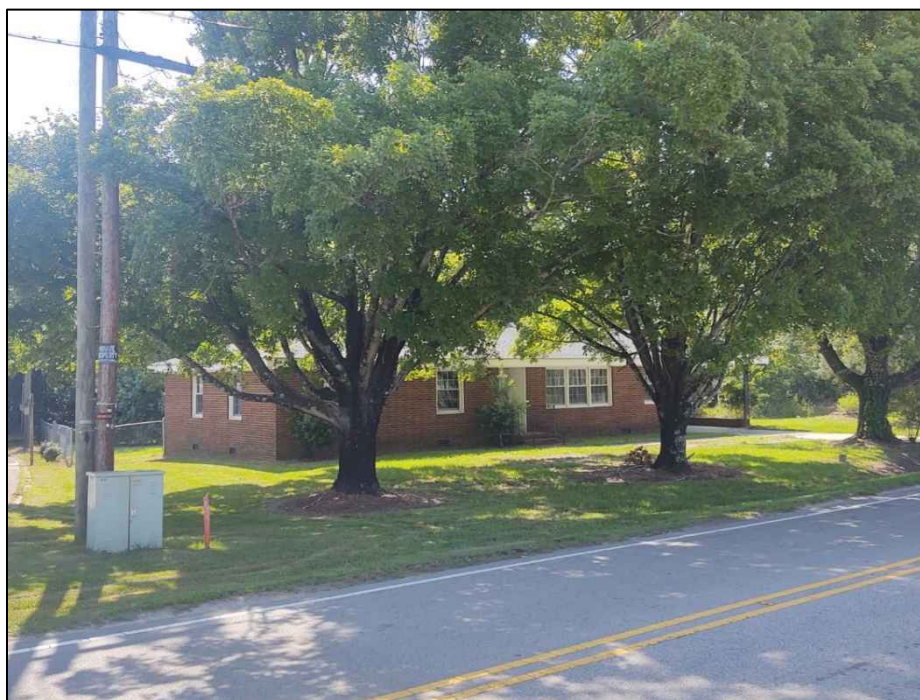
Figure 4.25. Structure WA7044, facing southeast.
