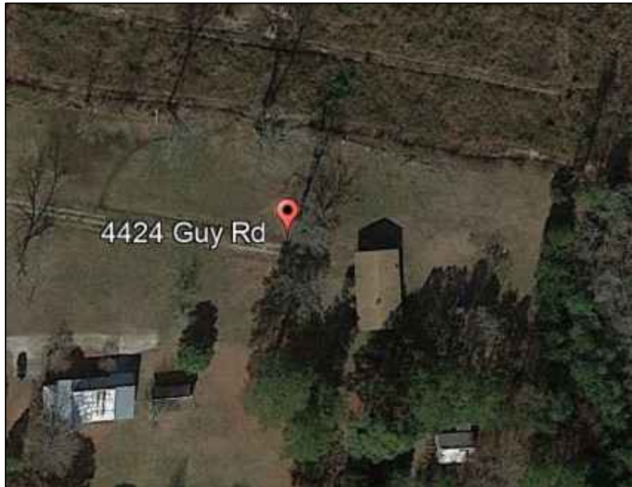
Figure 4.9. One-story brick veneer structure, WA7042 (Google Earth February 2019).
