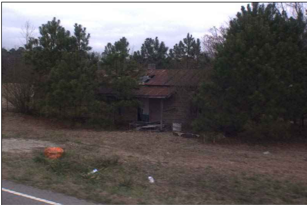
Figure 4.12. Structure, circa 1900, on the proposed laydown area parcel (Wake County Tax Assessor 2013).
