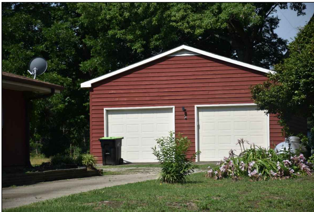
Figure 4.49. Structure WA7047, modern garage, facing southwest.
