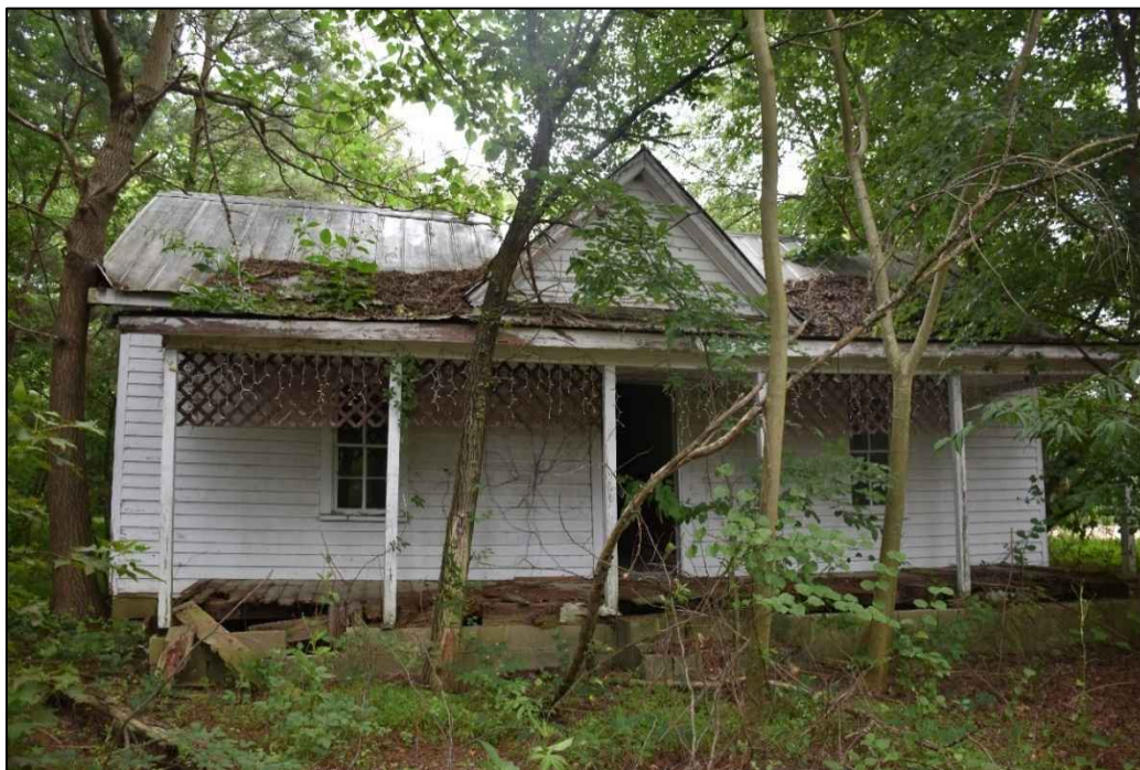
Figure 4.82. Structure JT2038, facing east.
