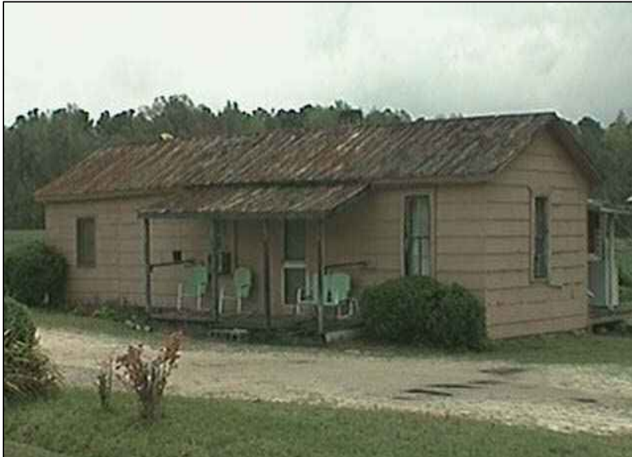
Figure 4.11. Structure, circa 1900, on the proposed laydown area parcel (Wake County Tax Assessor 1996).
