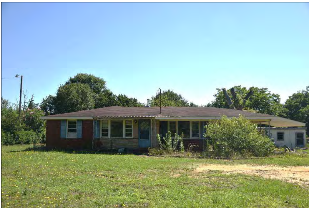
Figure 2.32. Unsurveyed house, 1412 Old US Highway 70, circa 1955, northeast.
