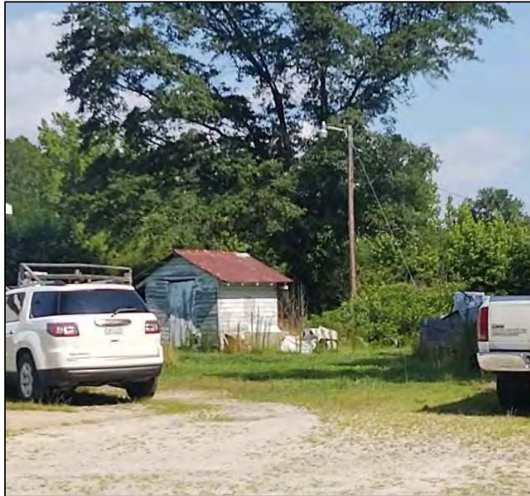
Figure 4.39. Structure WA8325, circa 1959 shed, facing northeast.
