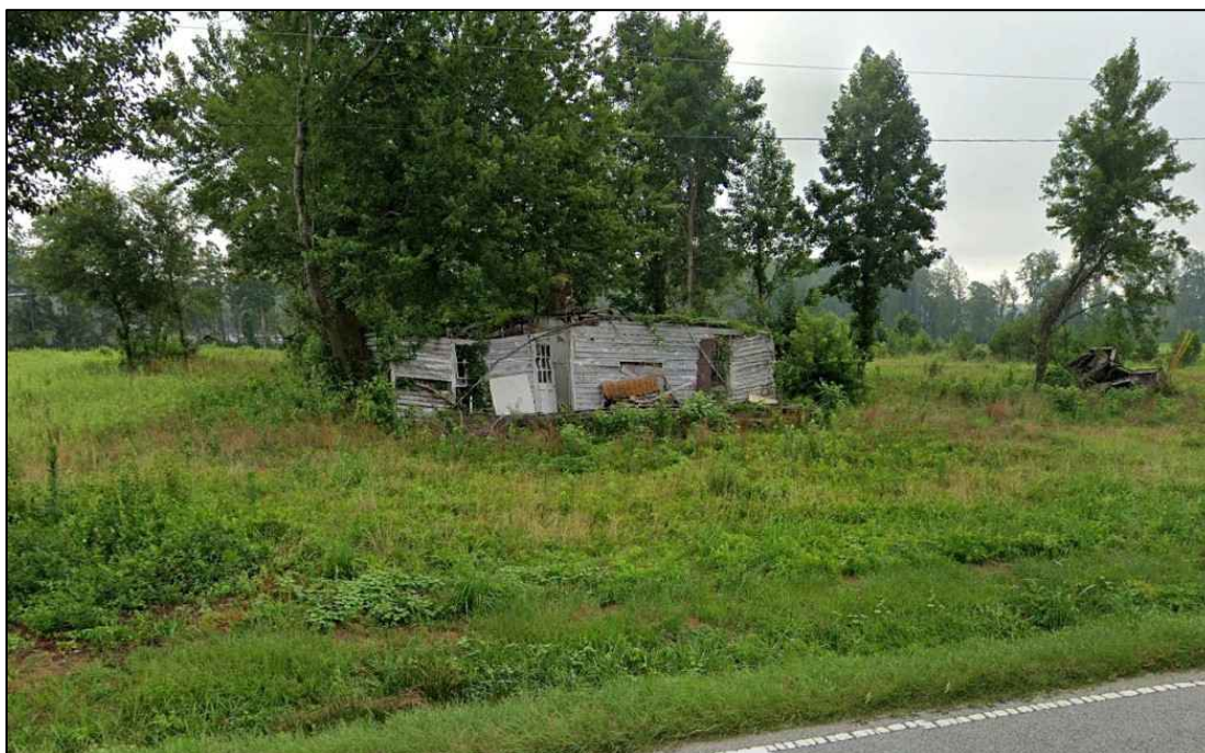
Figure 4.22. Structure WA7043 (Google Earth 2019).
