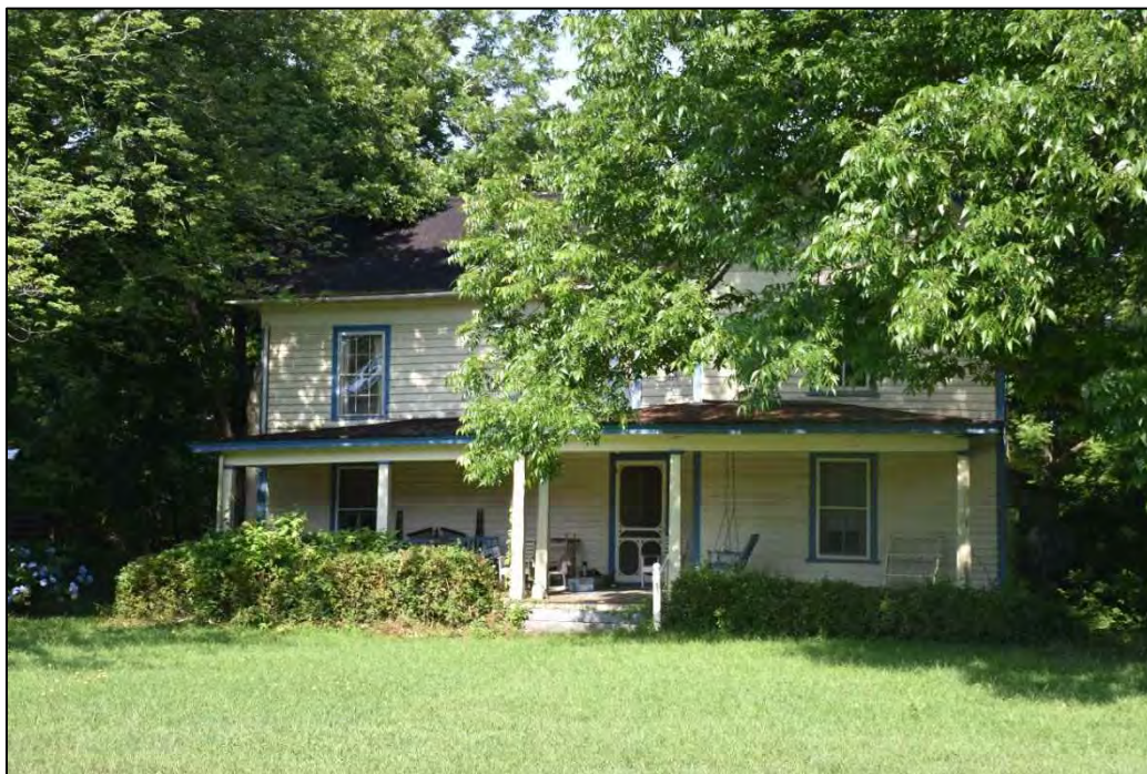
Figure 4.1. Gowers House (WA0290), facing west.
