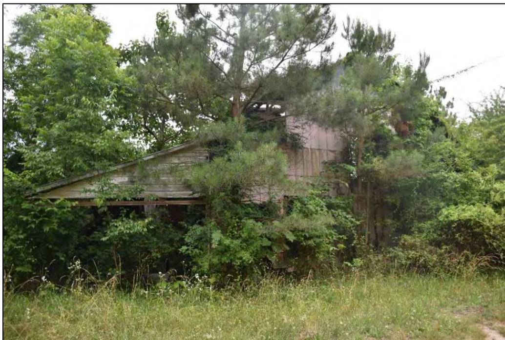
Figure 4.63. Structure JT0791, barn, facing north.
