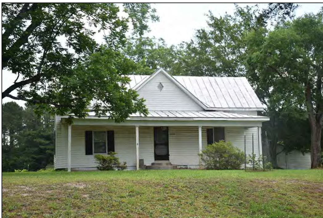
Figure 2.8. Unsurveyed House, 6309 Mial Plantation Road, facing west.
