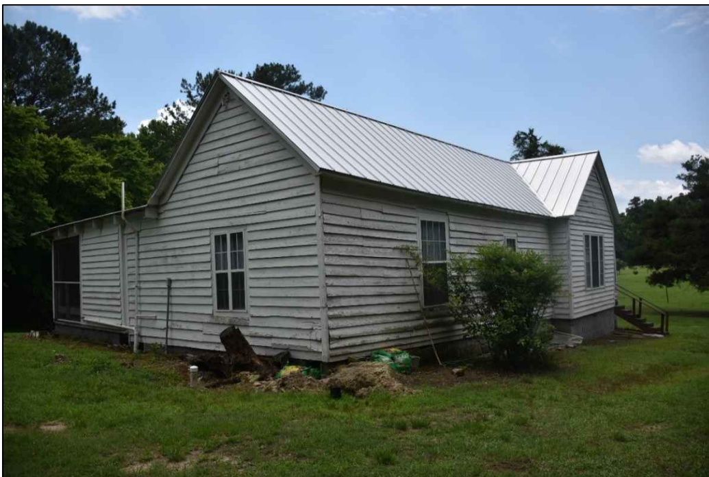
Figure 4.79. Single farmhouse, JT2037, facing southeast.
