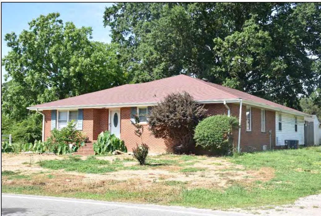
Figure 4.41. Structure WA7045, facing southwest.
