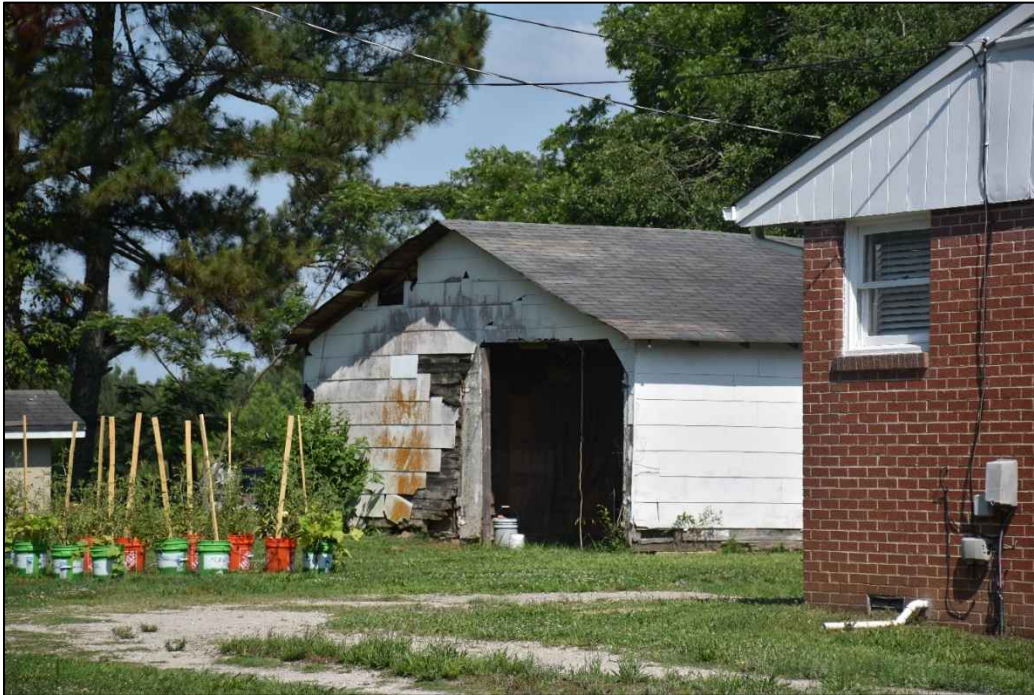
Figure 4.46. Garage associated with WA7046, facing northwest.
