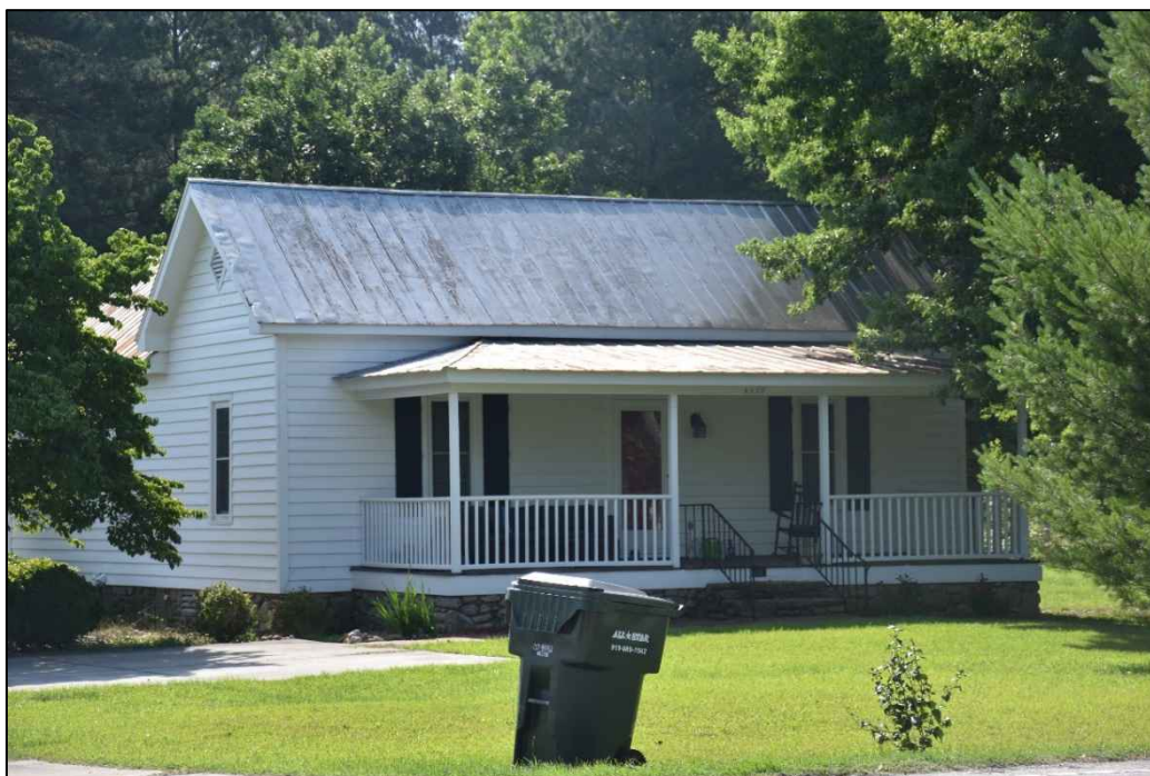
Figure 4.6. WA0291 William Coats House facing southeast.
