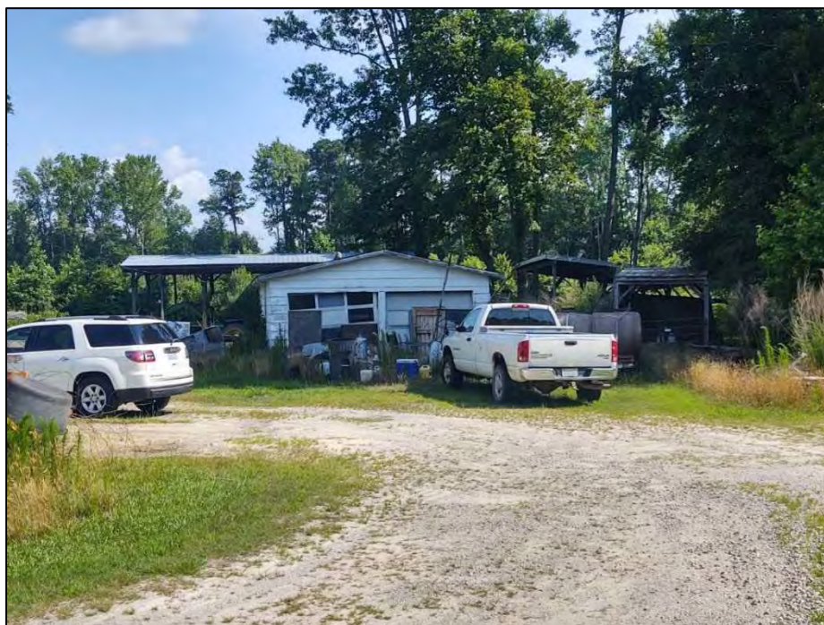
Figure 4.38. Structure WA8325, circa 1970 garage, facing west.
