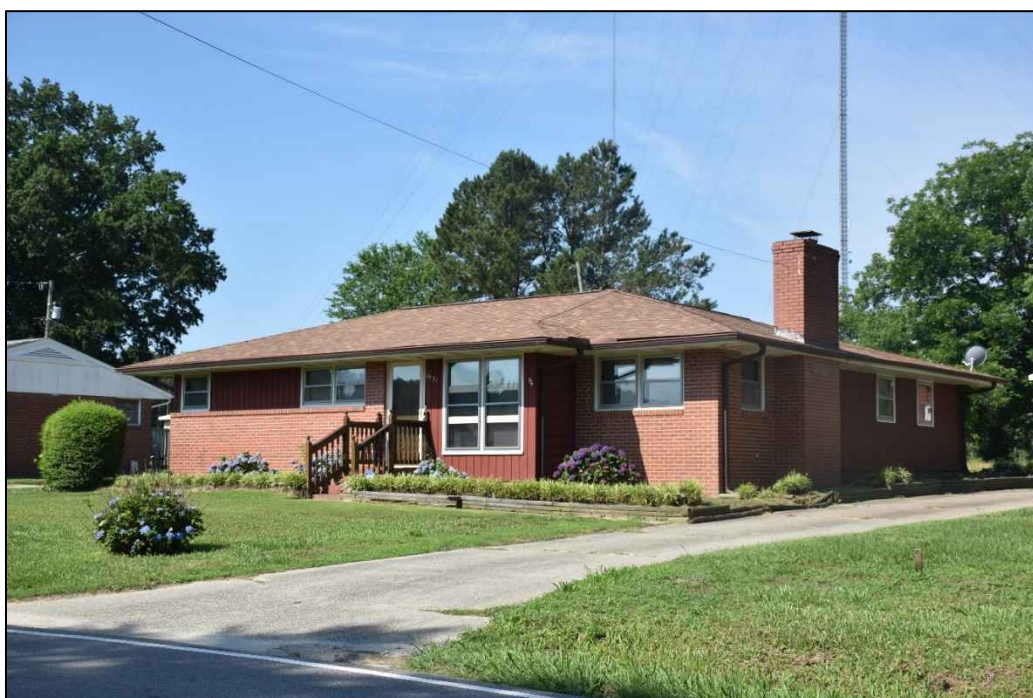
Figure 4.48. WA7047, facing southwest.
