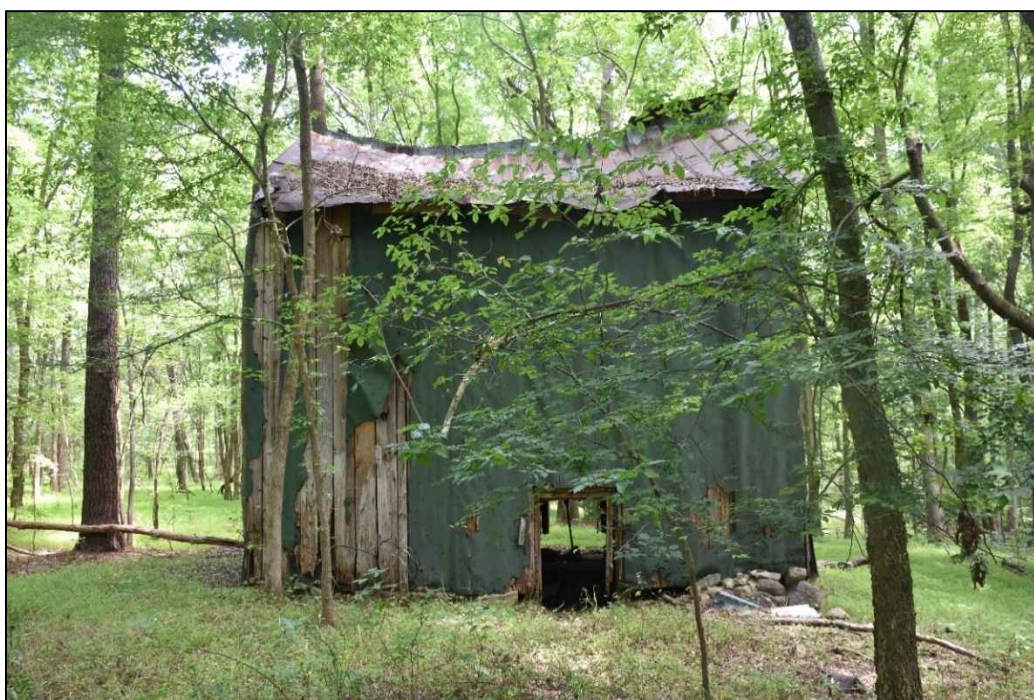
Figure 4.73. Tobacco barn associated with duplex farmhouse along access road, facing east.
