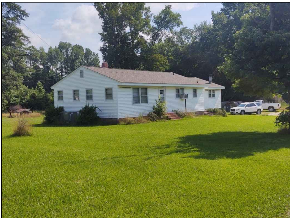
Figure 4.36. Structure WA8325, facing northeast.
