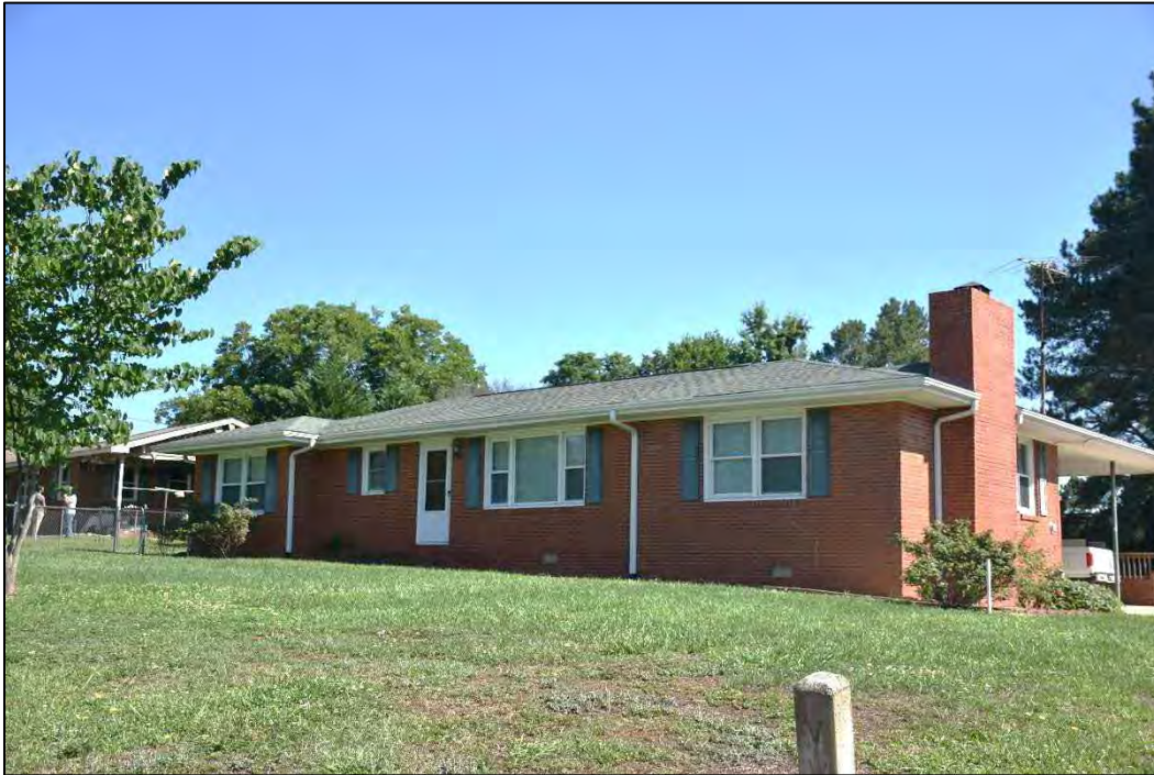
Figure 2.31. Unsurveyed house, 1402 Old US Highway 70, circa 1960, facing northeast.
