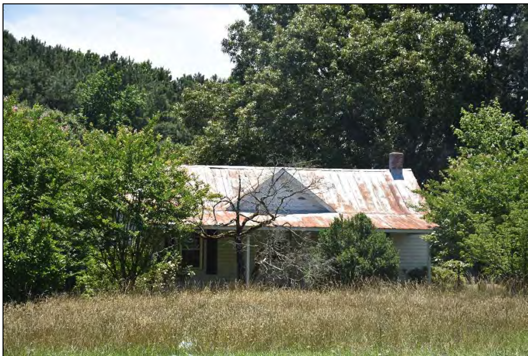
Figure 2.9. Unsurveyed house, 2129 Auburn Knightdale Road, facing east.
