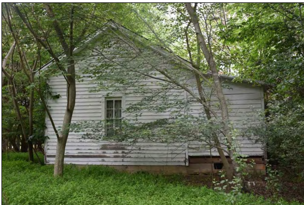
Figure 4.83. Structure JT2038, facing south.
