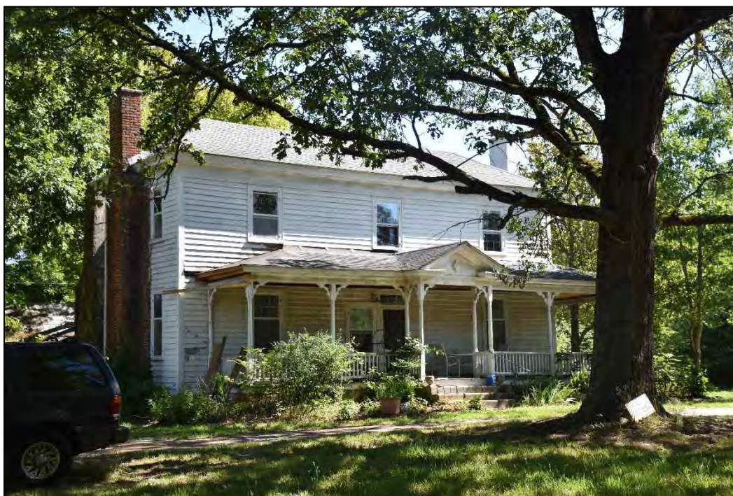
Figure 2.15. Baucom-Stallings House (WA0287), circa 1851, NRHP eligible, facing north.
