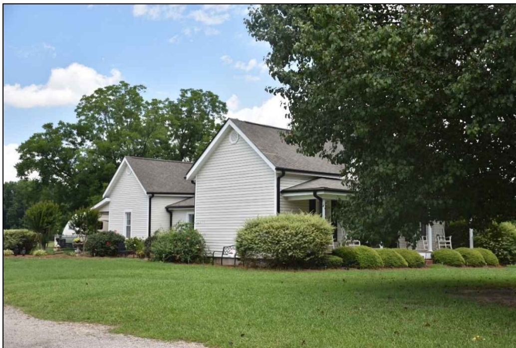
Figure 4.93. Structure JT2042, facing southwest.
