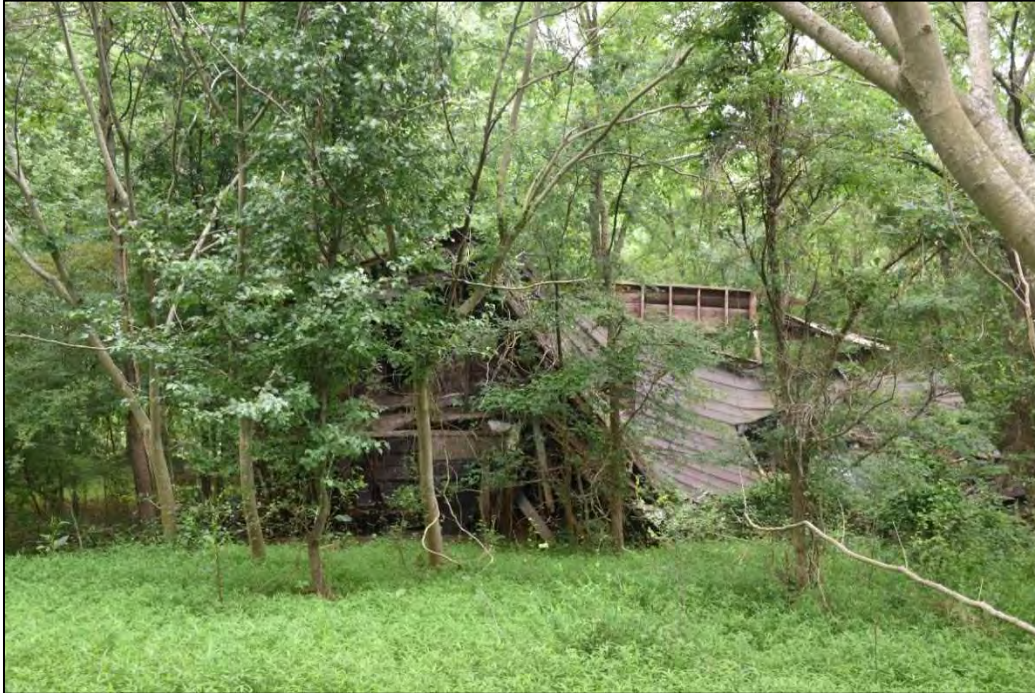
Figure 4.84. Barn associated with Structure JT2038, facing south.
