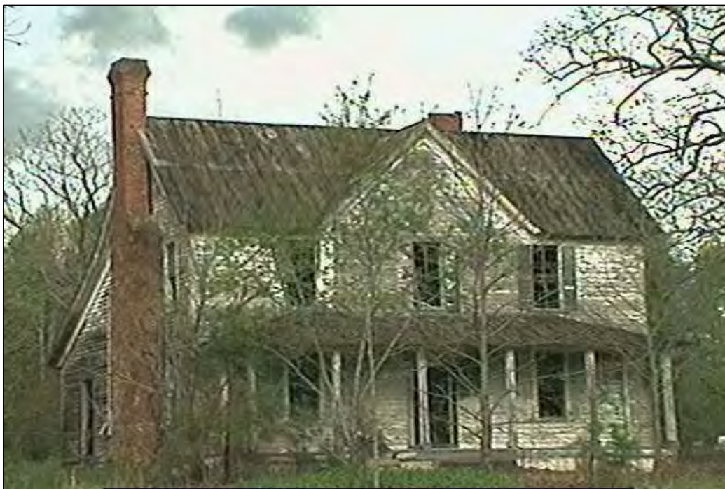
Figure 4.17. Kelly-Smith House, WA0292 (Wake County Tax Assessor 1996).
