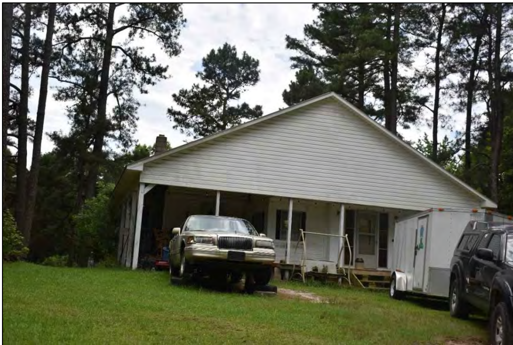
Figure 4.86. Current structure surrounding Structure JT2039, facing south.
