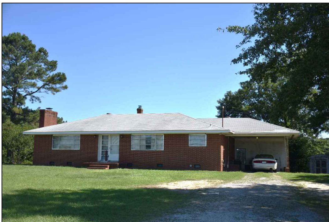
Figure 2.33. Unsurveyed house, 8513 Old Baucom Road, circa 1960, facing north.
