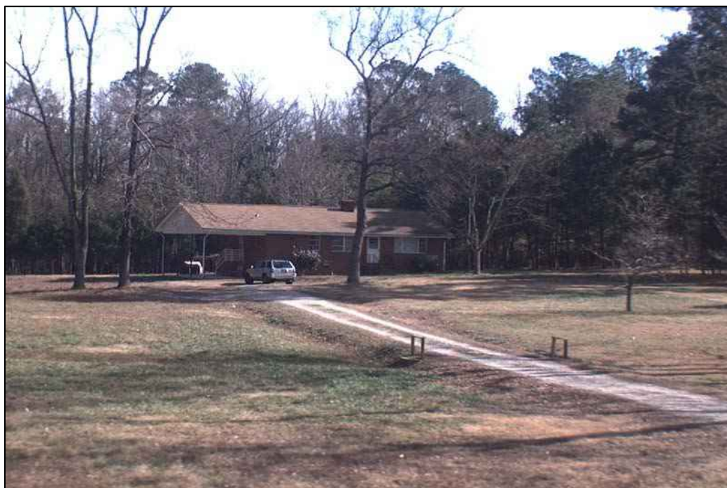
Figure 4.8. One-story brick veneer structure, WA7042 (Wake County Tax Assessor 2012).
