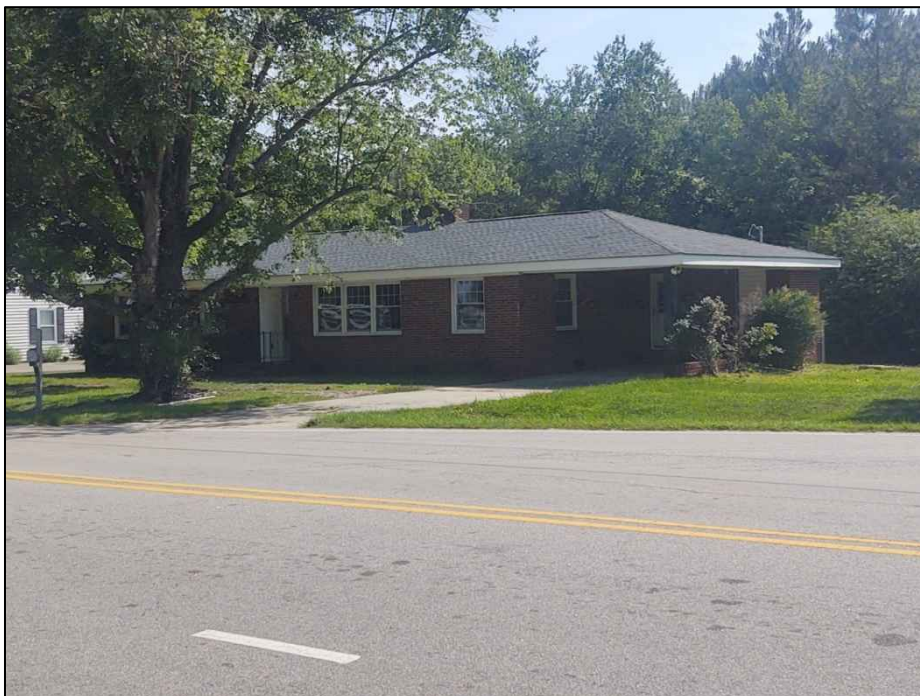
Figure 4.24. Structure WA7044, facing north.
