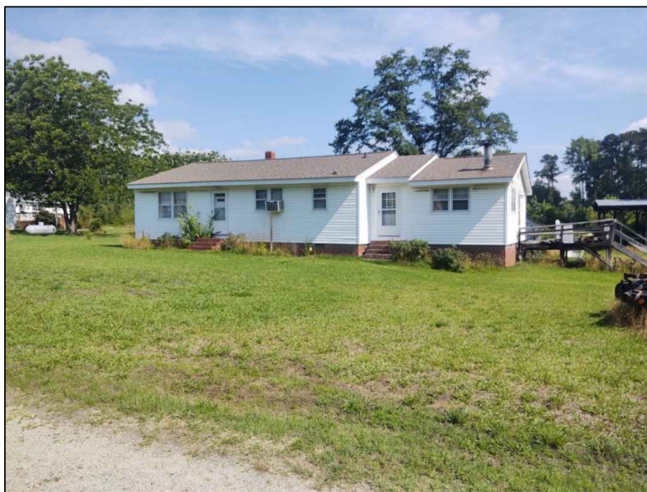
Figure 4.37. Structure WA8325, facing northwest.
