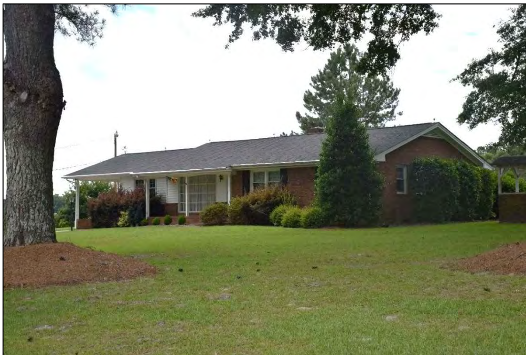
Figure 4.87. Structure JT2040, facing southwest.
