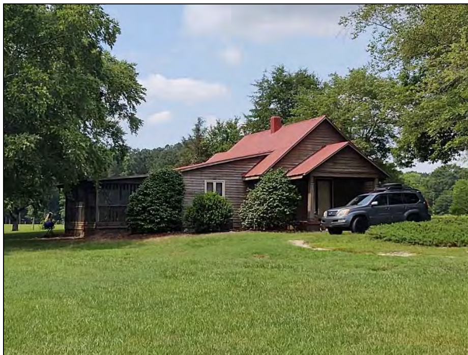
Figure 4.55. Structure WA8327, facing southwest.
