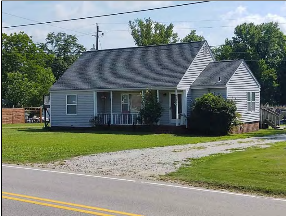
Figure 4.33. Structure WA8324, facing northeast.
