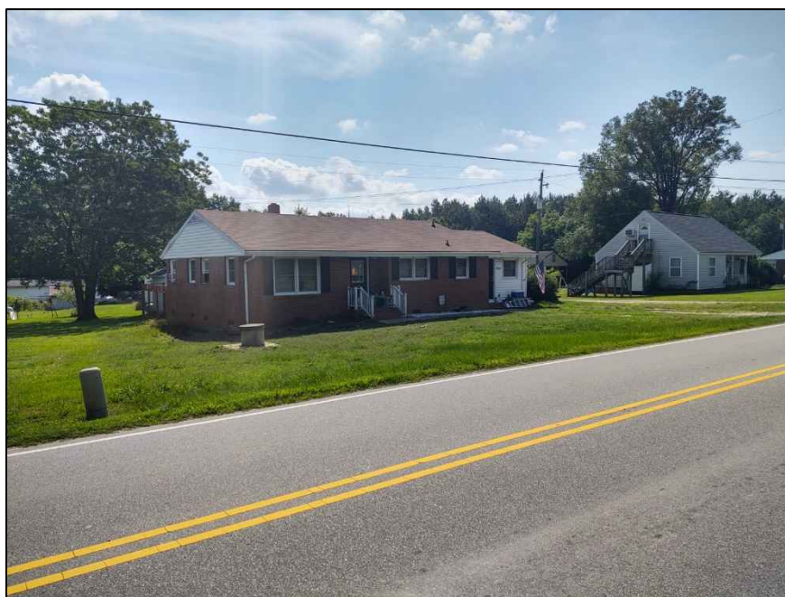
Figure 4.43. Structure WA8326, facing southeast.
