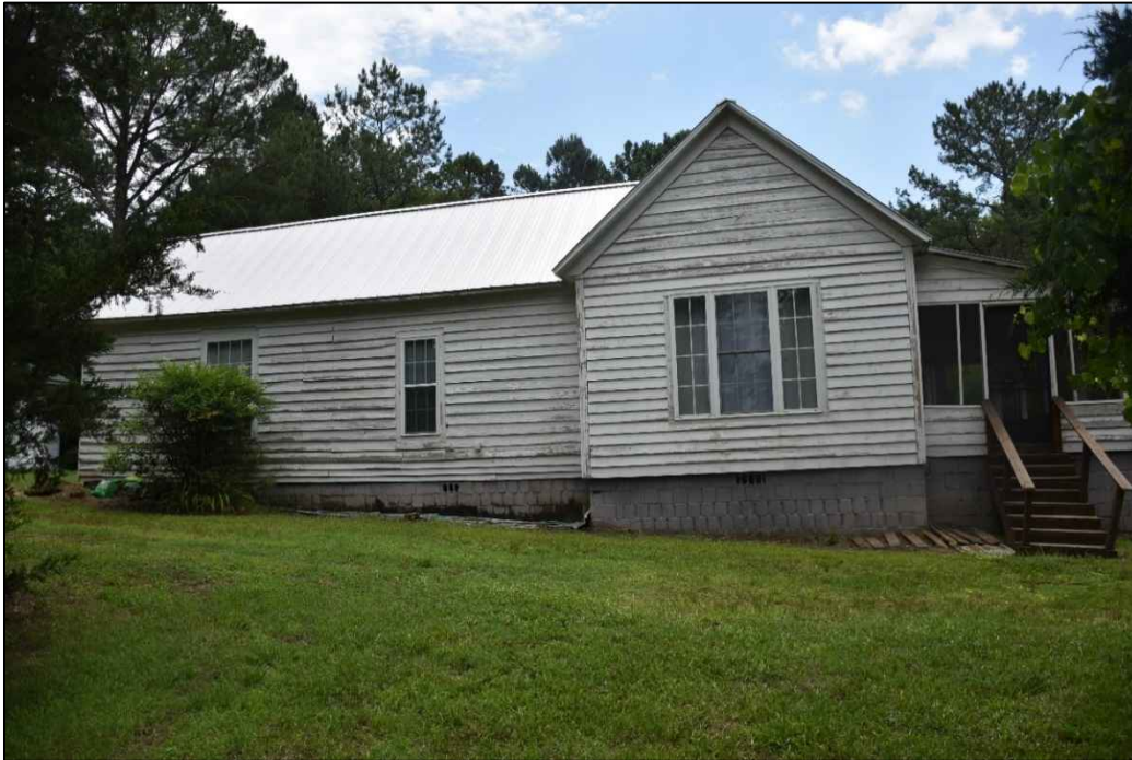
Figure 4.78. Single farmhouse, JT2037, facing east.
