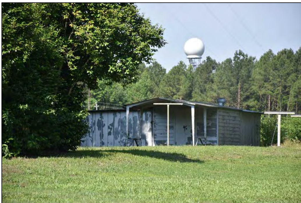
Figure 4.50. Structure WA7047, circa 1957 shed, facing southwest.
