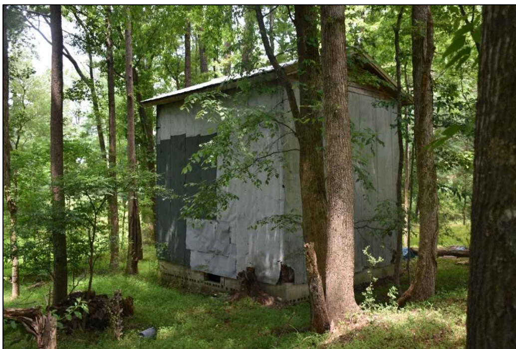
Figure 4.76. Tobacco barn, JT2037, facing northwest.
