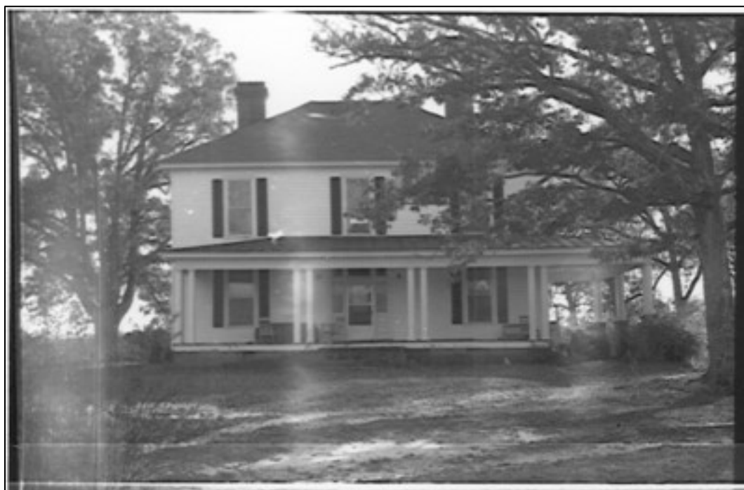
Figure 4.56. Baucom House (WA0281), survey photograph (Survey File 1988).
