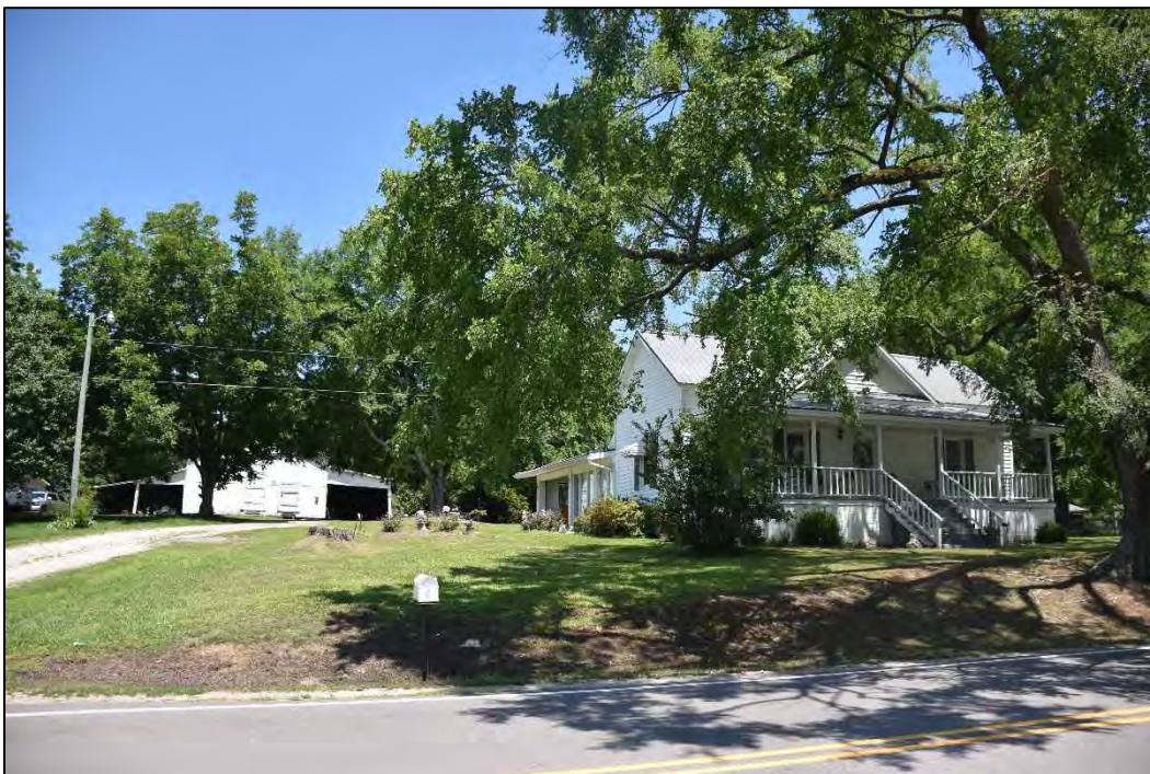
Figure 2.6. House (WA7075), circa 1900, and associated barn, facing north.
