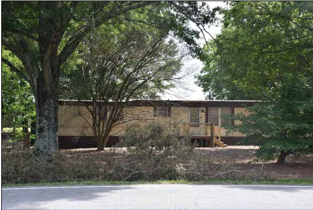
Figure 2.38. Unsurveyed house, 8604 White Oak Road, circa 1960, facing north.
