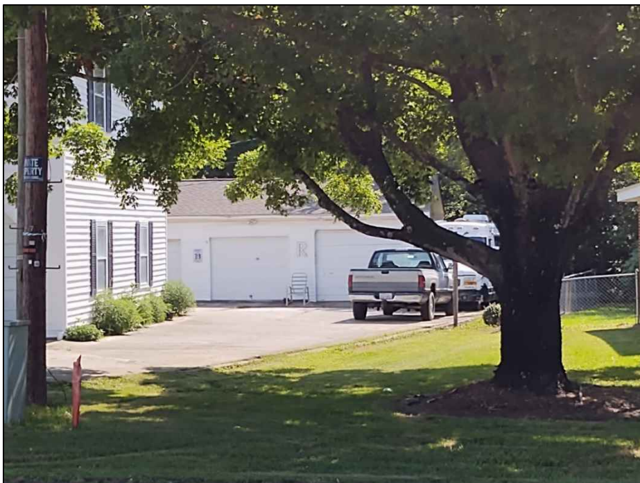
Figure 4.28. Structure WA7048, associated garage, facing east.
