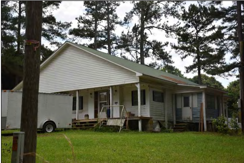
Figure 4.85. Structure JT2039, blue projecting section is only visible part of original structure, facing south.
