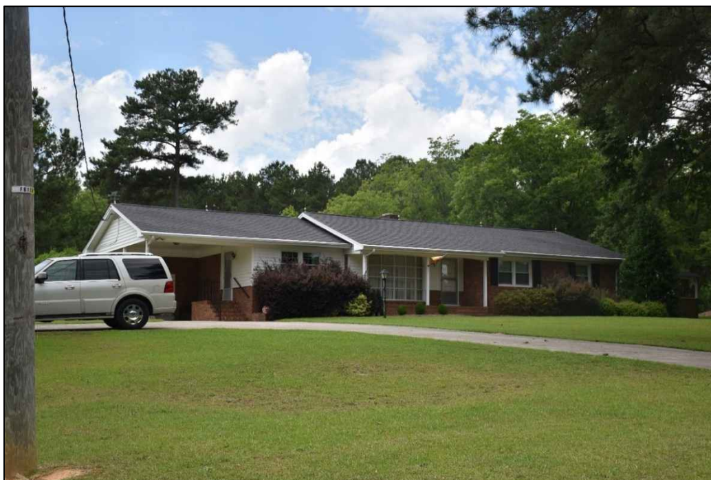
Figure 4.88. Structure JT2040, facing northwest.
