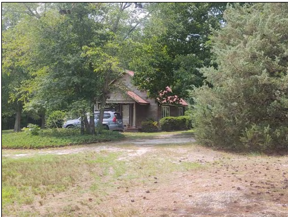
Figure 4.54. Structure WA8327, facing southeast.
