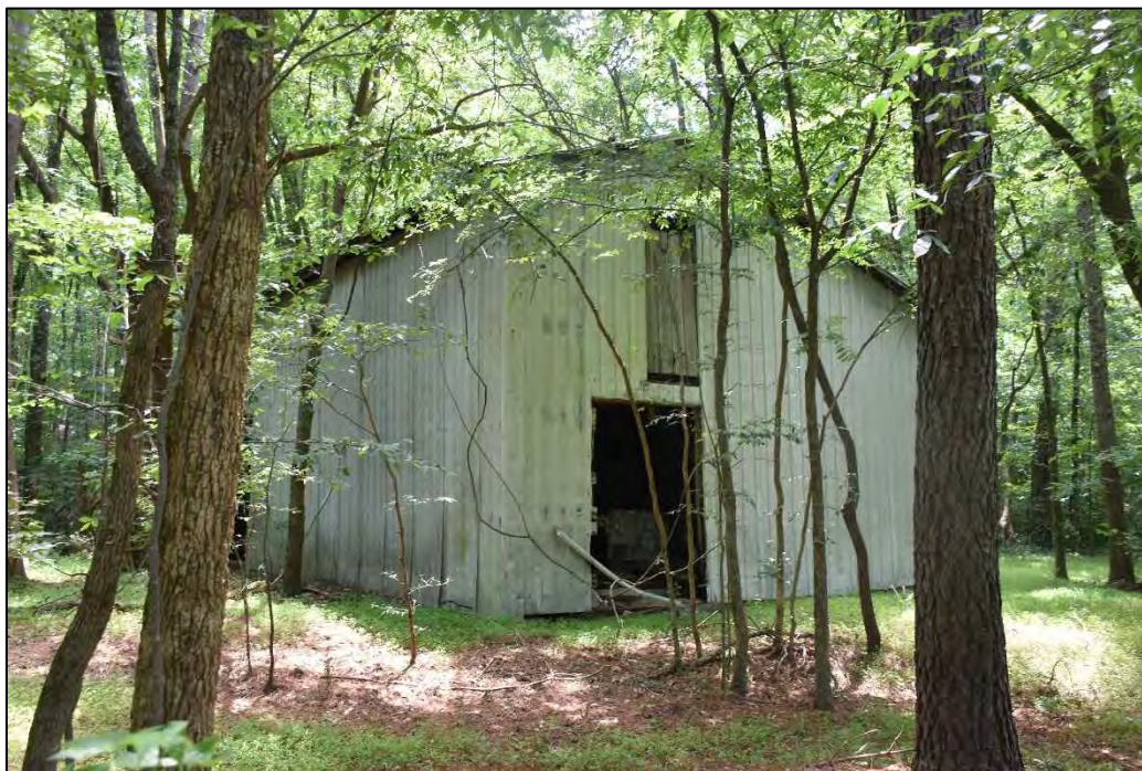
Figure 4.70. Frame barn with corrugated siding, JT2037, facing north.
