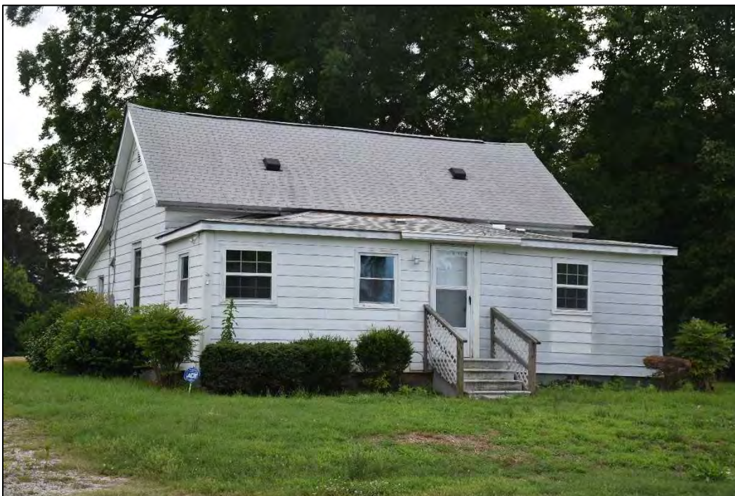
Figure 2.1. House (WA6350), circa 1890, facing southwest.
