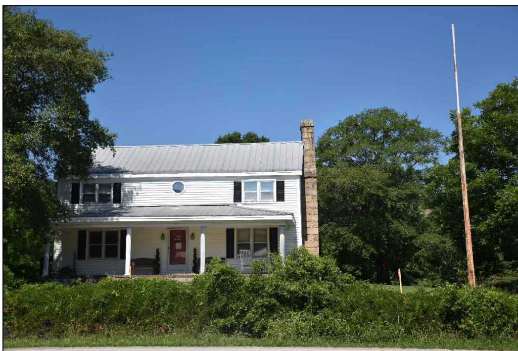
Figure 2.16. Bertie C. Richardson House (JT0918), circa 1880, facing west.
