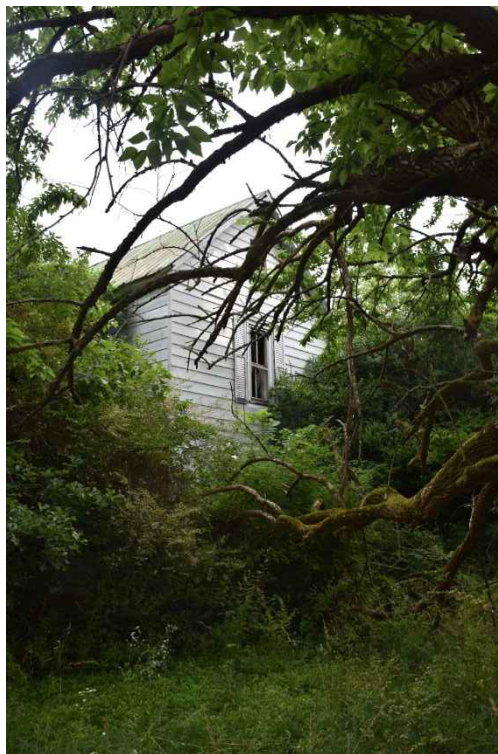
Figure 4.61. Structure JT0791, facing northeast.
