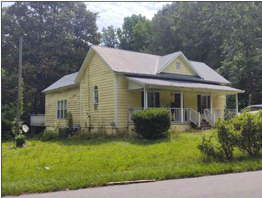
Figure 4.60. Structure JT2036, facing southeast.
