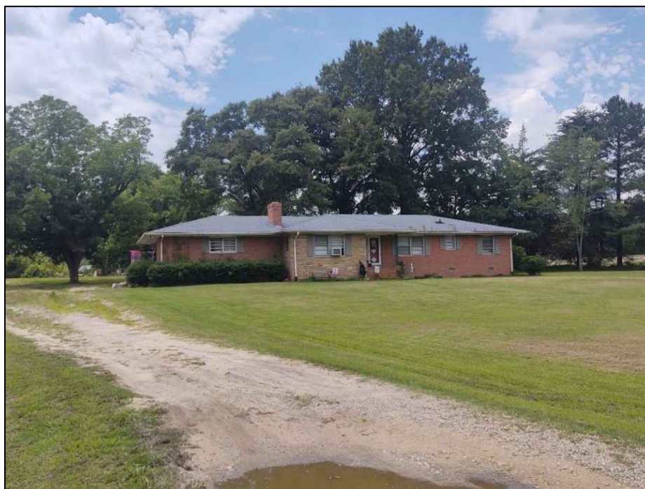
Figure 4.90. Structure JT2041, facing northwest.
