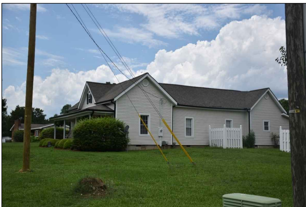
Figure 4.92. Structure JT2042, facing west.
