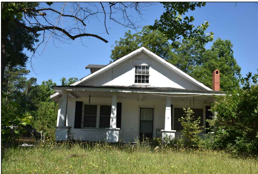
Figure 2.21. Unsurveyed house, 507 Medlin Road, circa 1945, facing west.
