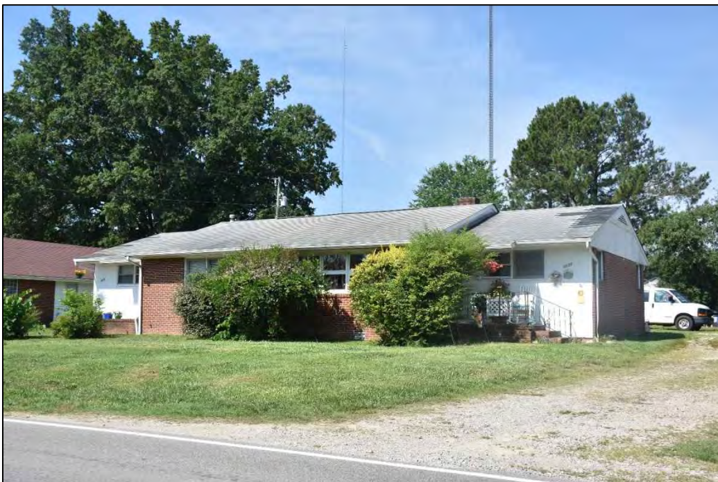
Figure 4.45. WA7046, facing southwest.
