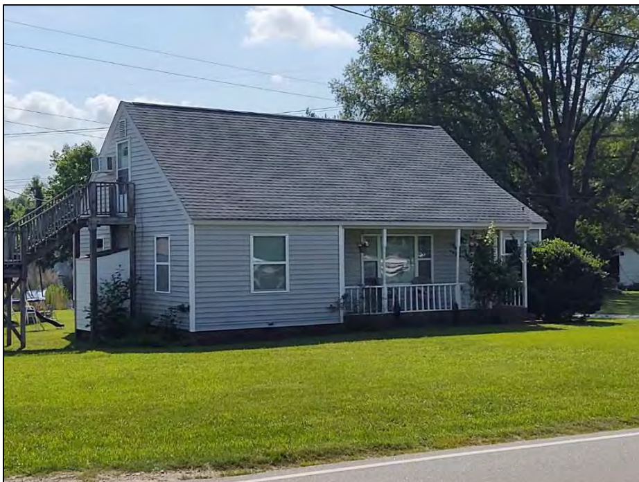
Figure 4.34 Structure WA8324, facing southeast.
