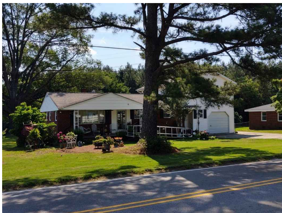
Figure 4.26. Structure WA7048, facing southeast.
