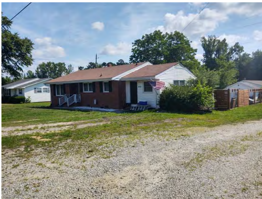
Figure 4.42. Structure WA8326, facing northeast.
