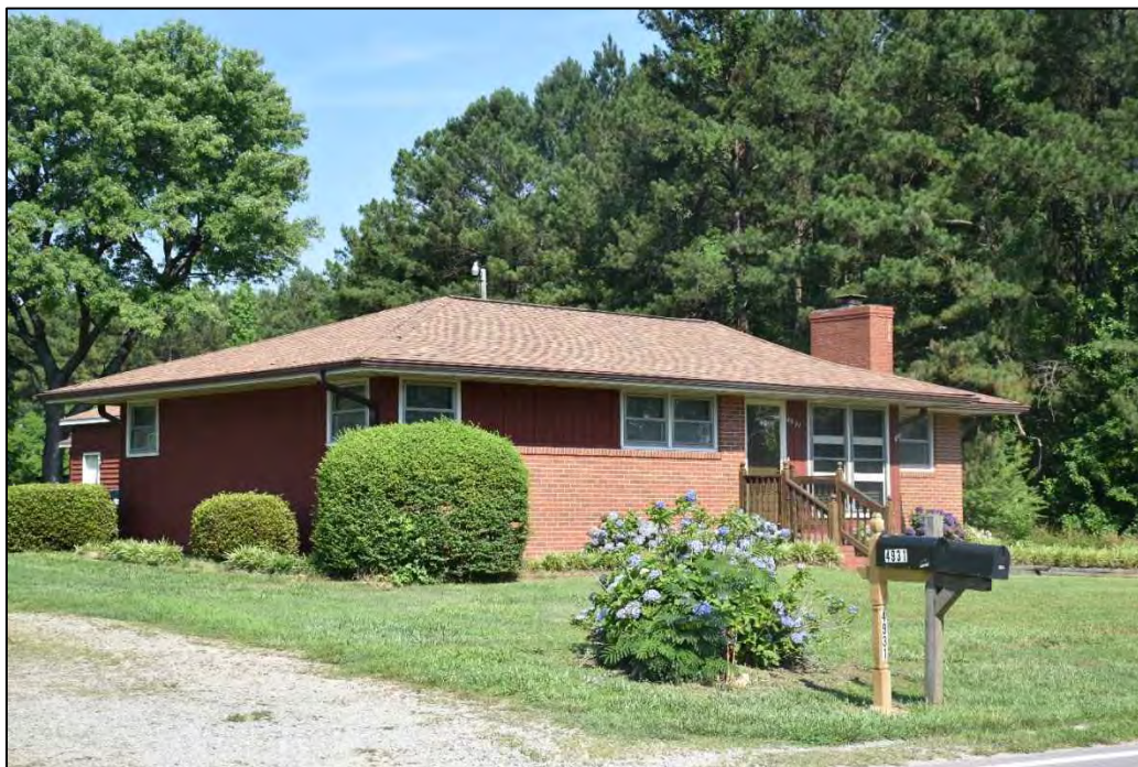
Figure 4.47. Structure WA7047, facing northwest.
