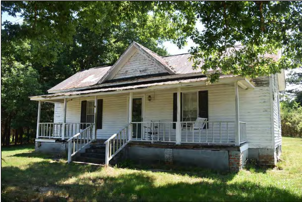
Figure 2.5. House (WA7067), circa 1900, facing northeast.
