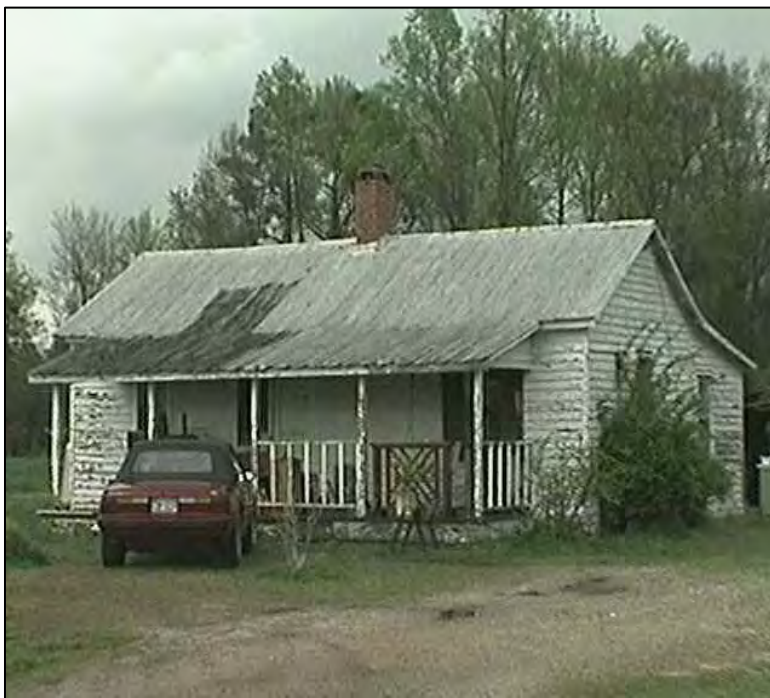
Figure 4.21. Structure WA7043 (Wake County Tax Assessor 1996).
