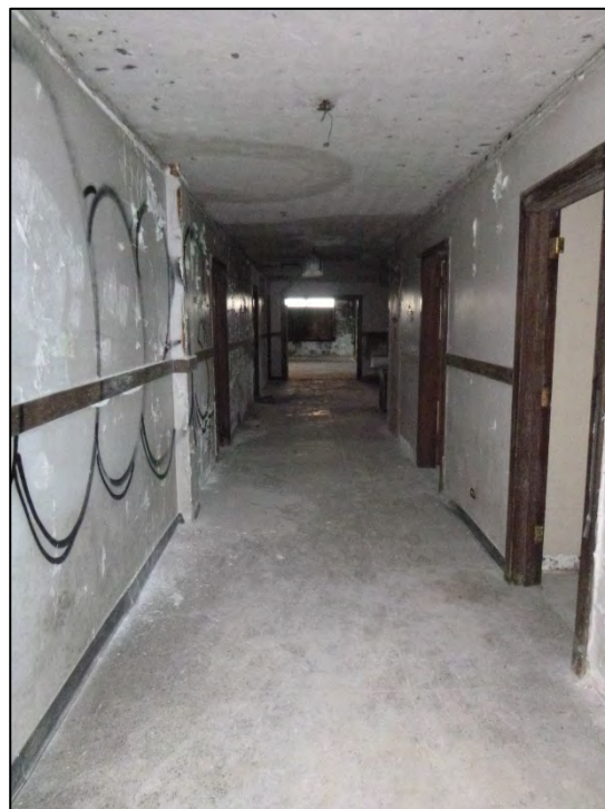
Figure 4.25. First-floor hallway, facing west.
