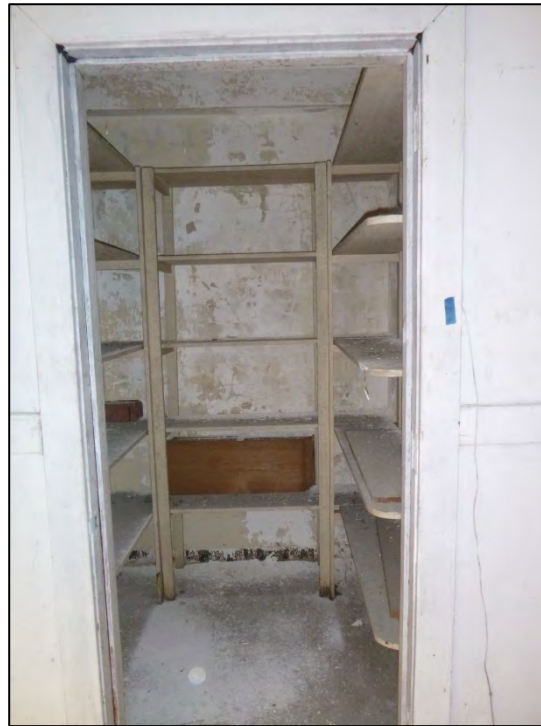
Figure 4.38. Second floor storage closet, facing south.
