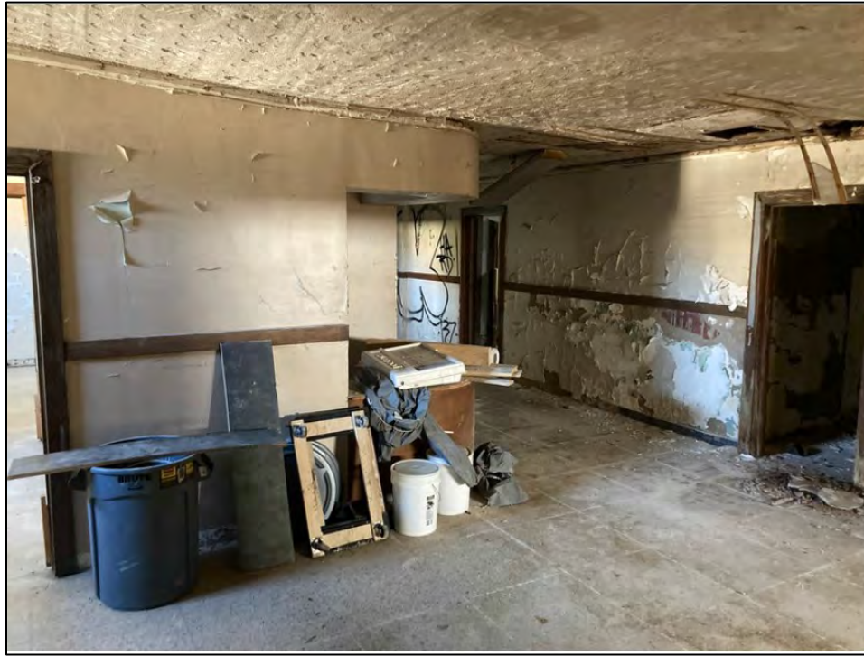
Figure 4.19. Reception desk, facing southeast.
