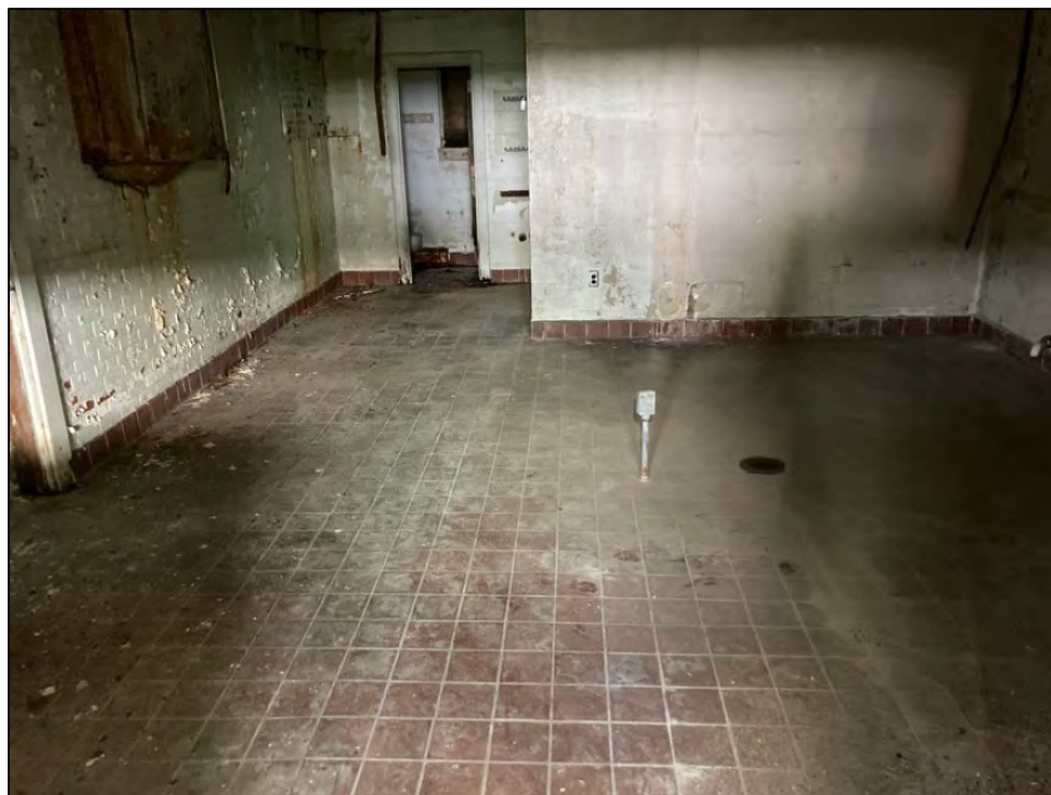
Figure 4.21. Kitchen, facing east.
