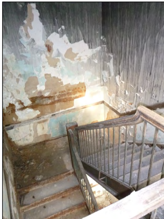
Figure 4.28. Stairwell from third to second floor, facing northwest.
