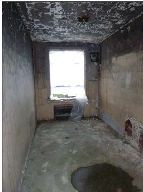
Figure 4.40. Third floor apartment, facing south.
