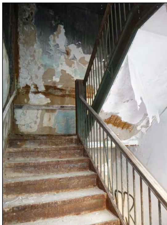
Figure 4.26. Stairwell from second to third floor, facing northwest.
