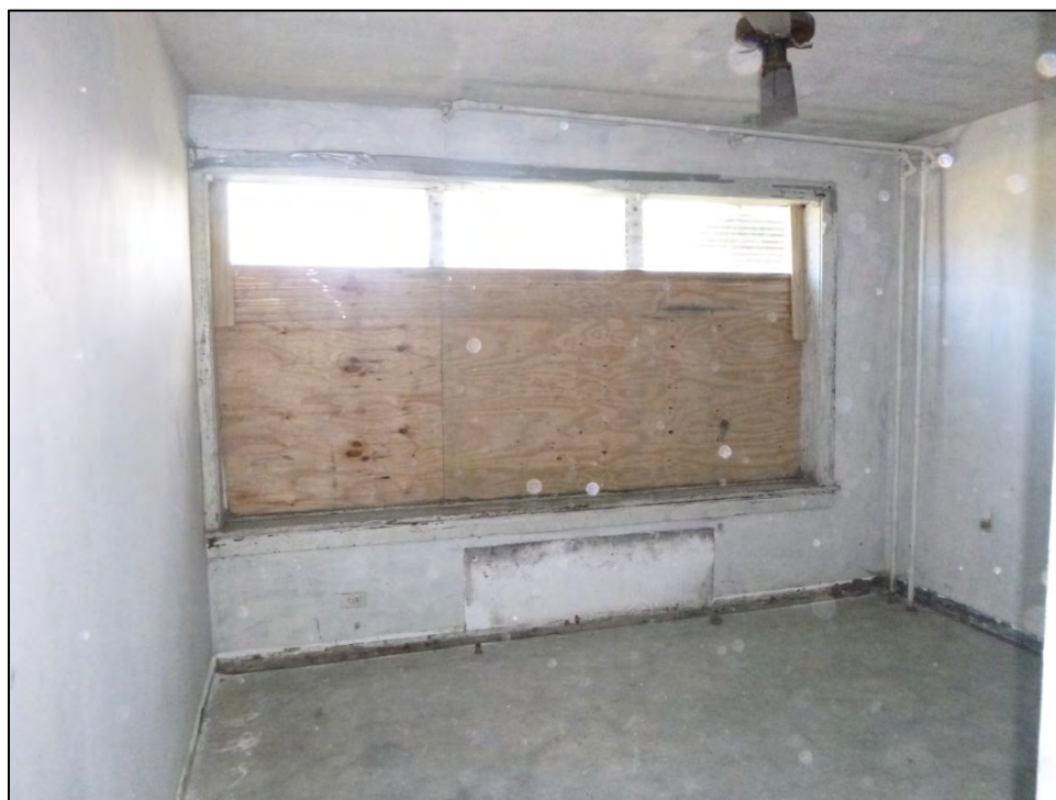
Figure 4.30. Typical windows for apartments on north side, facing northeast.
