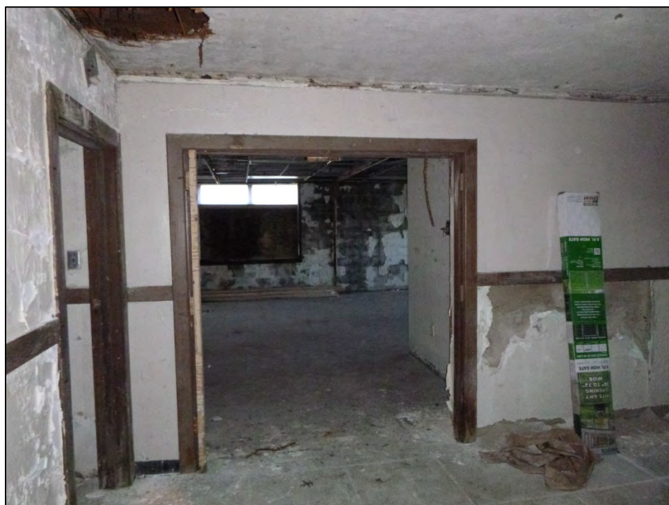
Figure 4.18. Community room from reception area, facing west.
