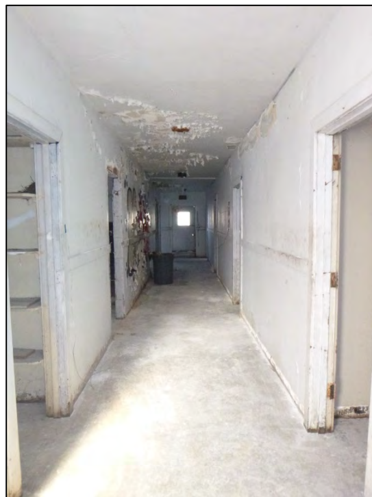
Figure 4.35. Second floor hallway, facing west.
