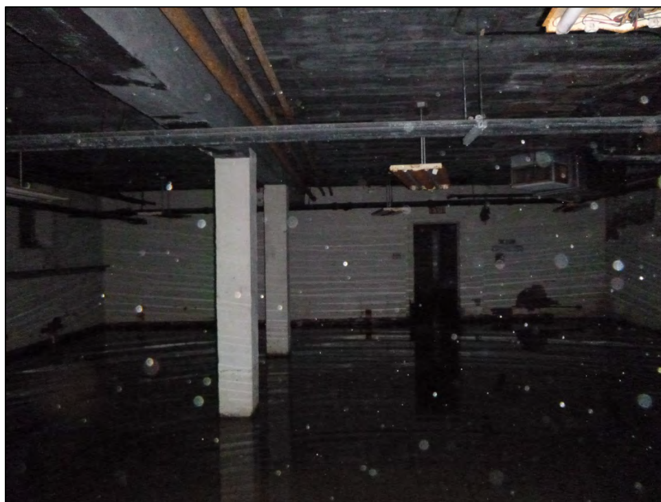
Figure 4.41. Main basement room, facing east.
