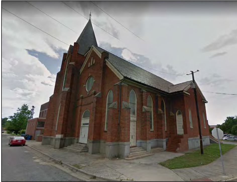
Figure 2.1. St. Joseph's African Methodist Episcopal Church (from Google Streetview).
