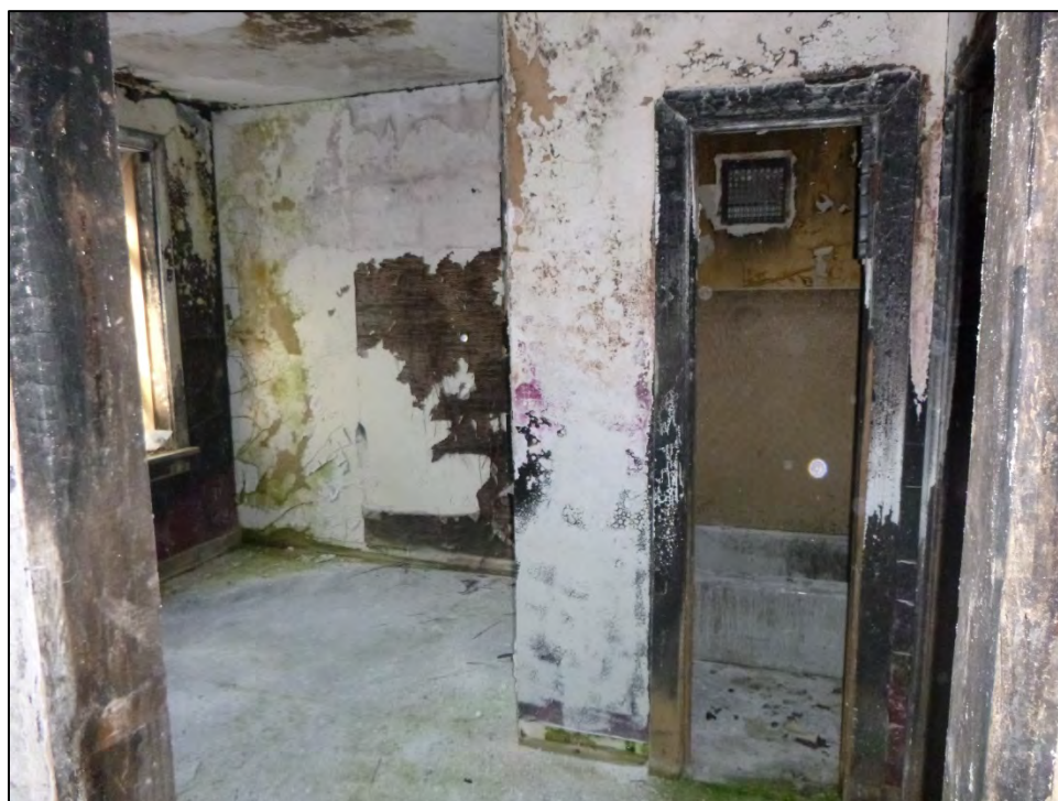
Figure 4.37. Second floor two room apartment, facing southwest.
