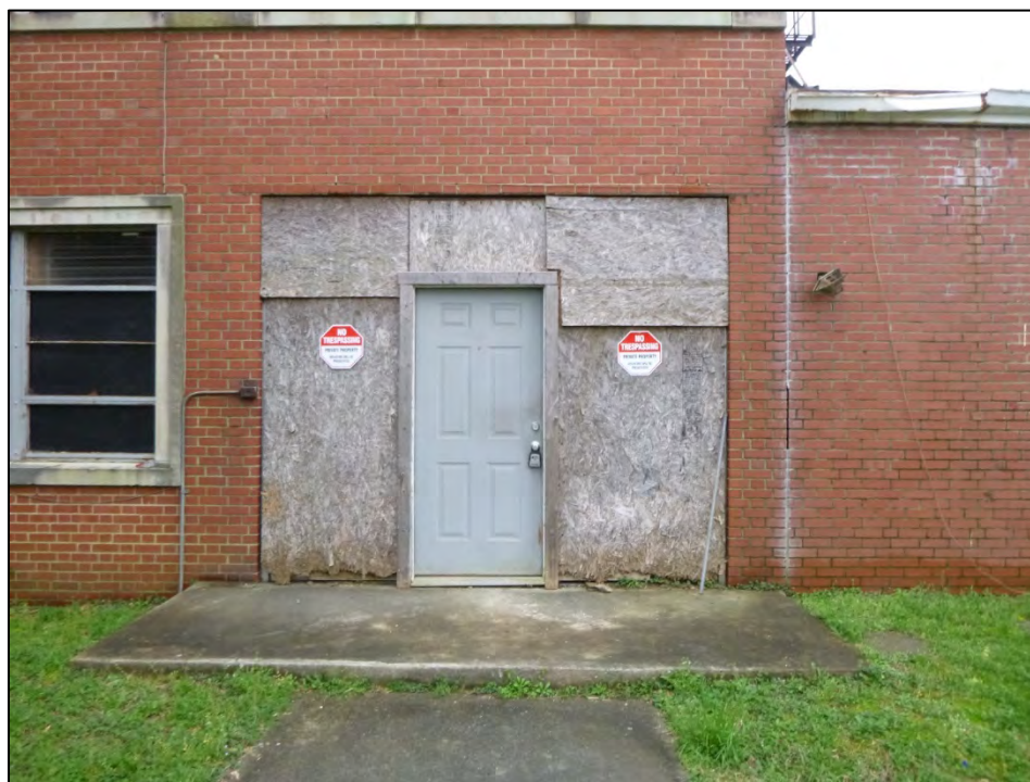
Figure 4.7. Harriet’s Place, main entrance showing replacement of original entrance and difference of brick bond patterns from the main building and addition.
