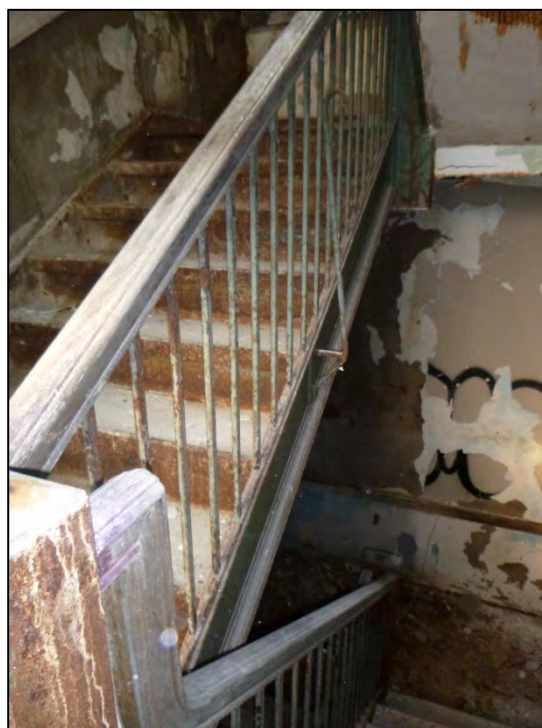
Figure 4.29. Wrought iron support, facing southwest.
