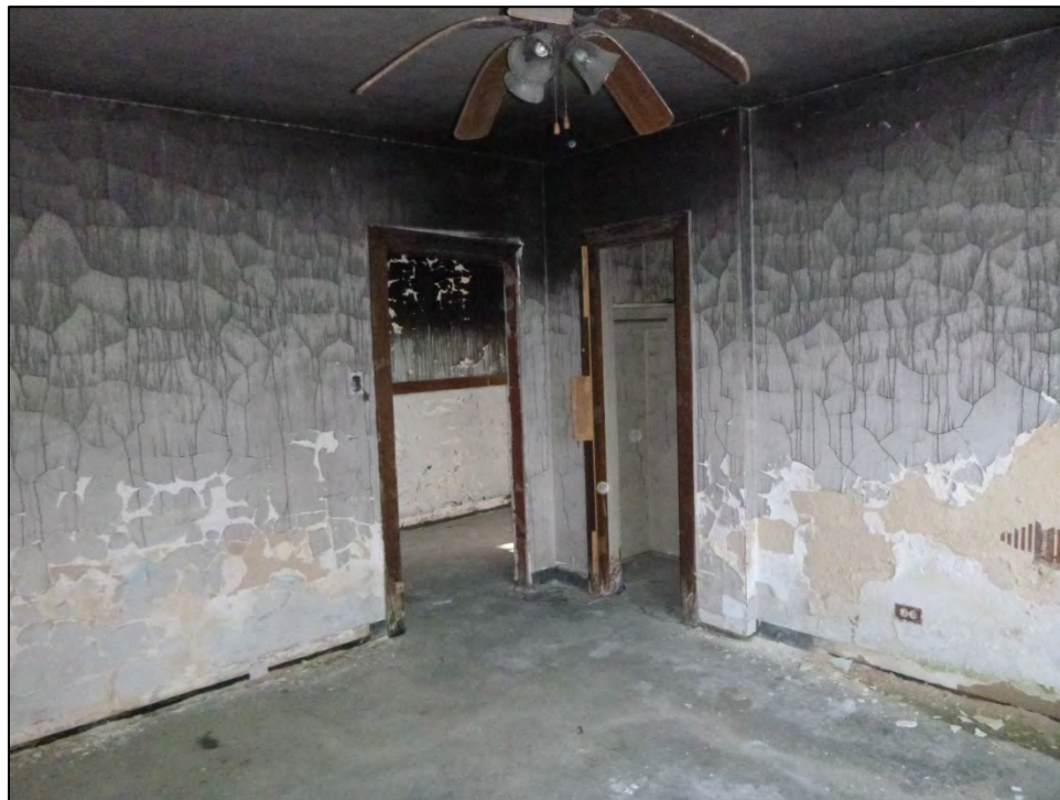
Figure 4.39. Third floor apartment, facing northeast.
