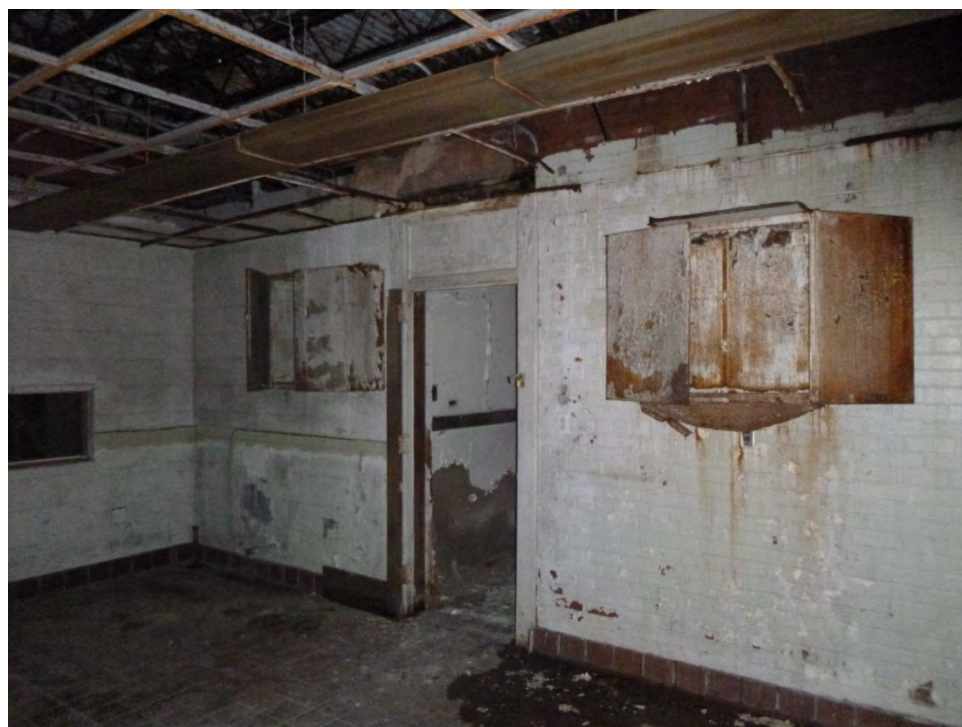
Figure 4.23. Kitchen, facing northwest.
