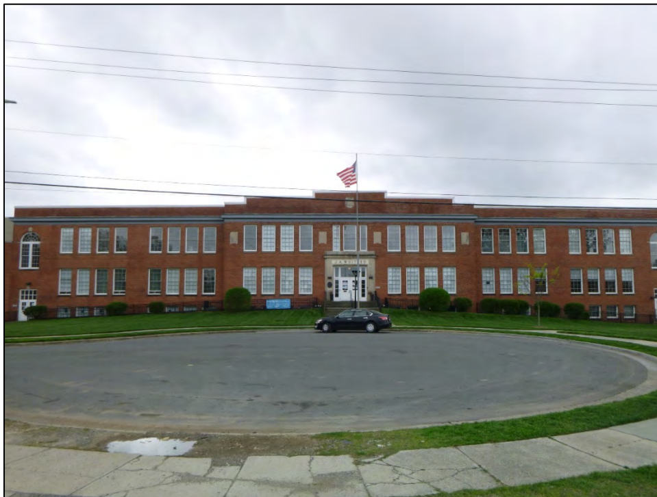
Figure 2.2. Hillside Park High School, facing south.
