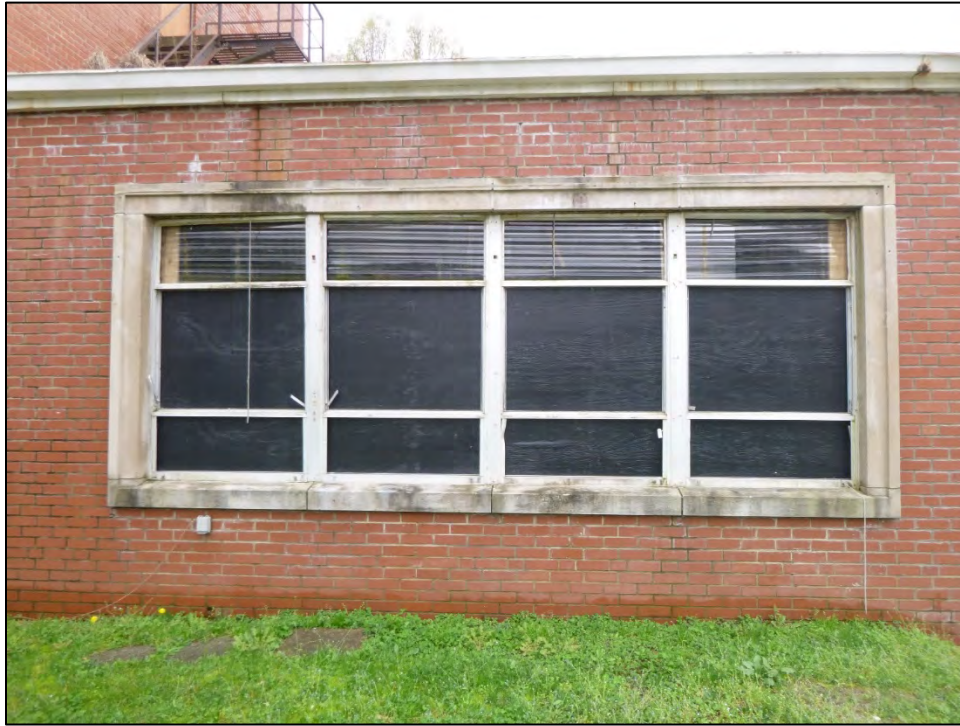
Figure 4.9. Harriet’s Place, addition window detail, facing south.
