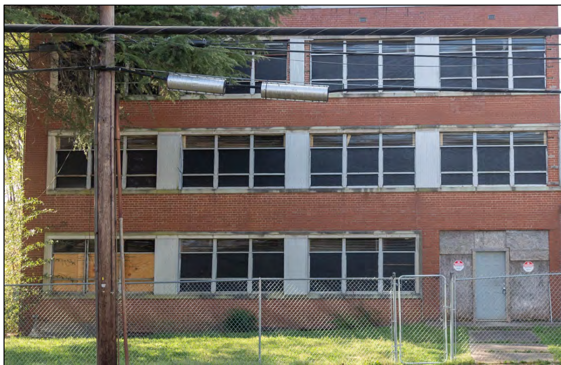
Figure 4.6. Harriet’s Place, window detail, facing south.
