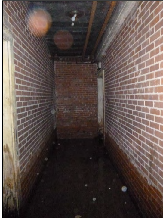
Figure 4.42. Hallway in basement, facing east.
