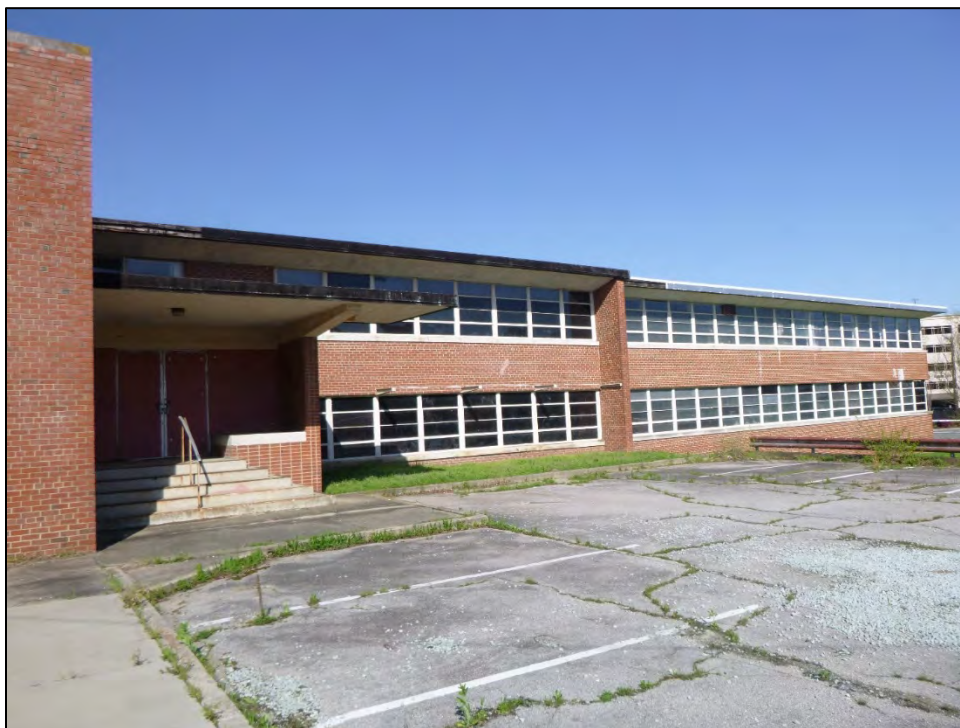
Figure 4.49. The Medical Arts building at 306 S Gregson, north.
