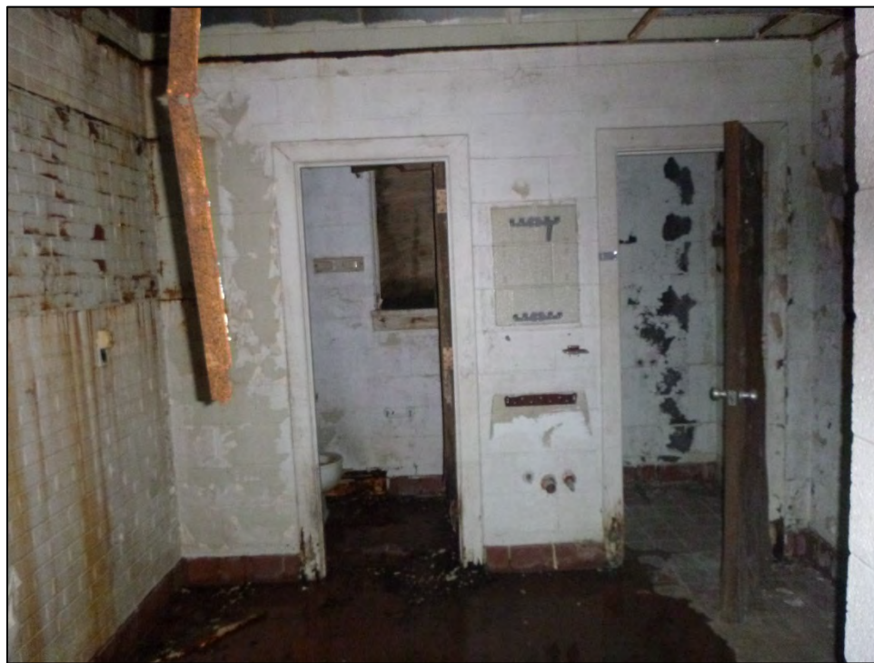
Figure 4.22. Kitchen bathrooms, facing east.
