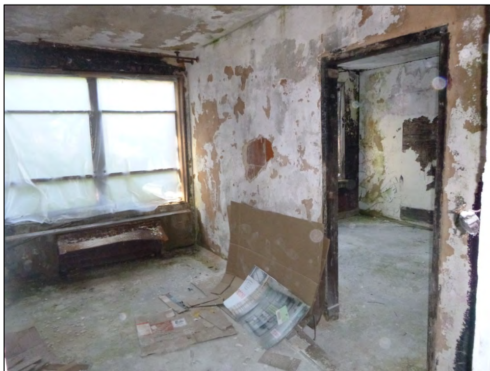
Figure 4.36. Second floor two room apartment, facing southwest.
