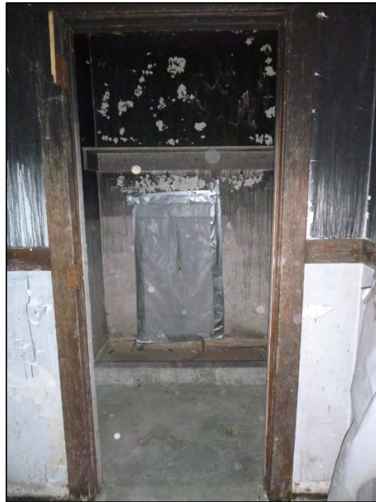
Figure 4.34. Typical washroom, facing south.
