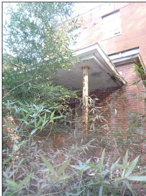
Figure 4.12. Harriet’s Place, rear entrance, facing northwest.
