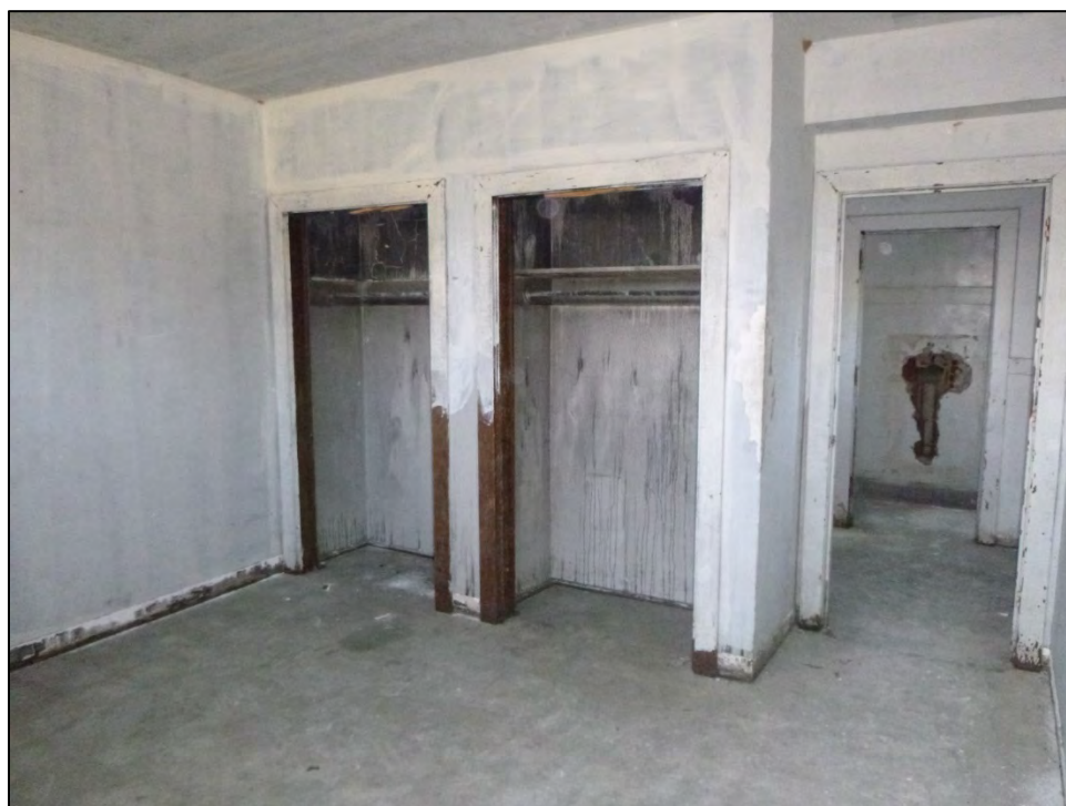
Figure 4.31. Typical closet and entrance for apartments on north side, facing southeast.
