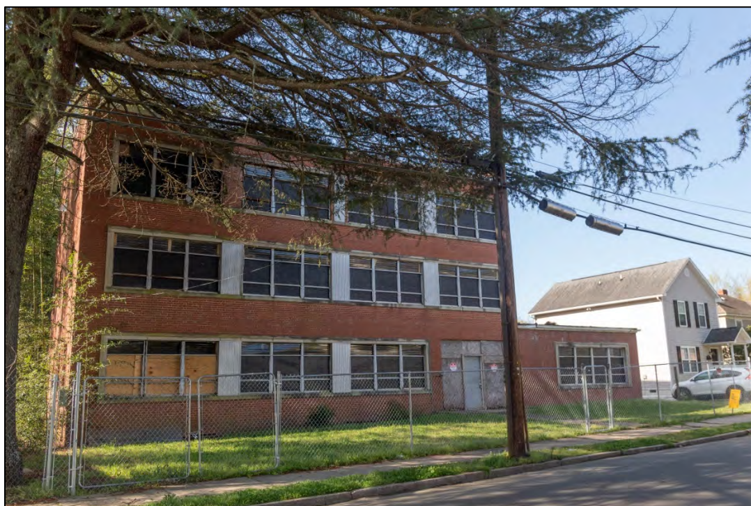
Figure 4.4. Harriet’s Place, facing southwest.
