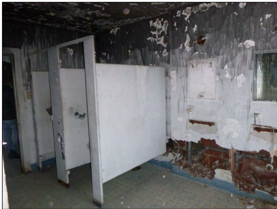
Figure 4.32. Typical bathroom stalls and sinks, facing northeast.
