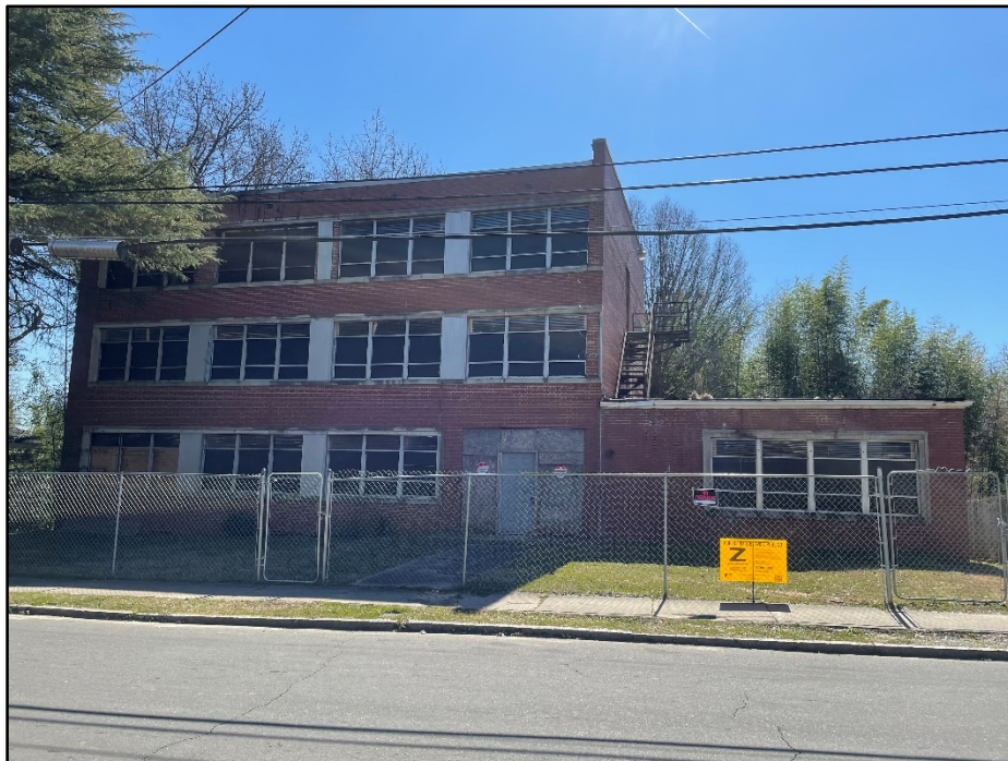
Figure 4. View of the former Harriet Tubman YWCA (DH2861), facing south.
