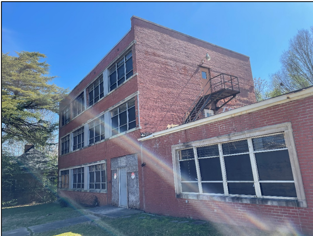
Figure 6. View of the former Harriet Tubman YWCA (DH2861), facing southeast.
