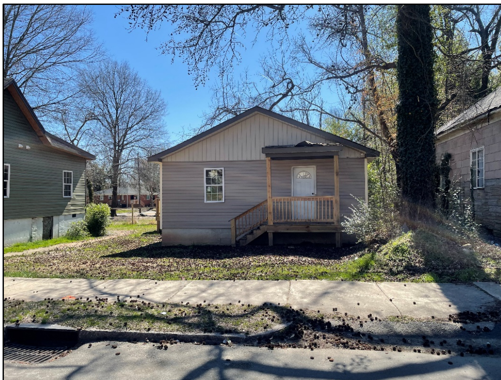
Figure 21. Modern alterations to structure at 318 East Umstead Street, facing south.
