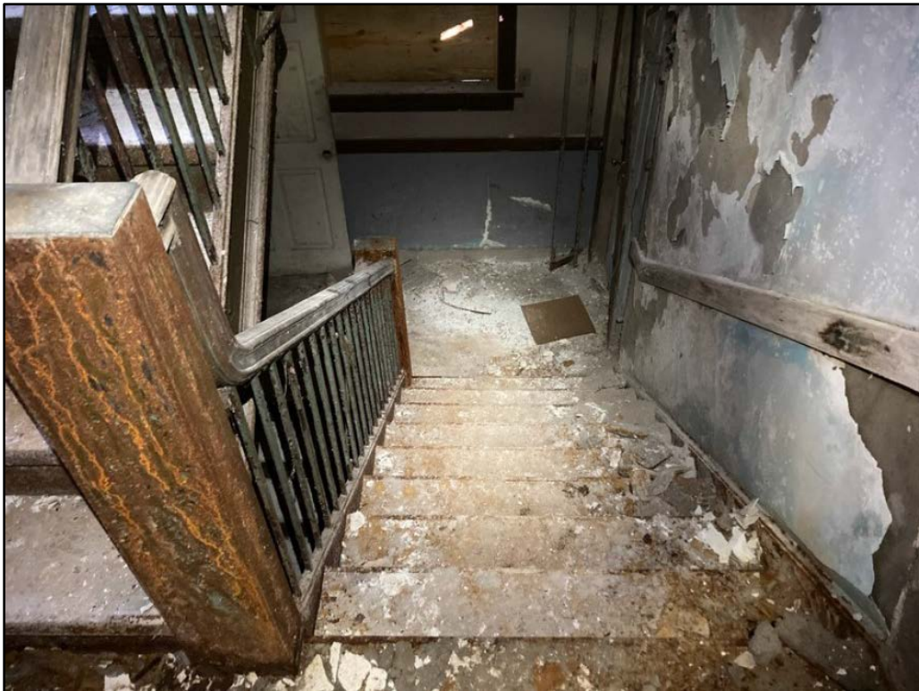
Figure 11. Interior of the former Harriet Tubman YWCA (DH2861), stairwell.
