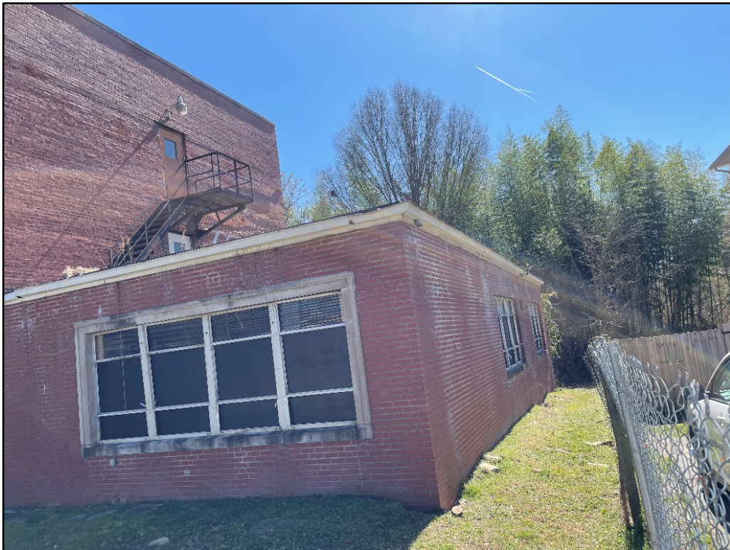
Figure 7. View of the former Harriet Tubman YWCA (DH2861), facing southeast.
