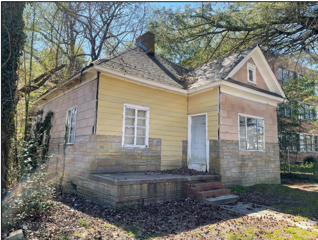
Figure 20. Modern alterations to structure at 316 East Umstead Street, facing southwest.
