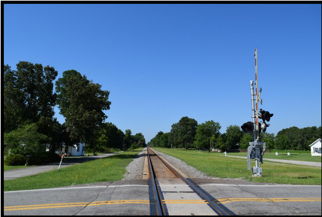
Figure 3.2-6: View of Fayetteville Cutoff (CD1450) as it Crosses Main Street in Godwin, North Carolina, Looking South.
