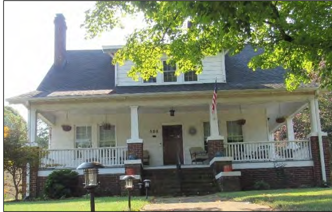
Photo 56: House at 508 S. Main St. Roxboro, West Elevation.
