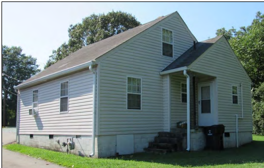
Photo 323: Parsonage, Northeast Oblique.
