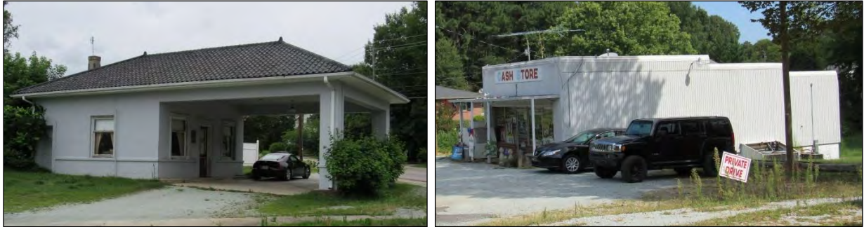
Photo 24: East Elevation of Former Gas Station at 122 Reams Avenue (Left) and Southwest Oblique of Store at 416 Chub Lake Road (Right).
