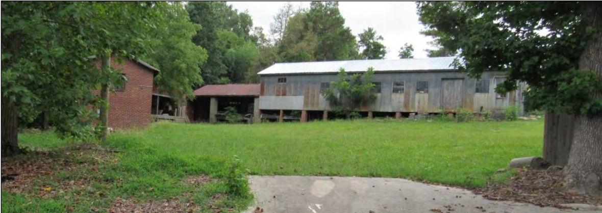
Photo 8: View of Circa-1925 Warehouses of George Kane at 225 Barnett Street, Looking South.
