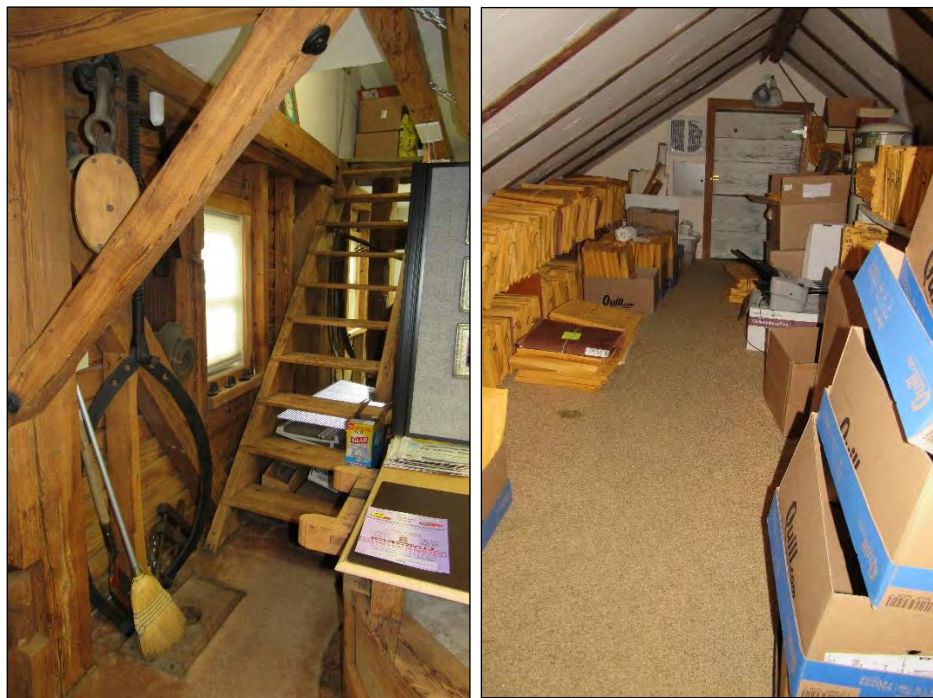
Photo 232: Stairs to Loft Area on Second Level of Mill.
