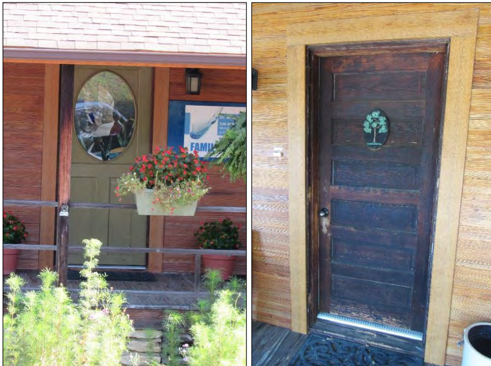
Photo 227: Detail of Main Entrance at Noblett Dentistry, South Elevation (Left) and Door on East Side of the South Elevation (Right).
