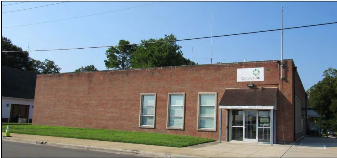
Photo 222: 33 Gordon Street, Looking South.
