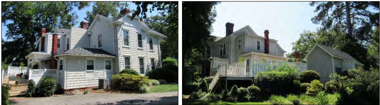
Photo 246: Southwest Oblique (Left) and Northwest Oblique (Right).
