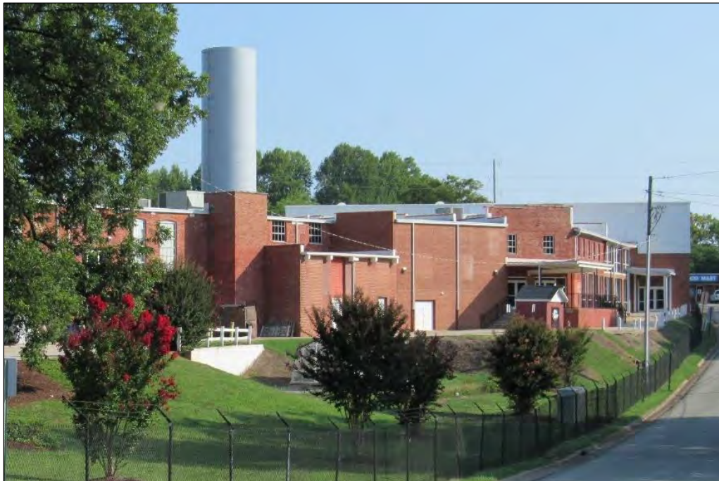
Photo 125: Roxboro Cotton Mill, Looking Northwest.
