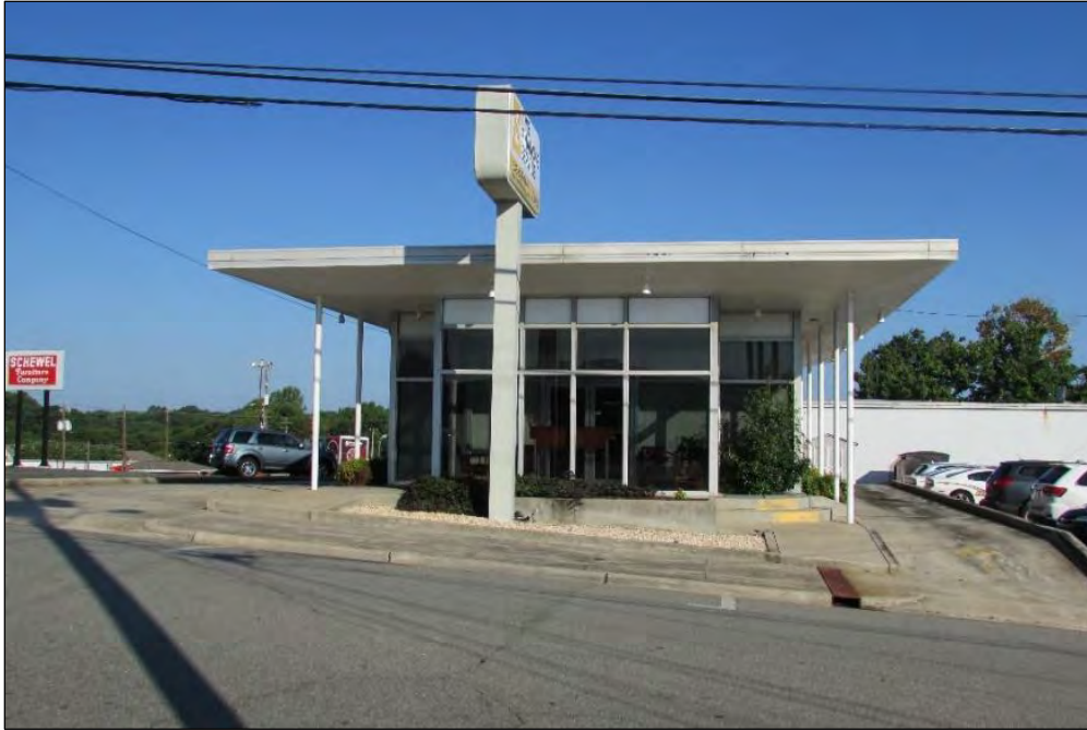
Photo 172: Southeast Elevation of Home Savings & Loan Association Building.
