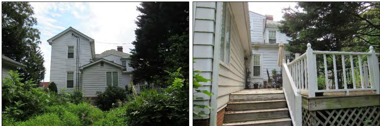
Photo 186: Rear (West) Elevation (Left) and Deck Detail, Looking East (Right).
