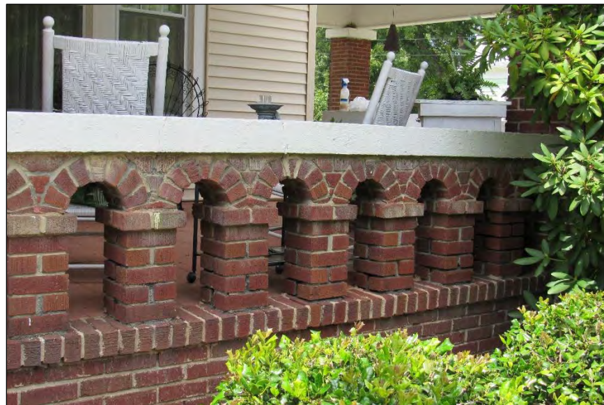
Photo 280: Brick Arcade Balustrade Detail on East Elevation.
