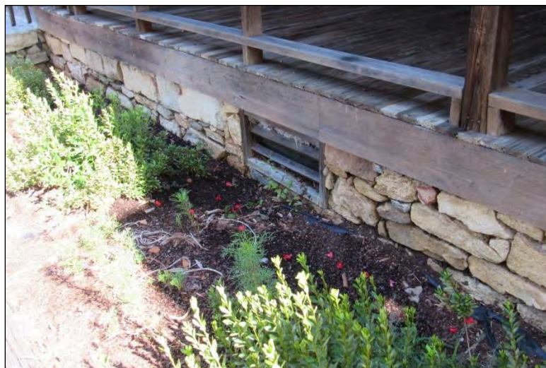
Photo 225: Stone Foundation on South Elevation of McGehee's Mill.
