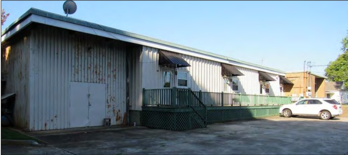
Photo 41: View of Converted Loading Dock Area Facing West.
