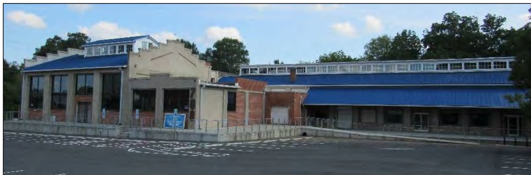
Photo 37: Commercial Building (Former Dye House) at 708 Gilbert Street, Durham, Facing South.
