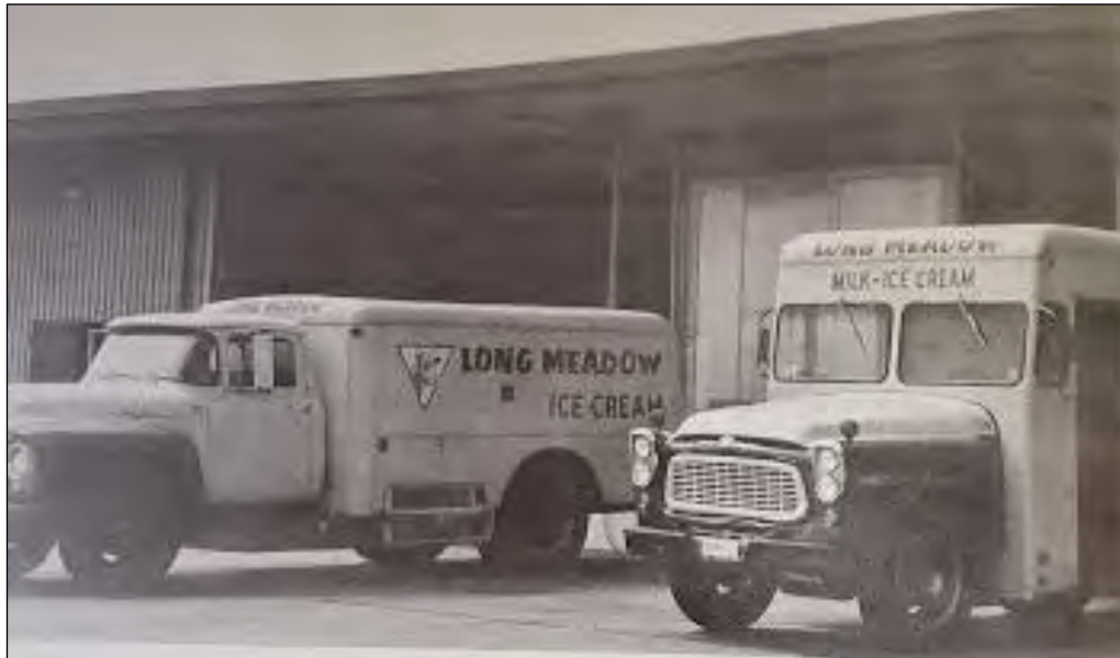
Figure 31: Circa-1971 Image of the Loading Dock Area. 91
