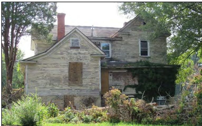
Photo 49: View of the Three Rear Additions, West Elevation.
