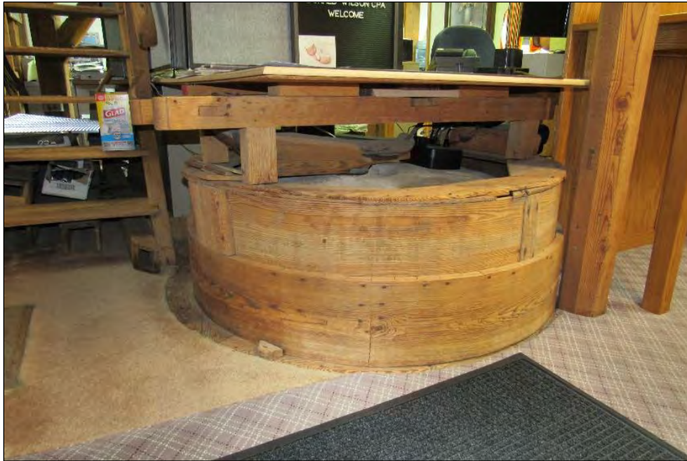
Photo 233: Millstone Enclosed in Wood Hoop on Second Level, Looking South.
