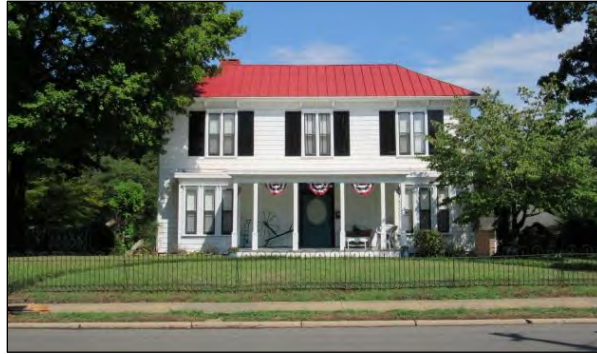
Photo 276: House, 314 S. Main Street, Looking East.
