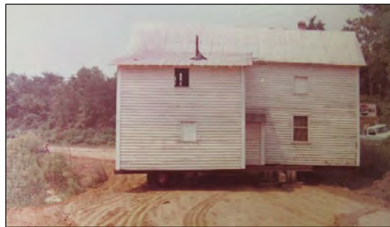
Photo 242: Move of the Mill to Temporary Location in 1973. 526
