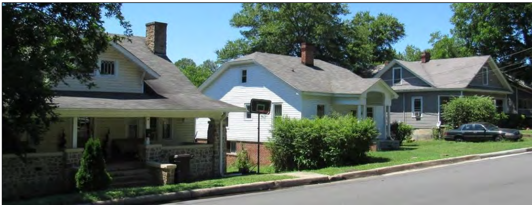
Photo 13: View Looking North at 421–413 S. Lamar Street.
