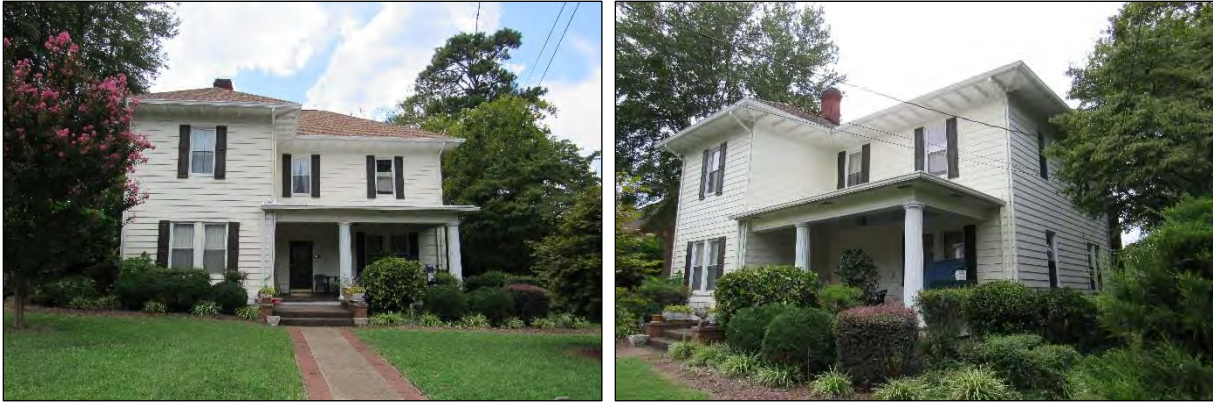
Photo 266: Façade (Left) and Northeast Oblique (Right).
