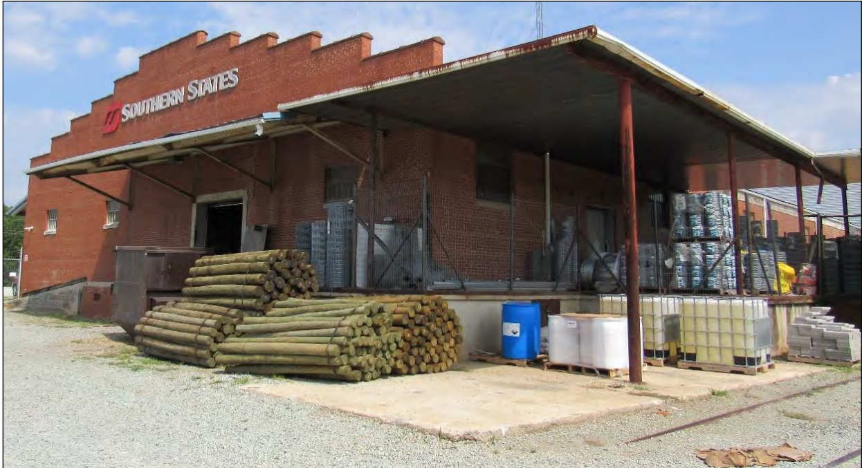
Photo 27: Detail of Southeast Oblique; Note Stepped Parapet and Loading Dock.
