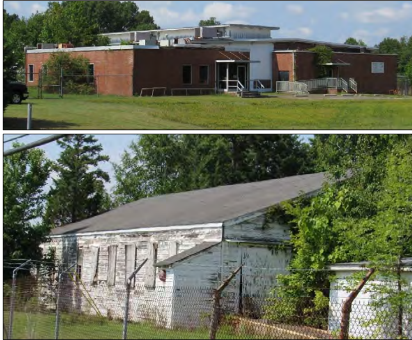
Photo 344: Northeast Oblique of the Primary Resource (Top) and Frame Warehouse (Bottom) of the Somerset Mills on Old Durham Road, Roxboro, North Carolina.
