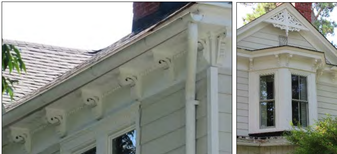
Photo 247: Queen Anne-Style Exterior Details, Looking East (Left) and Southwest (Right).
