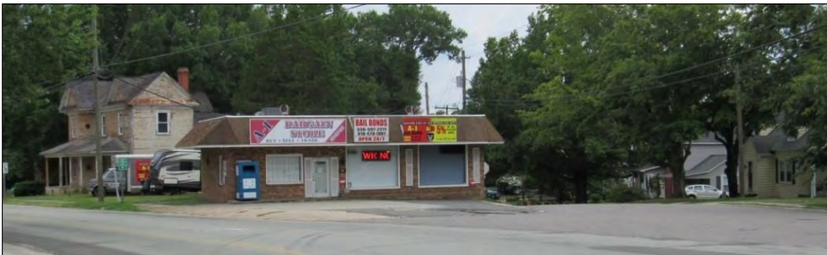
Photo 9: View of Commercial Building at 505 N. Main Street, Looking South Towards N. Lamar Street Intersection.
