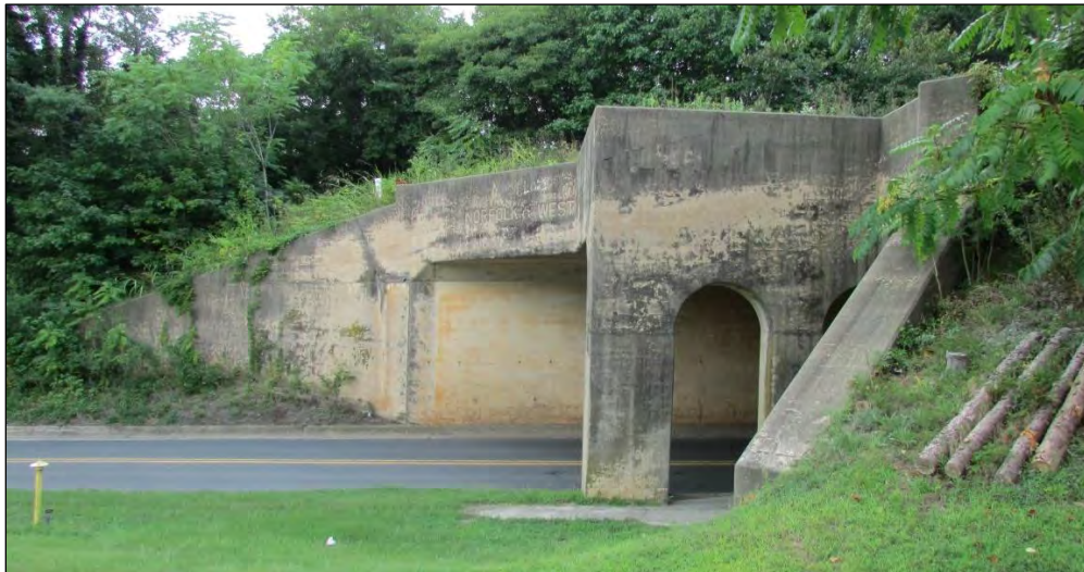
Photo 328: View of East Elevation, Looking Southwest.
