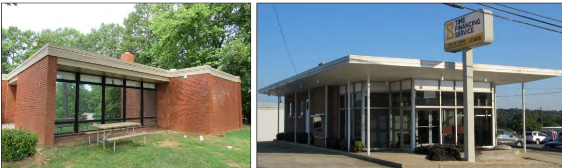
Photo 45: Former Person County Medical Center at 204 West Barden Street, South Oblique (Left), and Home Savings and Loan Association at 123 S. Lamar Street, South Oblique (Right).
