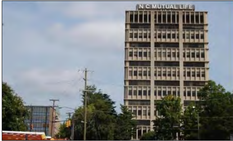
Photo 144: North Carolina Mutual Life Insurance Building, 411 West Chapel Hill Road, Durham. 326
