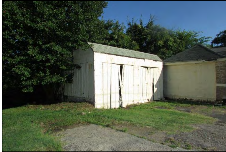
Photo 290: Auto Service Building at Rock Inn, Southeast Oblique.
