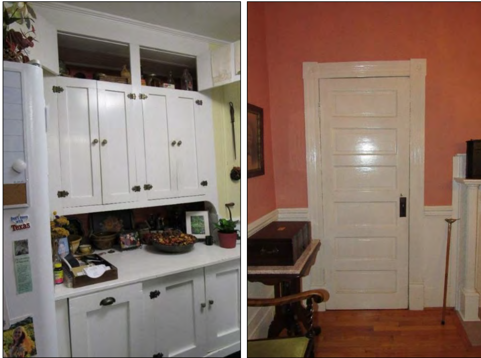
Photo 190: Original Built-In Kitchen Cabinet, Looking West (Left) and Door and Surround Detail in Current Dining Room (Former Master Bedroom) Looking East (Right).
