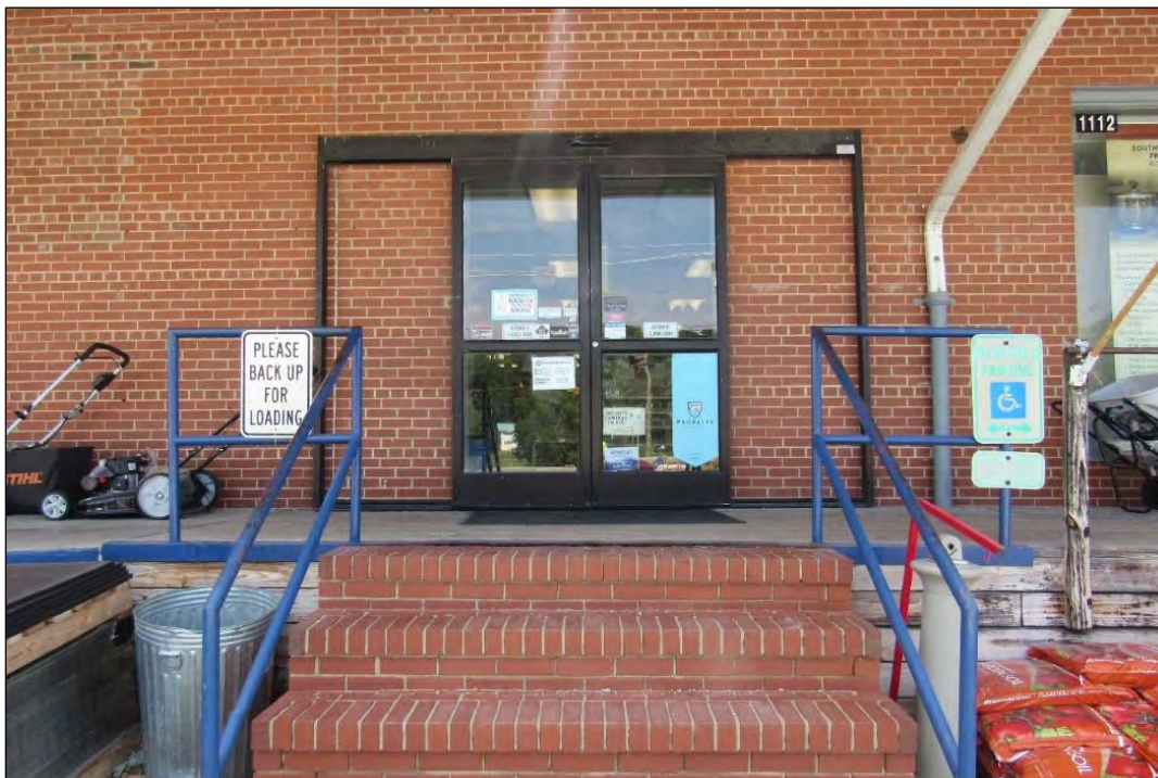
Photo 30: Detail of Primary Entry to Retail Store on West Elevation.
