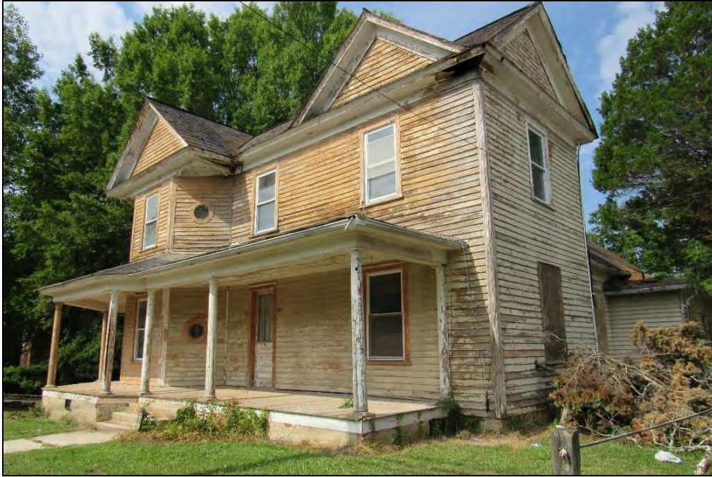
Photo 46: Newell House, Northeast Oblique.
