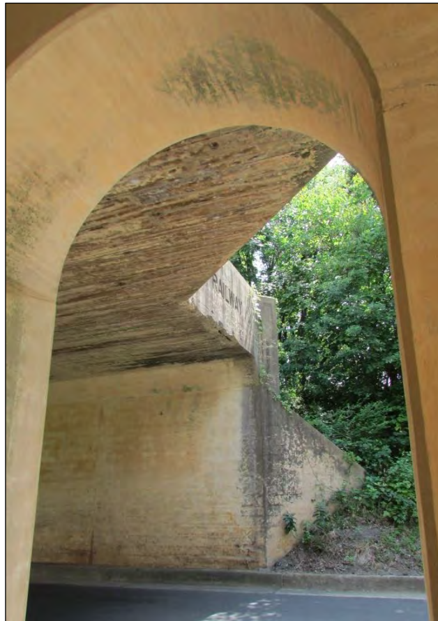
Photo 333: View of West Wall from Walkway Showing Various Form Marks.
