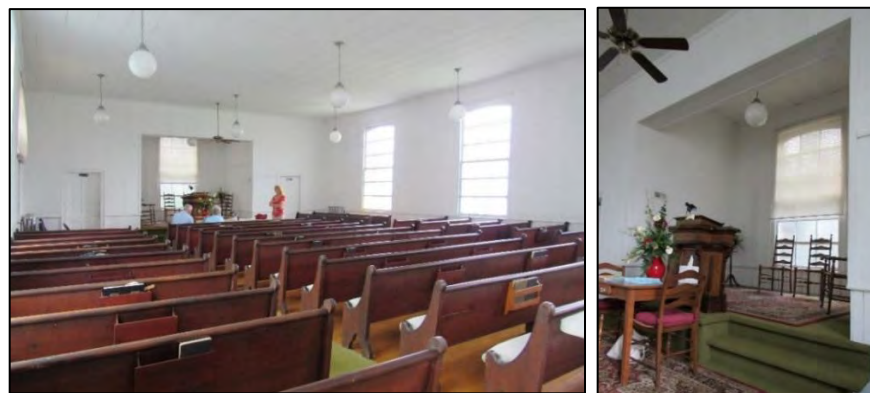
Photo 96: View of Sanctuary, Looking North (Left), and View of Chancel, Looking Southwest (Right).
