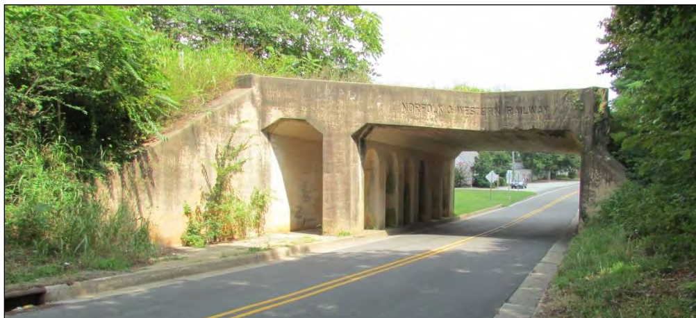
Photo 329: West Elevation of Underpass.
