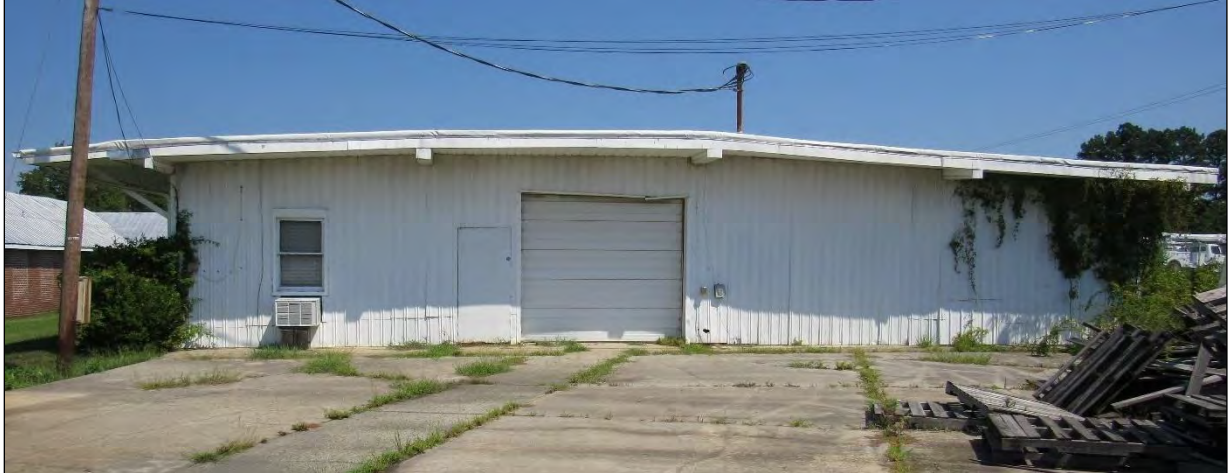
Photo 342: South Elevation of Frame Warehouse.
