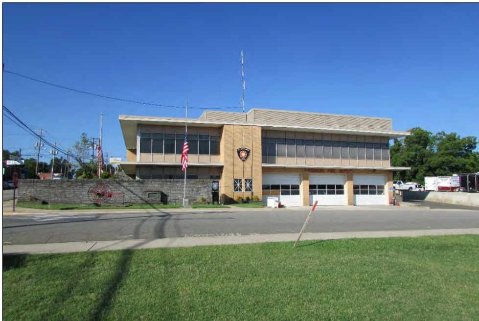
Photo 134: Northeast Elevation and Fire Station Entrance.
