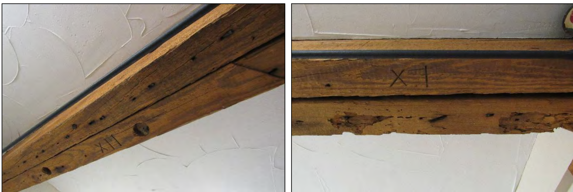
Photo 235: Roman Numeral Markings on Ceiling Beam in Second Floor Office Space.
