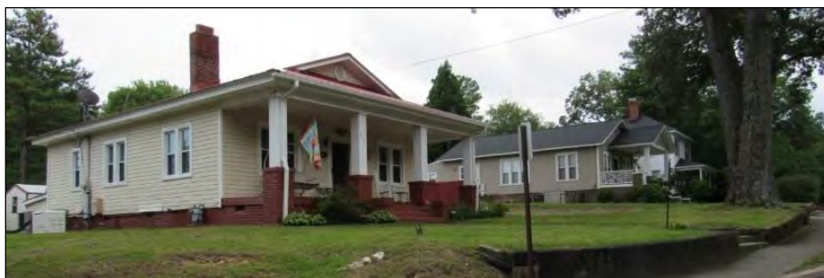
Photo 5: View Looking Southwest at 215–219 Barnett Street.
