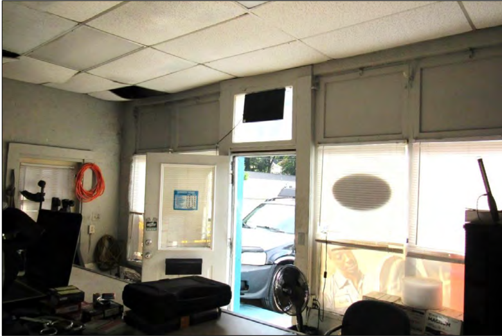
Photo 107: Interior View of Storefront, Looking East.
