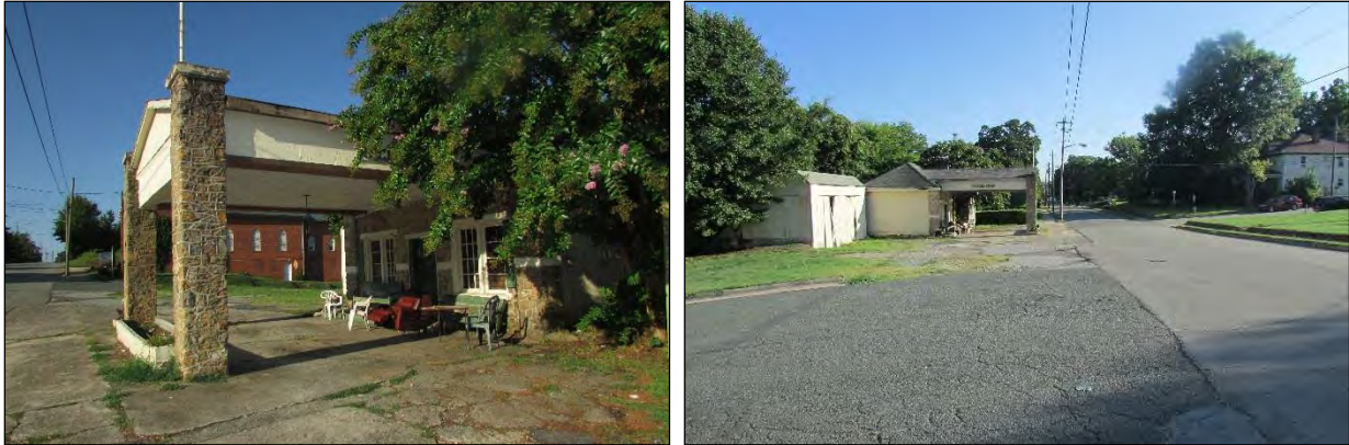
Photo 288: Northeast Oblique of Canopy (Left) and South Elevation (Right).
