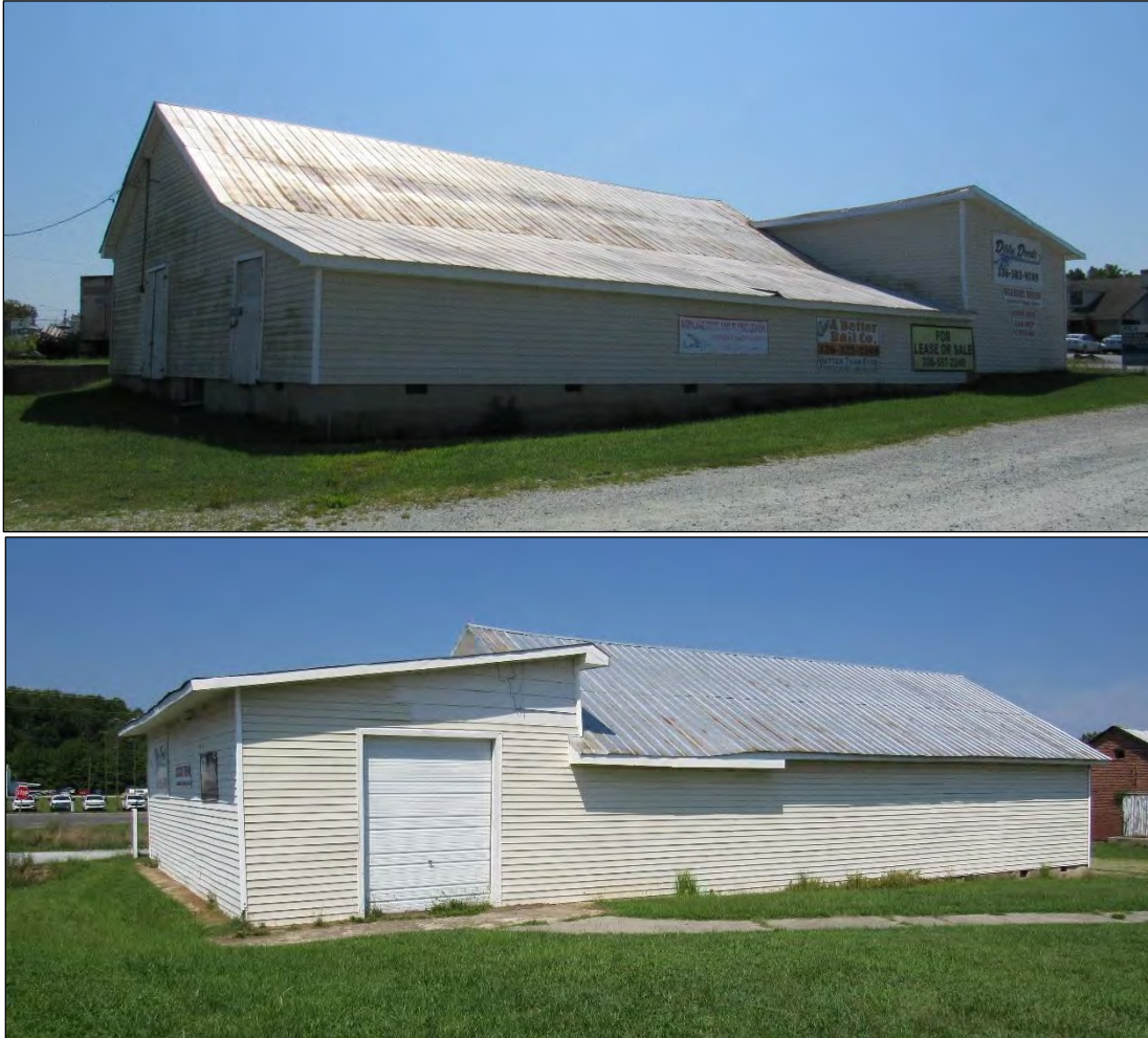
Photo 341: Northwest Oblique (Top) and Southeast Oblique (Bottom) of Circa-1920 Frame Warehouse.
