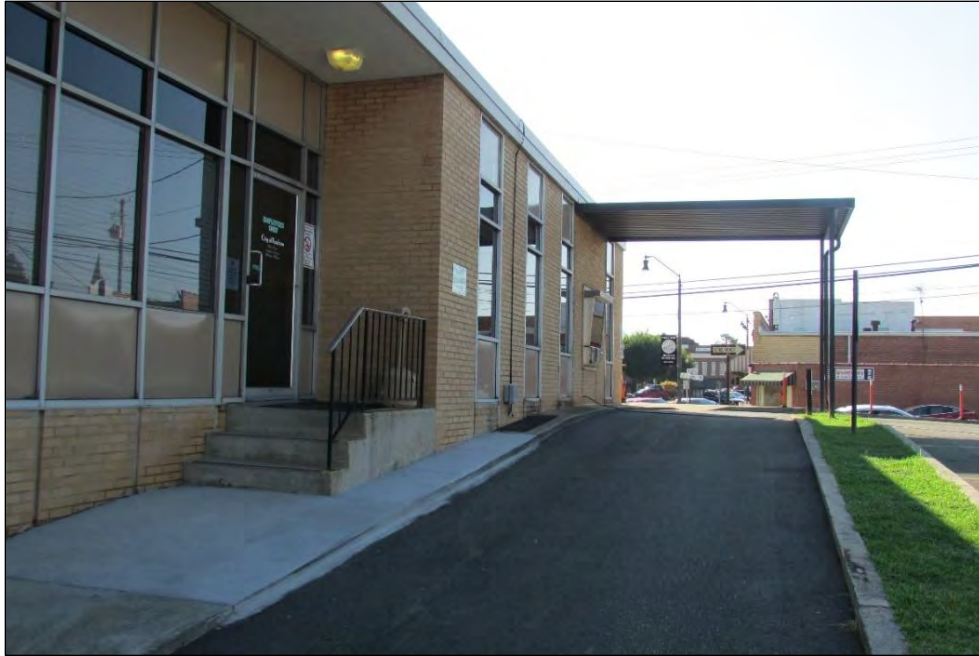
Photo 133: Detail of Drive-Thru Canopy Over Teller Window, Looking Southeast.
