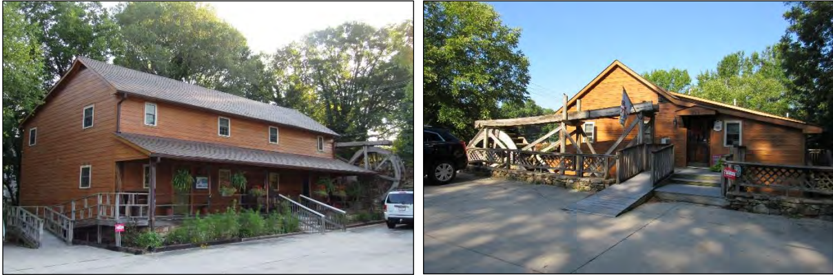
Photo 223: Southwest Oblique (Left) and East Elevation (Right).
