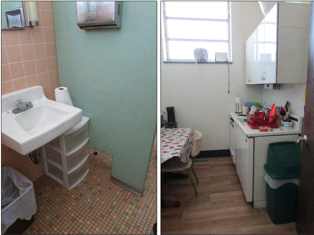
Photo 180: Bathroom Fixtures and Tile (Left) and Kitchen Cabinet, Stove, and Window (Right) at Home Savings & Loan Association.
