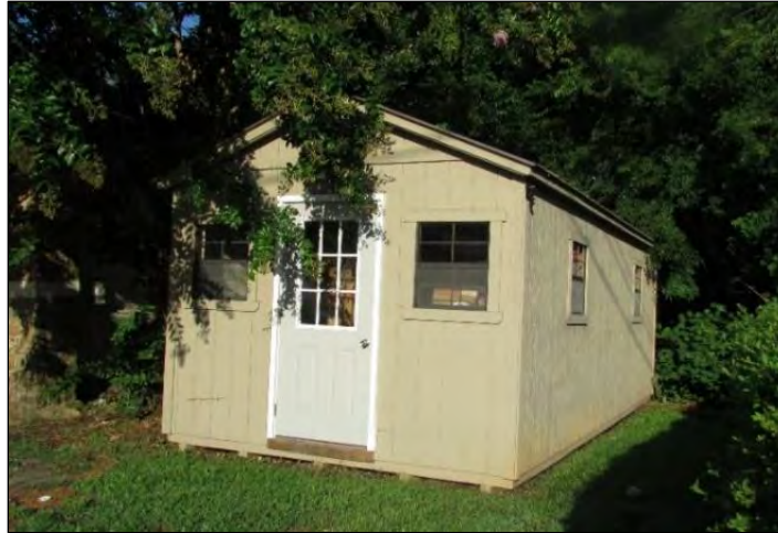
Photo 292: Circa-2018 Shed at Rock Inn, Northeast Oblique.
