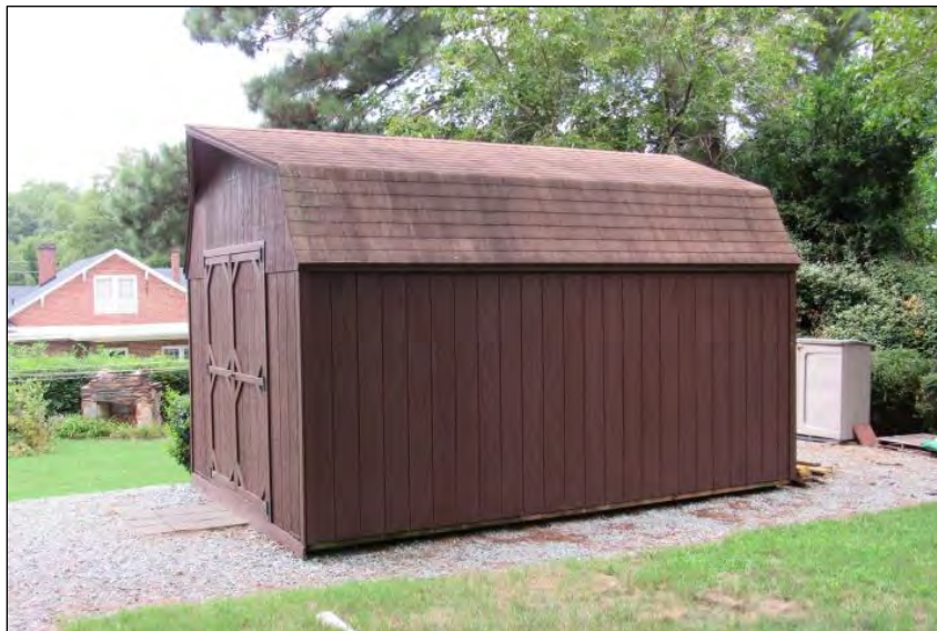
Photo 274: Shed, Looking Northwest.
