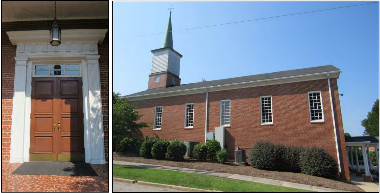
Photo 69: Detail of Primary Entrance, East Elevation (Left) and North Elevation (Right).
