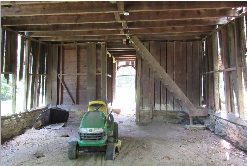
Photo 195: Interior of Stable, Looking East.
