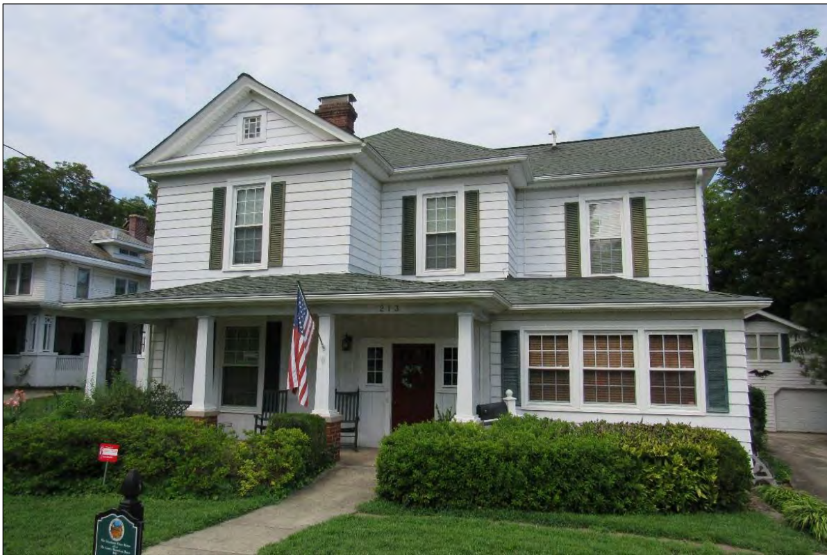
Photo 182: East Elevation (Façade).
