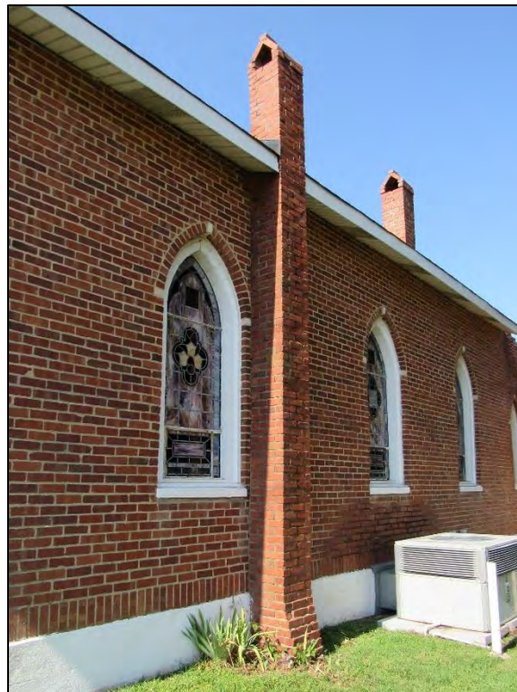
Photo 317: Detail of Foundation, Siding, and Chimneys, North Elevation.
