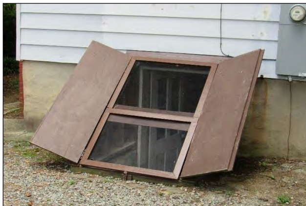
Photo 268: Bulkhead Door and Entrance to Basement on West Elevation.
