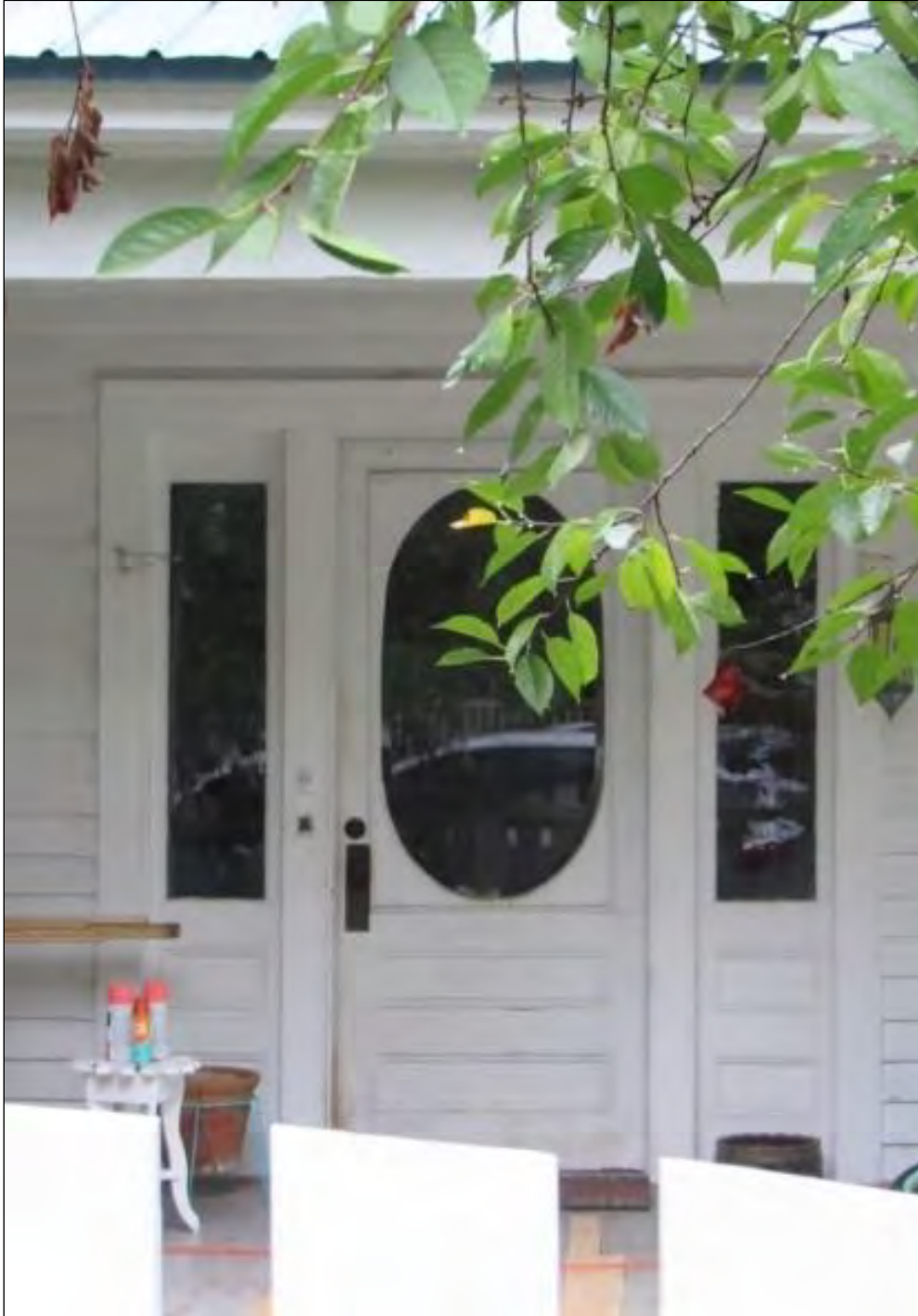
Photo 86: Primary Entry Detail on Northeast Elevation.
