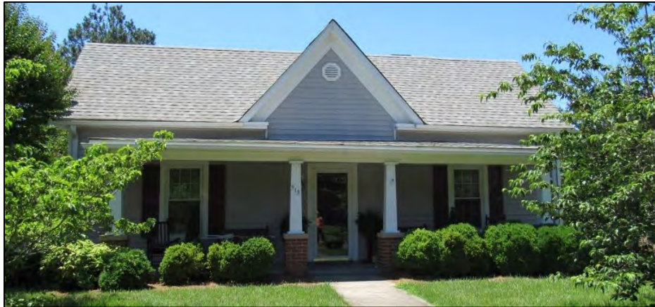
Photo 10: East Elevation of the House at 513 S. Main Street.
