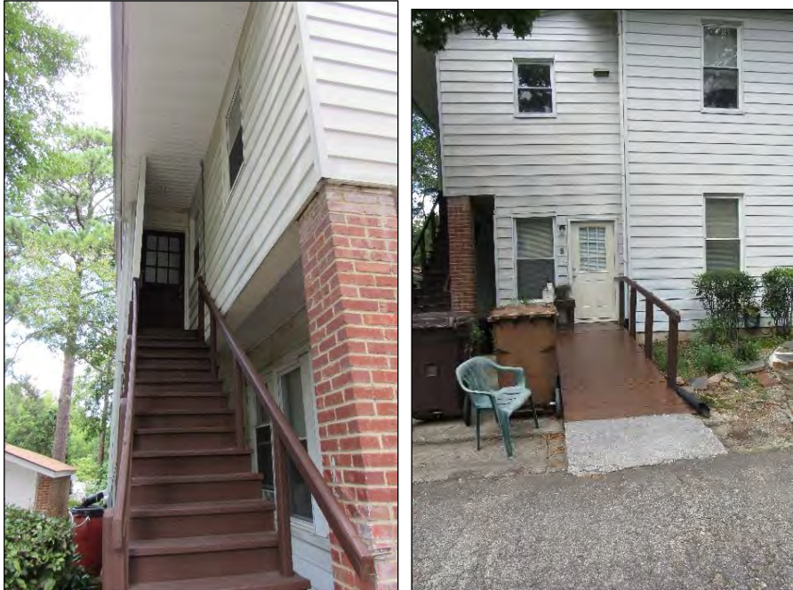
Photo 272: Rear Addition Entrances: Looking North (Left) and Looking North (Right).
