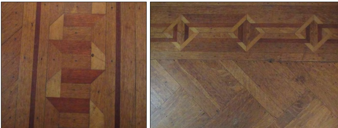
Photo 203: Details of Parquet Flooring in Lower Level.
