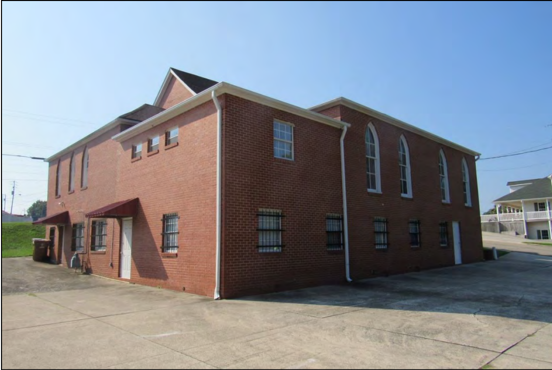
Photo 155: Circa-1995 Addition, North Oblique.
