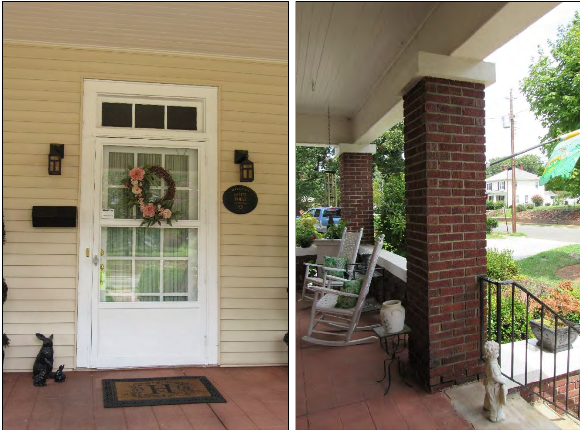
Photo 279: Primary Entrance (Left) and Column Detail (Right) on East Elevation.
