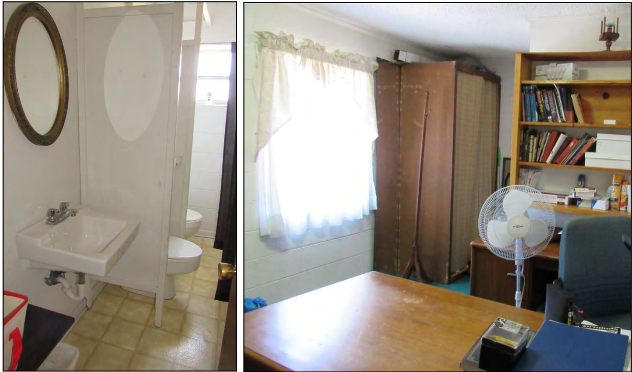
Photo 162: Bathroom, Looking Northeast (Left) and Office, Looking North (Right) in the Circa-1995 Addition.
