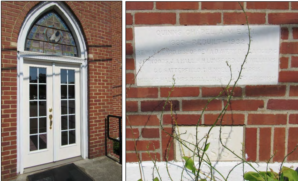
Photo 318: Primary Entrance Detail (Left) and Cornerstones (Right), Both on Façade.
