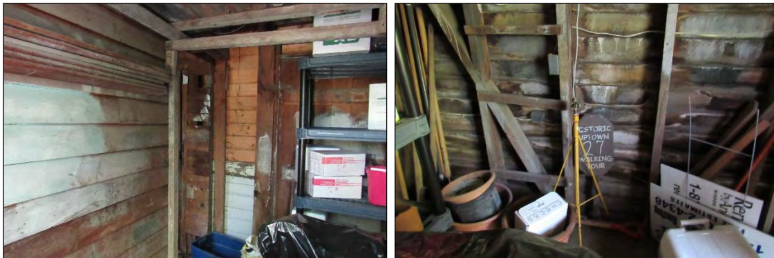
Photo 263: Interior Details of Shed: Looking East (Left) and Looking South (Right).
