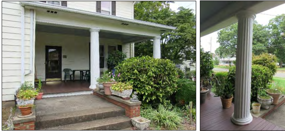
Photo 269: Porch on Façade (Left) and Porch Column Detail, Looking Northeast (Right).
