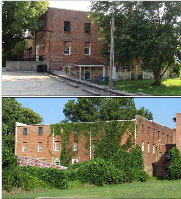
Photo 343: Southwest (Top) and Northeast (Bottom) Oblique of Brick Warehouse (PR0225).
