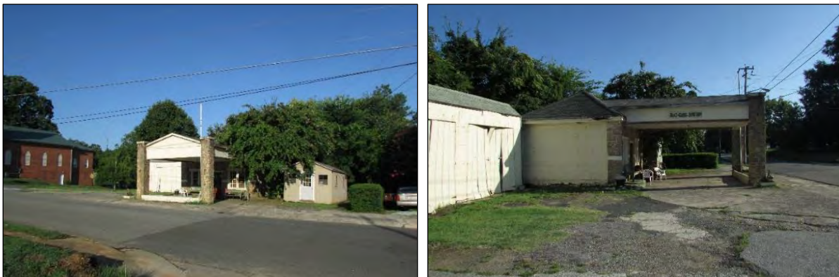
Photo 286: Northeast Oblique (Left) and South Elevation (Right).
