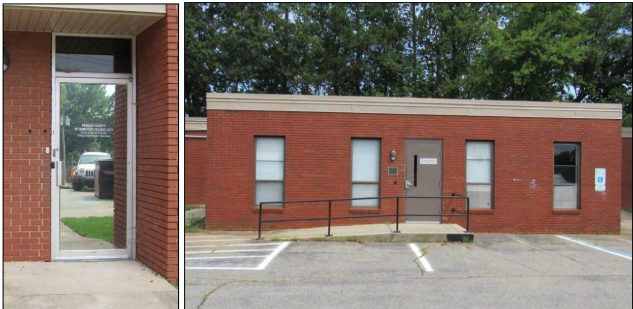
Photo 213: Primary Entrance (Left) and Secondary Entrance (Right) on the South Elevation.
