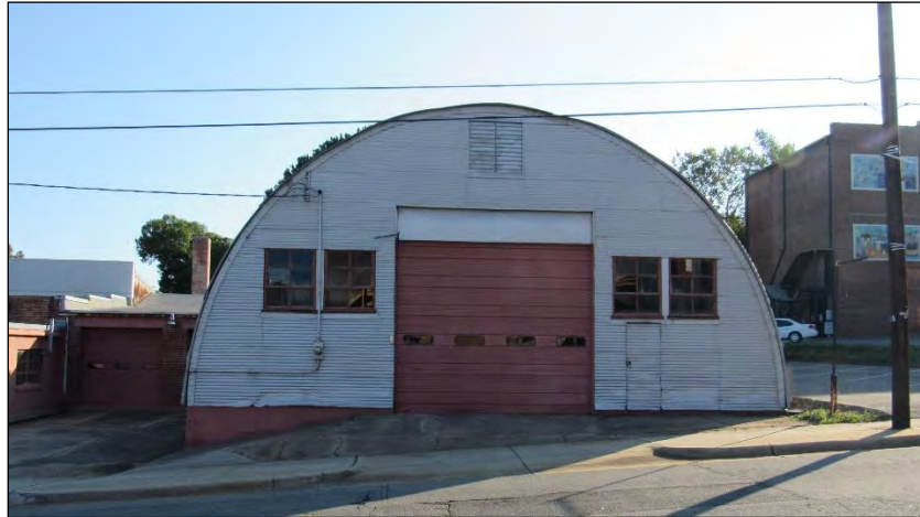
Photo 123: South Elevation of Quonset Hut from Reams Avenue.
