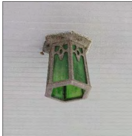
Photo 270: Original Porch Light Over Primary Entrance on East Elevation.
