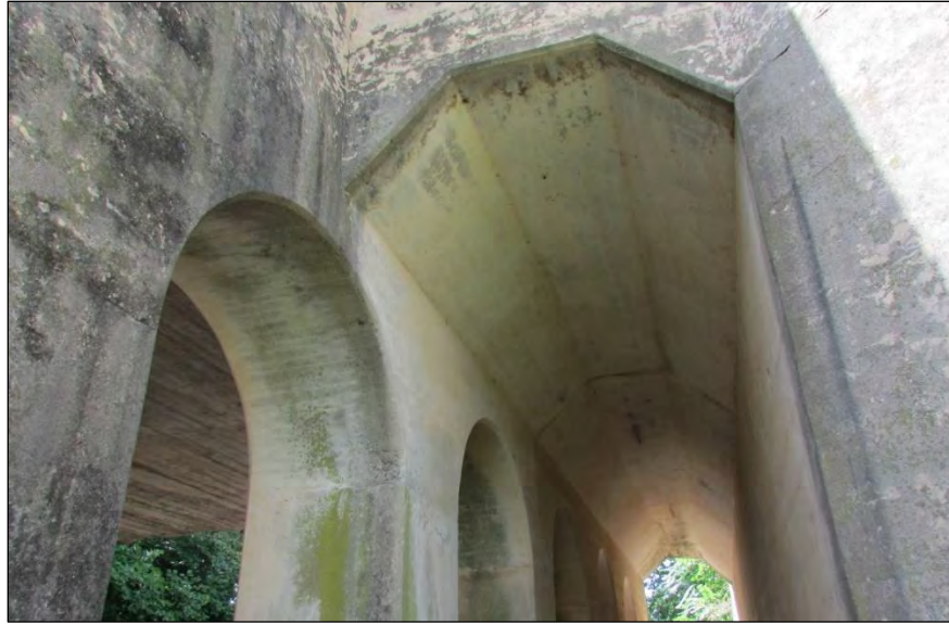
Photo 332: Detail of Pedestrian Walkway, East Elevation.
