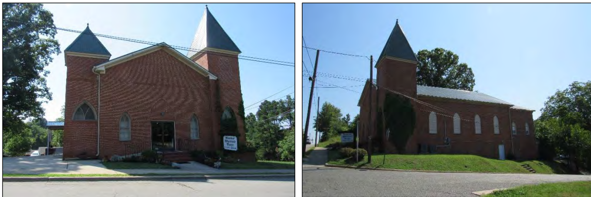
Photo 306: East Elevation (Left) and North Elevation (Right).
