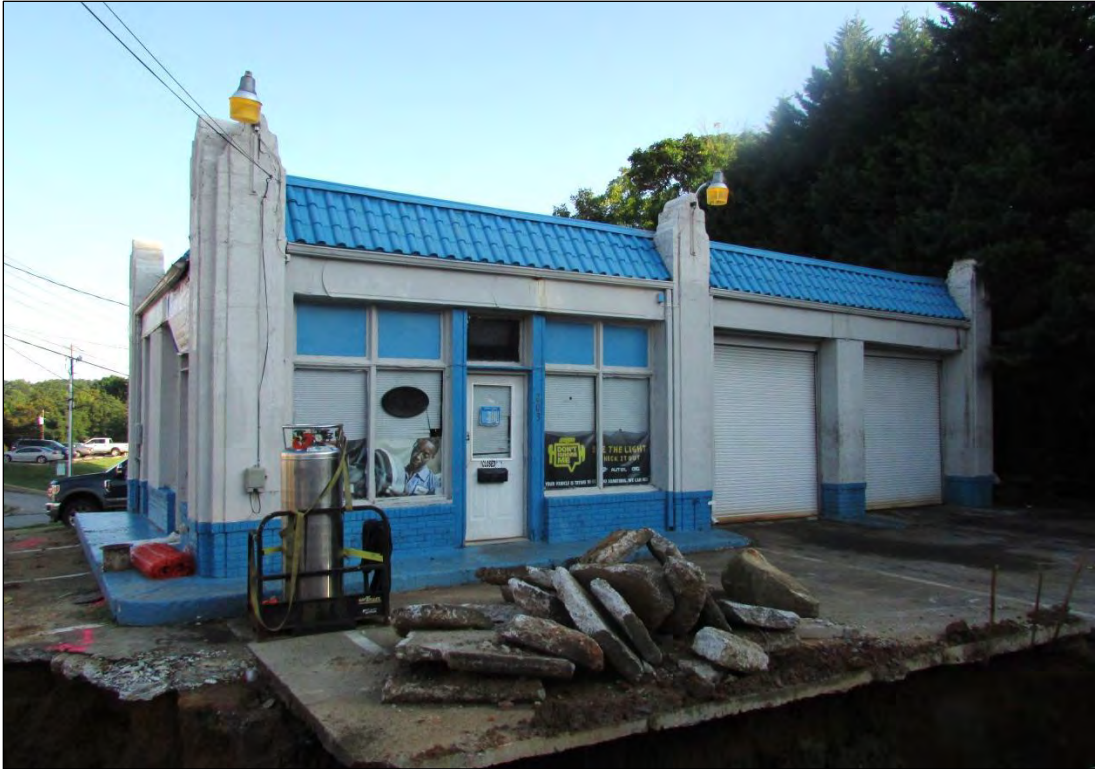
Photo 101: View of East Elevation, Showing Storefront and Service Bays.
