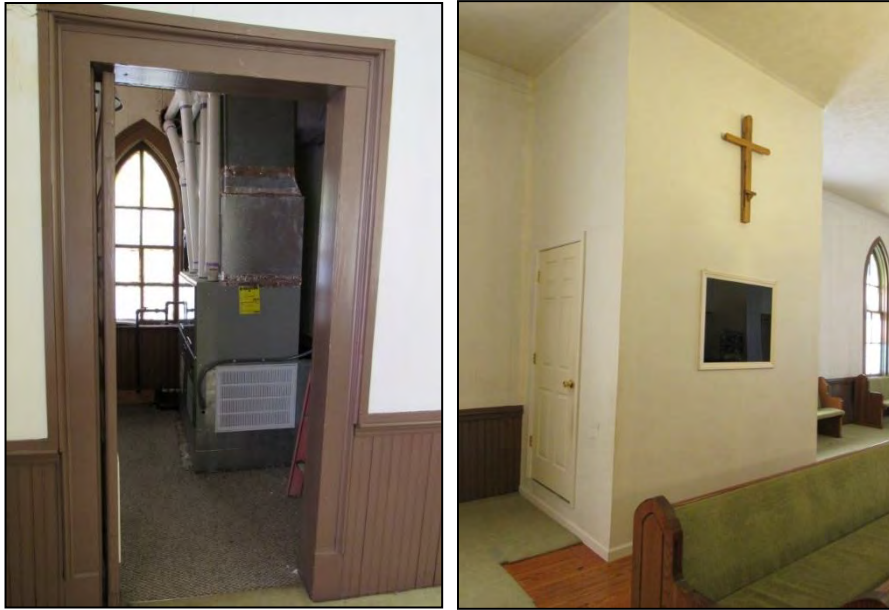
Photo 160: Boiler Room, Looking Northwest (Left), and Sound Room, Looking South (Right).
