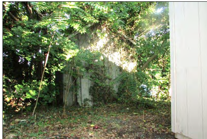
Photo 291: Circa-1935 Shed at Rock Inn, East Elevation.
