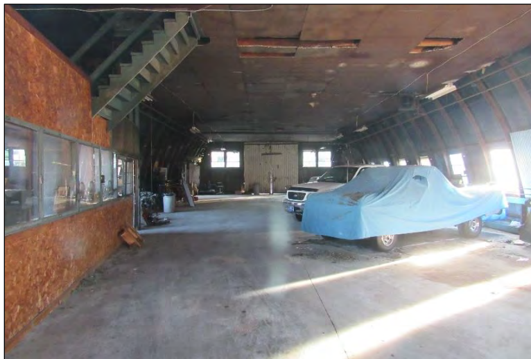
Photo 124: Interior of the Quonset Hut Addition, Facing North.
