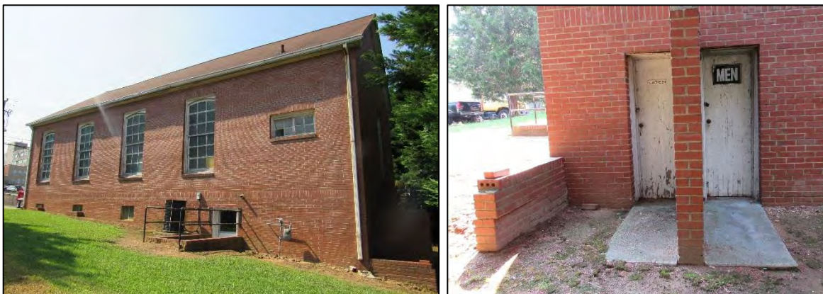
Photo 94: East Oblique (Left) and Bathroom Entrance Detail on Northeast Elevation (Right).
