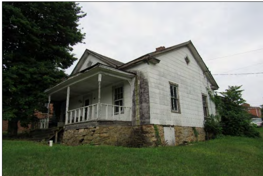
Photo 305: 102 Leasburg Road, Looking Southeast.
