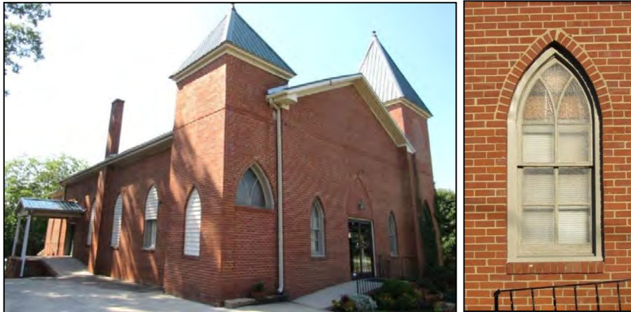
Photo 170: Former First Baptist Church (PR0321), Southeast Oblique (Left) and Window Detail (Right).
