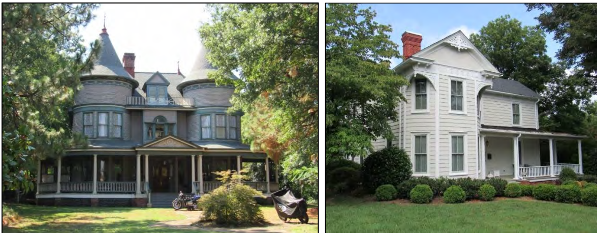
Photo 11: East Elevation of J.A. Long House at 217 S. Main Street (Left) and Southeast Oblique of James Sidney Bradsher House at 421 S. Main Street (Right).
