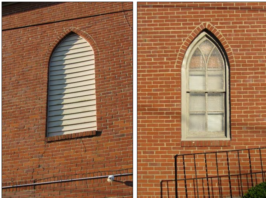
Photo 309: Window Details: North Elevation (Left) and East Elevation (Right).
