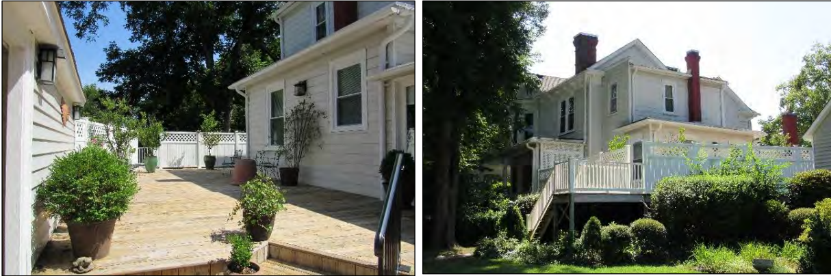
Photo 250: Rear Deck Details, Looking North (Left) and Southeast (Right).
