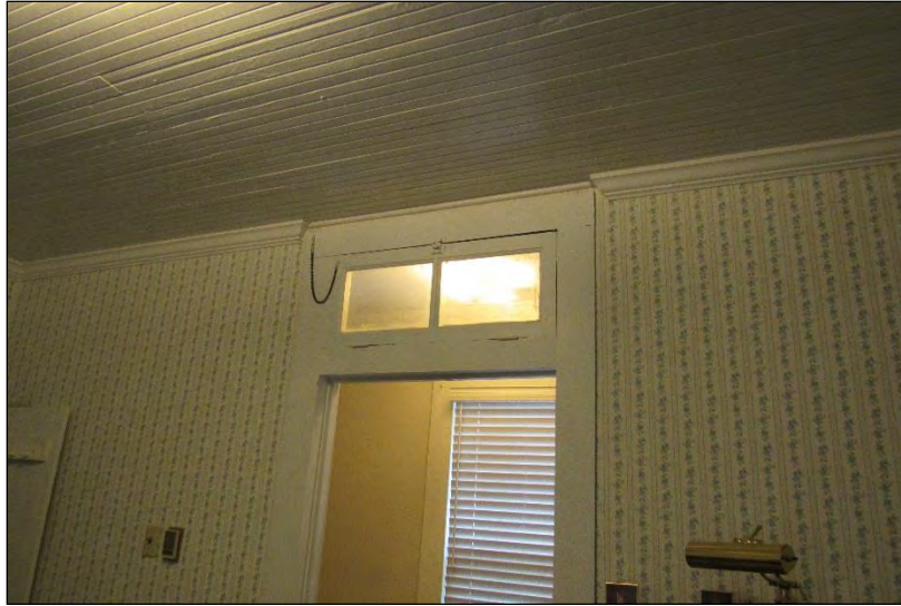
Photo 193: Ceiling and Transom Detail in Boarding House Bedroom Addition, Looking South.
