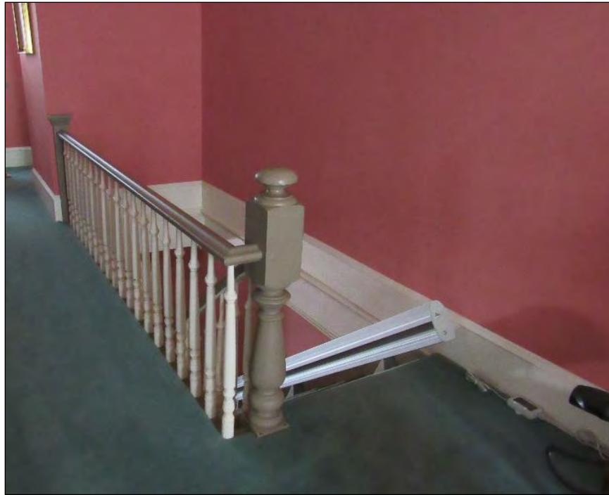
Photo 256: Staircase from Second Floor, Looking West.
