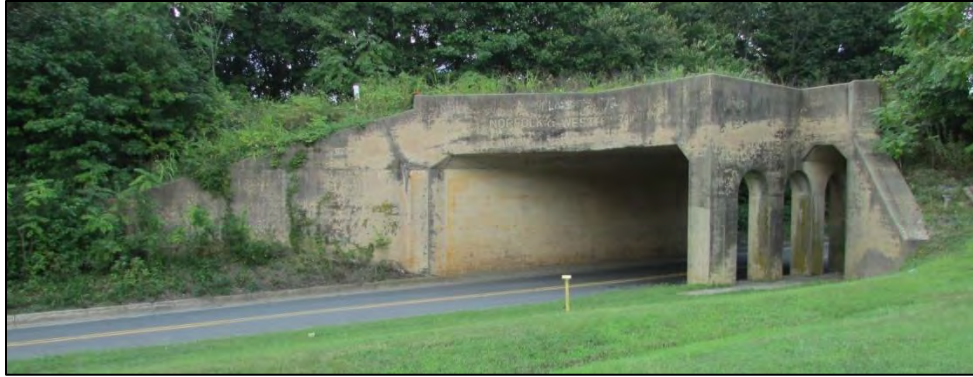
Photo 327: East Elevation of Underpass.
