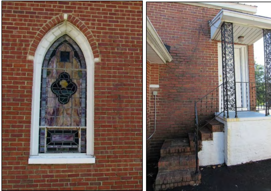
Photo 319: Window Detail (Left) and Addition Entrance on Northeast Corner (Right).
