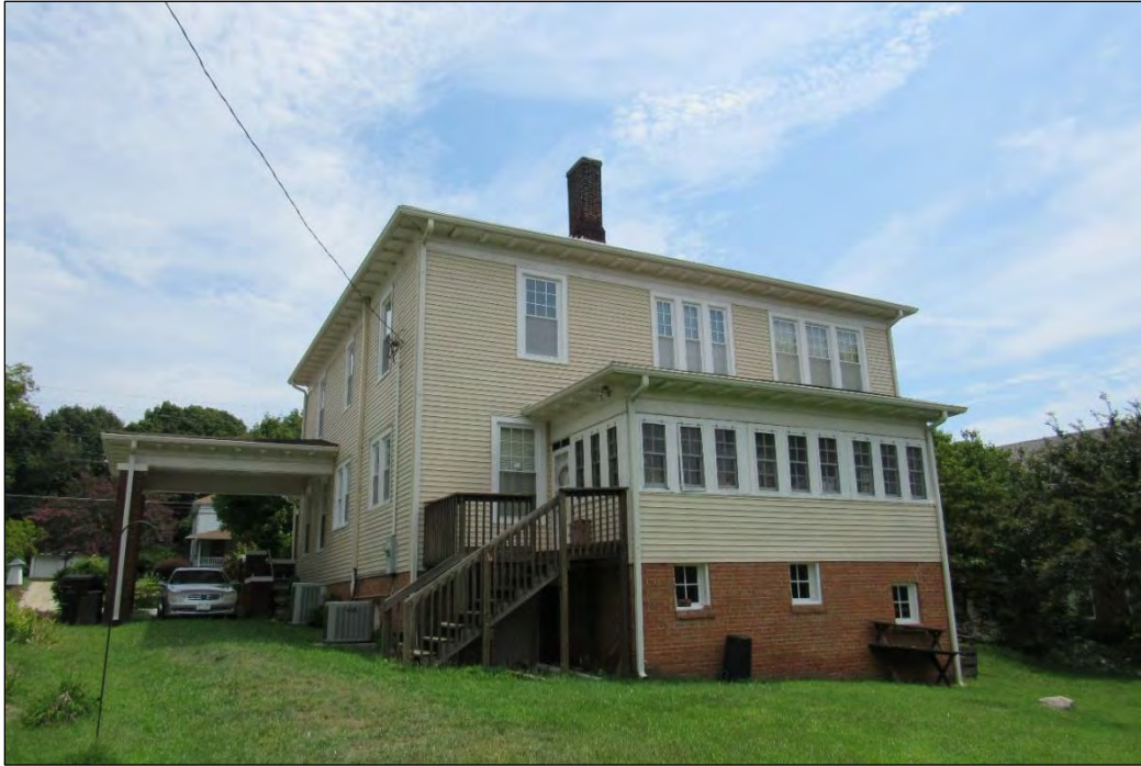
Photo 283: Rear (West) Elevation of Hester House.
