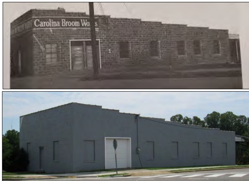
Photo 345: Historic Image of the Carolina Broom Works Building, West Elevation (Top) and Current View of Building, Northwest Oblique (Bottom). 802
