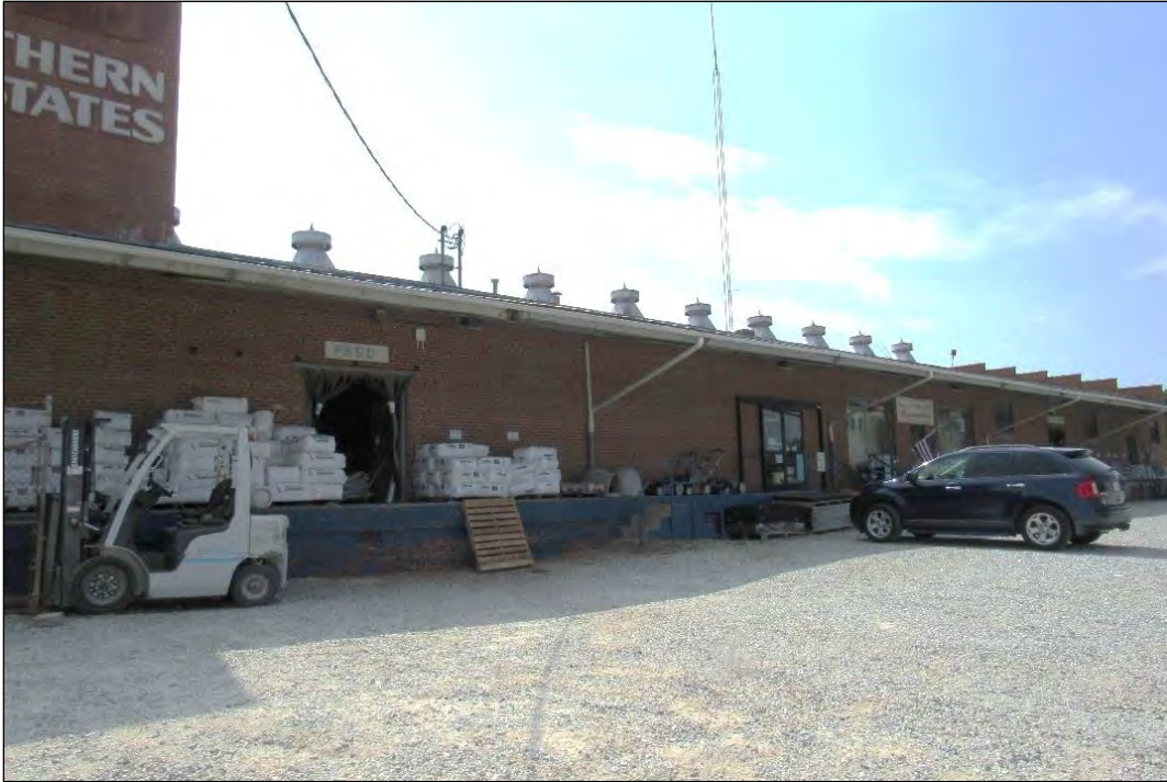
Photo 29: West Elevation Facing Southeast.
