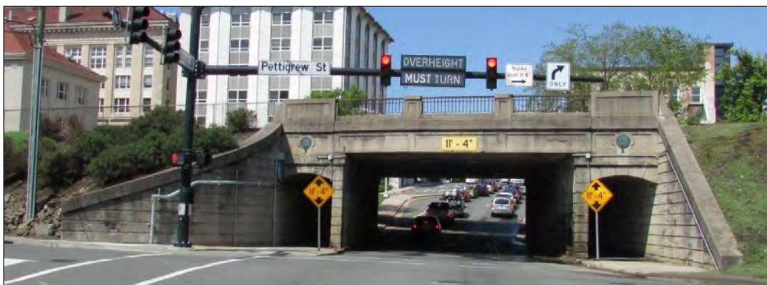
Photo 337: Southern Railway Bridge (DH2504) over S. Roxboro Street, Looking North.
