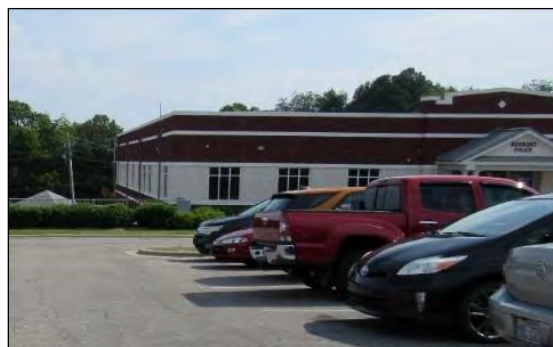
Photo 149: Roxboro Police Station at 109 N. Lamar Street, Looking Northeast.
