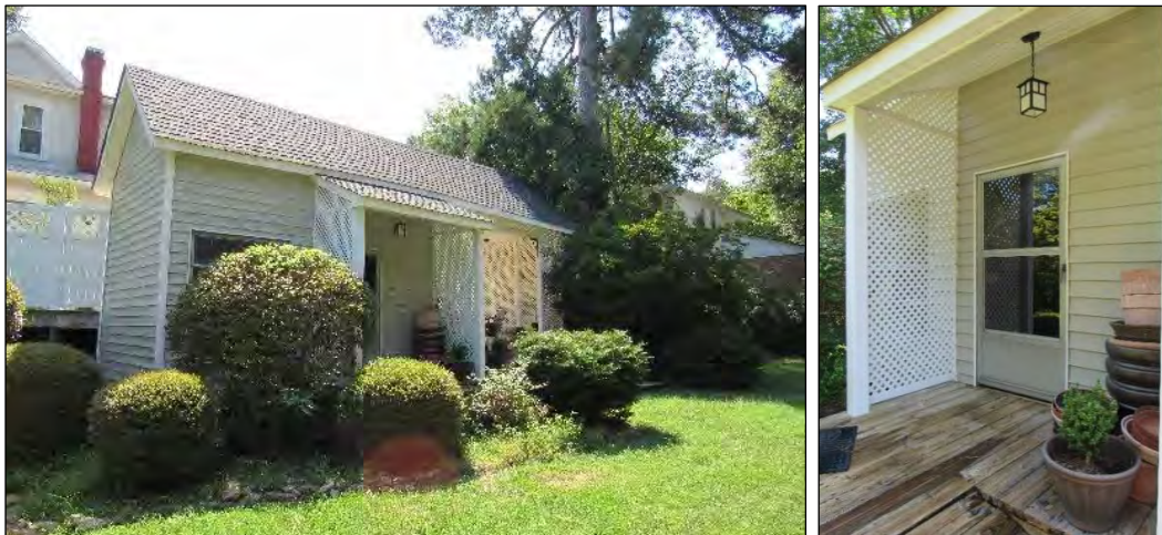
Photo 261: Shed, Looking East (Left) and Detail of Shed Entrance (Right).
