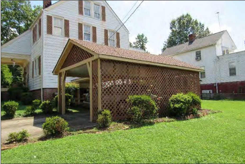
Photo 55: View of Carport, Facing Southeast.
