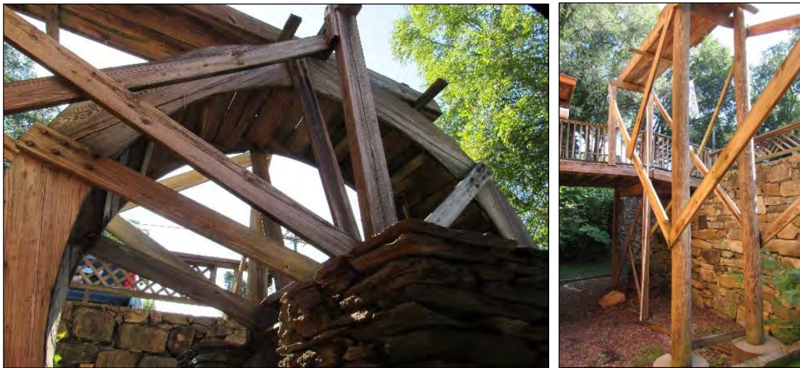
Photo 239: Details of Wood Work and Condition.
