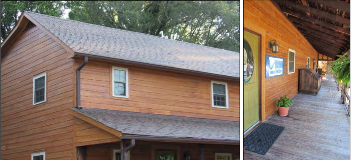
Photo 226: Roof Detail and Porch Detail on McGehee's Mill on South Elevation.
