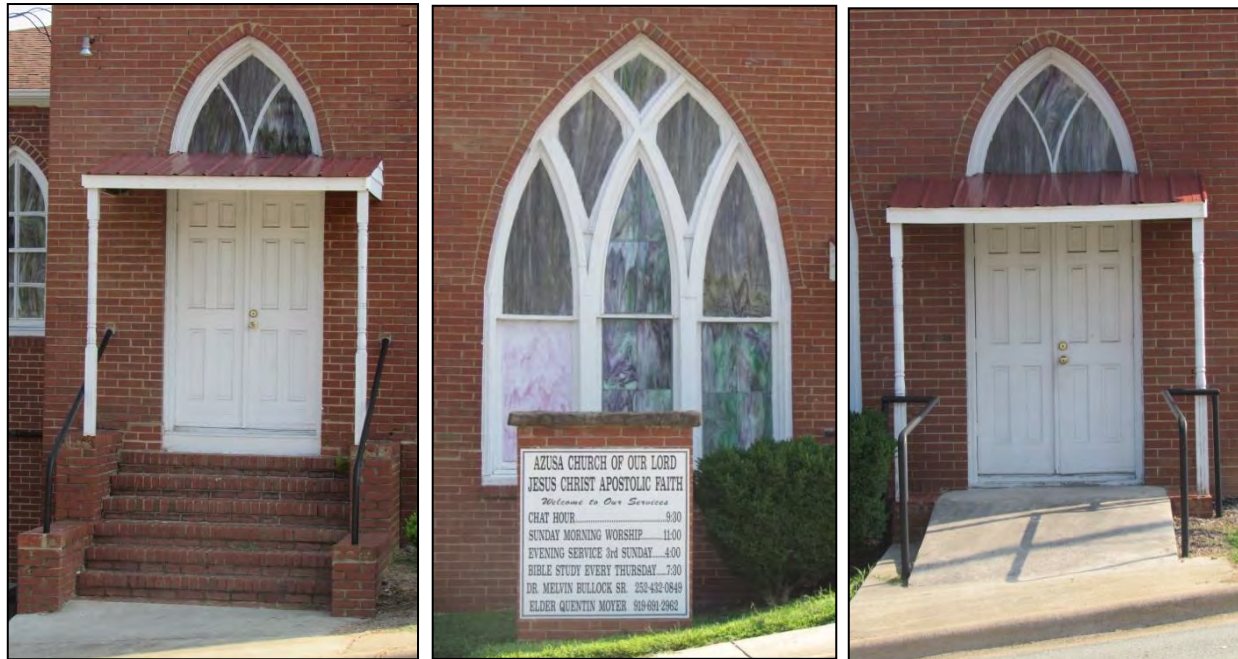
Photo 152: Primary Entrances and Window on the Southwest Elevation.
