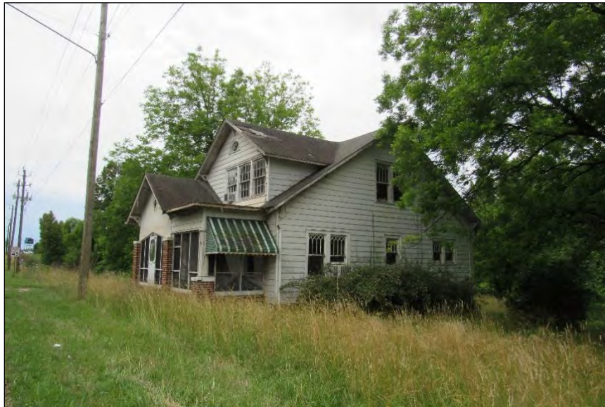
Photo 303: 1522 Durham Road, Looking Southwest.
