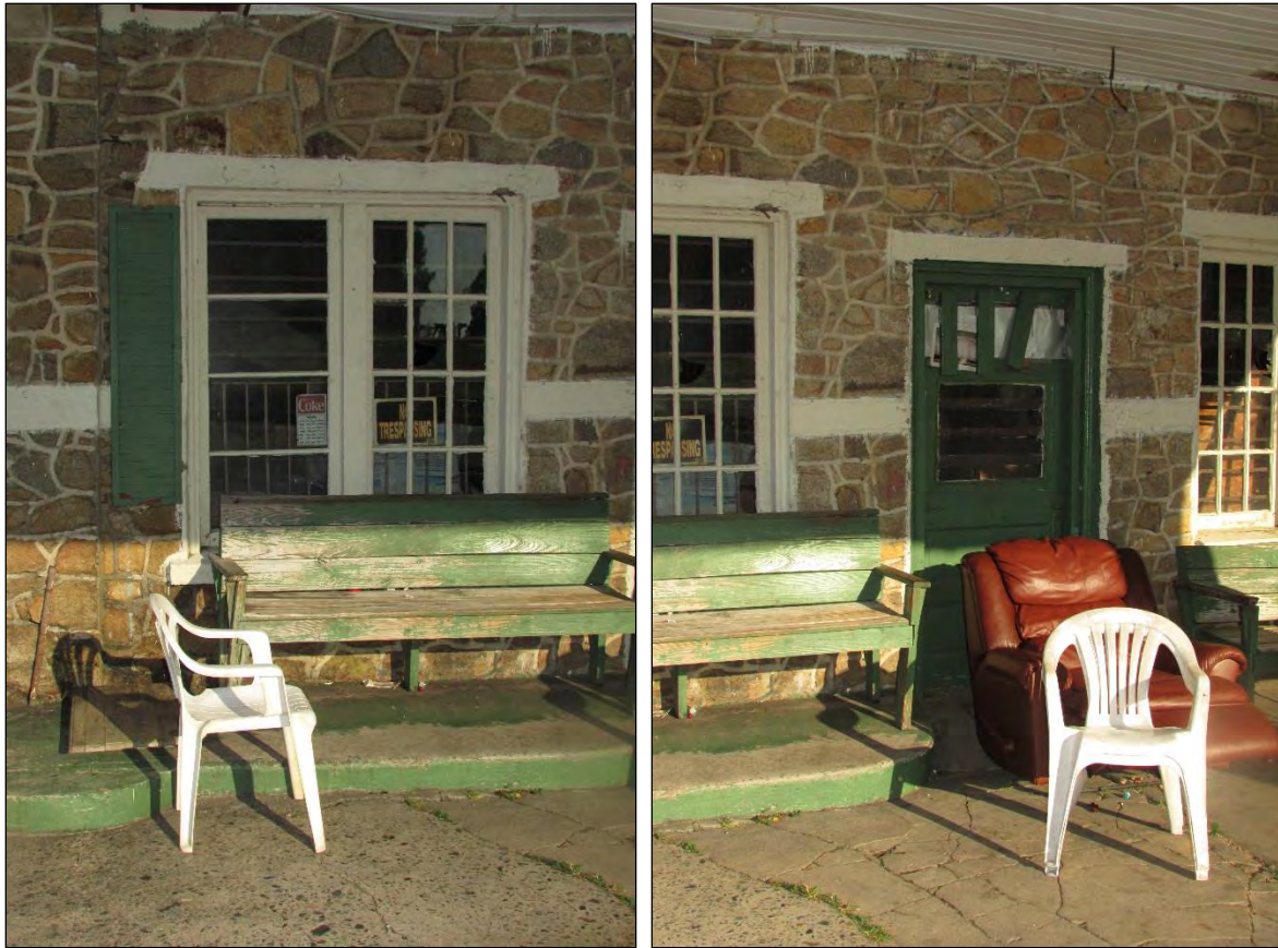
Photo 287: Window (Left) and Door (Right) Detail on the Façade.
