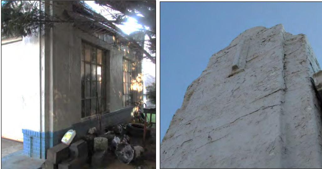
Photo 103: View of Northeast Corner and North Elevation (Left) and Detail of Sculpted Pinnacle at Southeast Corner (Right).
