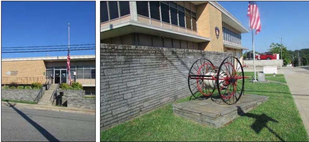
Photo 142: Flagpole at Entrance on S. Lamar Street (Left), Looking West and Memorial Area and Flagpole on Court Street (Right), Looking Southwest.
