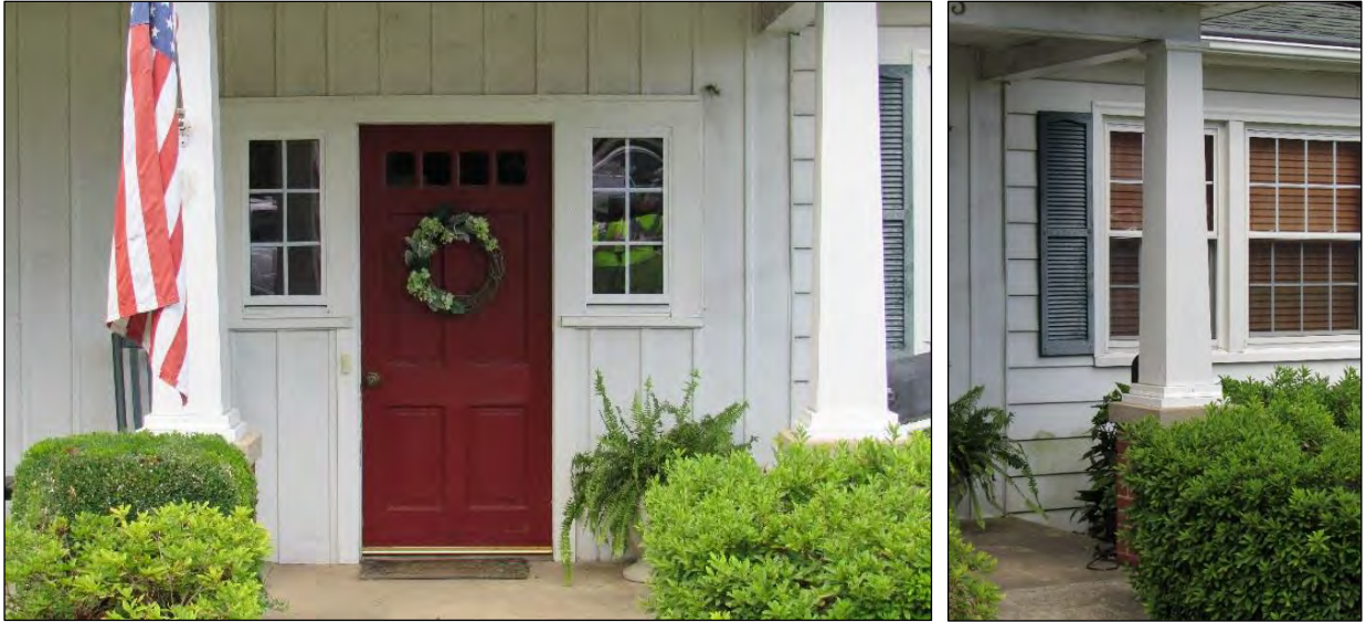
Photo 183: Primary Entrance (Left) and Column Detail (Right) on Façade.
