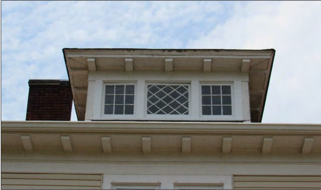
Photo 281: Detail of Dormer with Original Windows on East Elevation.
