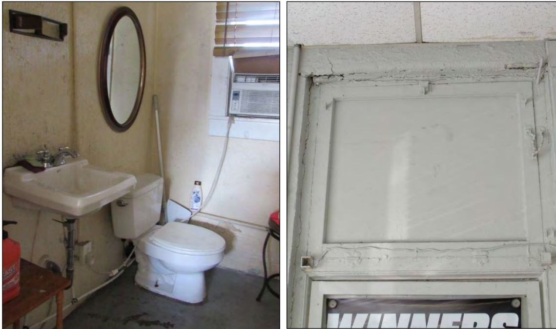
Photo 109: Detail of Private Restroom and Transom Above South Entry at Interior.
