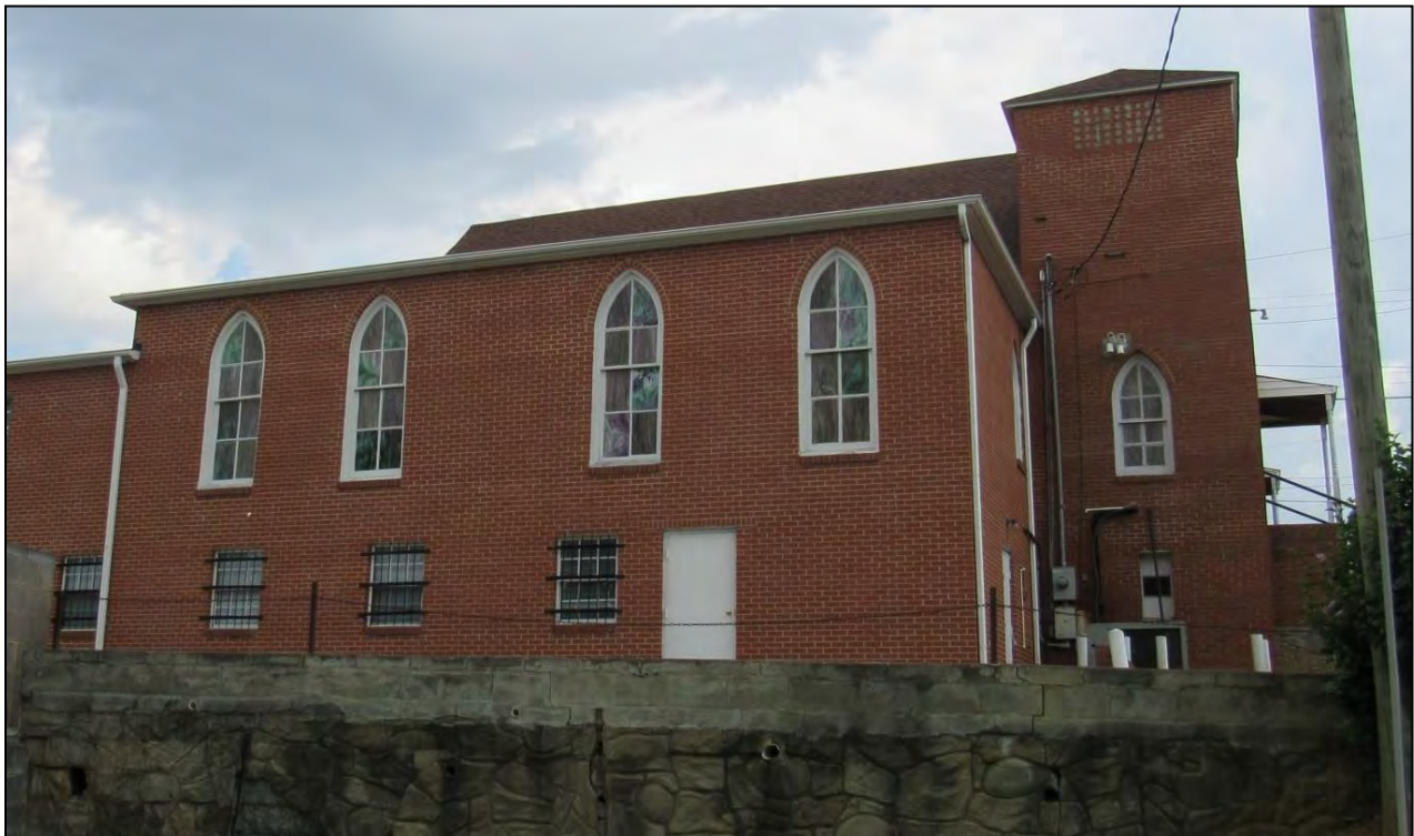
Photo 154: Circa-1985 Addition, Northwest Elevation.
