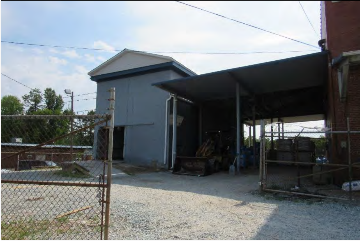
Photo 31: Southwest Oblique of Addition, Facing Northeast.
