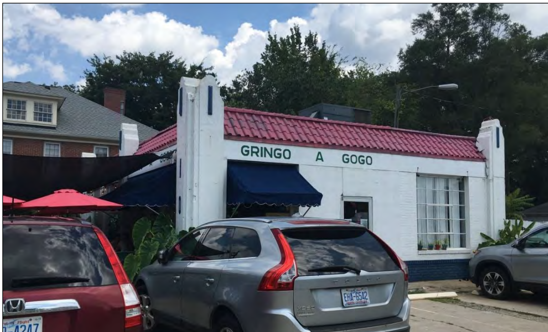
Photo 111: Current View of Former Blowes Esso Station Building, Looking Northeast.
