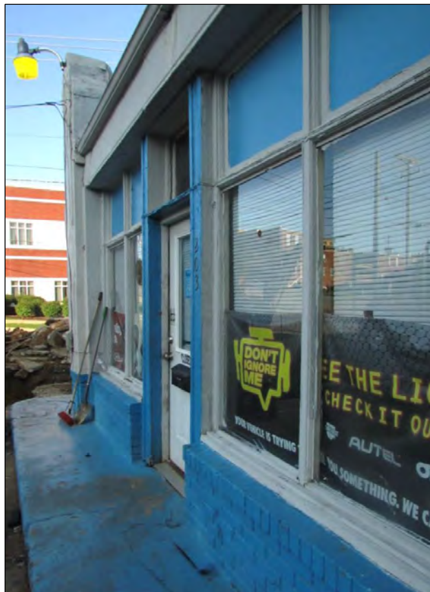
Photo 104: Detail of Storefront Looking South Along East Elevation.
