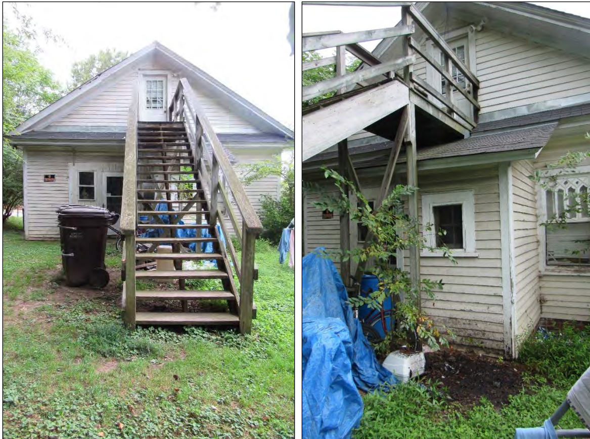
Photo 302: Rear (East) Elevation (Left) and Detail of Rear Addition (Right).
