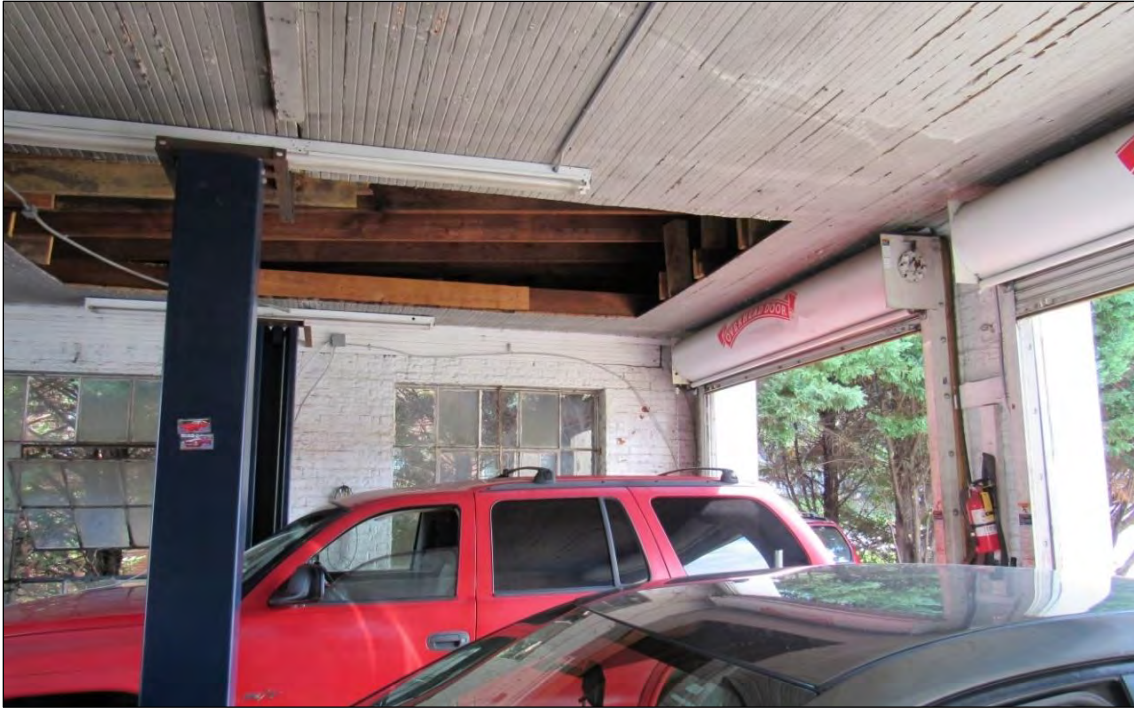
Photo 105: Interior View of Service Area, Looking North-Northeast.
