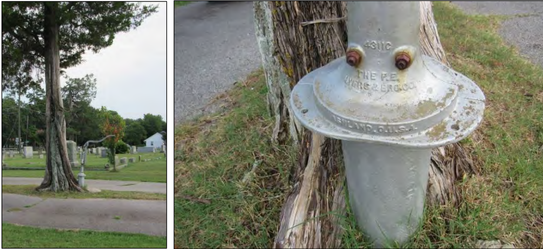
Photo 360: Water Pump, Looking Southeast.
