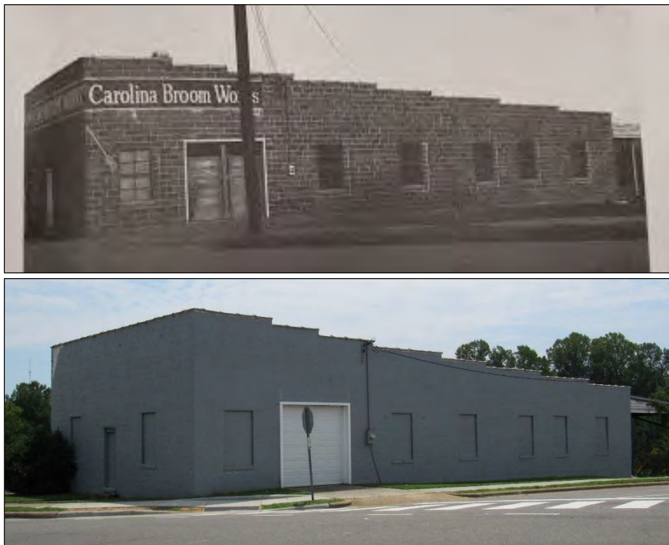
Photo 126: Historic Image of the Carolina Broom Works Building, West Elevation (Top) and Current View of Building, Northwest Oblique (Bottom). 291
