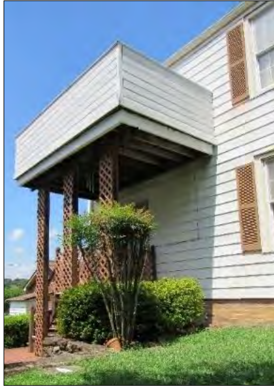
Photo 54: Detail of Deck on Southwest Elevation.
