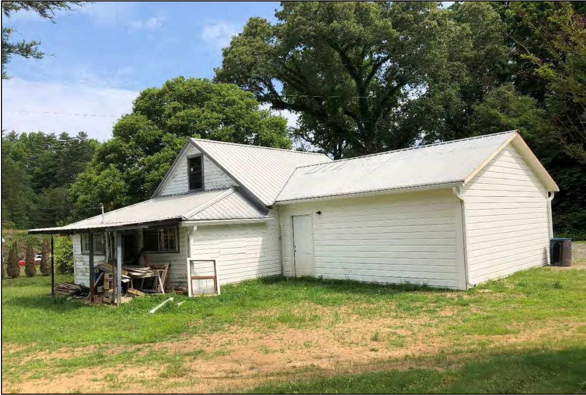
Figure 12. Architectural resource CE0246; view is north featuring the southwest (rear) elevation.
