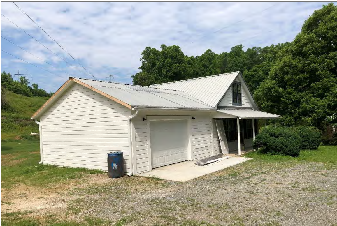
Figure 11. Architectural resource CE0246; view is west featuring the modern garage addition.
