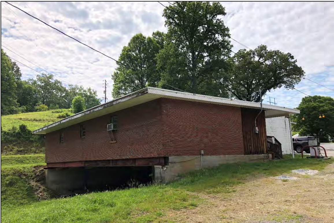
Figure 9. Architectural resource CE0245; view is southeast featuring the north (rear) addition.
