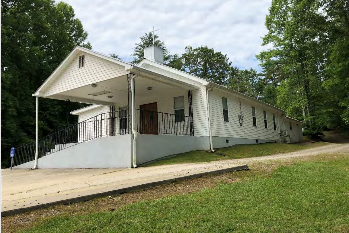
Figure 14. Architectural resource CE0247; view is southwest featuring the façade and northwest elevation.
