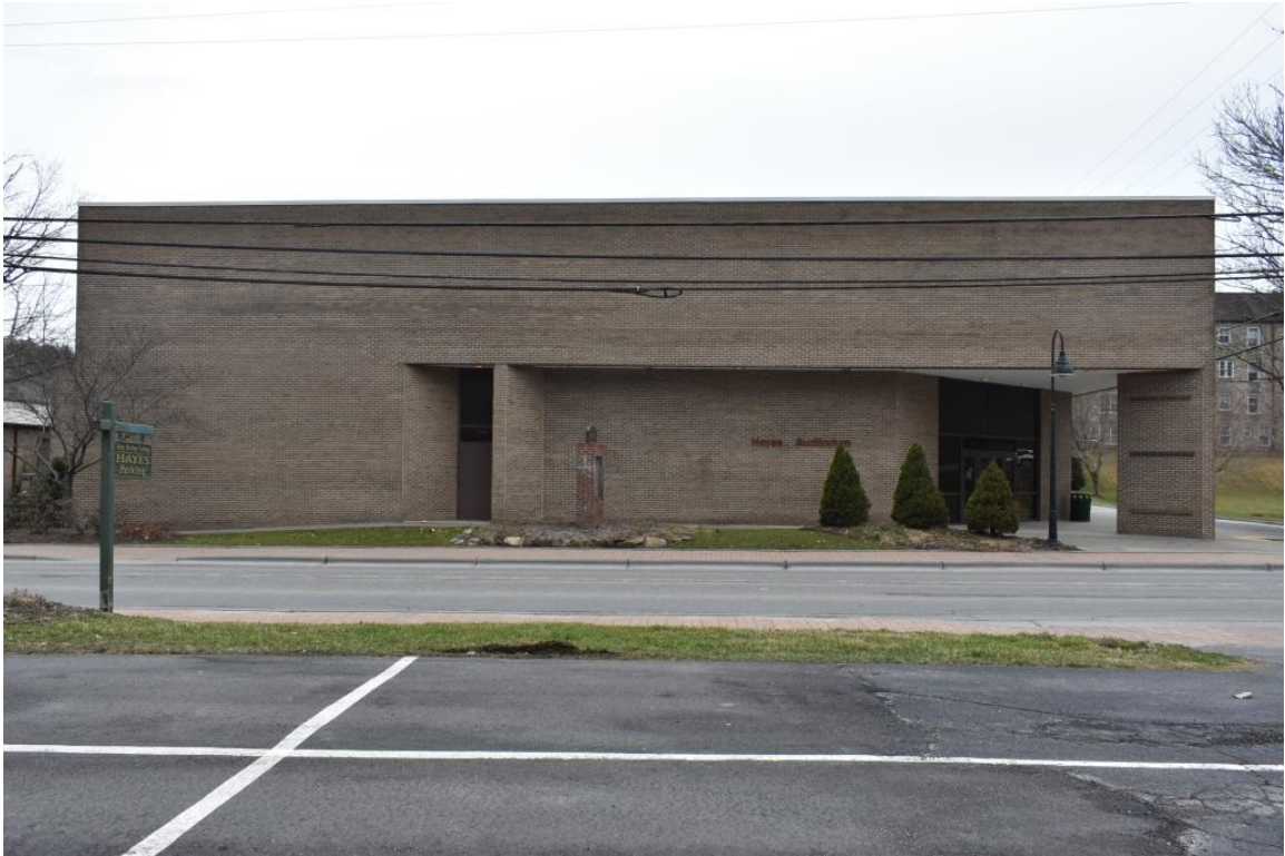
(#4) Hayes Auditorium (1975), façade, view to south
