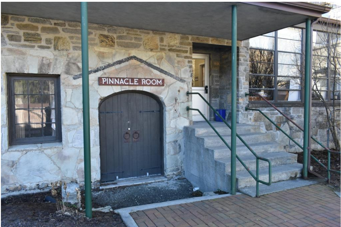
(#19) North Carolina Building Annex (1957), entrance, view to south
