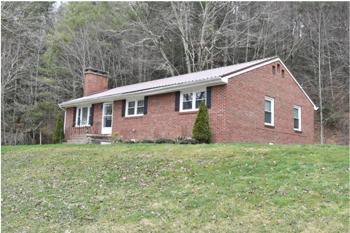
Staff Residence 5 (ca. 1963), 280 Bobcat Way, façade, oblique view to northwest
