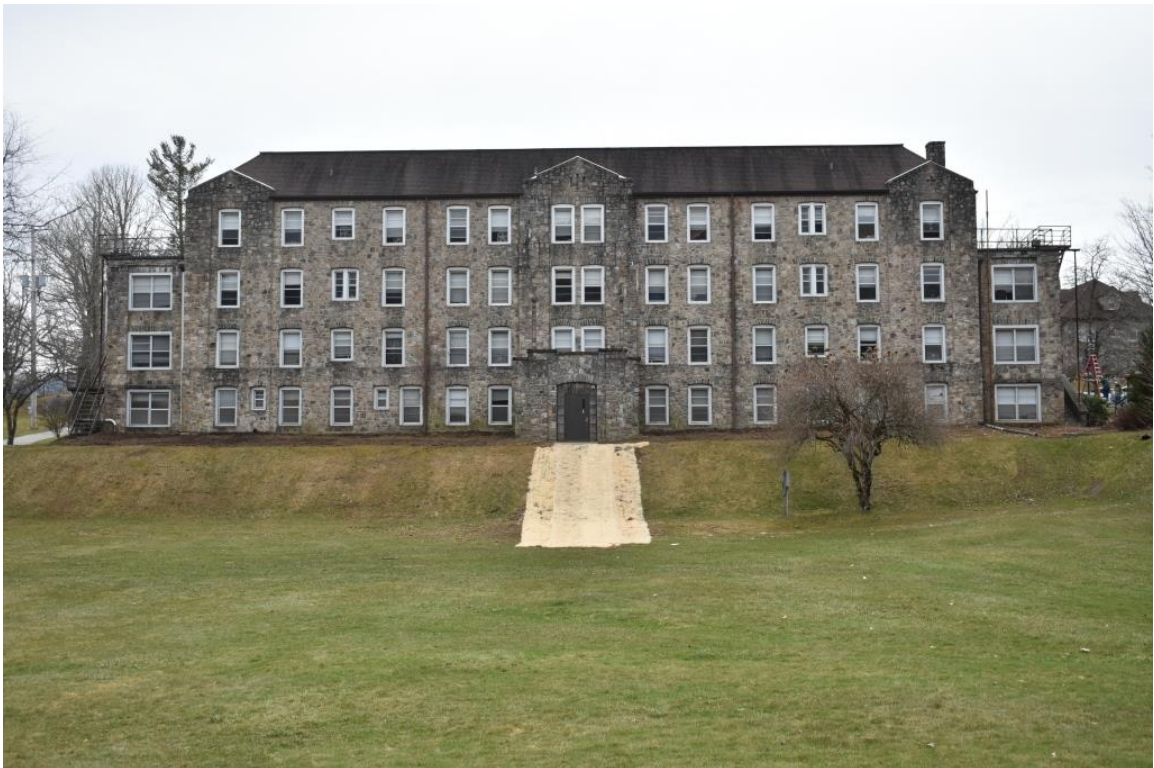
(#12) Tate Residence Hall (1932), façade, view to south
