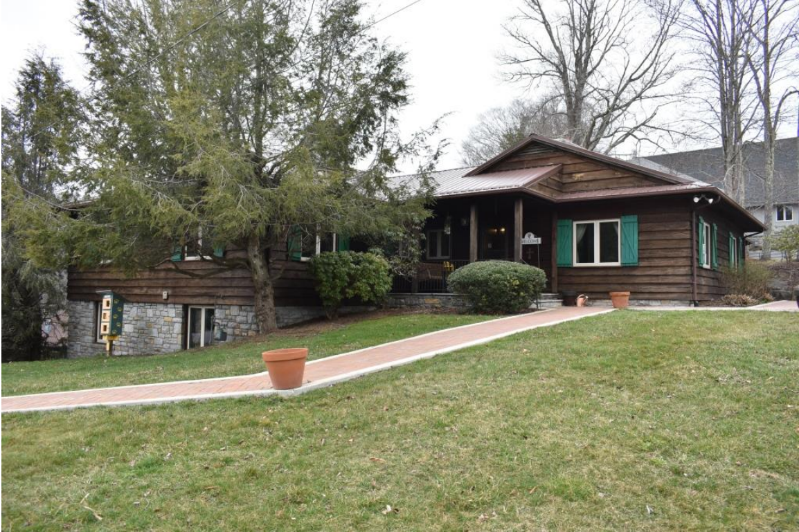
(#25) Needham Alumni House (ca. 1958), façade, view to west
