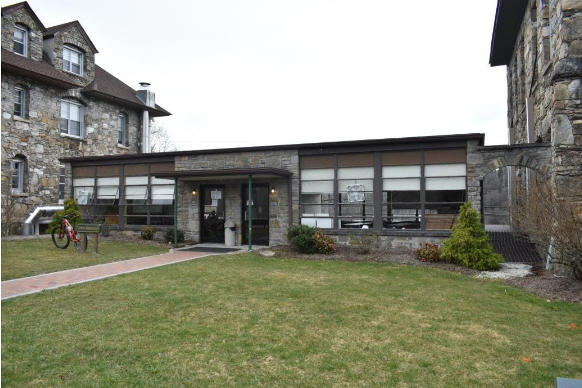
(#20) Cannon Classroom Building (1957), façade, view to south
