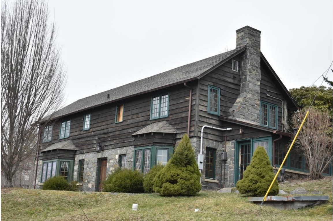
(#33) Daniel Boone VI Cottage (1935), rear elevation, view to northwest
