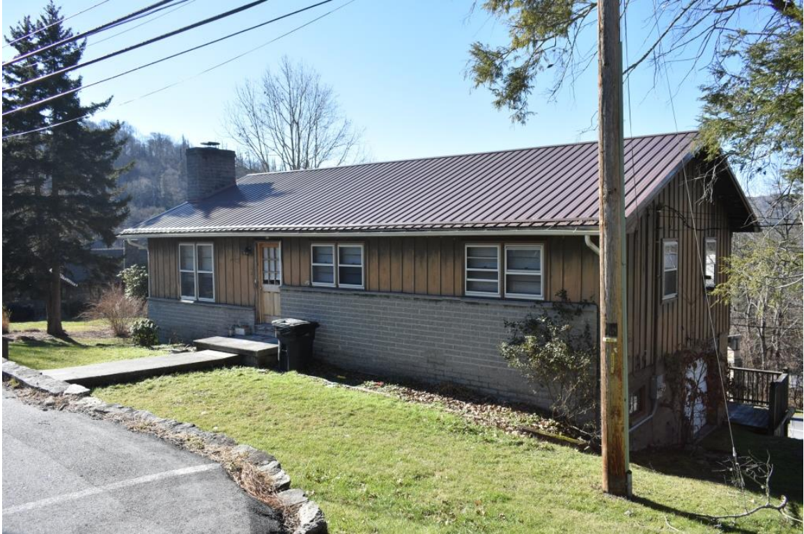
Student Residence House (ca. 1964), 168 Chestnut Way, oblique view to southwest
