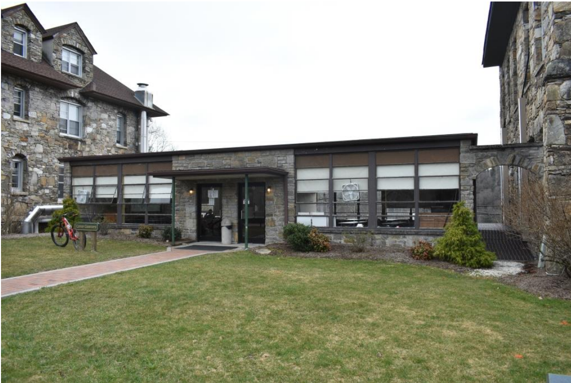
(#20) Cannon Classroom Building (1957), façade, view to south
