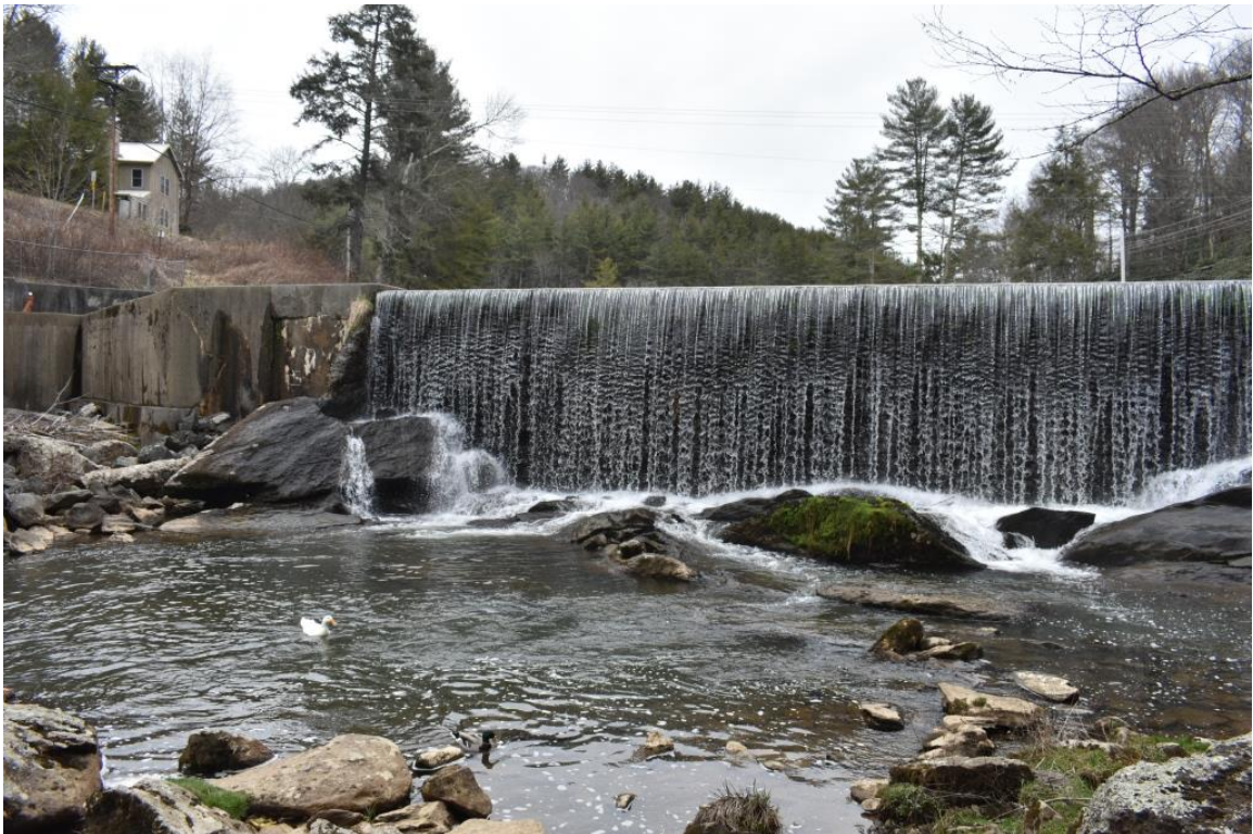
Elk River Dam (ca. 1912), view to southeast
