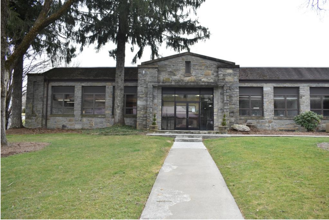
(#13) Chaffee Administration Building (1955), façade, view to south
