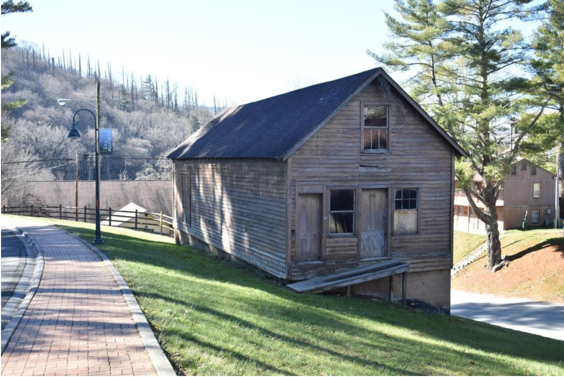
(#28) Carriage House (ca. 1890s), oblique view to southwest
