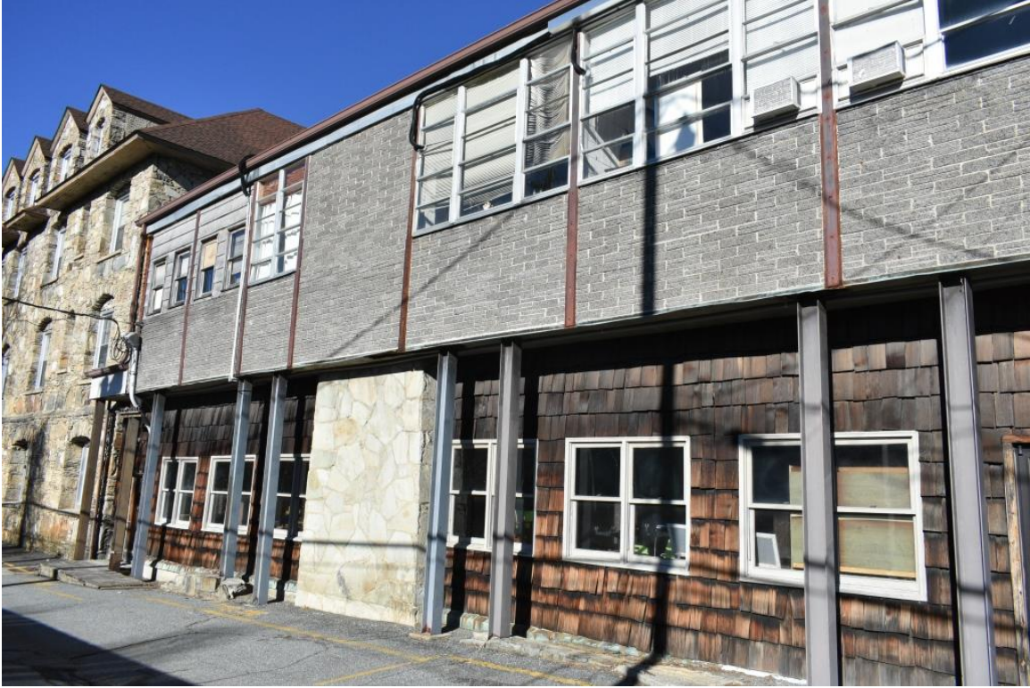
(#19) North Carolina Building Annex (1932 and 1957), rear elevation, view to northwest
