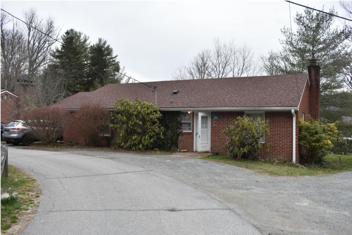
Student Residence 5 (ca. 1963), 306 Bobcat Way, rear elevation, view to southeast
