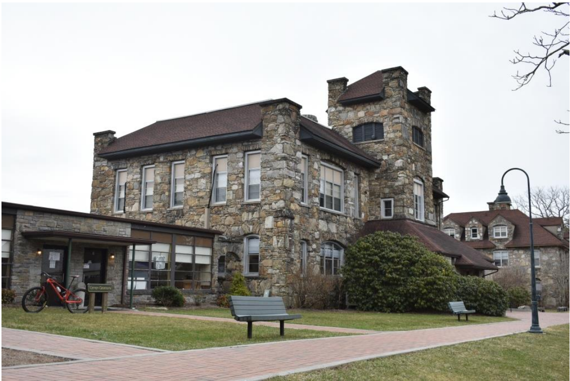
(#19) North Carolina Building (1923), oblique view to southwest
