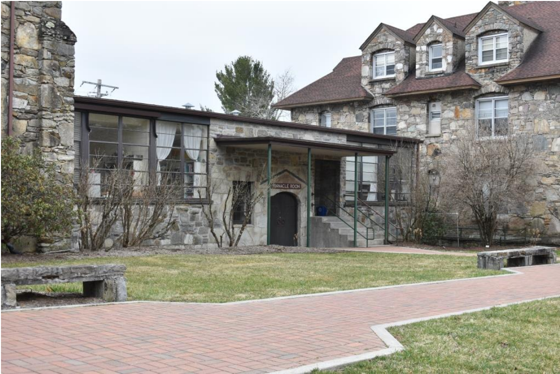
(#19) North Carolina Building Annex (1957), oblique view to southwest
