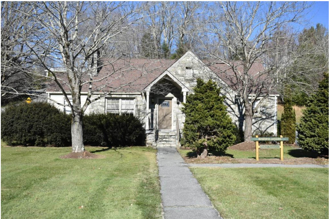
(#13) Business Affairs Office (ca. 1948), façade, view to north
