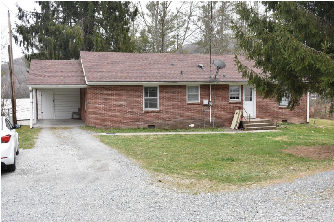
Student Residence 6 (ca. 1963), 300 Bobcat Way, rear elevation, view to south
