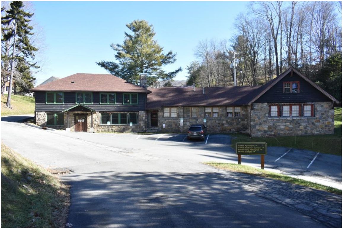
(#27) Whitesell Art Building and Costume Shop (ca. 1943), façade, view to east
