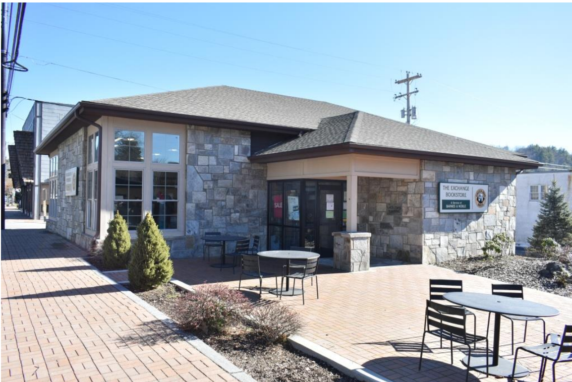
(#7) The Exchange Bookstore (Lauritsen Building) (ca. 1964), oblique view to southeast
