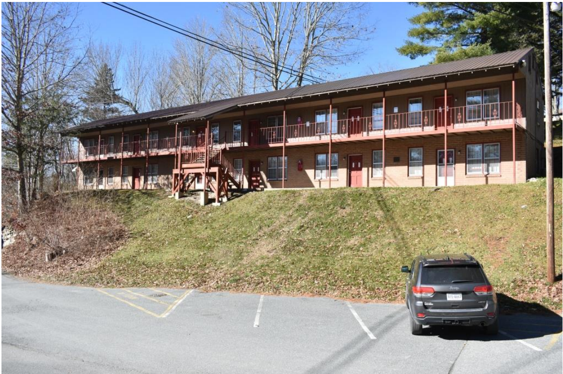
(#36) Student Apartments (ca. 1965), façade, view to northwest
