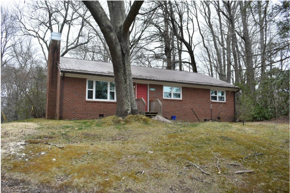
Staff Residence 4 (ca. 1963), 160 Bobcat Way, façade, view to north
