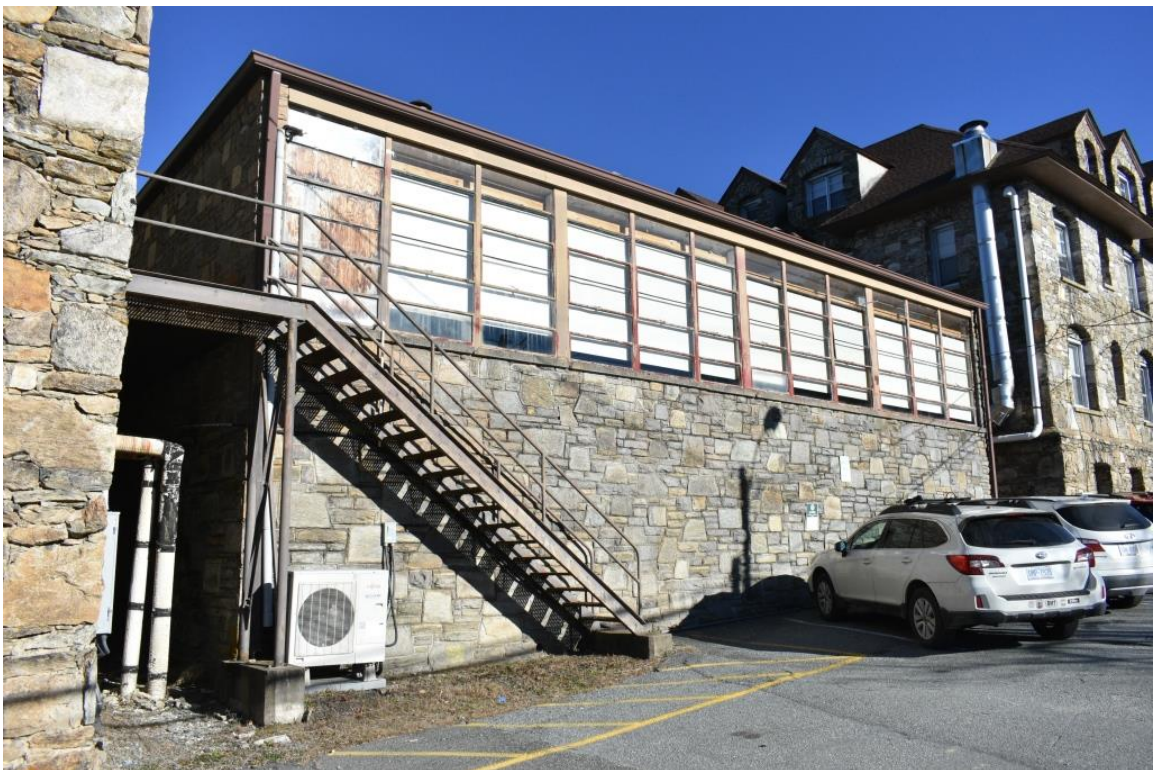
(#20) Cannon Classroom Building (1957), rear elevation, view to northeast
