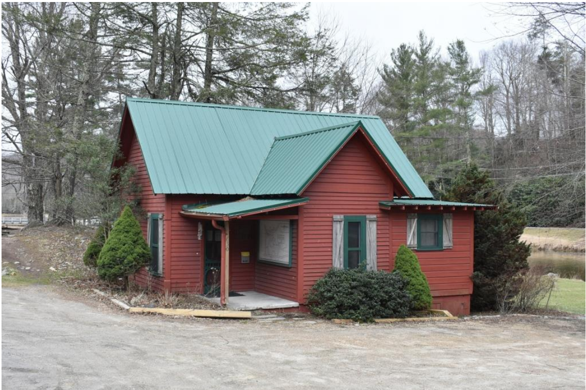
(#40) Historic Cheese House (ca. 1917), oblique view to south
