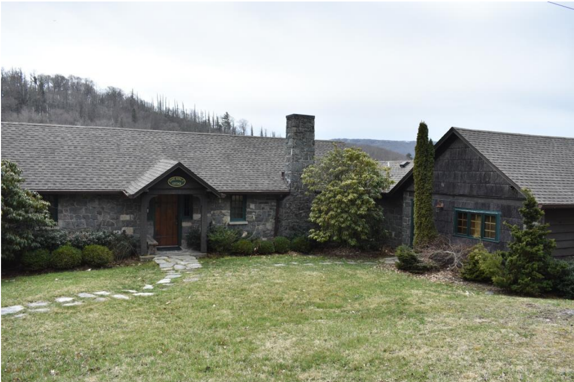
(#33) Daniel Boone VI Cottage (1935), façade, view to southwest
