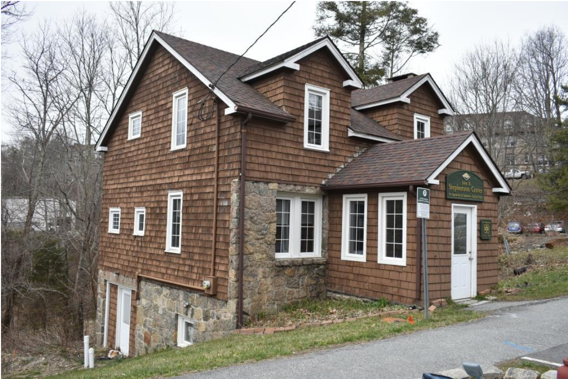
(#32) Stephenson Center for Appalachian Studies (ca. 1934), oblique view to northwest
