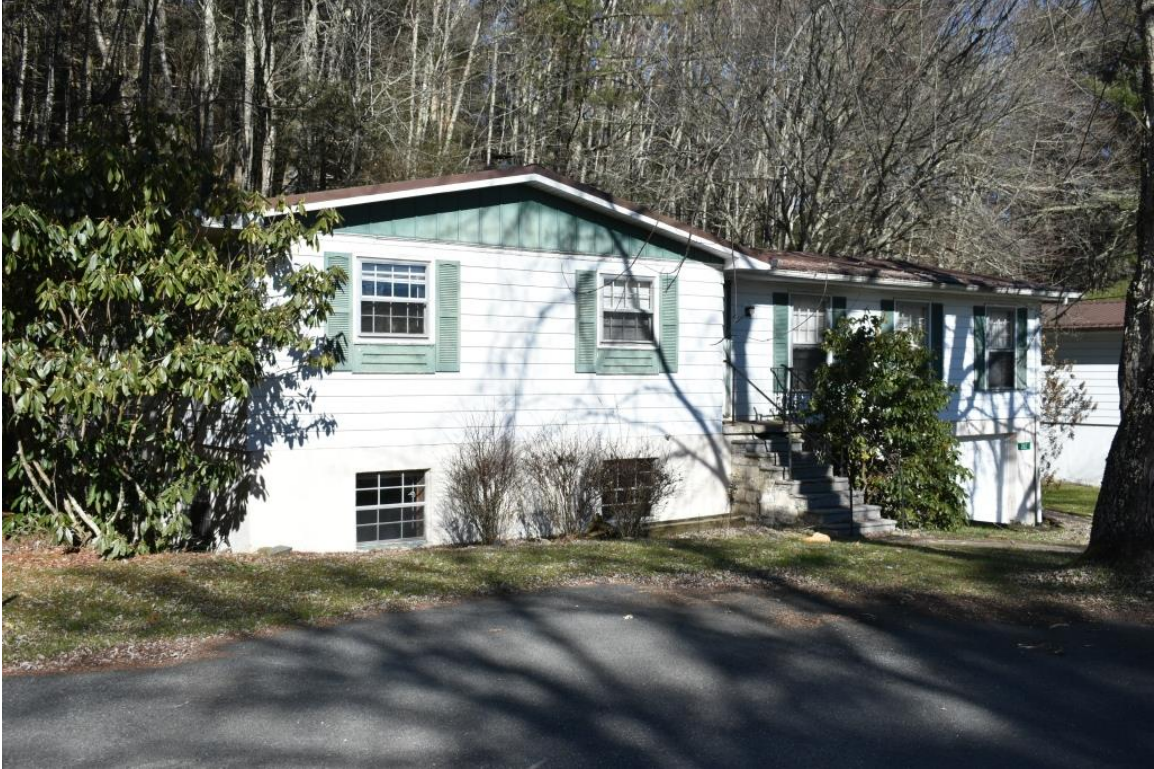
Student Residence 8 (ca. 1969), 262 Bobcat Way, oblique view to north
