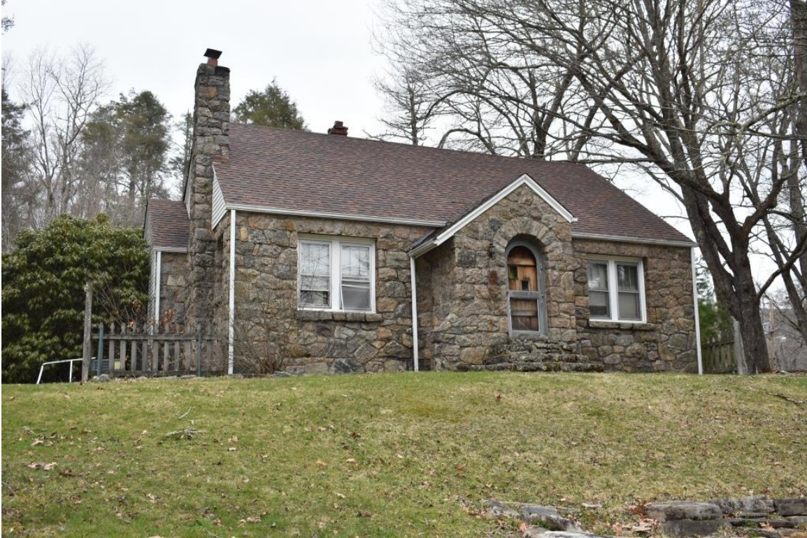
Athletic Offices (ca. 1938), 225 Bobcat Way, façade, view to north
