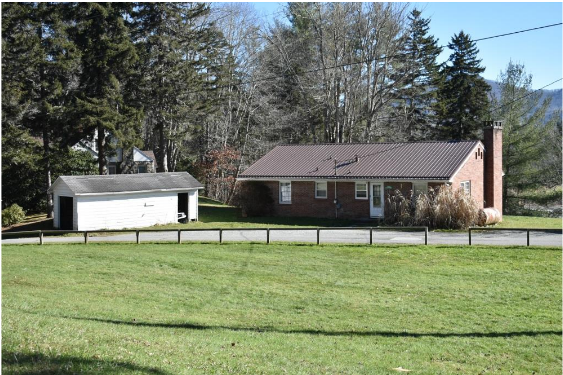
Student Residence 4 and Garage (ca. 1963), 320 Bobcat Way, rear elevation, view to southeast
