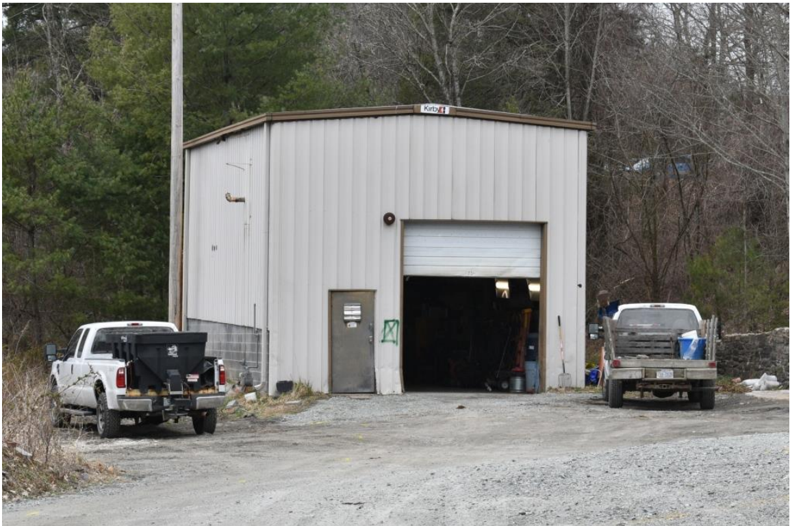
Physical Plant Operations Building (ca. 1992), view to west
