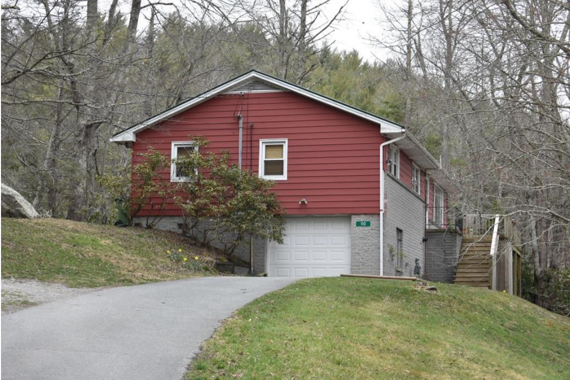
Staff Residence 1 (ca. 1961), 110 Bobcat Way, oblique view to east
