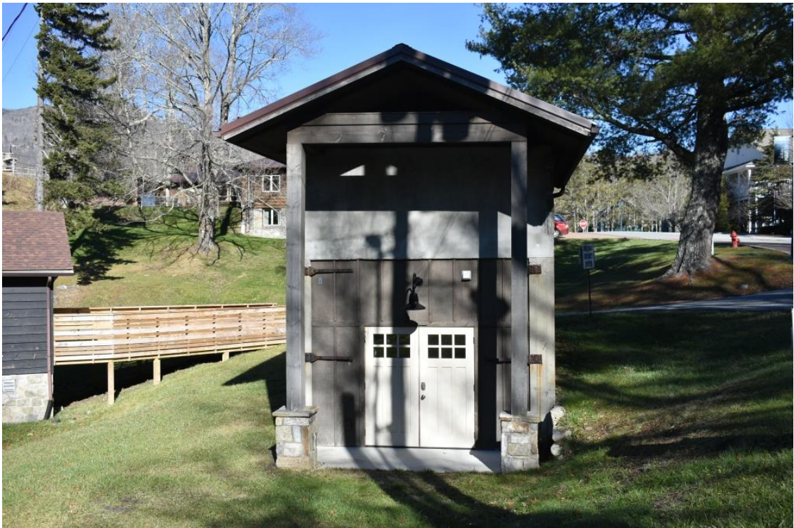
(#26) Kiln Building (ca. 1943), façade, view to north
