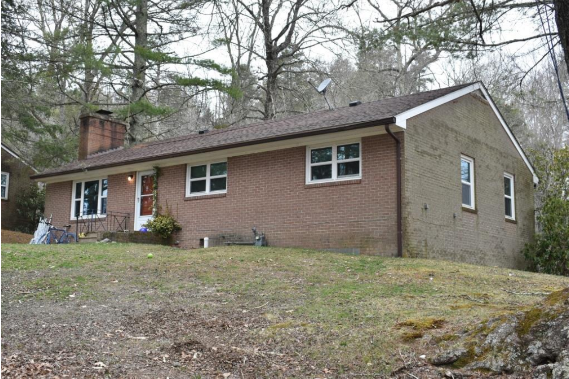
Student Residence 2 (ca. 1963), 193 Bobcat Way, façade, oblique view to northwest
