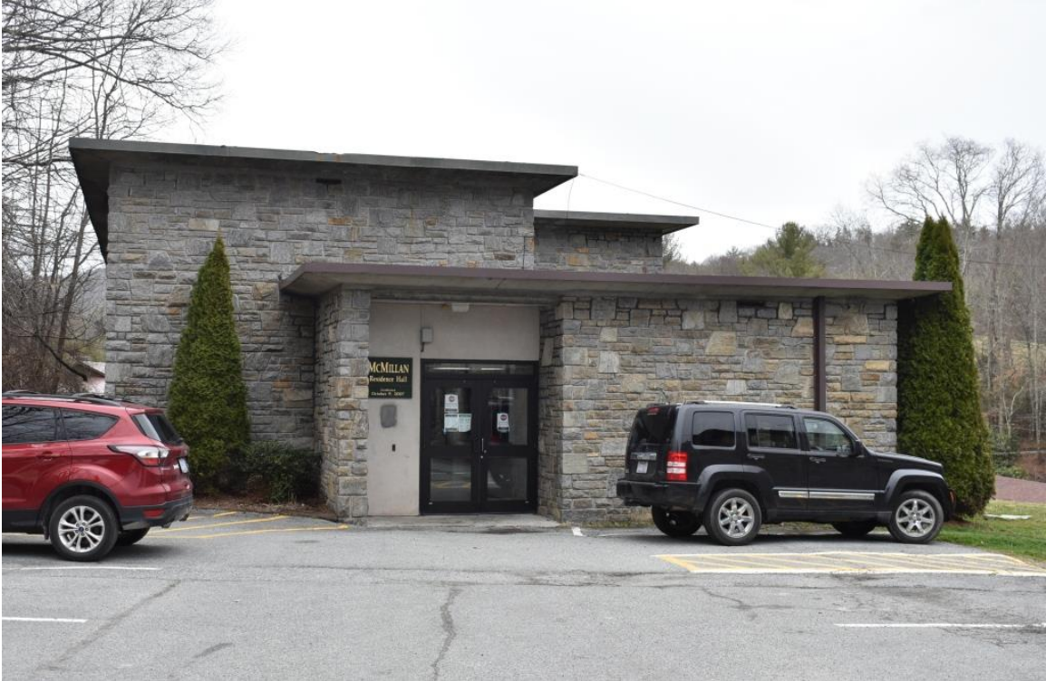
(#29) McMillan Residence Hall (1959), faced, view to east
