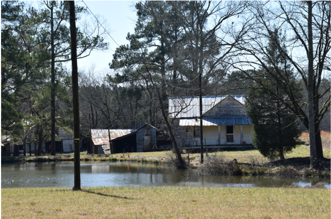
Outbuildings and tenant house, Goodwin Farm Complex, view south
