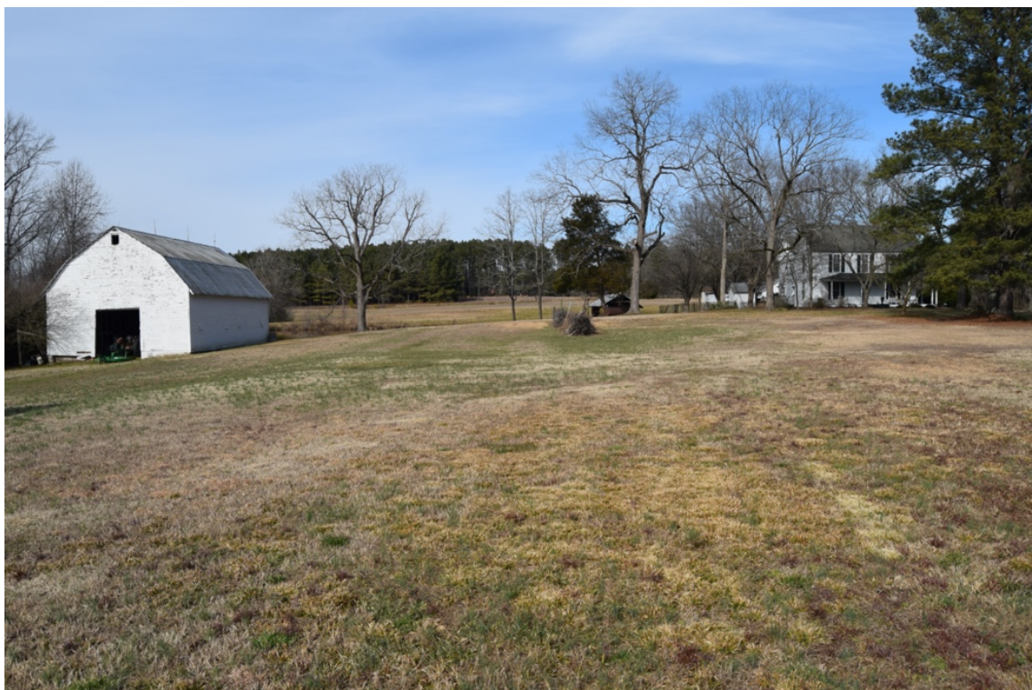
H. T. Lawrence farm, barn and dwelling as they appear on the approach from the main roadway, view north
