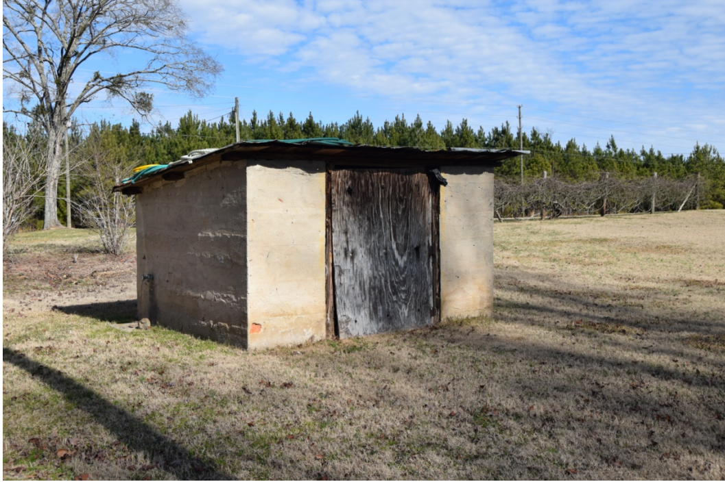
New well, Bartley Yates Farm, view to northeast.
