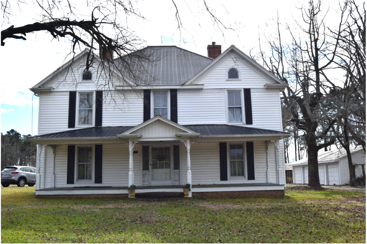
Dwelling, Bartley Yates Farm, façade (N elevation), view to south.
