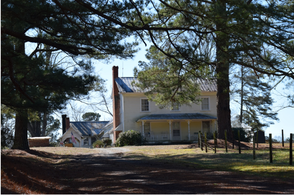
Outbuildings and Dwelling, Goodwin Farm Complex, view south
