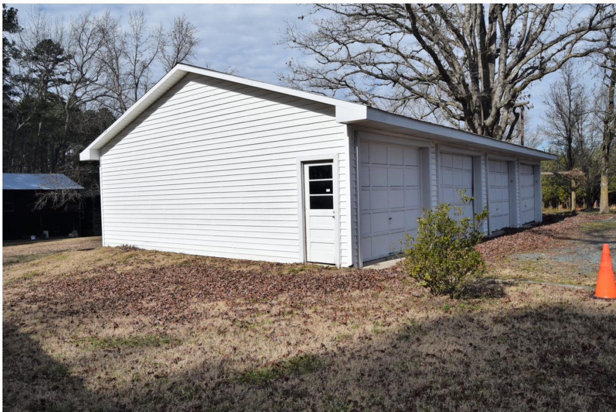
Garage, Bartley Yates Farm, view to northwest.
