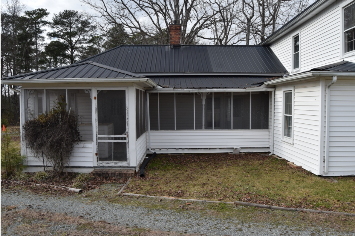
Dwelling, Bartley Yates Farm, enclosed well at S end of E screened porch, view to west.
