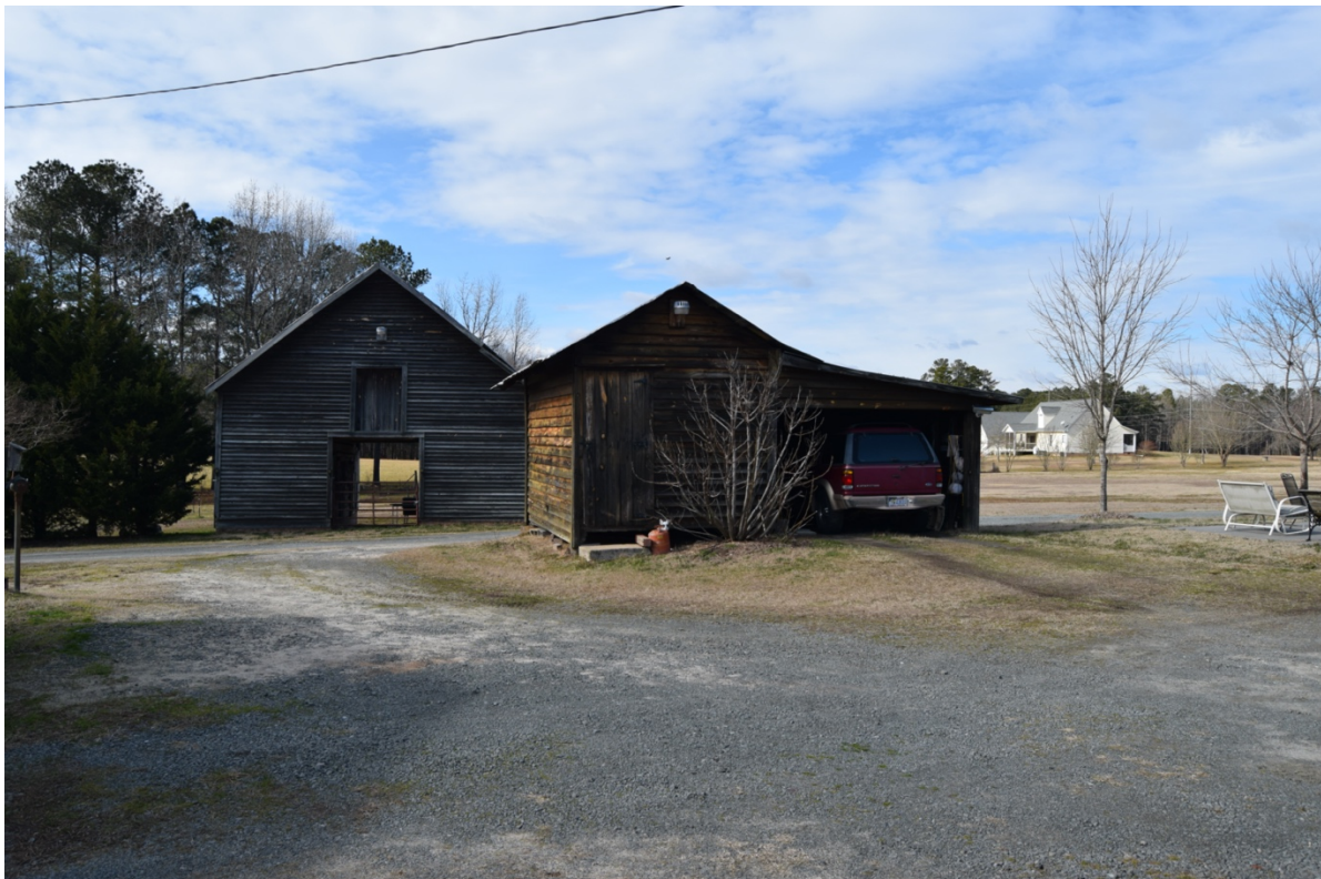
Mule barn and corn crib, Cannady-Brogden Farm, view northeast
