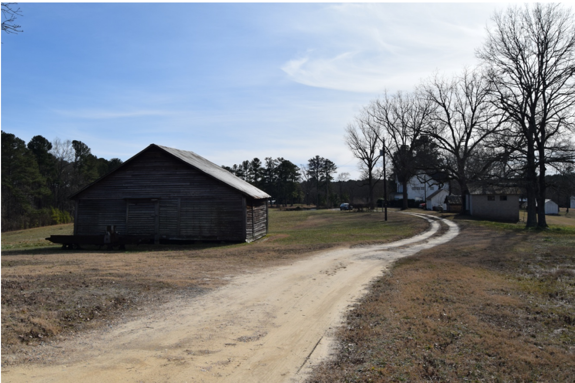
Packhouse on farm lane north of dwelling and outbuildings, H. T. Lawrence farm, view south
