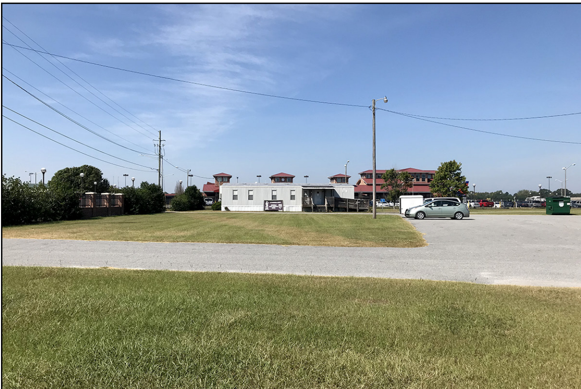
PLATE 38: Modular Support Building, East Elevation, Greenville National Guard Armory (PT3357), Pitt County, North Carolina
