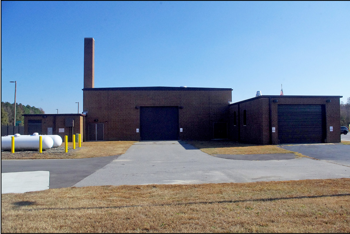
PLATE 48: West Elevation, Nashville National Guard Armory (NS1563), Nash County, North Carolina
