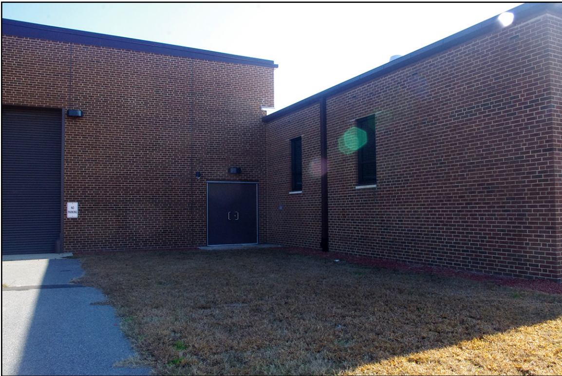
PLATE 49: Detail of North Elevation of Former Rifle Range Wing on West Elevation, Nashville National Guard Armory (NS1563), Nash County, North Carolina
