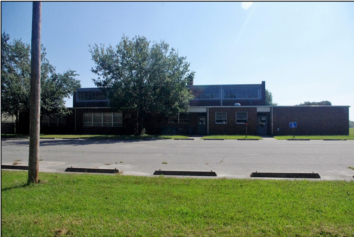
PLATE 15: West Elevation, Fremont National Guard Armory (WY1458), Wayne County, North Carolina
