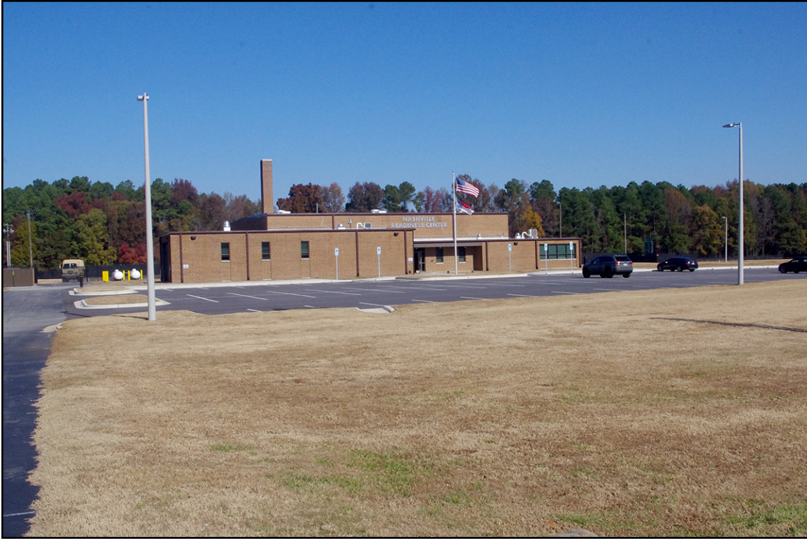
PLATE 41: Nashville National Guard Armory (NS1563) Property, Facing Northeast from Entrance on Eastern Avenue, Nash County, North Carolina
