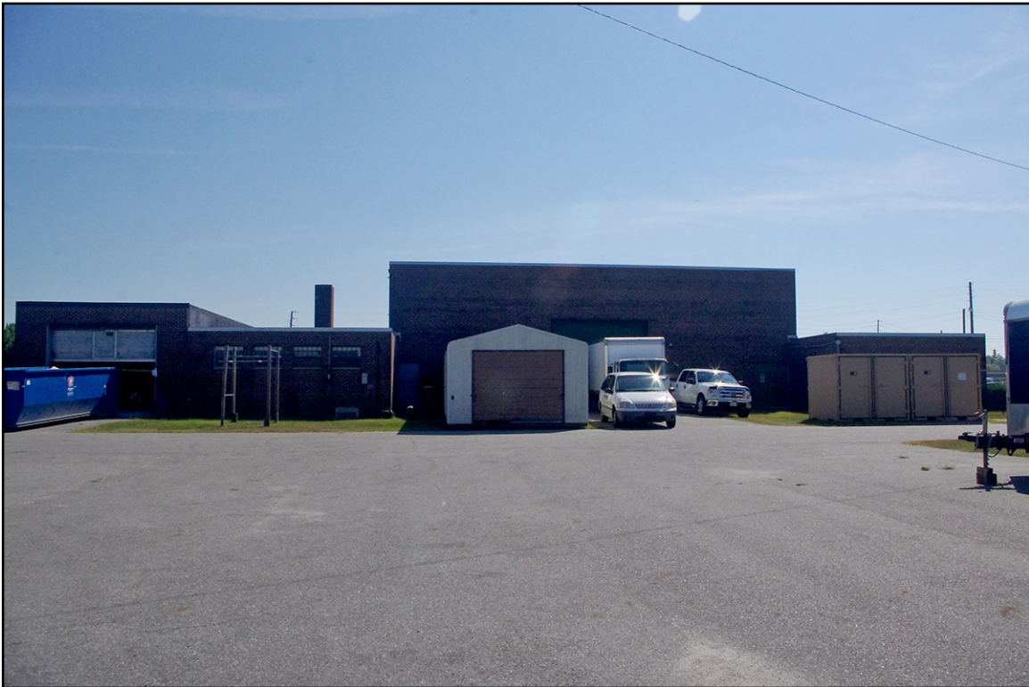
PLATE 30: West Elevation, Greenville National Guard Armory (PT3357), Pitt County, North Carolina
