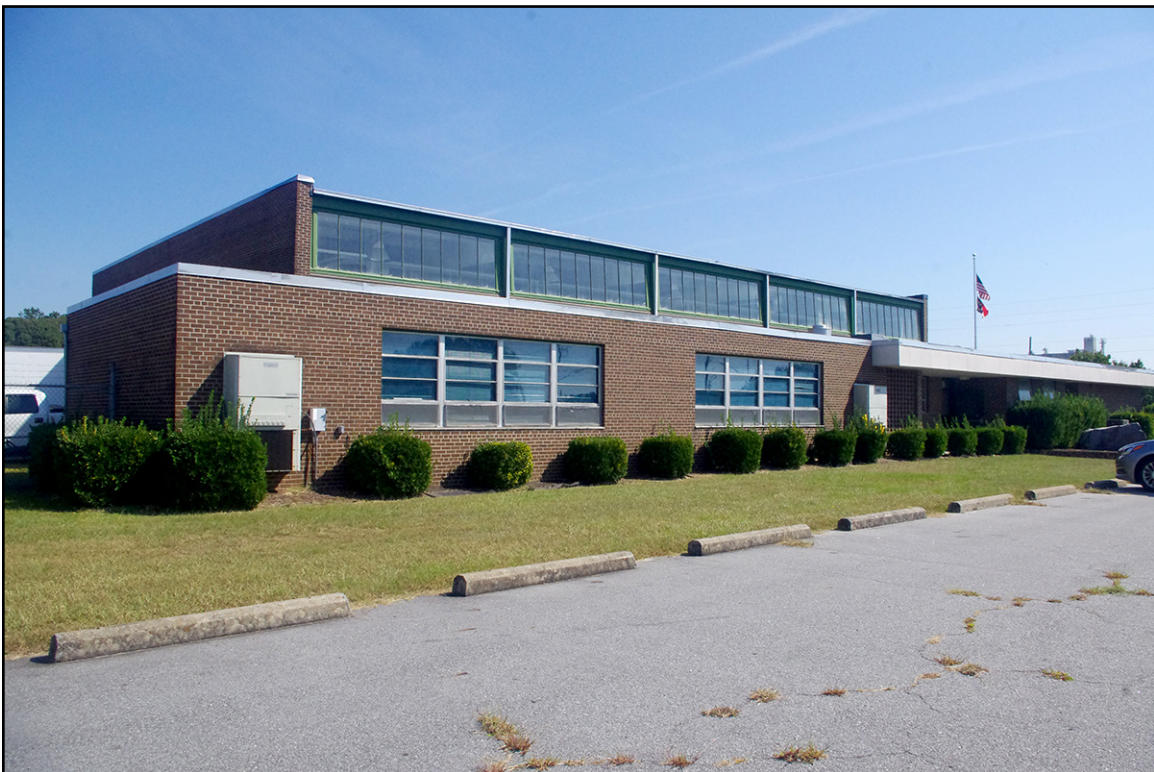
PLATE 40: Oblique View of South Elevation, Greenville National Guard Armory (PT3357), Pitt County, North Carolina
