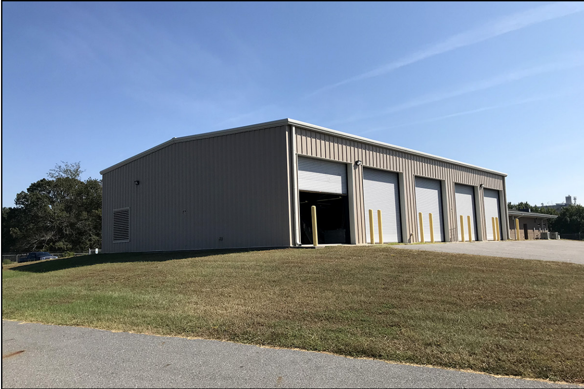
PLATE 37: Maintenance Bay/Garage, South Elevation, Greenville National Guard Armory (PT3357), Pitt County, North Carolina
