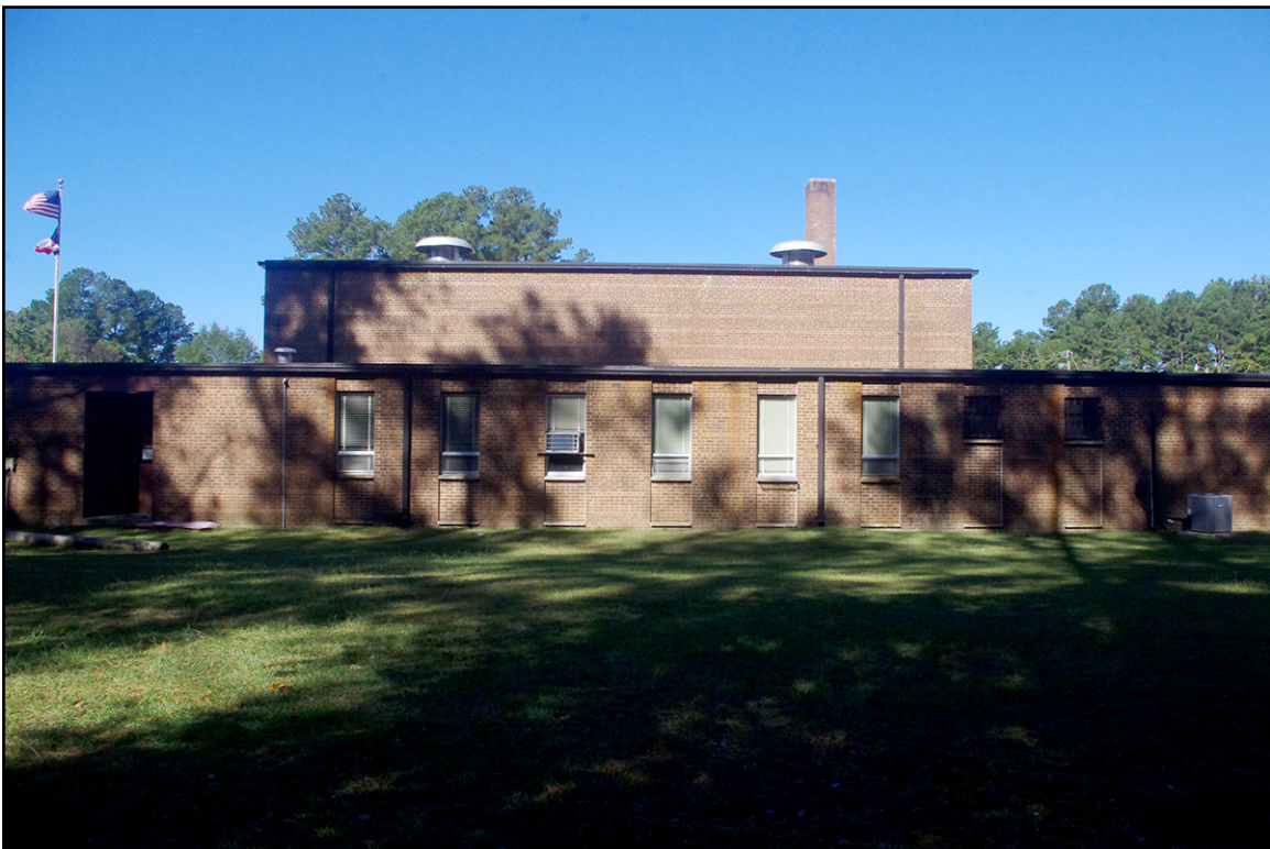
PLATE 61: East Elevation, Roseboro National Guard Armory (SP0769), Sampson County, North Carolina
