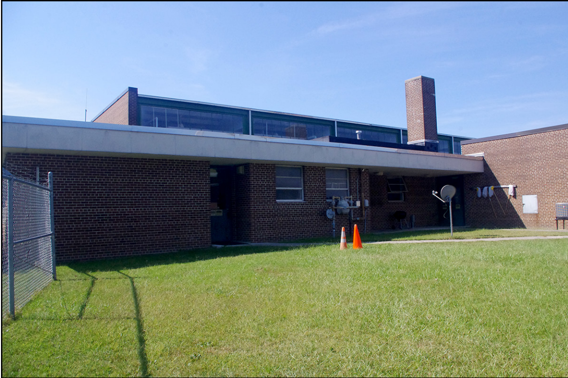
PLATE 31: North Elevation, Greenville National Guard Armory (PT3357), Pitt County, North Carolina
