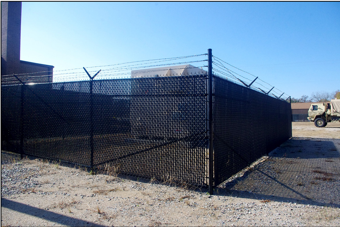
PLATE 42: Modular/Temporary Magazine, Oblique View of North and East Elevations, Nashville National Guard Armory (NS1563), Nash County, North Carolina
