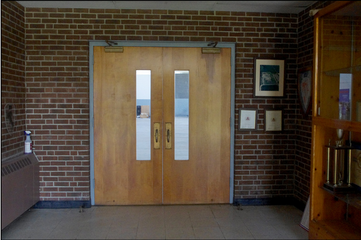
PLATE 23: Interior of Entry Leading to Drill Hall, Facing North, Fremont National Guard Armory (WY1458), Wayne County, North Carolina
