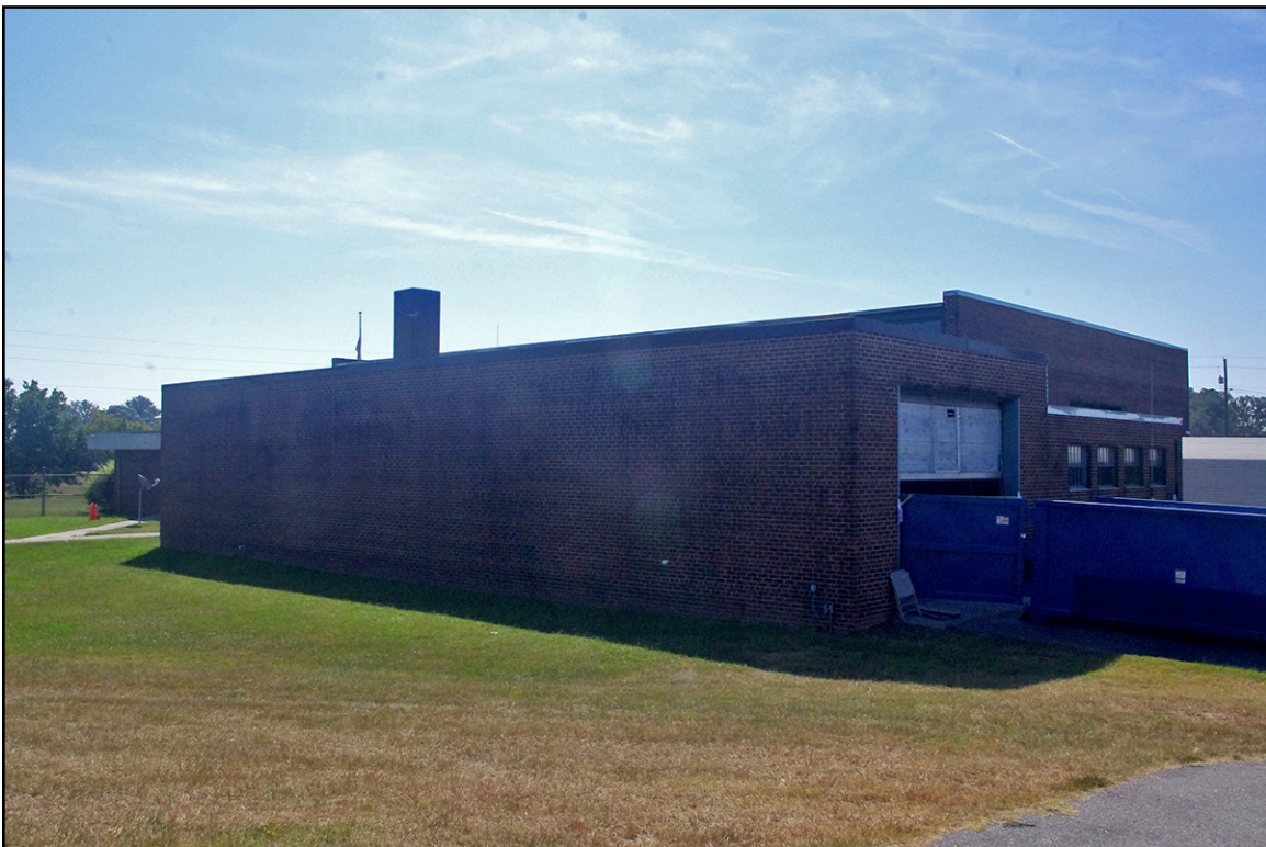
PLATE 32: Oblique View of North Elevation, Greenville National Guard Armory (PT3357), Pitt County, North Carolina
