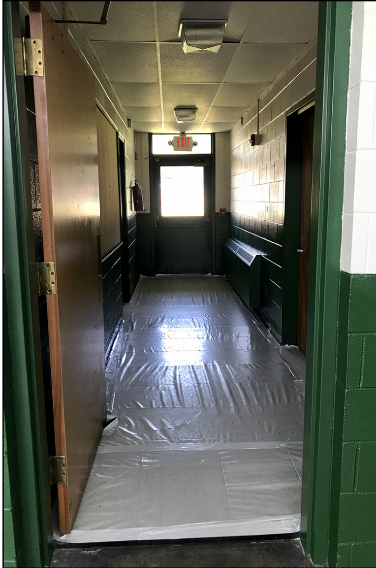
PLATE 34: Interior Corridor of Greenville National Guard Armory (PT3357), Facing North, Pitt County, North Carolina
