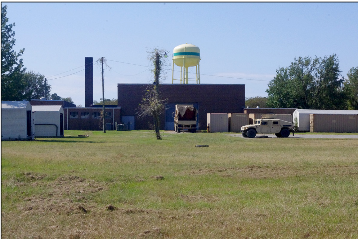
PLATE 18: North Elevation, Fremont National Guard Armory (WY1458), Wayne County, North Carolina
