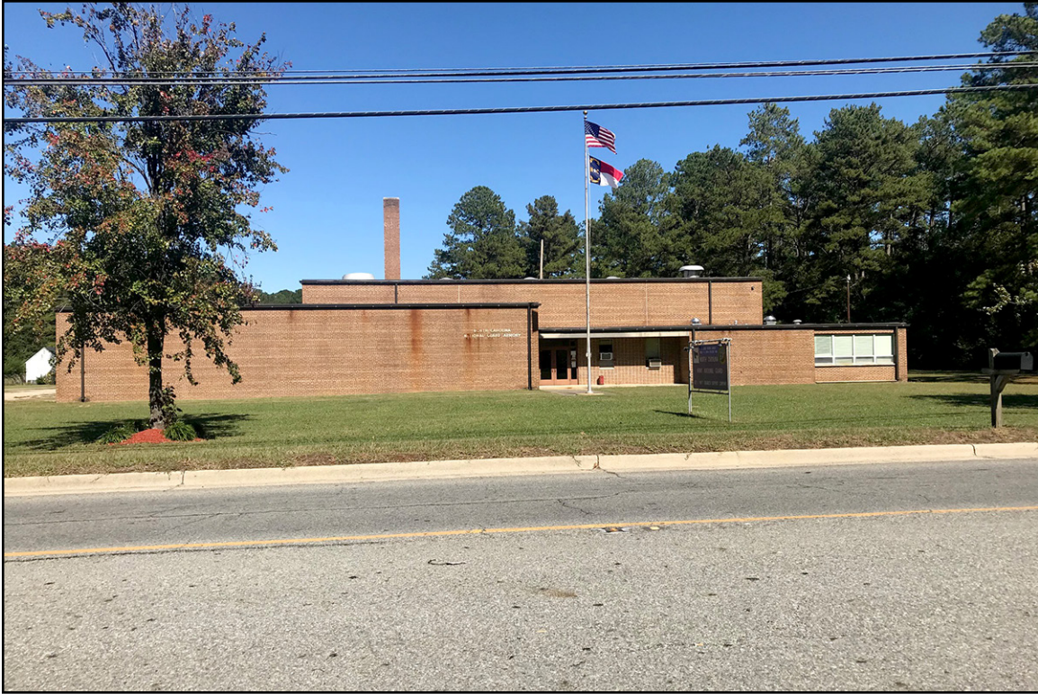
PLATE 60: South Elevation, Roseboro National Guard Armory (SP0769), Sampson County, North Carolina
