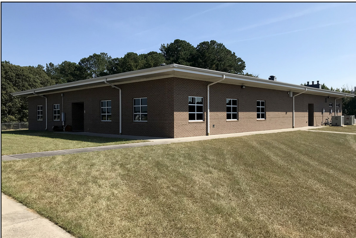
PLATE 36: Support Building, Oblique View of South and West Elevations, Greenville National Guard Armory (PT3357), Pitt County, North Carolina
