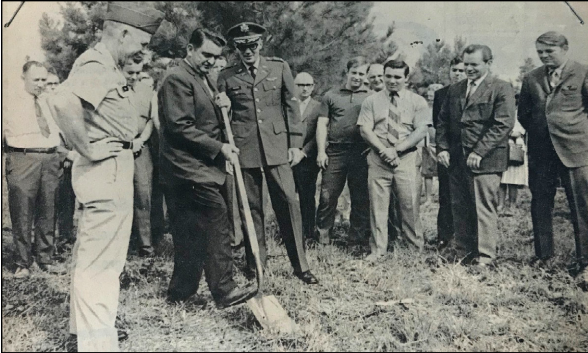
PLATE 73: Newspaper Clipping of Groundbreaking for Roseboro Armory ( The Sampsonian , 1970)
