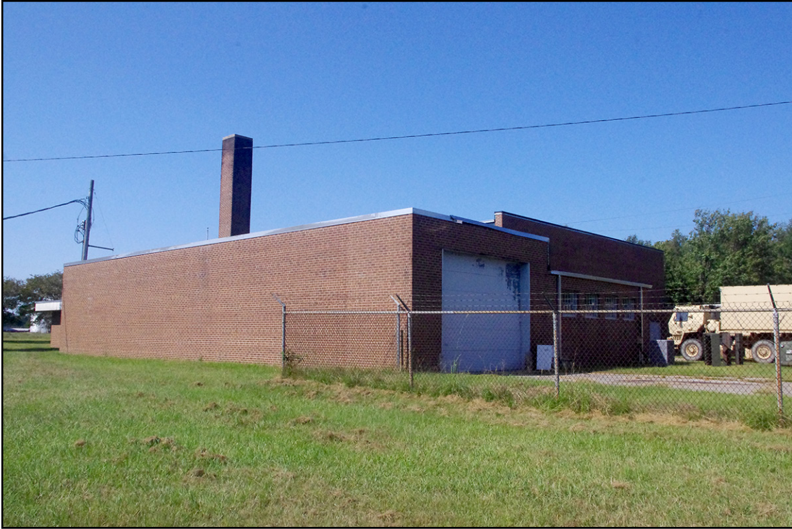
PLATE 17: Oblique View of North Elevation, Northeastern Corner Detail, Fremont National Guard Armory (WY1458), Wayne County, North Carolina
