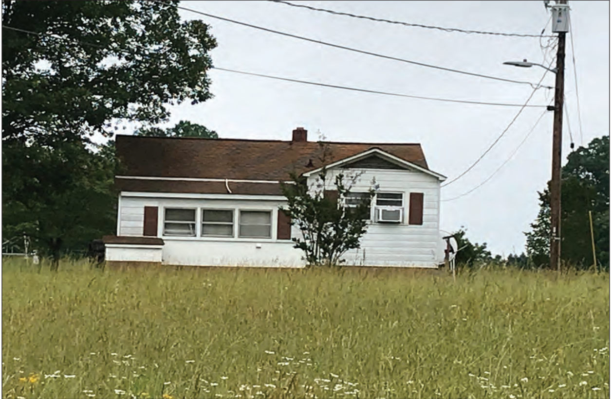
Figure 4.32 Resource BK0804 and pump house, west rear elevation.
