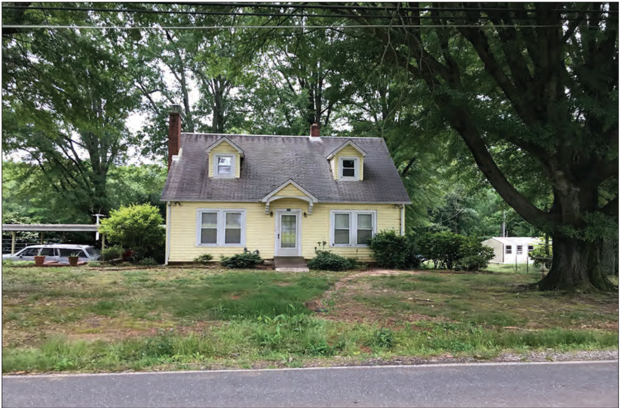
Figure 4.9 Minimal Traditional/Cape Cod Cottage in the project area on Cape Hickory Road, east front elevation.
