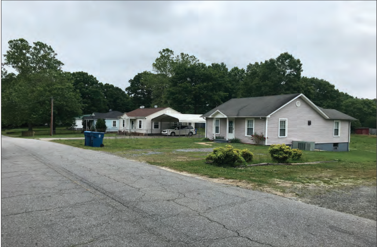
Figure 4.20 District streetscape with bungalows and Minimal Traditional houses on 40th Street NW, looking southwest.
