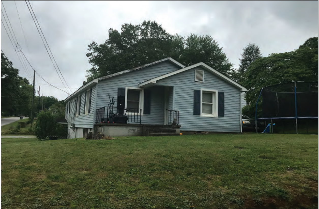
Figure 4.3 Bungalow in the project area on 38th Street NW, northwest oblique.
