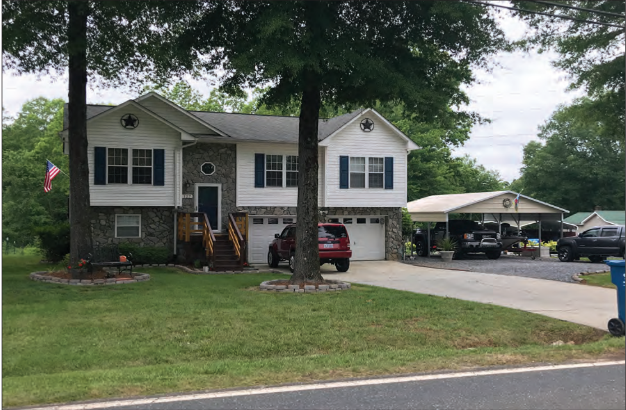
Figure 4.22 Non-historic infill house on Cape Hickory Road, east front elevation.
