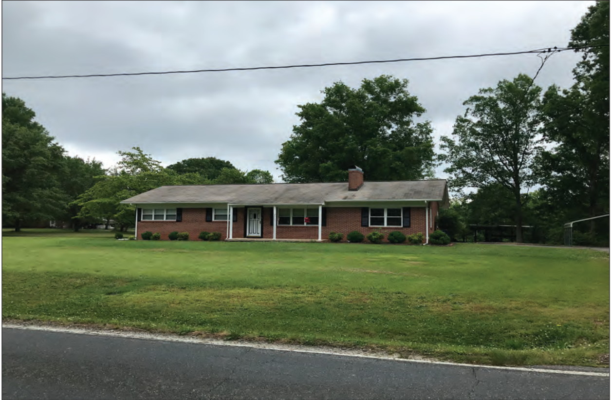
Figure 4.12 Side-gable Ranch house in the project area on Cape Hickory Road, west front elevation.
