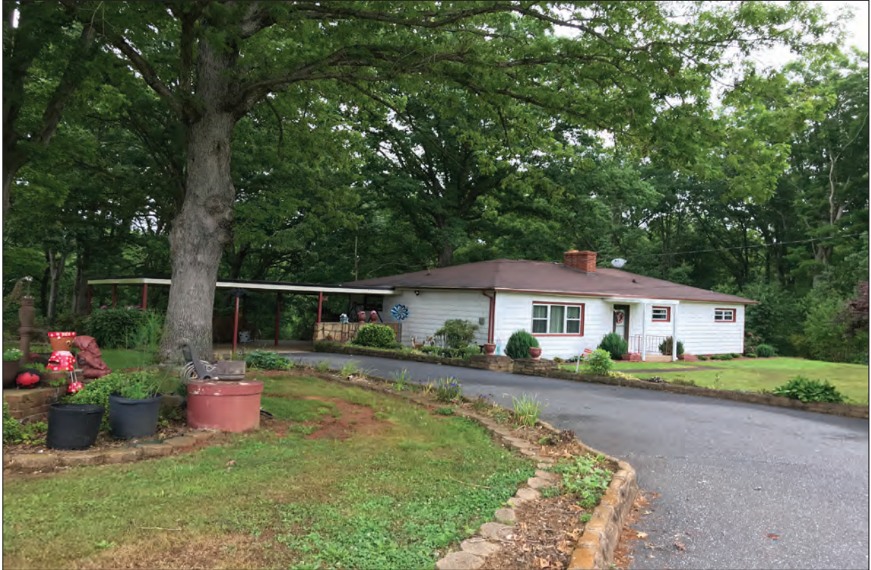
Figure 4.29 Resource BK0803, carport addition, southwest oblique.
