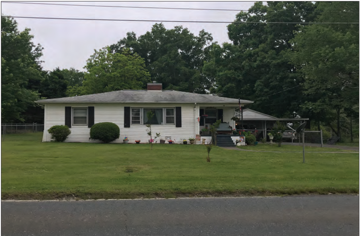
Figure 4.14 Hip-roof Ranch house in the project viewed on Cape Hickory Road, east front elevation.
