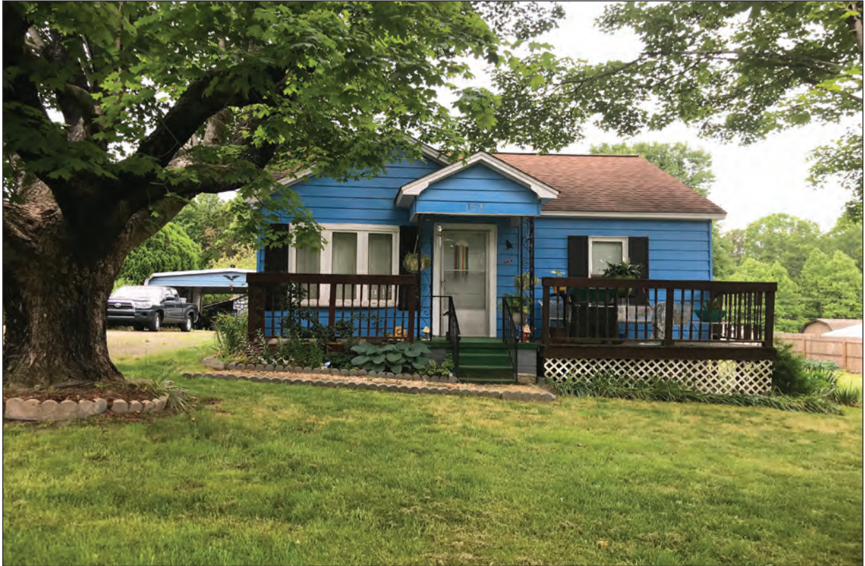
Figure 4.11 Minimal Traditional house in the project area on 38th Street NW, east front elevation.
