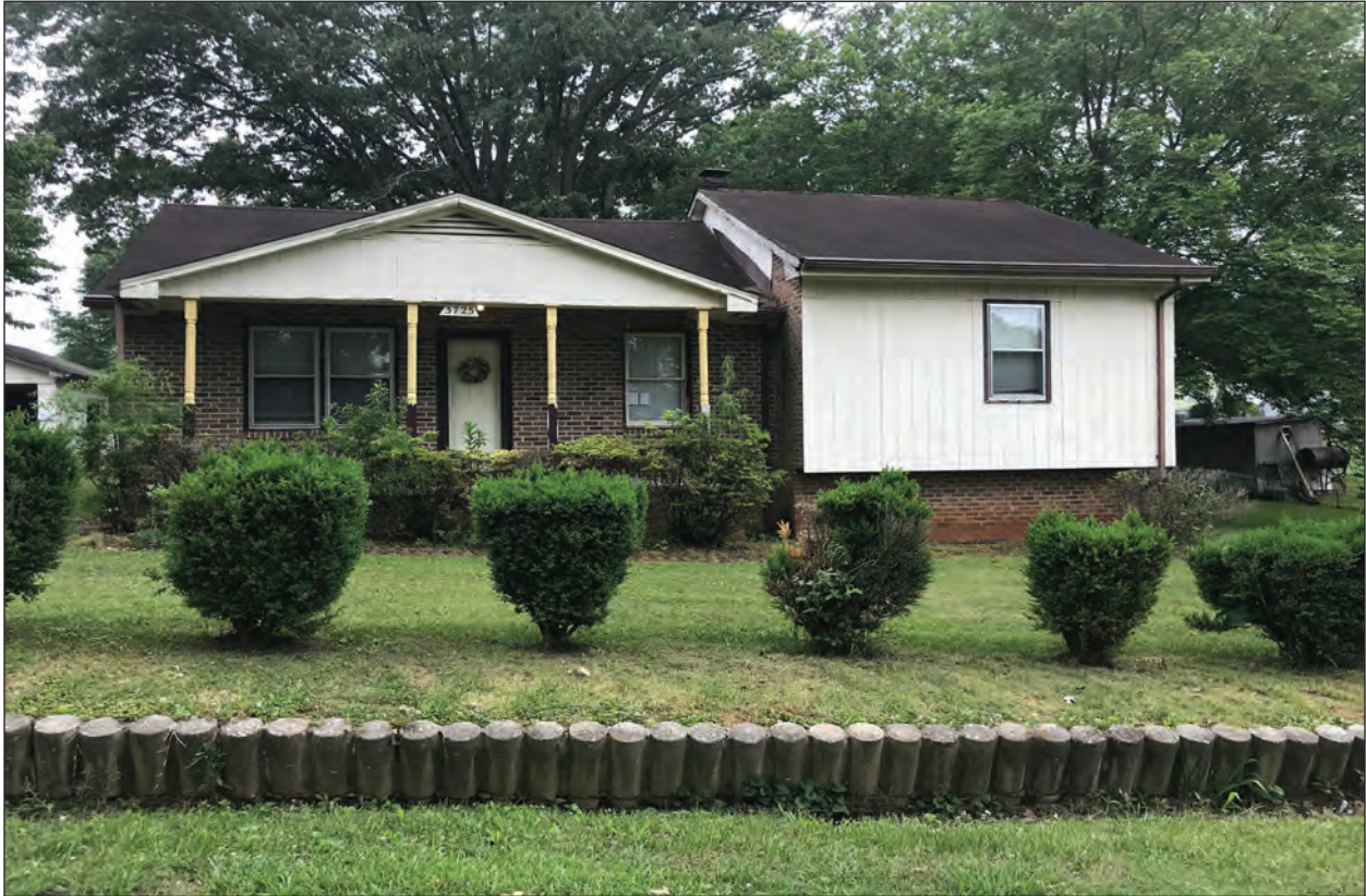
Figure 4.17 Side-gable ranch house with large side addition in the project area on 2nd Avenue NW, north front elevation.
