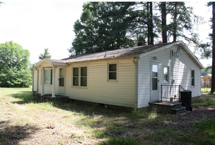
Plate 4.24: View of the primary and south elevations of the House.
