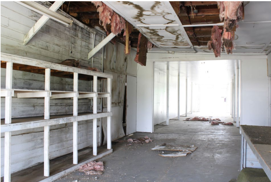
Plate 4.12: View of the interior of the westernmost wing of the Hangar.
