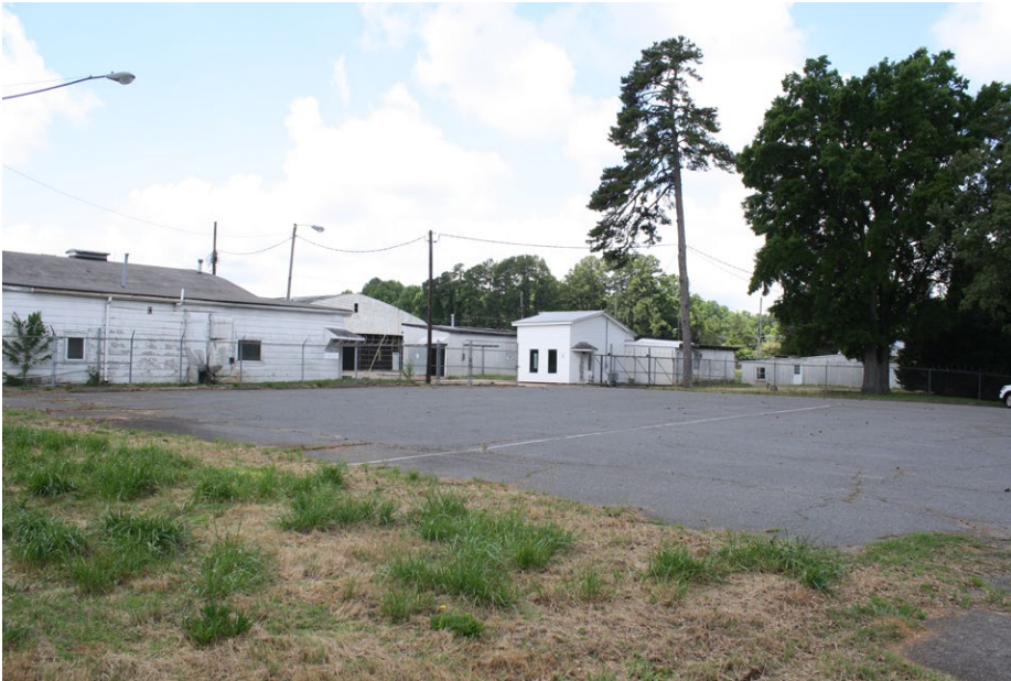
Plate 4.1: View of the entry into Grove Airport.
