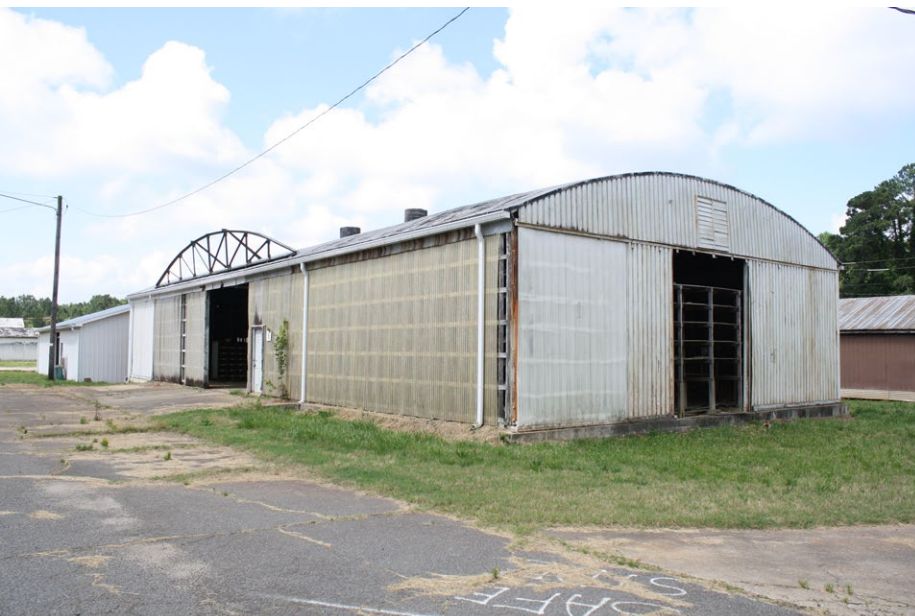
Plate 4.15: View of the primary and north elevations of Building 6.
