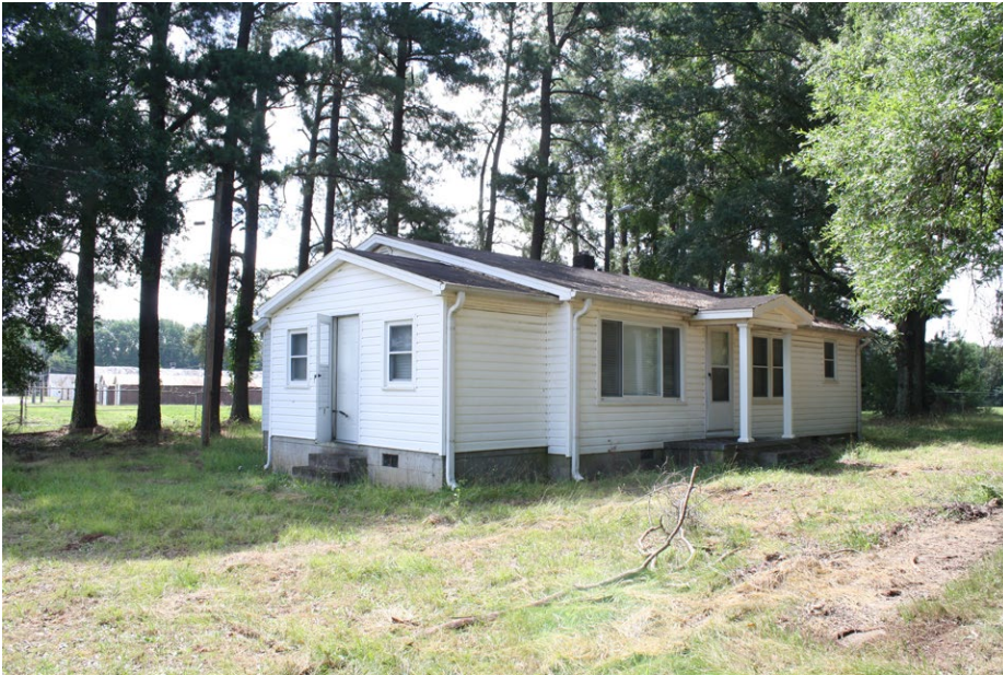
Plate 4.23: View of the primary and north elevations of the House.
