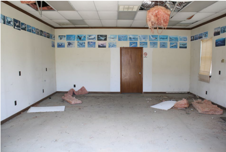
Plate 4.52: View of the office inside Building 90.
