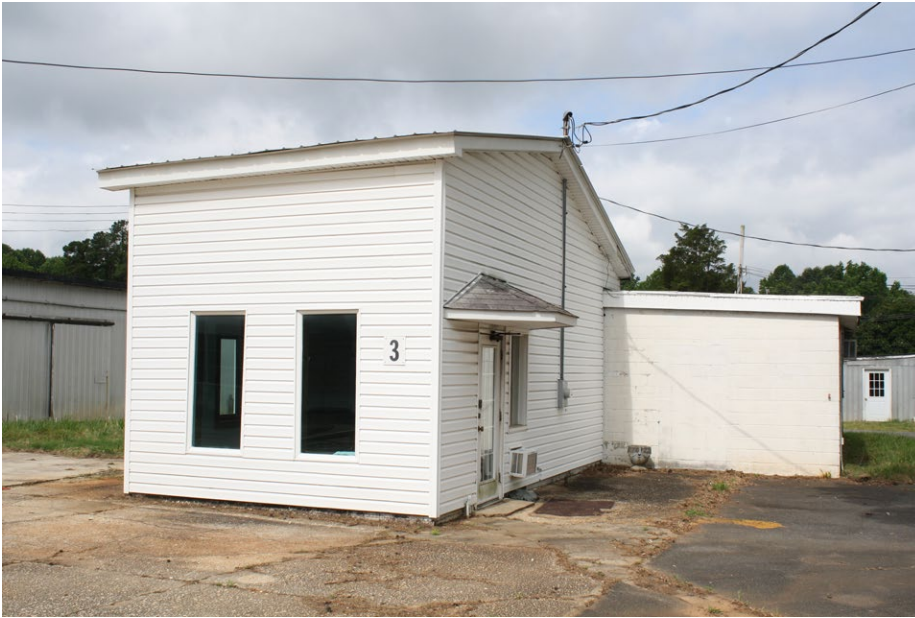
Plate 4.13: View of the primary elevation of Building 3.
