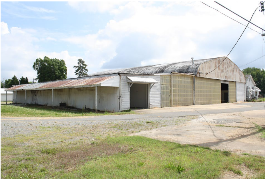
Plate 4.9: View of the rear elevation of the Hangar.
