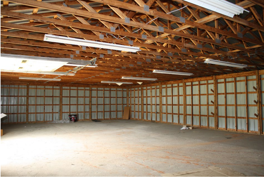
Plate 4.55: View of the interior of Building 74.
