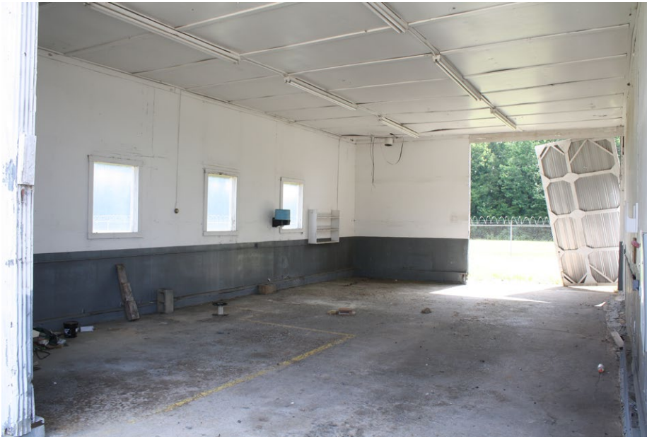
Plate 4.31: View of the interior of Building 11.
