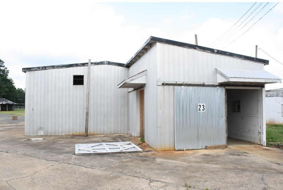
Plate 4.36: View of the east elevation of Building 23.
