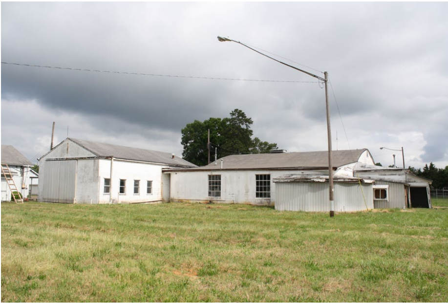
Plate 4.20: View of the rear elevation of Building 2 at the left of the photograph.
