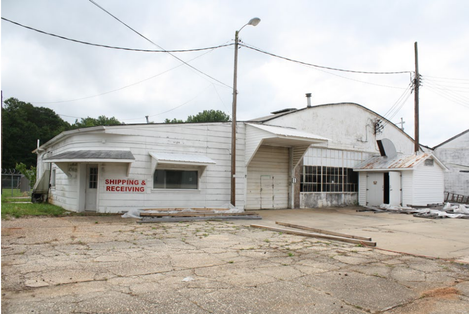
Plate 4.3: View of the primary elevation of Building 1.
