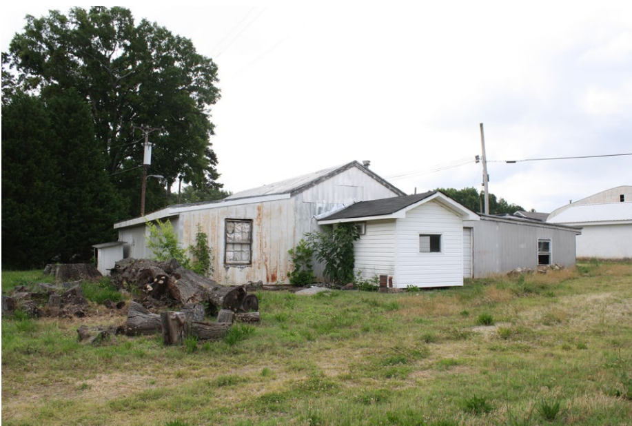
Plate 4.18: View of the north and west elevations of Building 4.
