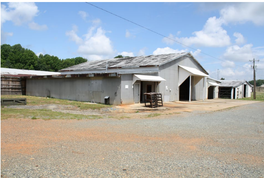
Plate 4.51: View of the primary and south elevations of Building 90.
