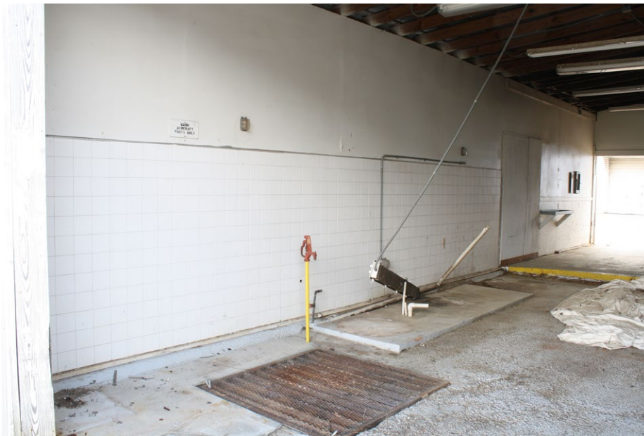
Plate 4.38: View of the interior of Building 23.
