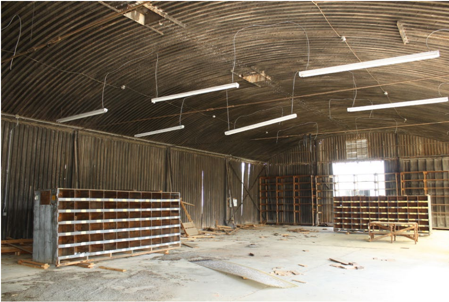
Plate 4.16: View of the interior of Building 6.
