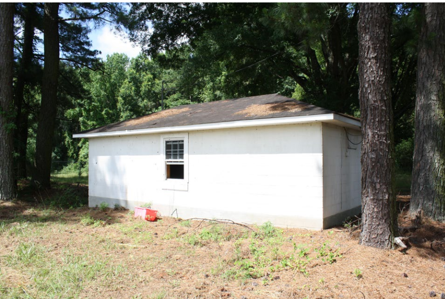
Plate 4.27: View of the rear elevation of the hipped roof residential building.
