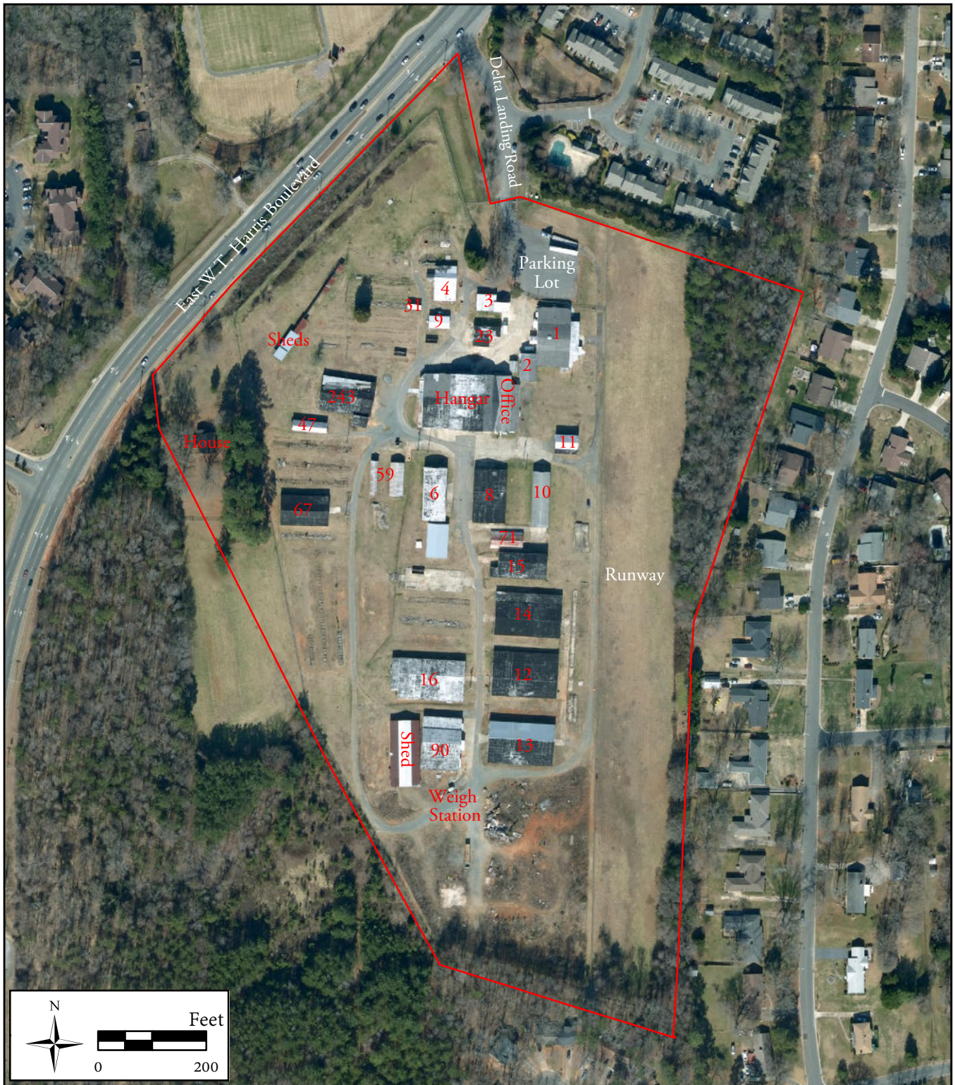
Figure 4.1: Overview of Grove Airport with building identification numbers (World Imagery, ESRI 2020).
