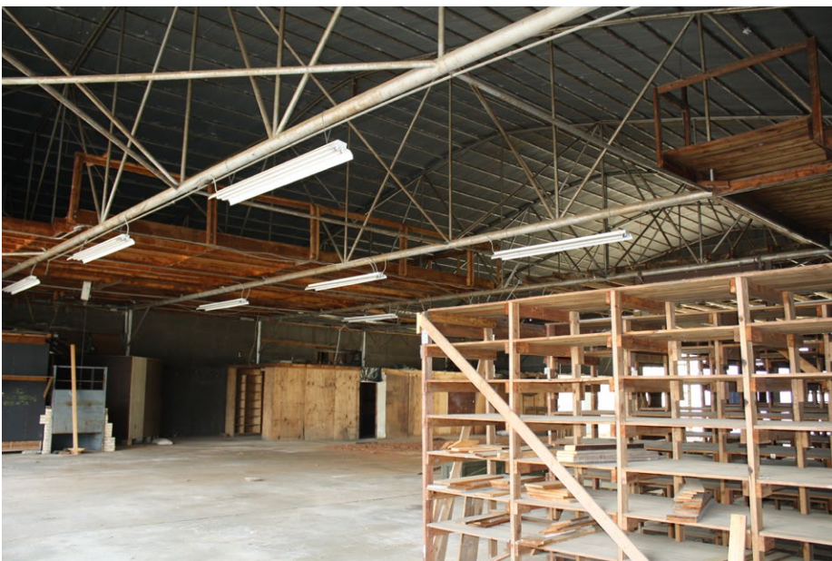
Plate 4.10: View of the interior of the Hangar.
