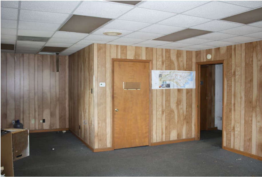
Plate 4.5: View of the interior of the office of Building 1.
