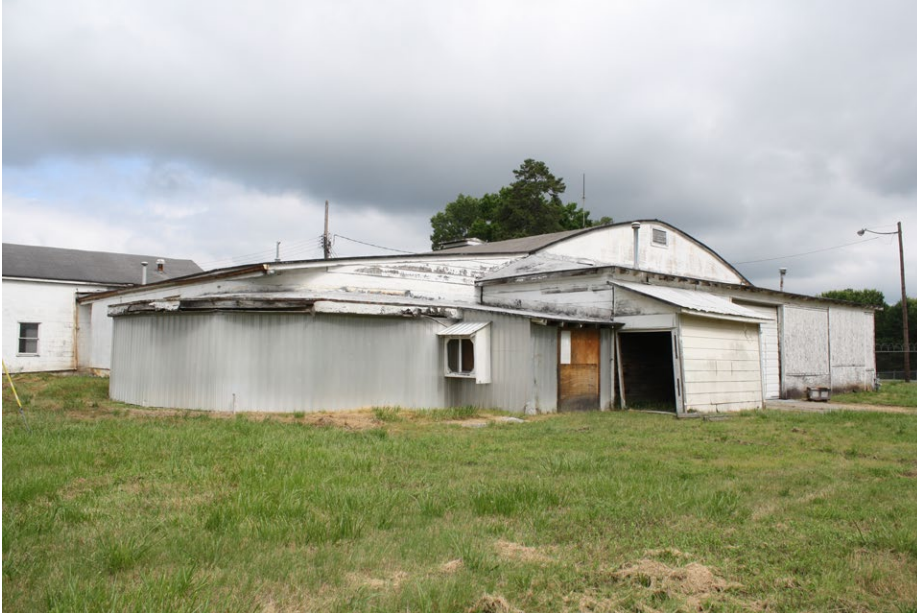
Plate 4.4: View of the rear elevation of Building 1.
