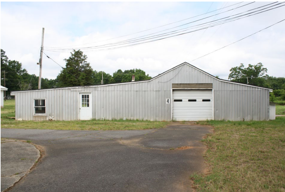
Plate 4.17: View of the primary elevation of Building 4.
