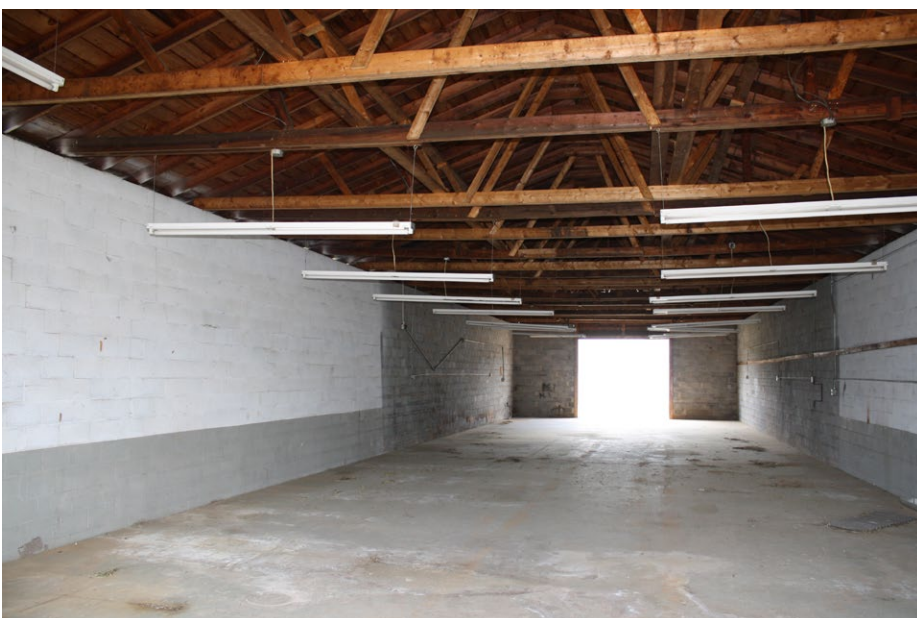
Plate 4.30: View of the interior of Building 10.
