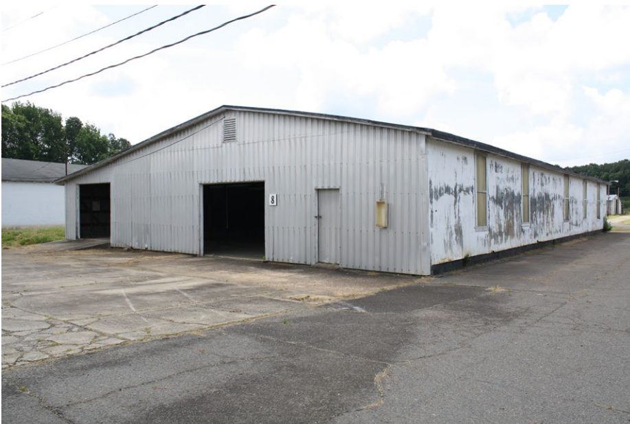
Plate 4.21: View of the north and west elevation of Building 8.
