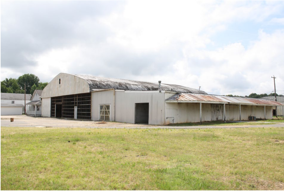
Plate 4.8: View of the primary (north) elevation of the Hangar.
