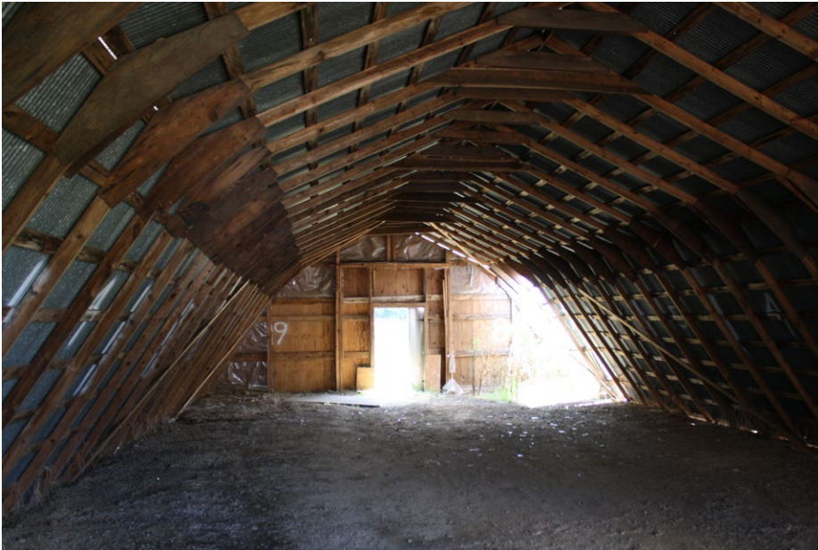
Plate 4.41: View of the interior of Building 71.
