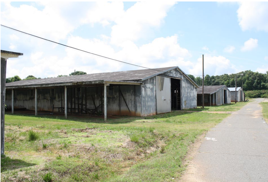
Plate 4.32: View of Buildings 14, 12, and 13.
