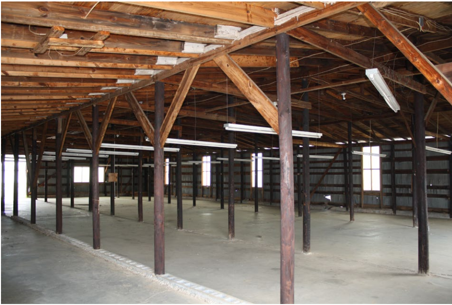
Plate 4.22: View of the interior of Building 8.
