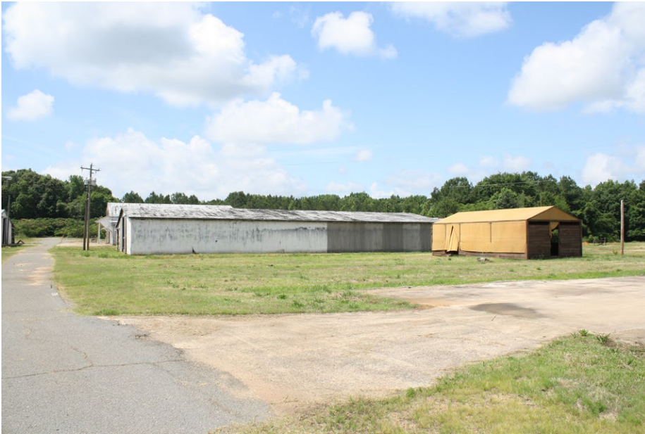
Plate 4.35: View of the north elevation of Building 16.
