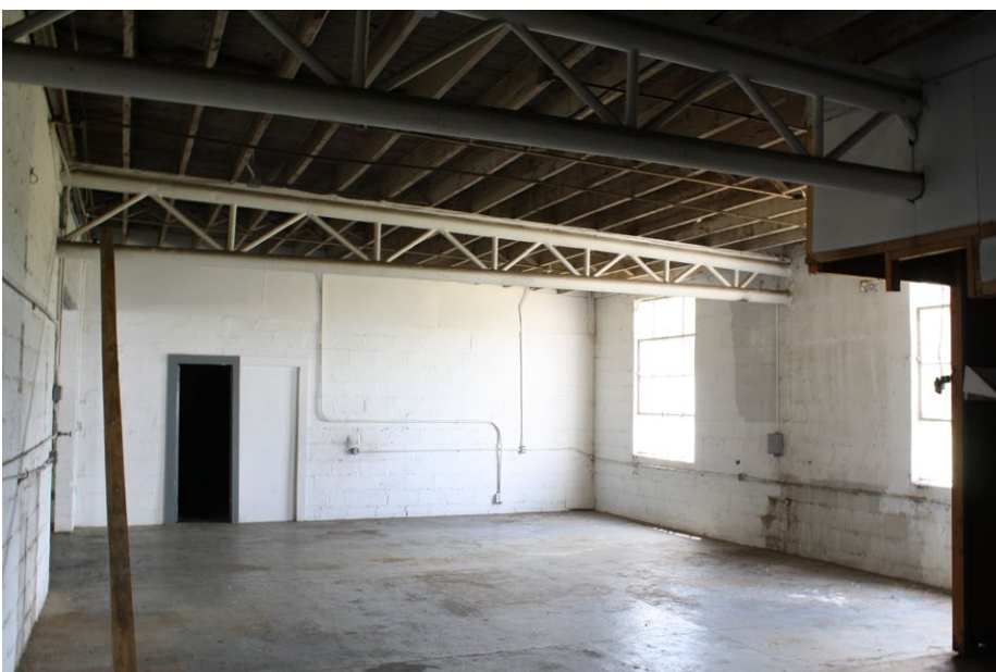
Plate 4.7: View of the interior of the south wing of Building 1.
