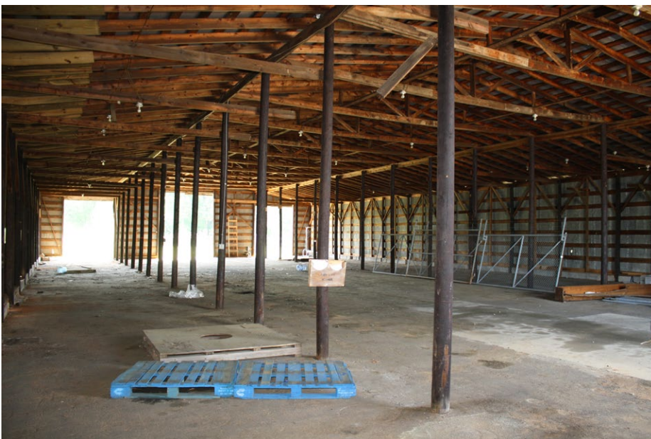
Plate 4.33: Interior view of Building 13, which is representative also of Buildings 12, 14, 15, 67, and 243.
