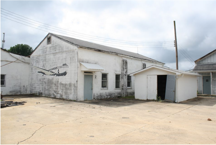
Plate 4.19: View of the primary elevation of Building 2.
