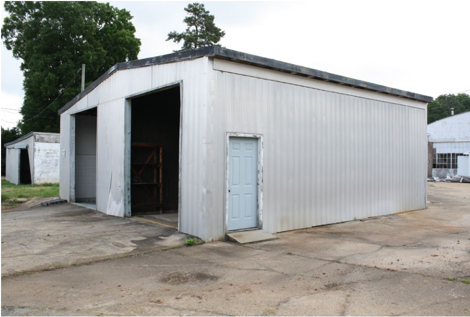
Plate 4.37: View of the rear and south elevations of Building 23.
