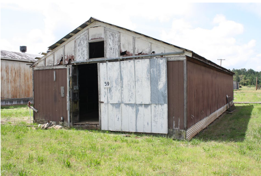
Plate 4.48: View of the north elevation of Building 59.
