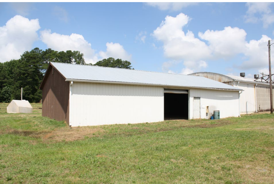
Plate 4.54: View of east elevation of Building 74.
