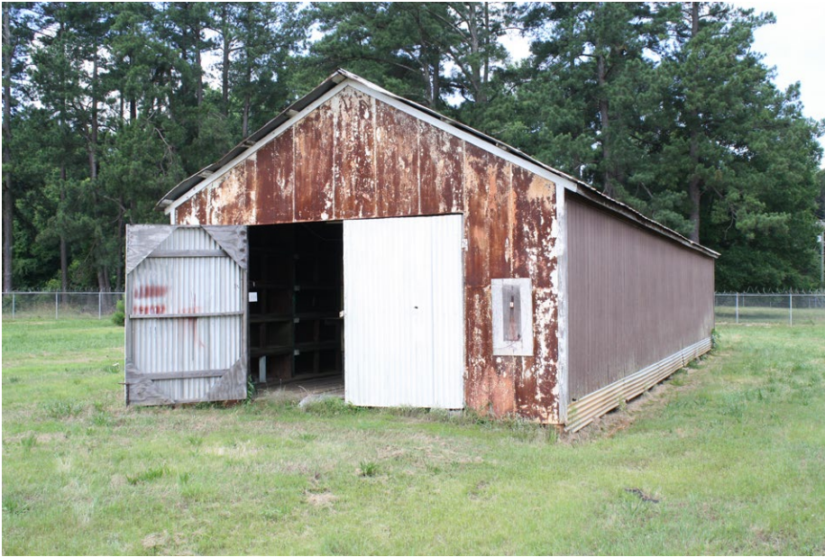
Plate 4.46: View of the east elevation of Building 47.
