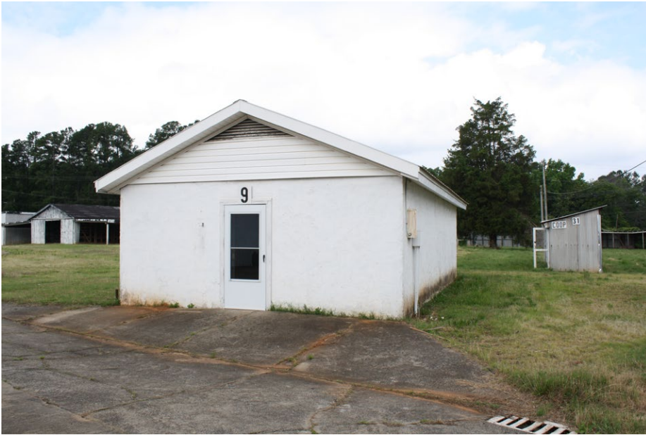
Plate 4.28: View of the primary elevation of Building 9.
