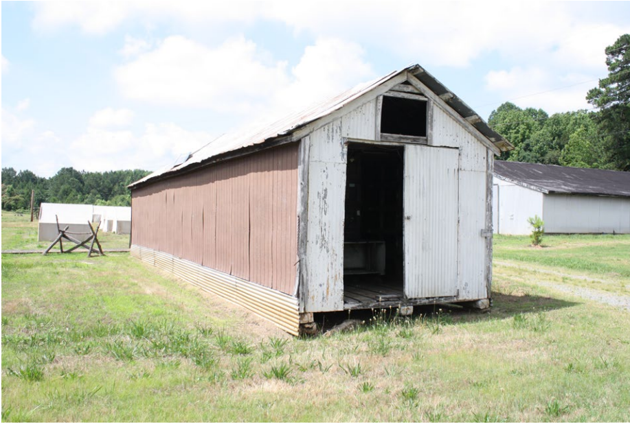
Plate 4.49: View of the building to the west of Building 59.
