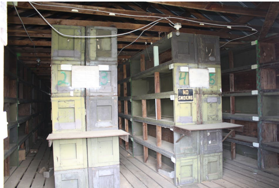
Plate 4.47: View of the interior of Building 47.
