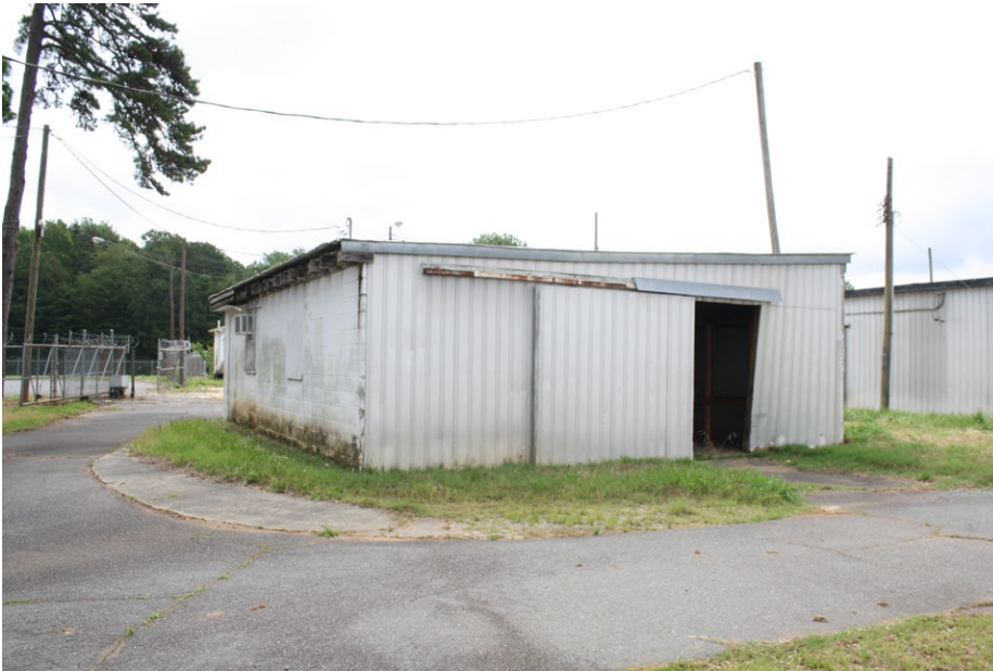
Plate 4.14: View of the rear elevation of Building 3.
