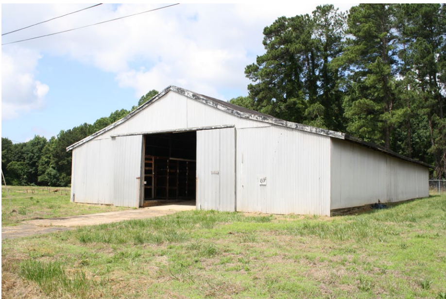
Plate 4.39: View of the east elevation of Building 67.
