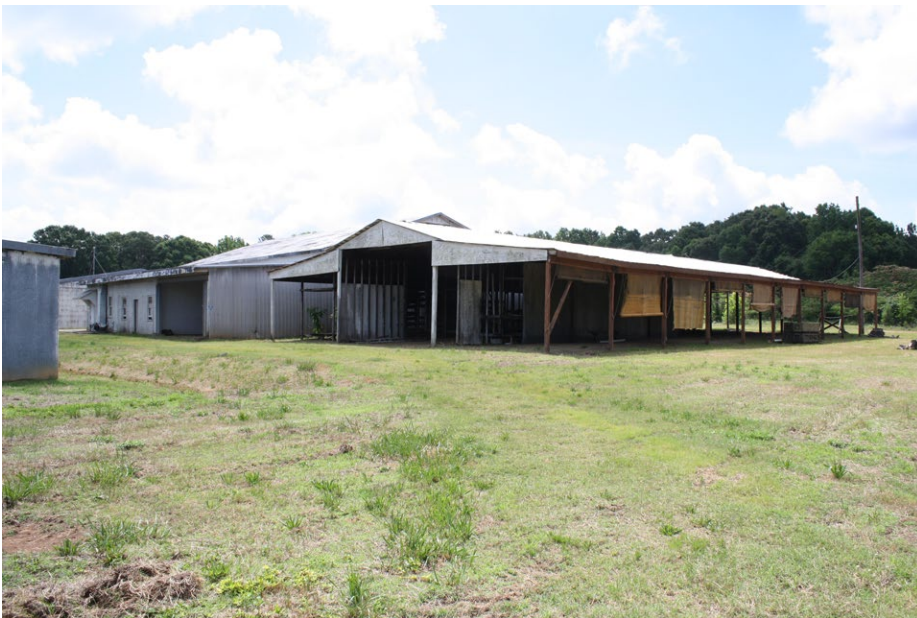
Plate 4.53: View of the shed behind Building 90.
