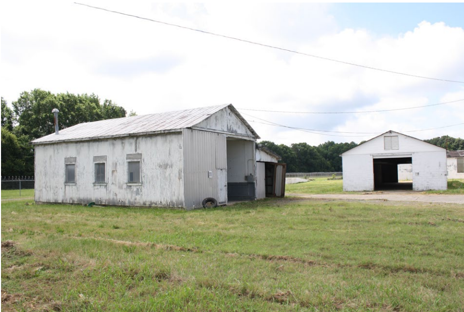
Plate 4.29: View of Buildings 10 and 11.
