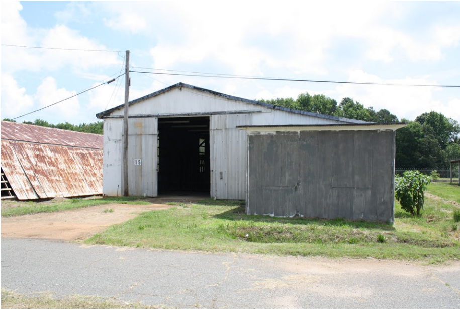
Plate 4.34: View of the east elevation of Building 15.
