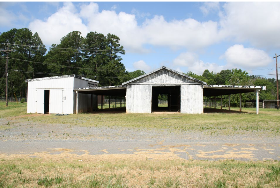
Plate 4.42: View of the east elevation of Building 243.
