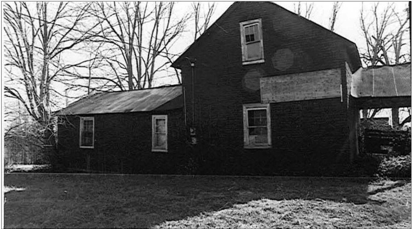
Figure 114: Northwestern elevation, 1981, showing later additions and siding (HPO Survey Files)
