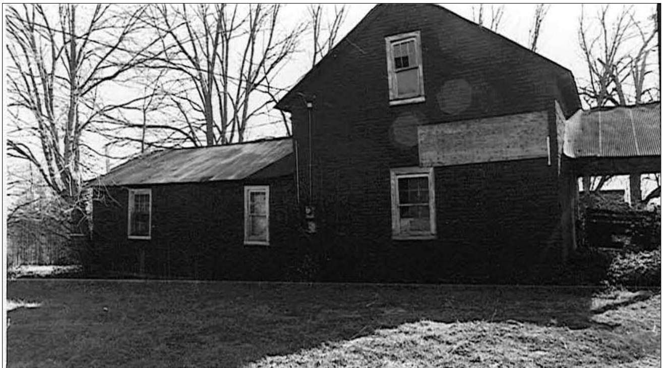
Figure 57: Snow House (SR0251), ca.1870 with later additions and asphalt siding, shown in 1981 before recent renovation (HPO Survey Files)
