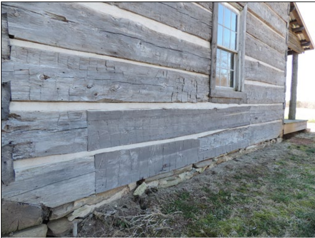
Figure 109: Detail of repaired original logs and new chinking on northwestern elevation
