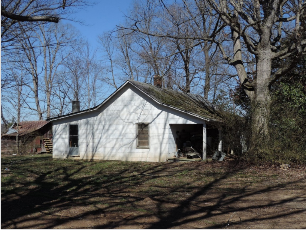
Figure 47: Farmhouse, likely expanded from nineteenth century log structure, 435 Highway 268, Pilot Mountain.
