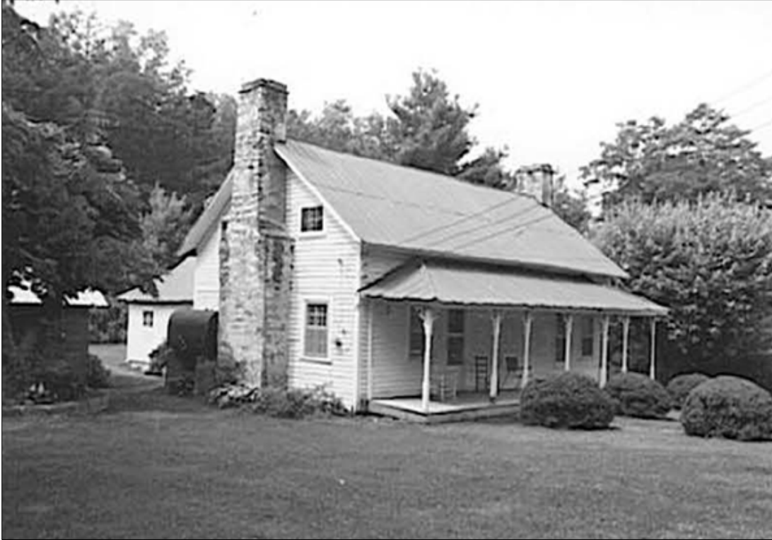
Figure 45: Chilton House (SR0027), ca 1895; SR 1799, Westfield Township (HPO Survey Files)
