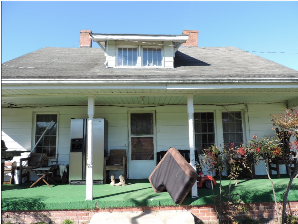
Figure 6: South elevation detail
