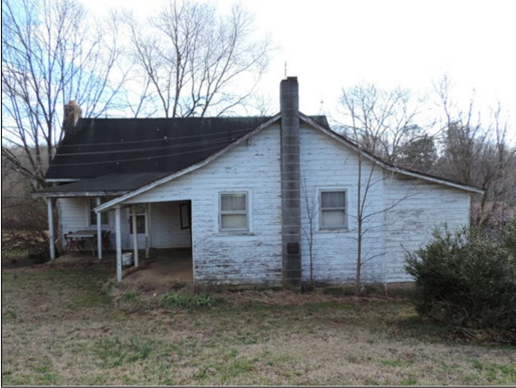
Figure 100: Draugh-Barnes House (SR1485), north (rear) elevation
