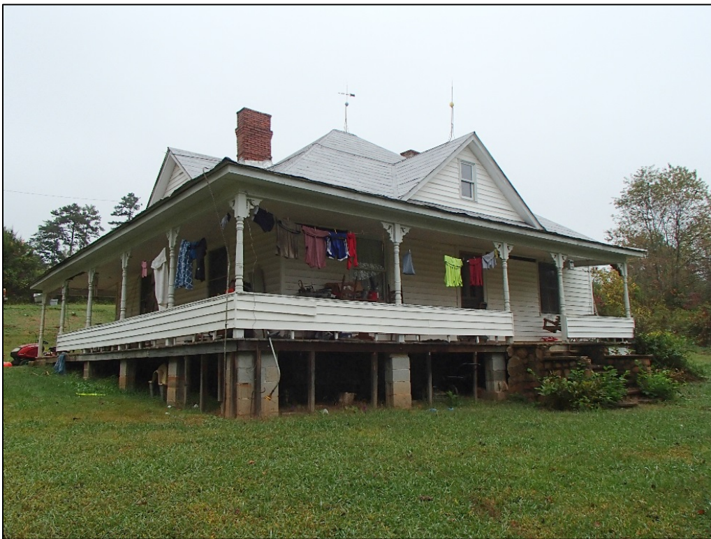
Figure 29: Cleveland Dobbins House (SR0554), ca. 1907, 167 Horse Haven Lane, Dobson
