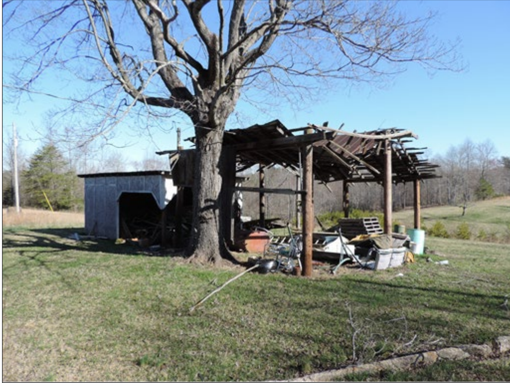
Figure 56: Remains of shed northwest of house
