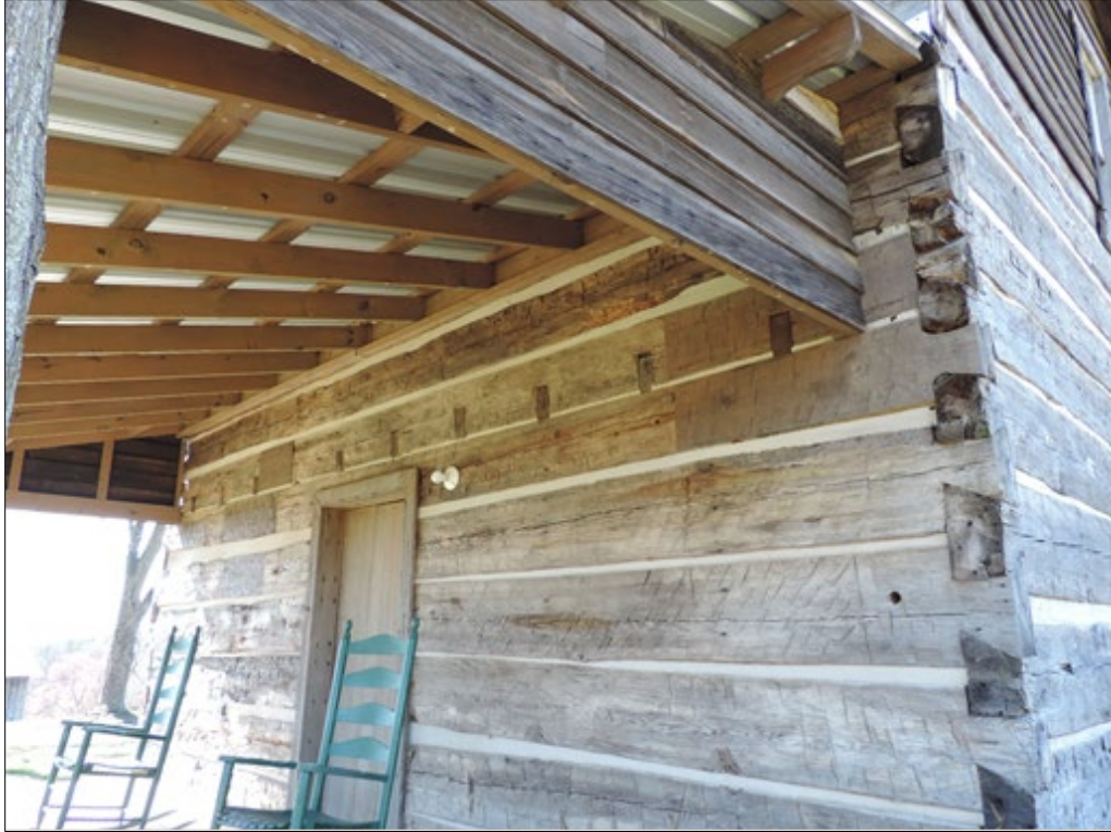
Figure 108: Detail of southwestern elevation wall and porch
