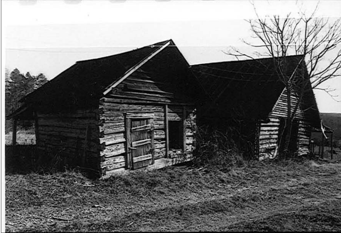
Figure 115: Nineteenth century log corncrib and barn, now destroyed (HPO Survey Files)
