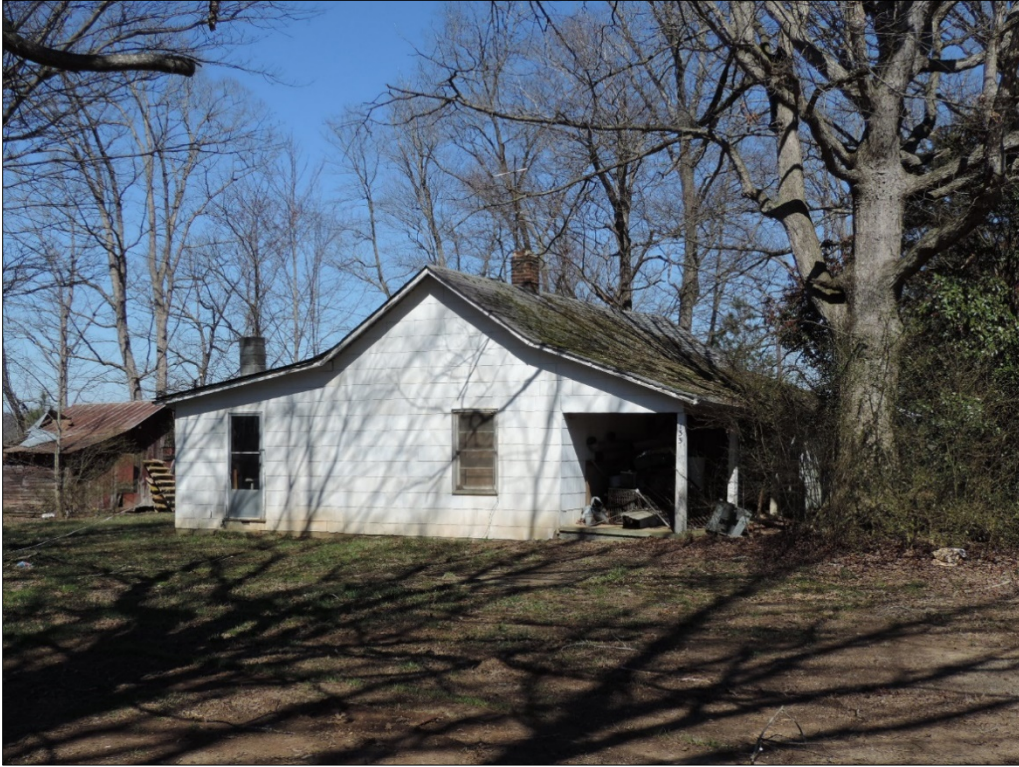
Figure 102: Farmhouse, likely expanded from nineteenth century log structure, 435 Highway 268, Pilot Mountain
