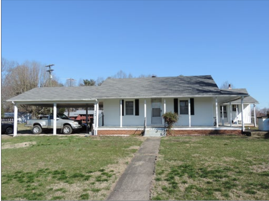
Figure 89: South (front) elevation
