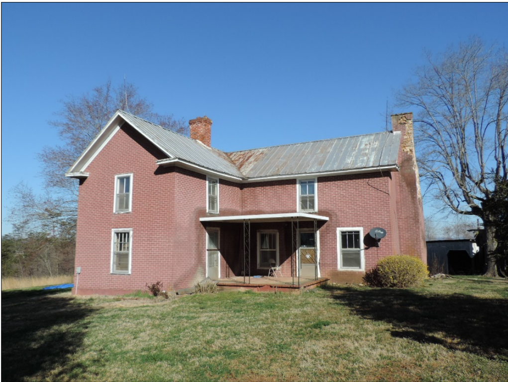
Figure 51: South (front) elevation
