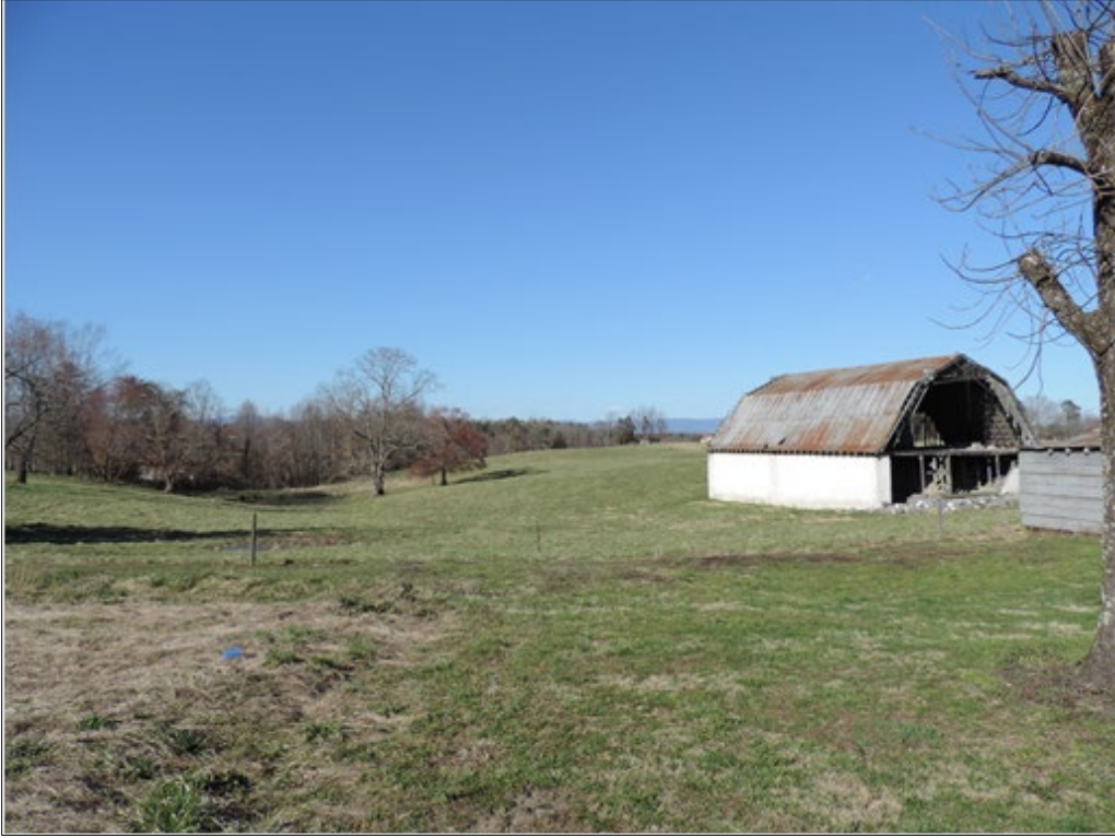
Figure 13: Looking northwest from the farmhouse; cinderblock and corrugated metal barn on the right
