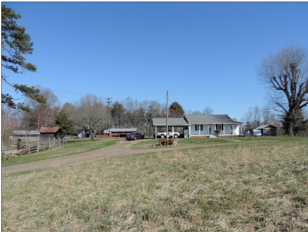
Figure 44: Wood-Hardy House, looking south, showing several outbuildings (SR1490)
