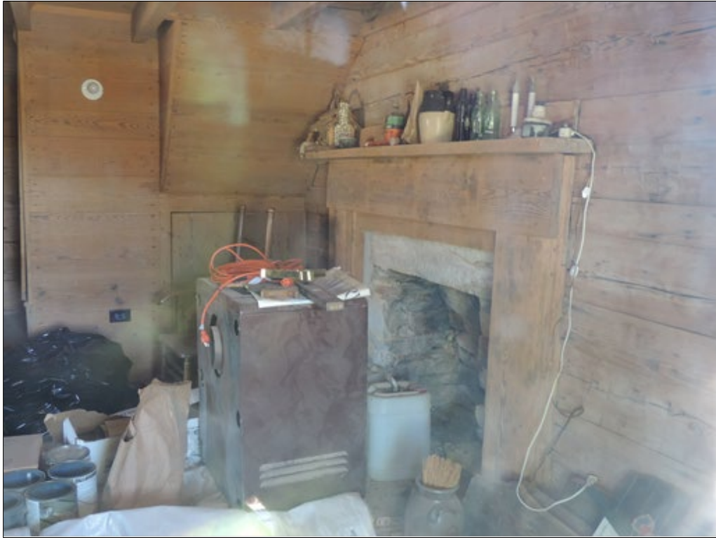
Figure 110: Interior view of the "hall," showing original plank walls, fireplace surround, and enclosed stairs to loft
