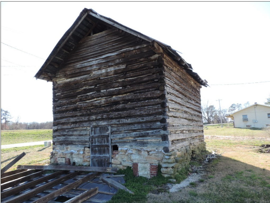
Figure 12: Log tobacco barn, 19th century. Southwestern side of property previously moved from another location.
