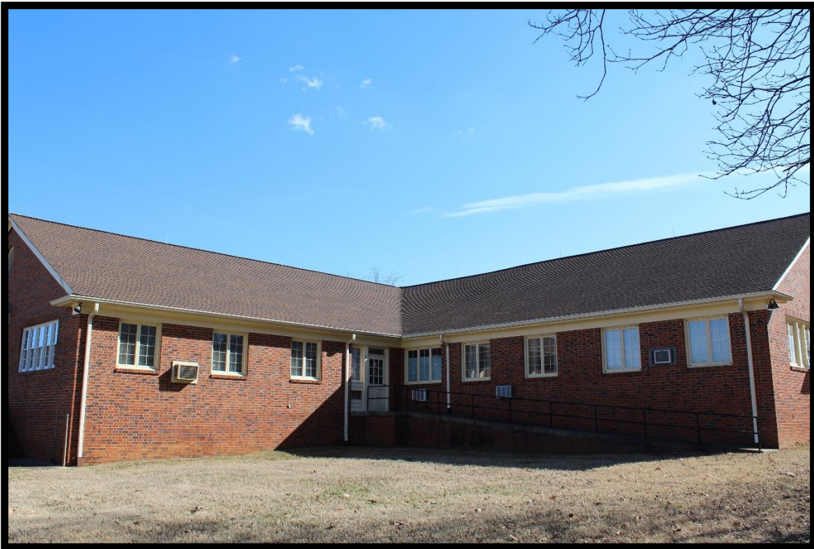
Figure 45: Hawfields Presbyterian Church, Educational Building, Looking Southeast.
