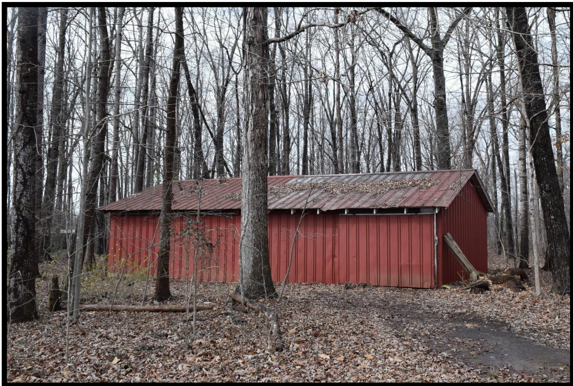
Figure 55: Hawfields Presbyterian Church, Shed, Looking Northwest.
