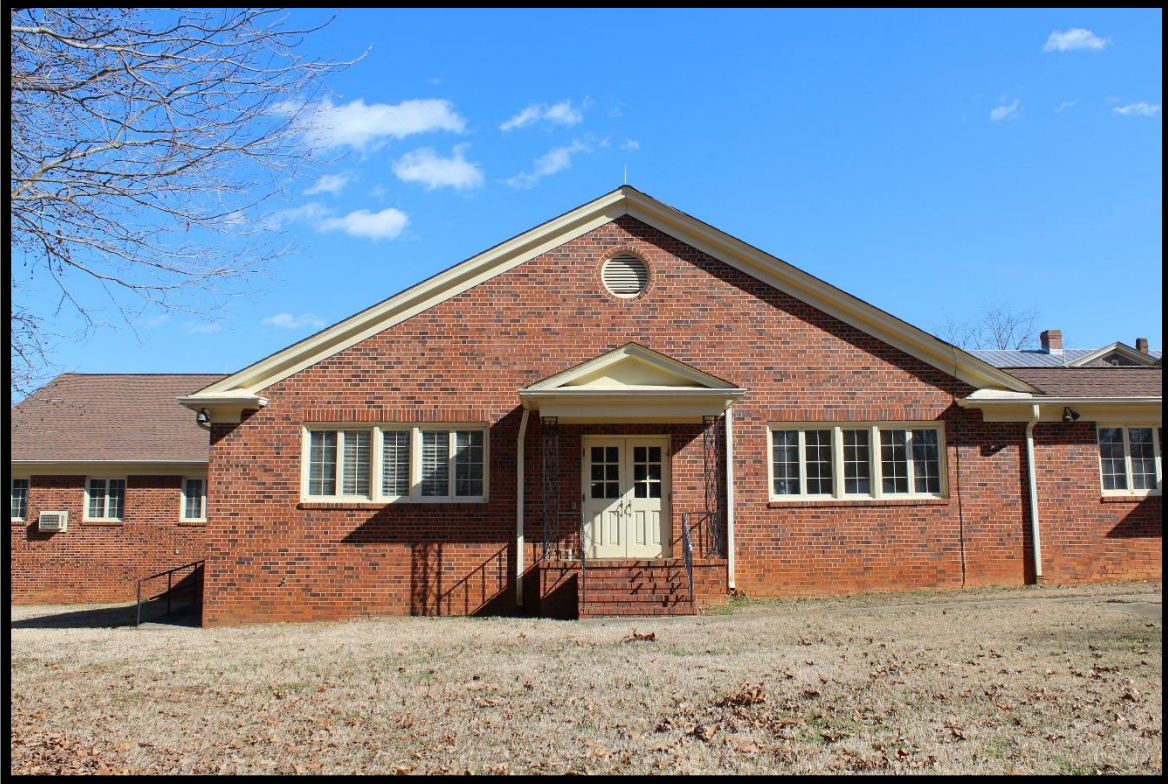
Figure 46: Hawfields Presbyterian Church, Educational Building, Looking Northeast.
