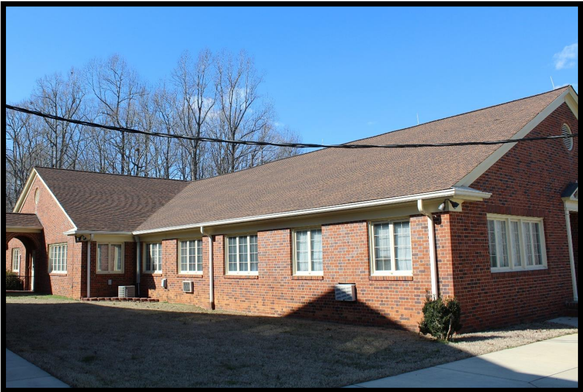
Figure 41: Hawfields Presbyterian Church, Educational Building, Looking Northwest.
