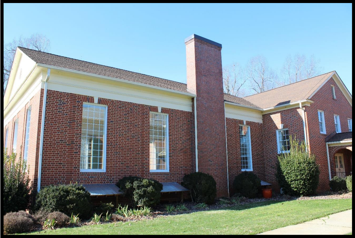
Figure 25: Hawfields Presbyterian Church, Fellowship Hall, Looking West.
