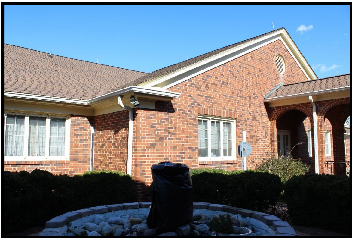
Figure 39: Hawfields Presbyterian Church, Educational Building, Looking Northeast.
