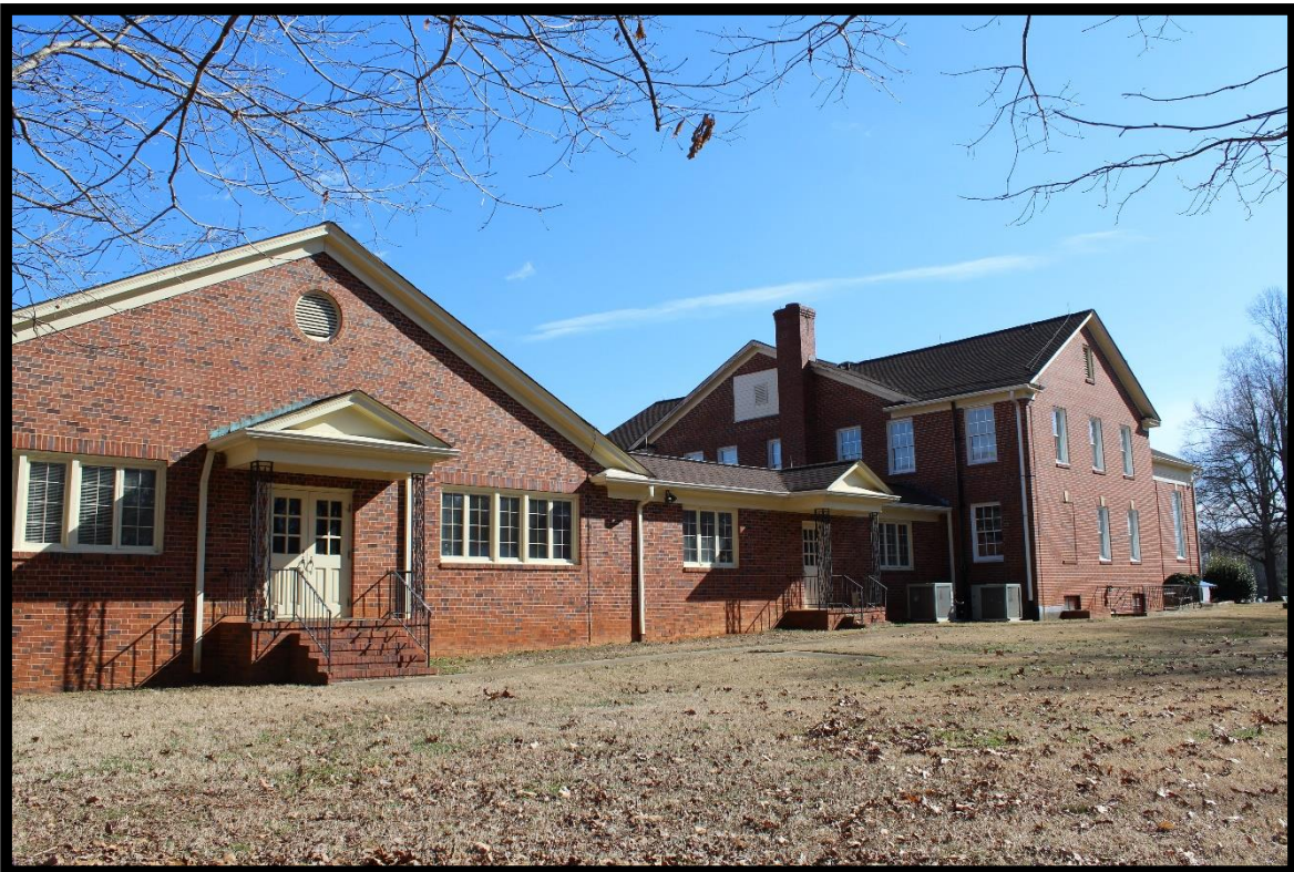
Figure 47: Hawfields Presbyterian Church, Educational Building, Hallway, and Fellowship Hall, Looking Southeast.
