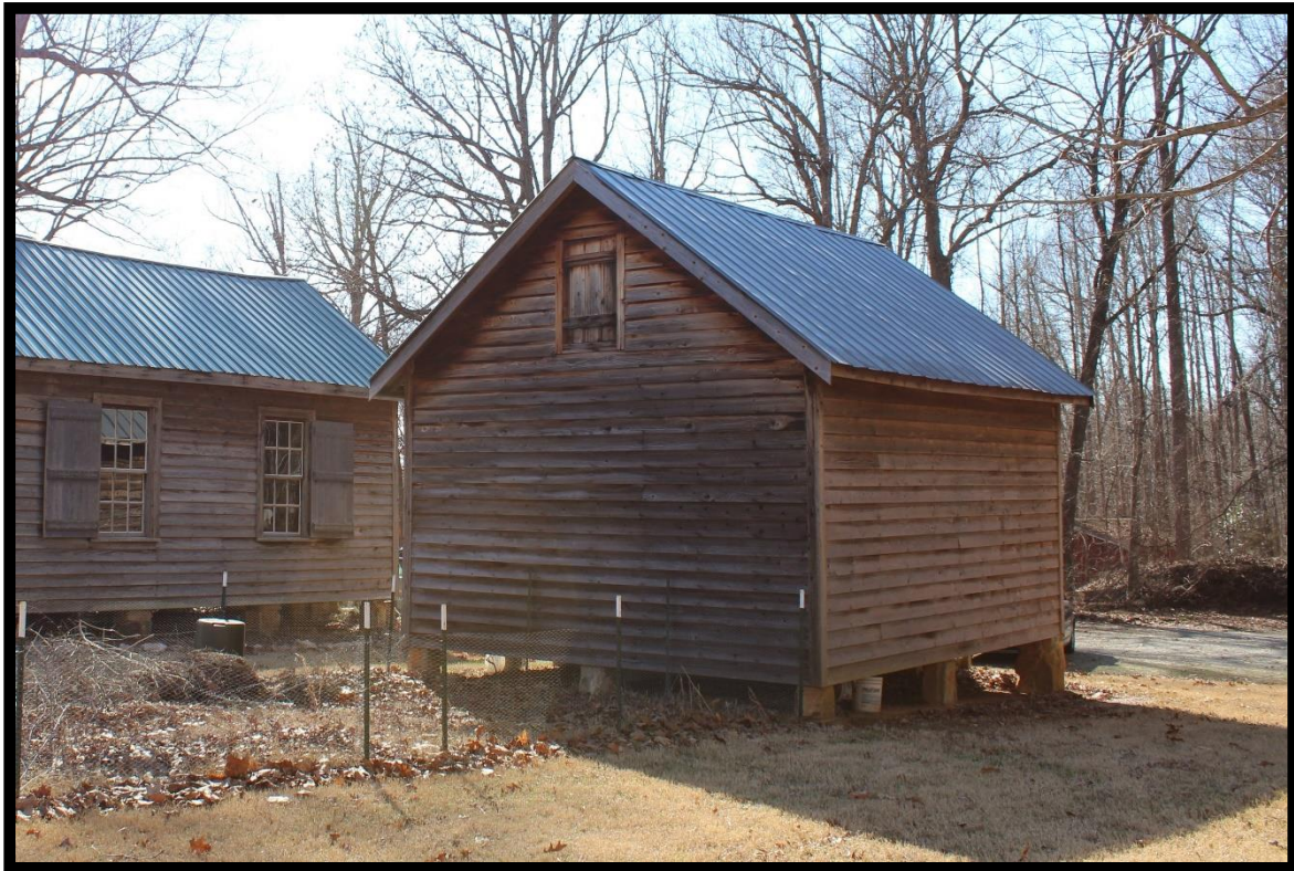
Figure 14: Albright Post Office, Looking Southwest.
