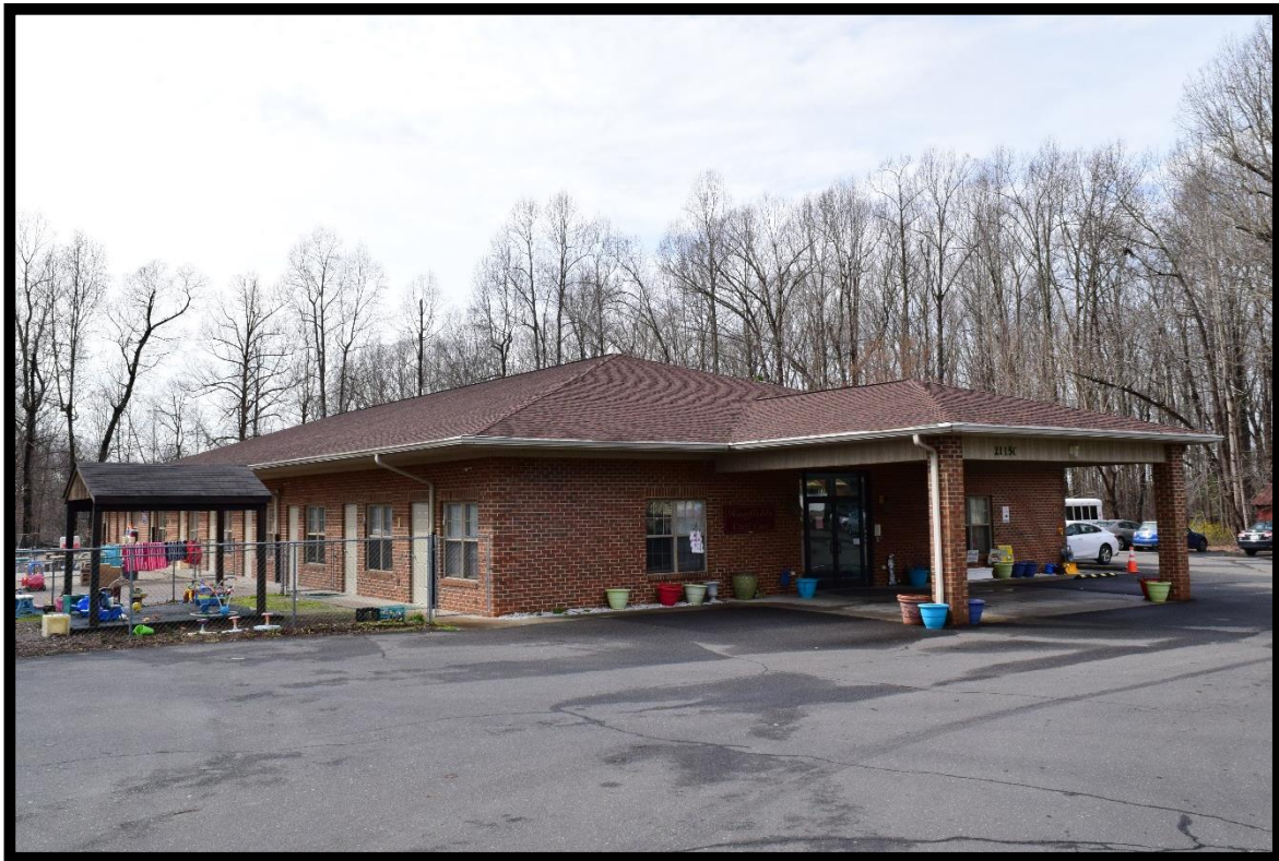
Figure 56: Hawfields Presbyterian Church, Childcare Center, Looking Northwest.
