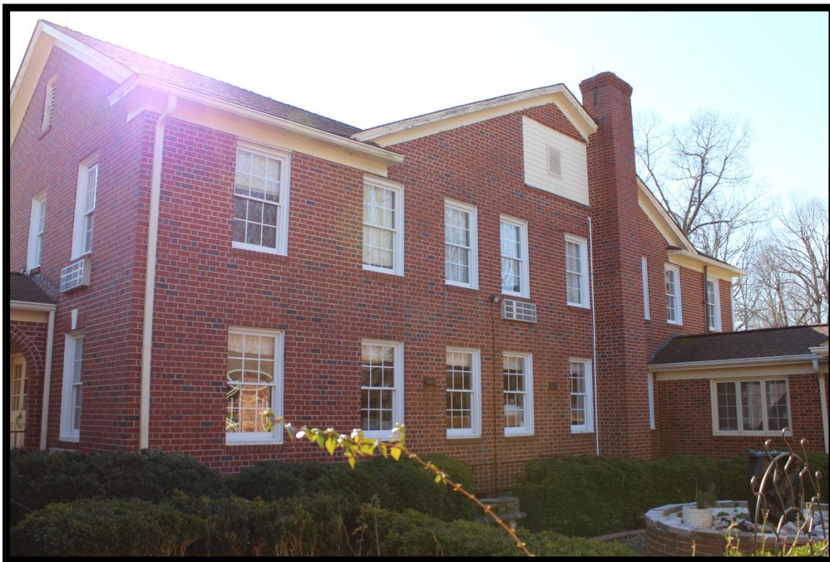
Figure 29: Hawfields Presbyterian Church, Fellowship Hall, Looking Southwest.
