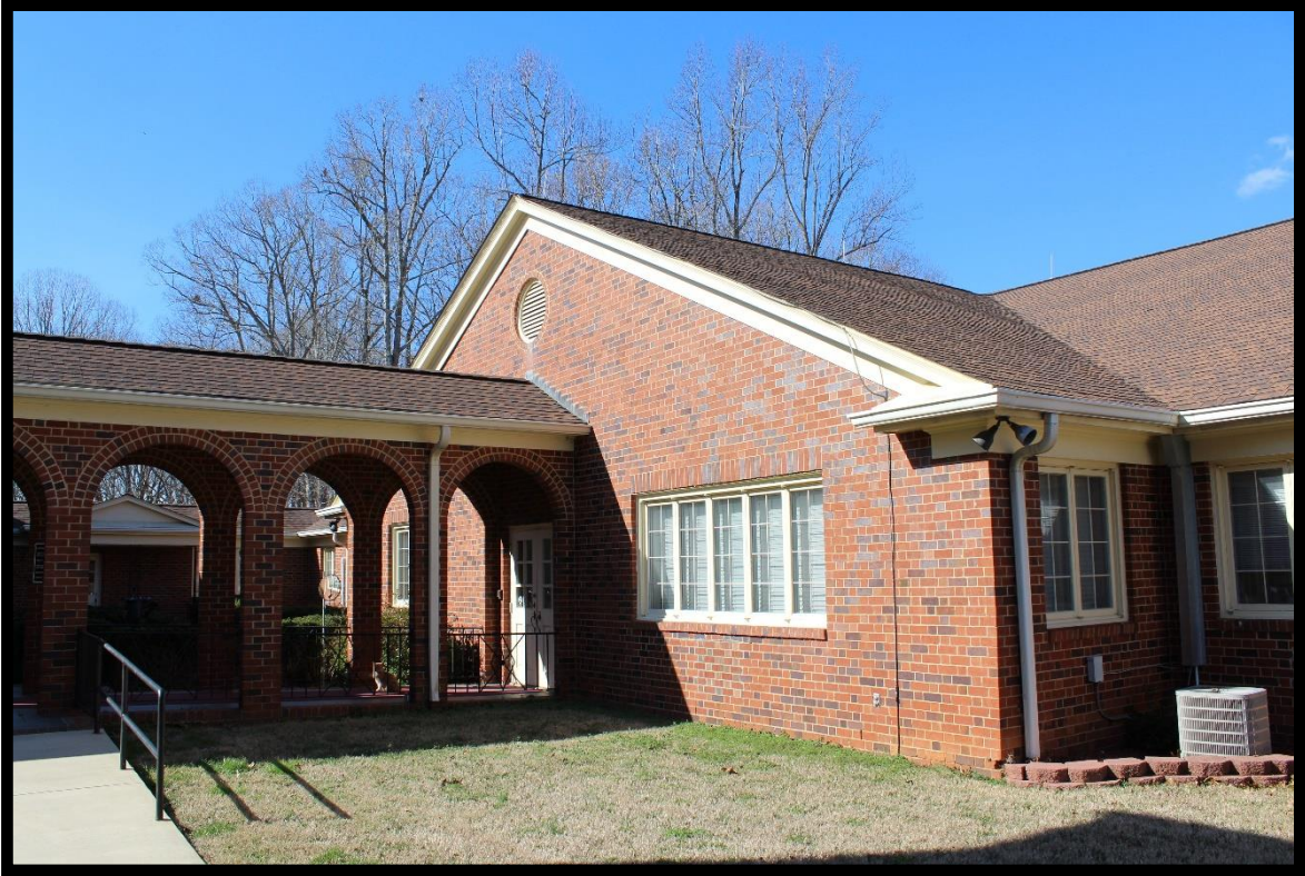
Figure 40: Hawfields Presbyterian Church, Educational Building, Looking West.
