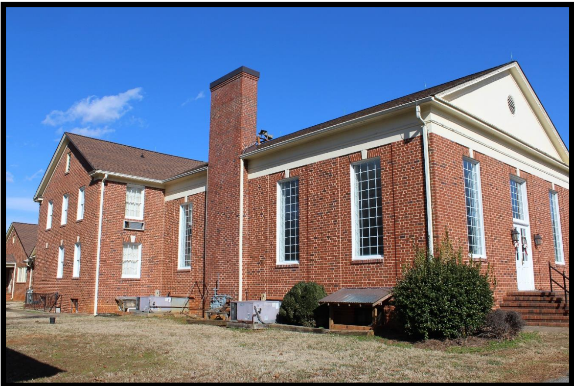
Figure 26: Hawfields Presbyterian Church, Fellowship Hall, Looking Northeast.
