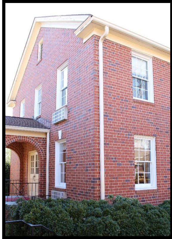
Figure 27: Hawfields Presbyterian Church, Fellowship Hall, Looking Southwest.
