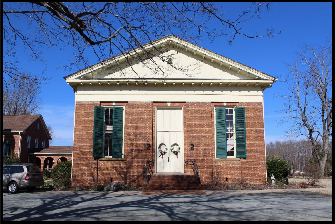
Figure 20: Hawfields Presbyterian Church, Looking North-Northwest.
