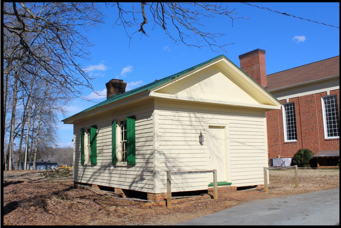
Figure 22: Hawfields Presbyterian Church, Session House, Looking Northeast.
