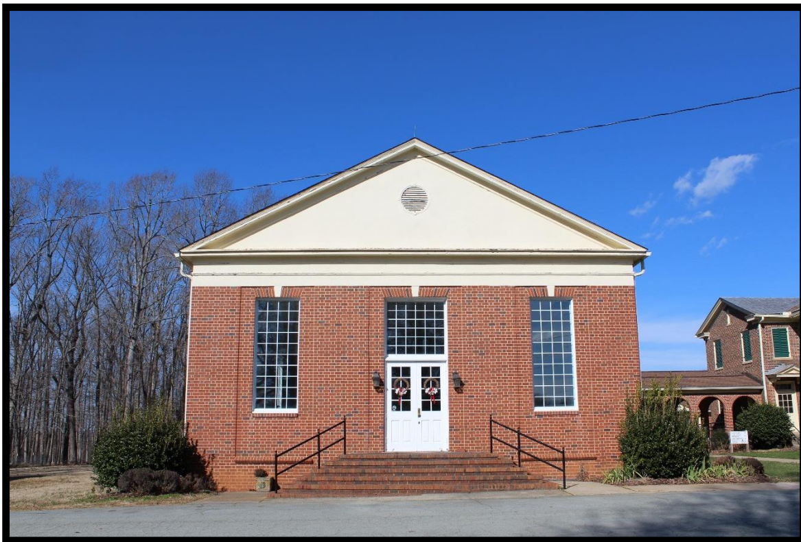
Figure 24: Hawfields Presbyterian Church, Fellowship Hall, Looking North-Northwest.
