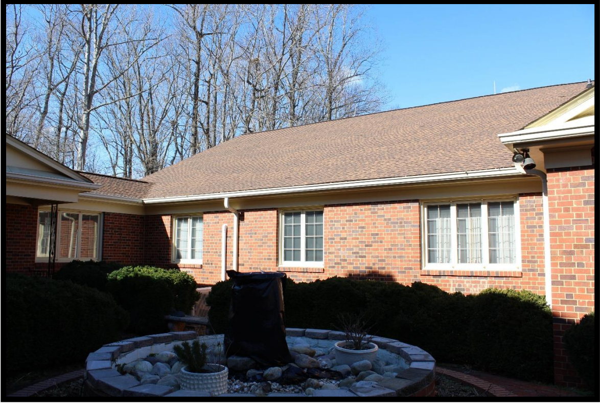
Figure 48: Hawfields Presbyterian Church, Educational Building, Looking Northwest.
