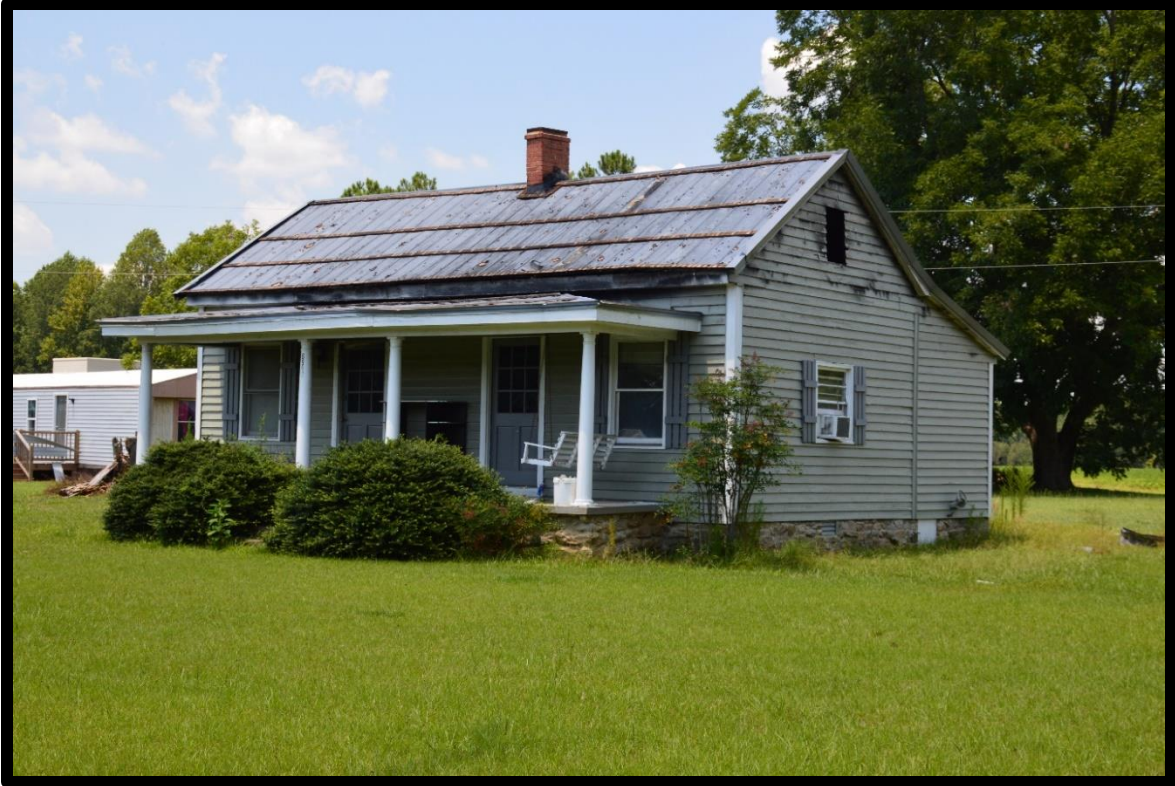
Figure 21: Wall House, 6602 Covered Bridge Road (JT1987).
