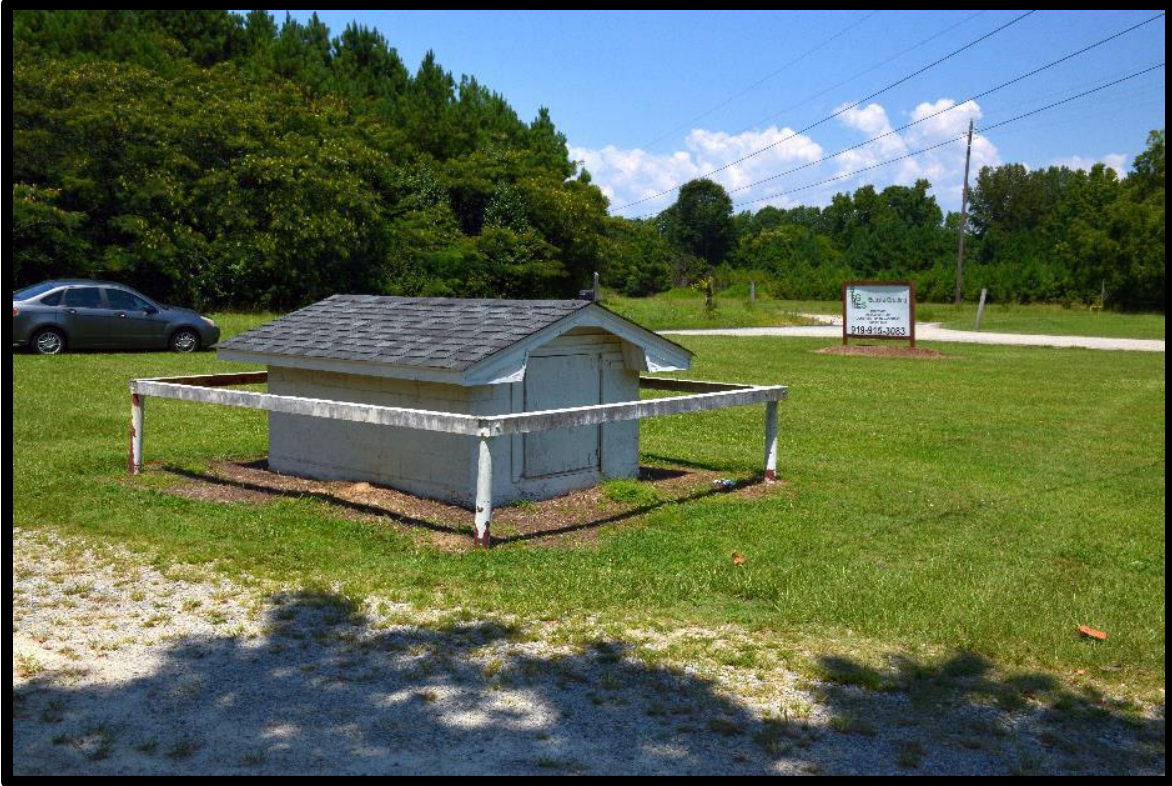
Figure 11: Ellis Tenant House, Well House, Looking Northeast.
