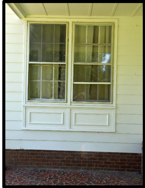
Figure 7: Ellis Tenant House, Window Detail.
