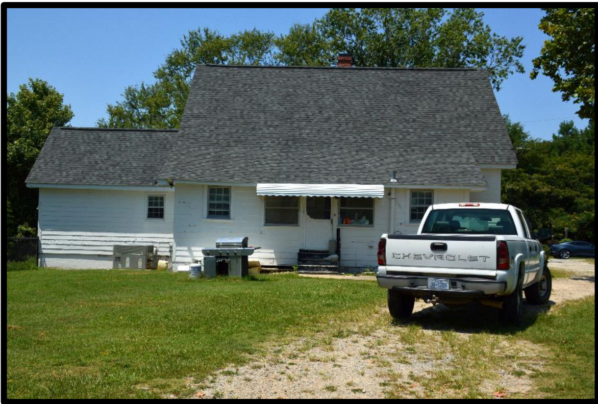
Figure 9: Ellis Tenant House, View West.
