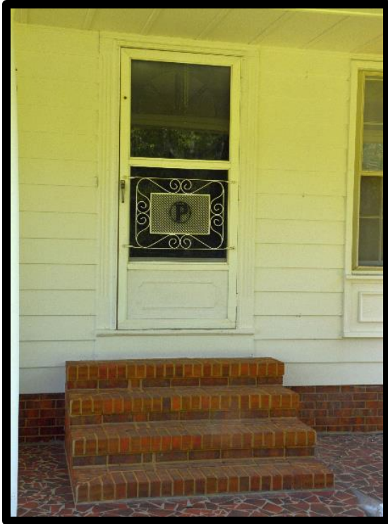
Figure 6: Ellis Tenant House, Entry Detail.
