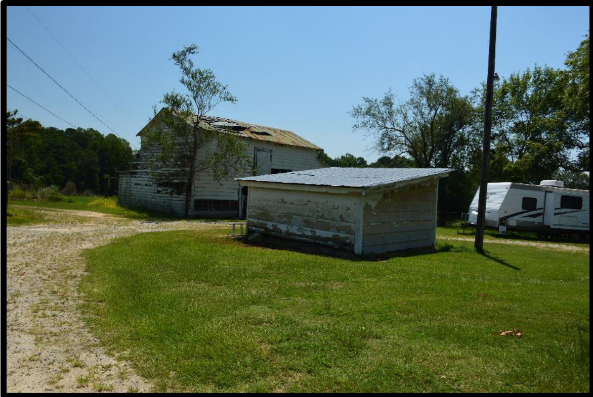
Figure 12: Ellis Tenant House, Chicken House (right) and Barn (left), Looking Southwest.
