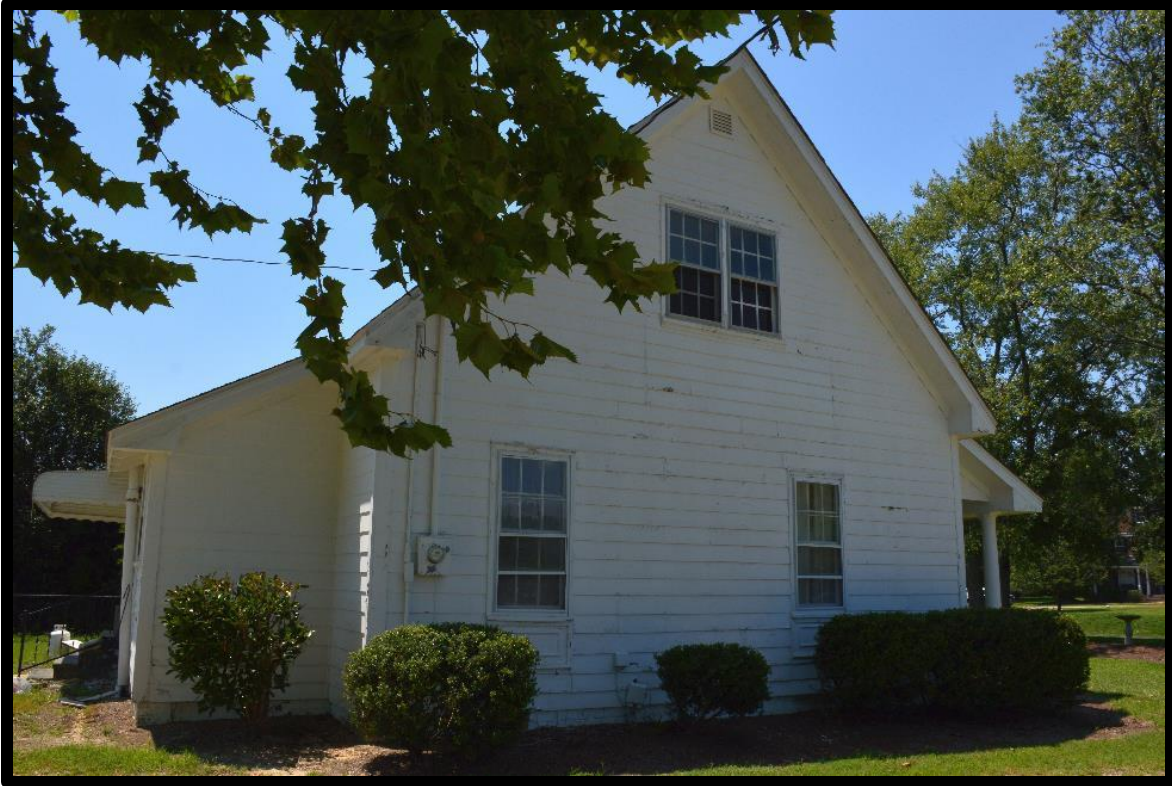
Figure 8: Ellis Tenant House, Looking South.
