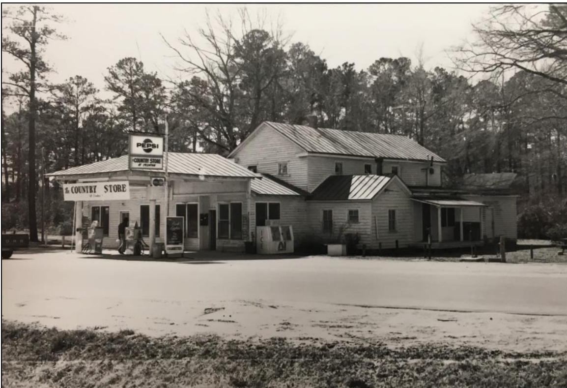
Figure 31: Survey Site Photograph, east and north elevation of store, January 1981.
