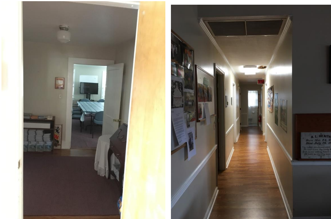
Figures 55 and 56: Vestibule and meeting room within one-story addition looking south, and hallway leading to Sunday school rooms, office, and bathrooms within fellowship hall addition, looking north.
