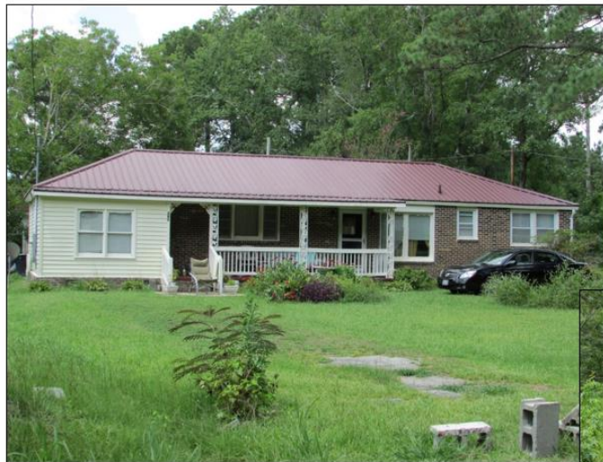
Address: 260 Green Avenue Date: 1960 Parcel: 7-054-025
