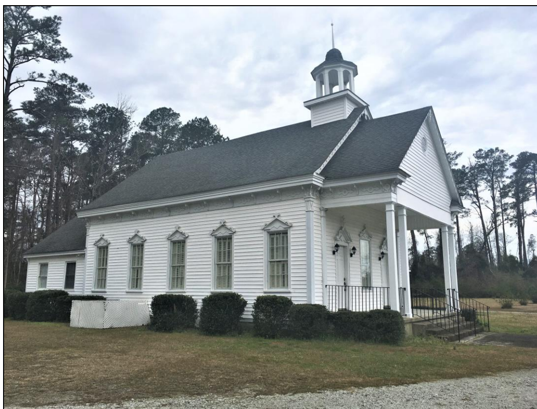
Figure 40: Croatan Presbyterian Church (CV1385) looking west.
