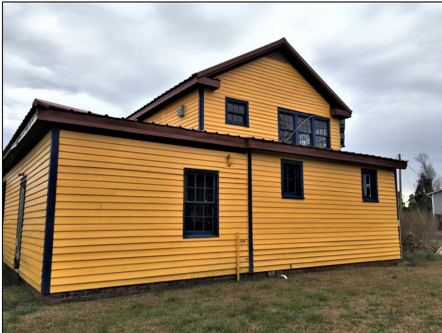
Figure 13: Tom Haywood Store, west elevation.
