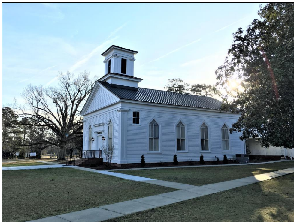
Figure 67: Grove Presbyterian Church (DP0013).
