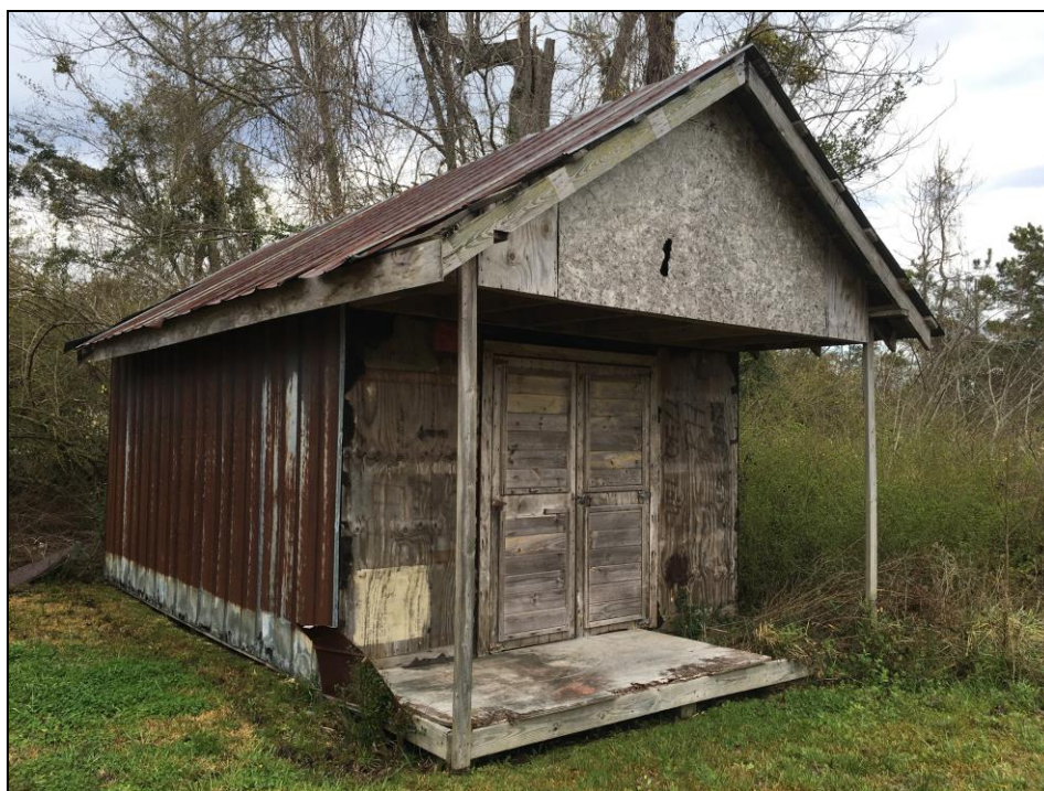
Figure 24: Shed, looking northwest.
