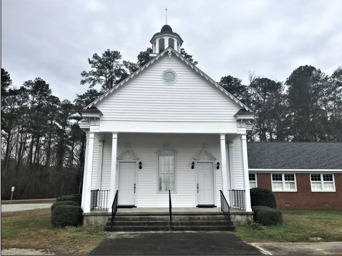
Figure 42: Northeast elevation of church looking southwest.
