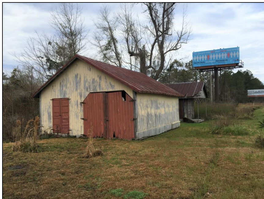
Figure 23: Garage, looking north.
