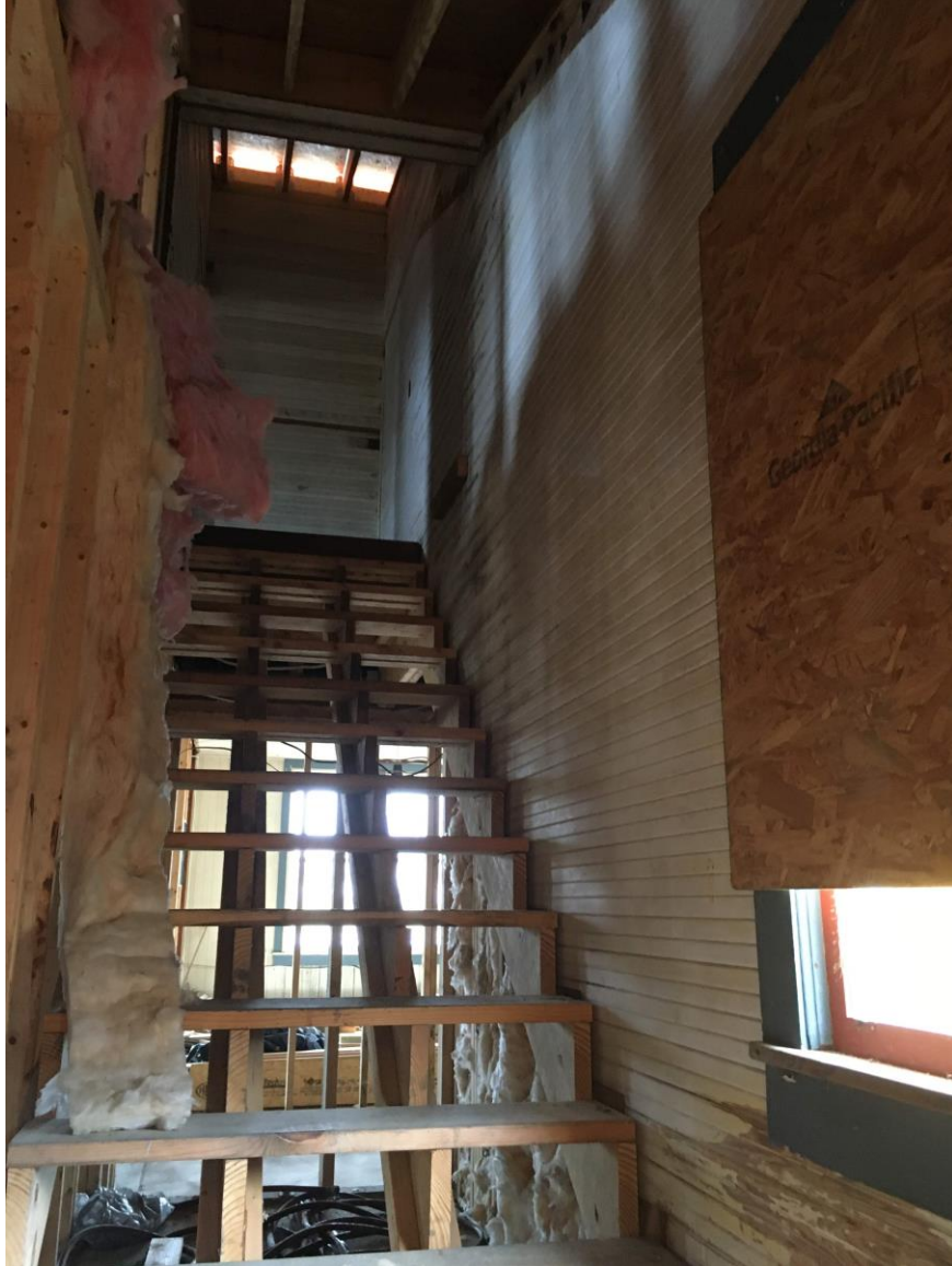
Figure 21: Exterior stairwell to second floor on south elevation, looking east.
