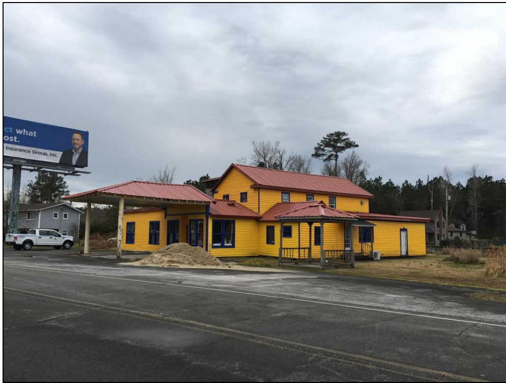
Figure 7: Tom Haywood Store (CV1044), looking southwest.
