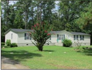
Address: 230 Green Avenue Date: 1969 Parcel: 7-053-010
