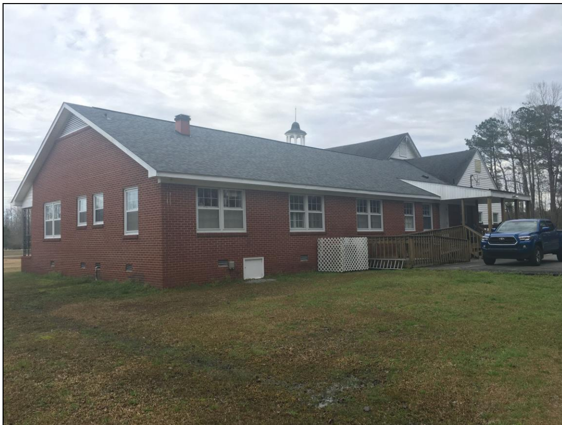
Figure 48: Sunday school and fellowship hall addition, looking east.
