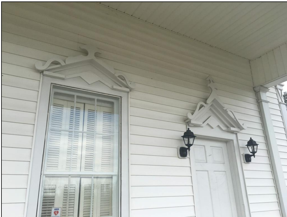
Figure 44: Detail of decorative triangular hoods over doors and windows on sanctuary.
