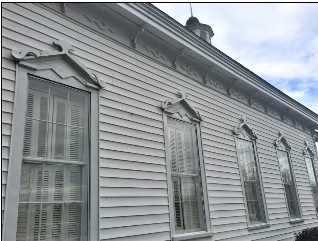
Figure 45: Detail of frieze with circle and arrow motif, southeast elevation.
