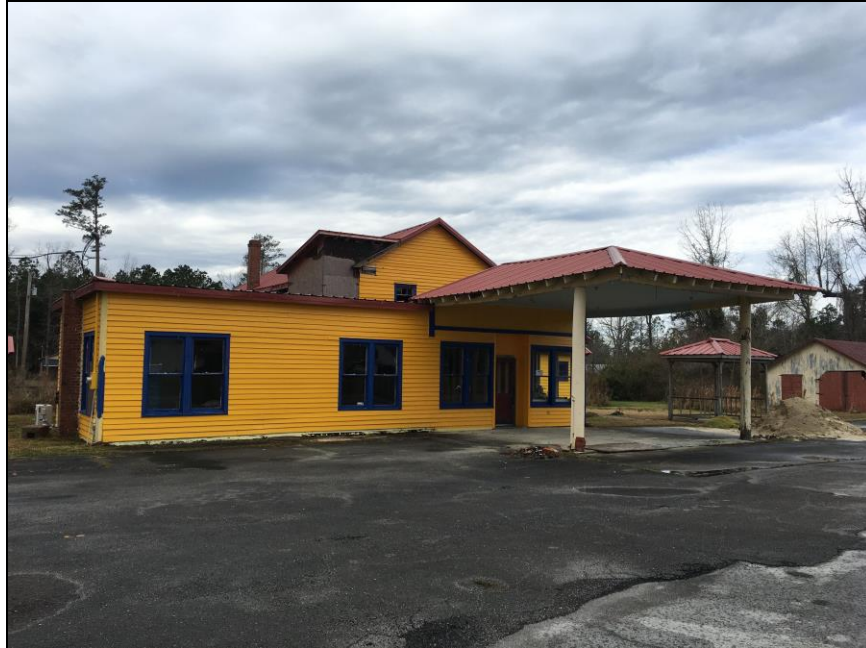
Figure 10: East elevation of Tom Haywood Store, looking northwest.
