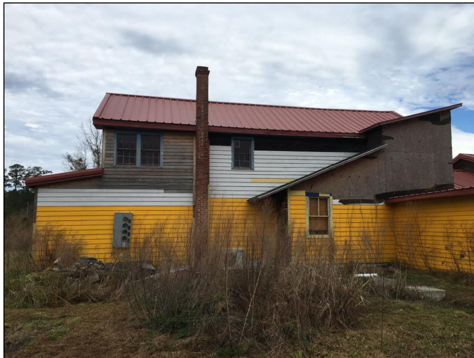
Figure 14: Tom Haywood Store, south elevation.
