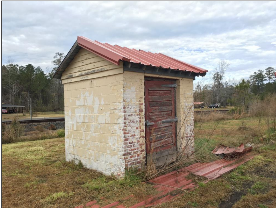
Figure 25: Pumphouse looking northwest.
