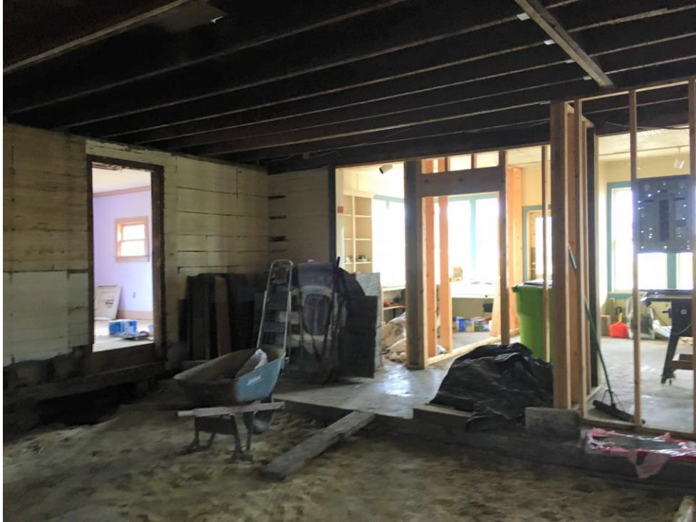
Figure 17: Interior of original two-story store portion, looking northeast.
