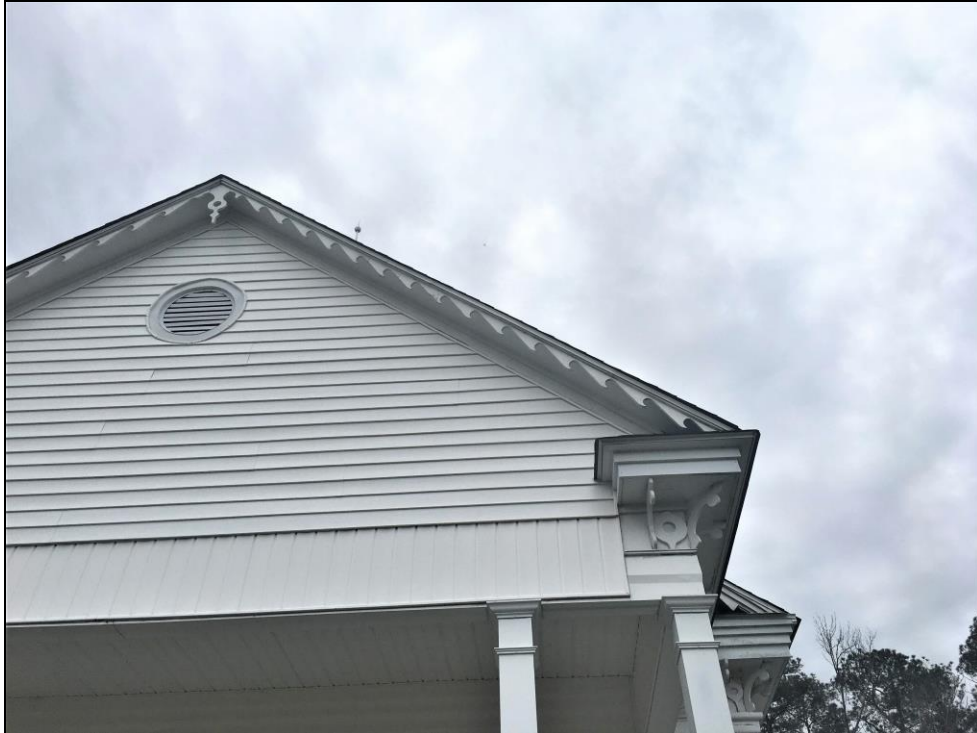
Figure 43: Detail of decorative sawn work on northeast elevation.
