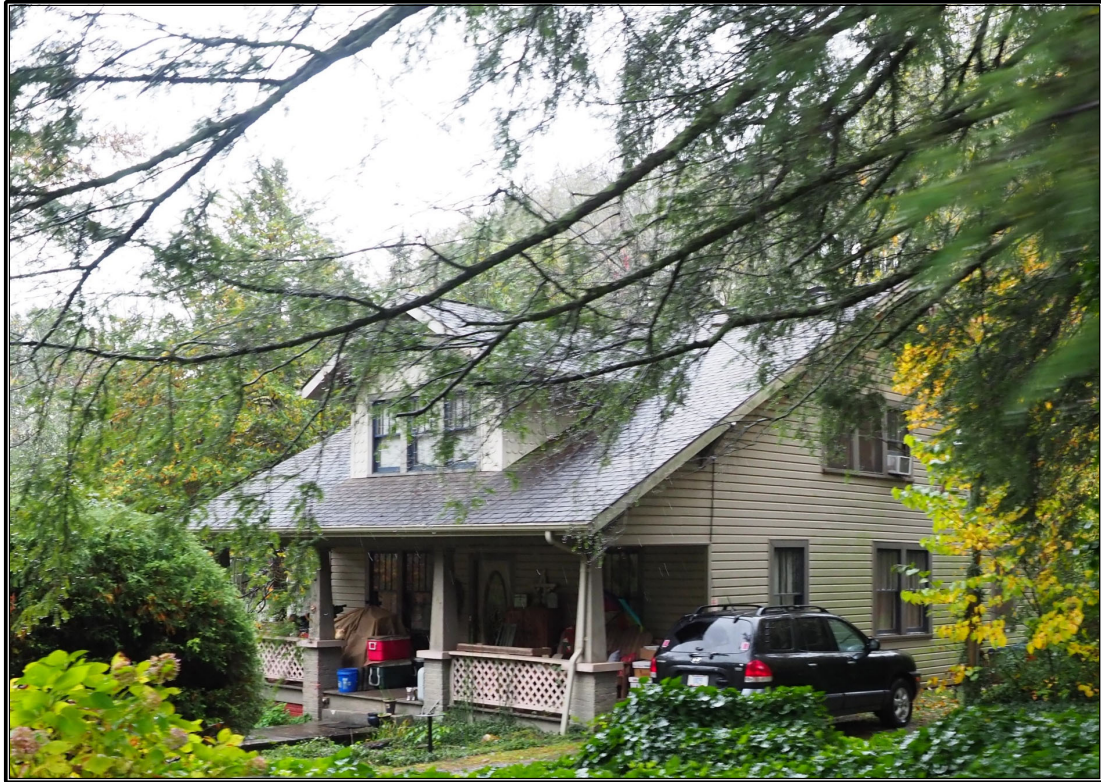
Figure 19. 147 Monteith Branch Road, Sylva, North Carolina.
