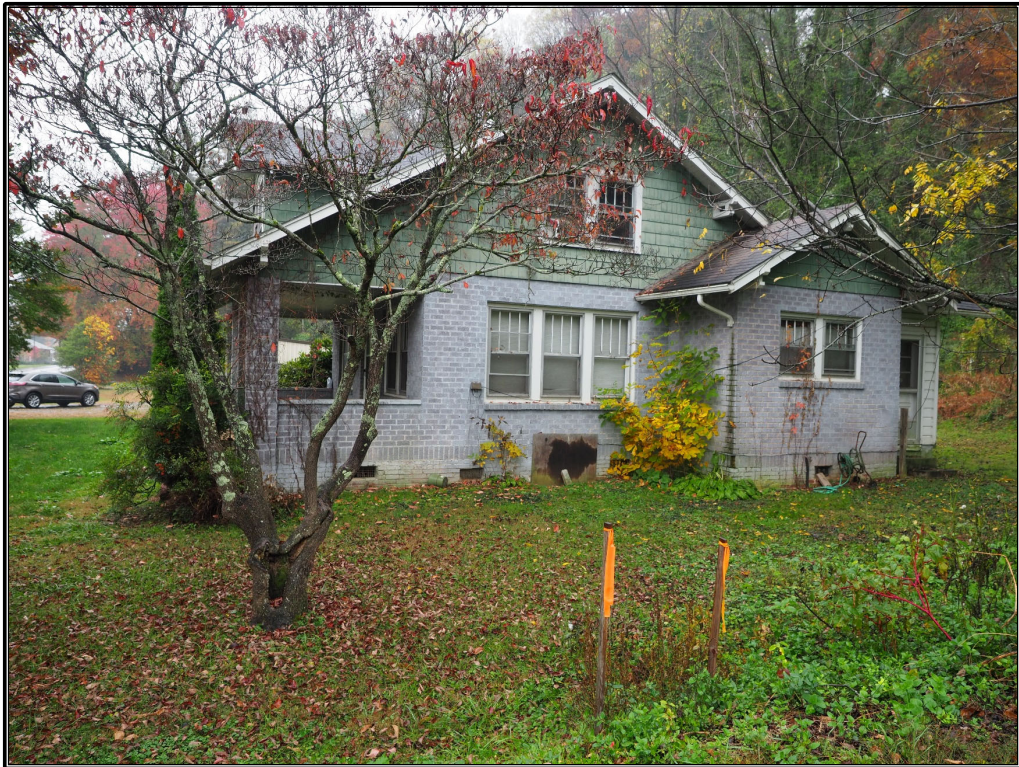
Figure 8. Northeast elevation, looking west.
