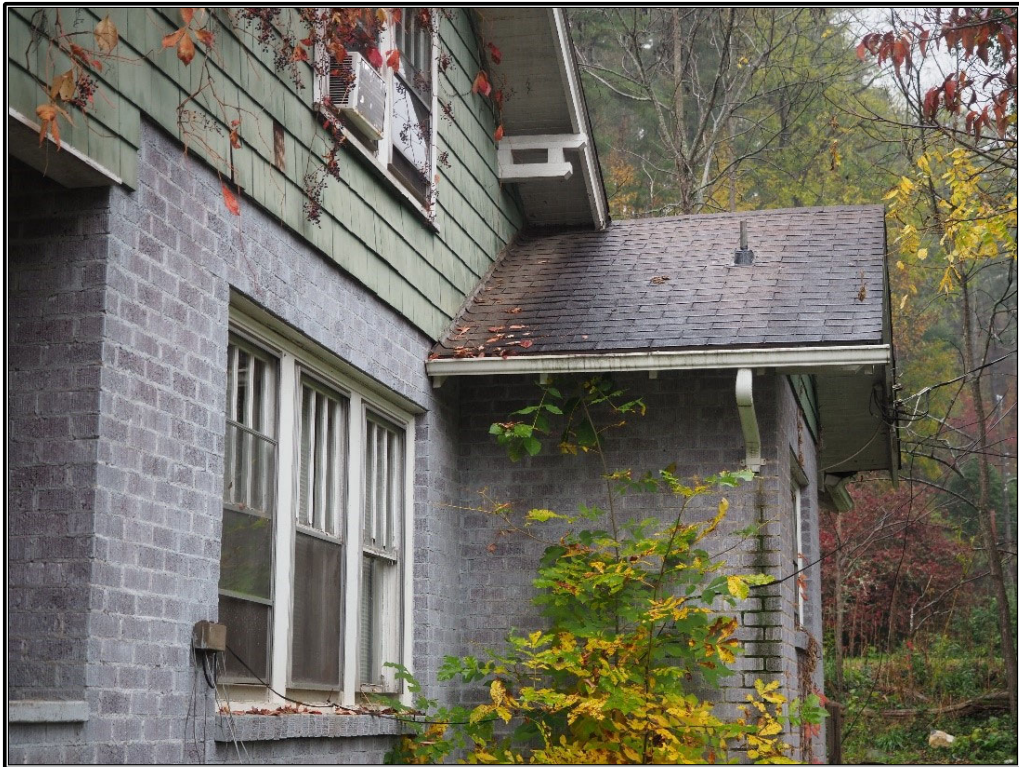
Figure 4. Bracket and shingle detailing.
