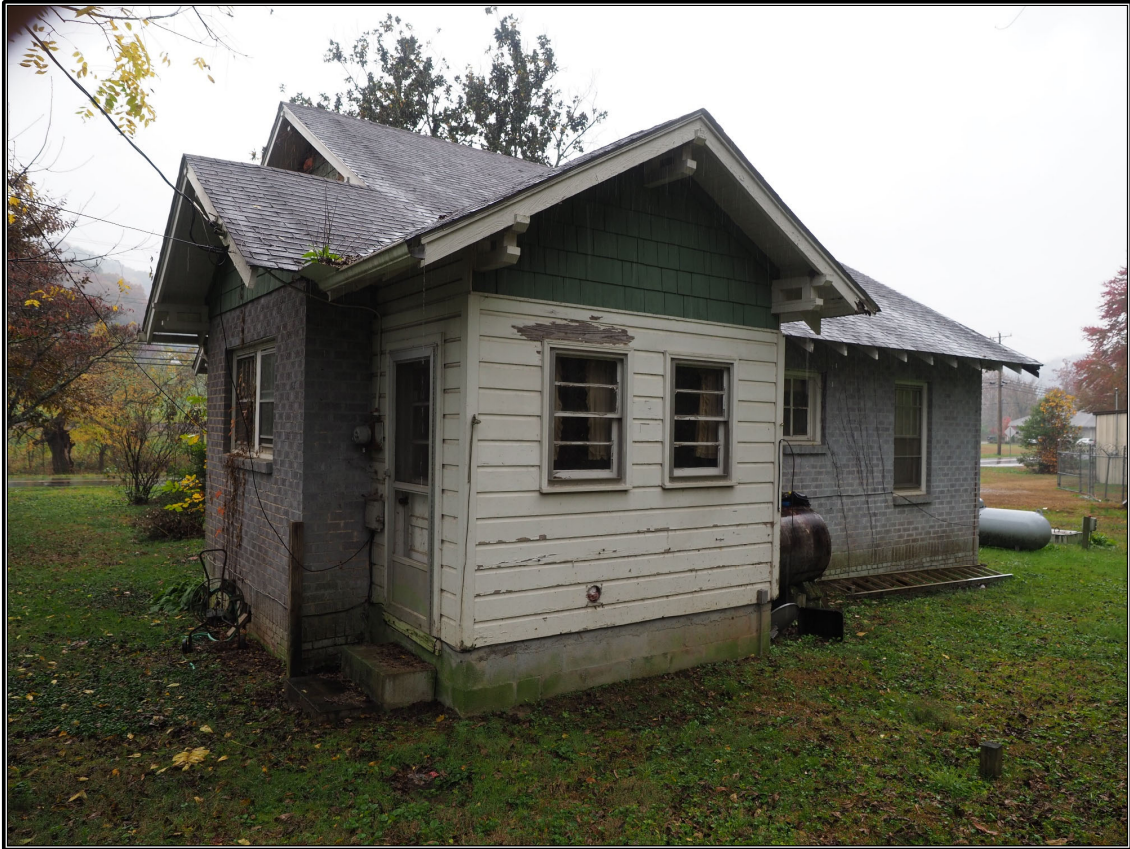
Figure 9. Northeast and rear elevations, looking south.
