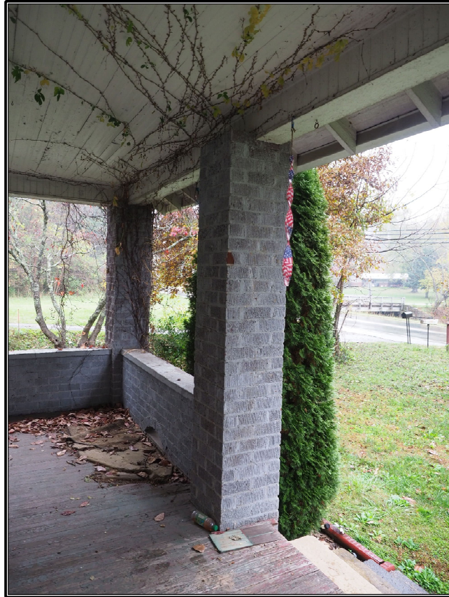
Figure 5. Porch column and balustrade arch detail on façade elevation.
