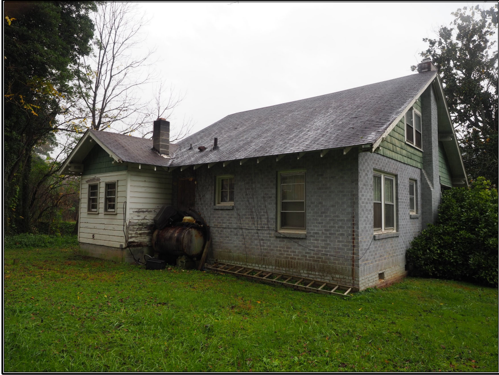
Figure 7. Rear and southwest elevations, looking northeast.
