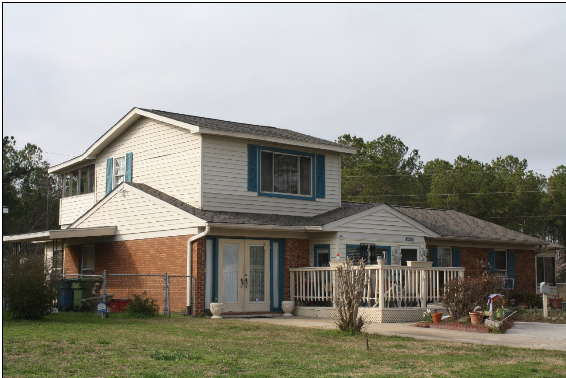
Figure 25: 1405 N. 26 th Street (House #13) enlarged one-story side-gable front entrance model
