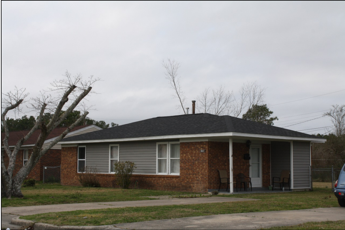
Figure 24: 2607 McClammy Street (House #12) hip-roofed, side gable model, newer vinyl siding and windows
