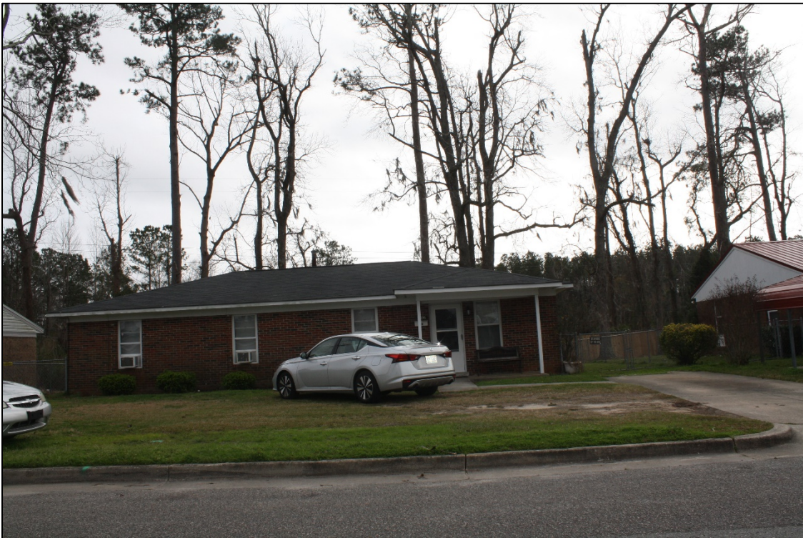
Figure 15: 2606 McClammy Street (House #3), hip-roofed, front entrance model
