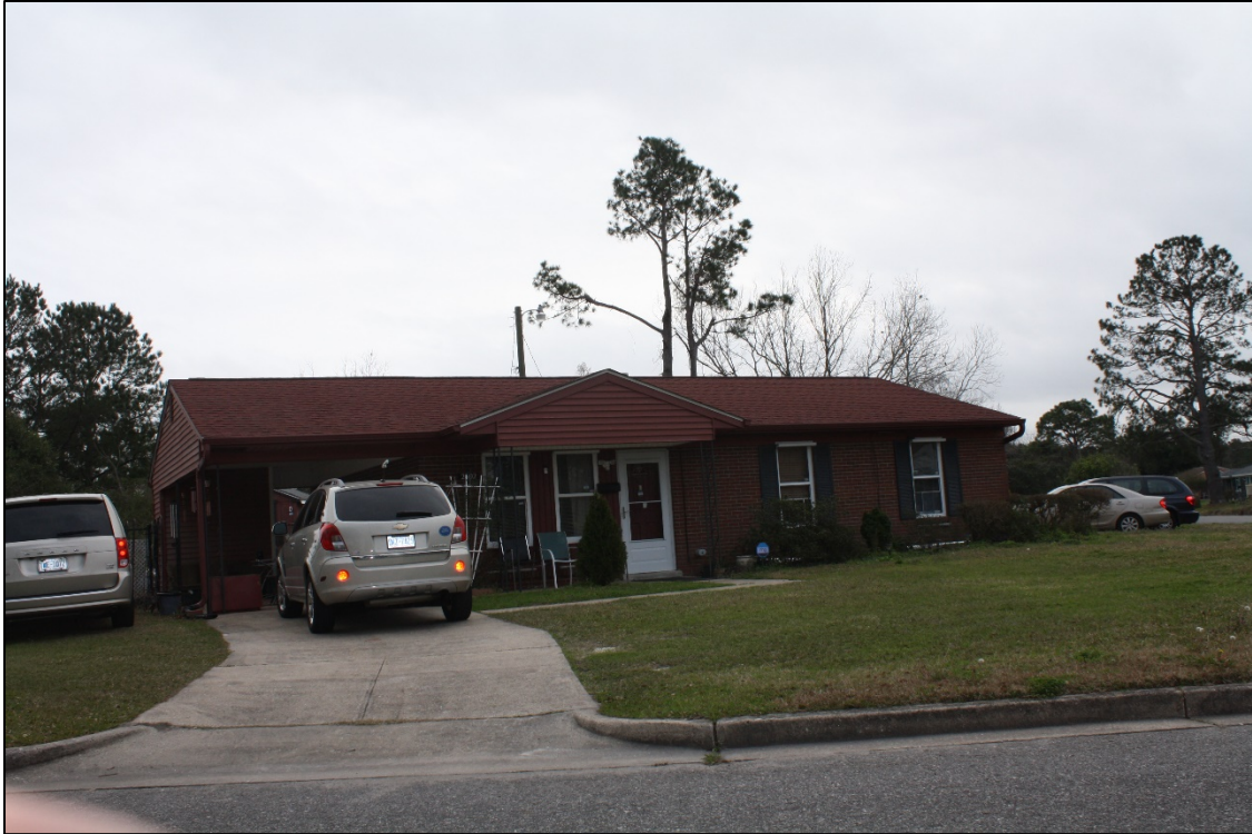
Figure 18: 2602 Bunche Street (House #6) side-gable front entrance with carport
