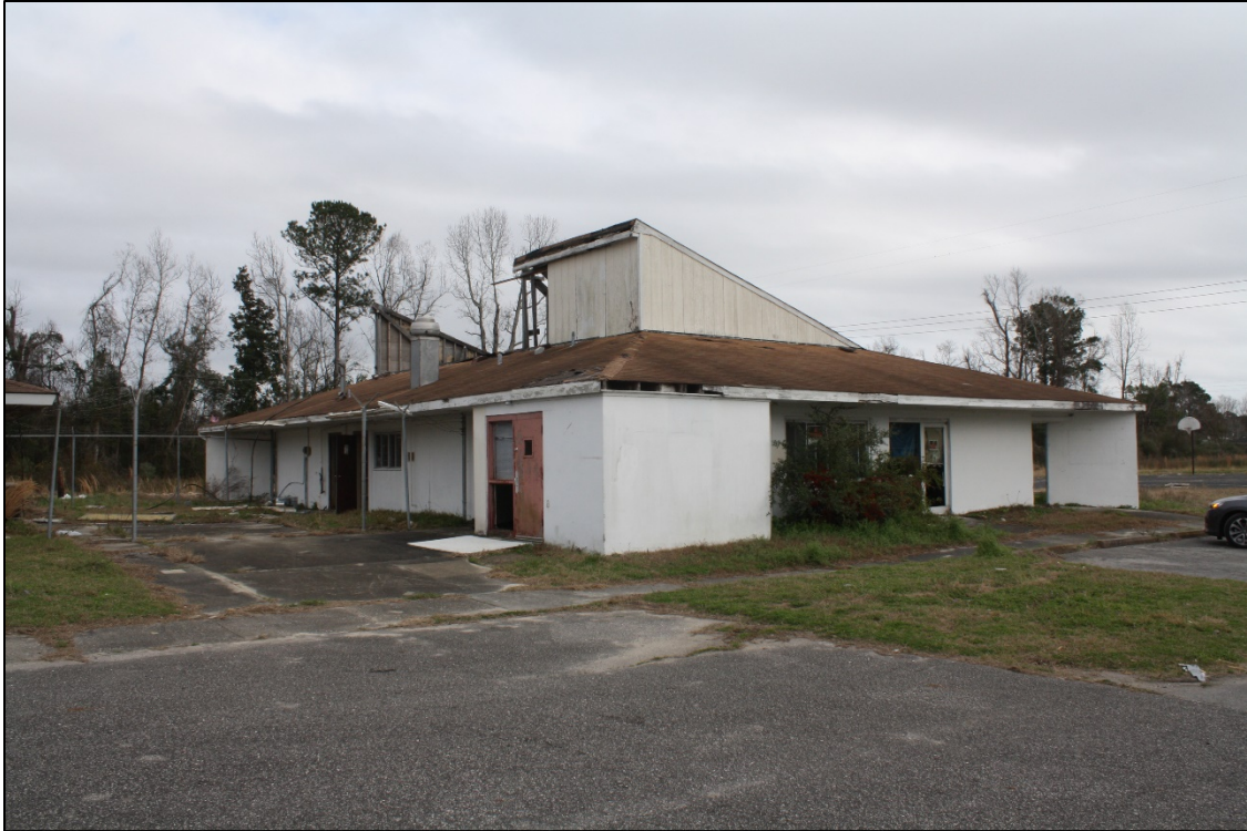
Figure 12: Looking east toward former Head Start building (now abandoned)
