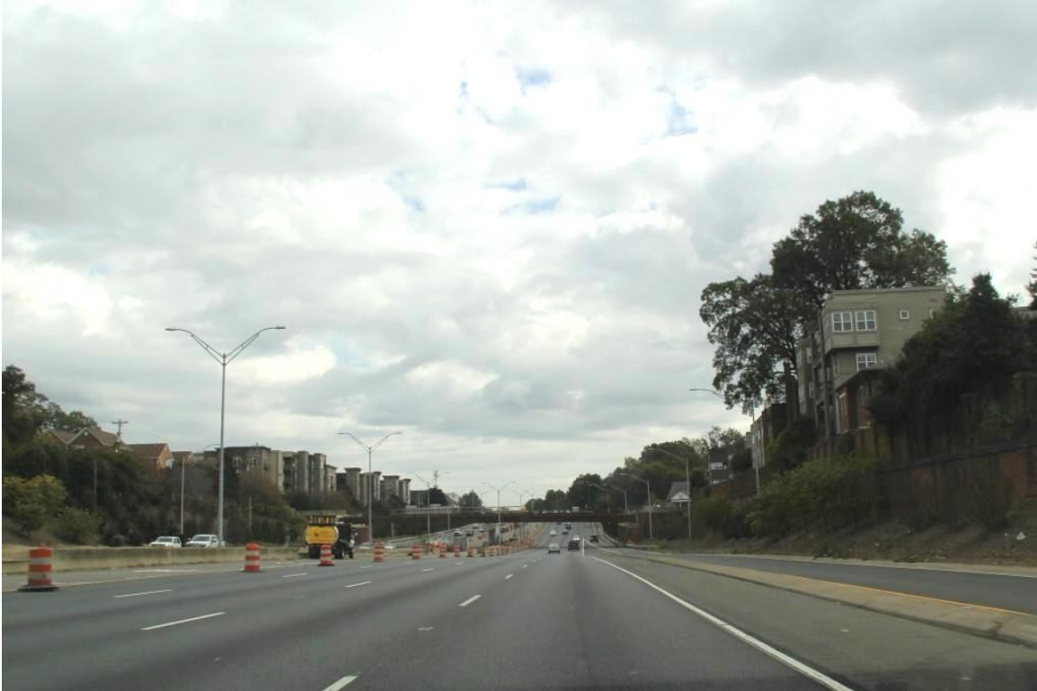
View east along Independence Boulevard (US 74) to Hawthorne Lane Bridge near project beginning
