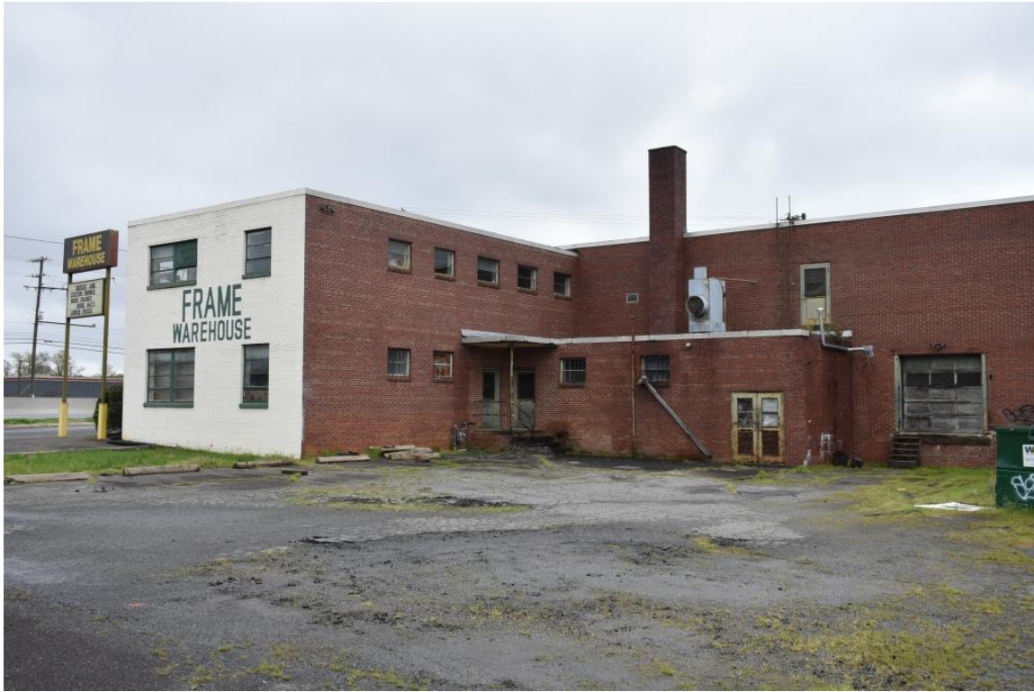
Barber Manufacturing Company, rear elevation, view to east
