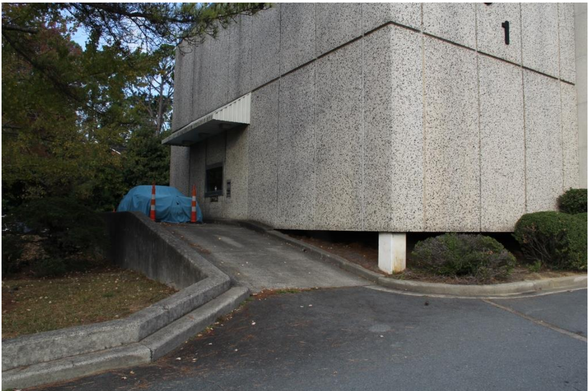
Allied Security Building, west elevation, oblique view to north
