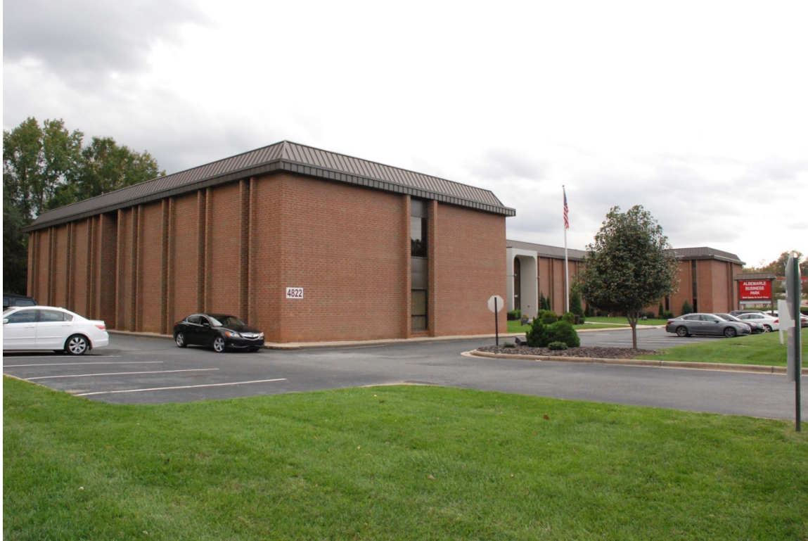
Albemarle Center, oblique front view to southwest
