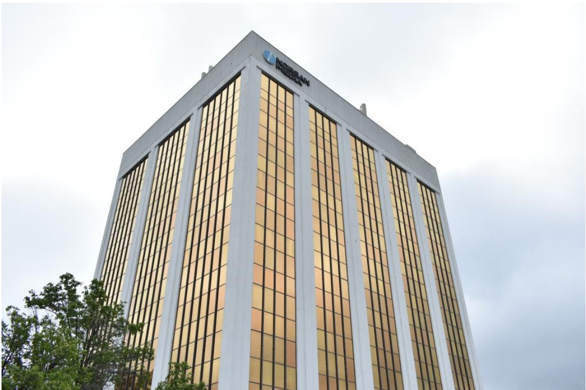
Independence Tower, oblique view to south
