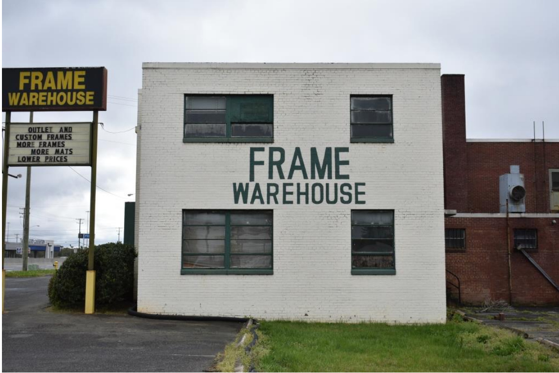
Barber Manufacturing Company, northwest elevation, view to southeast
