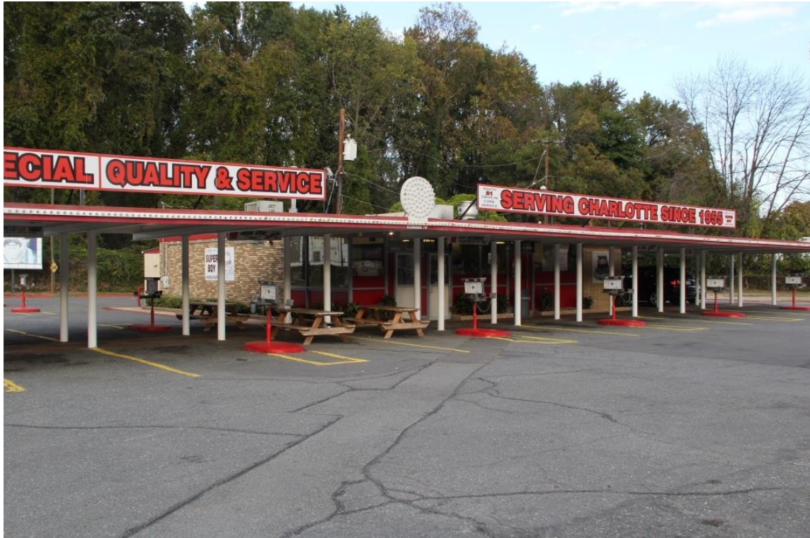
South 21 Drive-In No. 2, oblique front view to northeast
