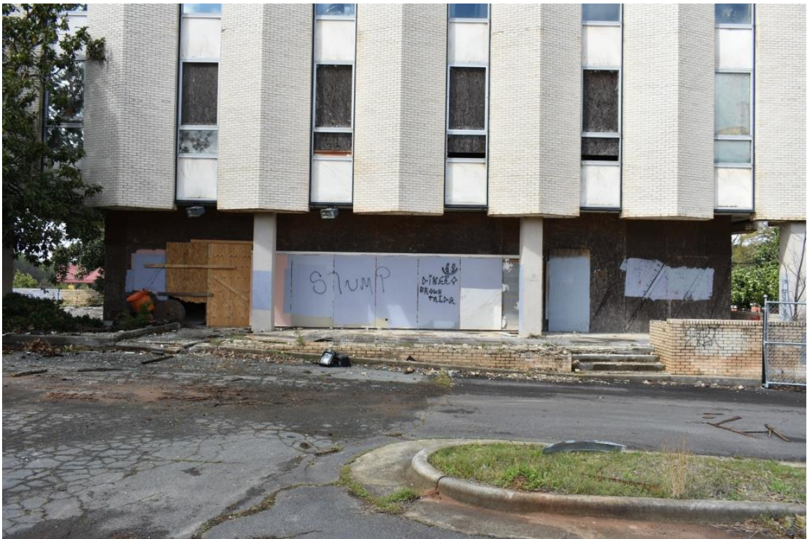
Ervin Building, east elevation, first floor detail, view to west
