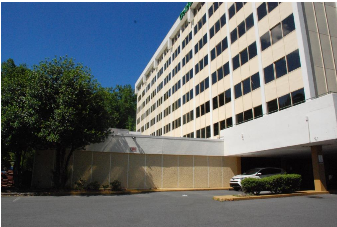
Coliseum Downtowner Motor Inn, east wing, view to north
