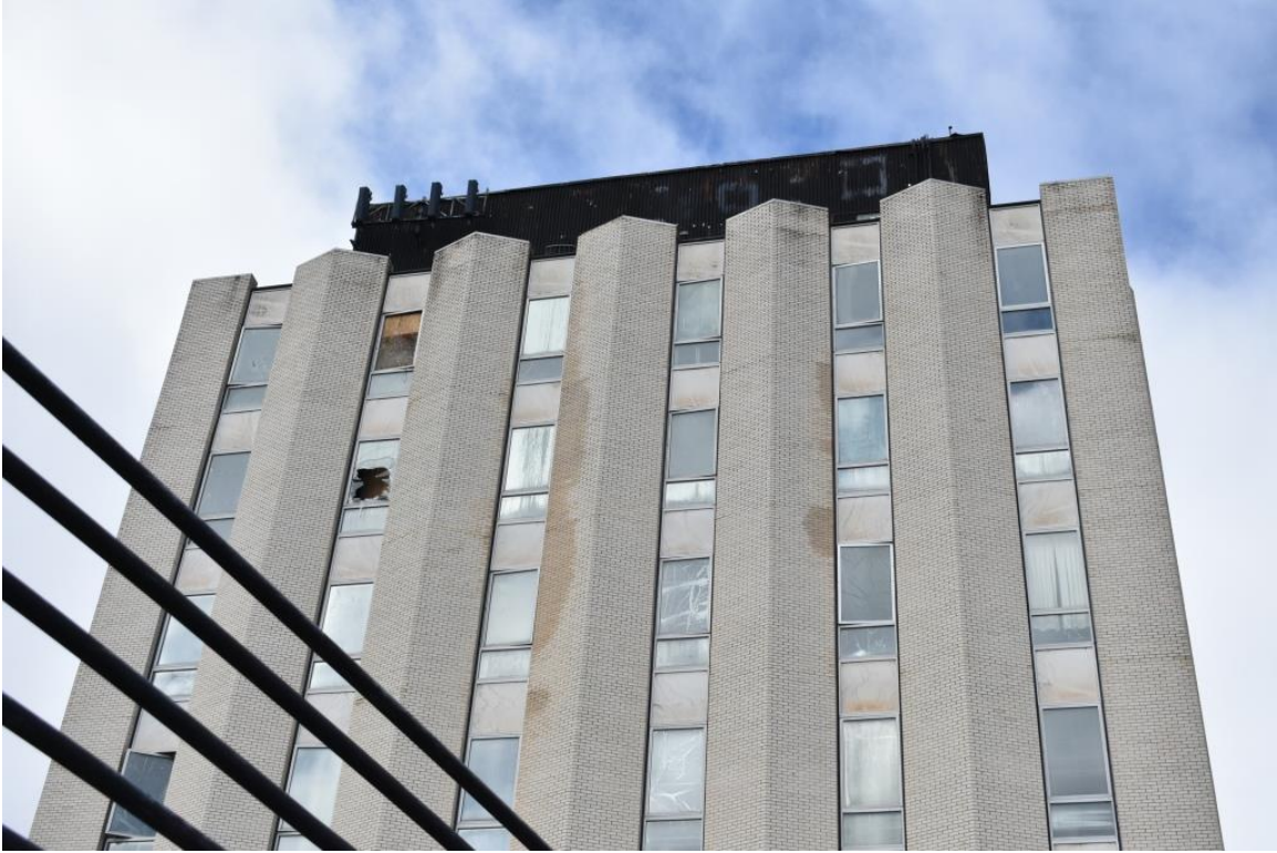
Ervin Building, east elevation detail, view to west
