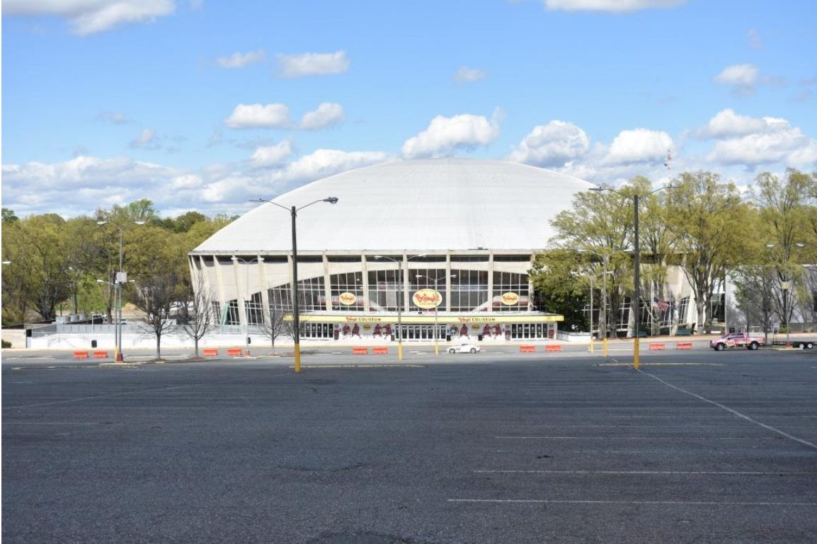
Charlotte Coliseum, façade, view to east
