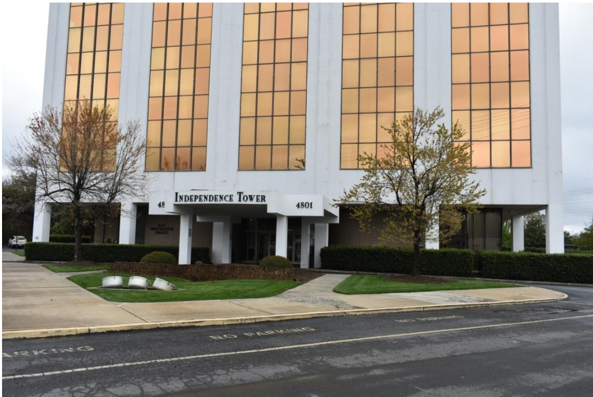
Independence Tower, entrance, view to east
