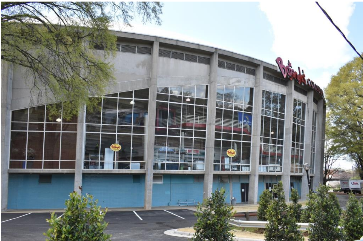
Charlotte Coliseum, oblique view to the west
