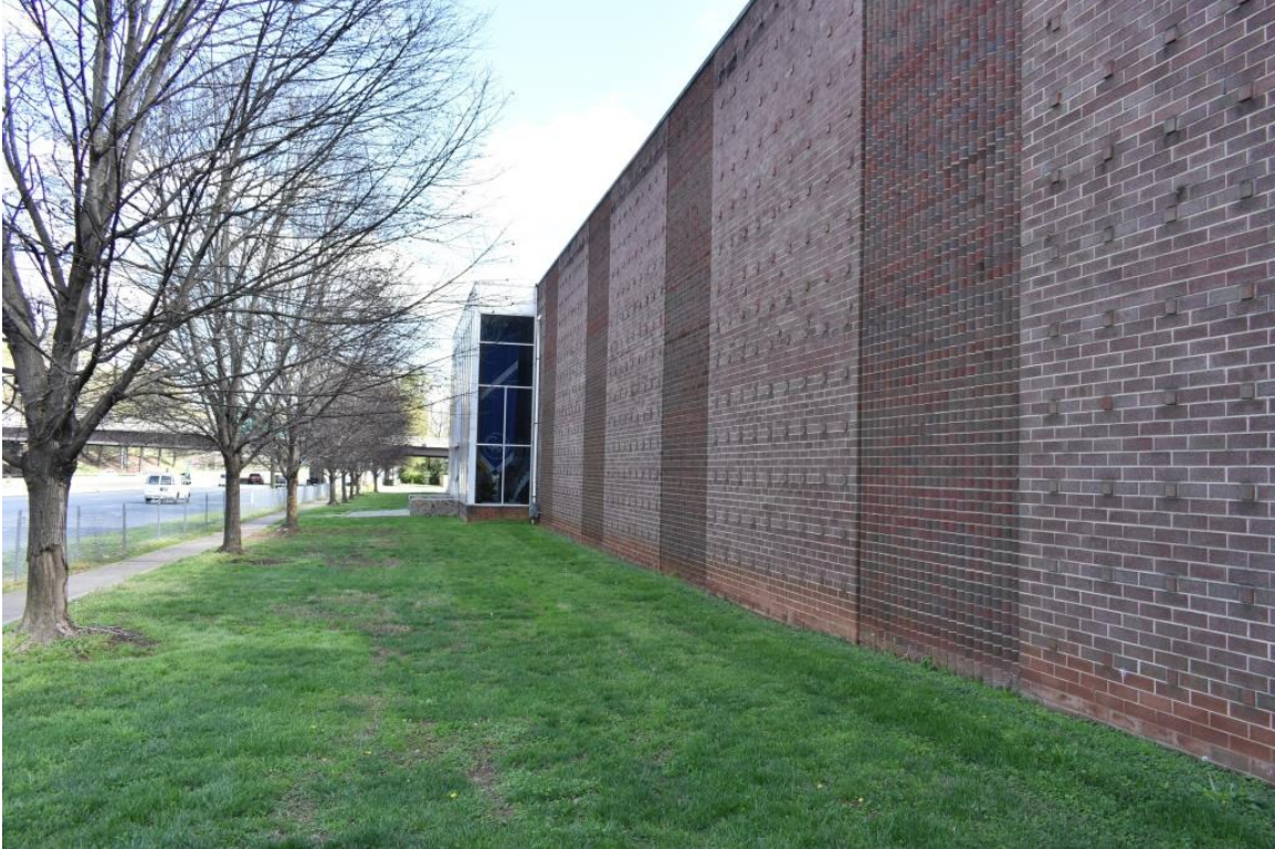
Charlotte Merchandise Mart, façade, oblique view to east
