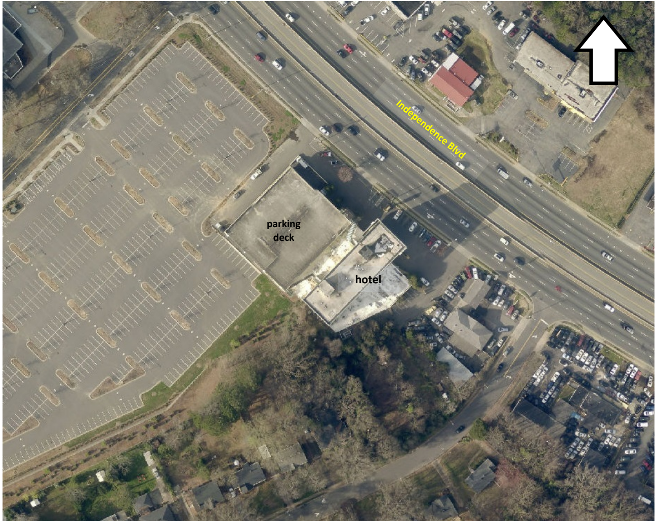
Site Plan – Coliseum Downtowner Motor Inn, 3024 E. Independence Boulevard (Source: Mecklenburg County GIS Polaris 3G)
