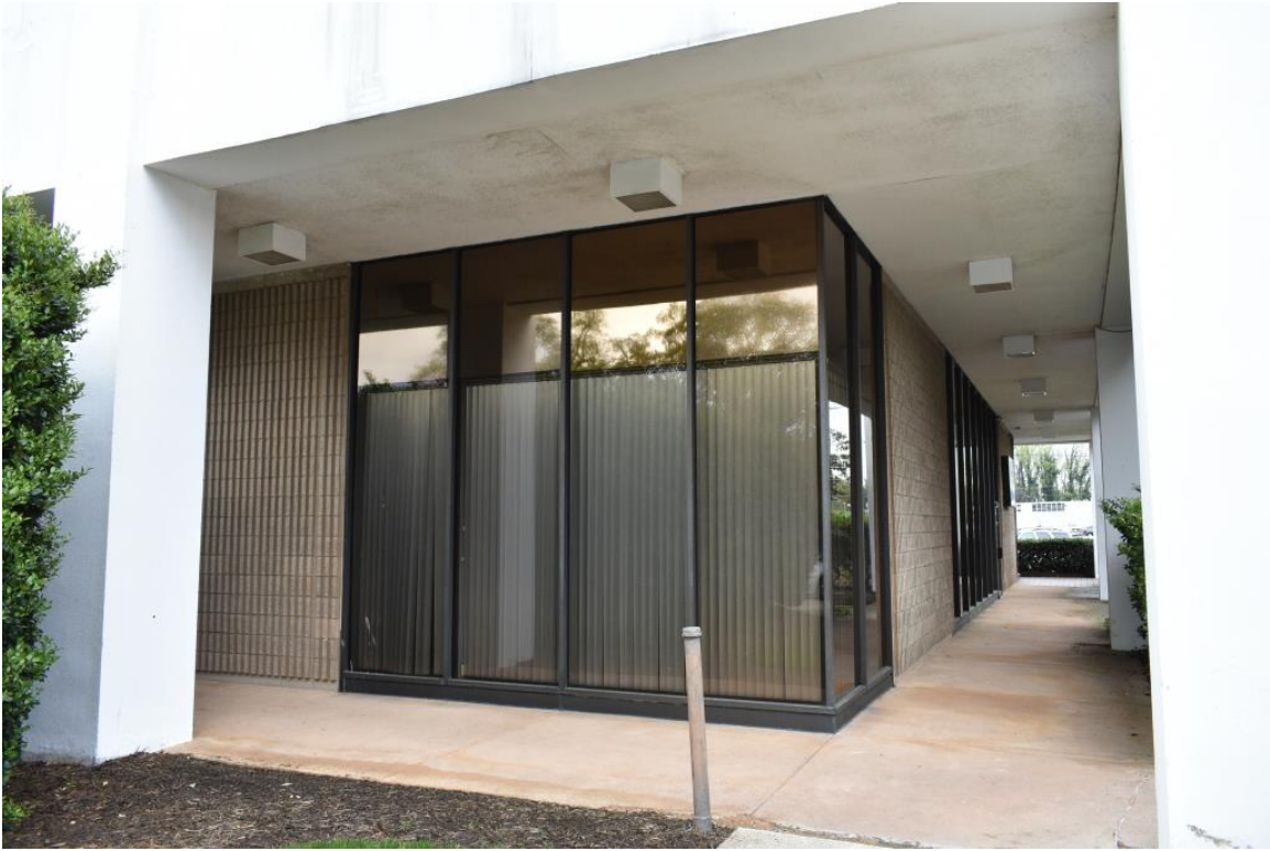
Independence Tower, first floor detail, view to west
