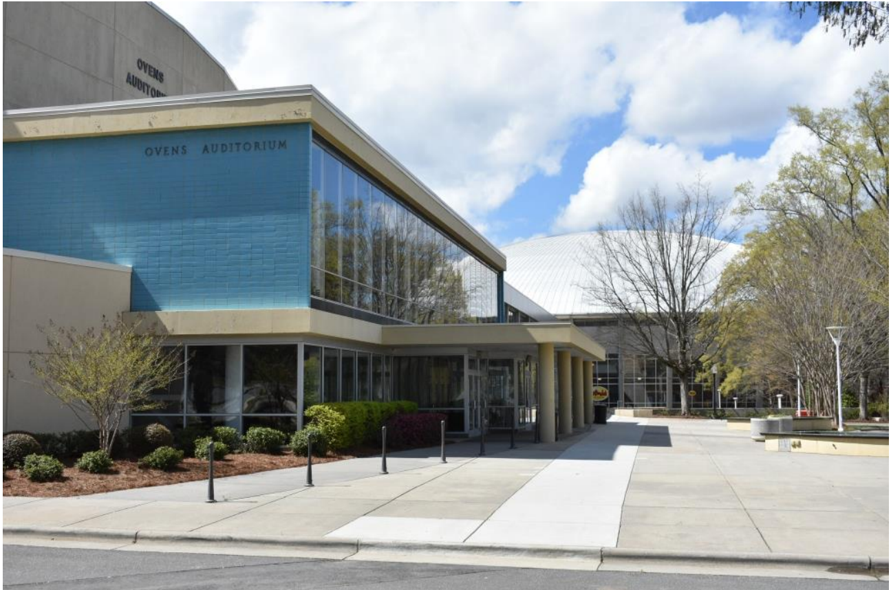
Old Charlotte Coliseum and Ovens Auditorium, view to northwest
