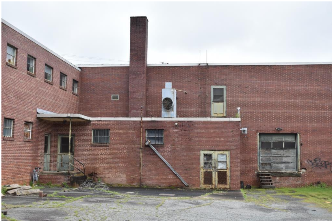
Barber Manufacturing Company, view to southeast
