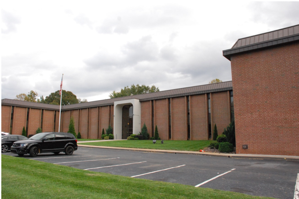
Albemarle Center, façade, oblique view to east
