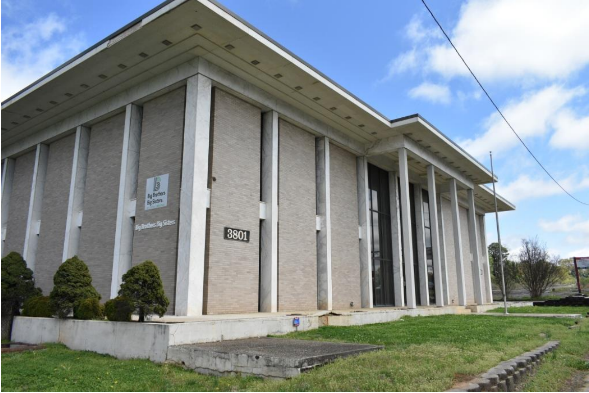
North Carolina Savings and Loan Building, façade, oblique view to northeast
