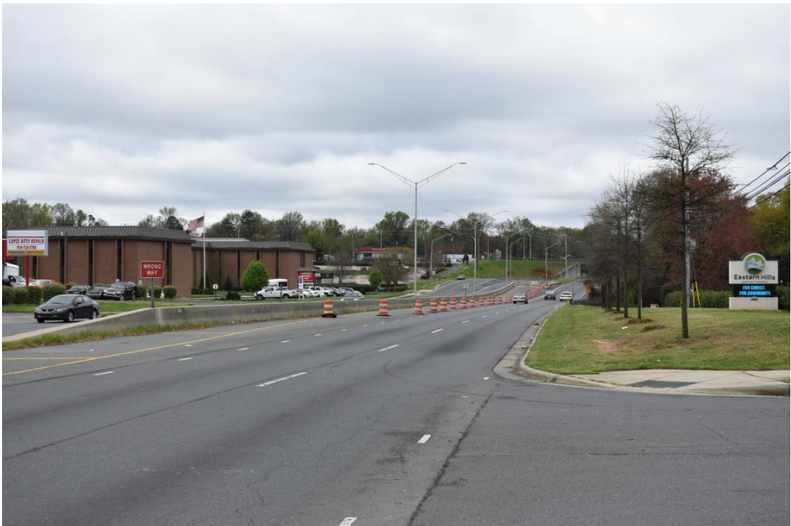
View southwest along Albemarle Road (NC 27) to intersection with Independence Boulevard
