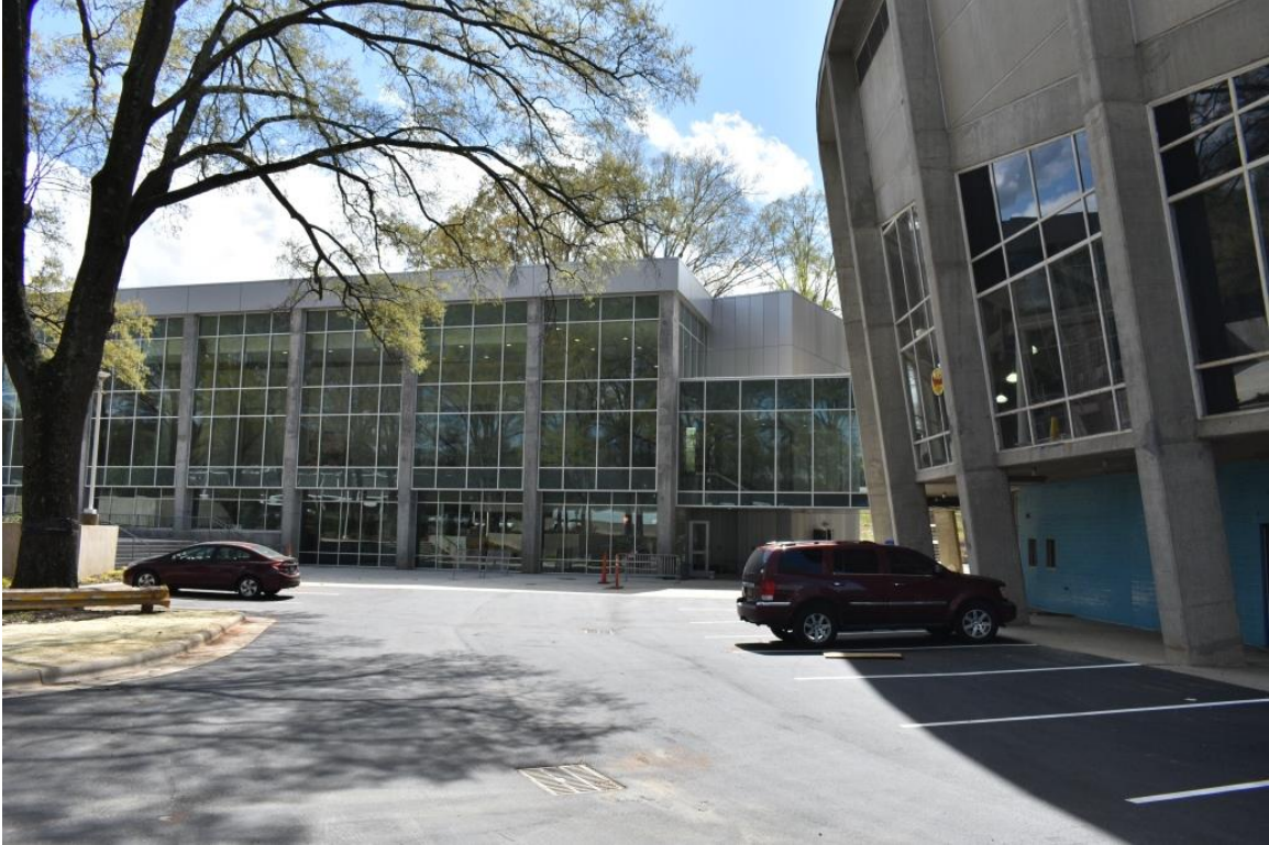
Charlotte Coliseum (r) and Coliseum-Auditorium LINK Connector Facility (l), view to west
