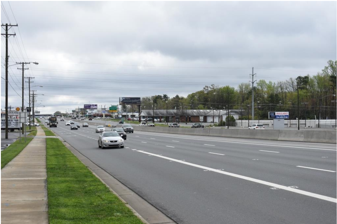
View southeast along Independence Boulevard from North Sharon Amity Road
