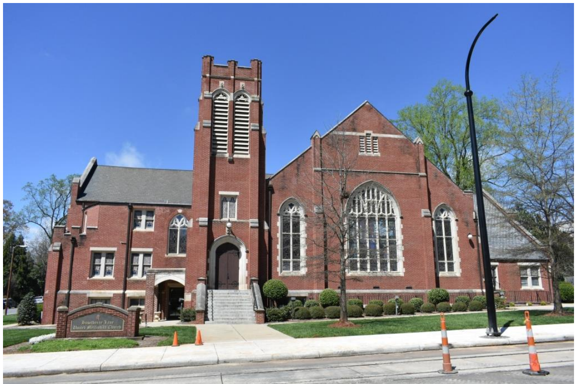
Hawthorne Lane United Methodist Church (MK0956), 501 Hawthorne Lane, view to northwest
