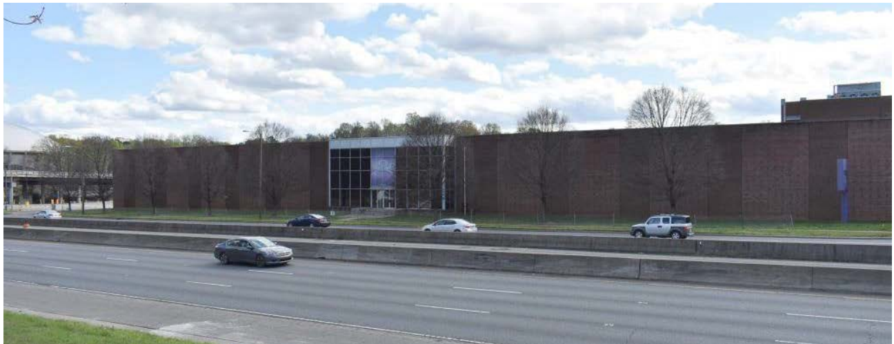
Charlotte Merchandise Mart, 800 Briar Creek Road, façade, view south across Independence Boulevard
