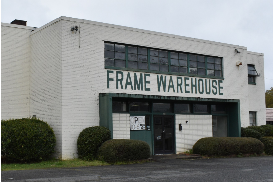
Barber Manufacturing Company, oblique front view to northwest
