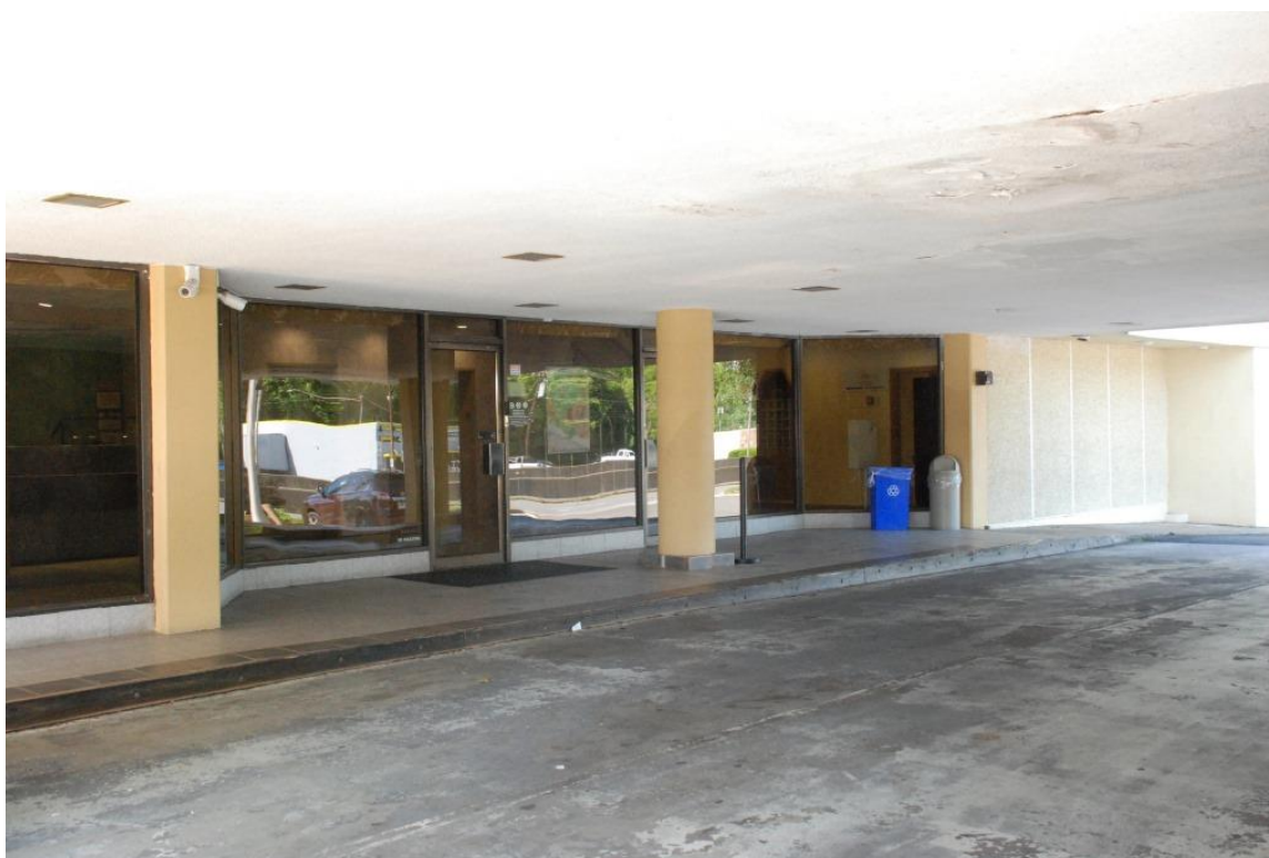
Coliseum Downtowner Motor Inn, entrance detail, view to west
