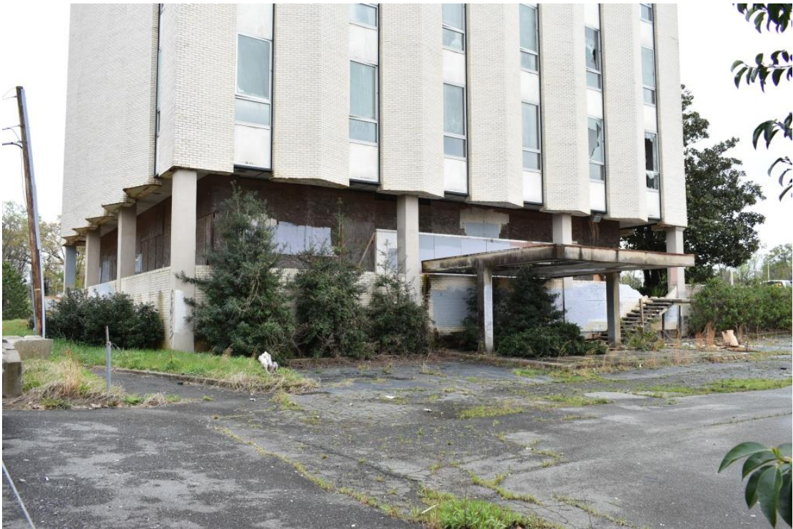
Ervin Building, west elevation detail, oblique view to south
