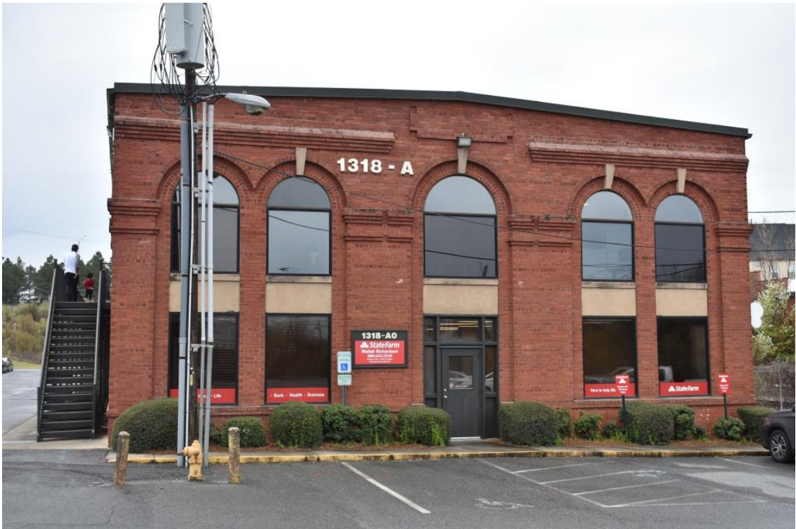
Heating Plant, north elevation, view to south
