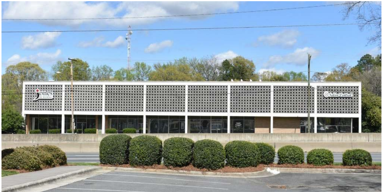
J. N. Pease Associates, 2925 East Independence Boulevard, façade, view to north
