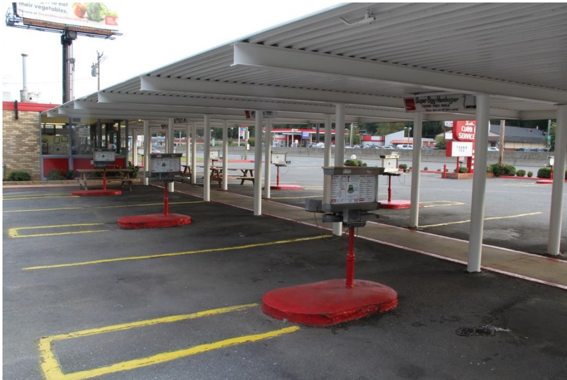
Menu stands and canopy rear view, view to southeast
