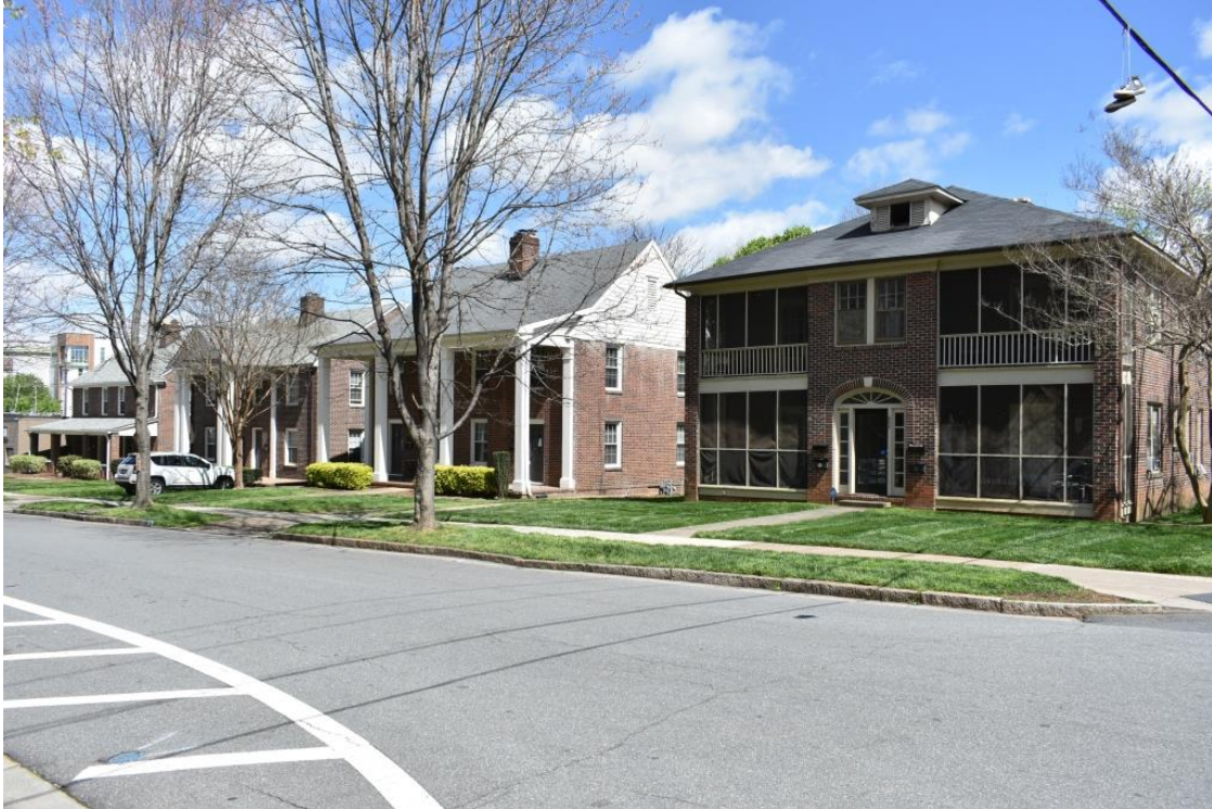
Elizabeth Historic District Boundary Reduction – contributing resources, 800 block Lamar Avenue, view to northeast
