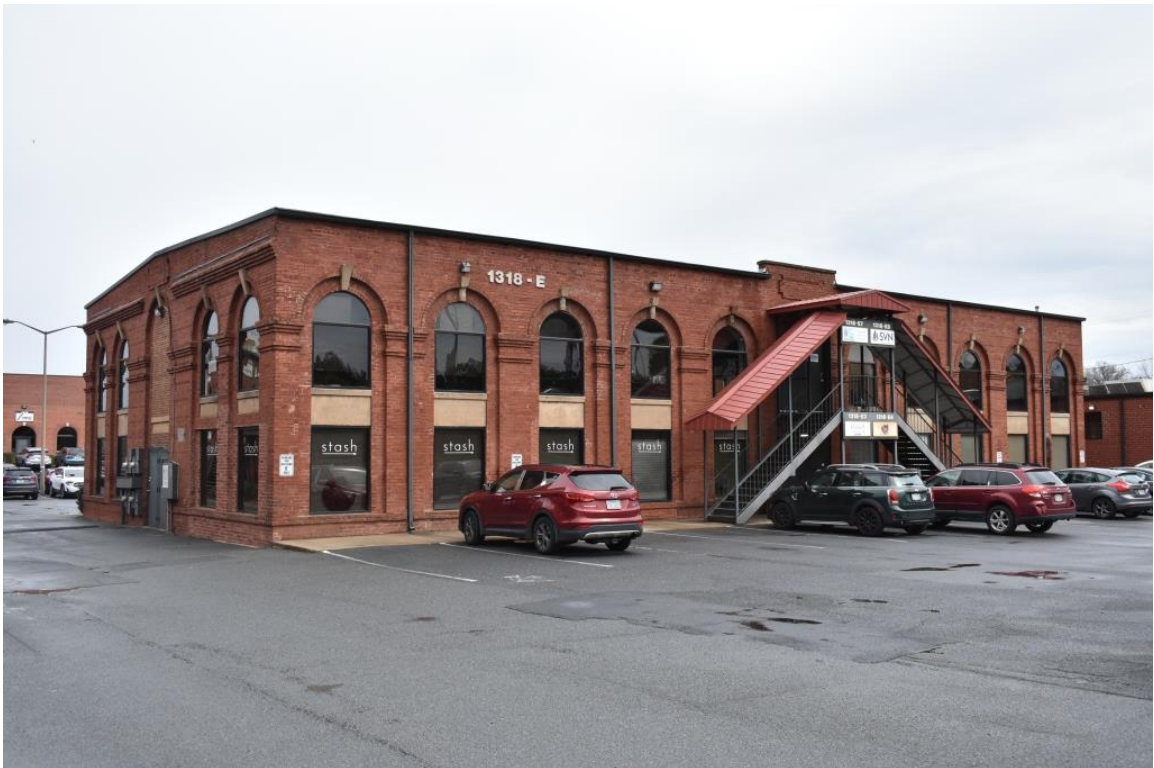
Machine Shop, oblique view to northeast
