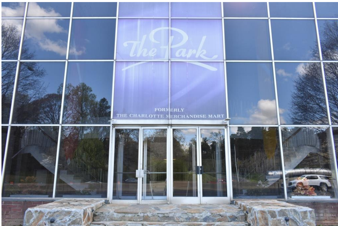
Charlotte Merchandise Mart, entrance pavilion, view to south
