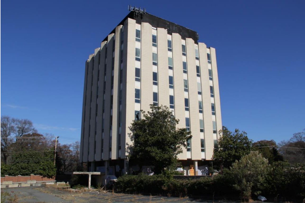
Ervin Building, oblique front view to northeast
