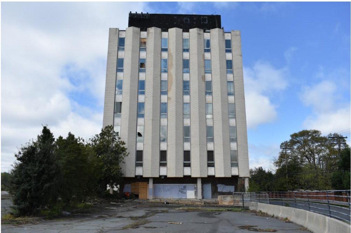
Ervin Building, east elevation, view to west
