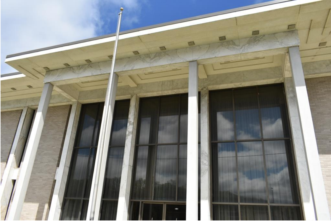
North Carolina Savings and Loan Building, entrance bay, view to north
