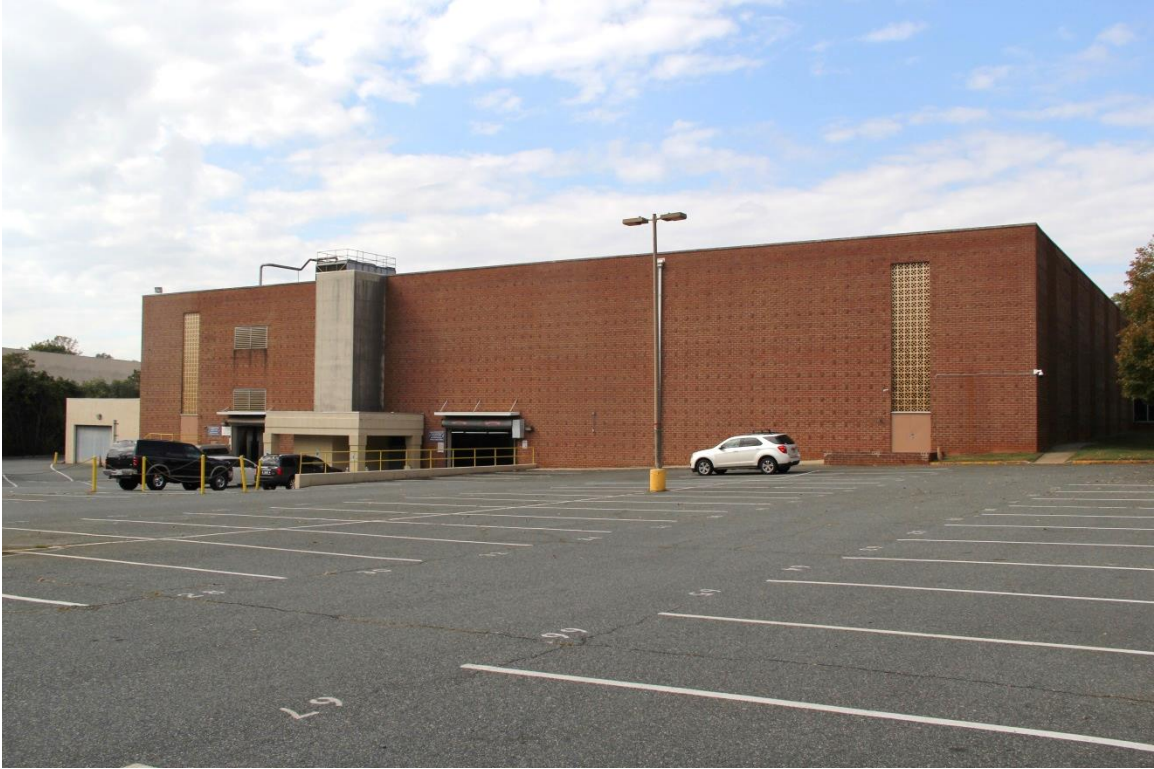
Charlotte Merchandise Mart, east elevation, view to west
