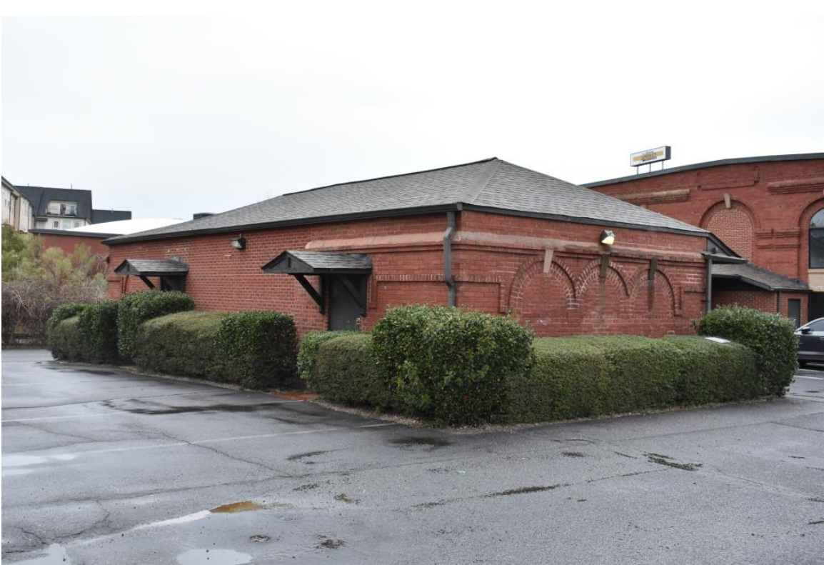
Heating Plant, view to northwest
