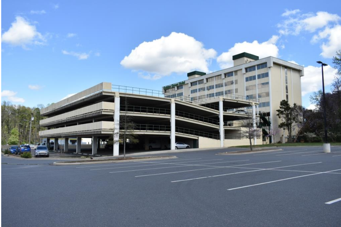
Coliseum Downtowner Motor Inn, parking deck, oblique rear view to east
