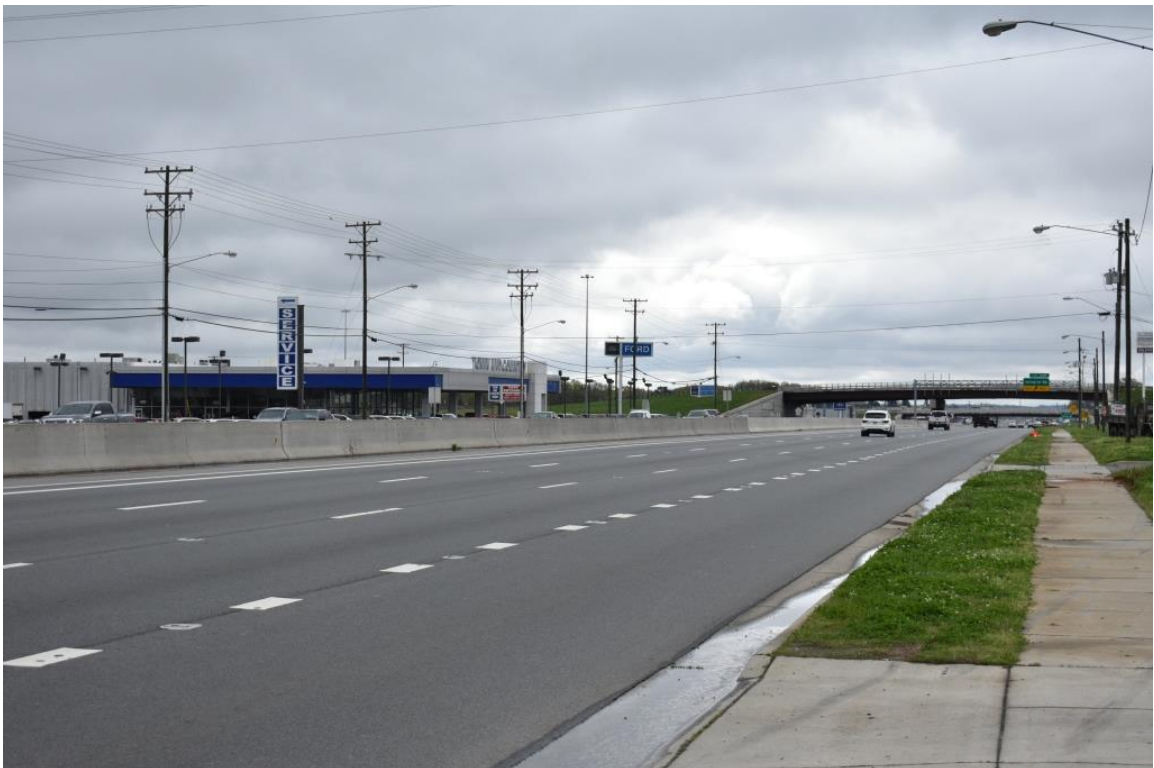
Project end, view southeast along Independence Boulevard to Idlewild Road (SR 3143)
