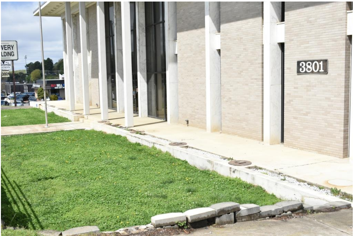
North Carolina Savings and Loan Building, view to northwest
