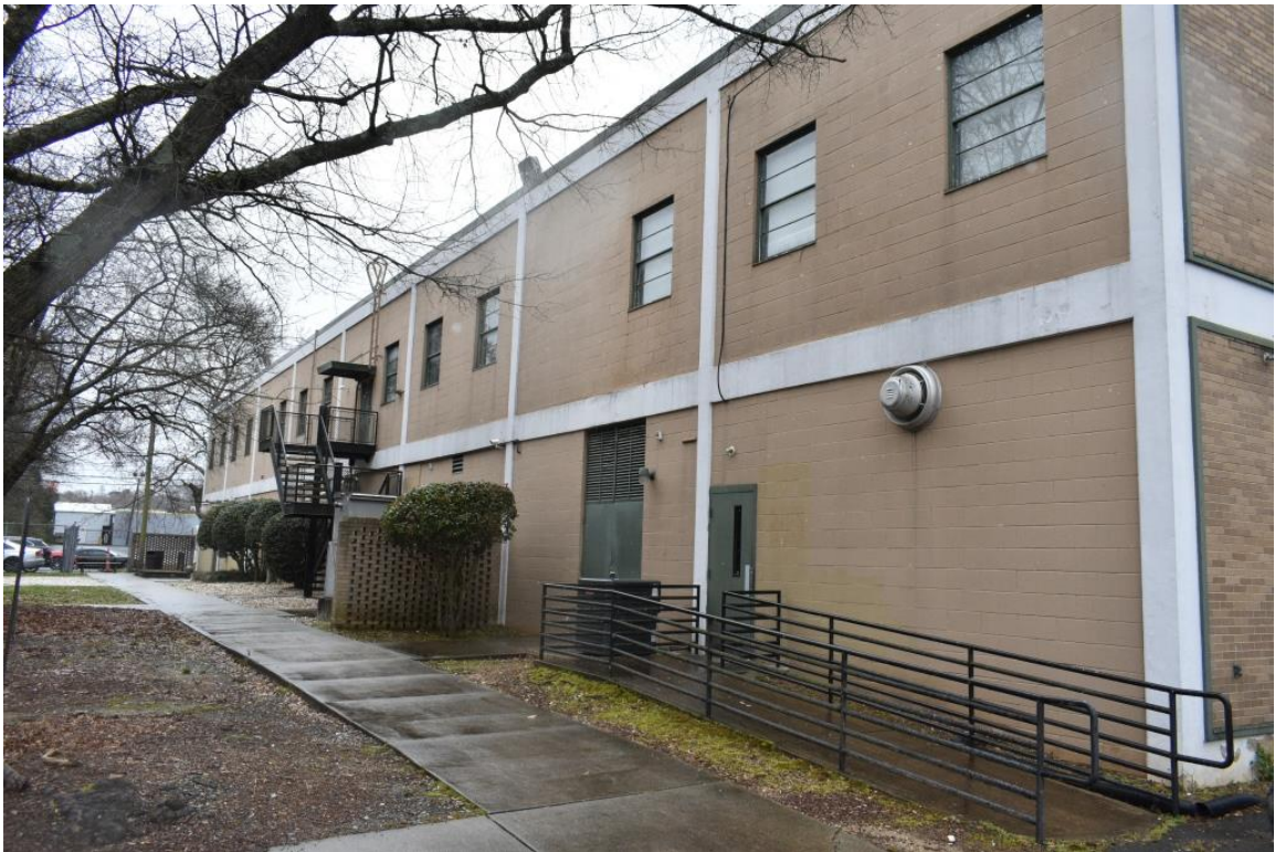
J. N. Pease Associates, north corner, view to south
