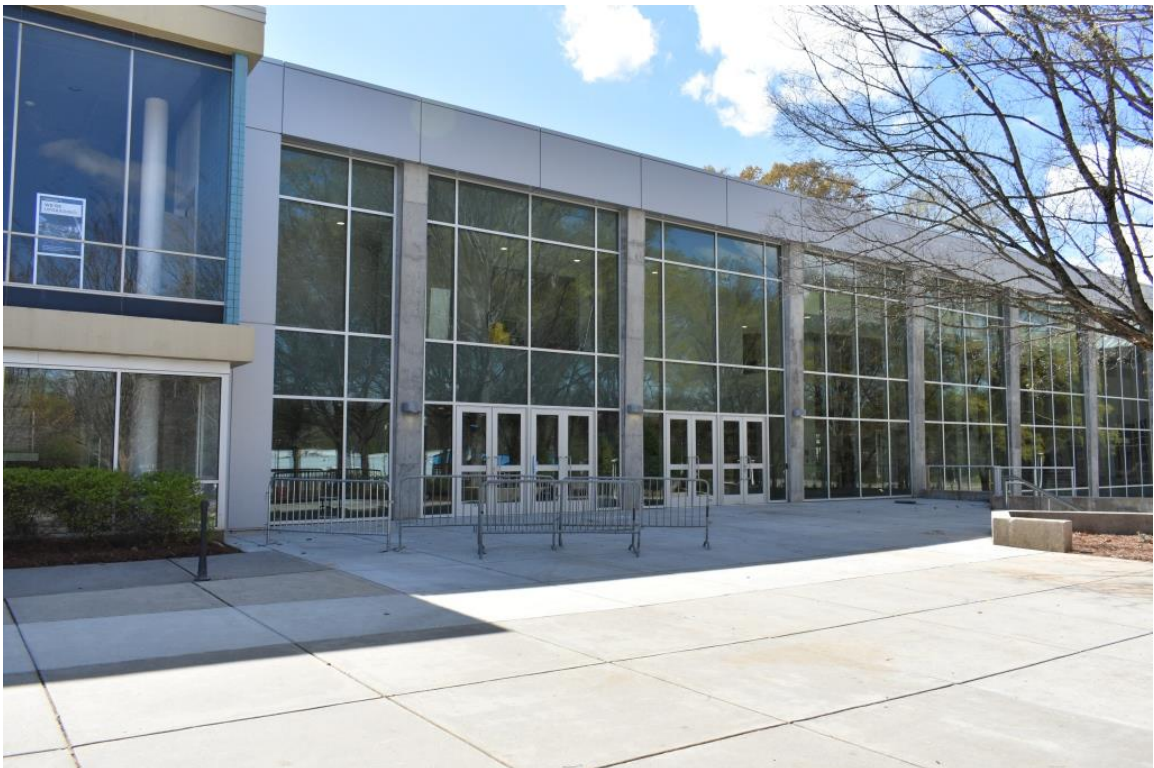
Coliseum-Auditorium LINK Connector Facility, view to west
