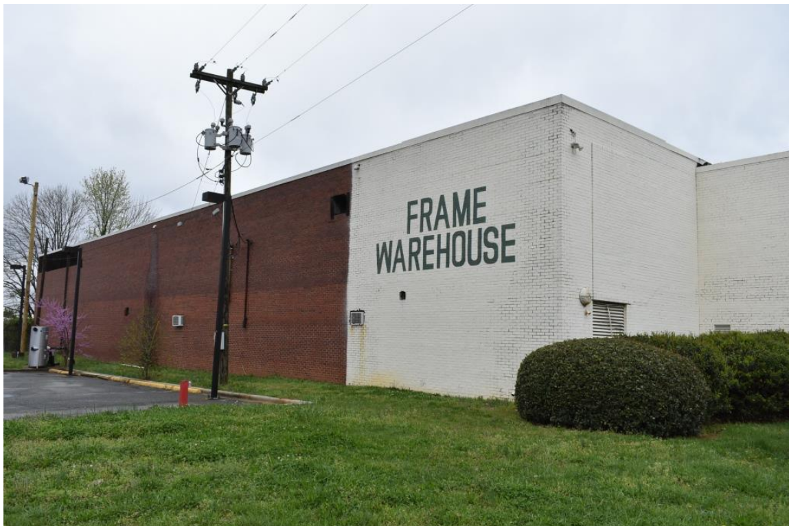
Barber Manufacturing Company, southeast elevation, oblique view to west
