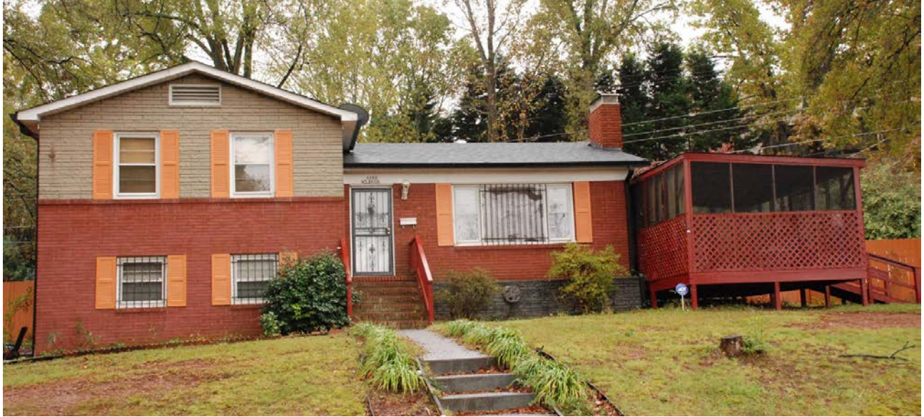
House, 4400 Holbrook Drive
