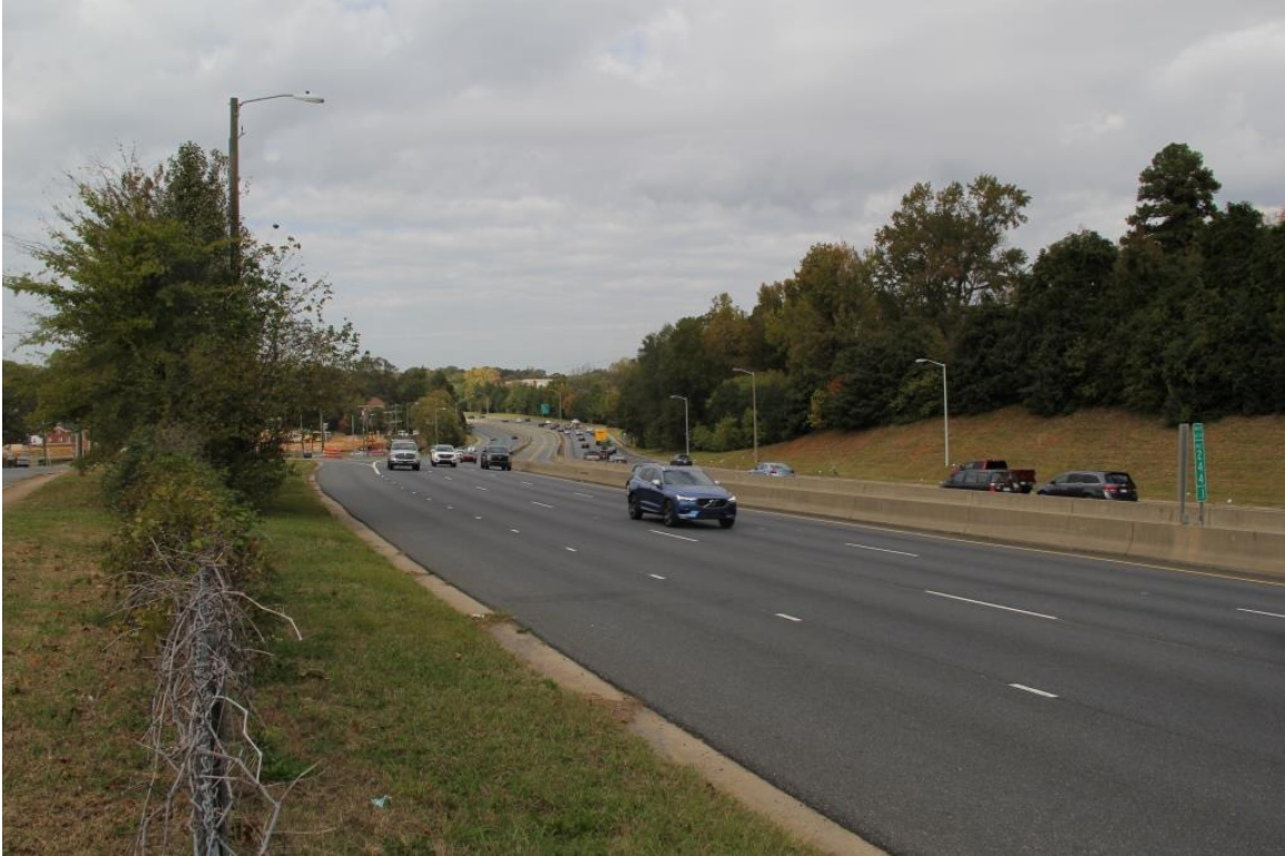
View northwest along Independence Boulevard near Rockway Drive
