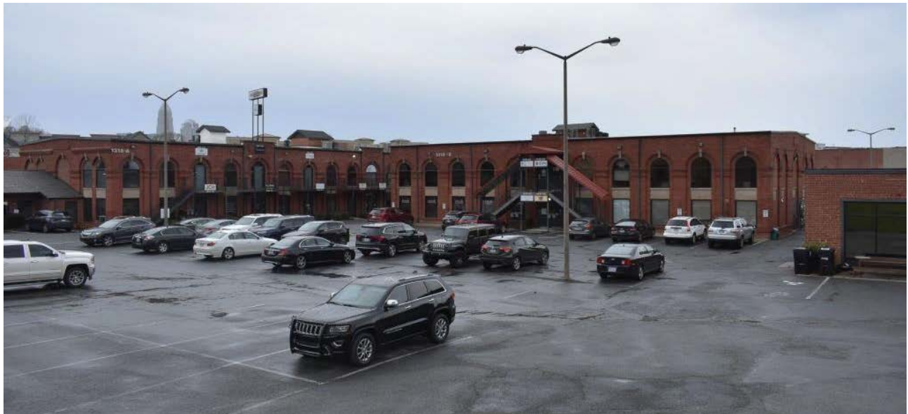
Cole Manufacturing Company Plant, 1318 Central Avenue, view to northwest
