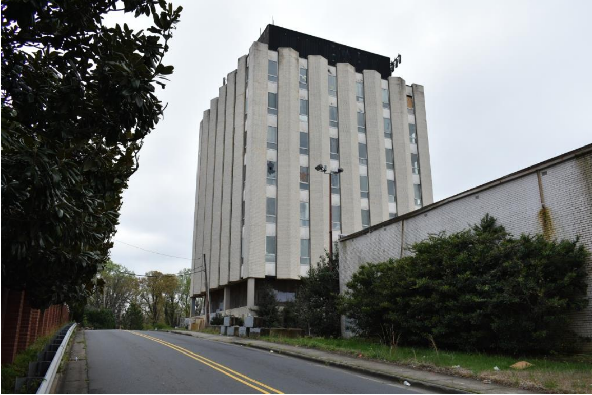
Ervin Building, oblique rear view to southeast along Bamboo Street
