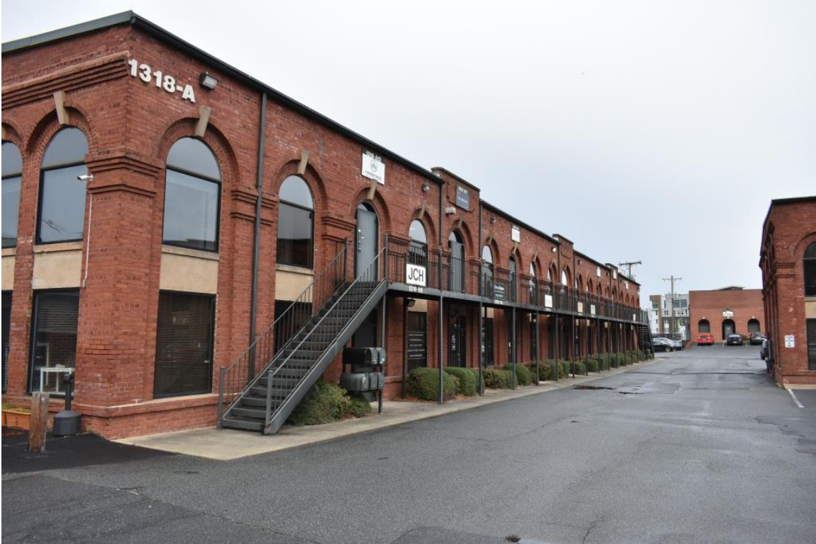
Assembly Building, east elevation, view to north
