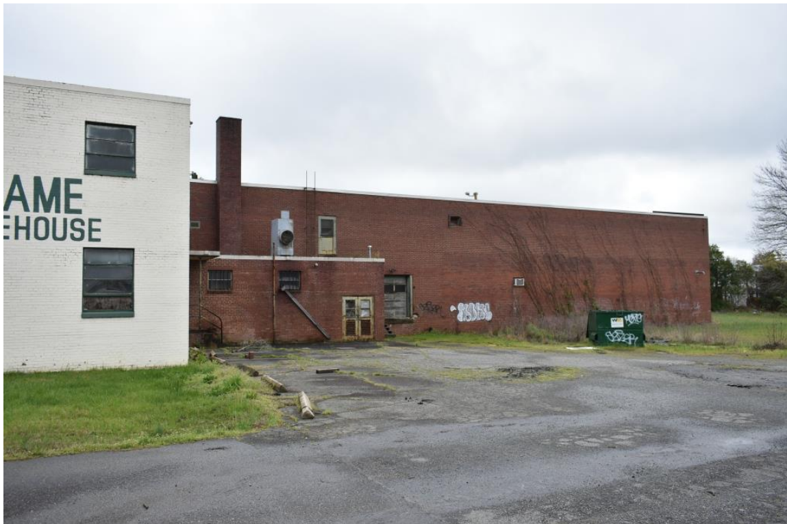
Barber Manufacturing Company, northwest elevation of production wing, oblique view to south
