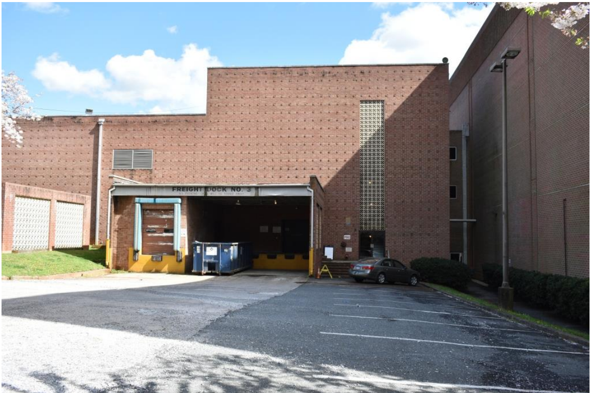
Charlotte Merchandise Mart, west elevation, view to east
