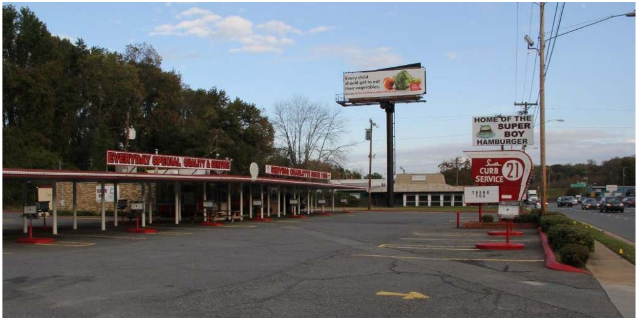
South 21 Drive-In No. 2, 3101 East Independence Boulevard, view to east
