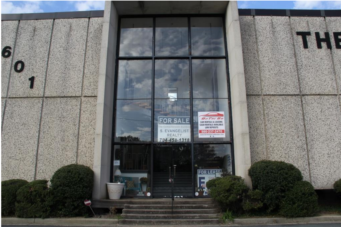
Allied Security Building, entrance bay, view to north
