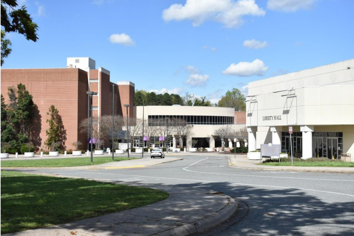
Charlotte Merchandise Mart, rear elevation, view to north
