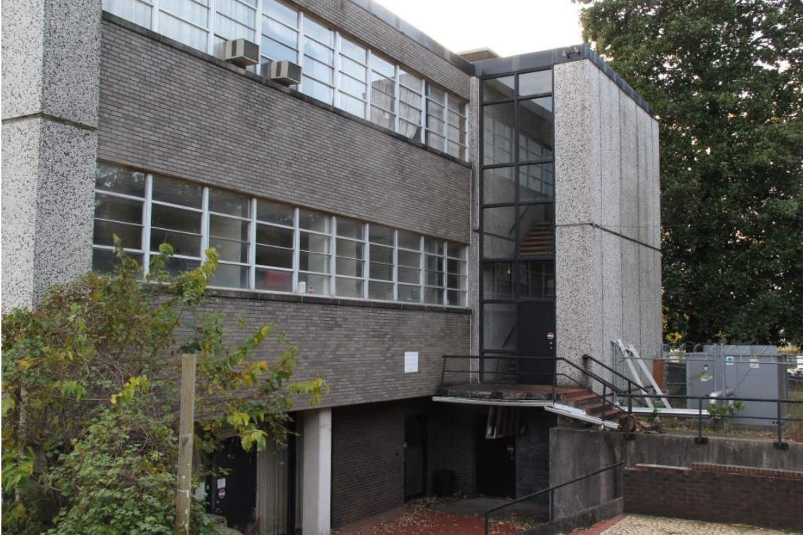
Allied Security Building, rear elevation, oblique view to west
