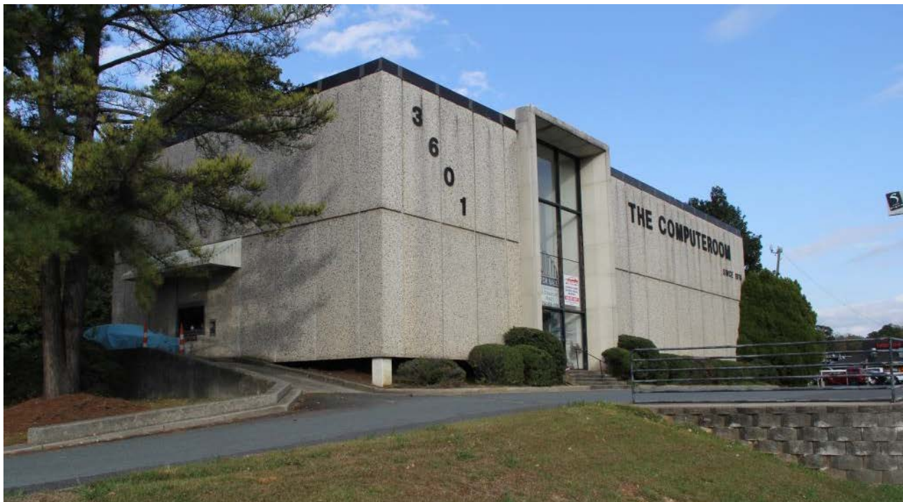
Allied Security Building, 3601 East Independence Boulevard, oblique front view to northeast
