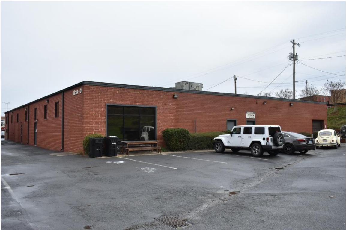
Warehouse, view to northeast
