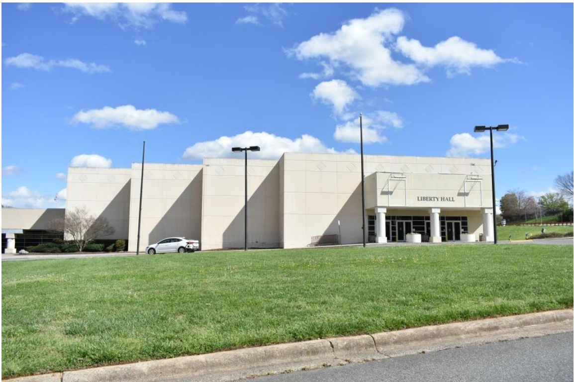
Charlotte Merchandise Mart, Liberty Hall façade, view to east
