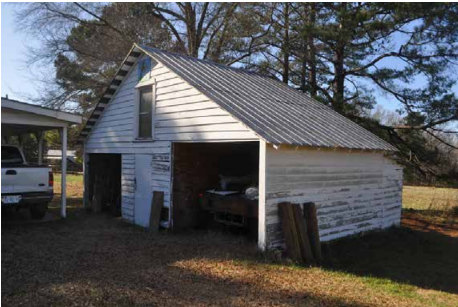
Plate 4.5: View of the detached garage on the subject parcel.
