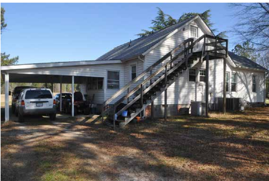
Plate 4.3: View of the northwest and southwest elevations of the Cleave A. Maynard House.
