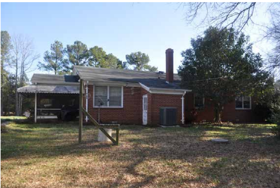
Plate 6.3: View of the rear (northwest) side of the William A. Poe House.
