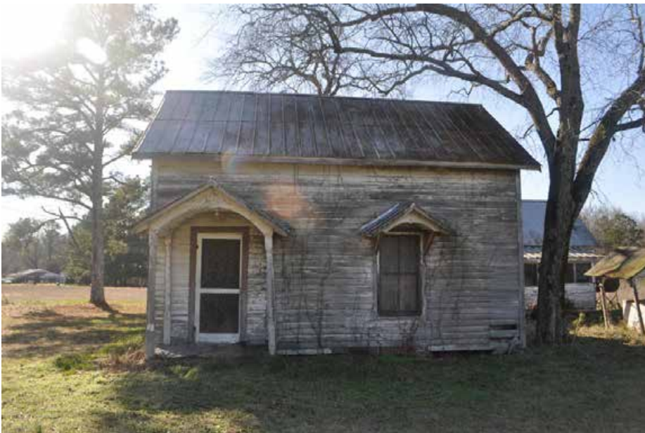
Plate 5.2: View of side addition (northeast side) of the Maynard Farm house.
