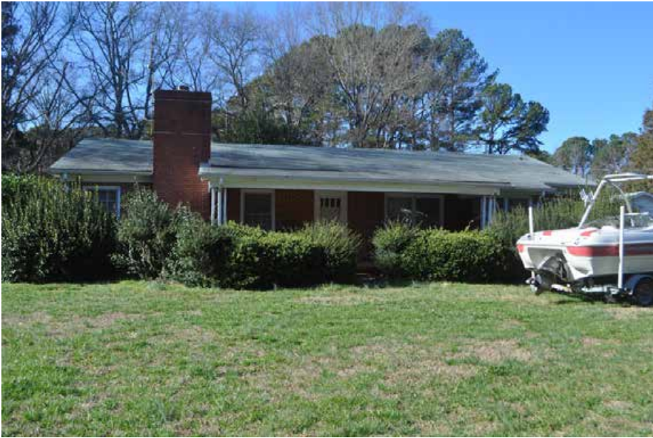
Plate 6.1: View of the primary façade (southeast side) of the William A. Poe House.
