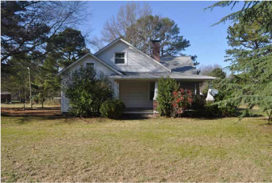
Plate 4.1: View of the primary façade (southeast side) of the Cleave A. Maynard House.
