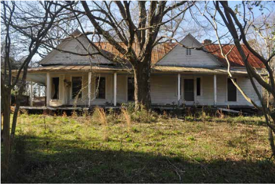
Plate 7.1: View of the primary façade (east side) of the Wood-Maynard Farm house.
