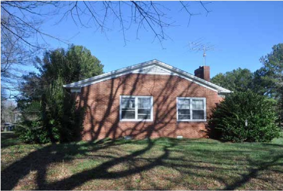
Plate 6.4: View of the southwest elevation of the William A. Poe House.
