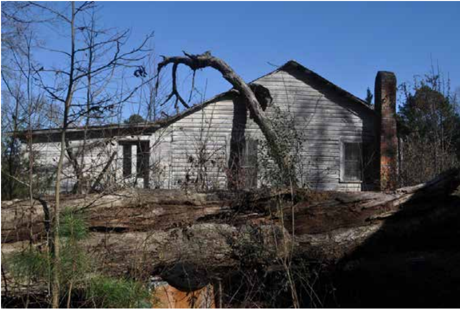
Plate 5.17: View of the tenant house on the subject parcel.
