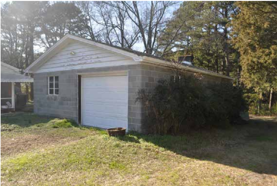
Plate 6.5: View of the detached garage on the subject parcel.
