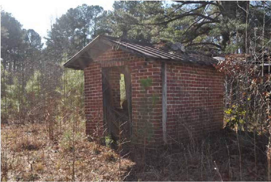
Plate 7.9: View of a brick shed on subject parcel.
