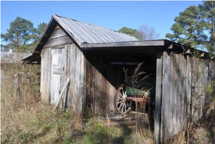
Plate 5.12: View of an equipment shed on the subject parcel.
