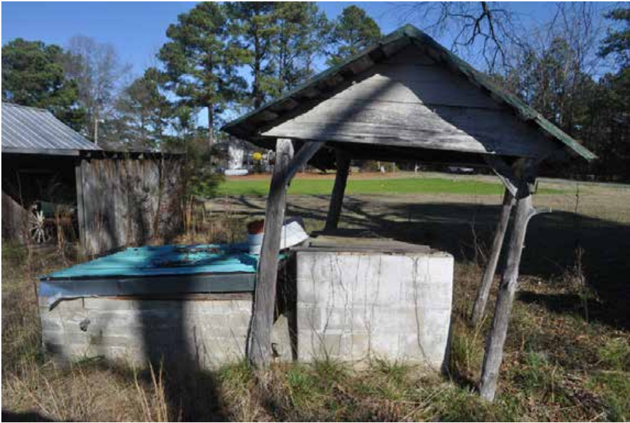
Plate 5.11: View of the well on the subject parcel.
