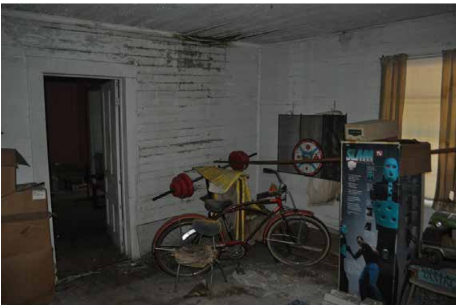
Plate 5.6: View of the east room in the main block of the Maynard Farm house.
