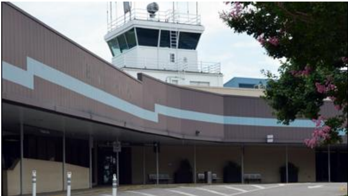
Photo 4. Raleigh-Durham pre-2014 demolition.
