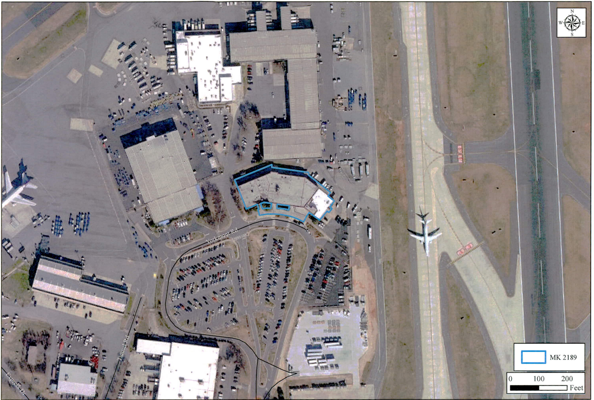
Figure 6 Addendum Historic Resource Report Charlotte Douglas International Airport Historical Resources Summary Project Mecklenburg County, North Carolina Aerial with MK 2189 (Old Terminal Building) Identified Aerial Provided by ArcGIS Online Environment & Archaeology LLC
