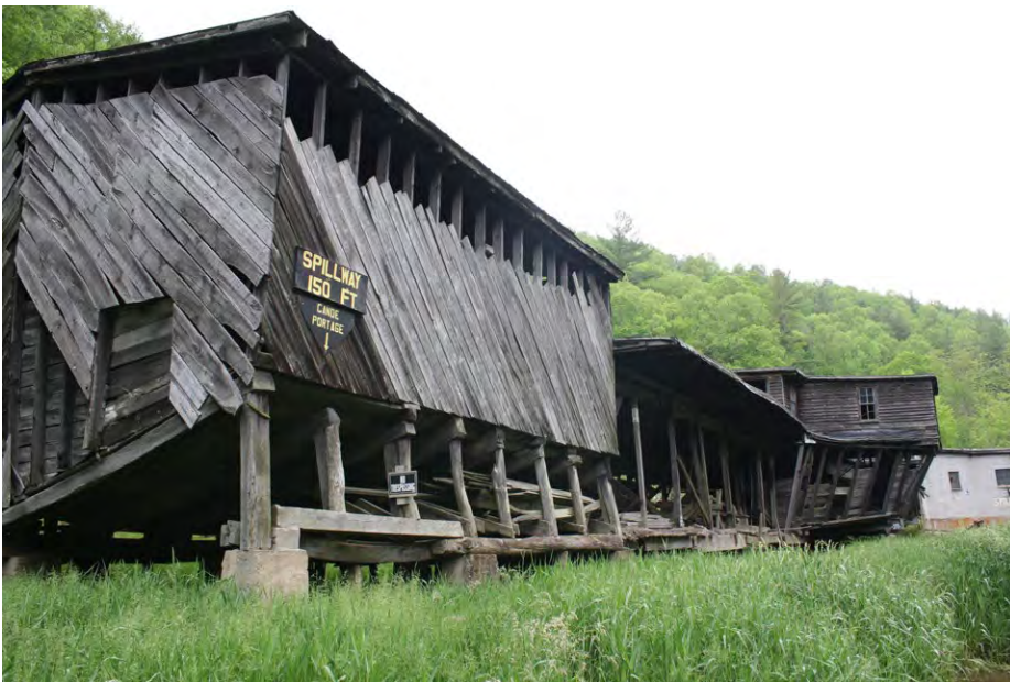
Plate 4.23: Sawmill storage bin section from the riverside.
