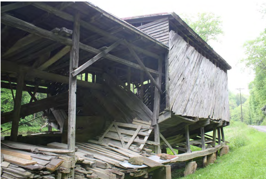
Plate 4.26: Storage bin and wood chute section.
