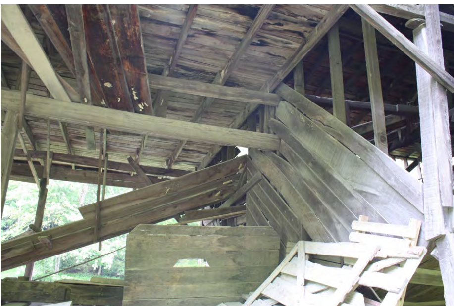
Plate 4.27: V-shaped wood chute leading up to the storage bin.
