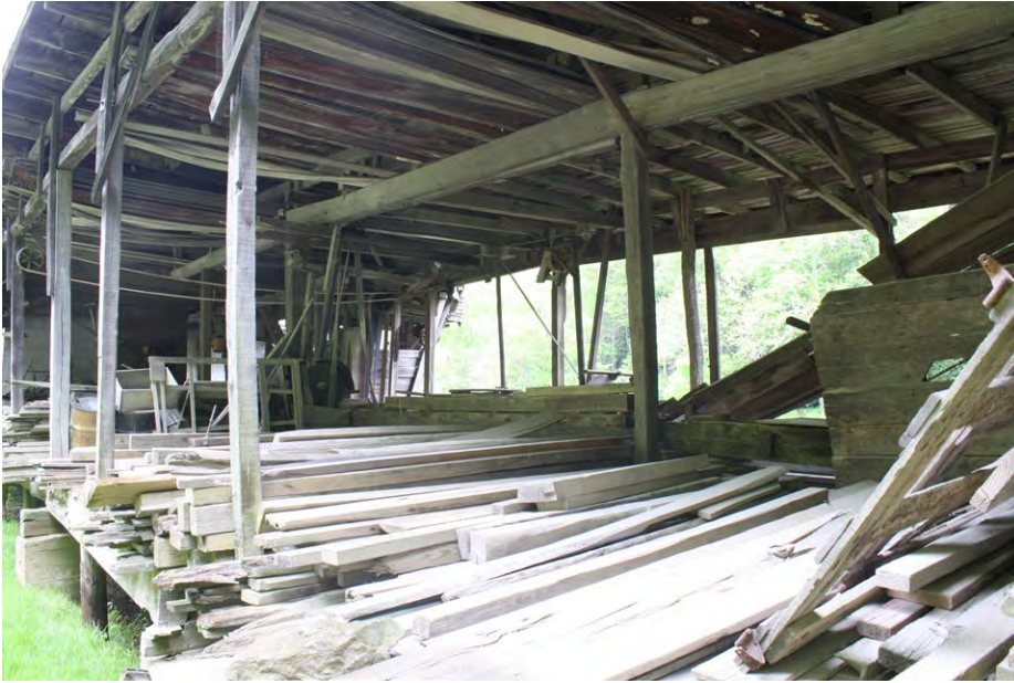
Plate 4.28: Sawmill interior looking toward the Machine Shop.
