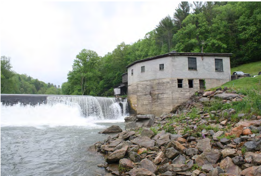
Plate 4.14: View of the Dam and Machine Shop.
