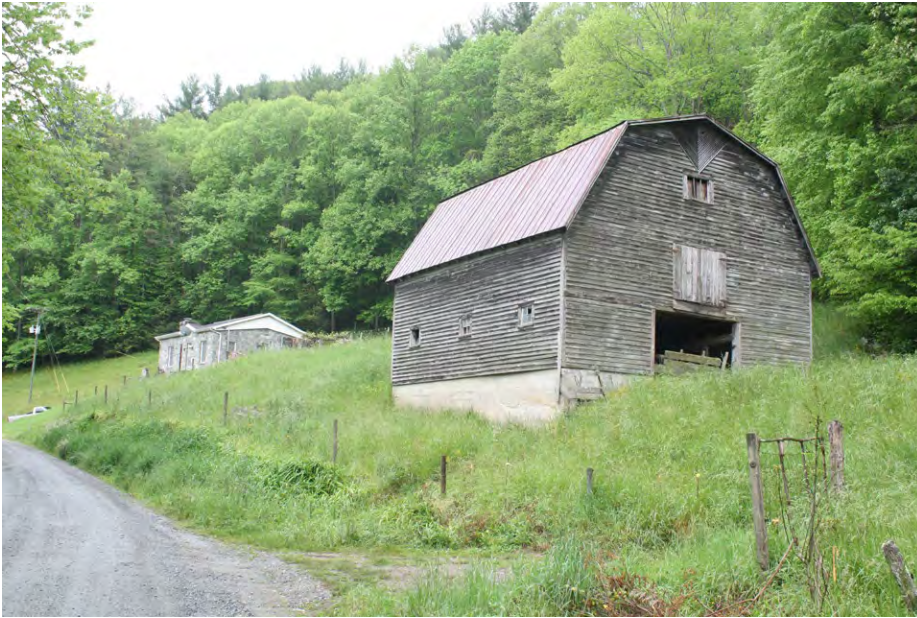
Plate 4.34: View of the Gambrel Roof Barn.
