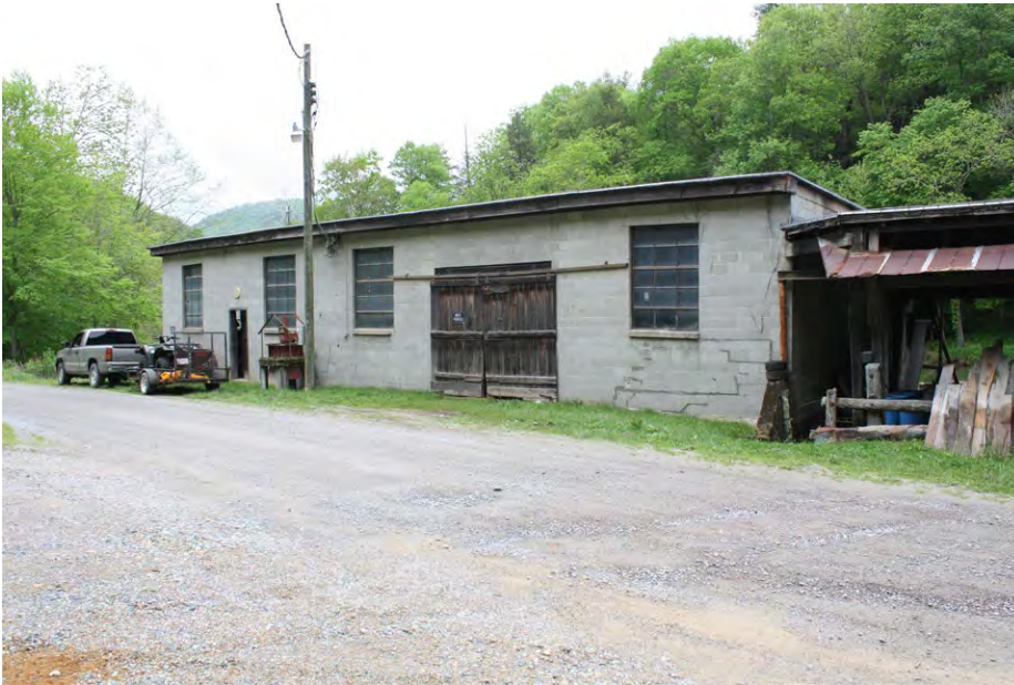
Plate 4.16: Machine Shop from Old Watauga Road.
