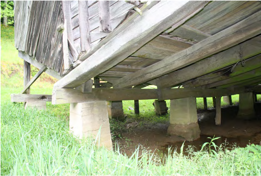
Plate 4.25: Storage bin floor system.
