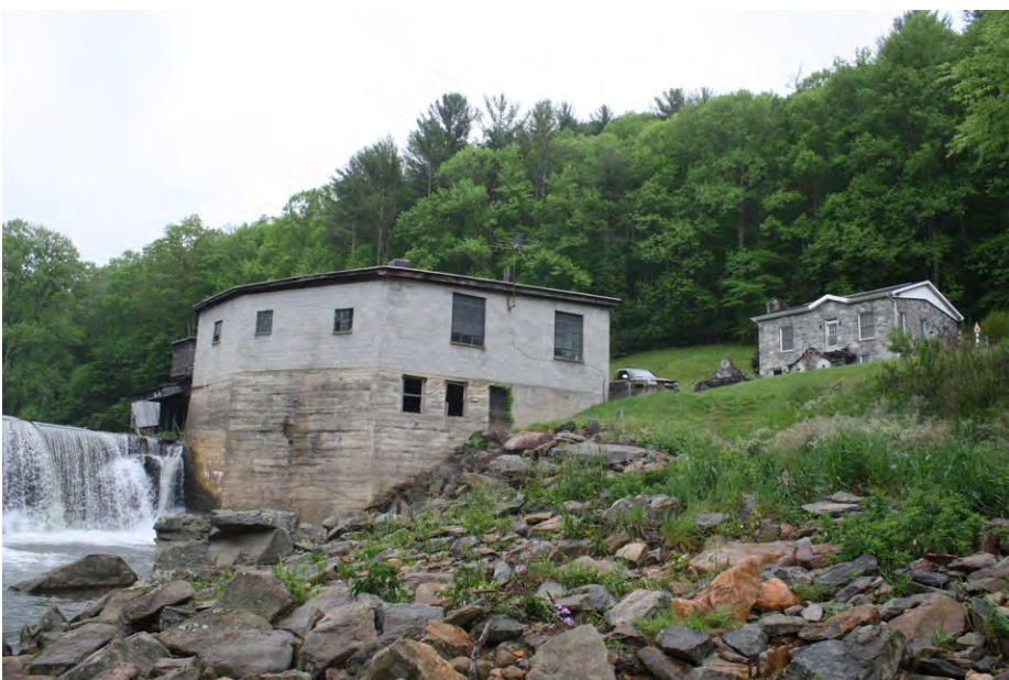
Plate 4.15: Machine Shop from riverbank with waterhouse section on right side.
