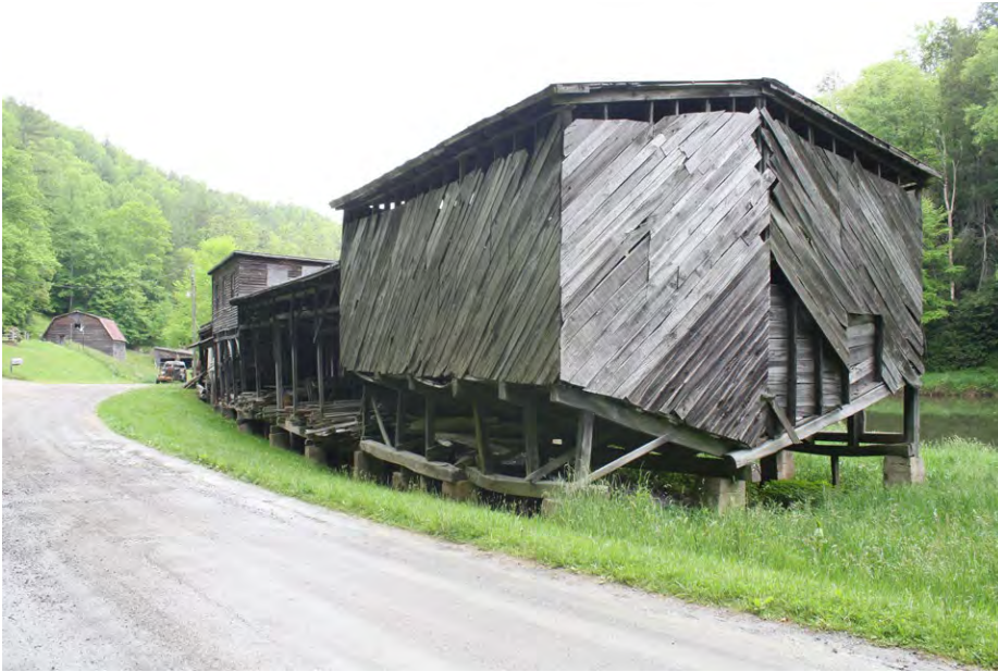
Plate 4.22: Sawmill storage bin section from the roadside.
