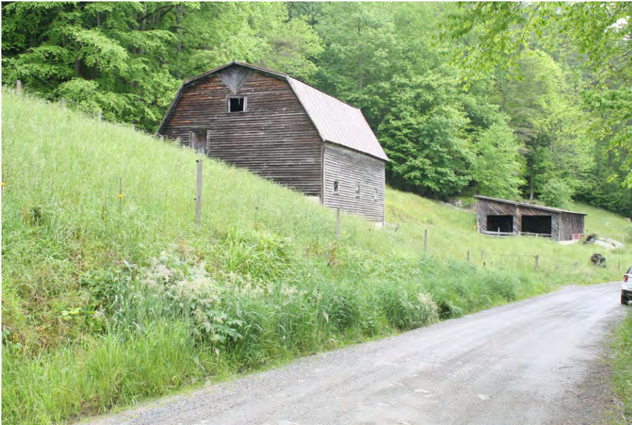
Plate 4.32: Gambrel Roof Barn (left) and Shed Roof Barn (right) from Old Watauga River Road.
