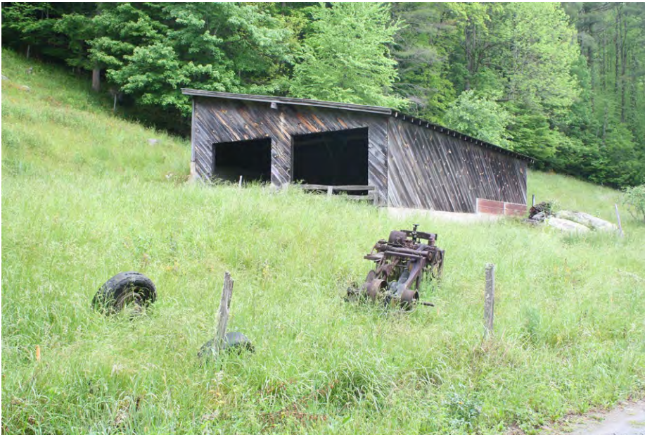
Plate 4.35: View of the Shed Roof Barn.
