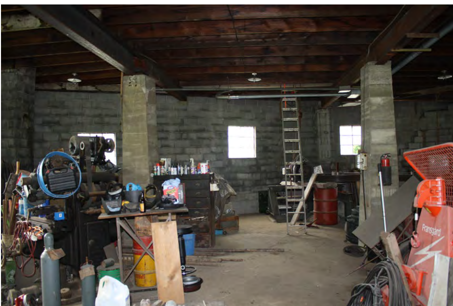
Plate 4.18: Machine Shop interior showing the pyramidal piers that support waterhouse section.
