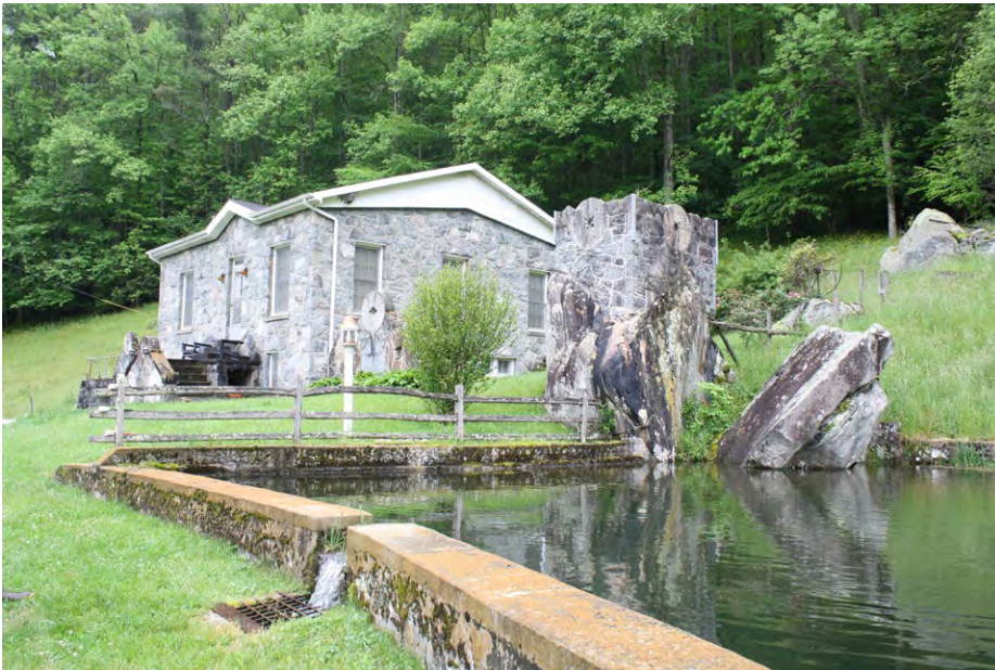
Plate 4.11: View of the Swimming Pool.
