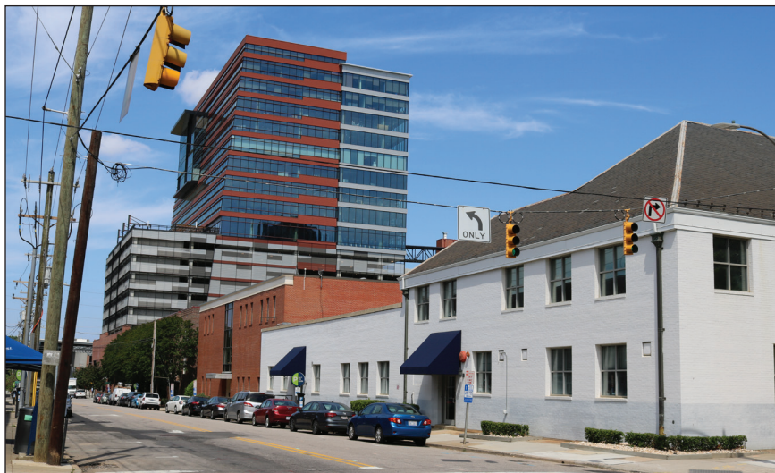
B. North Side of the 300 Block of West Martin Street, Facing Northwest
