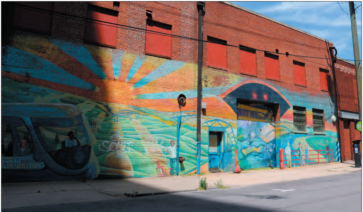
B. 210 South West Street, Facing Northwest
