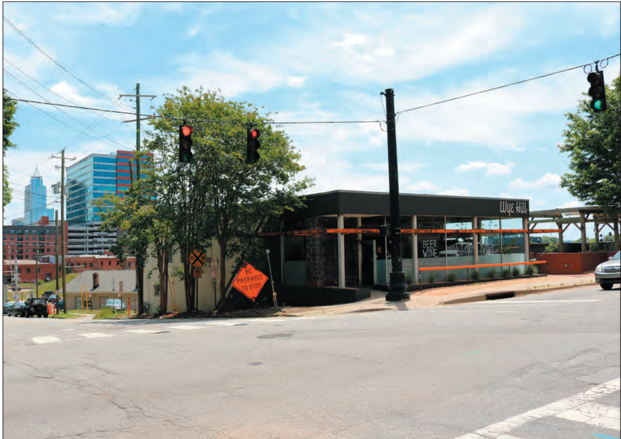
Figure 6.22. The EDS Equipment Design & Services Building, Facing Southeast
