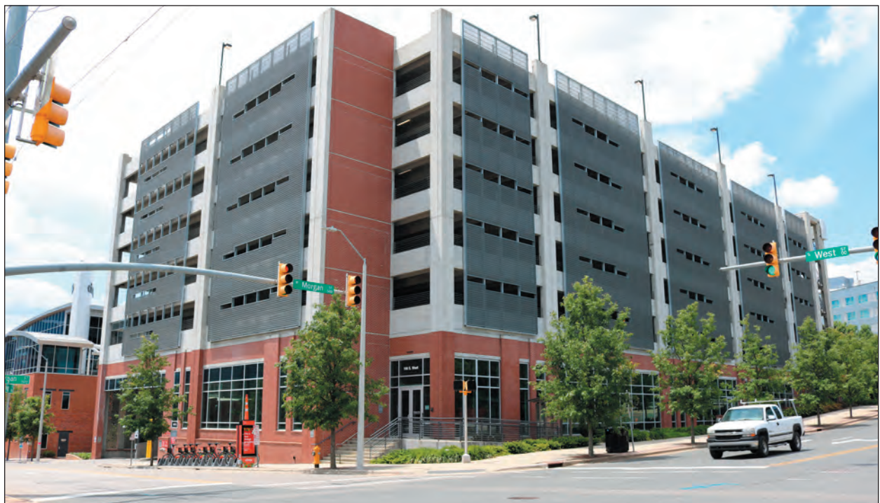
B. Citrix Office Building Parking Deck at 120 South West Street, Facing Southwest
