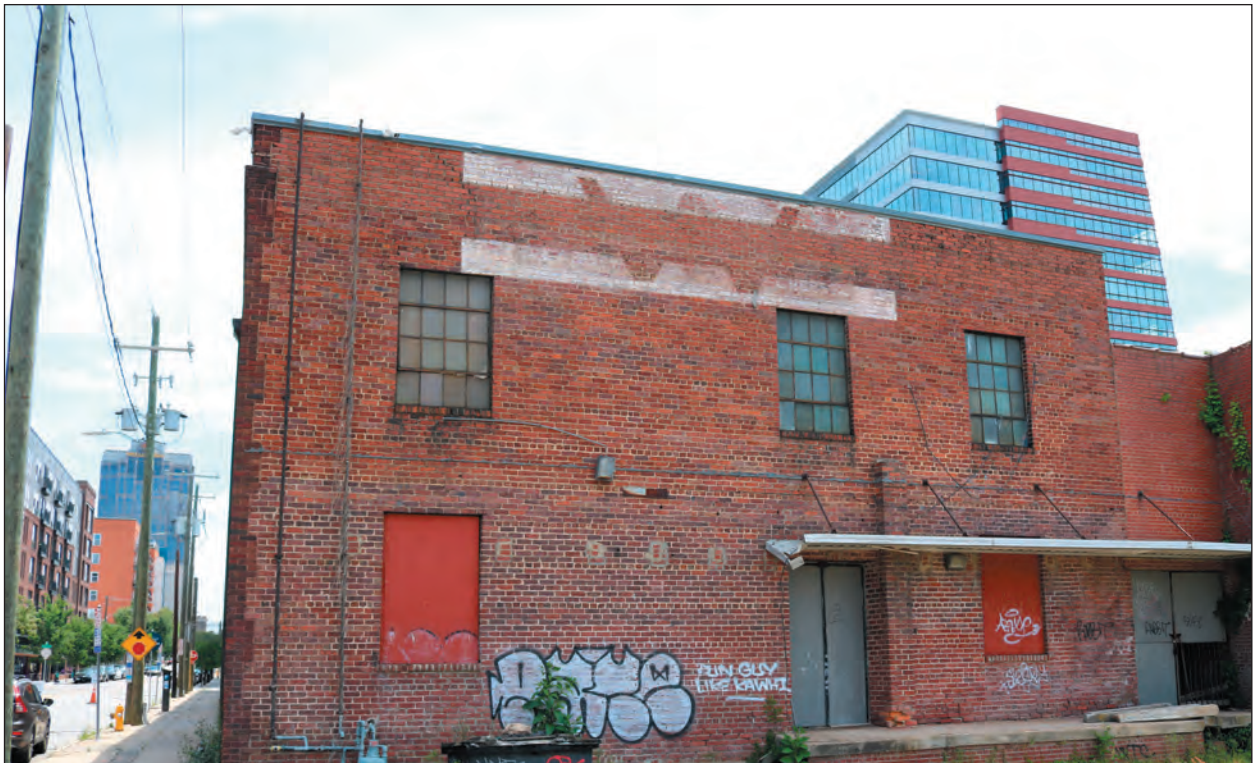
B. 200 South West Street, Facing East
