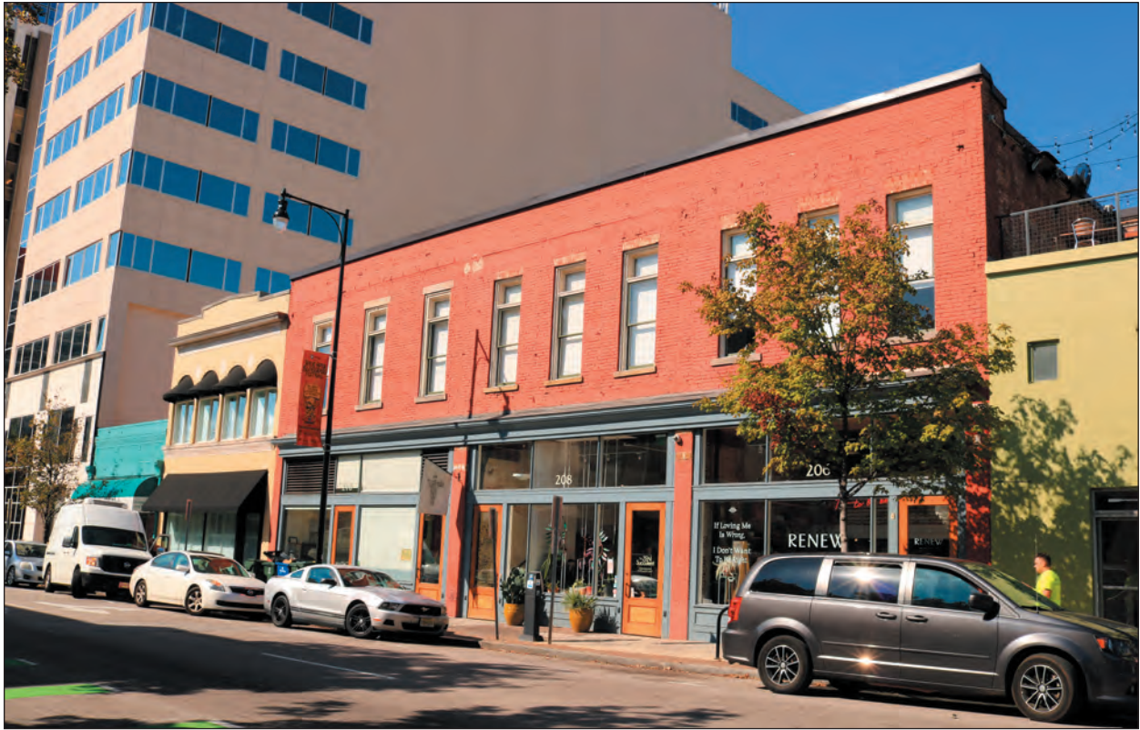
A. 200 Block of South Wilmington Street, Facing Southwest, 2019
