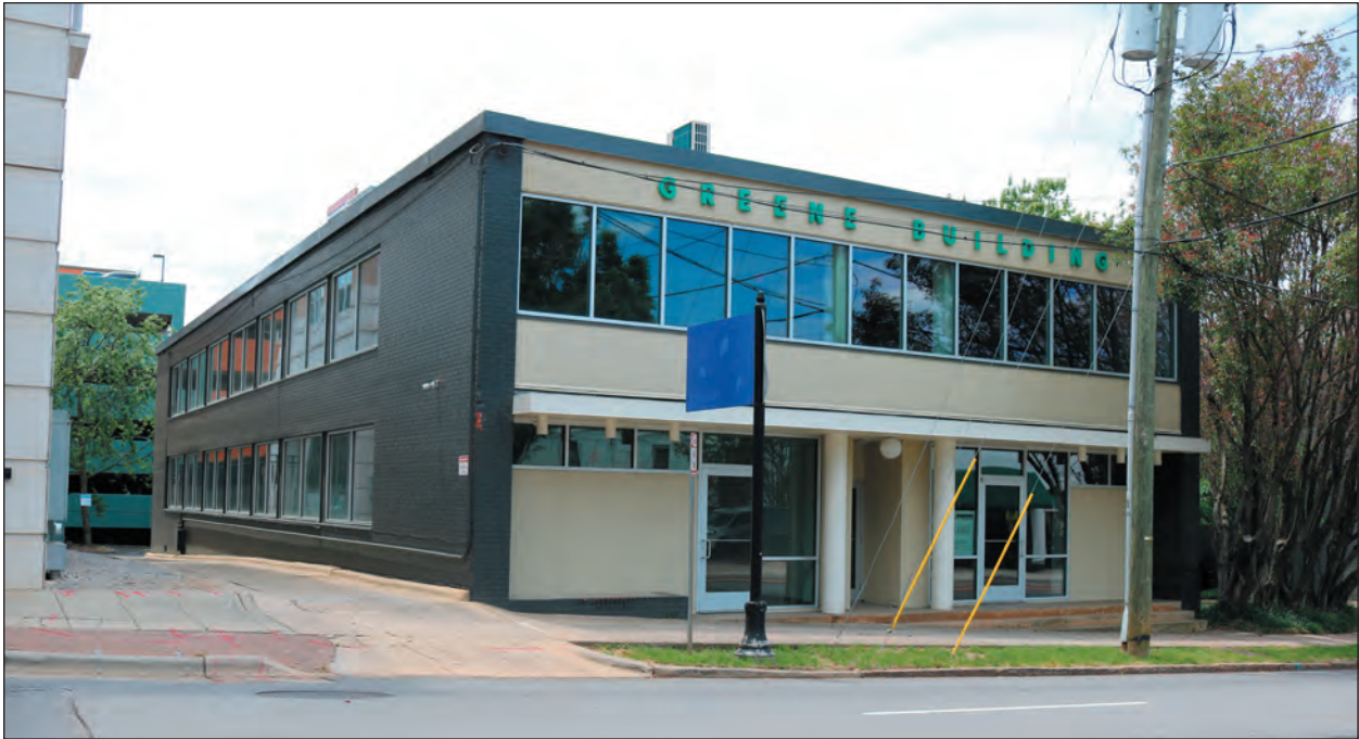
A. Facing Southwest
