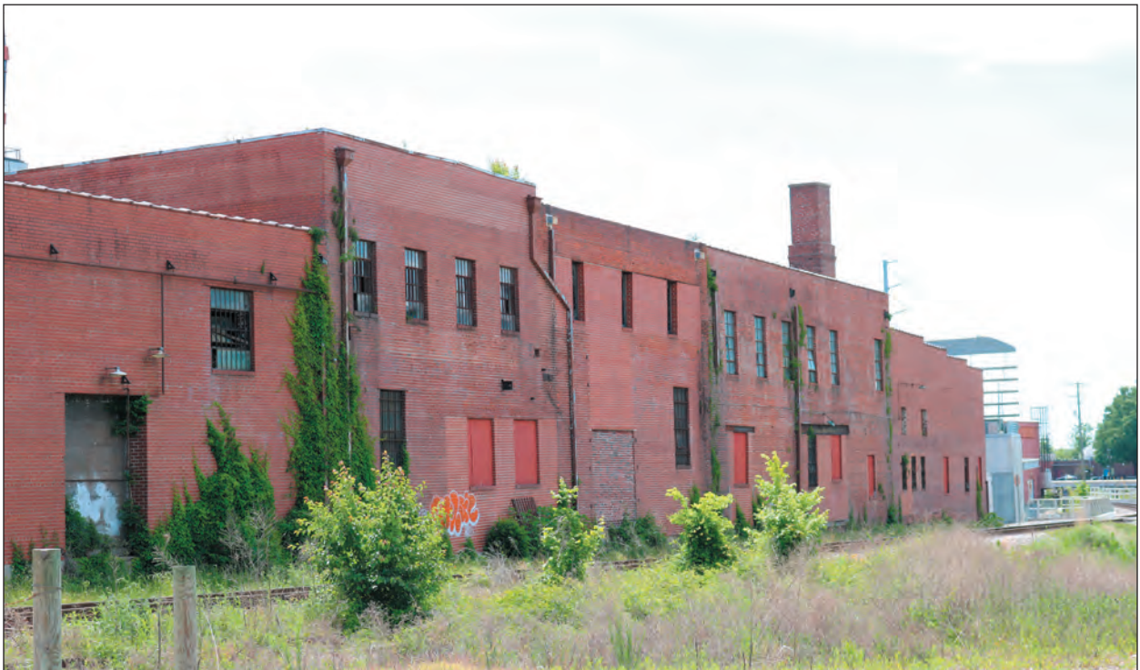
B. 210 South West Street, Southeast
