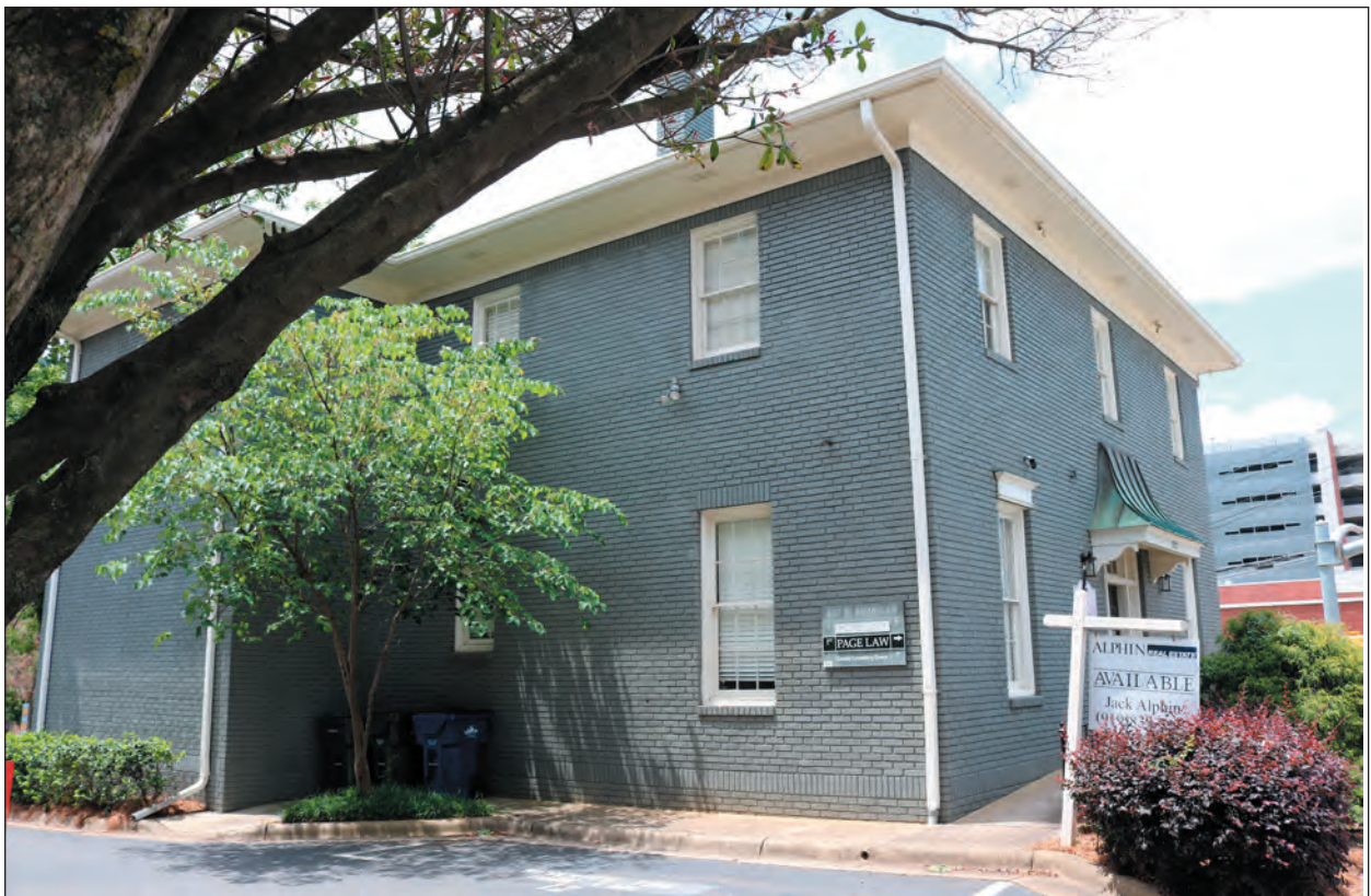
B. Facing Southwest
