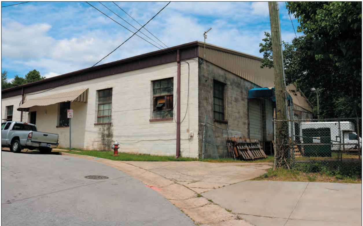
B. Facing Northwest
