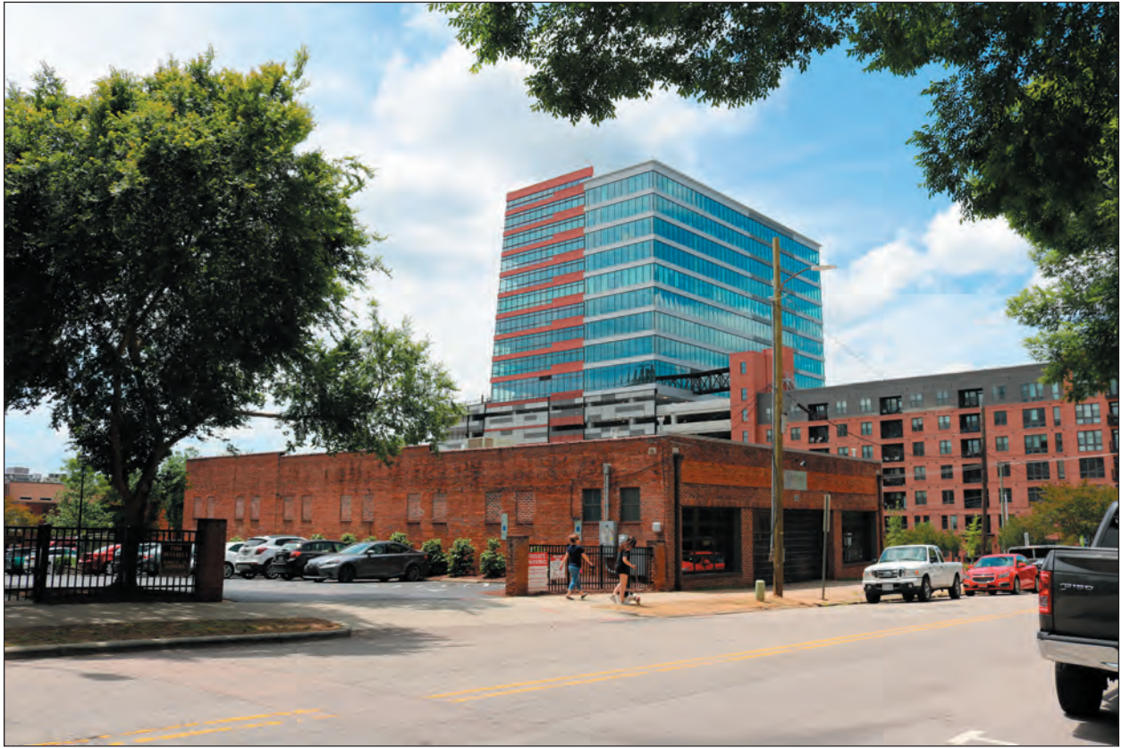
Figure 6.35. Royal Typewriter Company Building (WA8315), Facing Southwest
