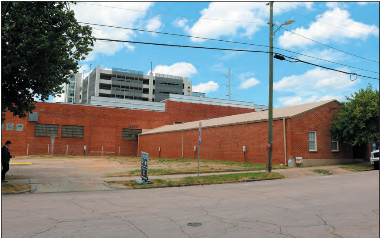
B. Facing Northwest
