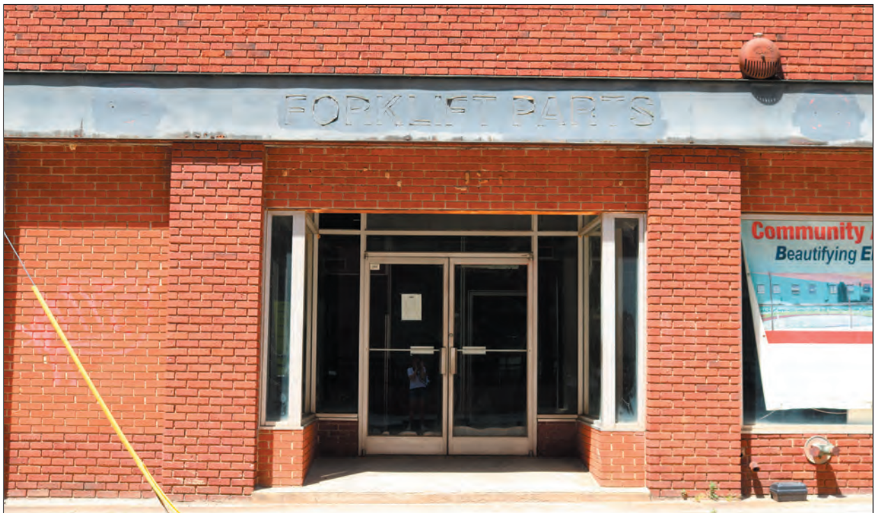
B. 206 South West Street, Main Entrance, Facing West
