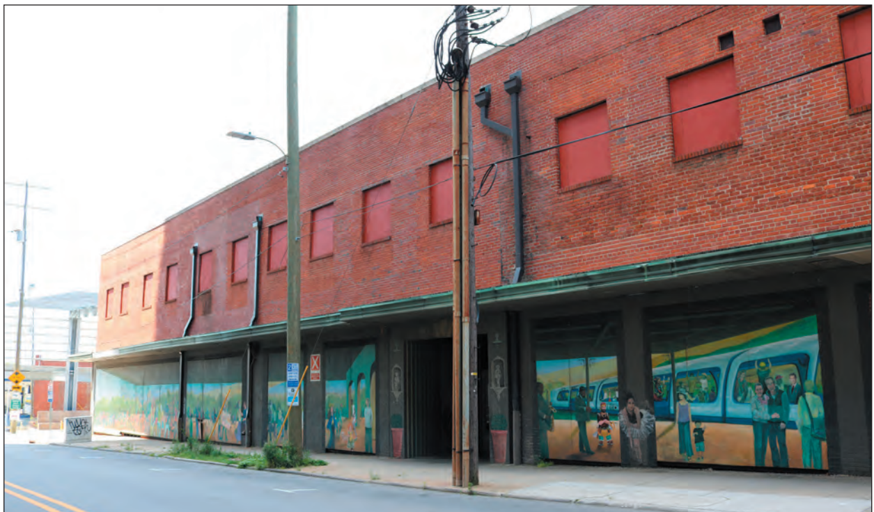
B. 210 South West Street, Main Entrance, Facing Southwest
