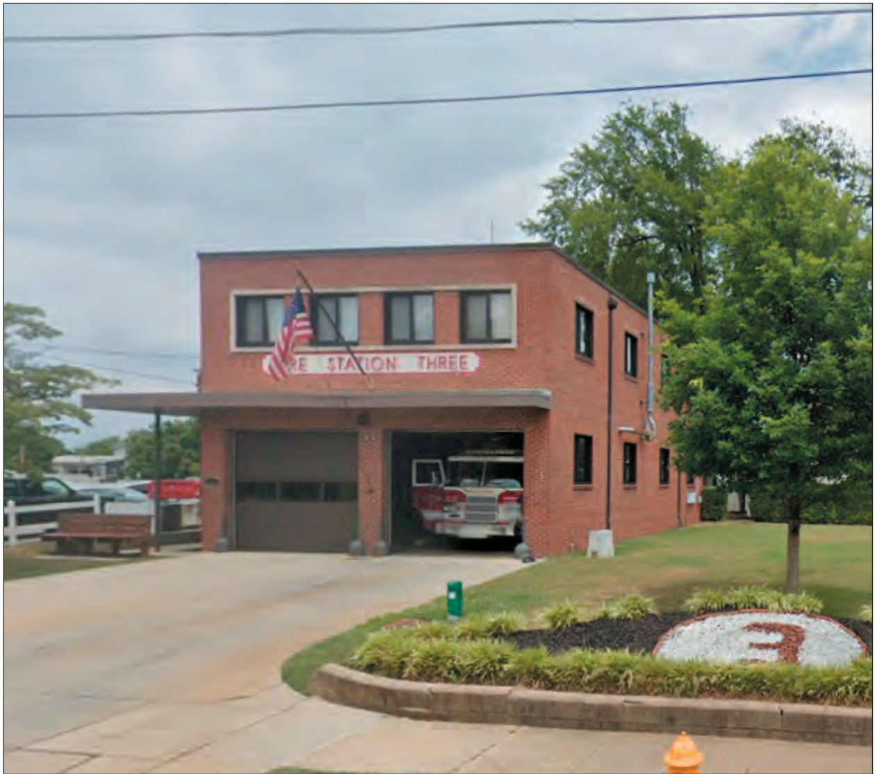
Figure 6.30. Station No. 3 (WA4557), Facing Northwest, 2019
