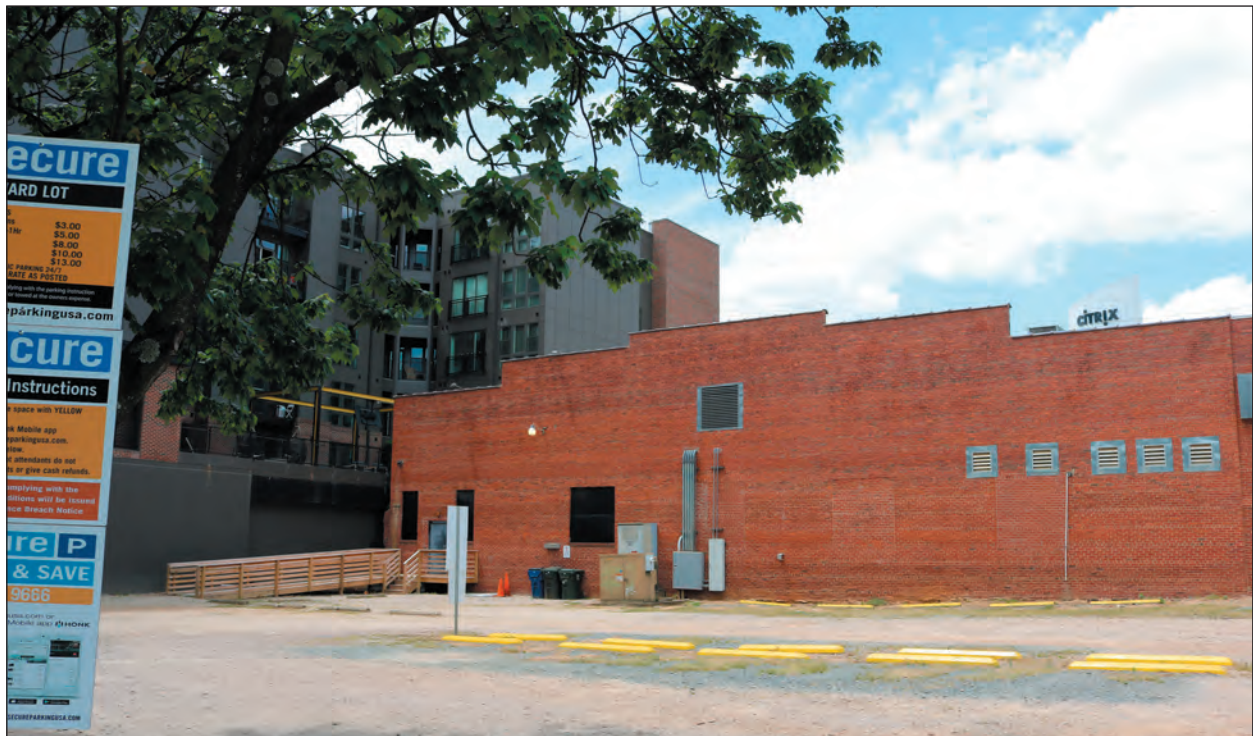
B. 117-121 South West Street, Facing West
