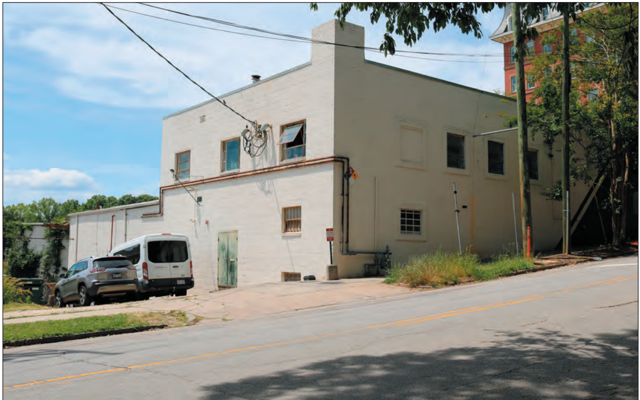
B. Facing Southwest
