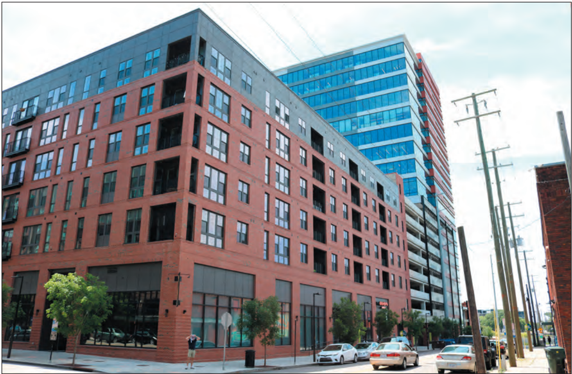
B. The Dillon at 223 South West Street, Facing Southeast
