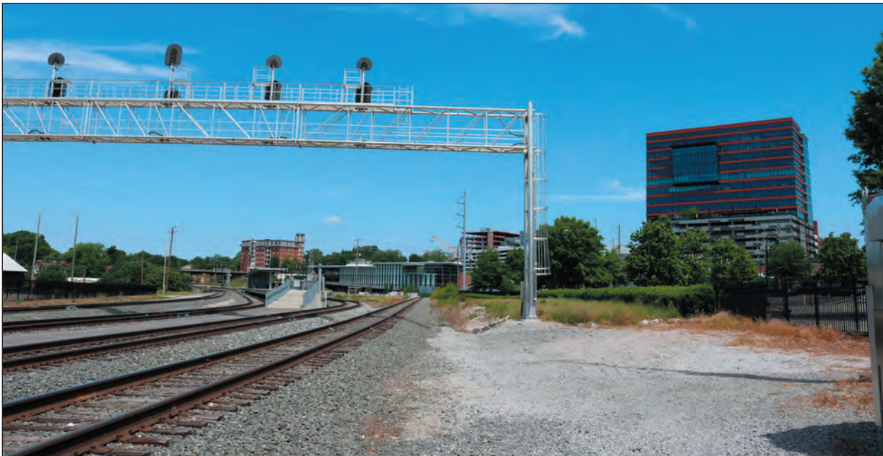
B. View of North of Rail Lines from the Southwest Corner of the Depot Historic District (WA0724)
