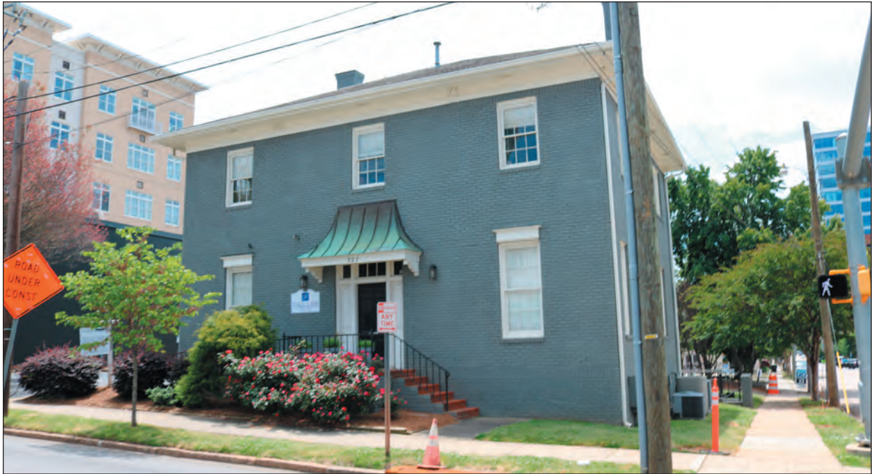
A. Facing South
