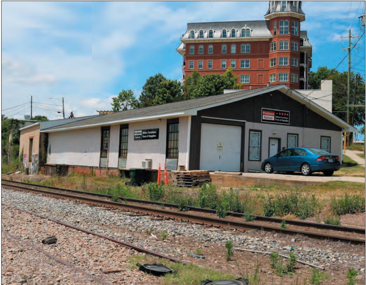
Figure 6.24. U.S. National Youth Administration Warehouse (WA7412), Facing Southwest
