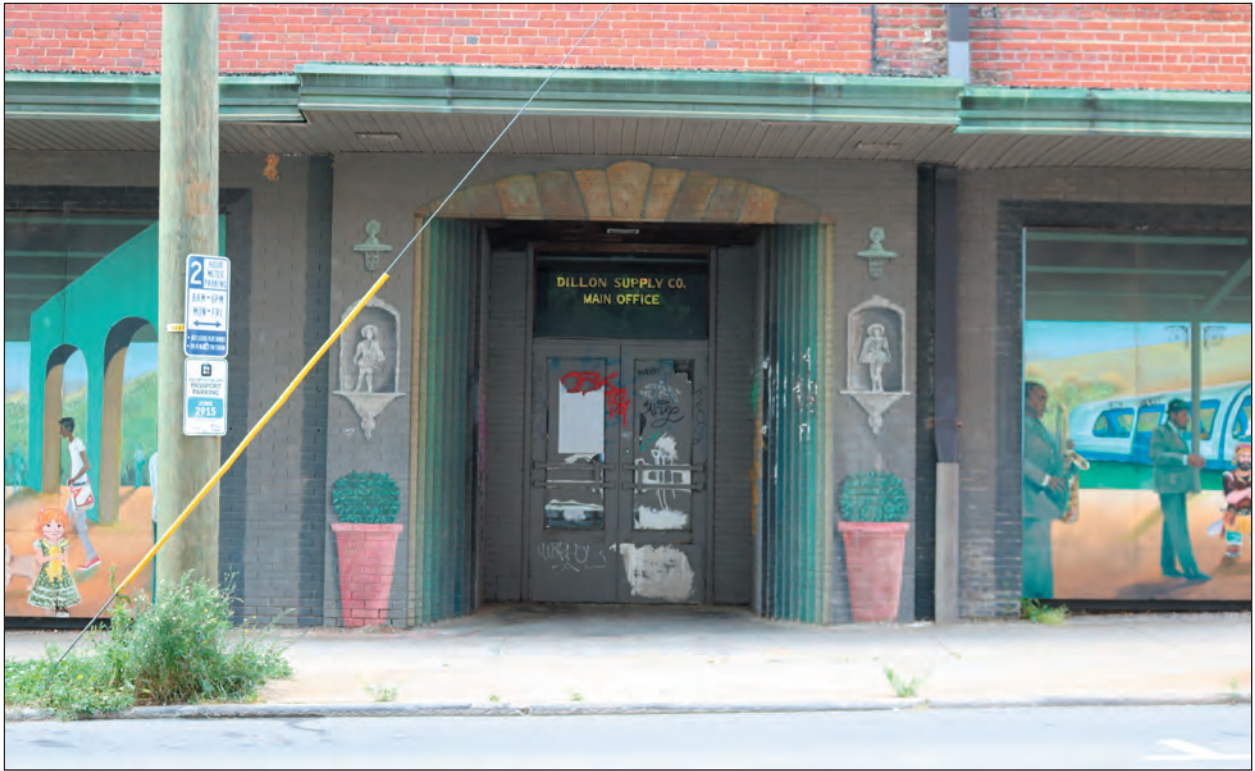
A. 210 South West Street, Main Entrance, Facing West
