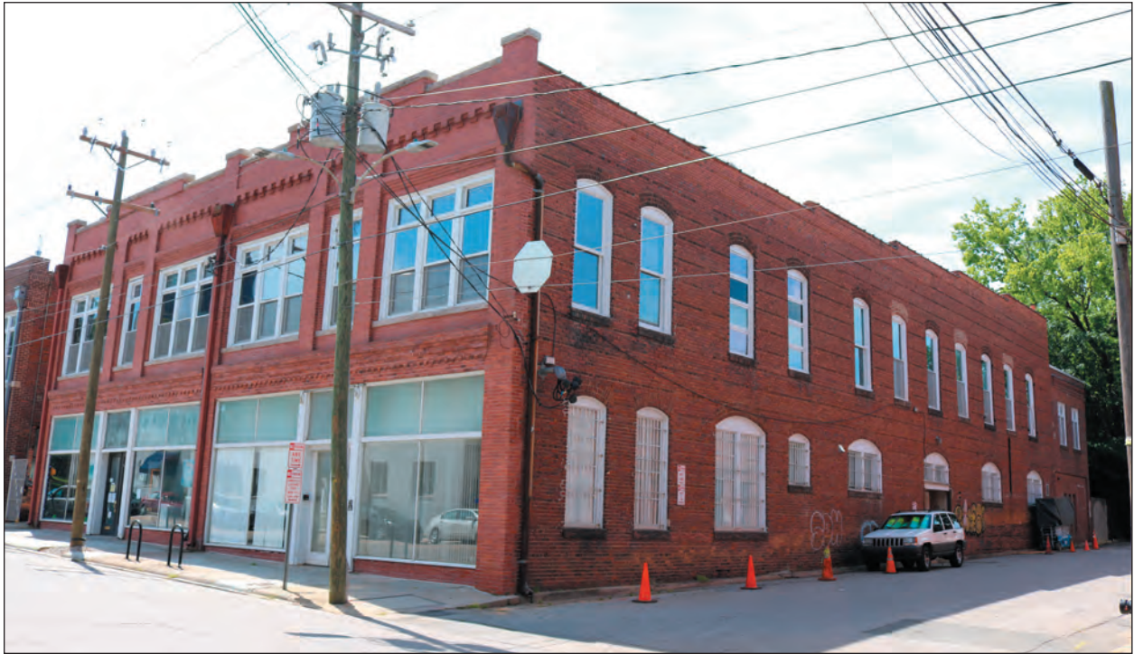
A. B.F. Goodrich Rubber Company (WA2982) at 311 West Martin Street, Facing Southeast
