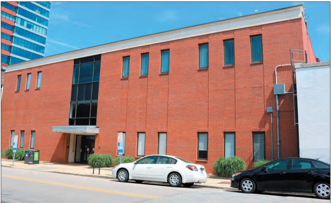
B. Facing Northwest
