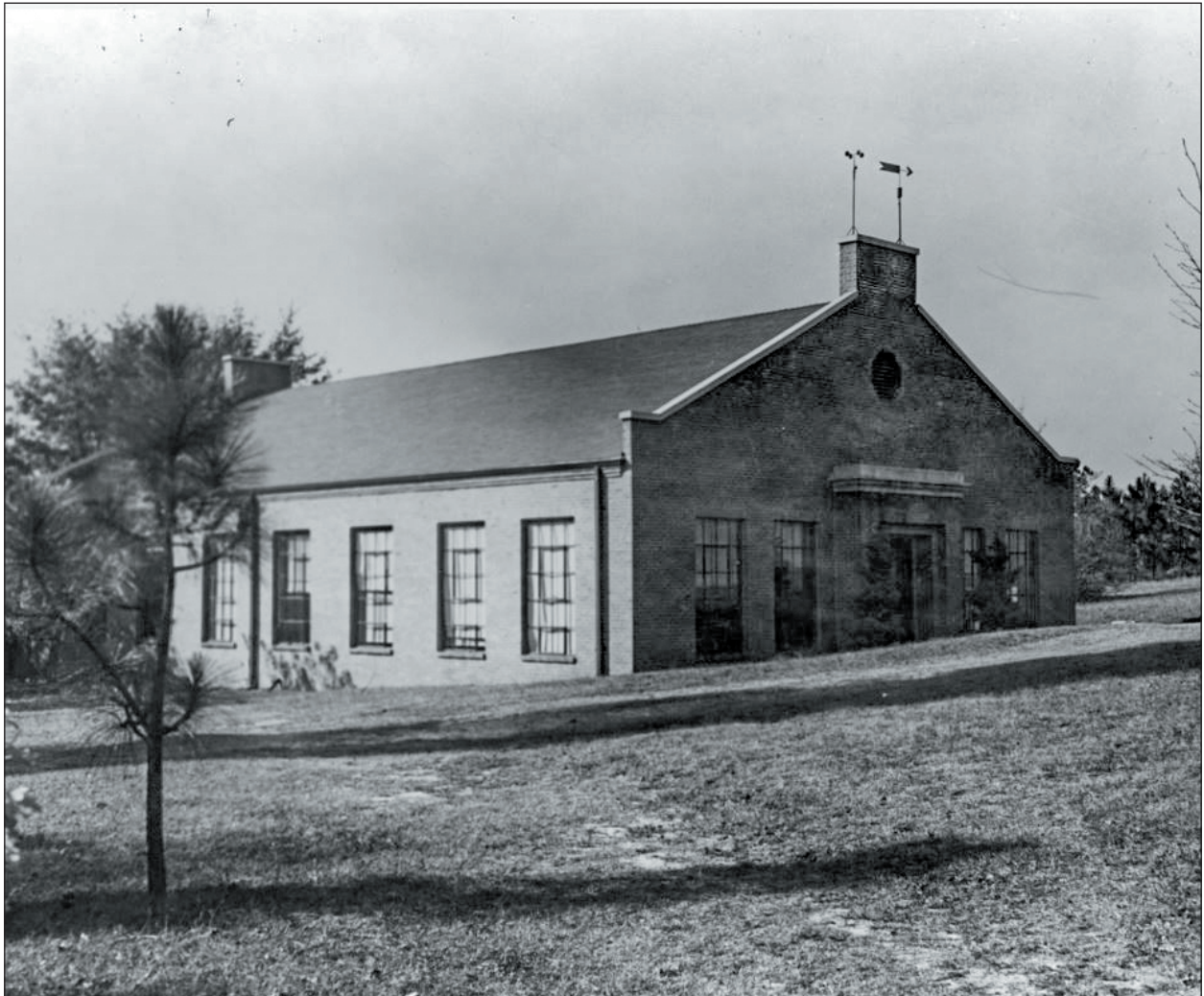
Figure 6.26. U.S. National Youth Administration building on the campus of NC State College, 1939
