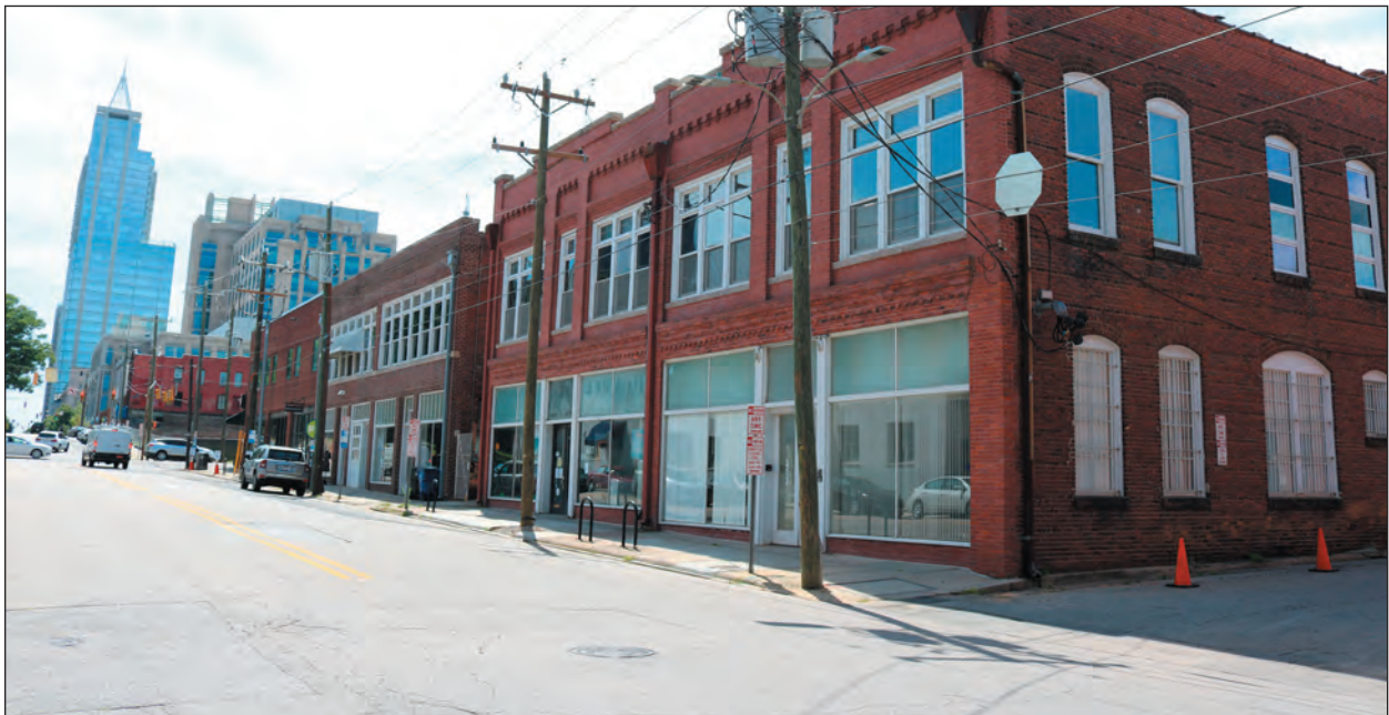
B. 320 Block of South Harrington Street, Facing Northeast
