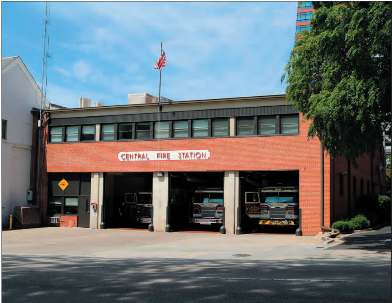
Figure 6.27. Nash Square Fire Station (WA8078), Facing Southwest
