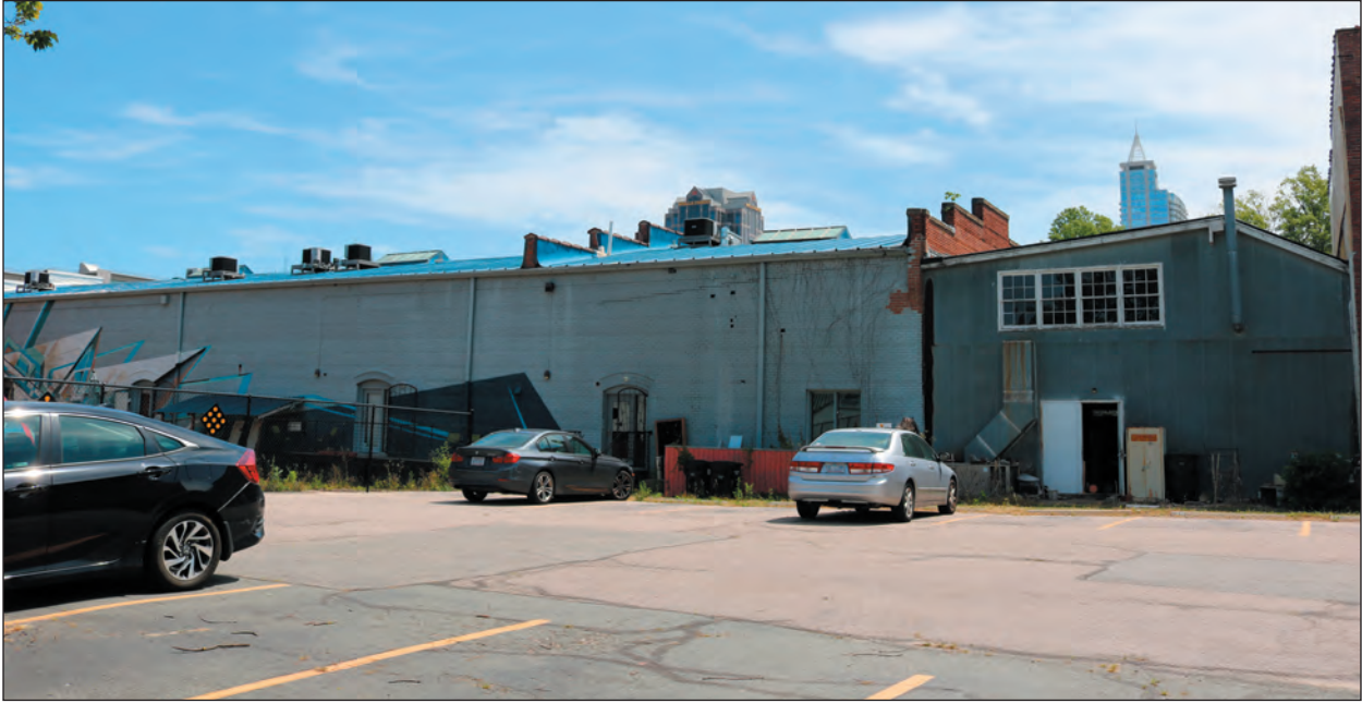
B. 310 Block of South Harrington Street, Facing Northeast
