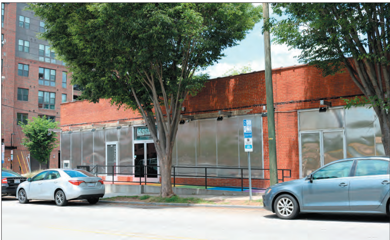
B. Facing Northwest
