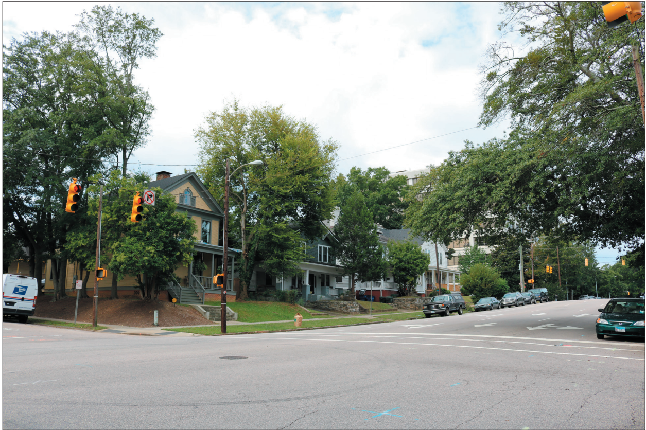
Figure 3.20. Contributing Dwellings on the South Side of the 400 Block of New Bern Avenue, Facing Southwest
