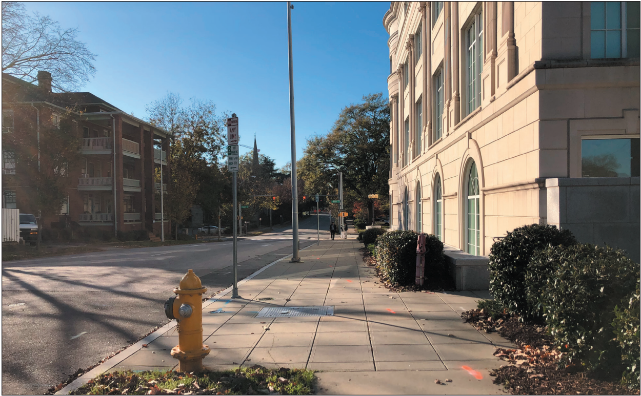
A. View Southeast into the Capitol Area Historic District from the Proposed Stop Location
