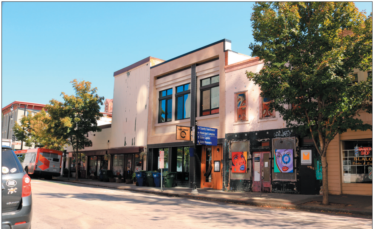
B. 200 Block of South Wilmington Street, Facing Northeast
