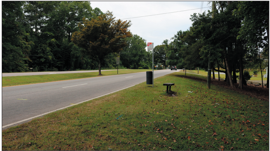
A. Existing Roadside Bus Stop near Dickens Drive, Facing Southeast
