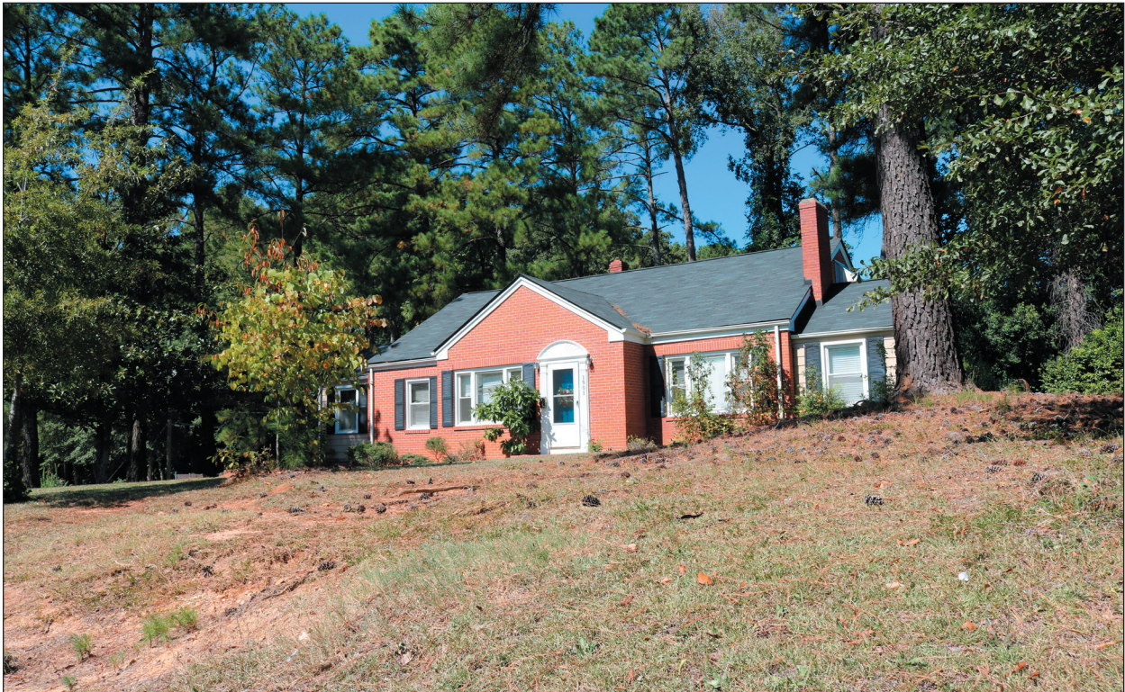
B. Richard Hall HoUse at 1901 New Bern Avenue
