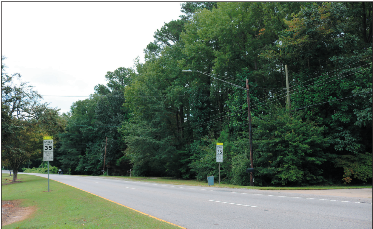
B. 2300 Block of New Bern Avenue, Facing Southeast
