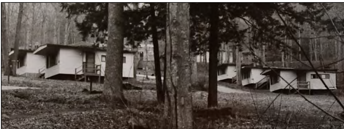
Figure 22. No-longer-extant, prefabricated A-6 trailer-type houses in 1997 (source: HPO file GH0061)
