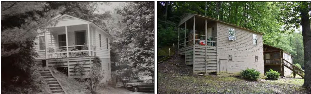
Figure 28. 19 Park Way (Fontana Village cabin 745) in 1974 (source: HPO file GH0061) and at present—perhaps originally a temporary house type J; note 37 Park Way (Fontana Village cabin 747-749), at far right,
