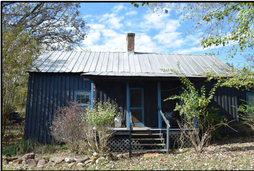
Facade, view to the west
