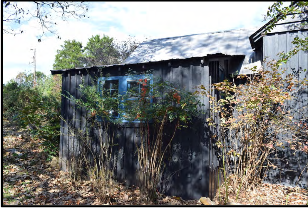
1993 kitchen addition on south elevation, view to the north-northwest
