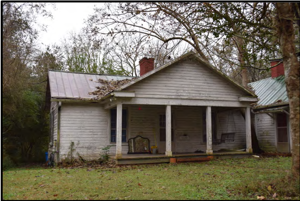
Main block, view to the east
