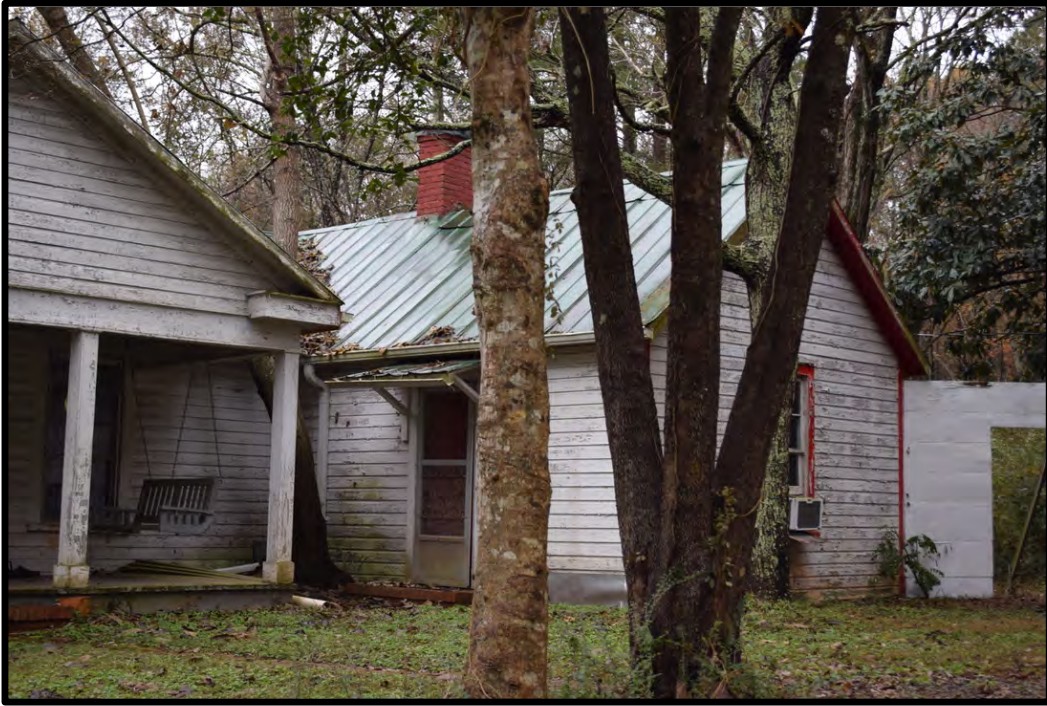
Front-gabled wing, view to the southeast
