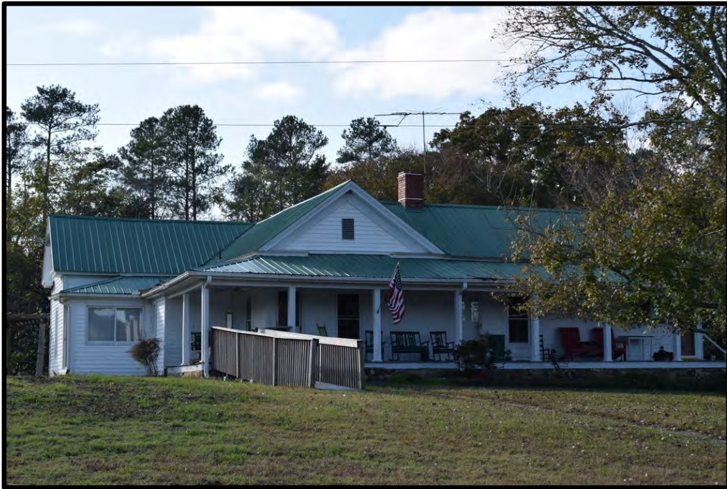
Burns House at 2388 Chatham Church Road
