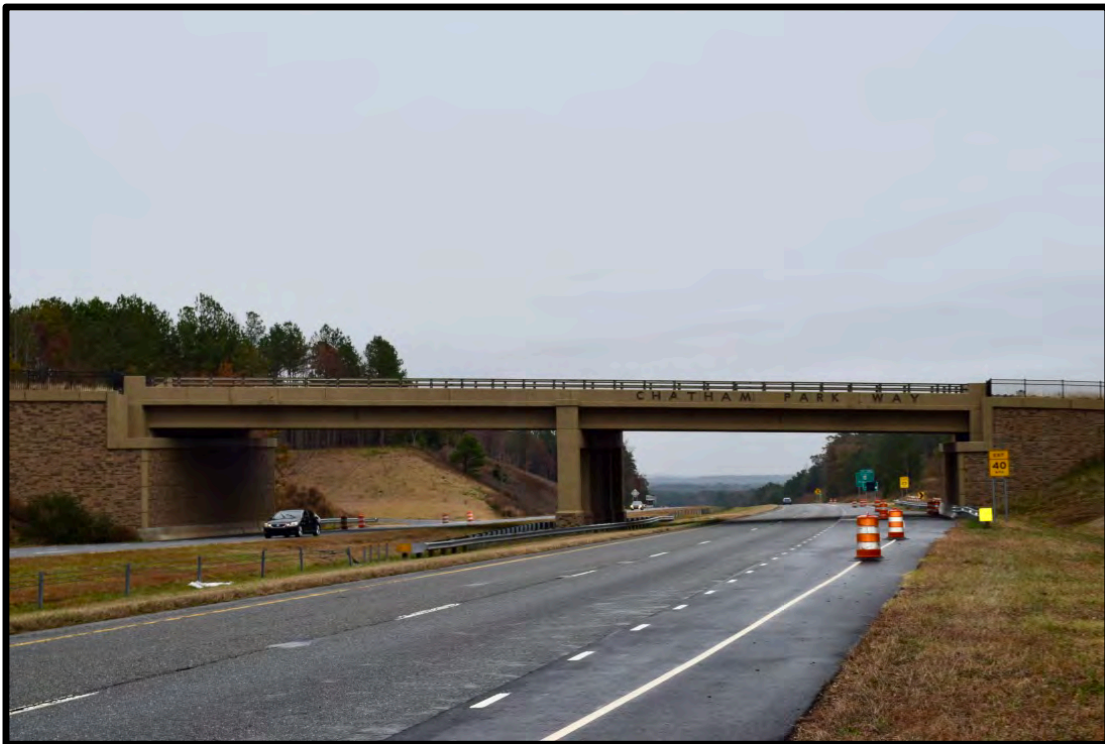
South end of project area on US 64 Business east of Pittsboro, view to the east
