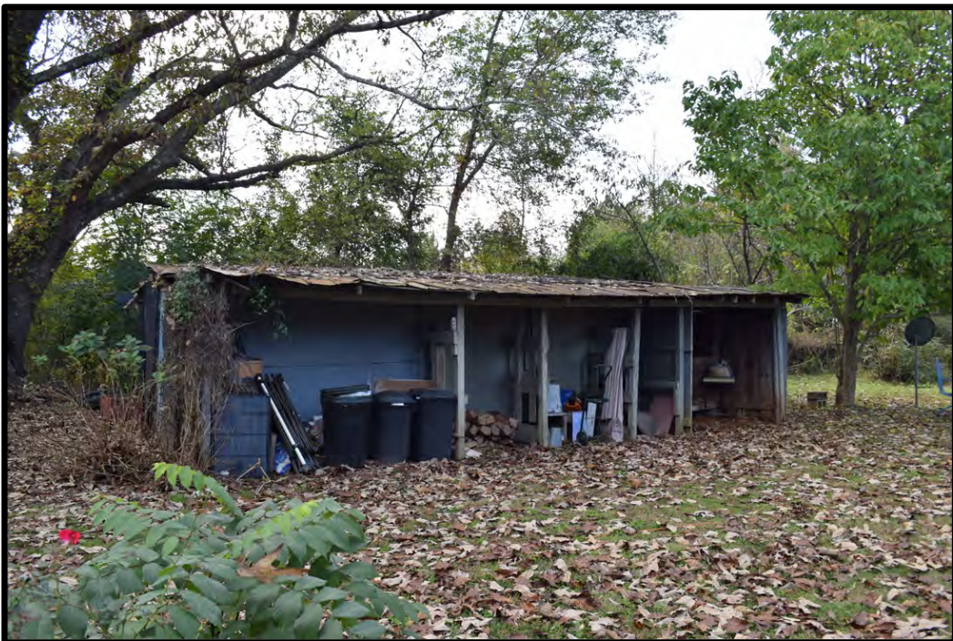
Shed built circa 1993, view to the west-southwest
