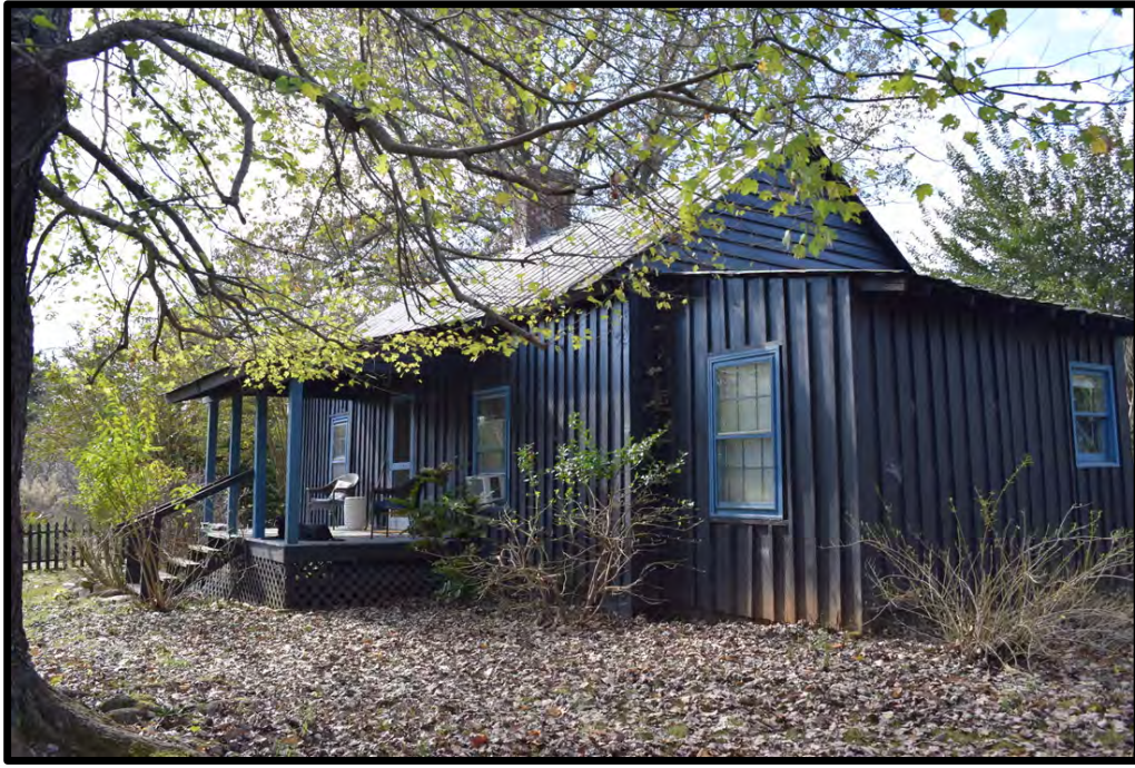
Northeast (front) corner of the house, view to the southwest
