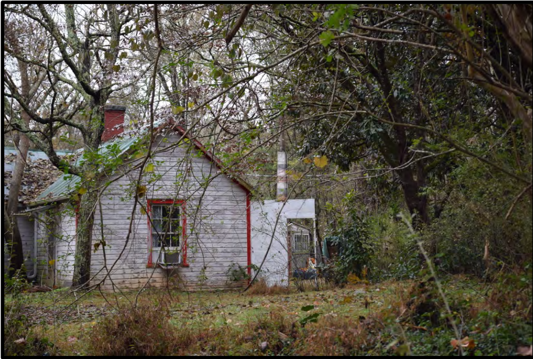
Front-gabled wing with part of greenhouse visible, view to the southeast
