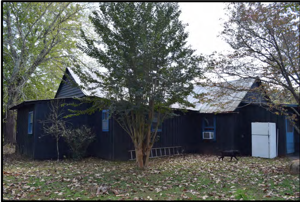
Northwest (rear) corner, view to the southeast
