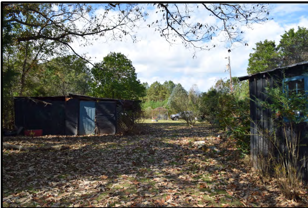
Circa 1993 shed (left) and portion of kitchen addition (right), view to the west
