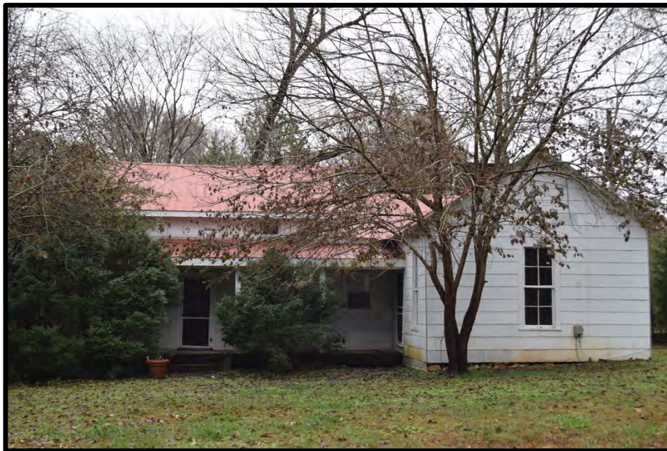
Will Harris House (CH0310), view to the north
