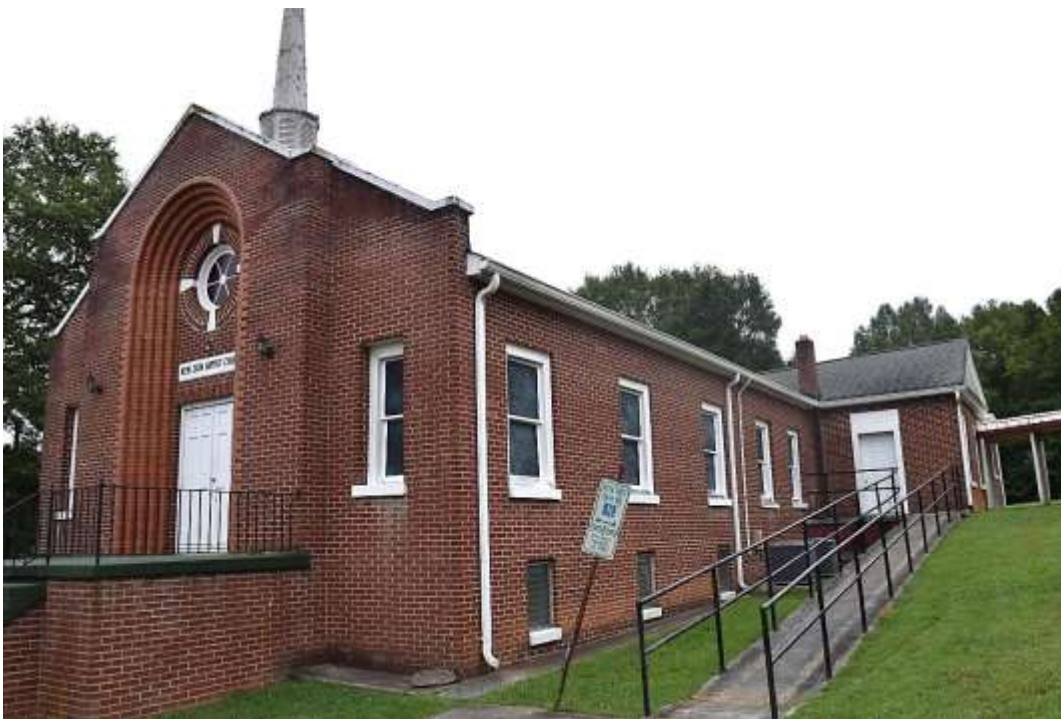
New Zion Baptist Church and Cemetery, Church Façade and Side (West) Elevation, Looking South.
