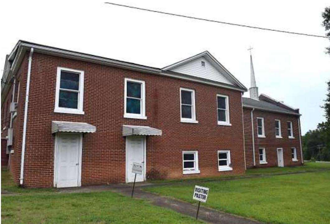
New Zion Baptist Church and Cemetery, Side (East) Elevation of Church and Rear Wing, Looking West.
