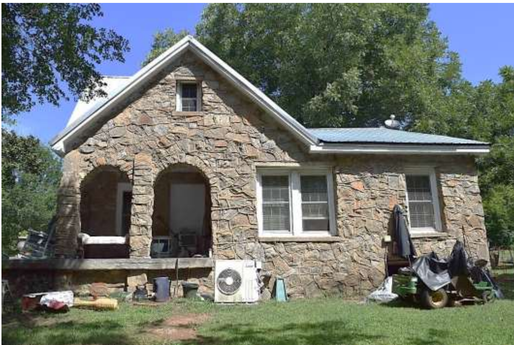
Walter and Emily Phillips House, Side (South) Elevation, Looking North.
