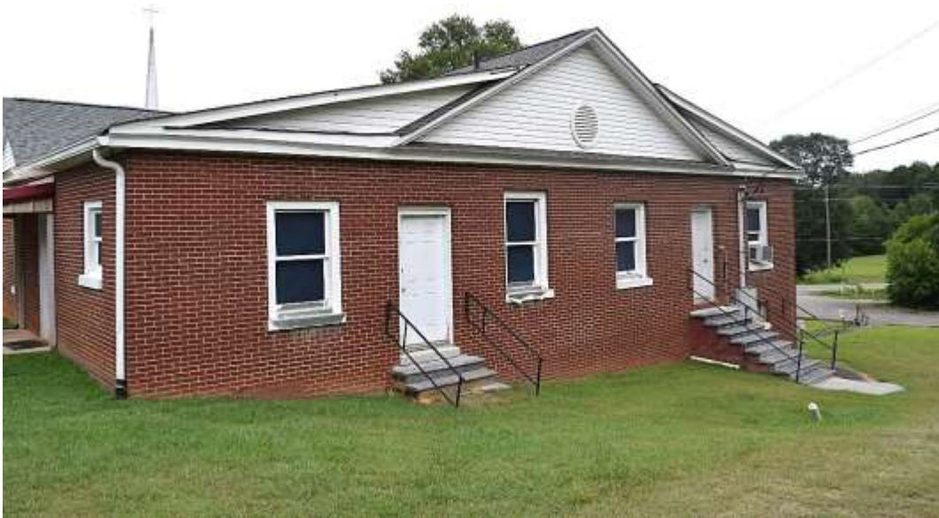
New Zion Baptist Church and Cemetery, Rear (South) Elevation of Church, Looking North.
