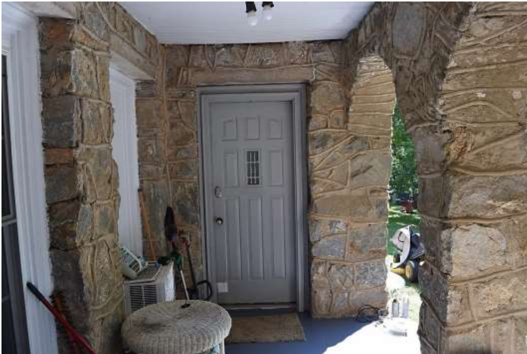
Walter and Emily Phillips House, Porch, Modern Entrance, Looking East.
