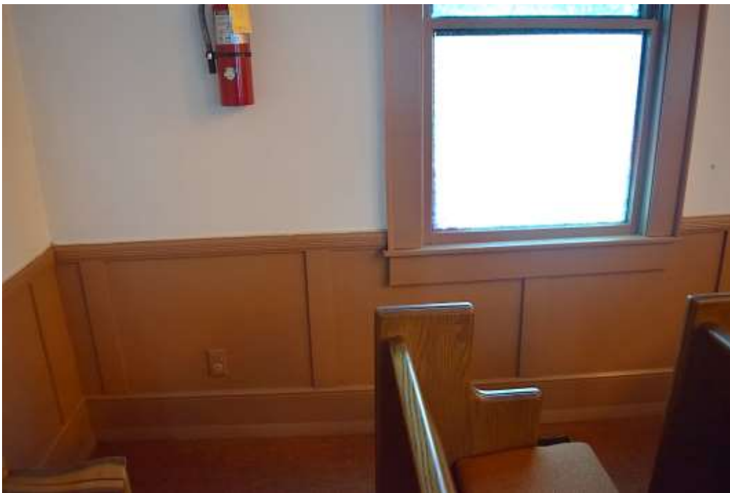
New Zion Baptist Church and Cemetery, Interior, Nave, Detail of Wainscoting.
