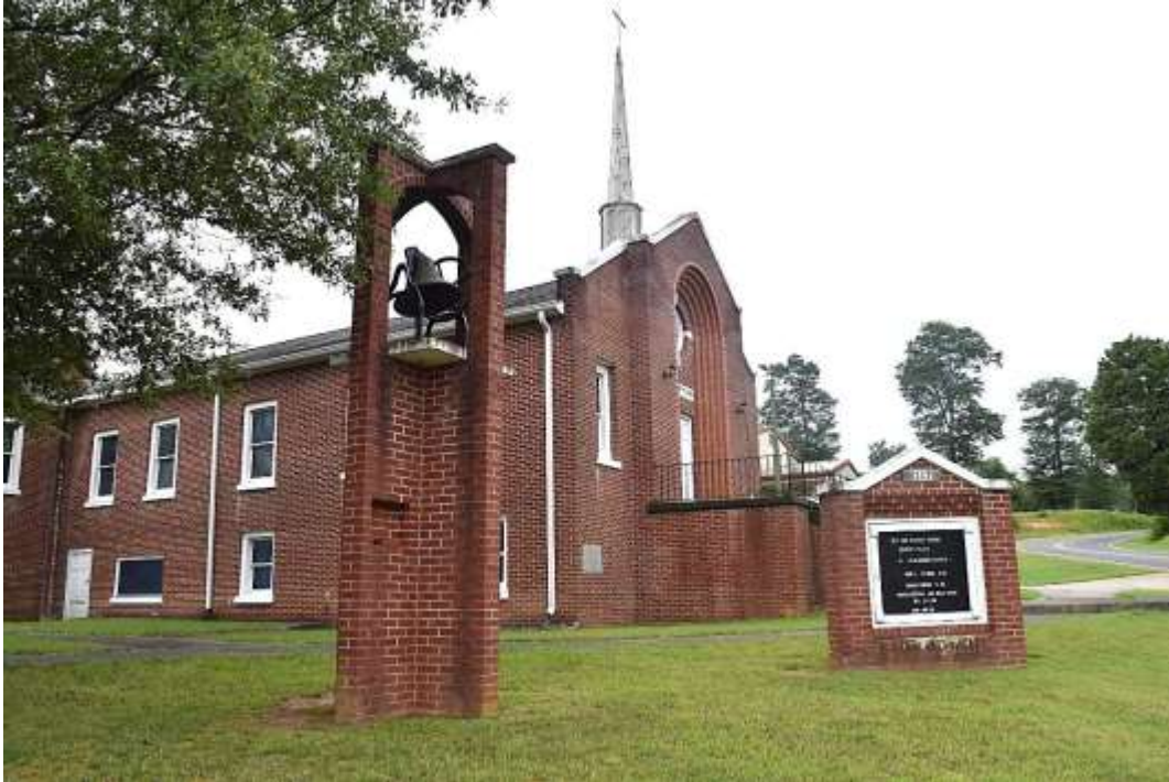
New Zion Baptist Church and Cemetery, Church, Belfry, and Church Sign, Looking West.
