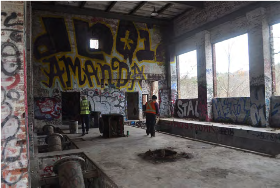
Plate 5.7: American ENKA Corporation Water Intake interior.
