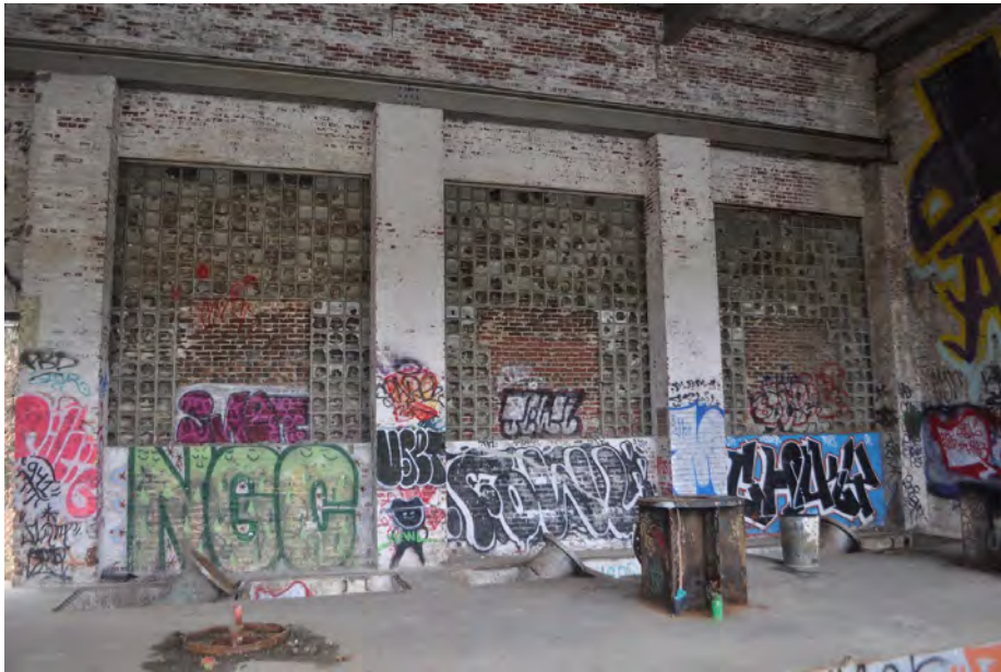
Plate 5.10: American ENKA Corporation Water Intake interior showing glass block windows infilled with brick.
