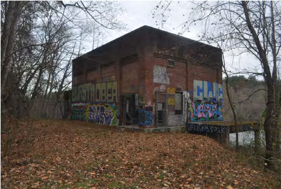
Plate 5.2: American ENKA Corporation Water Intake.
