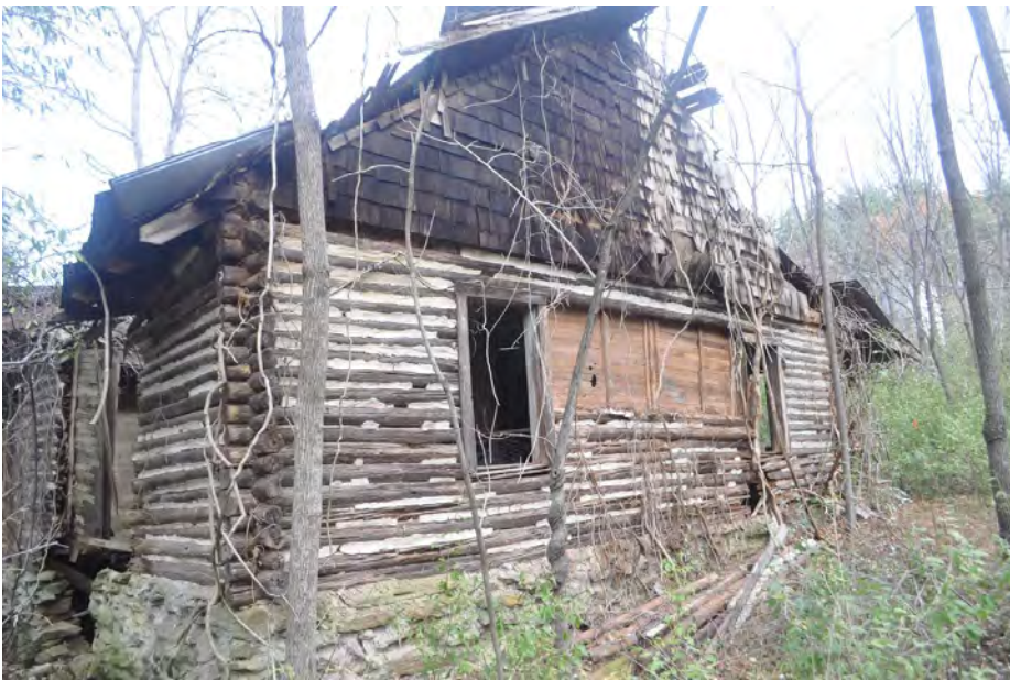
Plate 6.7: South and west sides of Log House.
