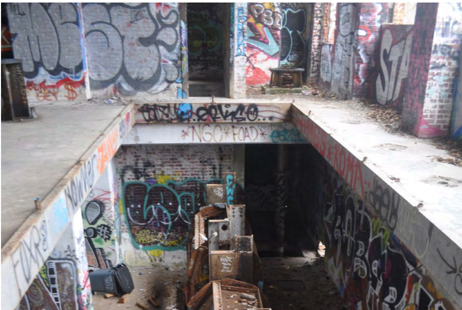
Plate 5.8: American ENKA Corporation Water Intake interior equipment.
