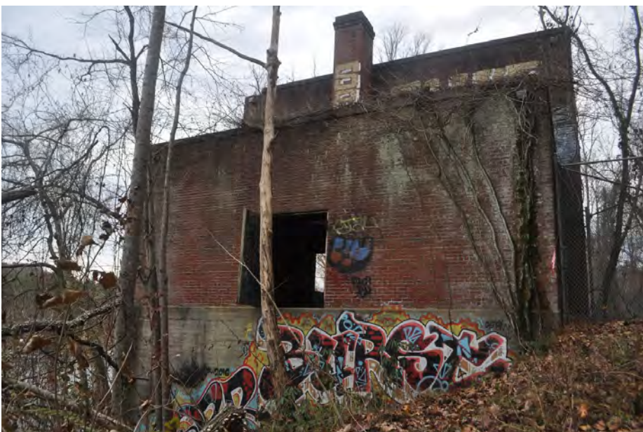
Plate 5.3: American ENKA Corporation Water Intake.
