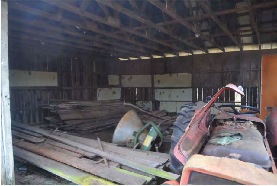
Plate 6.3: Shed interior. Photo view: South Photographer: Ellen Turco Date: November 20, 2019
