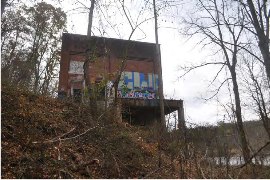
Plate 5.4: American ENKA Corporation Water Intake.
