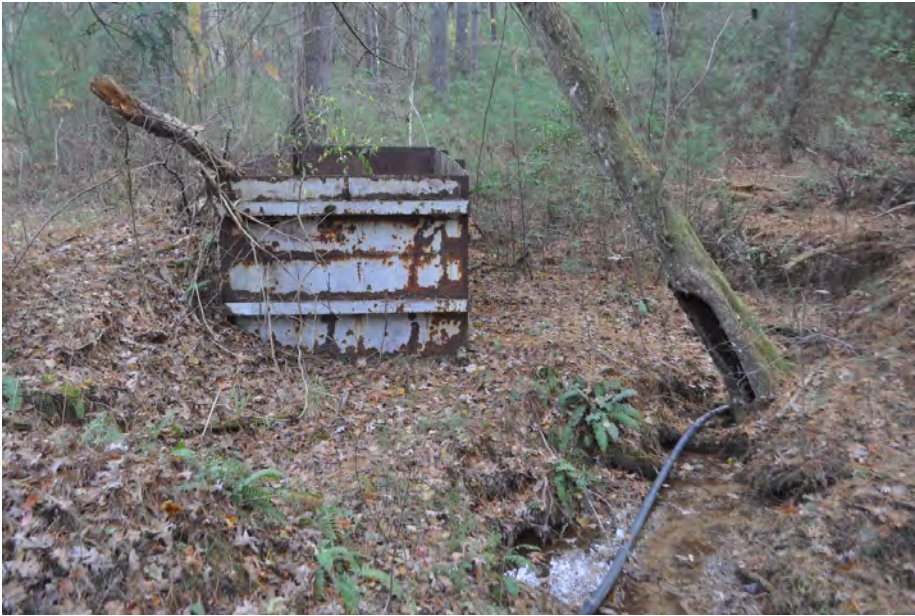
Plate 7.6: Metal box reservoir.
