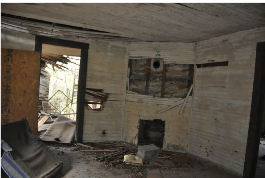
Plate 6.8: Log House interior, southeast front room.
