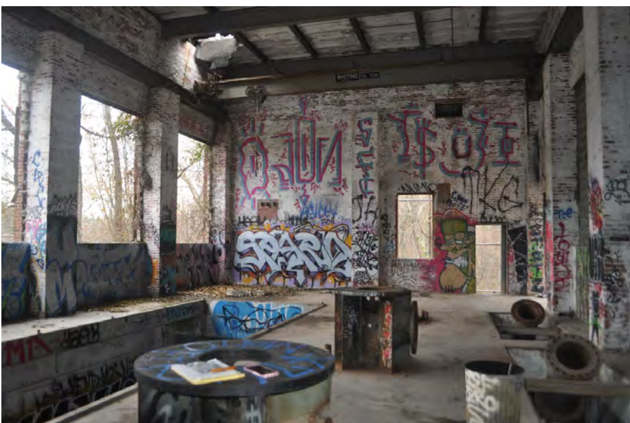
Plate 5.9: American ENKA Corporation Water Intake interior.
