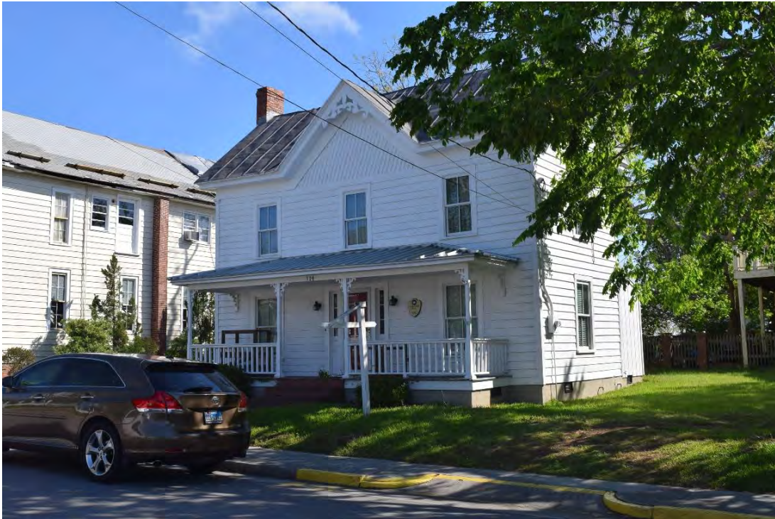
David G. Ward House, ca. 1902, 114 Street Main Street, Swansboro Historic District.
