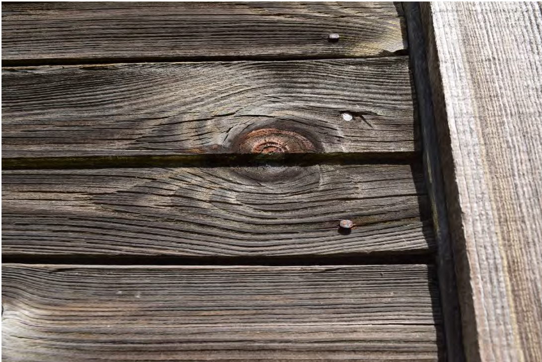
Edney Chapel School, Weatherboard Siding with Cut Nails.
