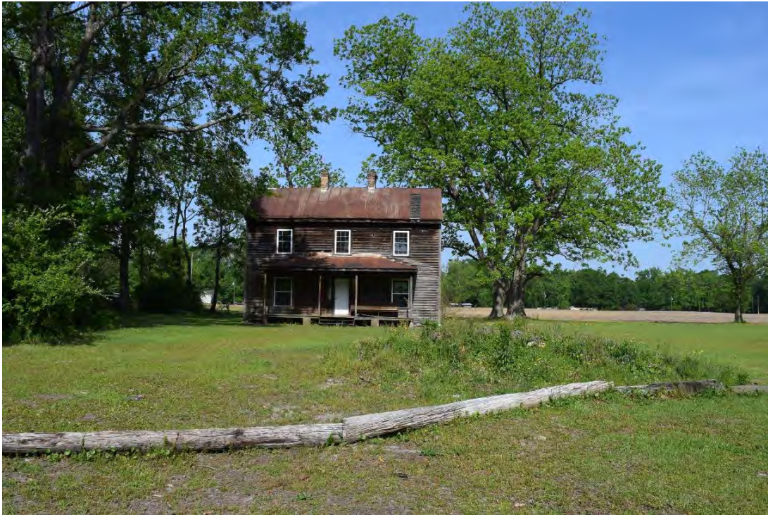
James S. and Sarah R. Heritage House, House and Setting, Looking East.
