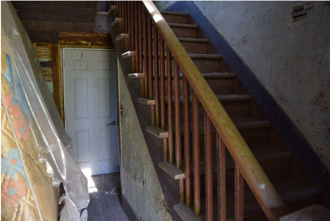
James S. and Sarah R. Heritage House, Interior, First-Floor Stair Hall.
