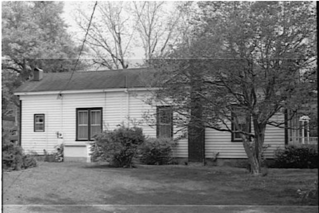
Jefferson D. Greer House, Side (North) Elevation. Survey Photograph. Source: HPO File, 1988.
