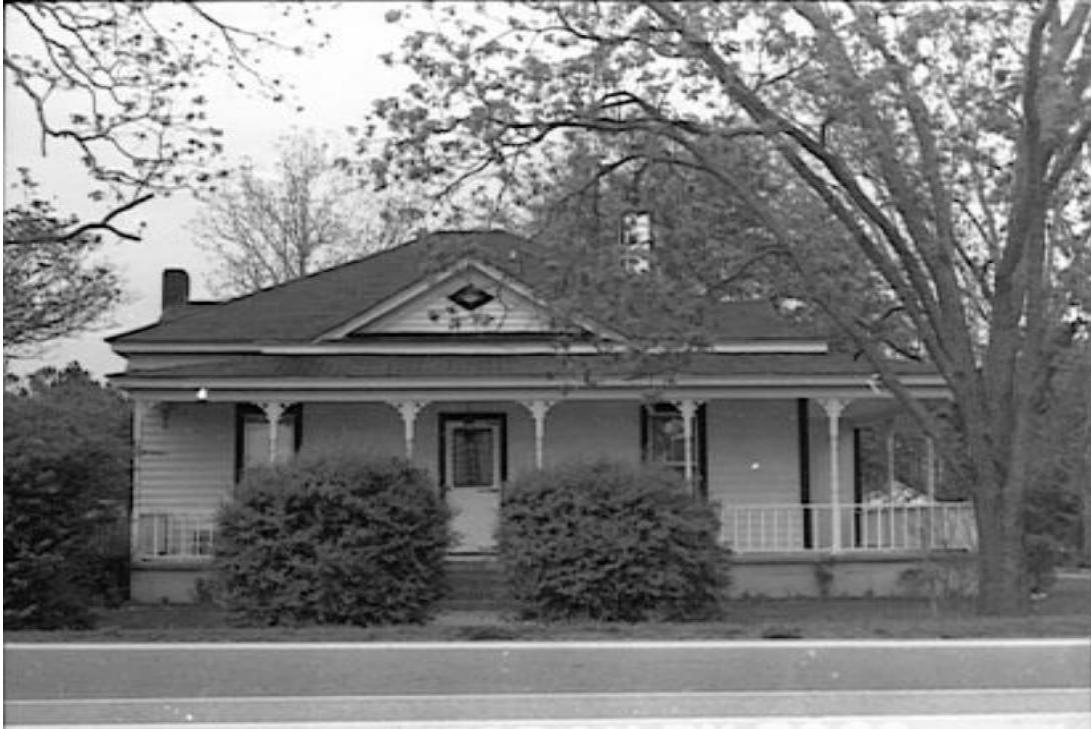
Jefferson D. Greer House, Façade. Survey Photograph. Source: HPO File, 1988.
