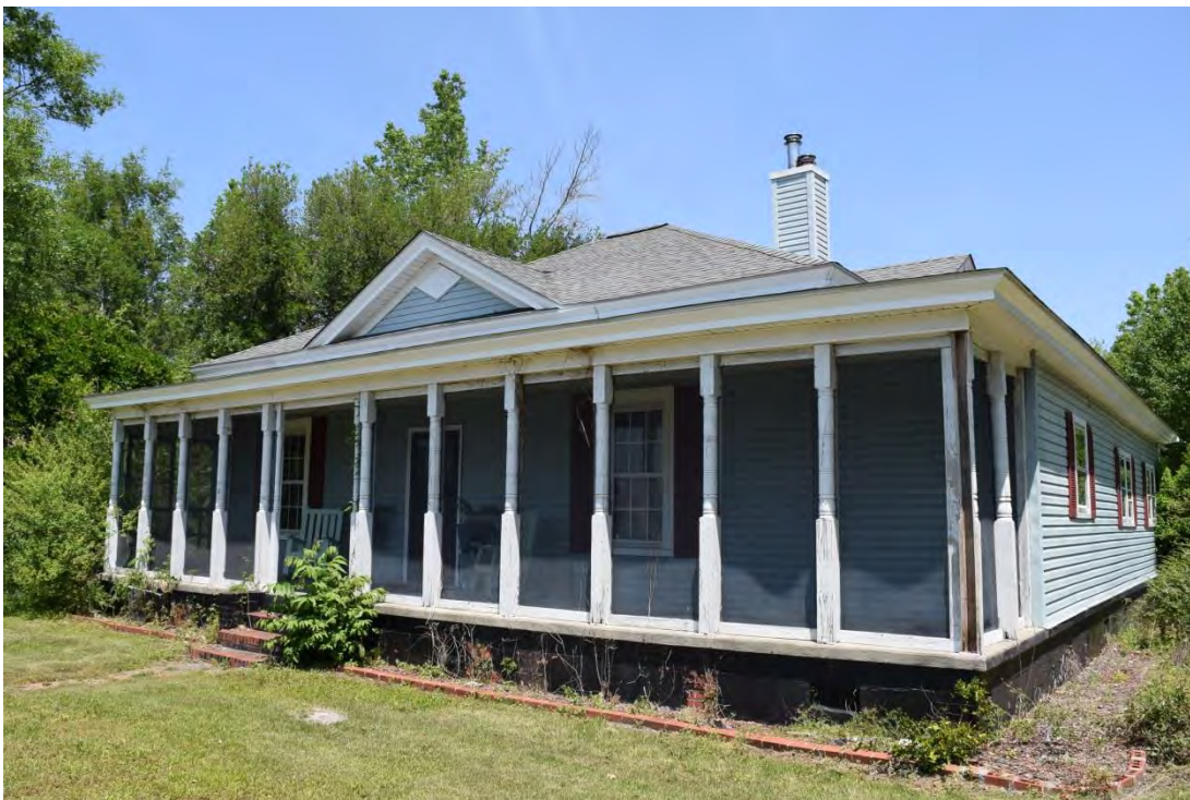
Jefferson D. Greer House, Façade, Looking East.
