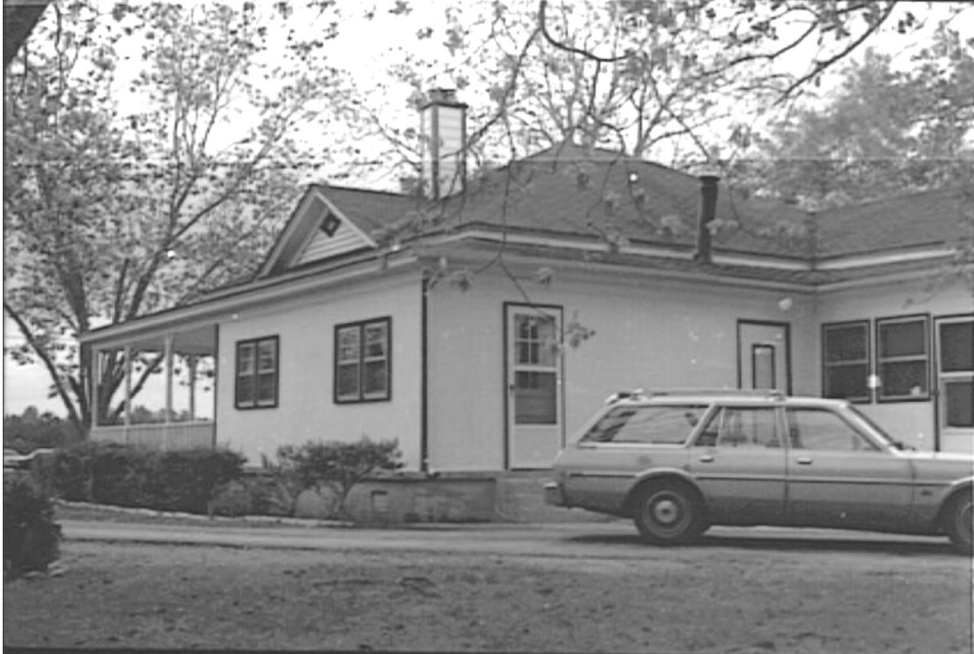
Jefferson D. Greer House, Side (South) and Rear (East) Elevations. Survey Photograph. Source: HPO File, 1988.
