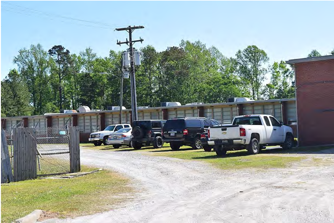
Silverdale Elementary School, Silverdale Vicinity, 1954 Rear Classroom Wing, Looking North.
