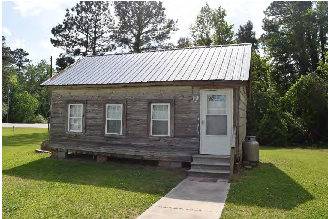
Edney Chapel School, Main (East) Elevation), Looking West.
