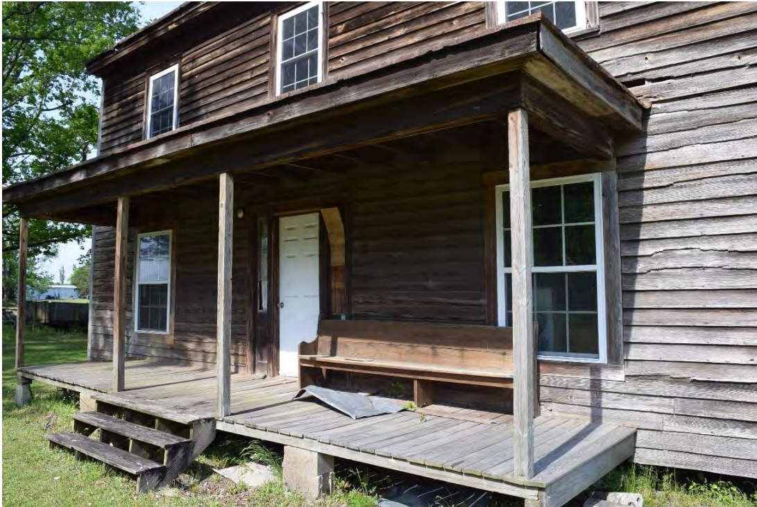
James S. and Sarah R. Heritage House, Façade, Looking East.
