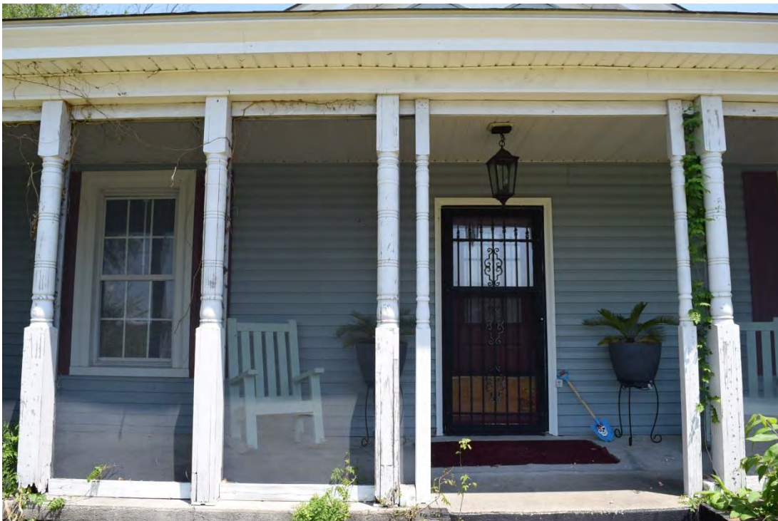
Jefferson D. Greer House, Façade, Showing Front Door, Porch Posts, and Replacement Windows.
