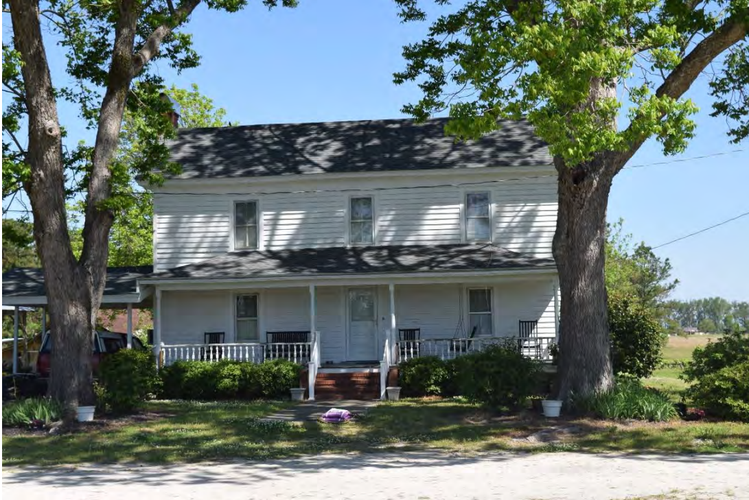
Benton House, ca. 1900, 386 Ramsey Road, Pumpkin Center Vicinity.
