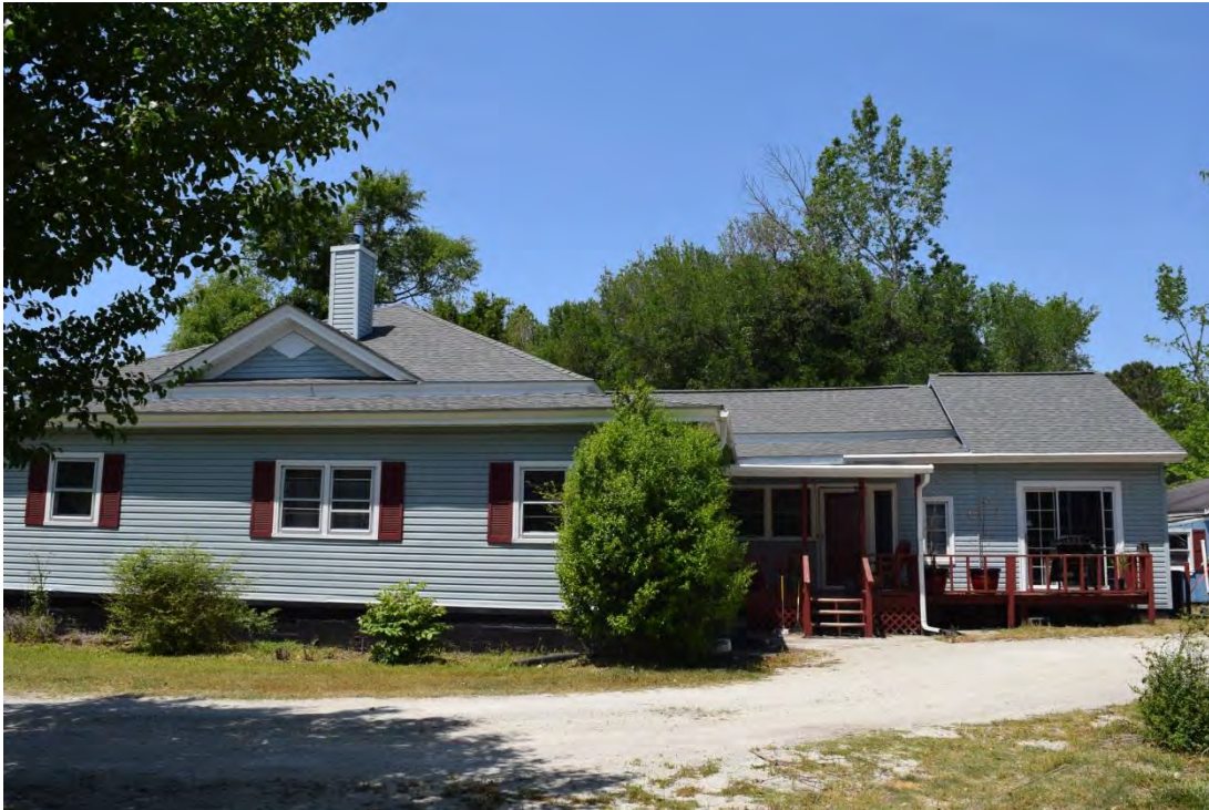
Jefferson D. Greer House, Side (South) Elevation, Rear Ell, and Rear Extension, Looking North.
