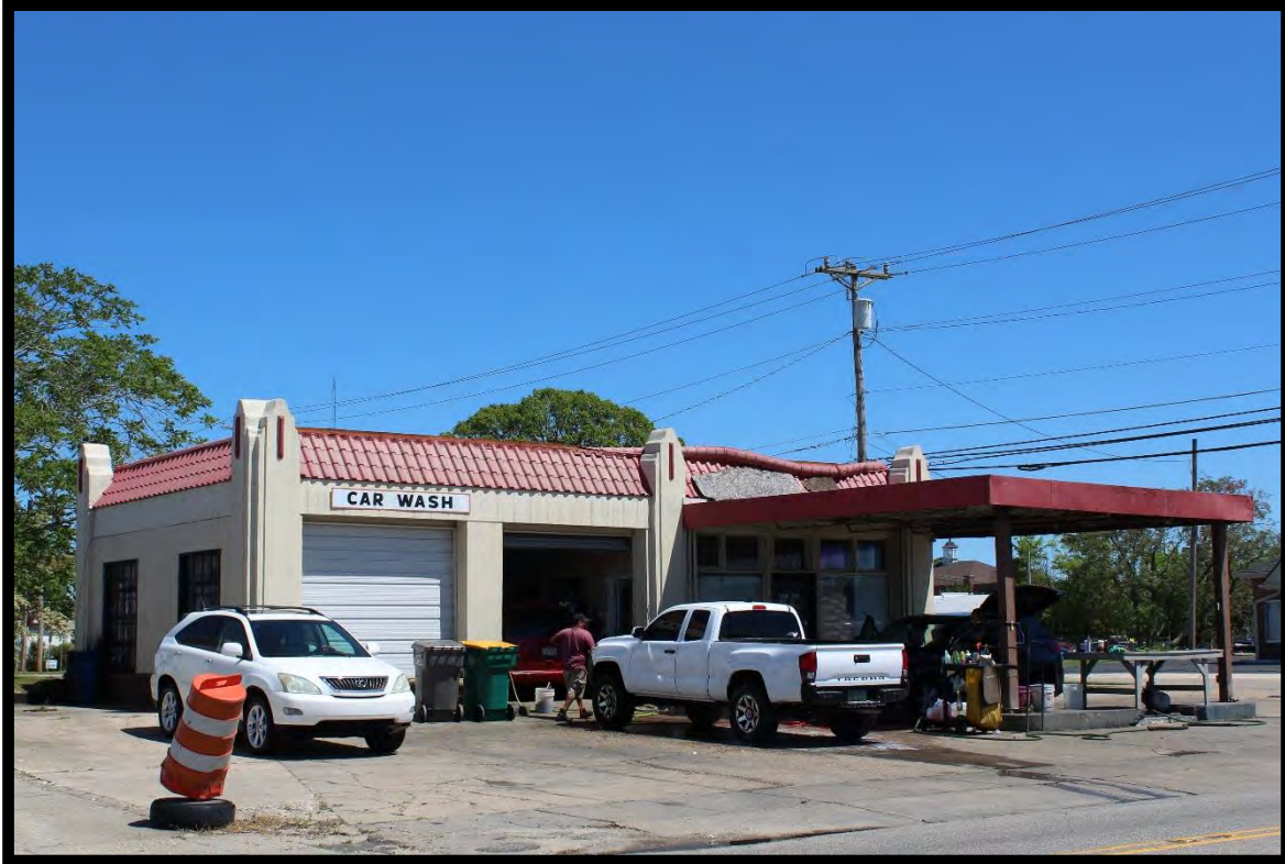
Figure 64: Gas Station (RB0230), Looking Northeast.
