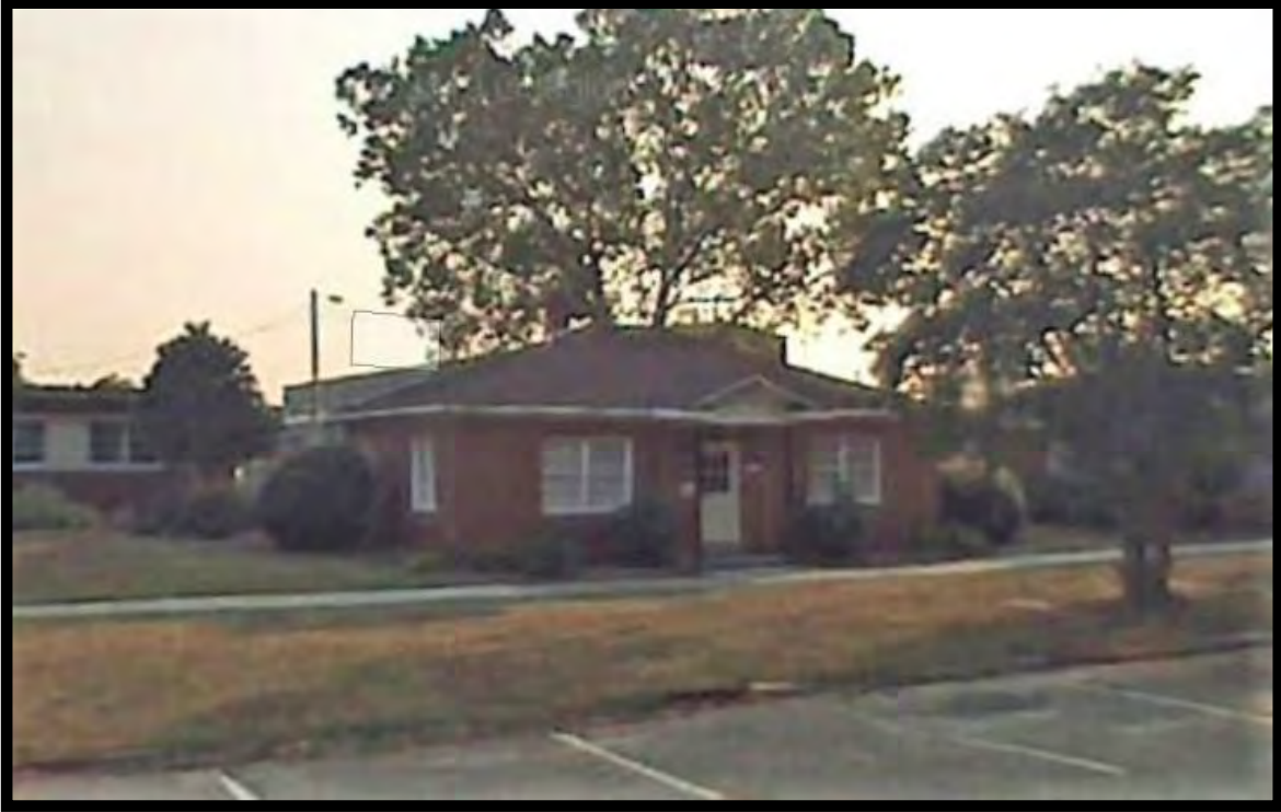
Figure 139: Demolished Building on Transportation Drive, Fayetteville, NC, Looking Southwest (Google Streetview).
