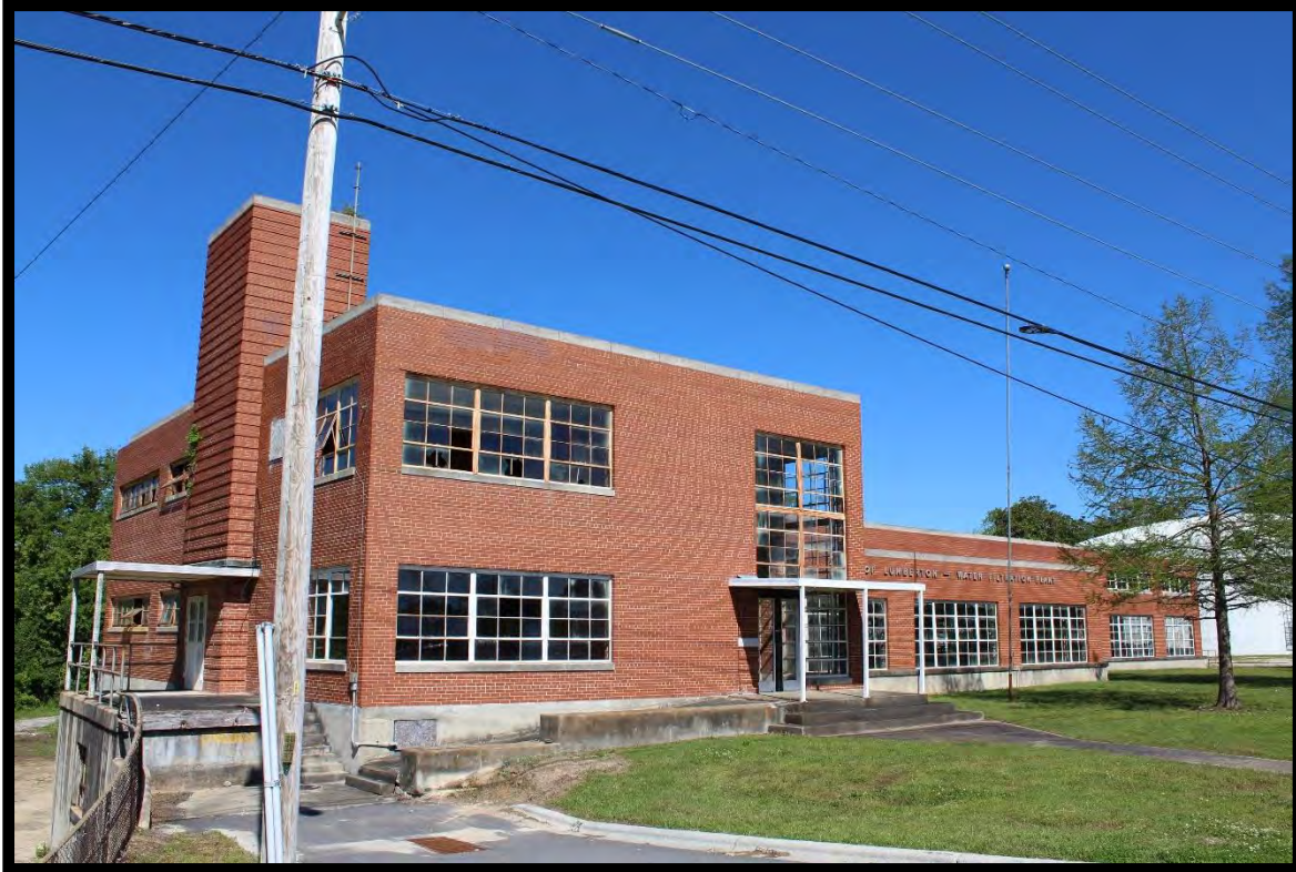
Figure 17: Lumberton Water Treatment Plant, Looking Northwest.
