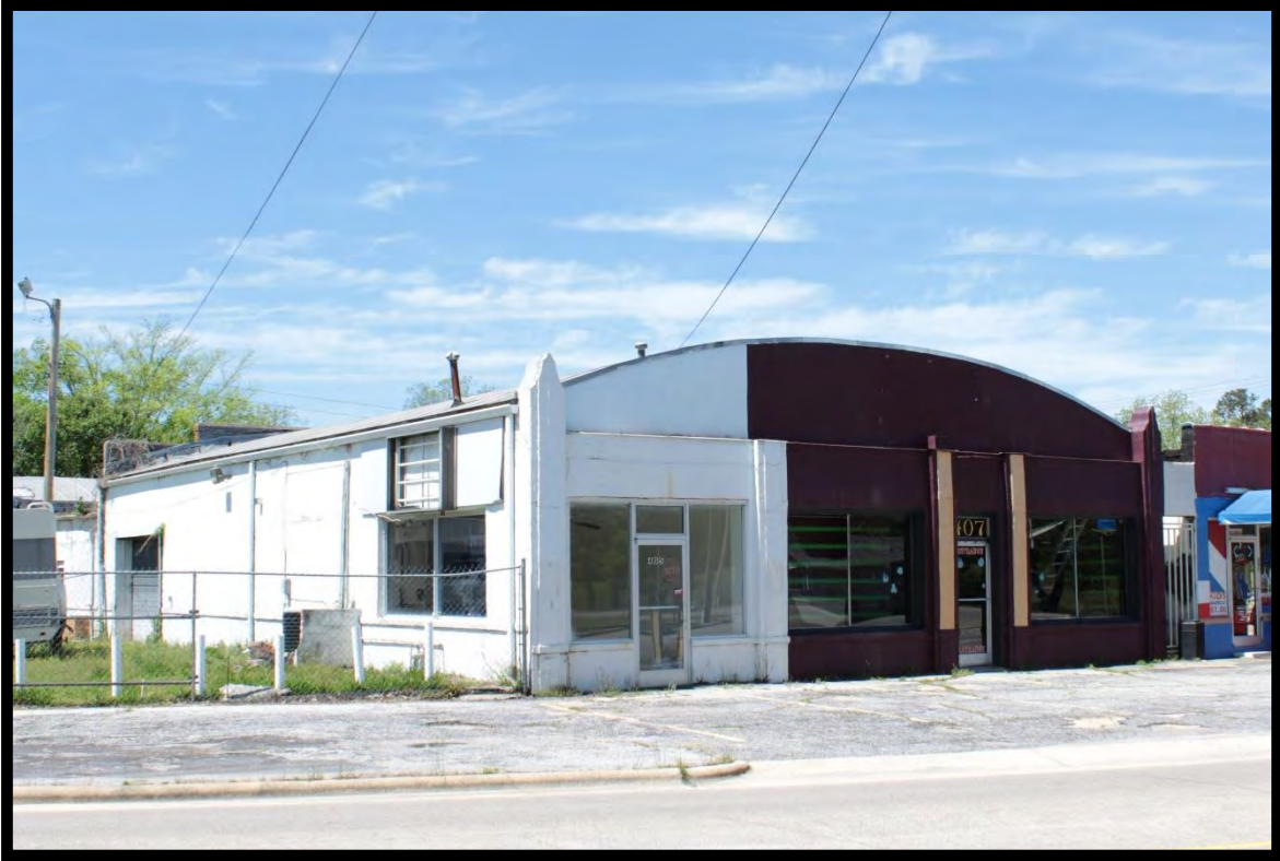
Figure 49: West Fifth Street Stores, Looking Northwest.
