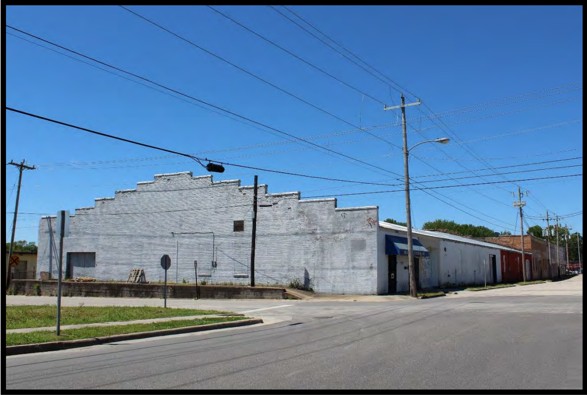
Figure 95: Warehouses (RB0466), Looking Southwest.
