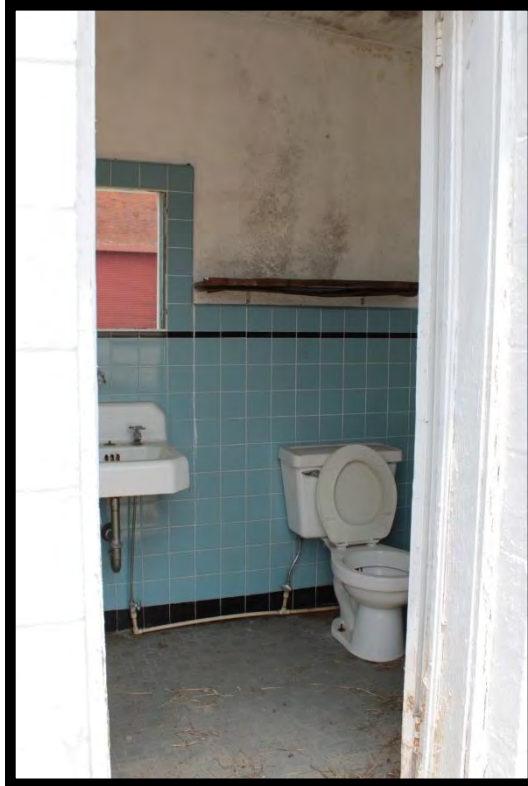
Figure 119: Filling Station, Restroom, Looking Northeast.
