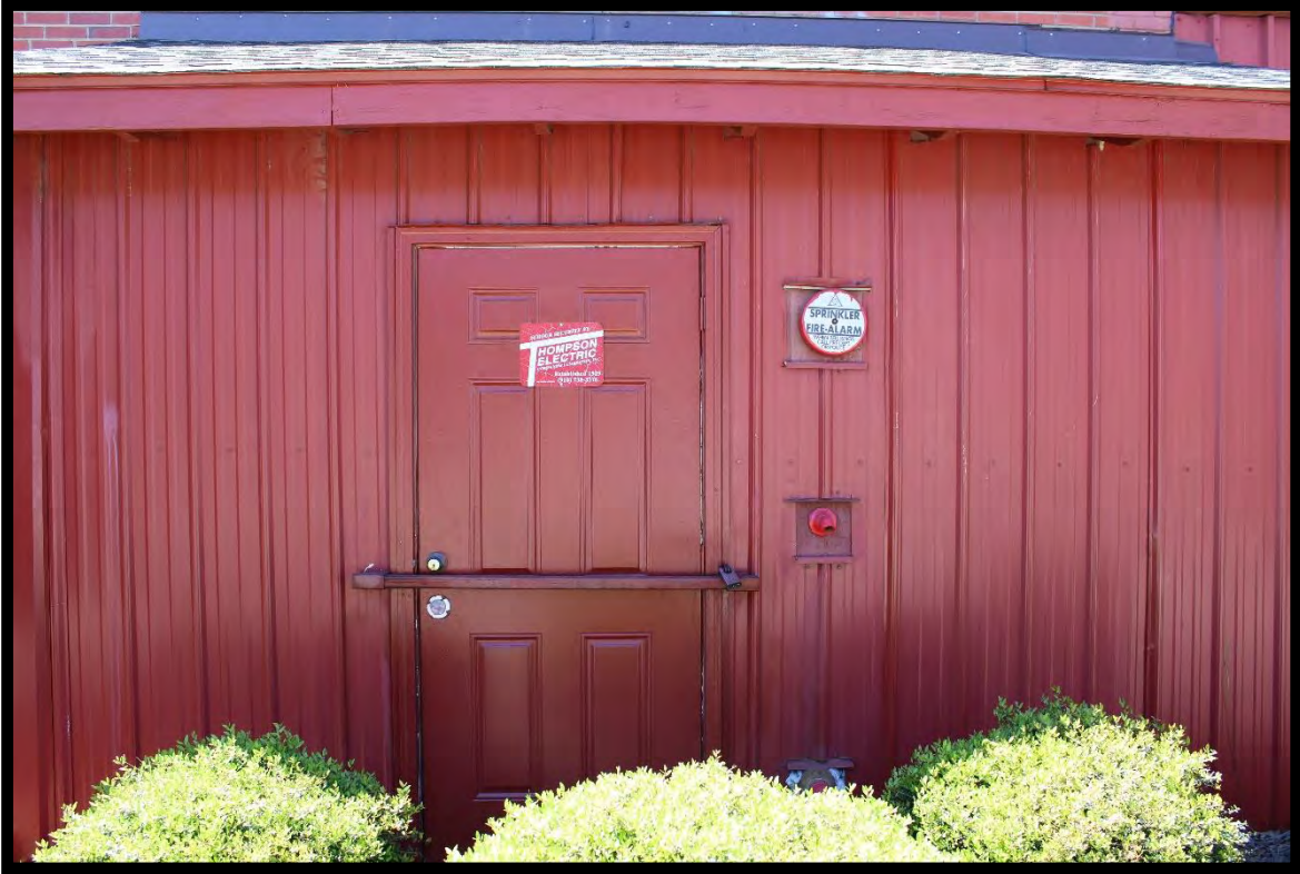
Figure 81: Planters Warehouse, Typical Door, Looking Southwest.
