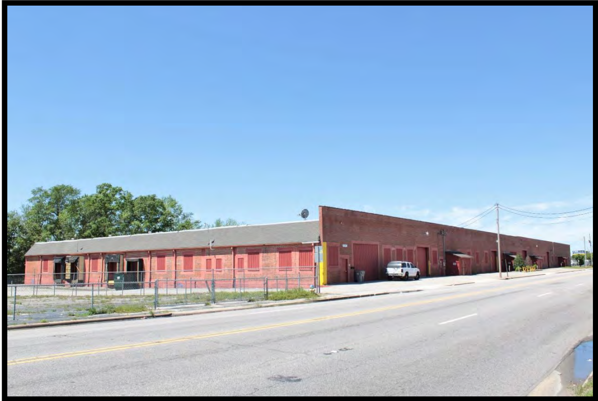
Figure 79: Planters Warehouse, Looking Southwest.
