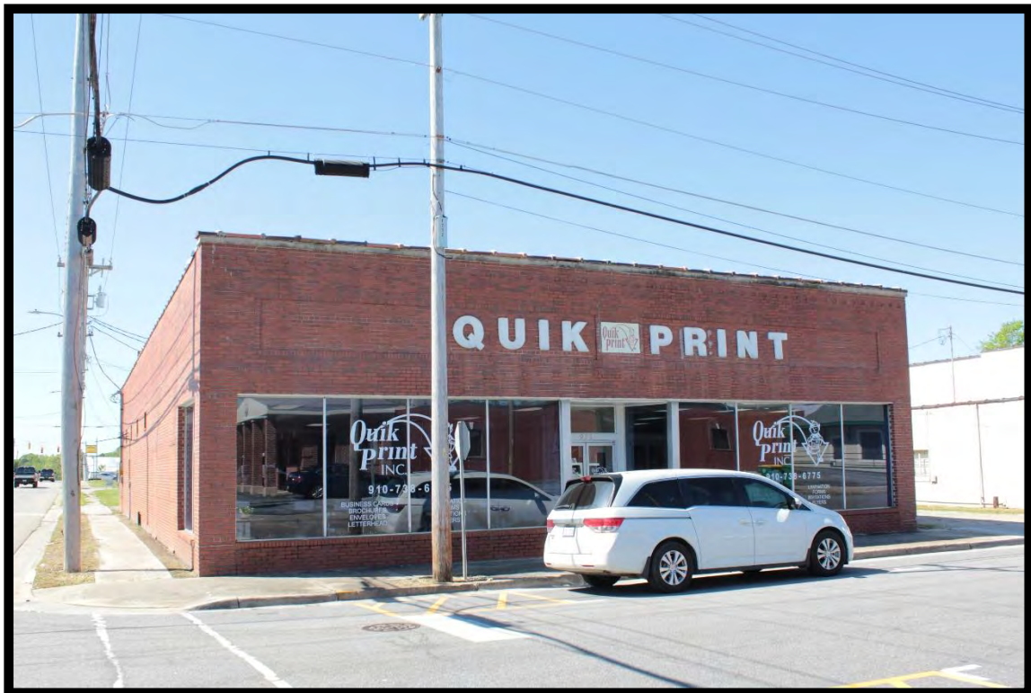
Figure 16: Store, 232 East 4 th Street (RB0246), Looking Southwest.
