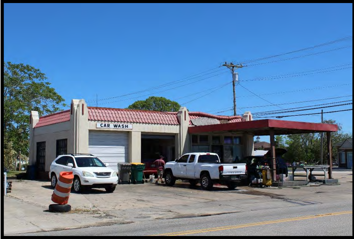
Figure 124: Gas Station (RB0230), Looking Northeast.
