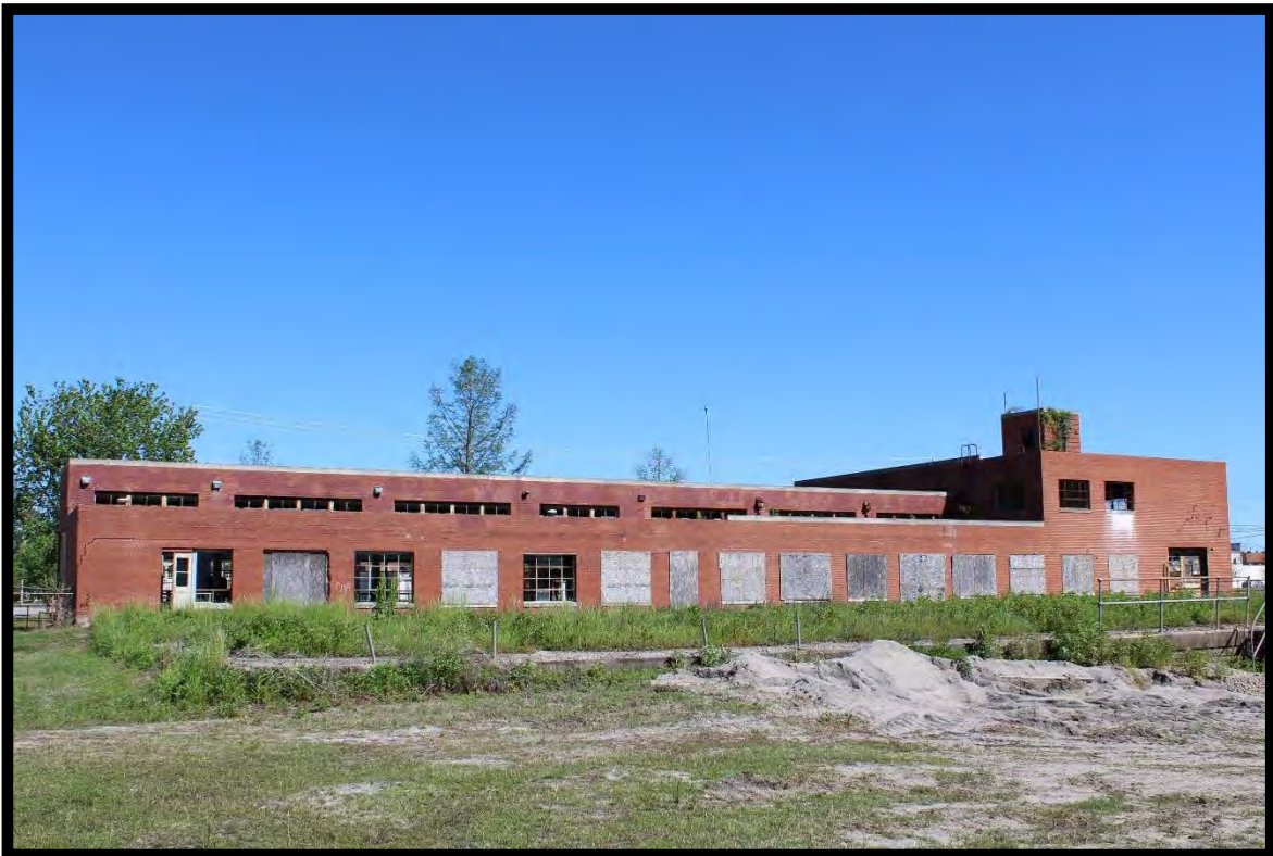
Figure 24: Lumberton Water Treatment Plant, Looking Southeast.
