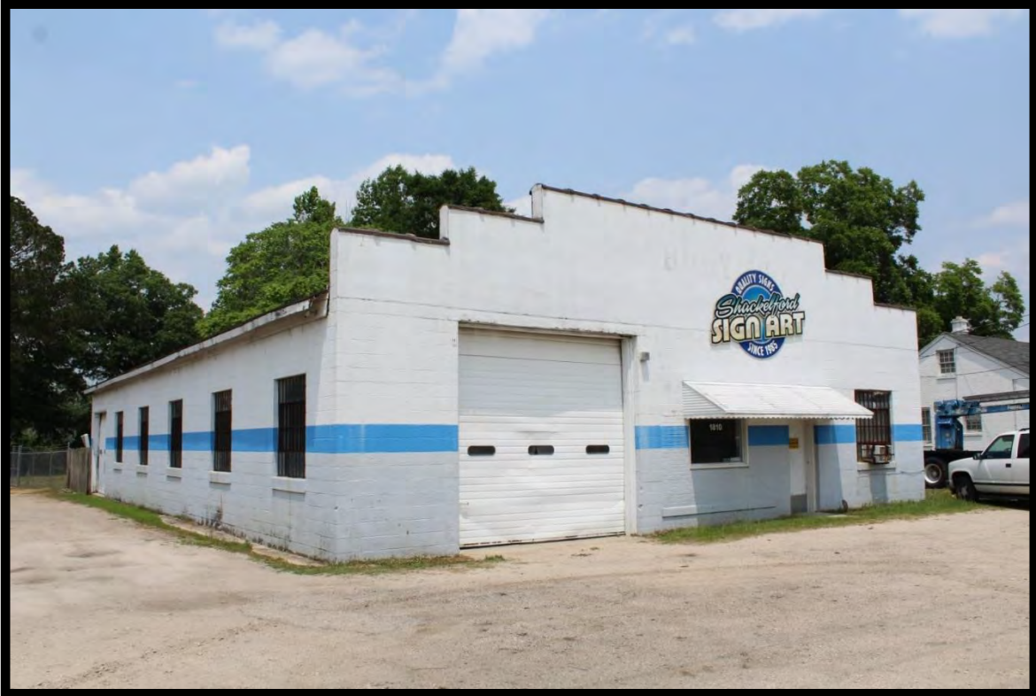
Figure 122: 1810 West 5 th Street, Lumberton, NC, Looking East.
