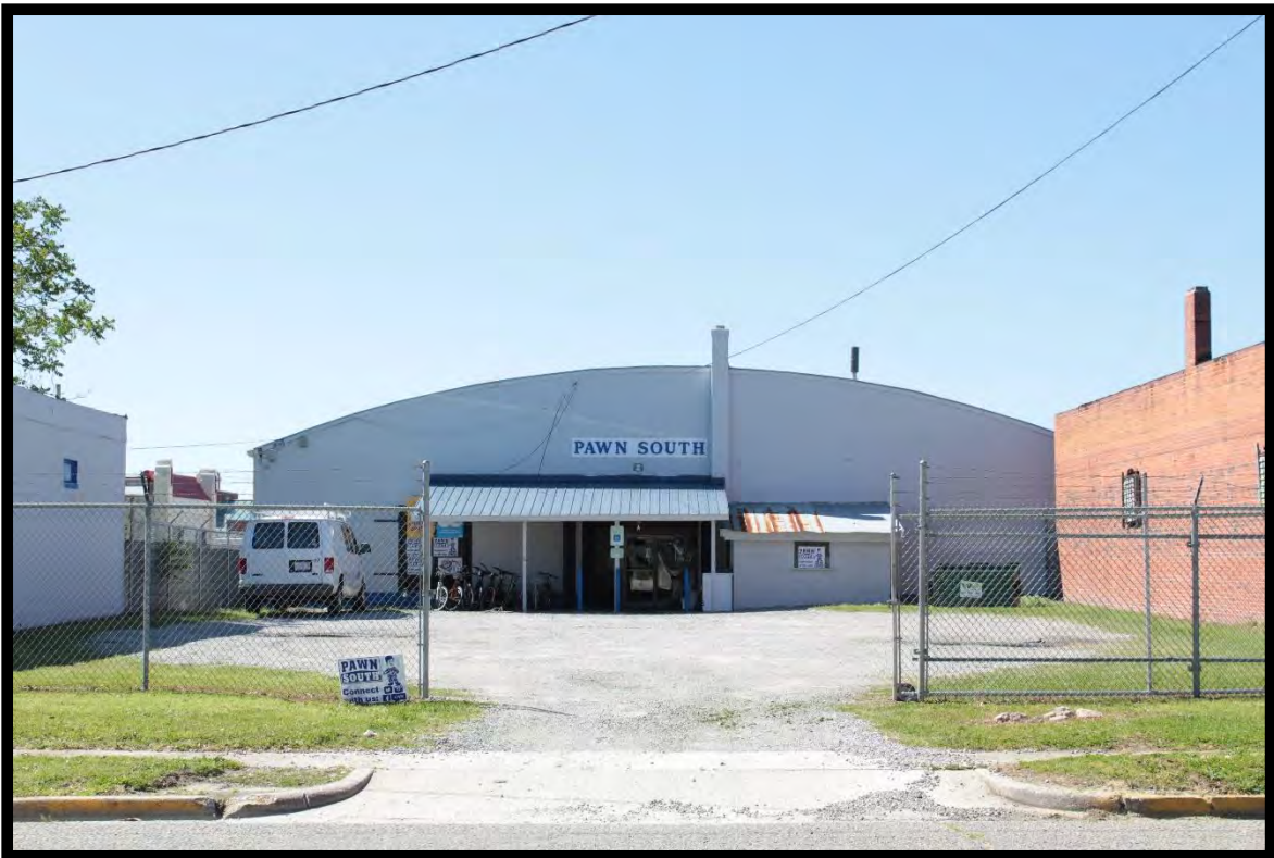
Figure 63: Store (RB0229), Looking South.
