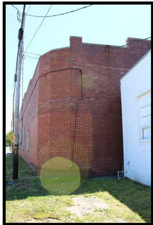
Figure 100: Automobile Sales Center, Looking Southeast.
