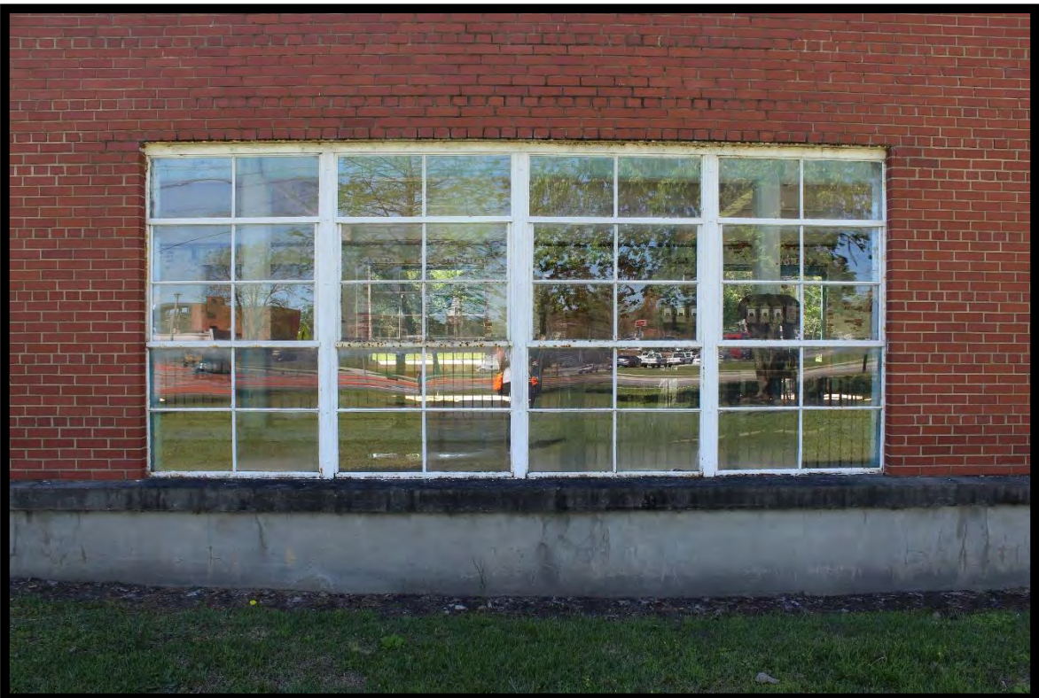
Figure 23: Lumberton Water Treatment Plant, Typical Windows.
