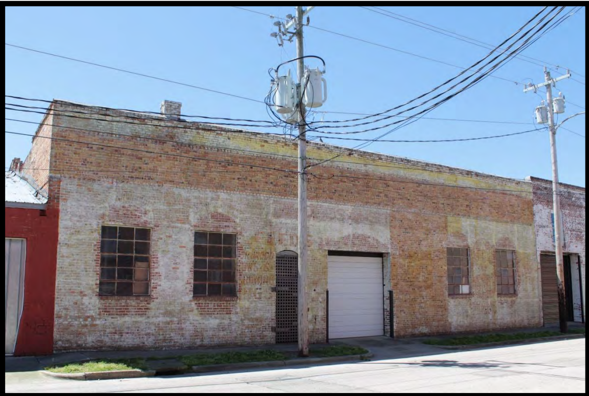
Figure 96: Warehouses (RB0466), Center Warehouse, Looking Southwest.
