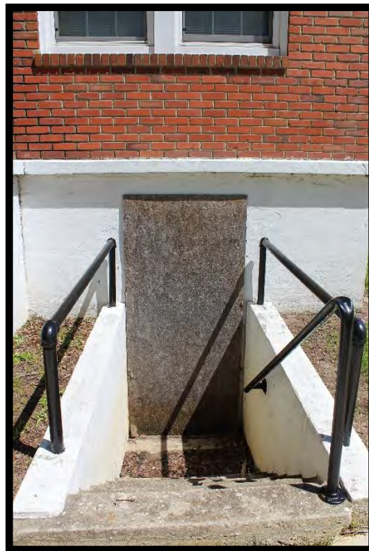
Figure 129: NCDOT Office, Looking South.
