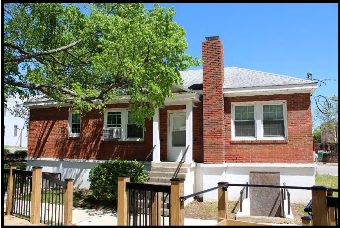
Figure 128: NCDOT Office, Looking South.
