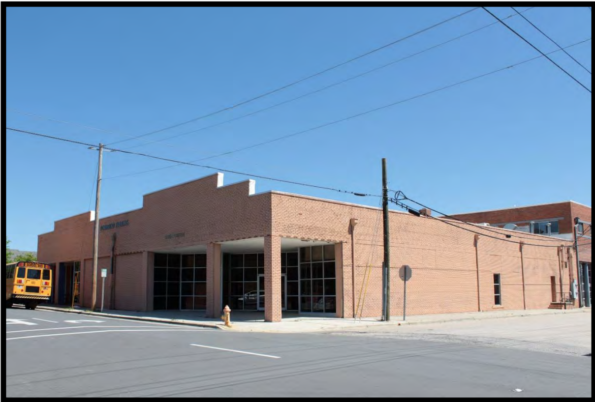
Figure 94: Warehouse (Lumberton Trading) (RB0163), Looking Northeast.
