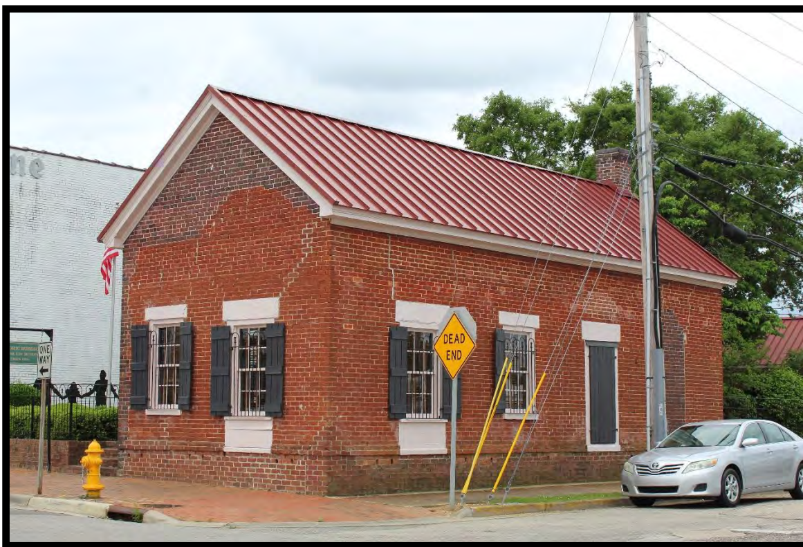
Figure 110: Proctor Law Office (RB0179), Looking Southwest.
