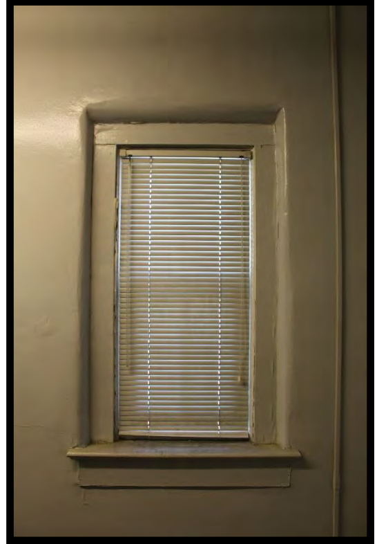
Figure 136: NCDOT Office, Typical Window.
