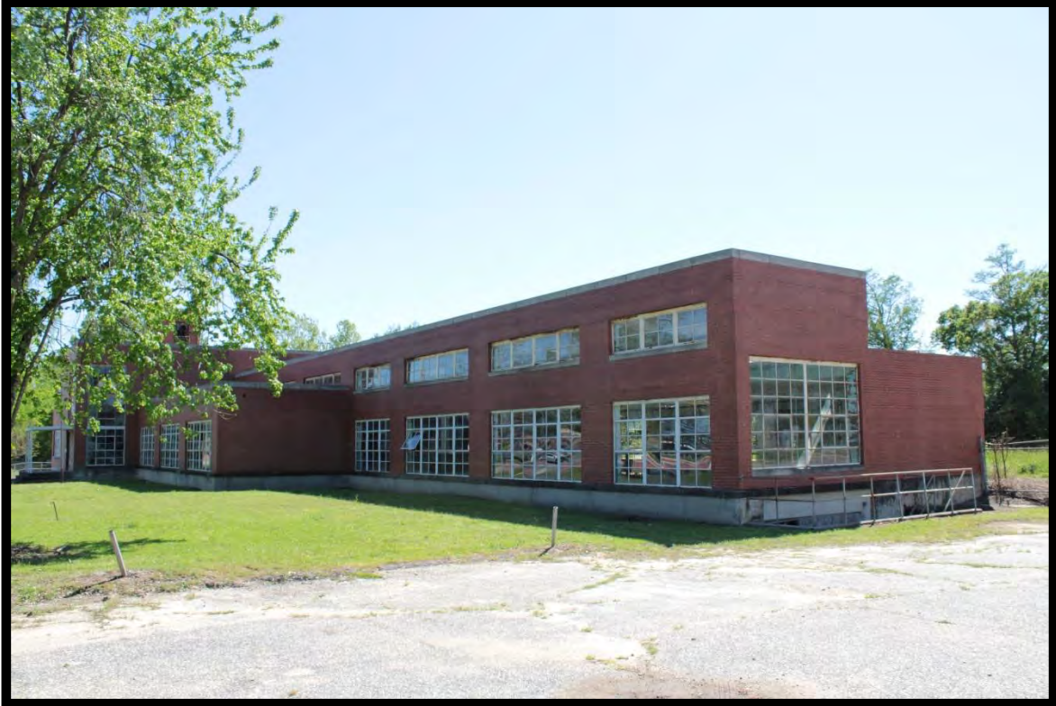
Figure 22: Lumberton Water Treatment Plant, Looking Southwest.
