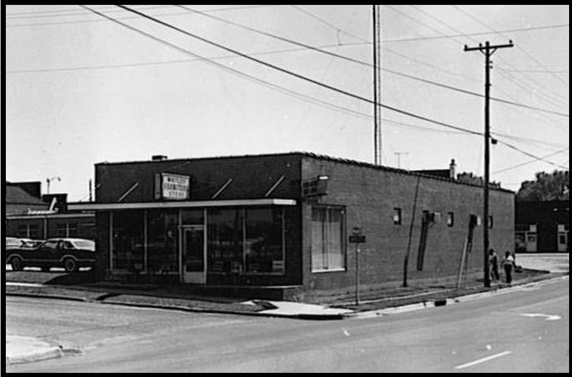
Figure 12: Whitley Furniture Company, Looking Southeast (Survey File, RB0234, 1979).
