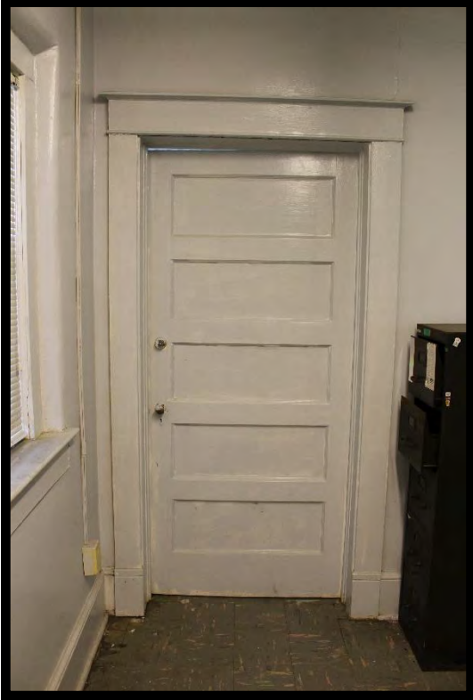
Figure 135: NCDOT Office, Typical Wooden Door.
