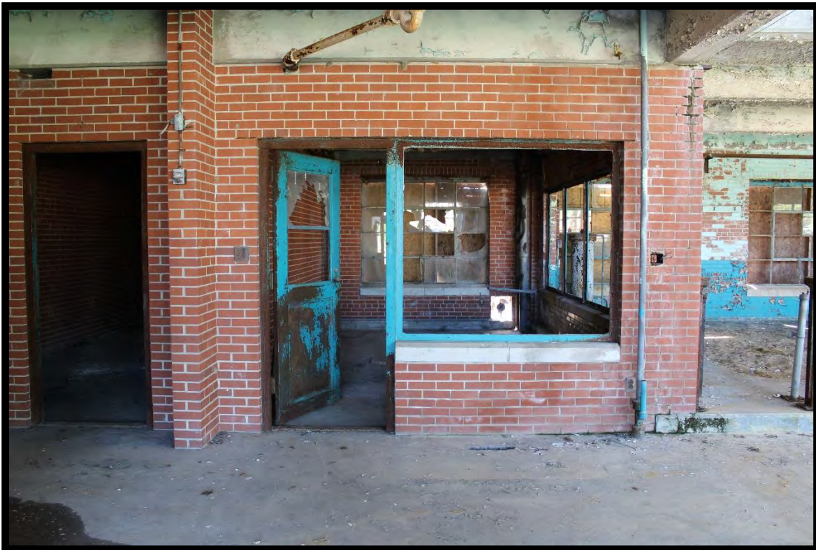
Figure 28: Lumberton Water Treatment Plant, Interior, Office.
