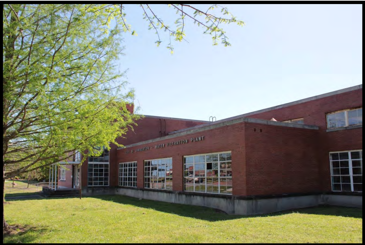
Figure 21: Lumberton Water Treatment Plant, Looking Southwest.
