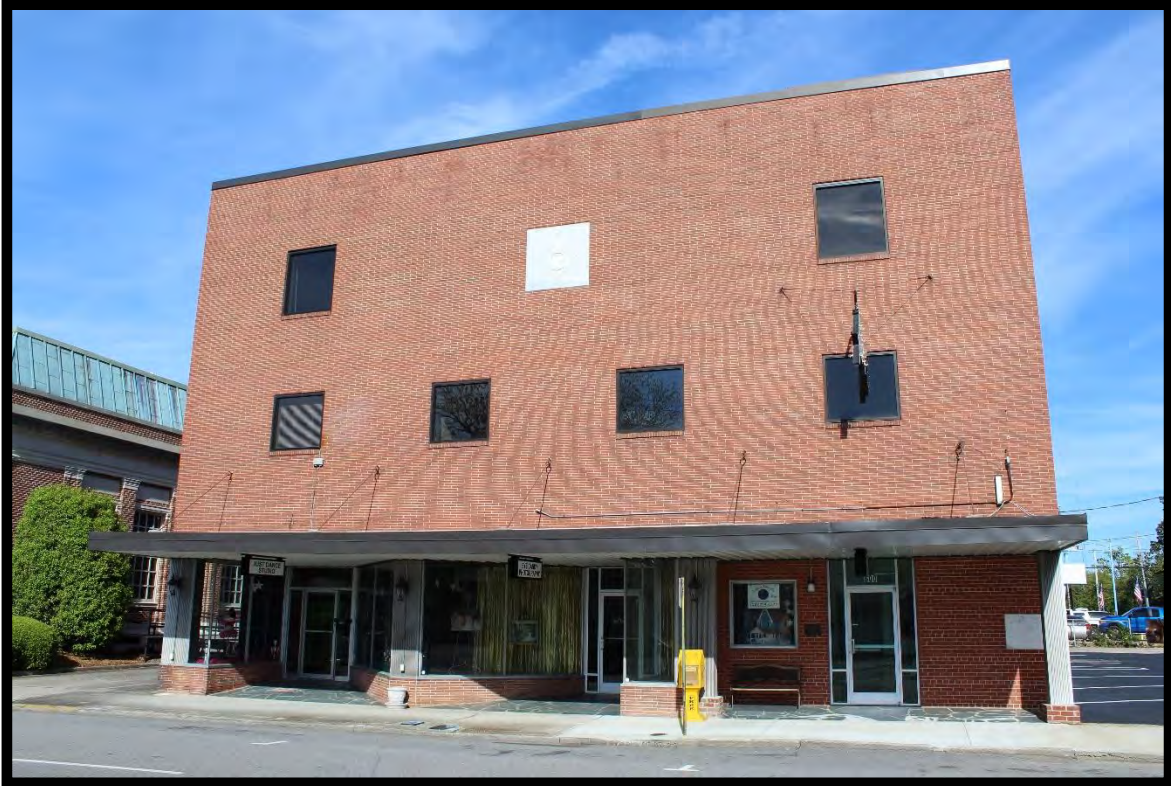
Figure 78: Masonic Building (RB0164), Looking Northeast.
