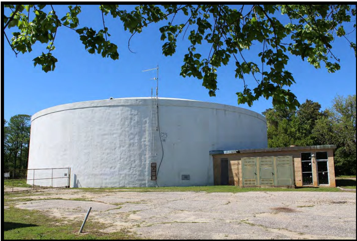
Figure 32: Lumberton Water Treatment Plant, Water Tank and Mechanical Building, Looking Northwest.
