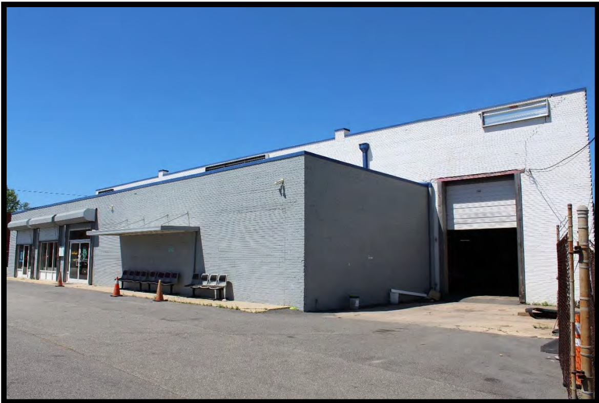
Figure 103: Automobile Sales Center, Looking Southeast.
