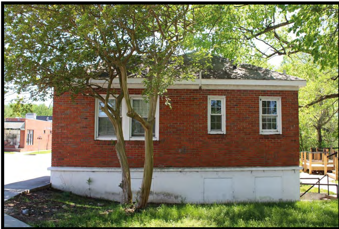
Figure 127: NCDOT Office, Looking South.
