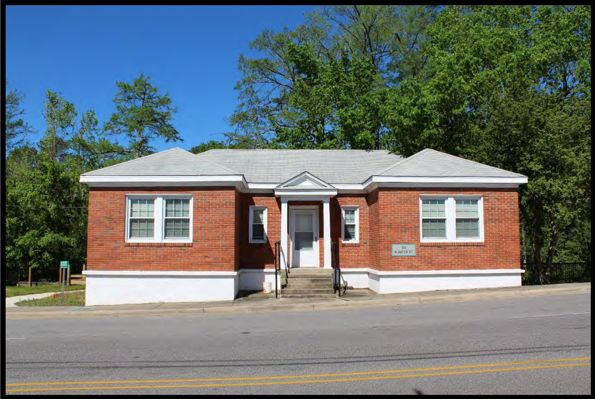
Figure 125: NCDOT Office, Looking West.
