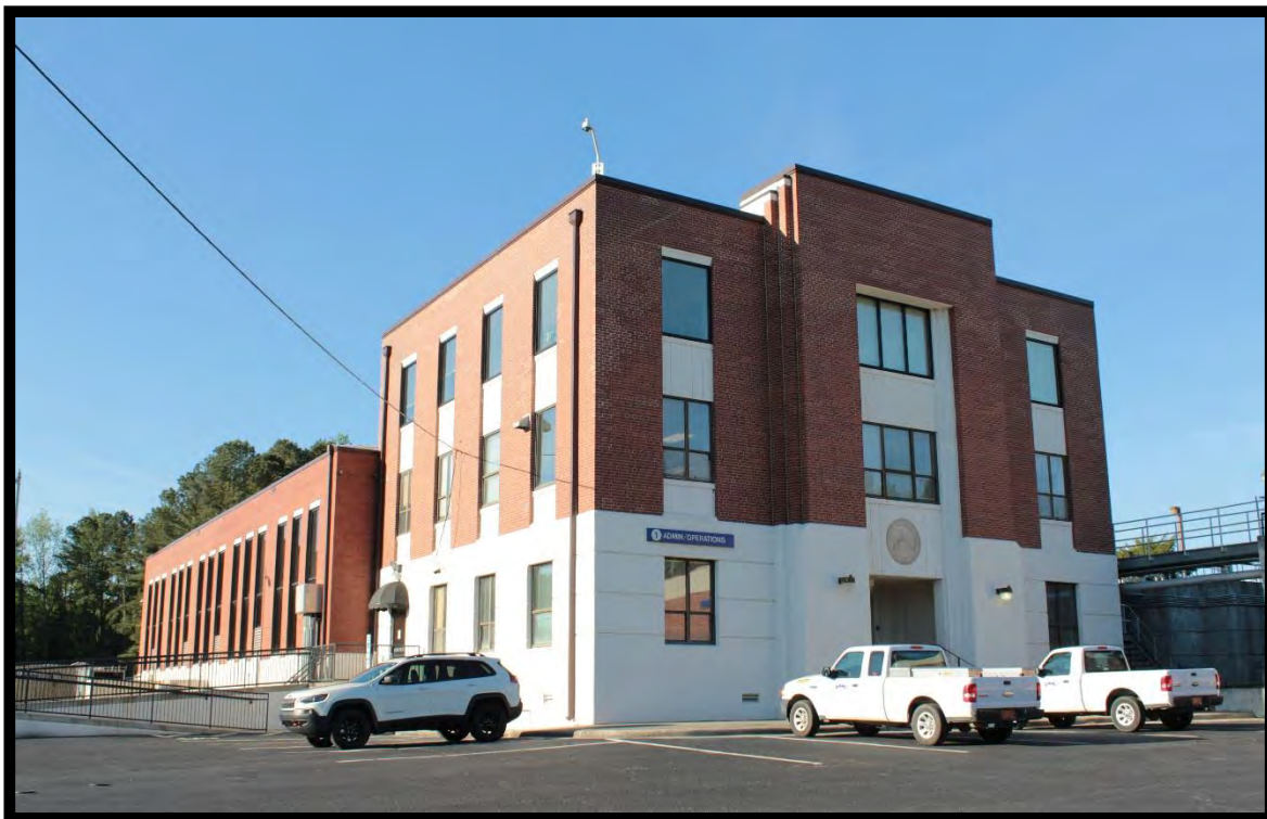
Figure 41: Glenville Water Treatment Plant, 628 Filter Plant Drive, Fayetteville, North Carolina, Looking Northeast.
