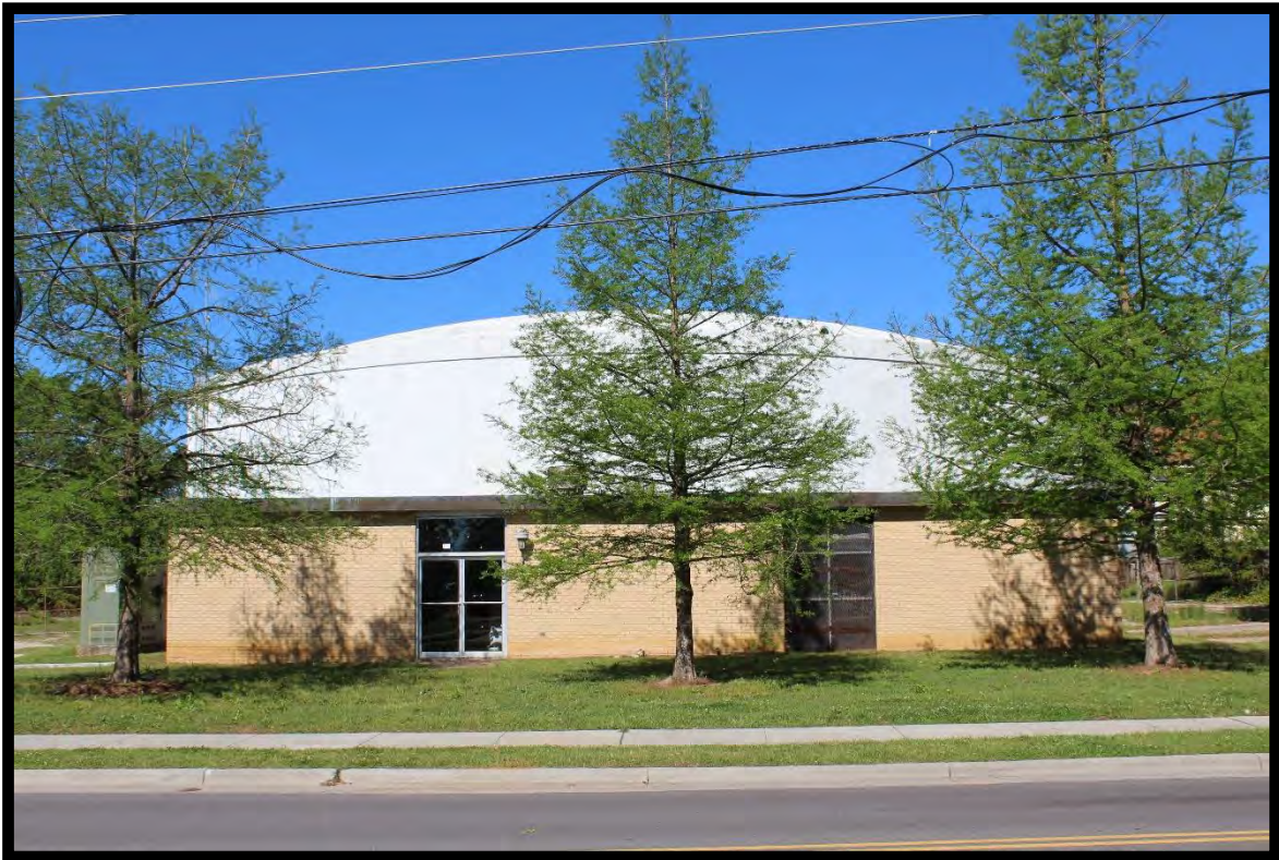
Figure 33: Lumberton Water Treatment Plant, Water Tank and Mechanical Building, Looking West.
