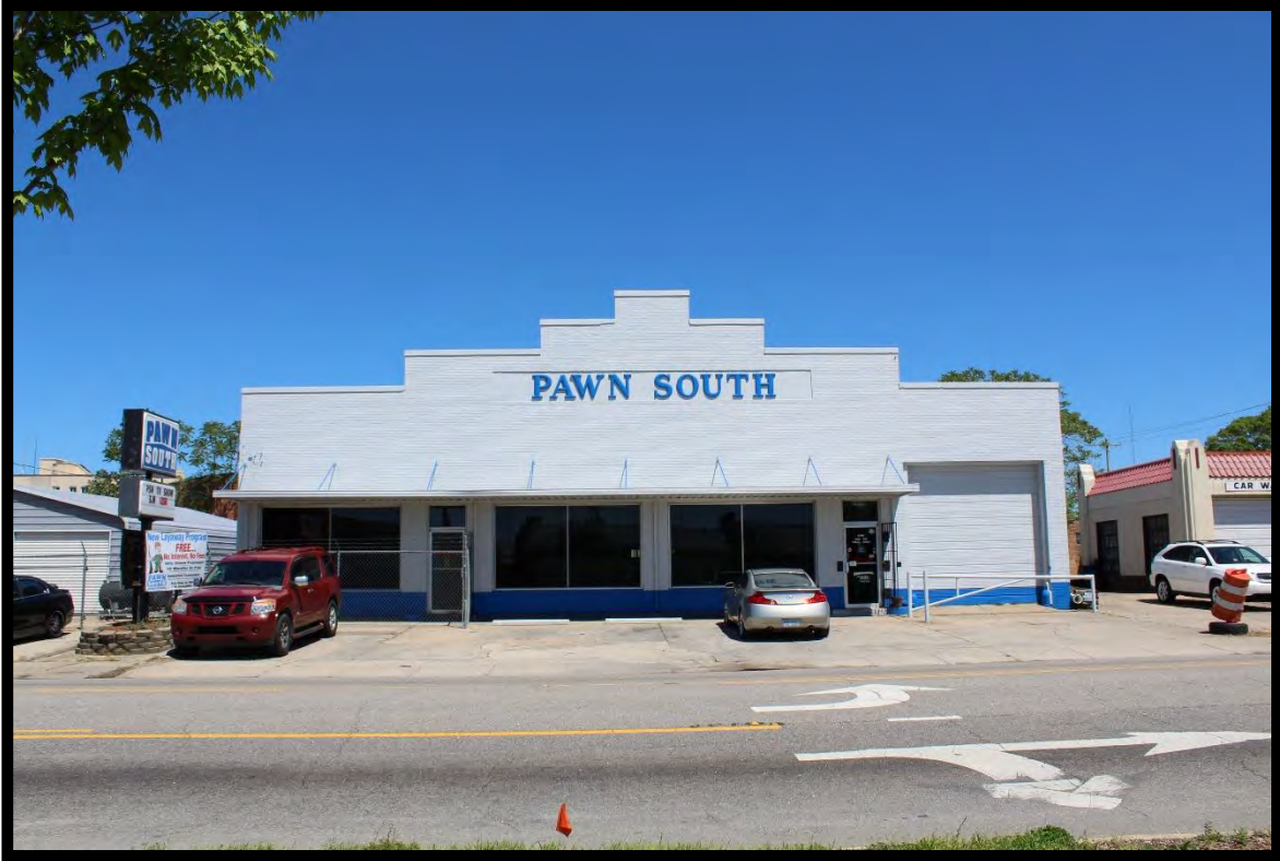
Figure 62: Store (RB0229), Looking North.
