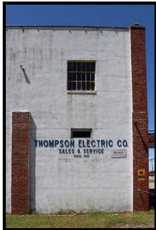
Figure 72: Thompson Electric Company, Sign, Looking West.
