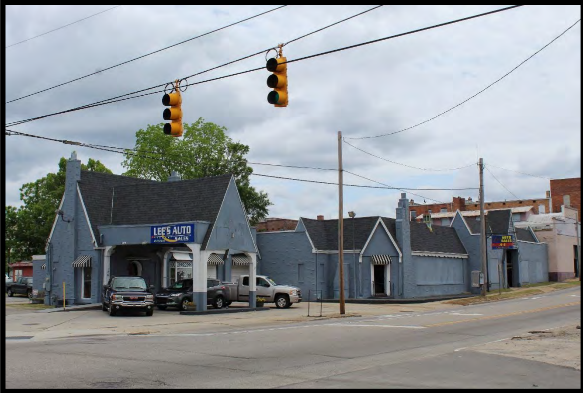
Figure 111: Pure Oil Filing Station (RB0180), Looking Northeast.
