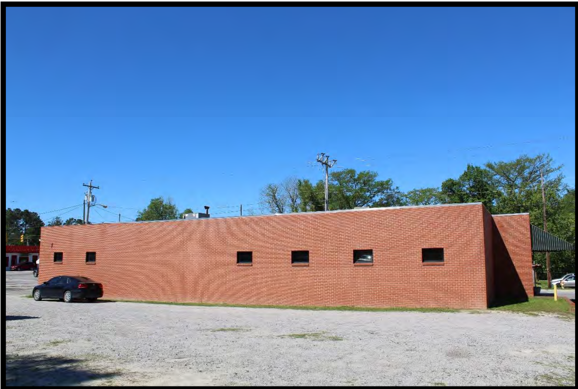
Figure 7: Whitley Furniture Company, Looking Southwest.
