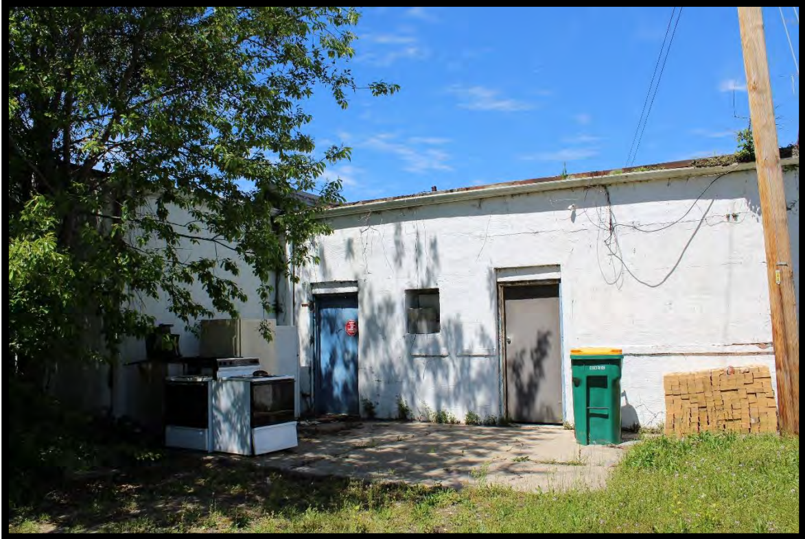
Figure 50: West Fifth Street Stores, Looking Northwest.
