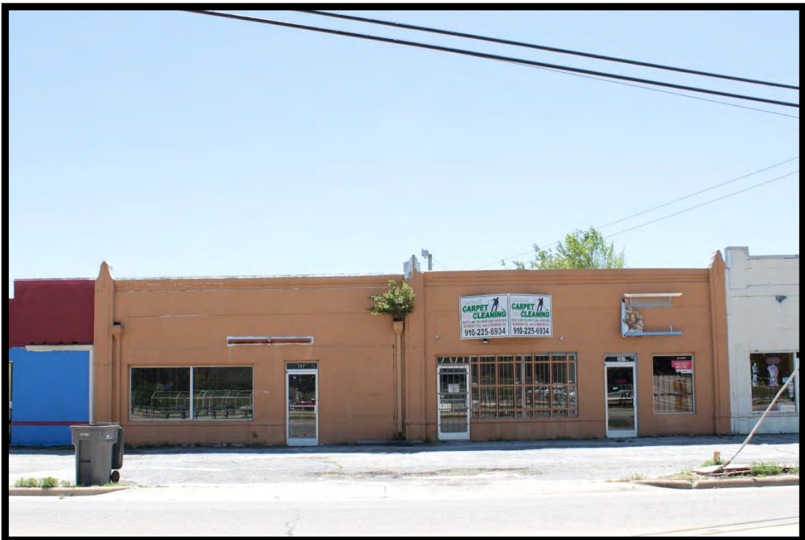
Figure 51: West Fifth Street Stores, Looking South.
