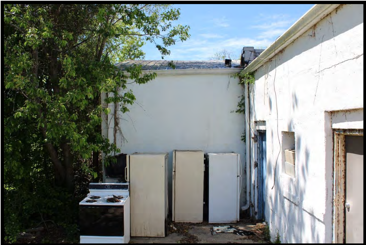
Figure 48: West Fifth Street Stores, Looking West.
