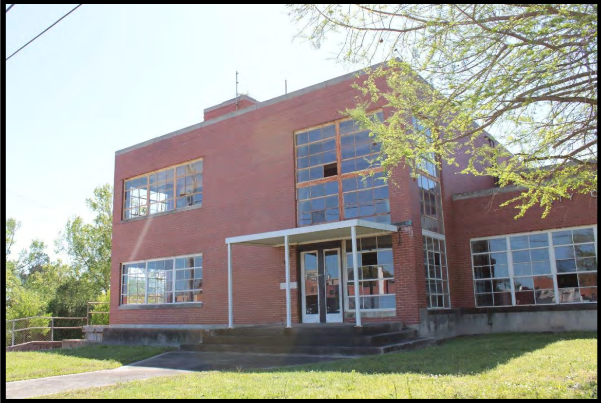
Figure 20: Lumberton Water Treatment Plant, Looking Southwest.
