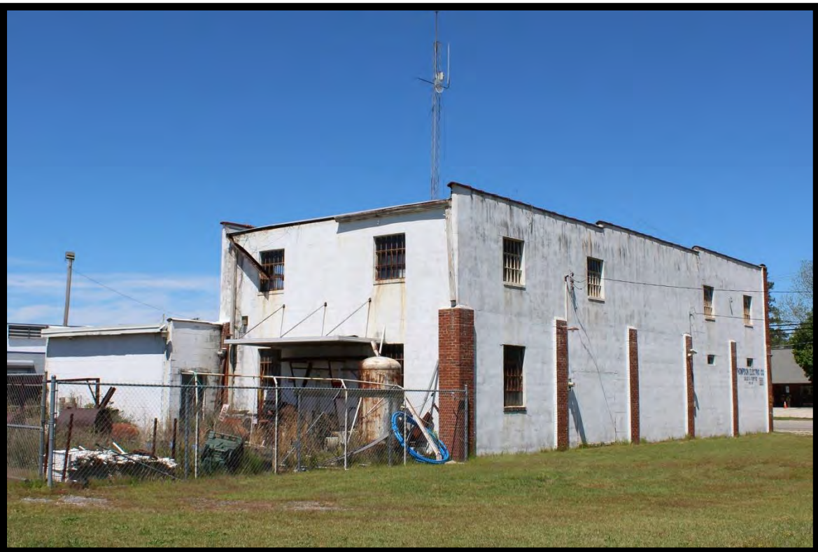
Figure 70: Thompson Electric Company, Looking Northwest.
