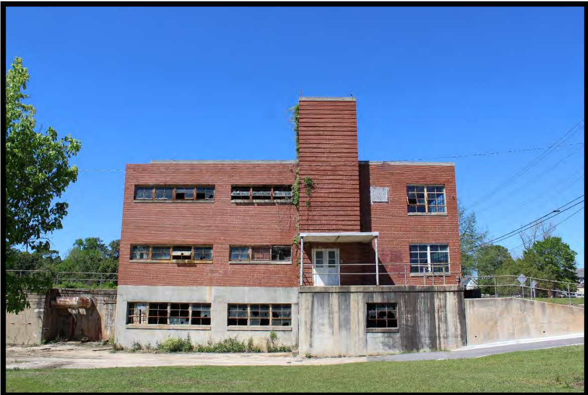
Figure 26: Lumberton Water Treatment Plant, Looking North.
