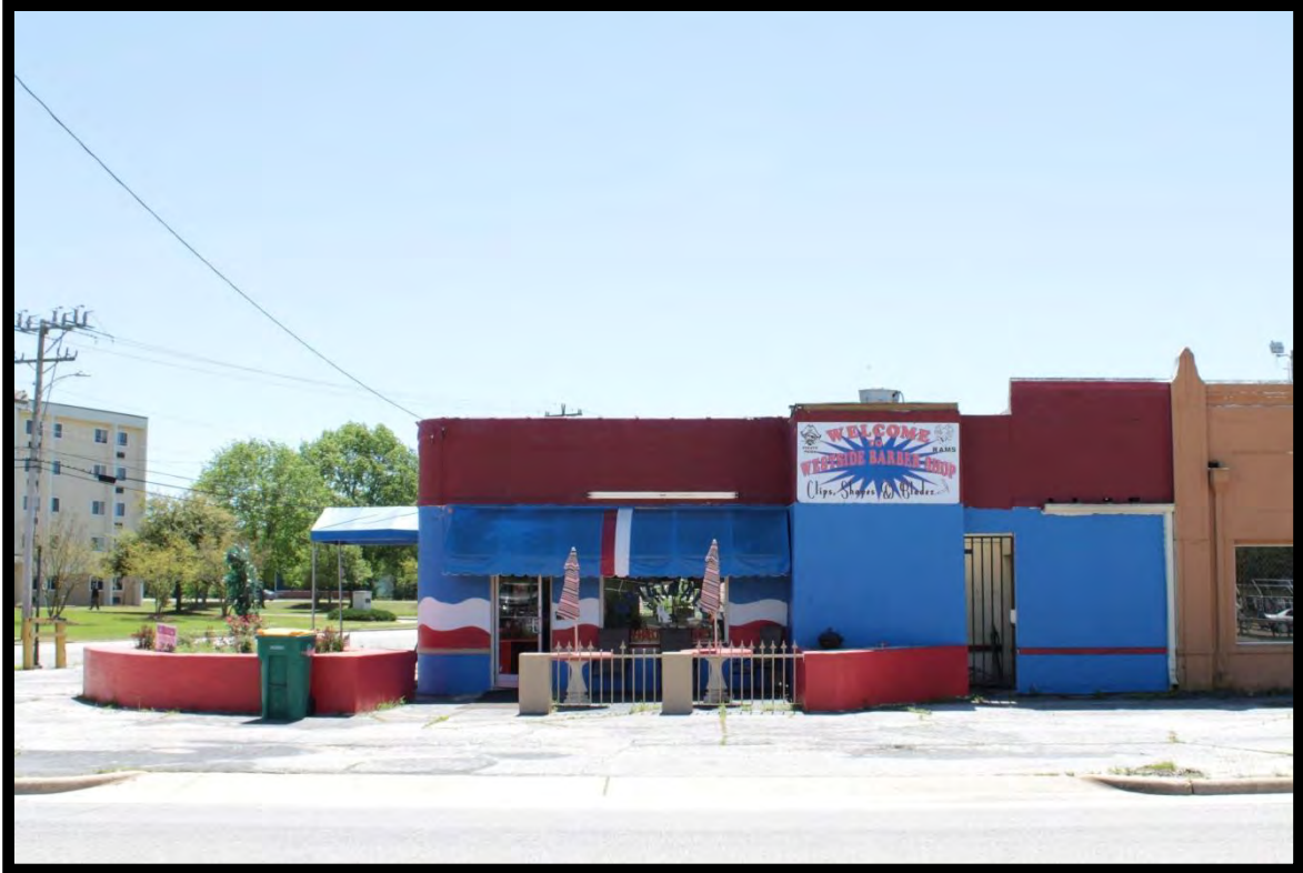
Figure 52: West Fifth Street Stores, Looking South.
