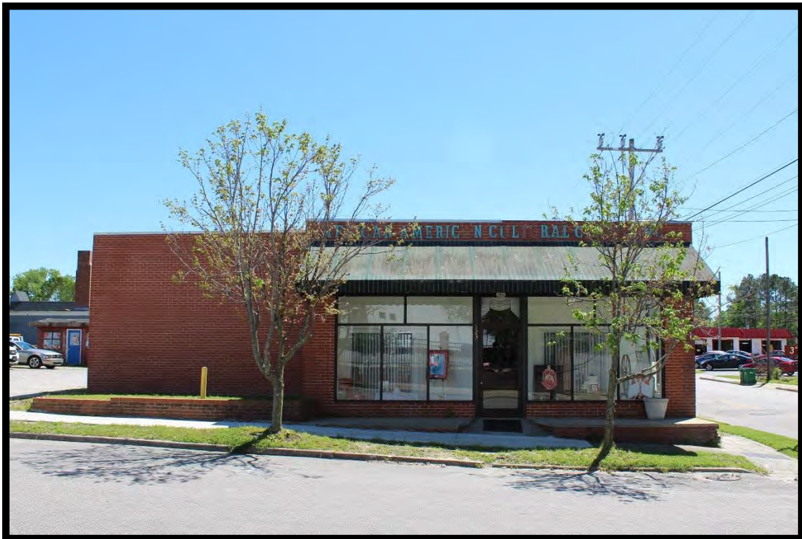
Figure 3: Whitley Furniture Company, Looking South.
