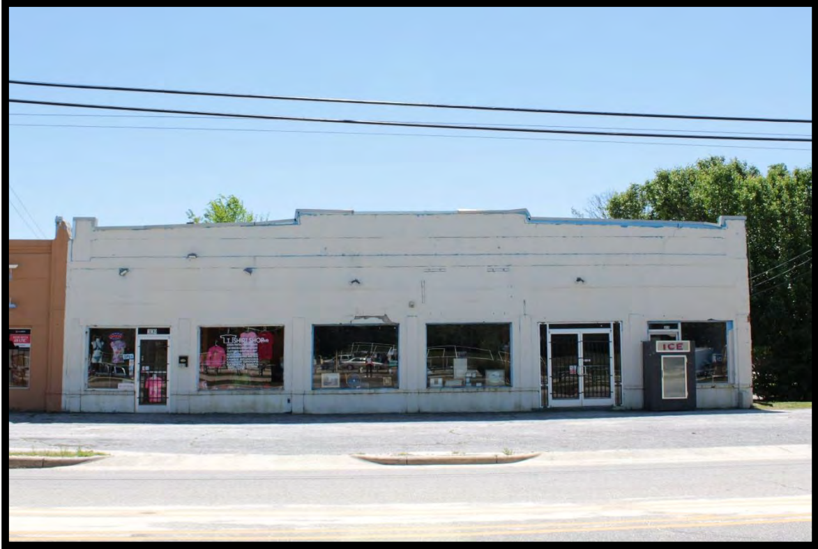
Figure 45: West Fifth Street Stores, Looking South.
