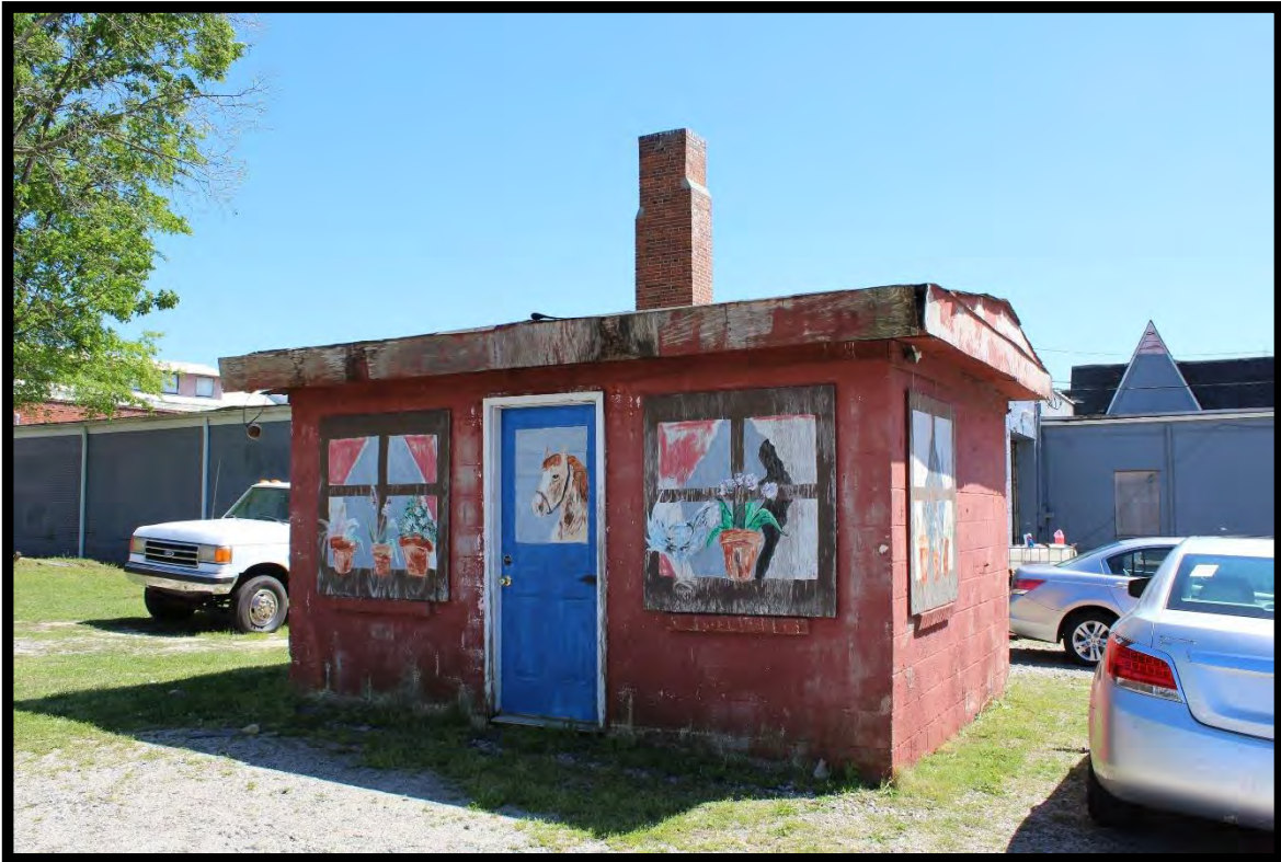
Figure 9: Whitley Furniture Company, Shed, Looking Southeast.
