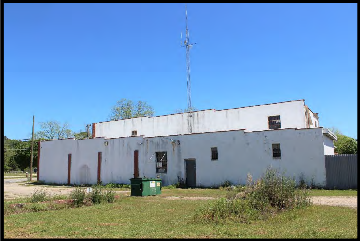
Figure 69: Thompson Electric Company, Looking Northeast.
