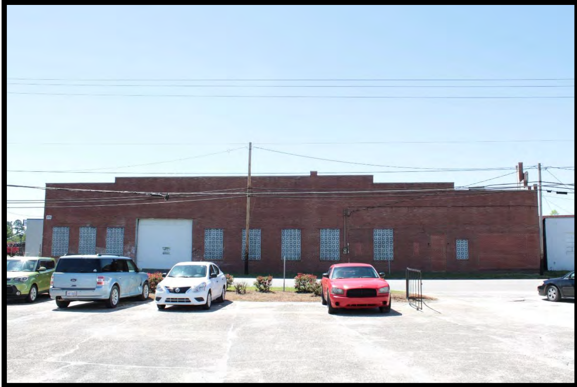
Figure 101: Automobile Sales Center, Looking South.
