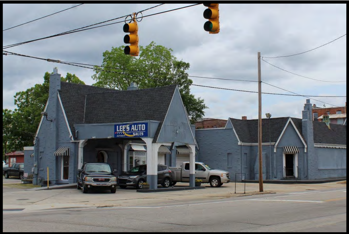
Figure 123: Pure Oil Filing Station (RB0180), Looking Northeast.
