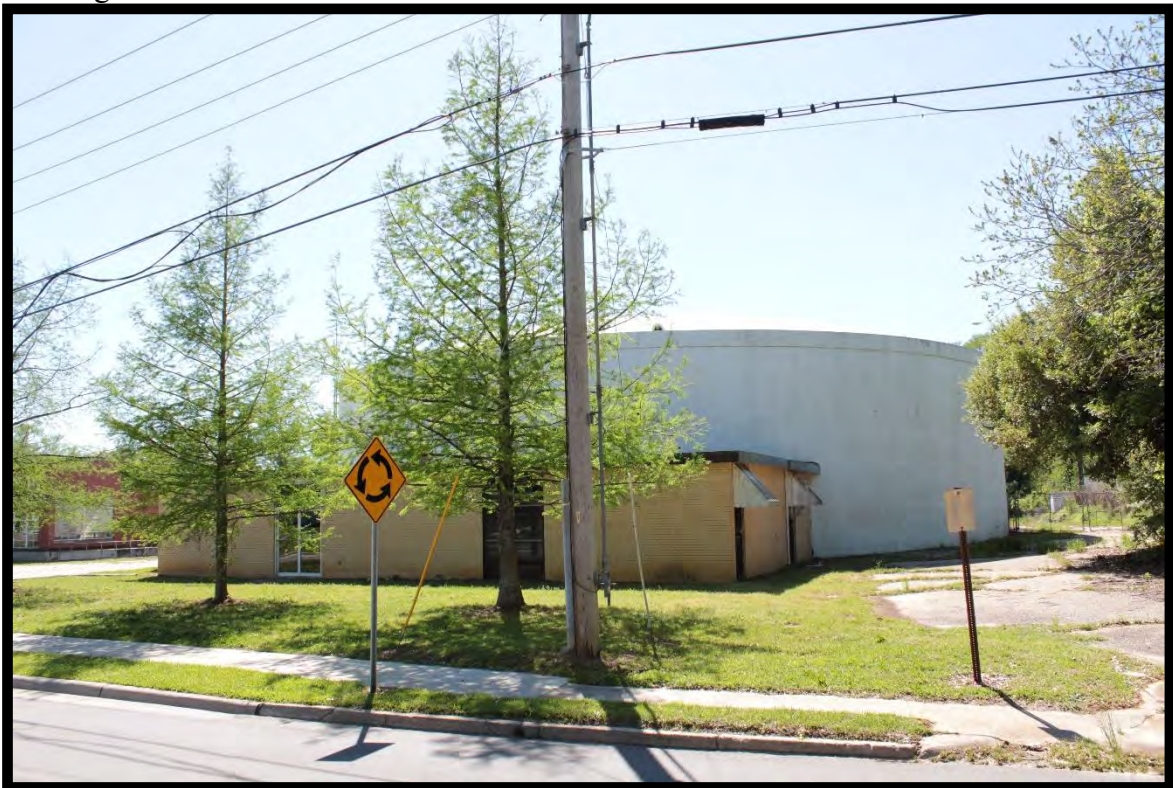
Figure 34: Lumberton Water Treatment Plant, Water Tank and Mechanical Building, Looking Northwest.
