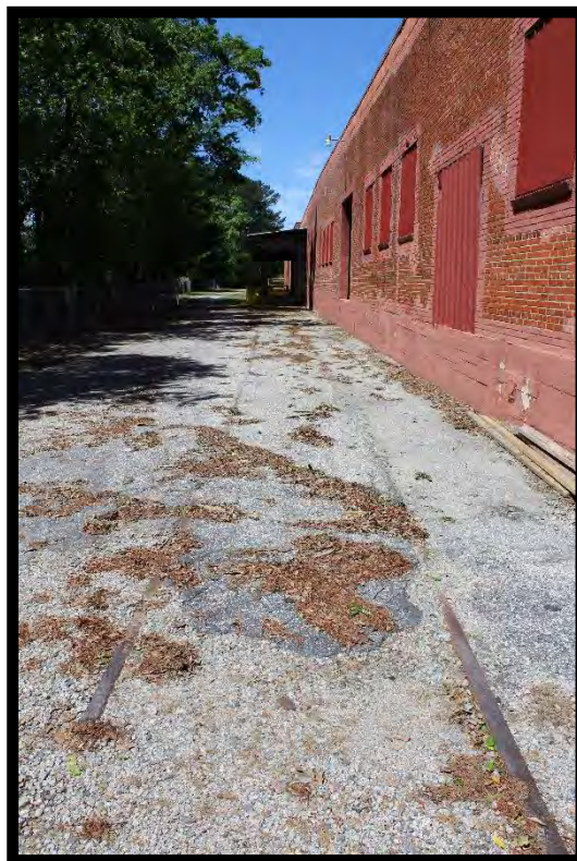
Figure 88: Planters Warehouse, Railroad Spur, Looking West.
