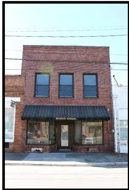
Figure 76: Store (RB0239), Looking South.
