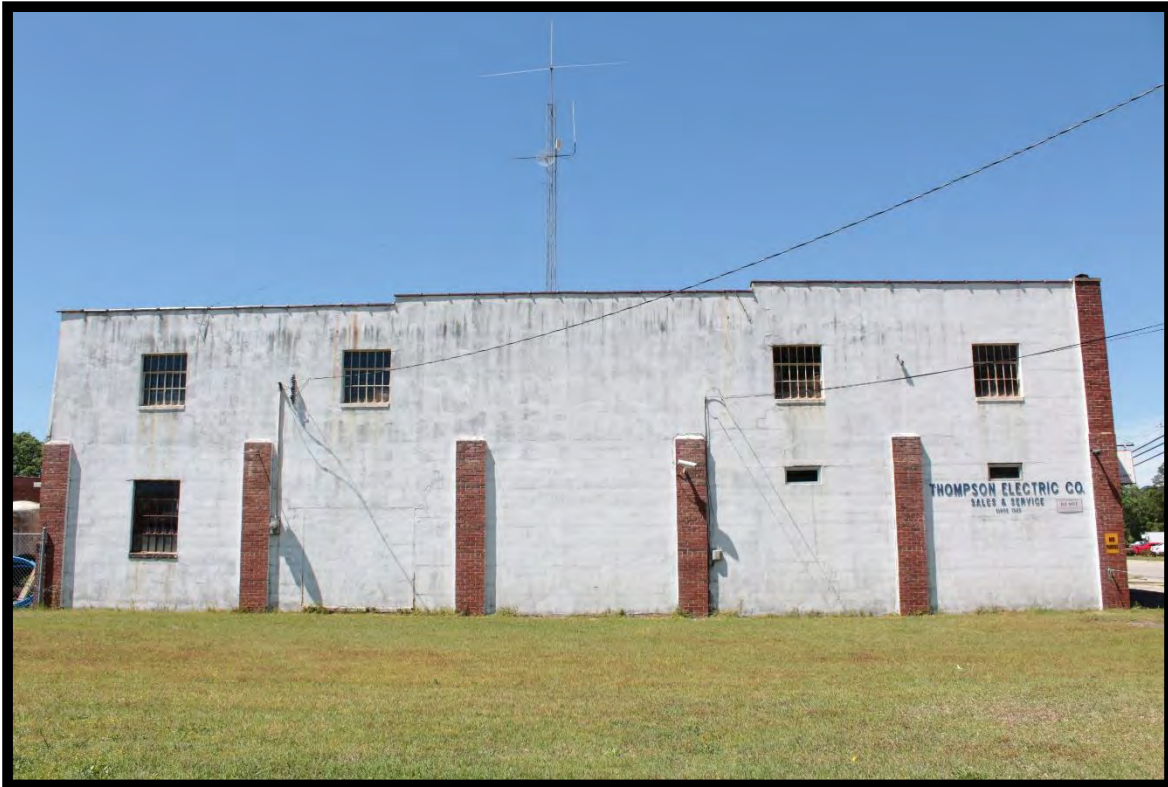
Figure 71: Thompson Electric Company, Looking West.
