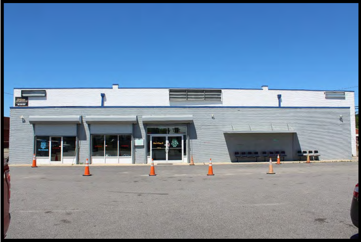
Figure 104: Automobile Sales Center, Looking West.
