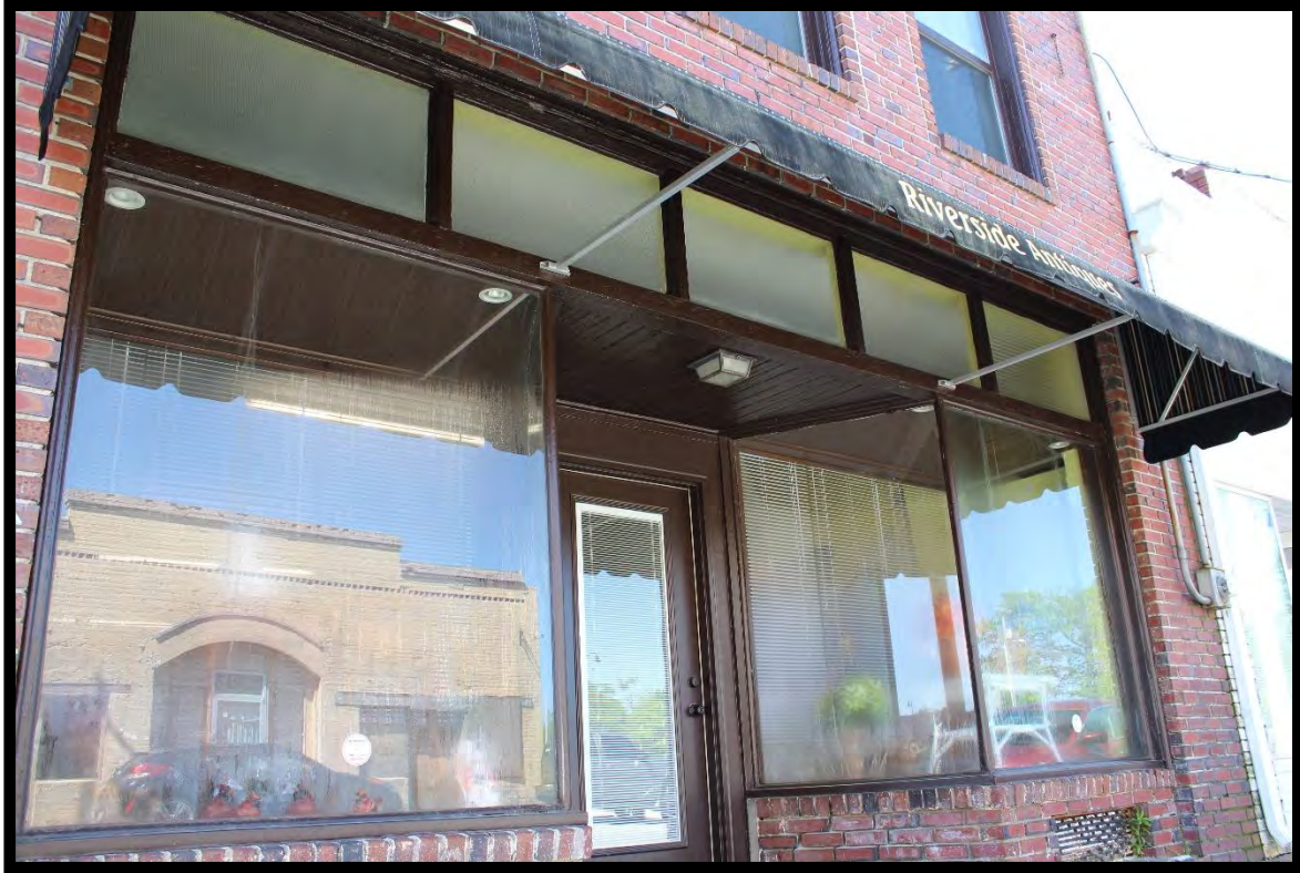
Figure 77: Store (RB0239), Detail of Storefront and Transom Windows.
