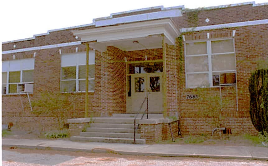
CB0067_CerroGordoSchool-1926 Classroom Building_M.Funk_09-15-2020_004_EntryPortico.jpg
