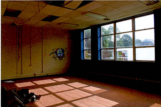
CB0067_CerroGordoSchool-1926 Classroom Building_M.Funk_09-15-2020_022_TypicalClassroom( Remodeled).jpg
