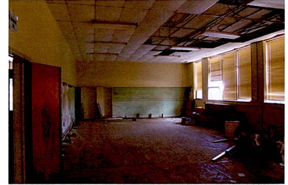
CB0067_CerroGordoSchool-1926 Classroom Building_M.Funk_09-15-2020_021_TypicalClassroom( OriginalMaterials).jpg
