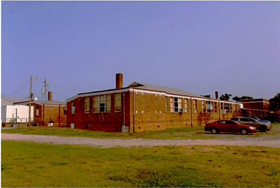
CB0067_CerroGordoSchool-1926 Classroom Building_M.Funk_09-15-2020_013_LookingNorth.jpg
