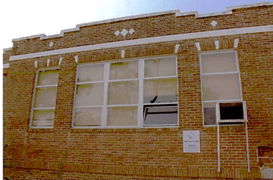
CB0067_CerroGordoSchool-1926 Classroom Building_M.Funk_09-15-2020_005_TypicalWindowBay.jpg
