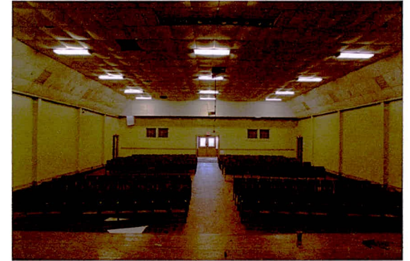
CB0067_CerroGordoSchool-1926 Classroom Building_M.Funk_09-15-2020_015_AuditoriumLookingNortheast.jpg
