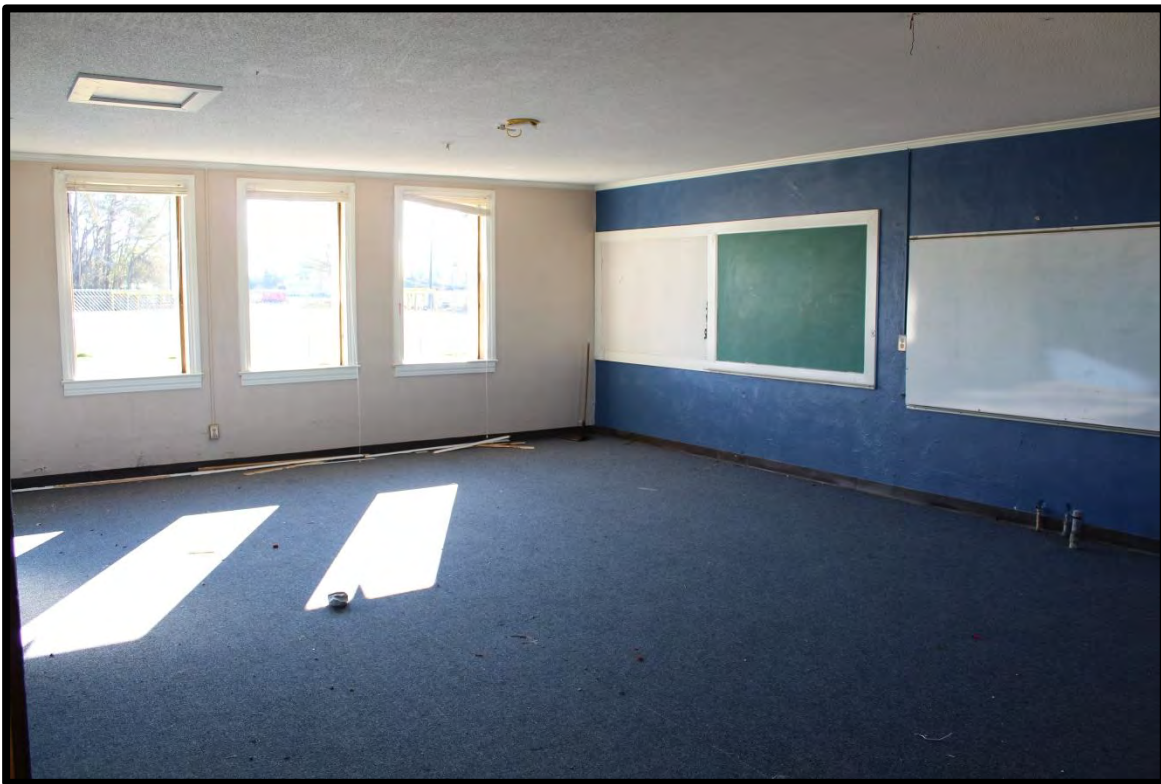
Figure 28: Cerro Gordo School, Field House, Band Classroom.
