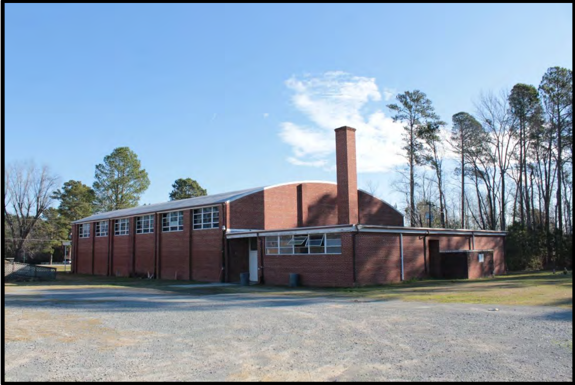
Figure 24: Cerro Gordo School, Gymnasium, Looking South.
