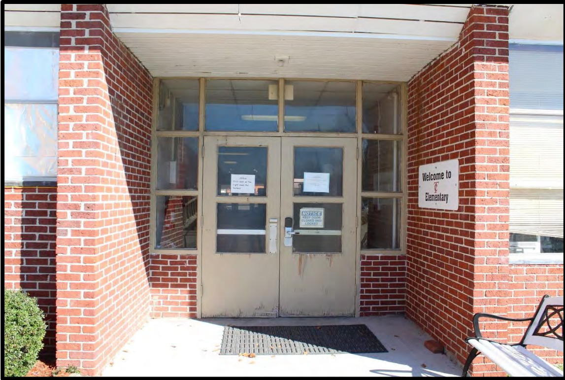
Figure 100: Tabor City School, 1950s Classroom Building, Looking Northeast.
