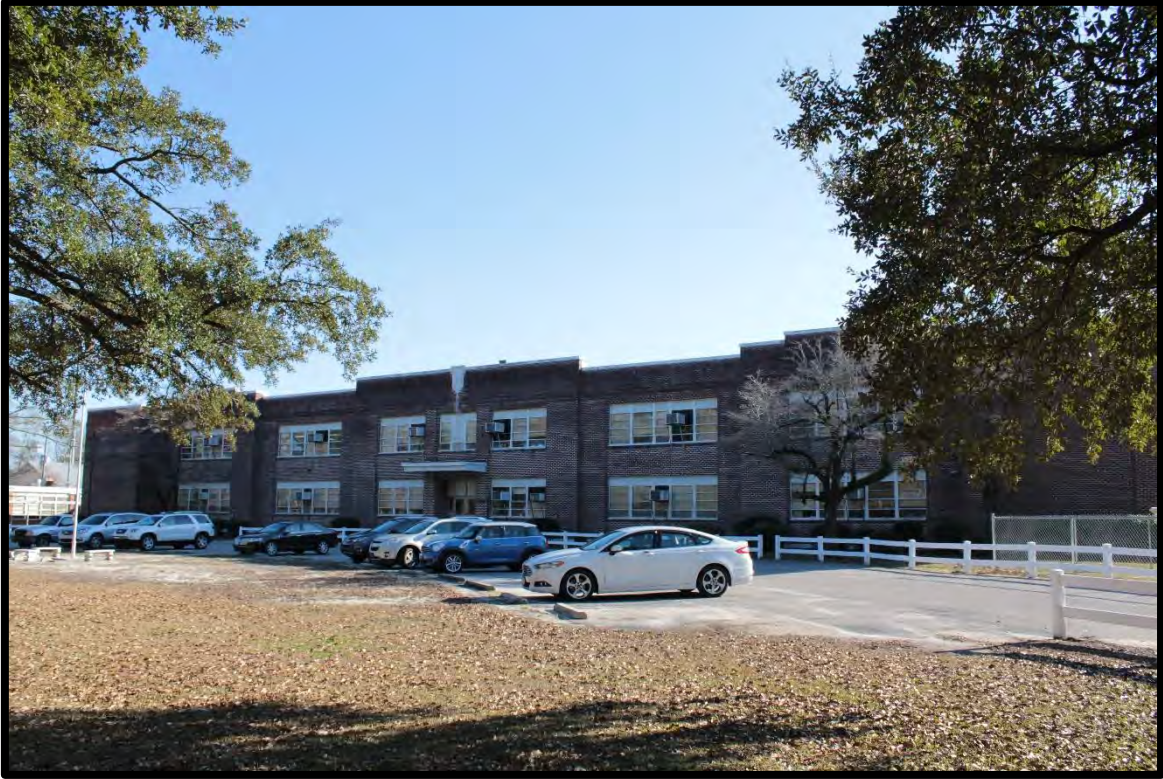
Figure 54: Evergreen School, Looking Southeast.
