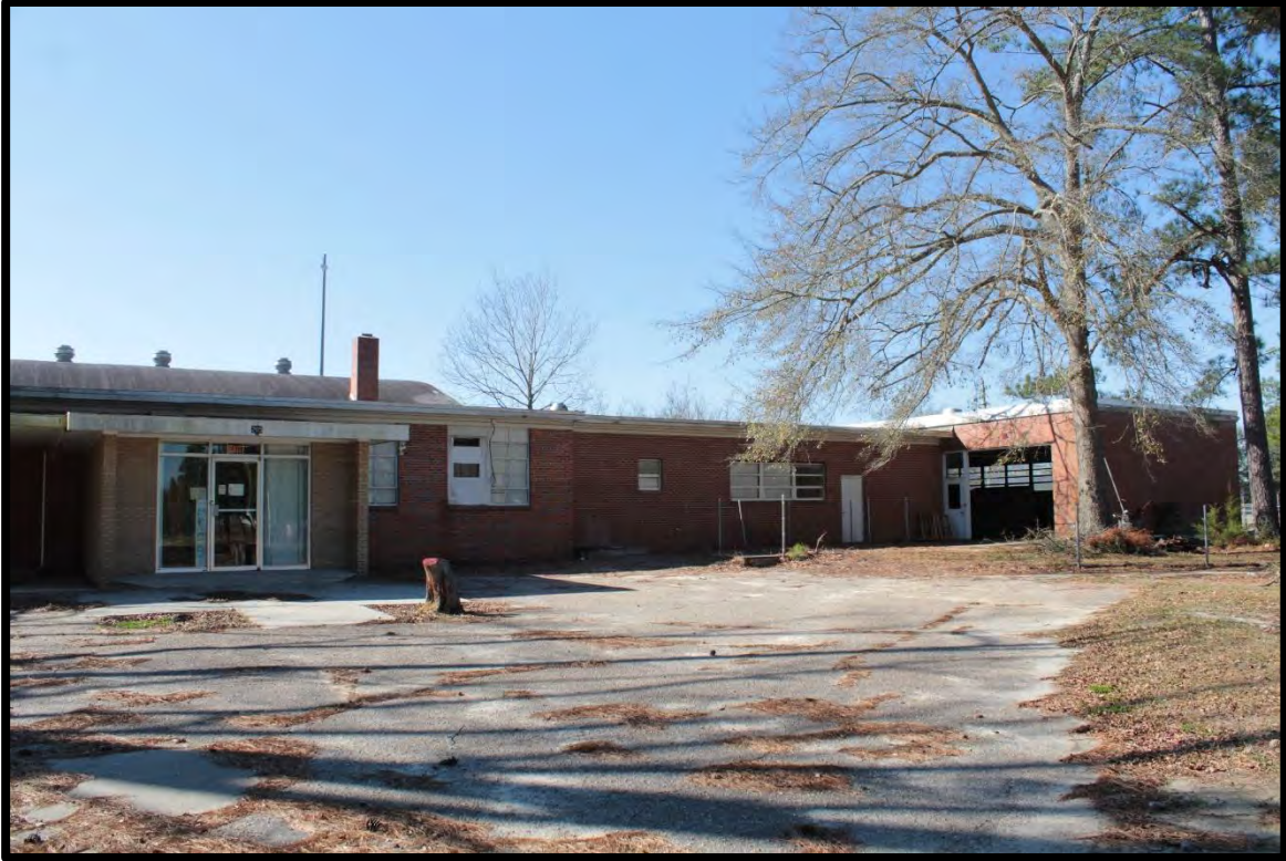
Figure 85: Tabor City School, Occupational Trades Building, Looking West.
