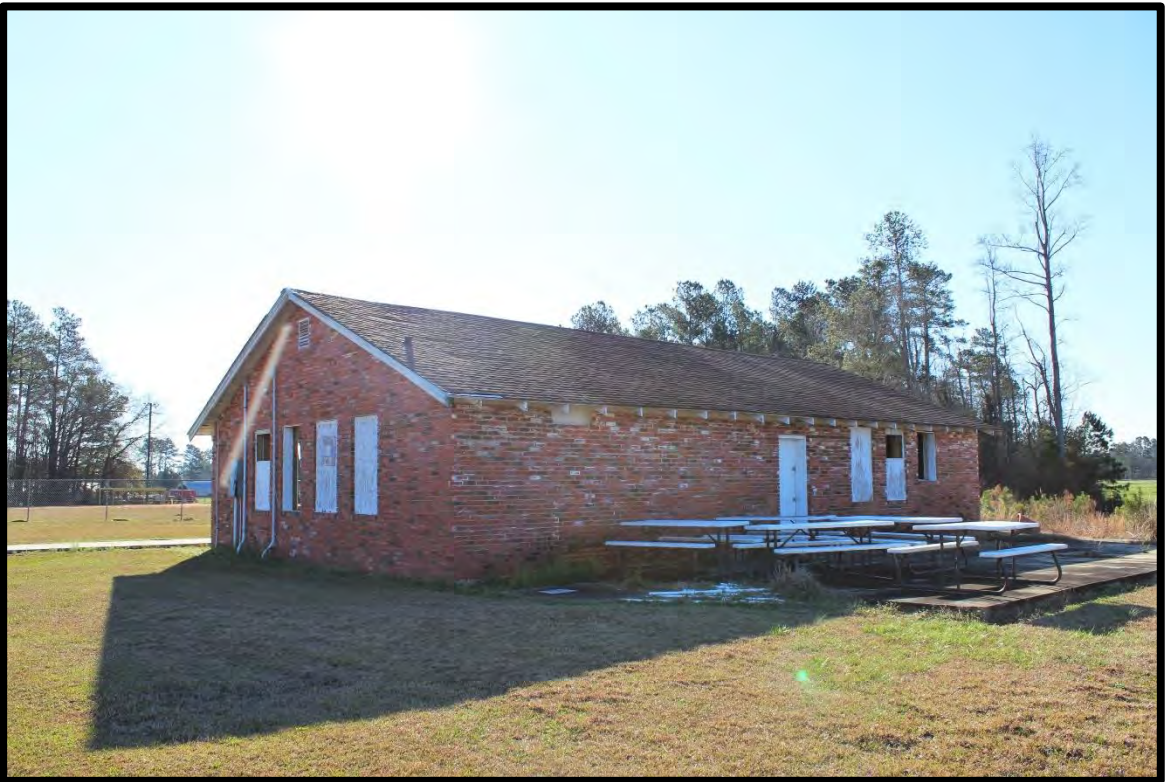
Figure 26: Cerro Gordo School, Field House, Looking South.
