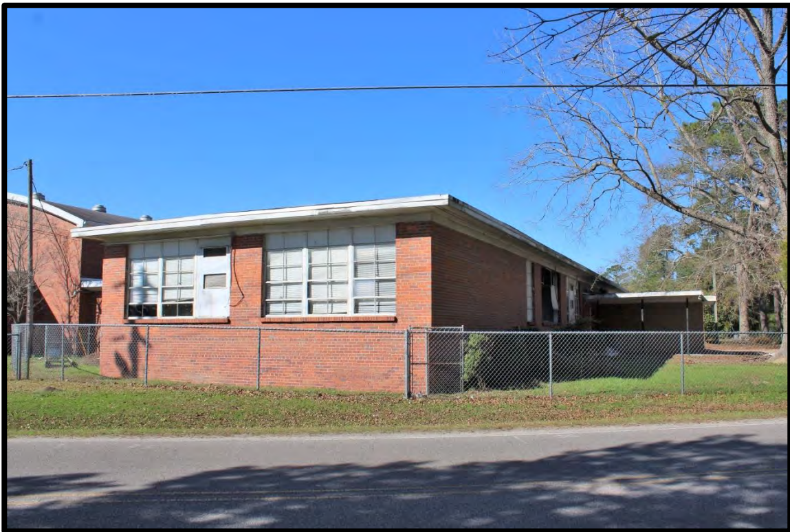
Figure 86: Tabor City School, Occupational Trades Building, Looking Northwest.
