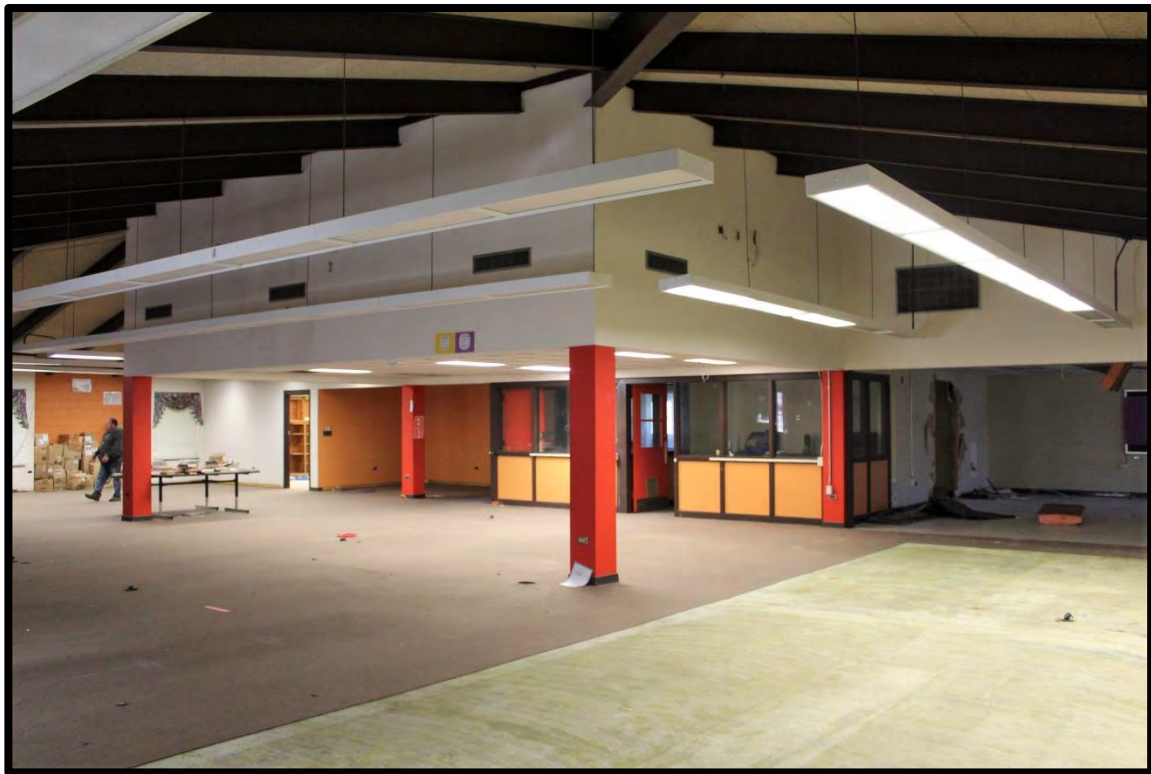
Figure 97: Tabor City School, Media Center, Library Space Looking Toward Office.
