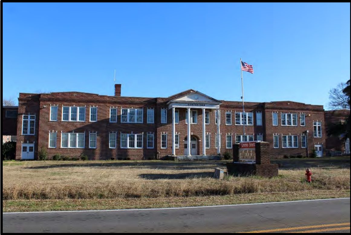
Figure 116: Contentnea School (LR0800), Looking South.
