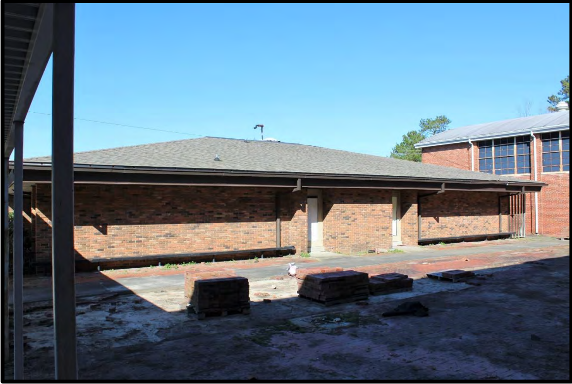
Figure 92: Tabor City School, Science Building, Looking North.
