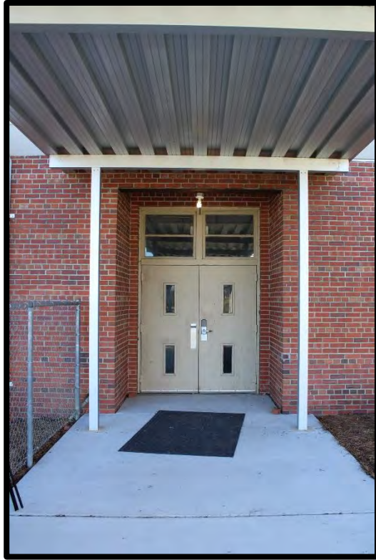
Figure 31: Cerro Gordo School, Ca. 1950 Classroom Building, Exterior Doors Below Metal Canopy.
