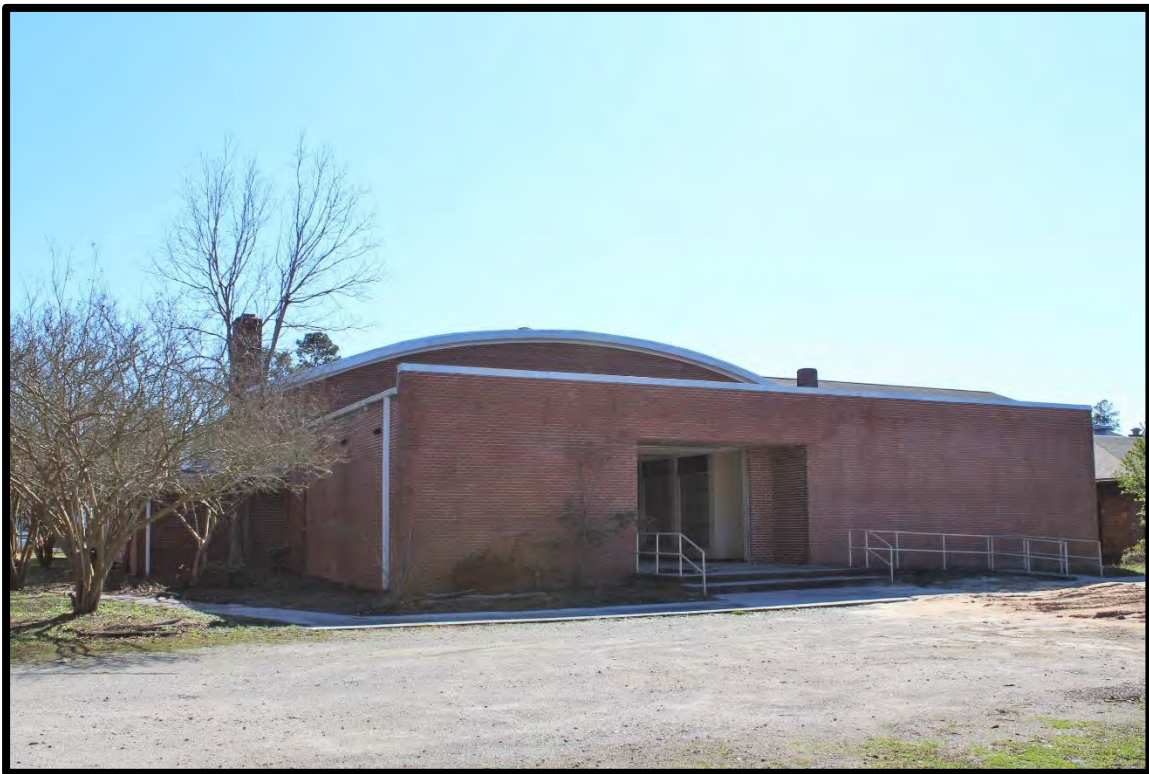
Figure 77: Tabor City School, Gymnasium, Looking South.
