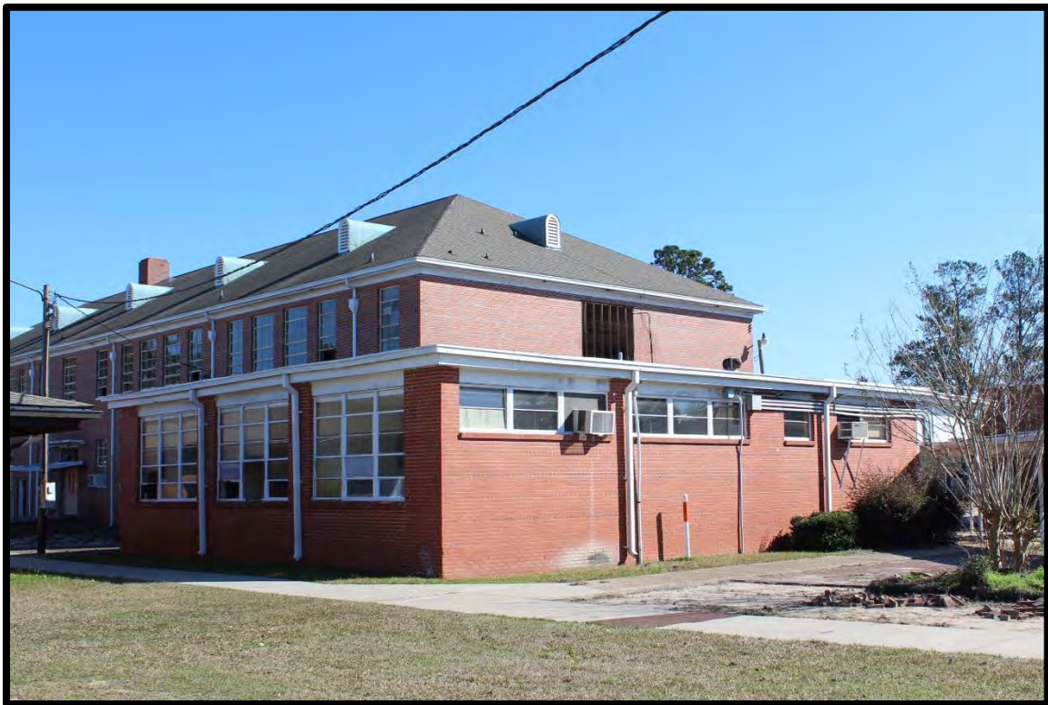
Figure 68: Tabor City School, Home Economics Wing with 1948 High School in Background, Looking East.
