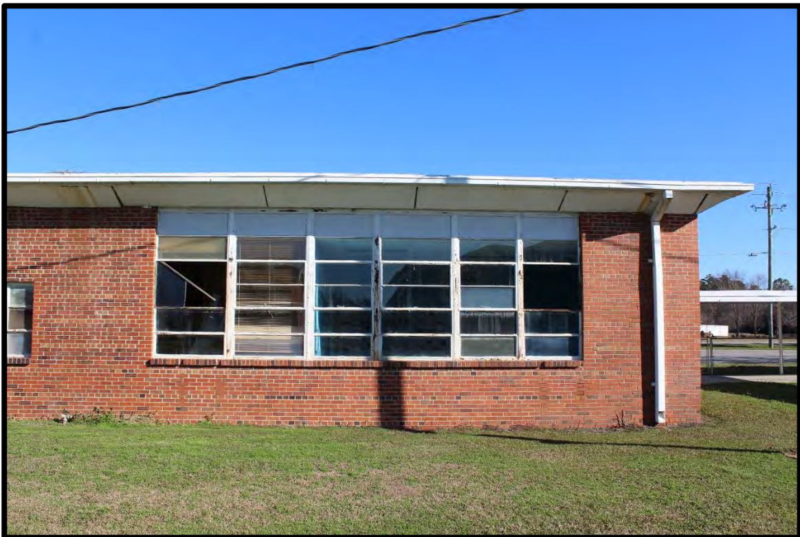
Figure 32: Cerro Gordo School, Ca. 1950 Classroom Building, Typical Windows.
