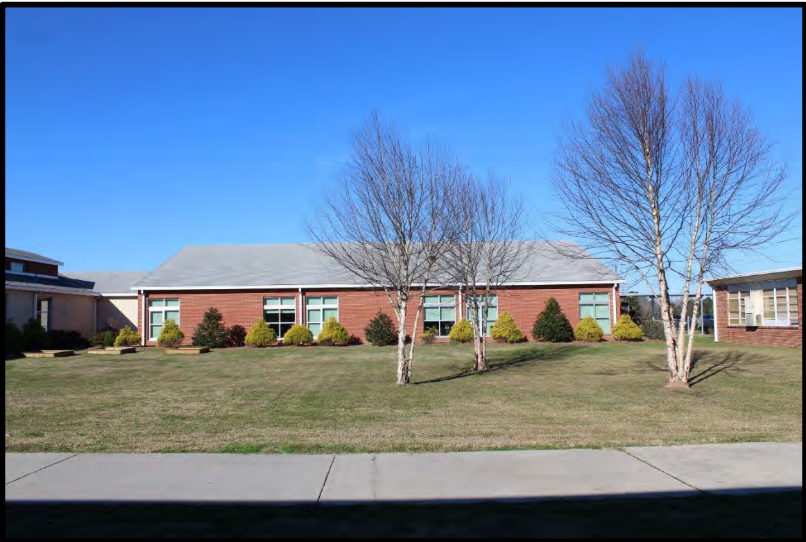
Figure 40: Cerro Gordo School, 2014 Classroom Building, Looking West-Northwest.
