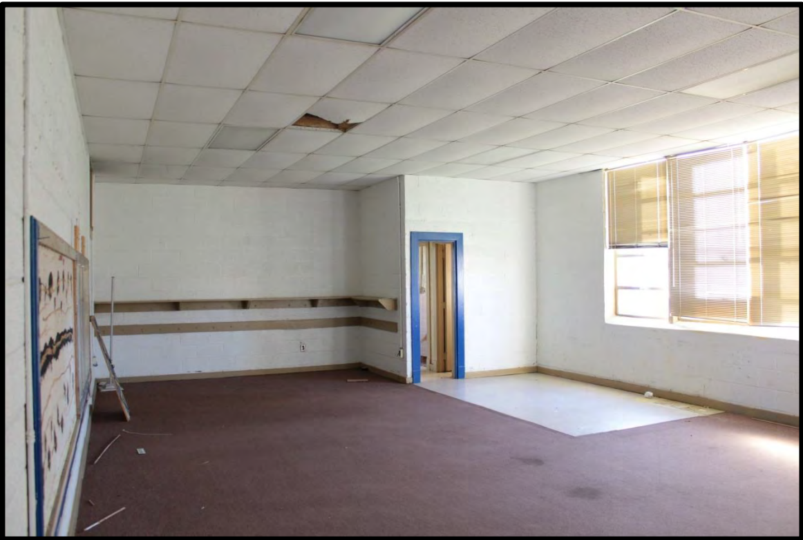
Figure 34: Cerro Gordo School, Ca. 1950 Classroom Building, Typical Classroom with Attached Restroom.
