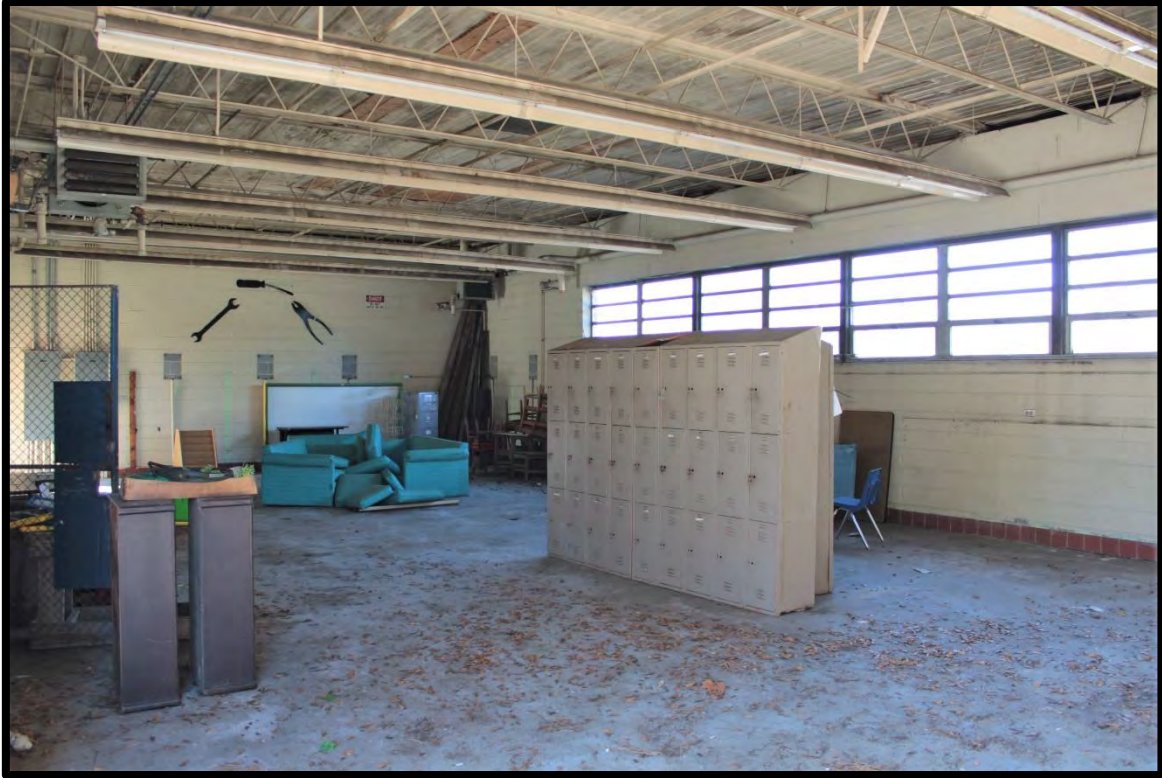
Figure 89: Tabor City School, Occupational Trades Building, Garage/Shop Rear Addition.
