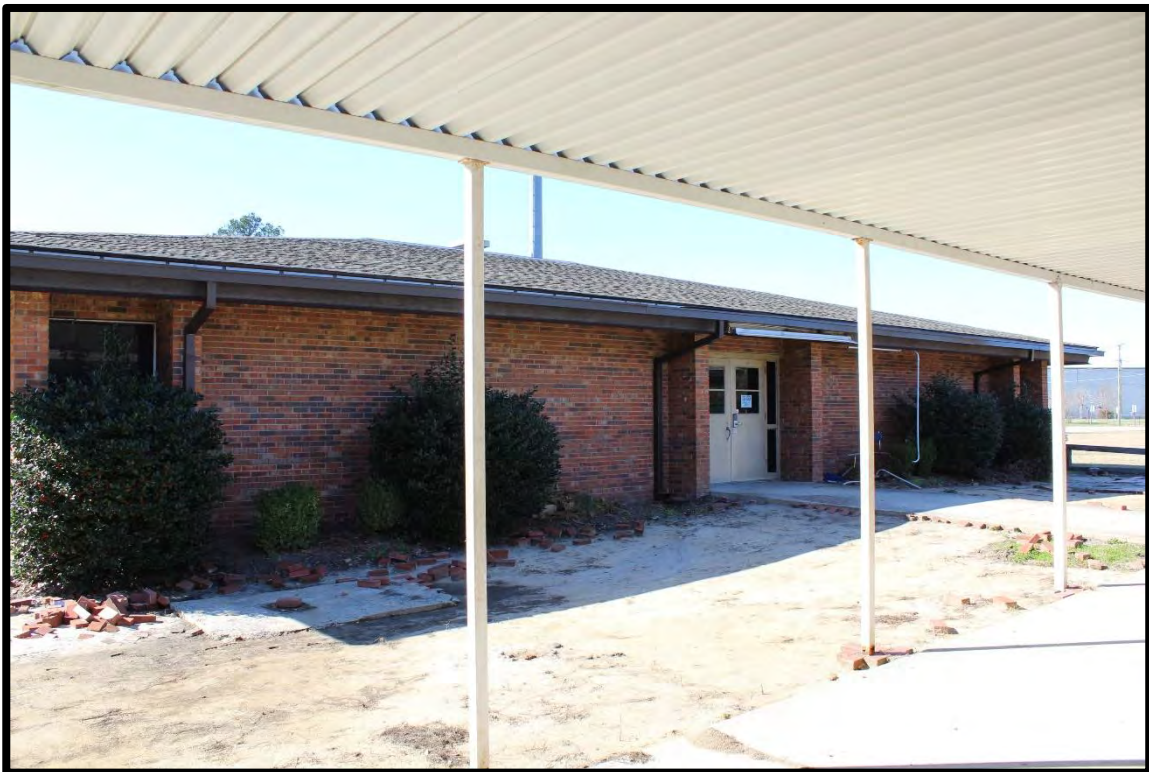
Figure 91: Tabor City School, Media Center, Looking Northwest.
