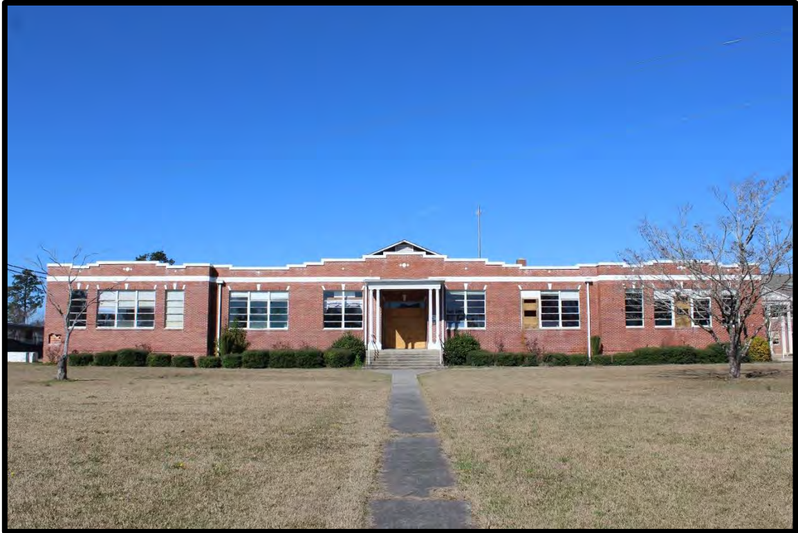
Figure 57: Tabor City School, Looking Northwest.
