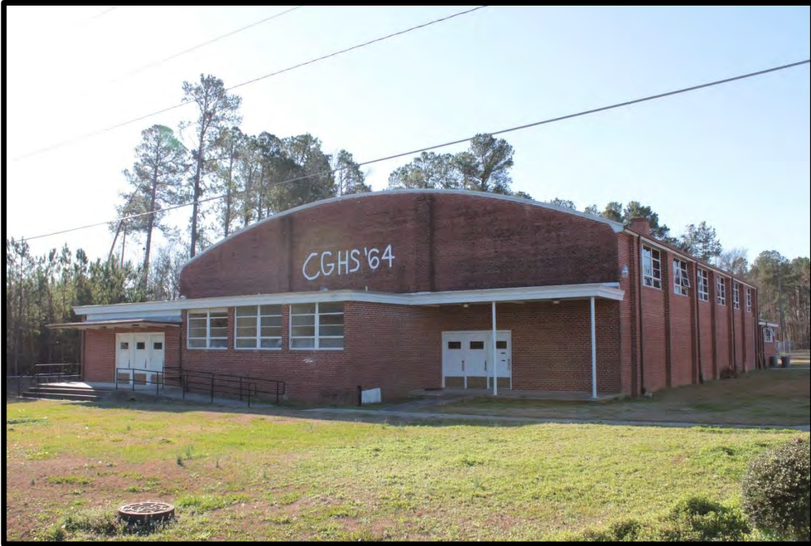
Figure 22: Cerro Gordo School, Gymnasium, Looking South.
