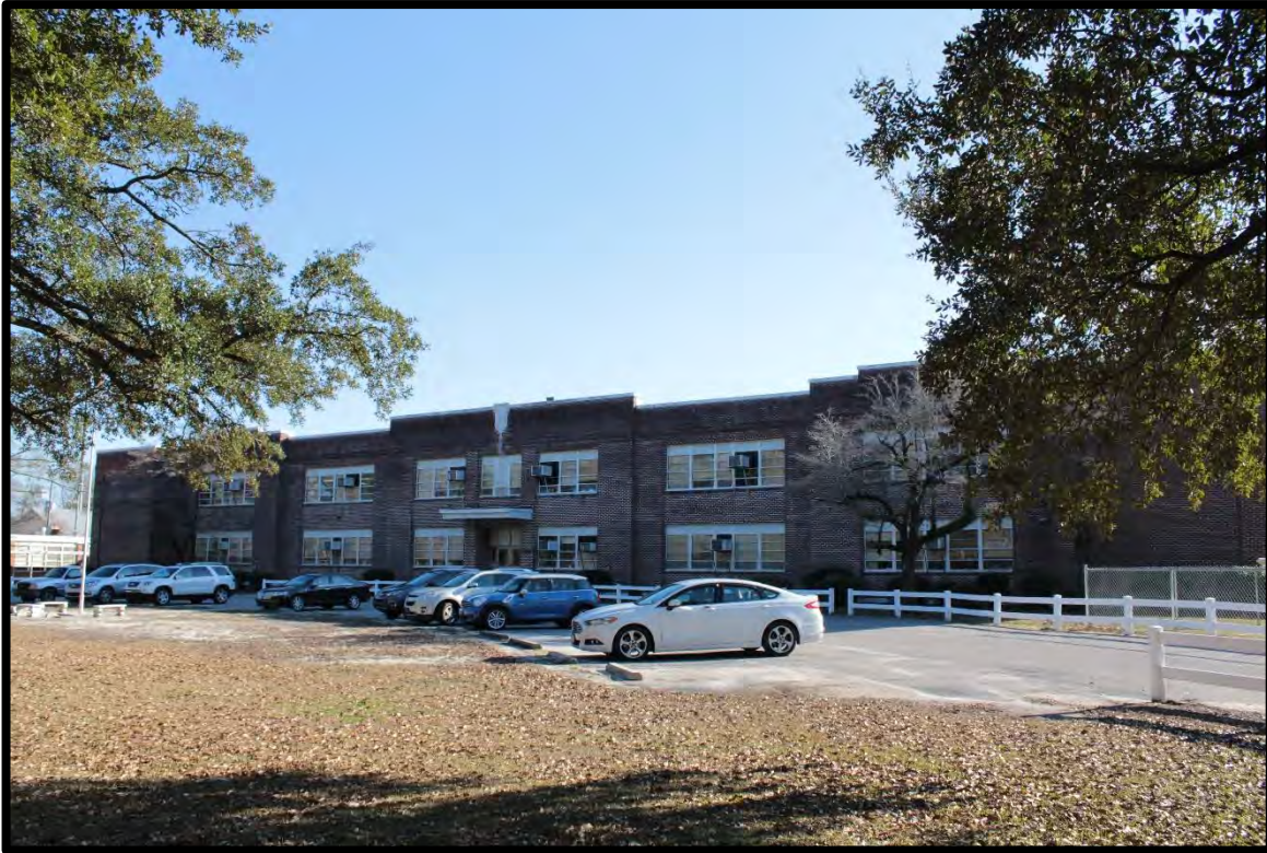
Figure 117: Evergreen School, Looking Southeast.
