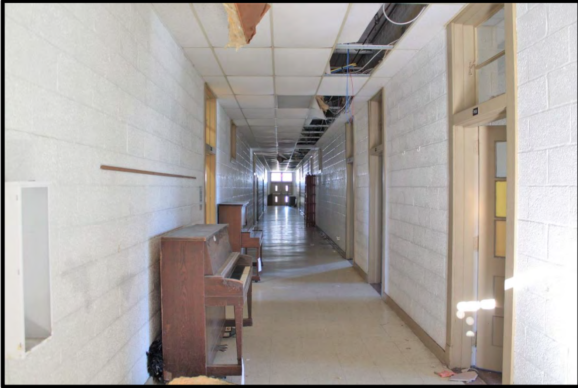
Figure 33: Cerro Gordo School, Ca. 1950 Classroom Building, Double-Loaded Corridor.
