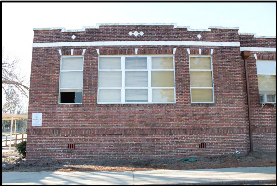
Figure 4: Cerro Gordo School, Looking South-Southwest.
