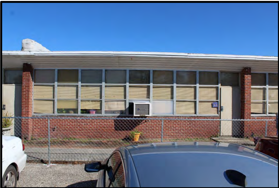
Figure 99: Tabor City School, 1950s Classroom Building, Looking Northeast.
