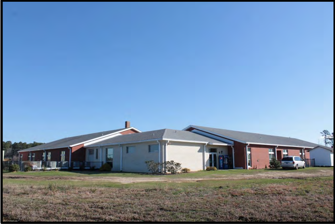
Figure 41: Cerro Gordo School, 2014 Classroom Building, Looking Northeast.
