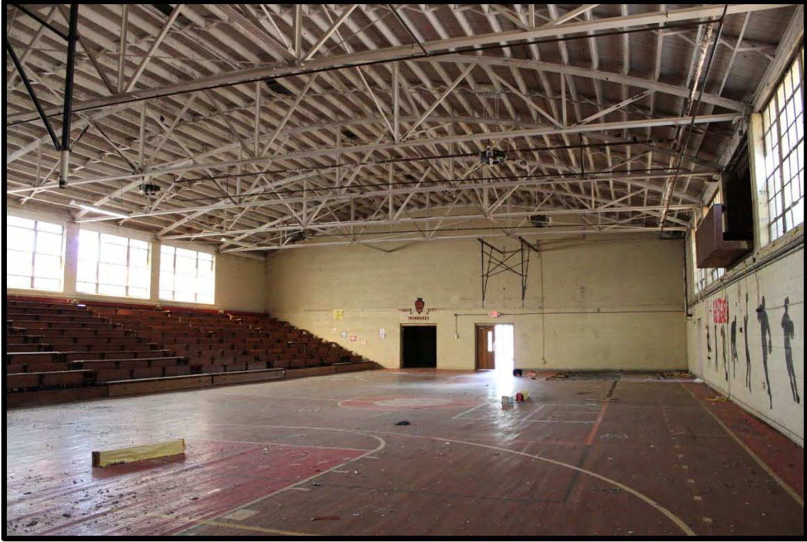
Figure 82: Tabor City School, Gymnasium Showing Hardwood Floor, Built-In Bleachers, and Added Announcer's Box (Right Elevation).
