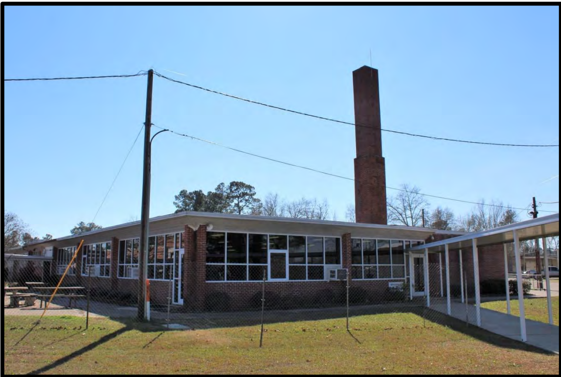
Figure 101: Tabor City School, 1950s Classroom Building, Looking South.
