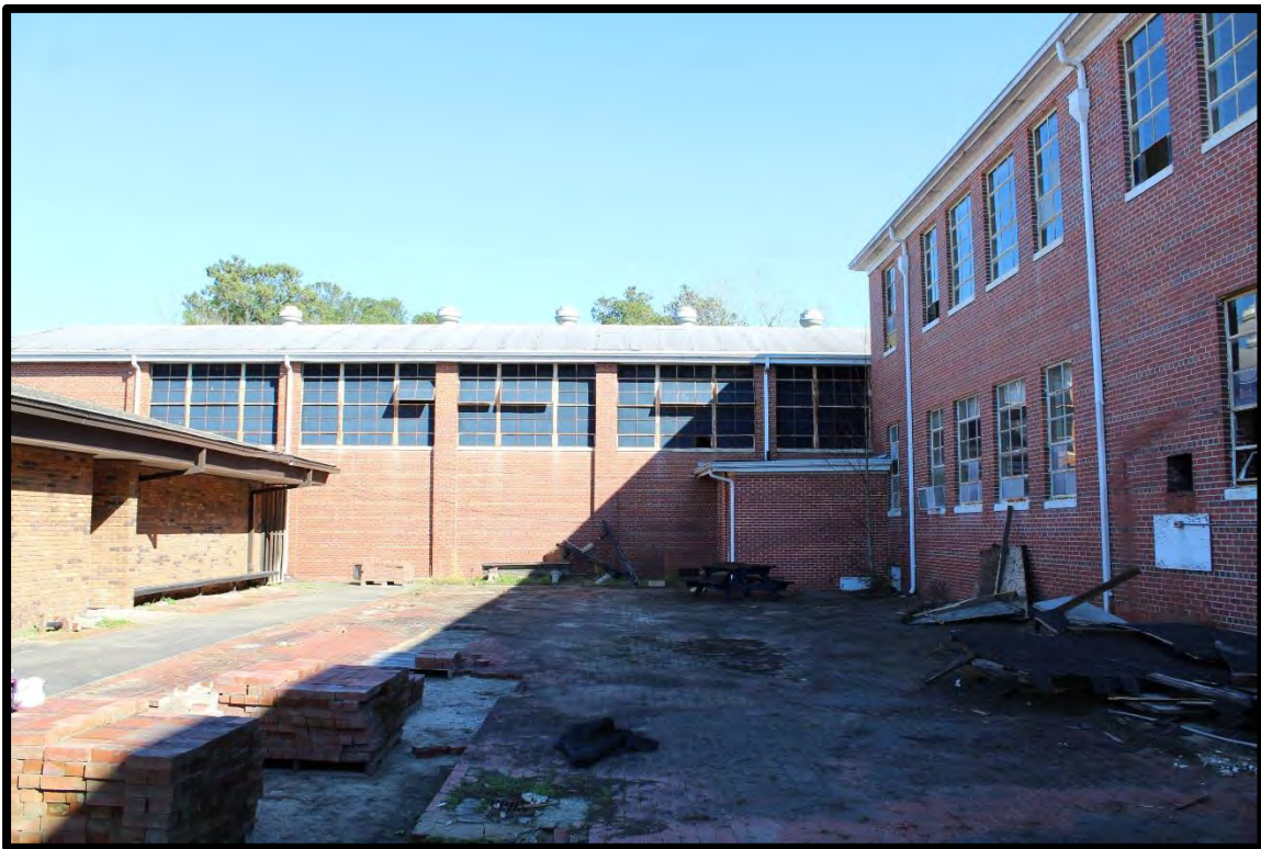
Figure 79: Tabor City School, Gymnasium, Looking Northeast.
