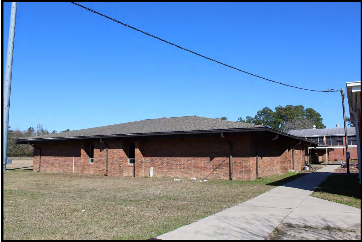
Figure 96: Tabor City School, Media Center, Looking Northeast.
