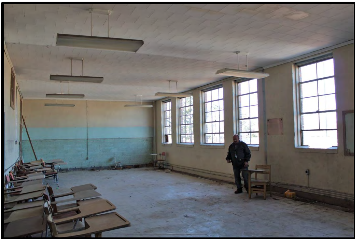
Figure 74: Tabor City School, 1948 High School, Interior of Second Floor Library Which was Created by Combining Two Classrooms. Also Note Earlier Materials.
