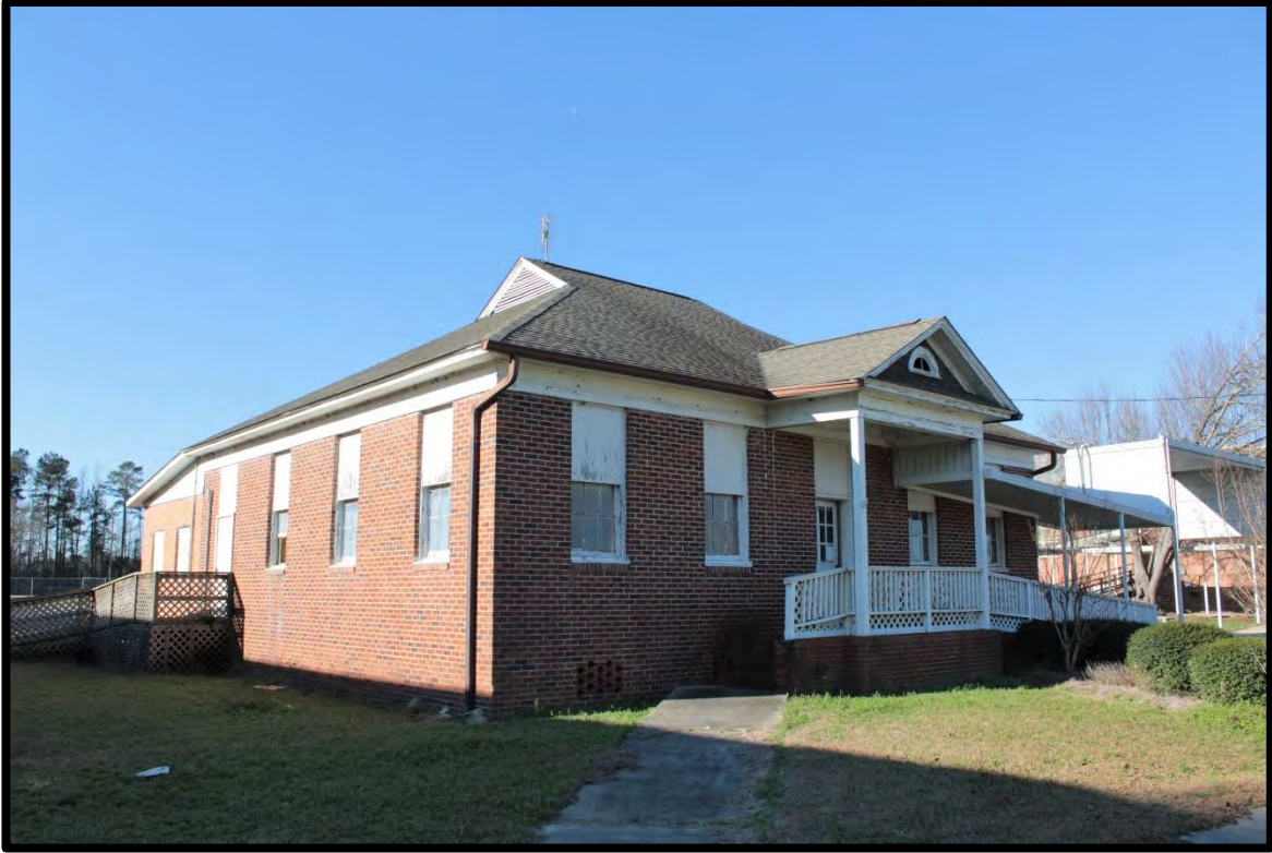
Figure 17: Cerro Gordo School, Agricultural Building, Looking Southwest.
