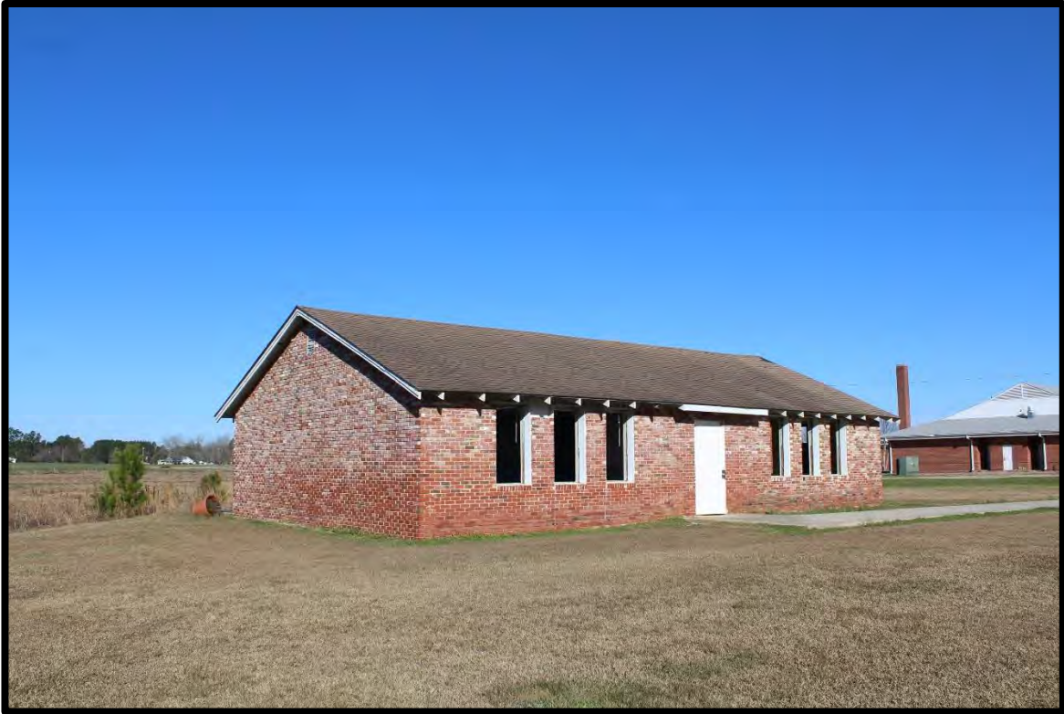
Figure 25: Cerro Gordo School, Field House, Looking North.
