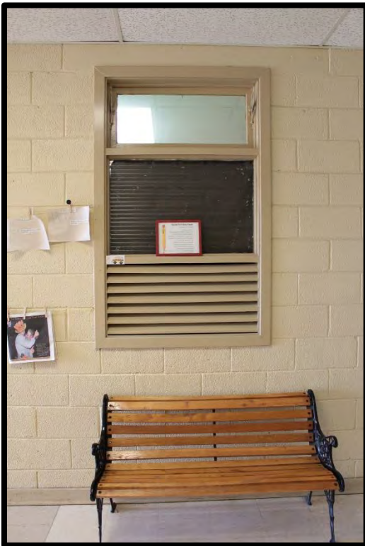
Figure 105: Tabor City School, 1950s Classroom Building, Vent/Transom Unit.
