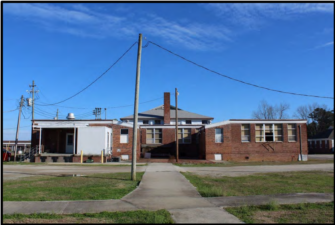
Figure 8: Cerro Gordo School, Looking North-Northeast.
