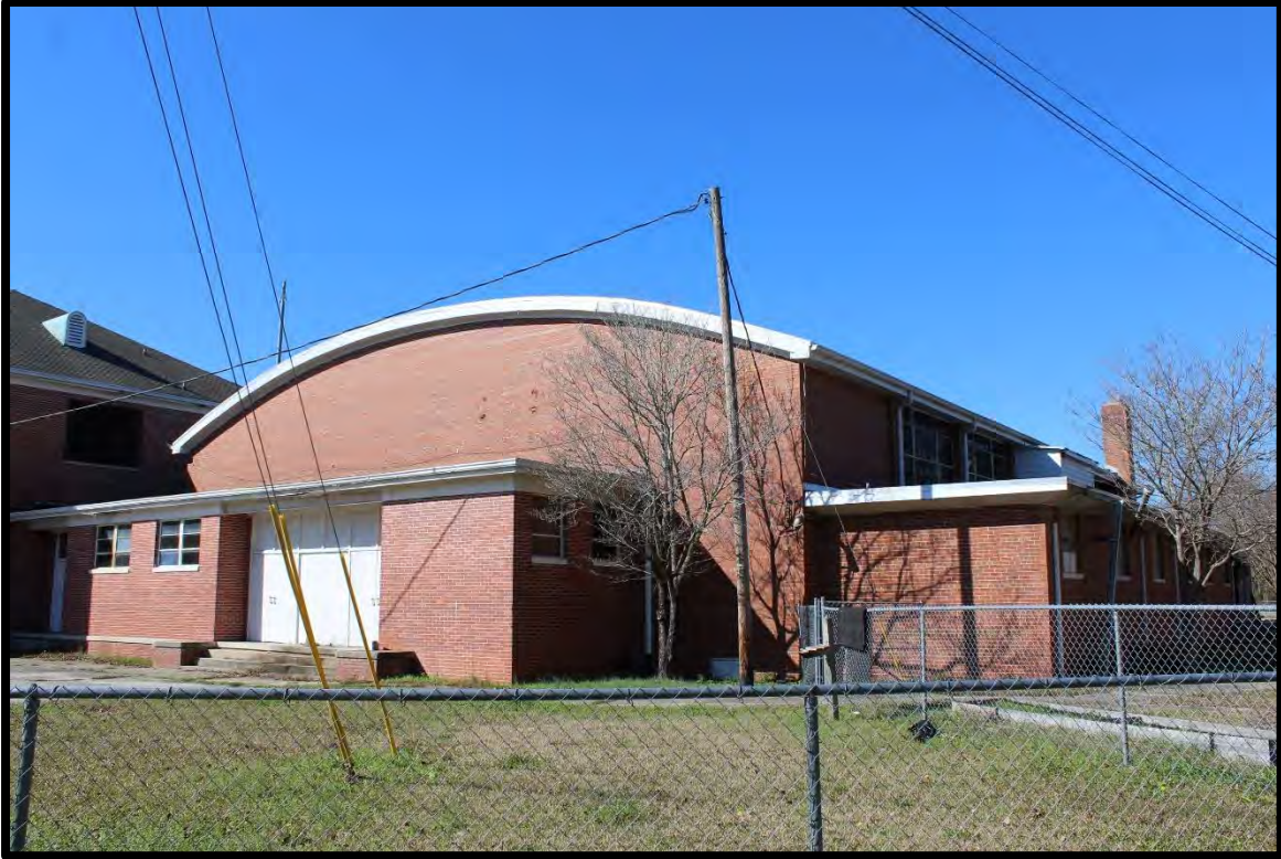
Figure 76: Tabor City School, Gymnasium, Looking Northwest.
