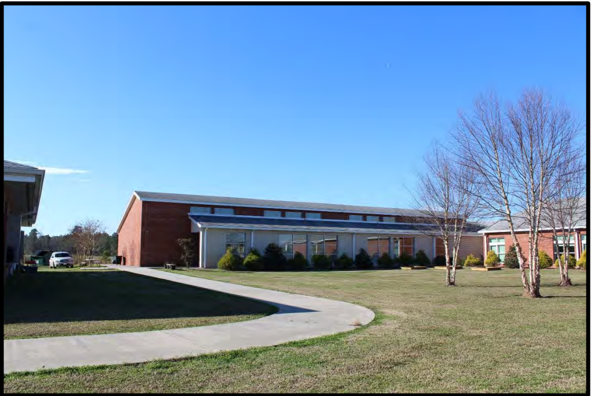
Figure 42: Cerro Gordo School, 2014 Classroom Building, Looking Southwest.
