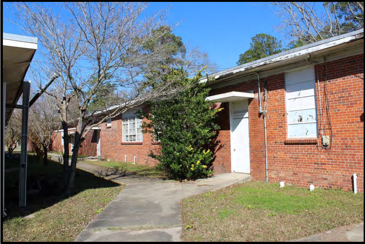
Figure 83: Tabor City School, Occupational Trades Building, Looking North.
