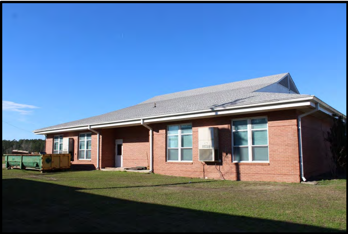
Figure 37: Cerro Gordo School, “Pod” -Style Classroom Building, Looking East.
