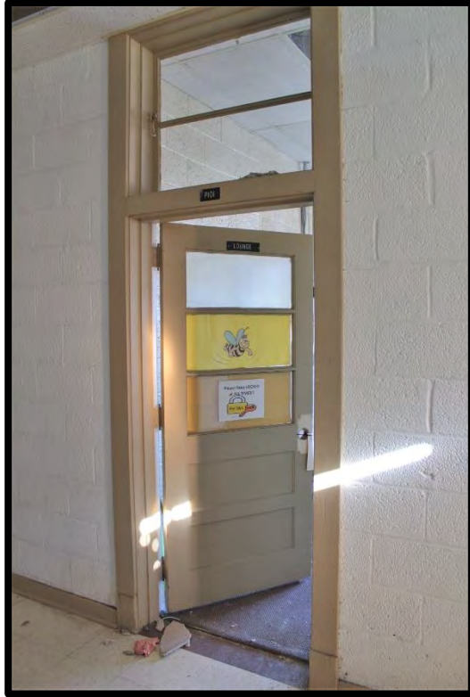
Figure 35: Cerro Gordo School, Ca. 1950 Classroom Building, Typical Interior Door and Transom.
