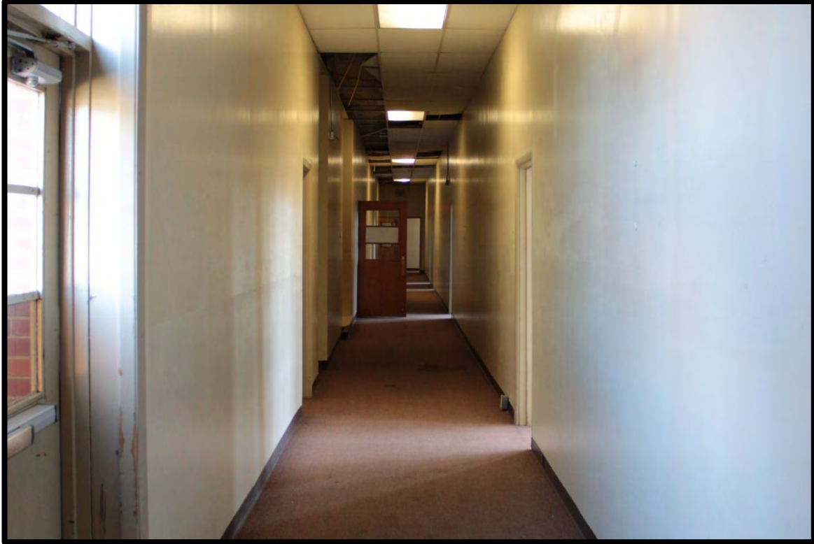
Figure 63: Tabor City School, Hallway. Note Drywall, Acoustic Tile Ceiling, Carpeting and Absence of Transoms from Classrooms.
