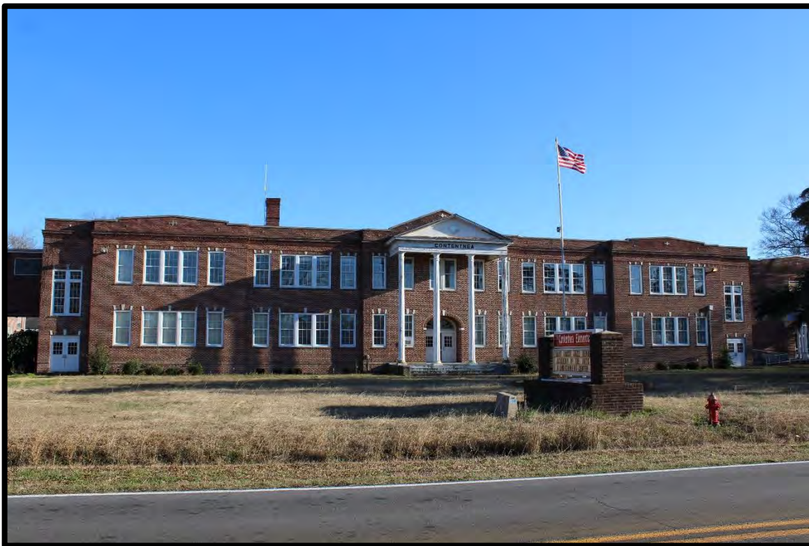
Figure 53: Contentnea School (LR0800), Looking South.
