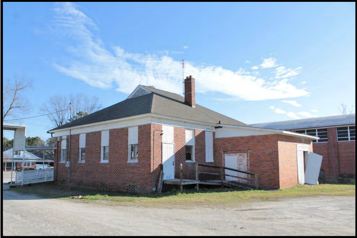
Figure 19: Cerro Gordo School, Agricultural Building, Looking Southwest.
