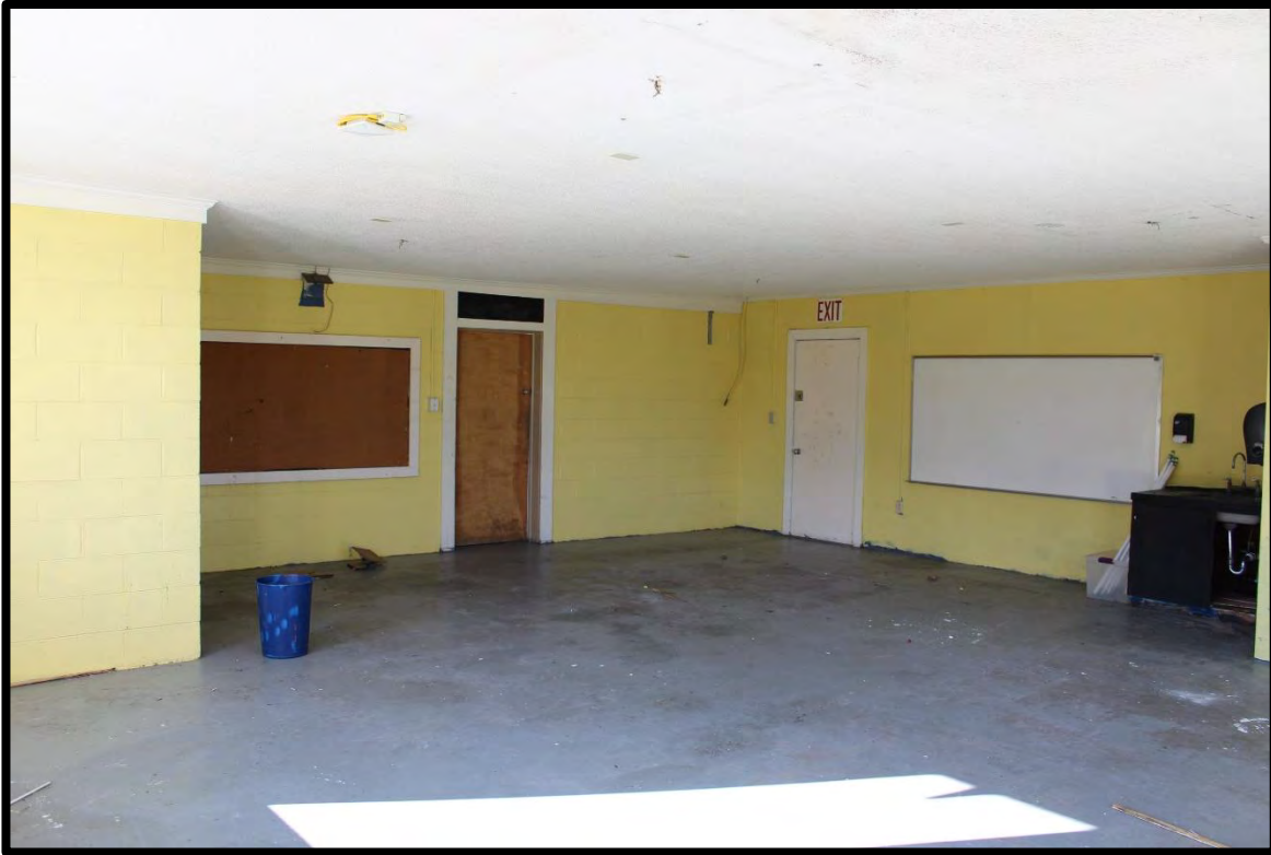
Figure 27: Cerro Gordo School, Field House, Art Classroom.
