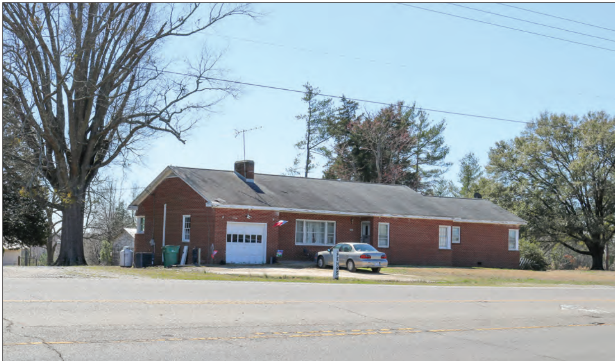
Figure 7.6. 2415 Tramway Road, Facing Southeast
