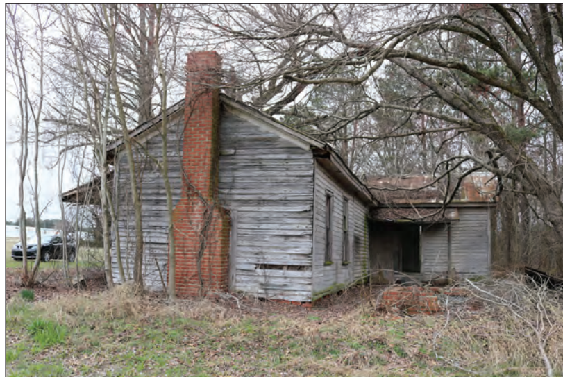
Figure 13.4. Lucy A. Lawrence House, West and North Elevations, Facing Southwest
