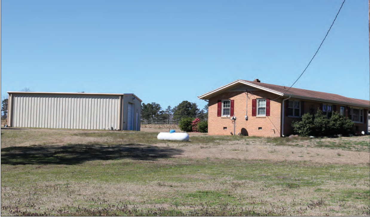
Figure 9.4. Frame Garage, Facing Northwest
