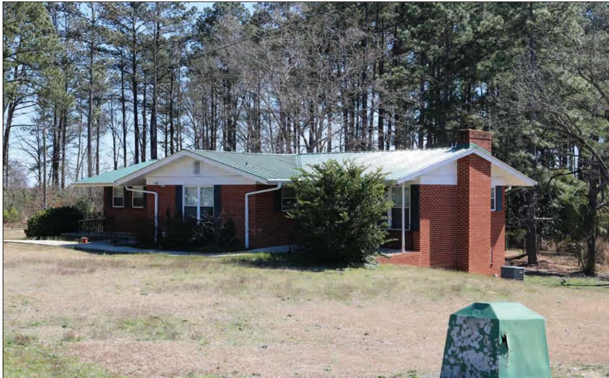
Figure 9.7. 2407 Hickory House Road, Facing Southeast
