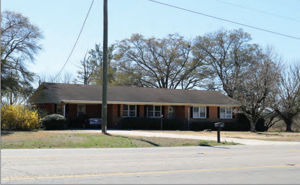
Figure 9.6. 2476 Tramway Road, Facing South
