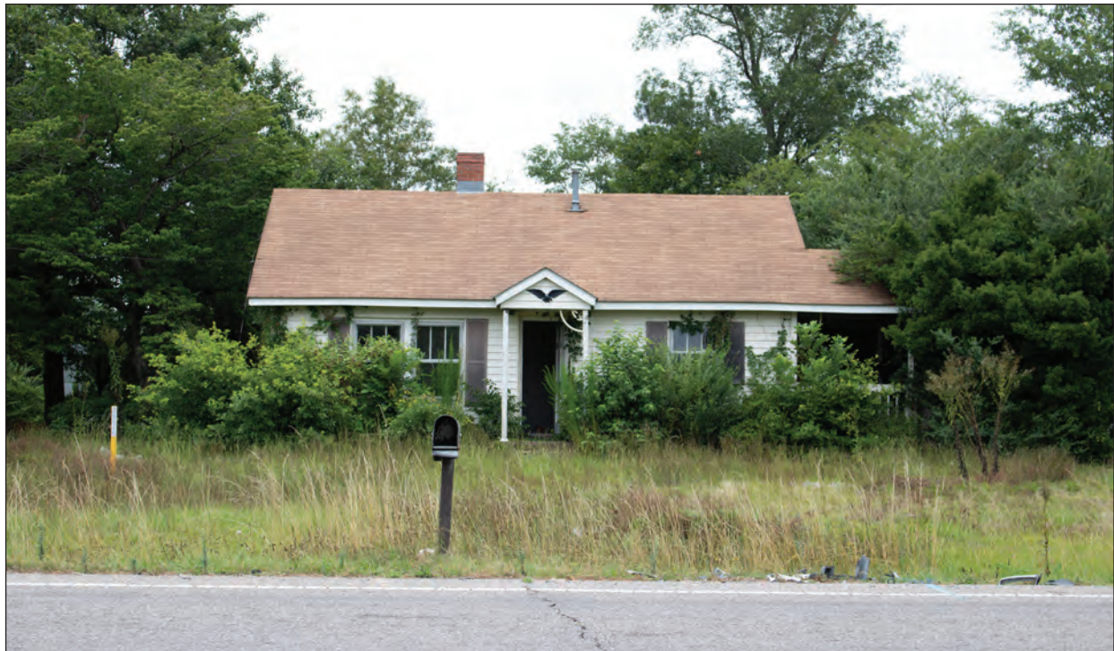
Figure 3.7. 1205 Broadway Road (LE0407), Facing North
