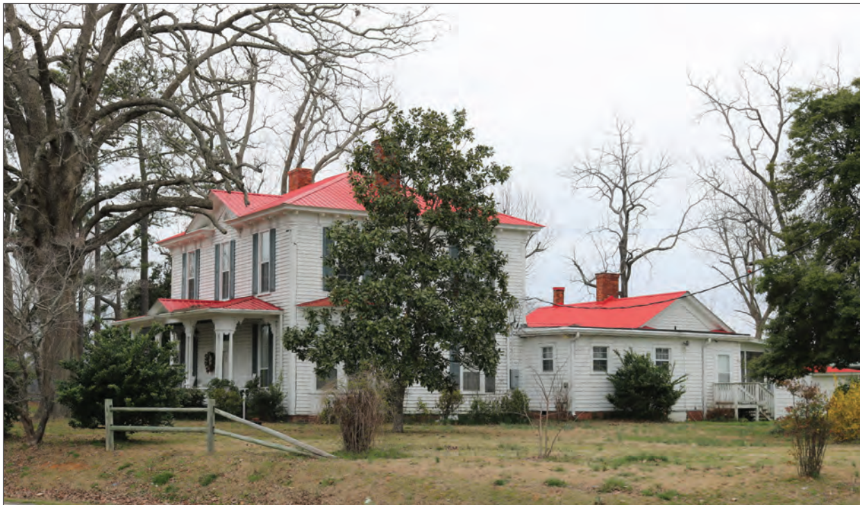
Figure 12.5. Kenneth H. Worthy House, Façade and East Elevation, Facing Northwest
