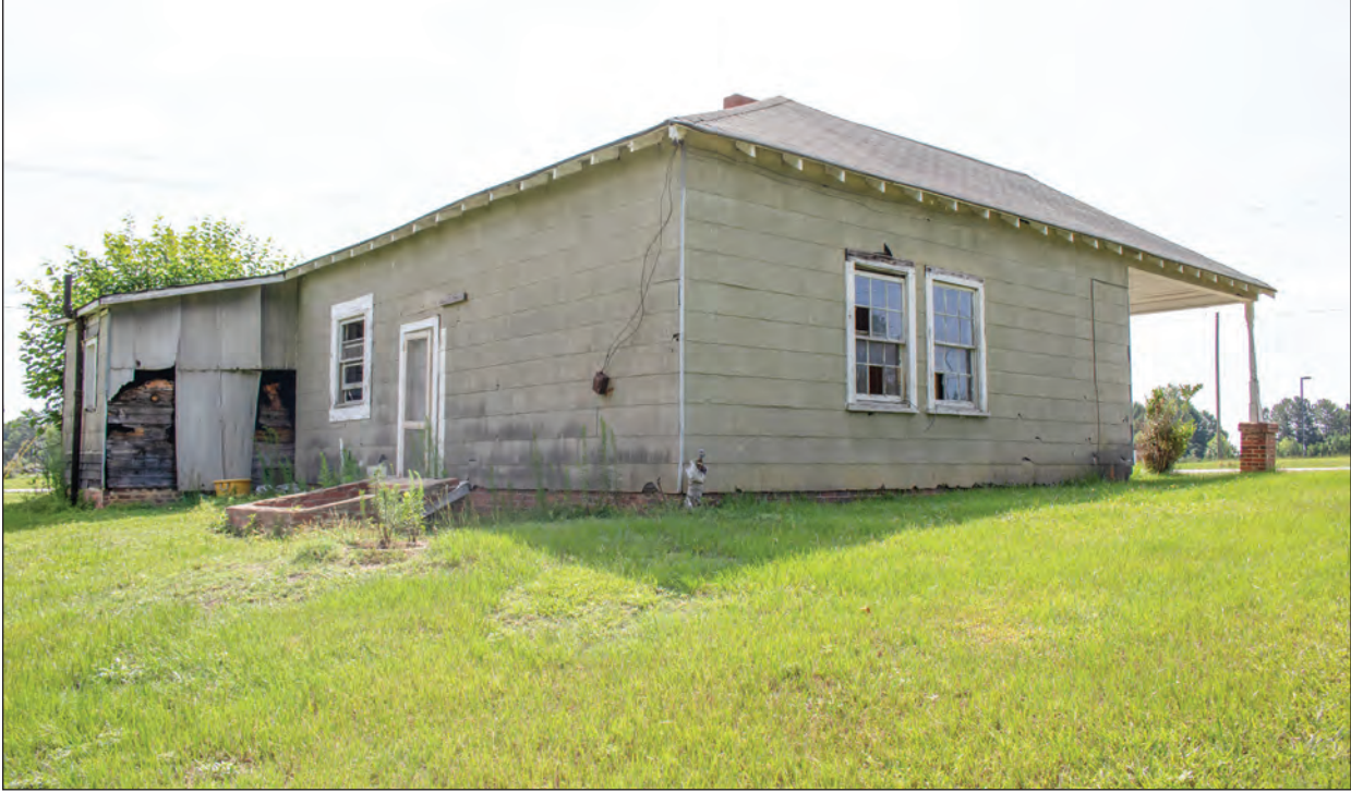
Figure 6.3. Robert Worthy Service Station, Facing Southeast
