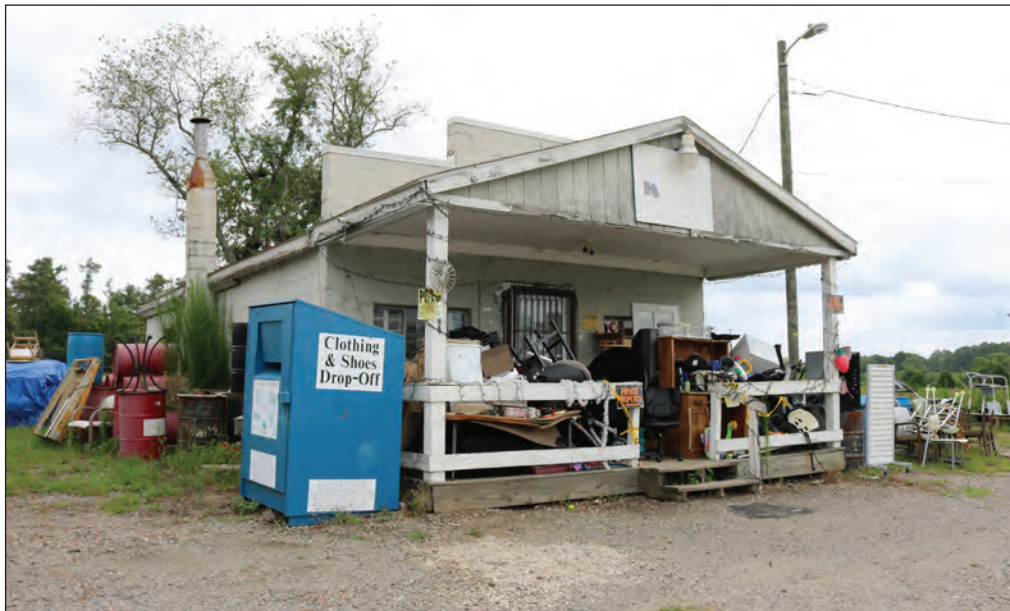
Figure 6.7. 1805 Broadway Road (LE0581), Facing Northeast
