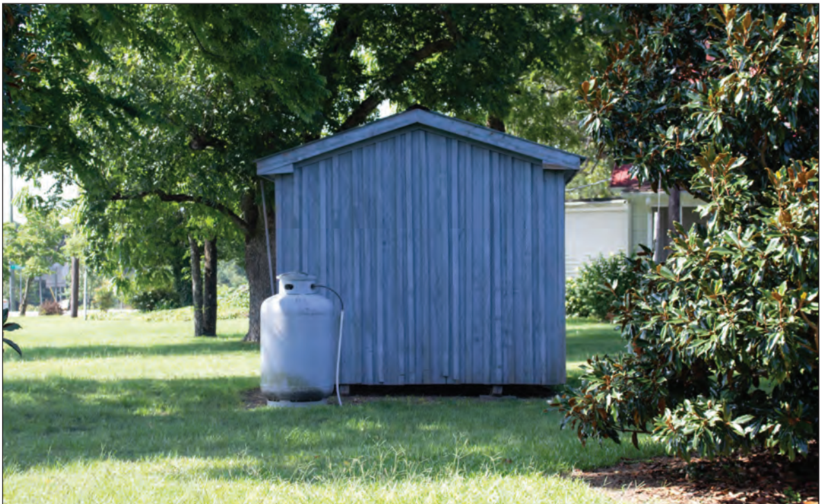
Figure 12.10. Gable-roof Storage Shed, Facing South
