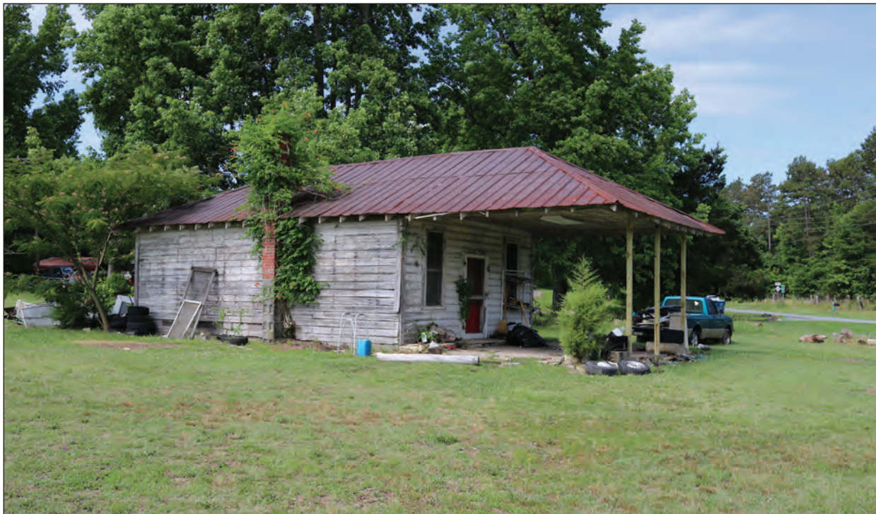
Figure 6.9. Coble Service Station (GF1924), Facing Southwest
