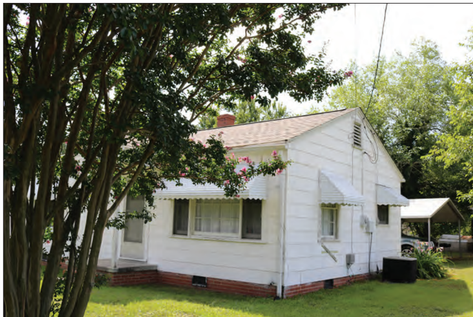
Figure 3.3. Makepeace House (LE0864), West Elevation, Facing Southeast
