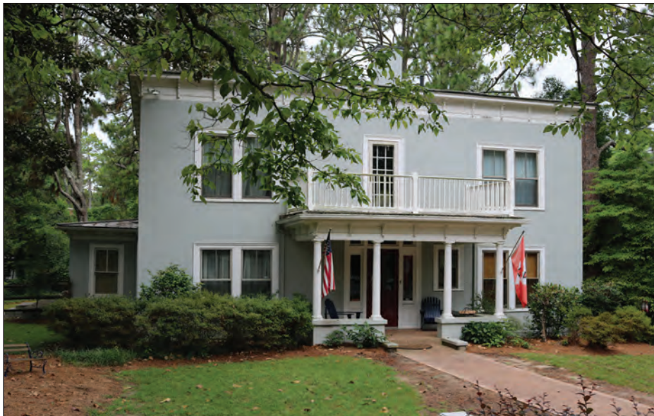
Figure 12.13. Dr. Holt House (MR0361), 560 E. Massachusetts Avenue in Southern Pines, Facing Southwest
