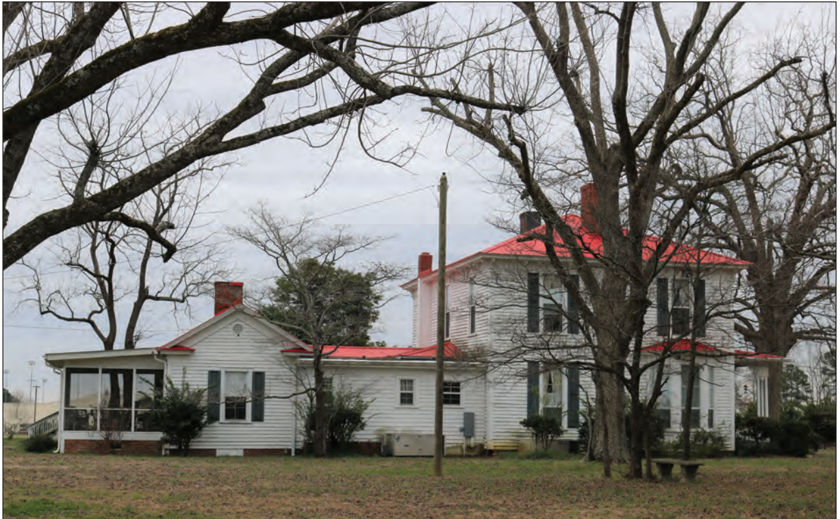
Figure 12.7. Kenneth H. Worthy House, West Elevation, Facing East
