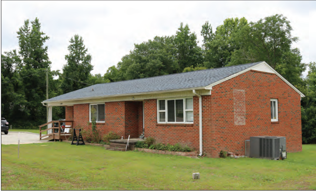
Figure 7.7. 1100 Broadway Road (LE0399), Facing Southeast
