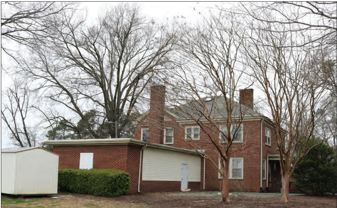
Figure 11.4. Raymond R. Knight Farm dwelling, South Elevation, Facing Northwest
