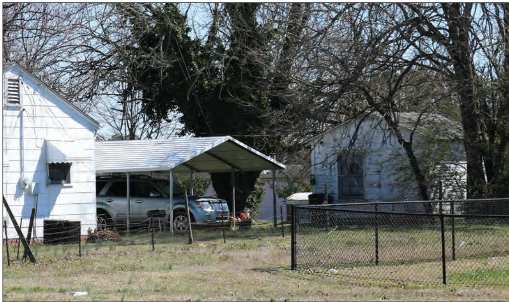
Figure 3.4. Makepeace House (LE0864), Outbuilding and Carport, Facing South
