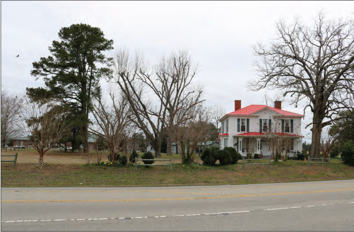
Figure 12.8. Kenneth H. Worthy House, Site and Lee County Co-op Extension, Facing South
