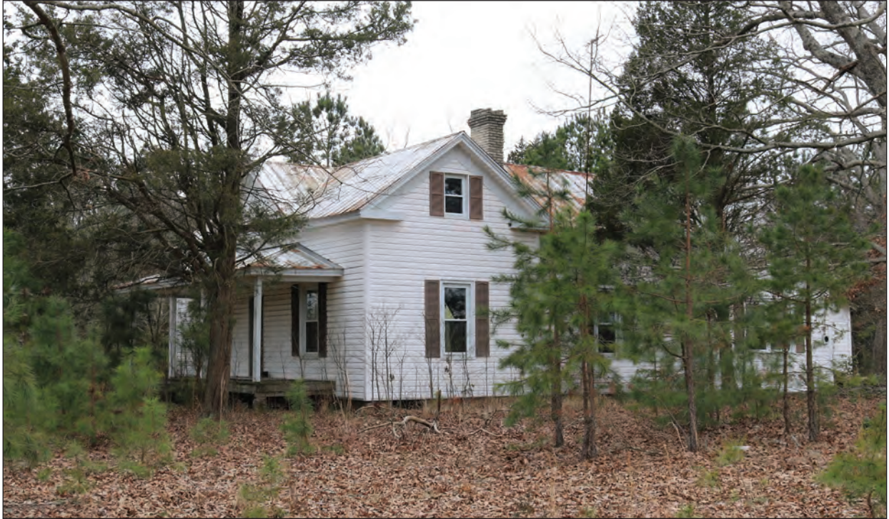
Figure 14.3. Shirley B. Wall House Façade and East Elevation, Facing Northwest
