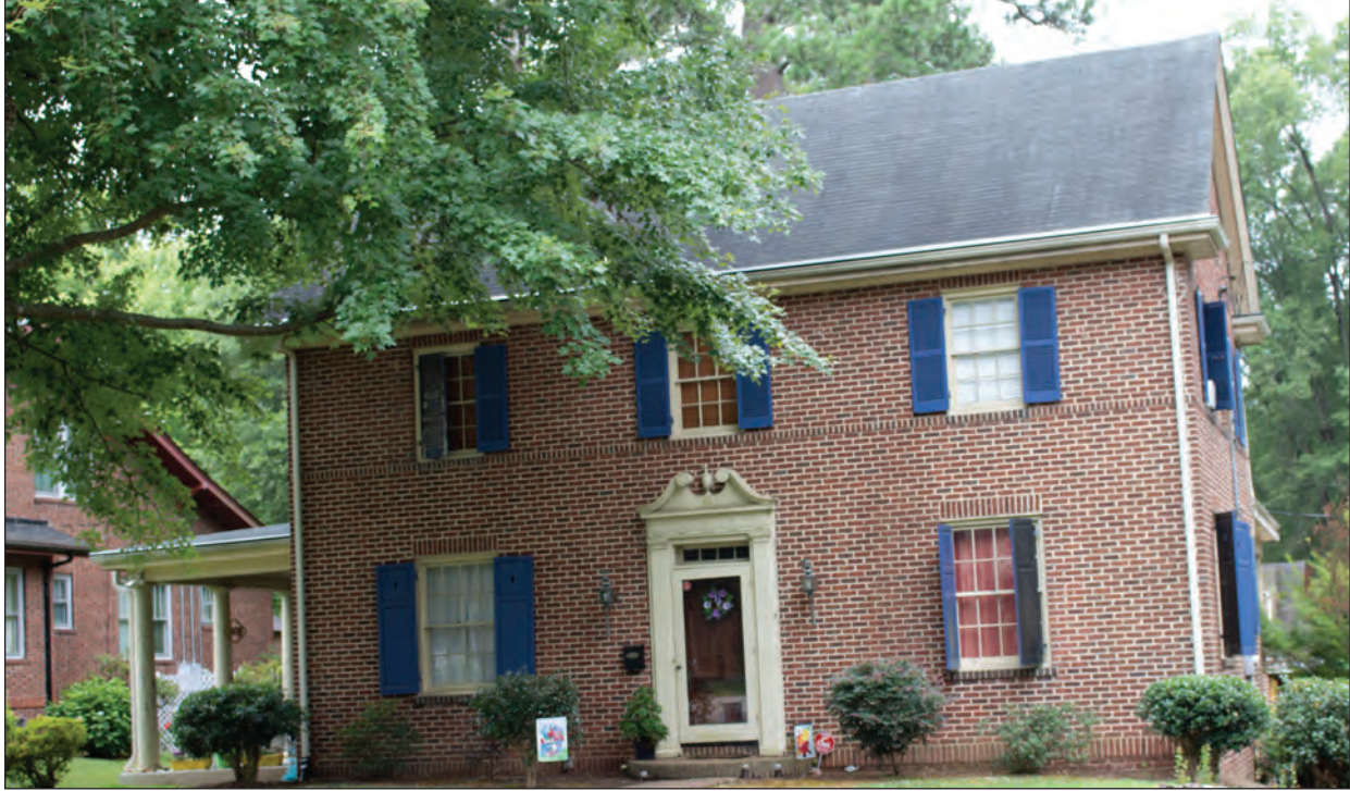
Figure 11.10. J.C. Pittman House, 311 N. Gulf Street, Facing Southeast
