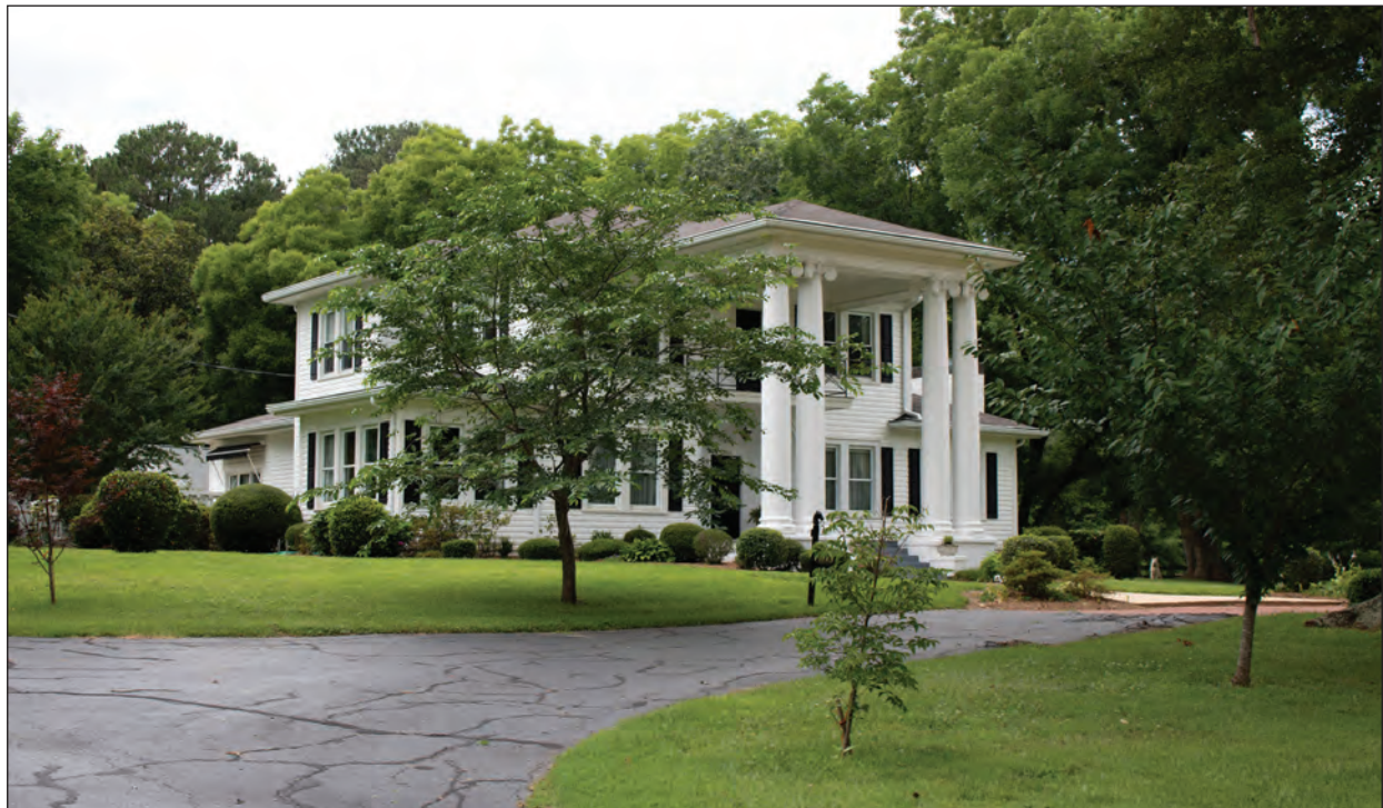
Figure 2.19. Buffalo Rural Historic District, Representative Anchor Dwelling
