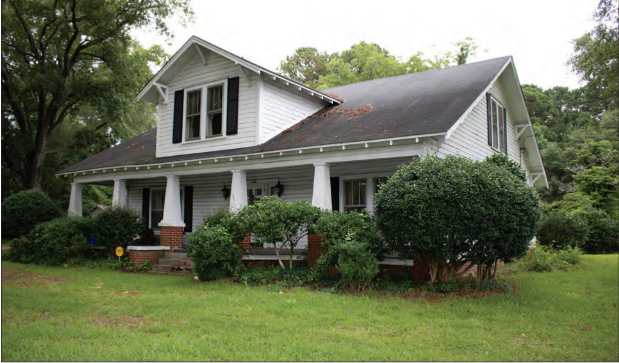
Figure 8.16. 1127 Broadway Road (LE0406), Facing Southeast
