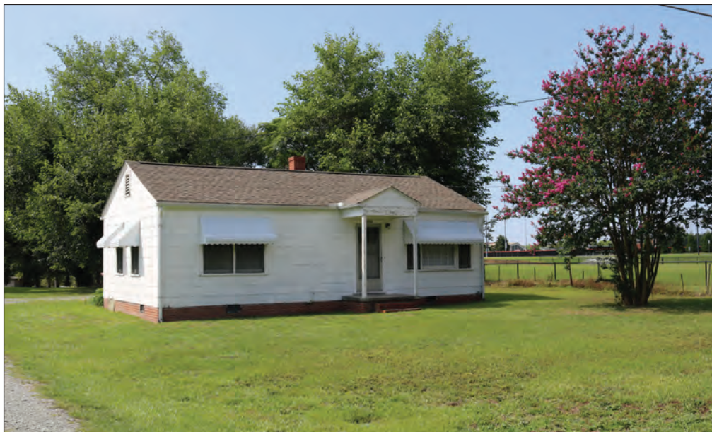
Figure 3.1. Makepeace House (LE0864), Façade and East Elevation, Facing Southwest
