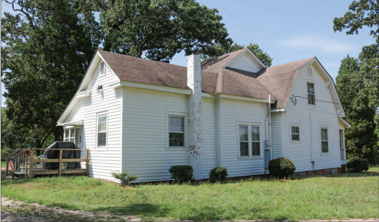
Figure 8.5. John W. Jackson Farm, North and East Elevations, Facing Southwest.
