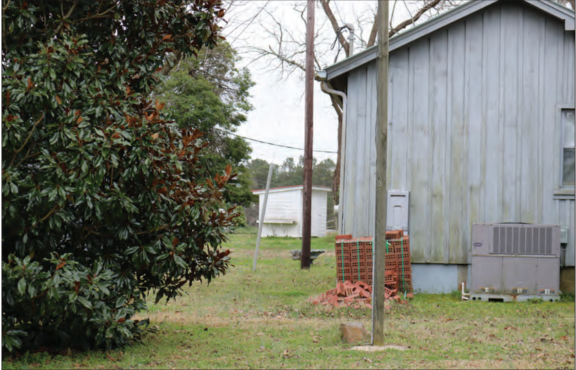
Figure 12.9. Storage Shed, Facing East
