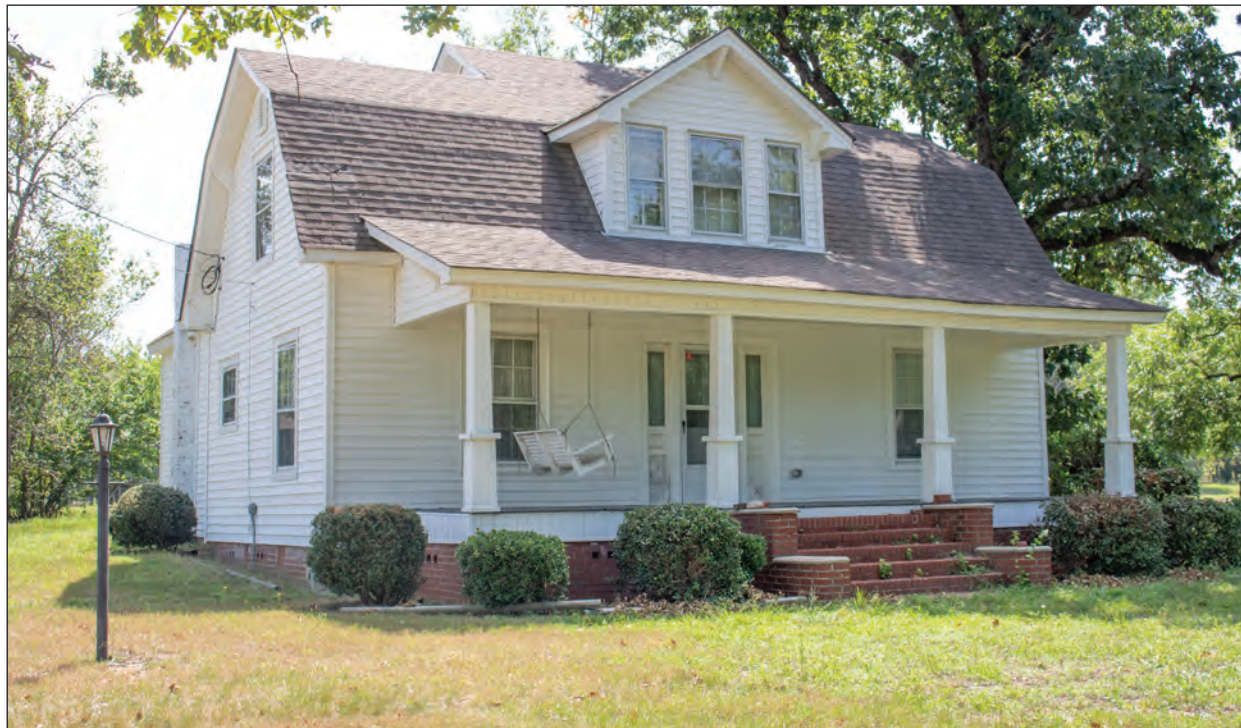
Figure 8.4. John W. Jackson Farm, Façade and North Elevation, Facing Southeast.
