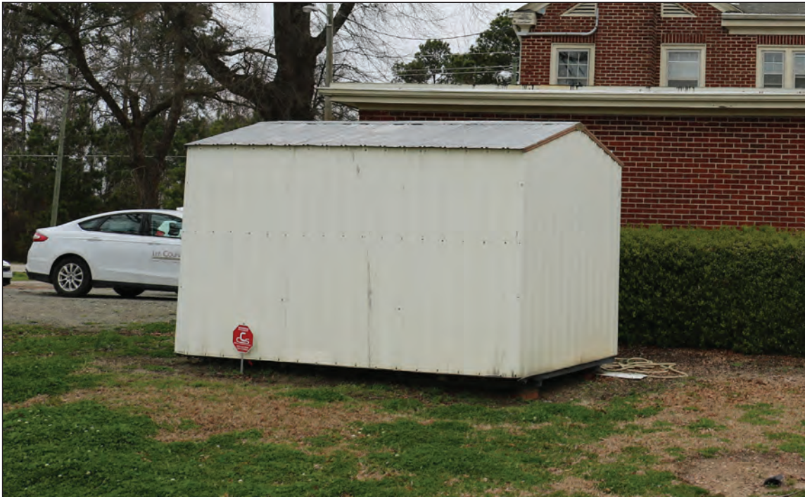
Figure 11.9. Pre-fabricated Storage Building, Facing Southeast
