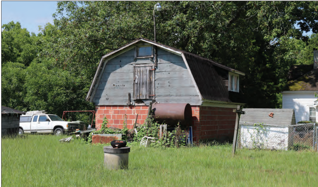
Figure 8.8. John W. Jackson Farm, Multi-use Garage, Facing Southwest
