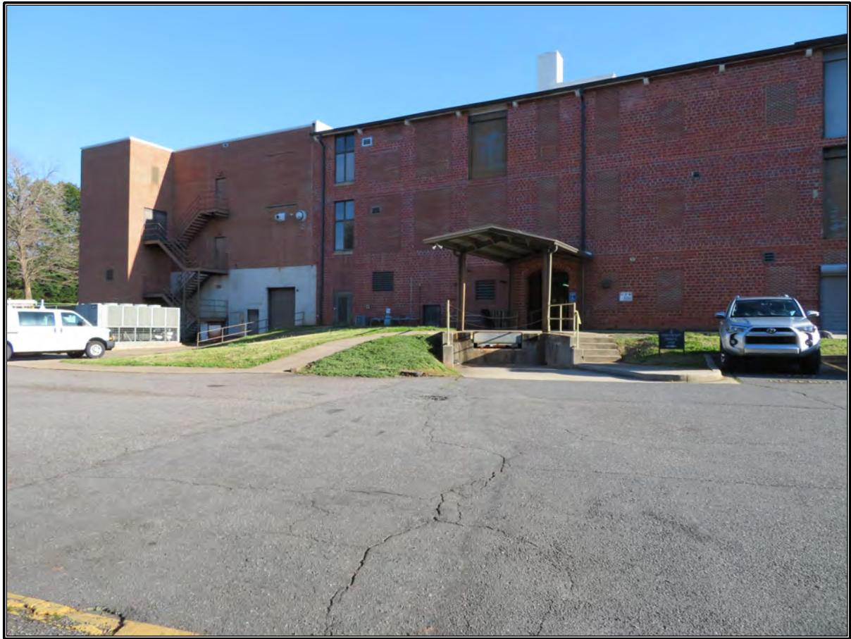
Figure 11. View of rear (south) elevation, looking northwest.
