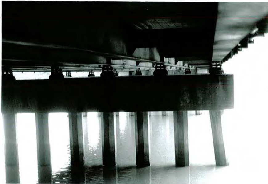
191:20. Underneath view of east span.
