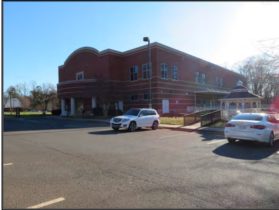
Figure 14. View of classroom building, rear (south) and west elevation, looking northeast.
