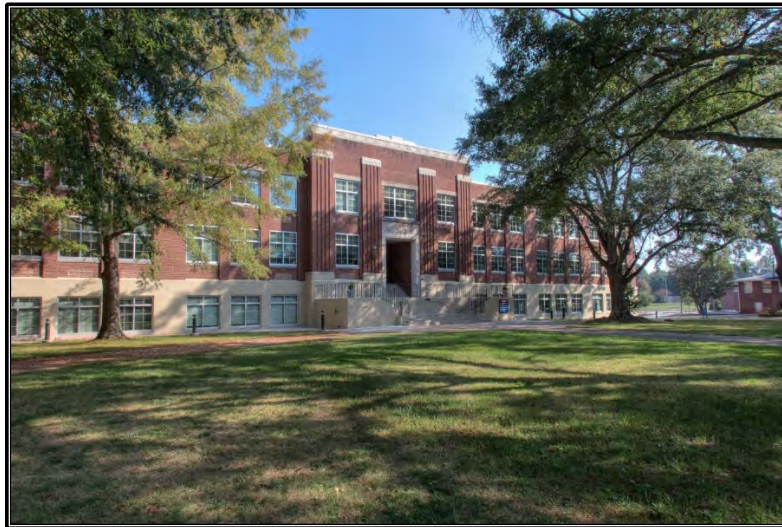
Figure 37. View of (former) Shelby High School, Shelby, North Carolina (Gailius 2015).
