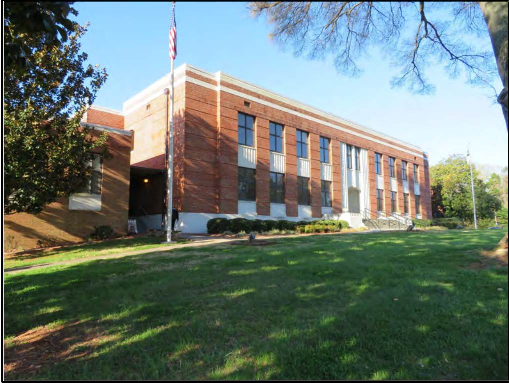
Figure 9. View of façade (north) elevation with east addition, looking southwest.
