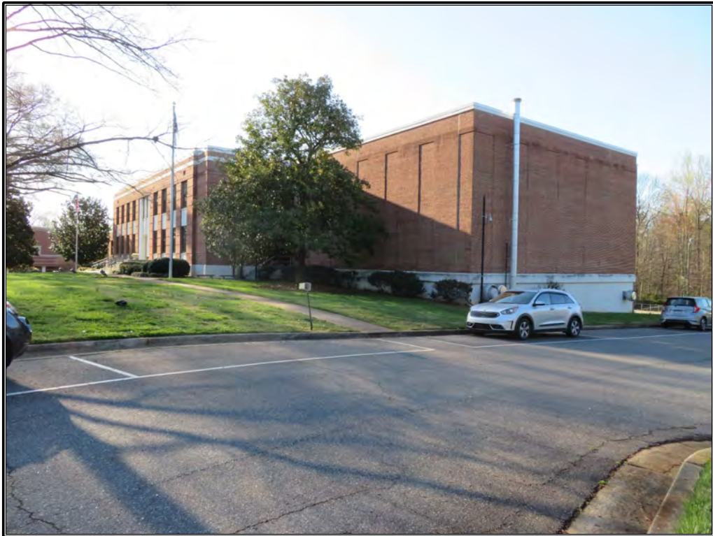
Figure 10. View of west elevation, looking southeast.
