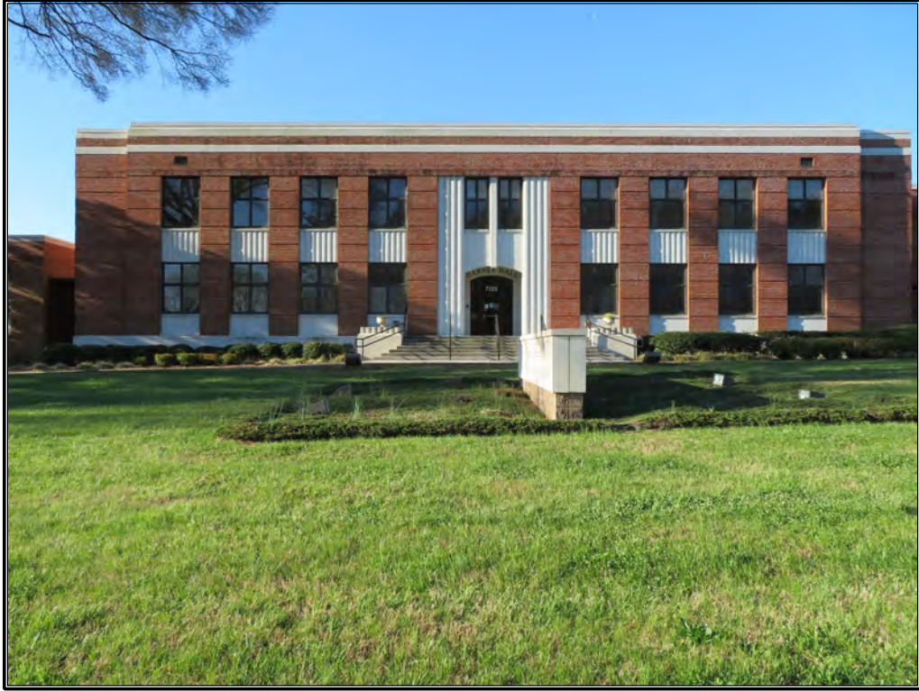
Figure 7. View of façade (north) elevation, looking south.
