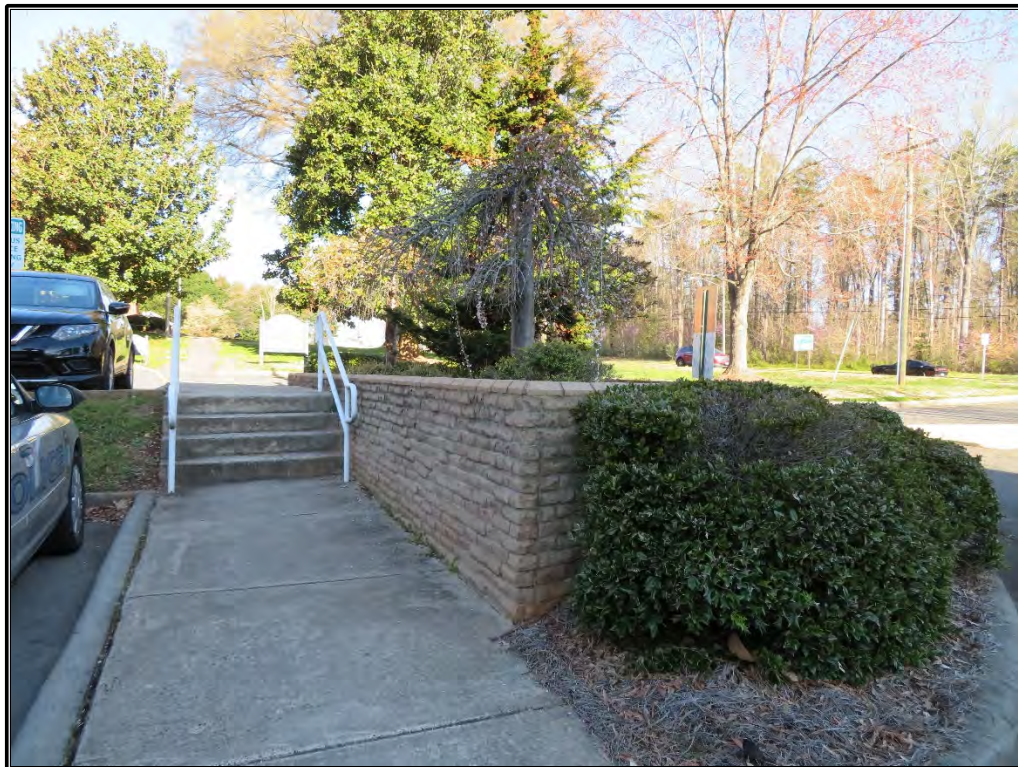
Figure 18. View of rusticated brick stair wall, looking northwest.
