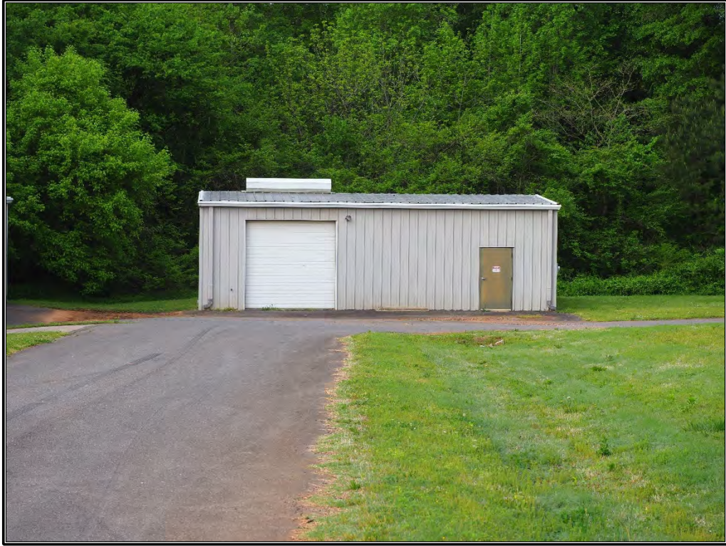
Figure 19. View of metal shed, looking southeast.
