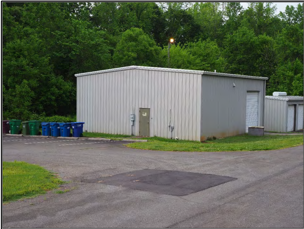
Figure 20. View of metal shed, looking south.
