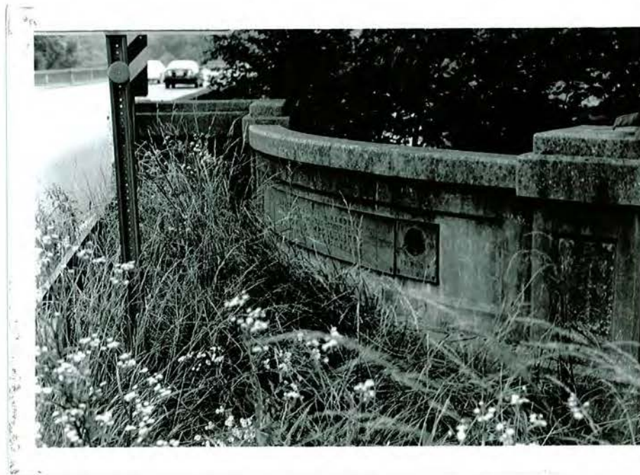
191:23. Memorial plaque and parapet at southwest corner.
