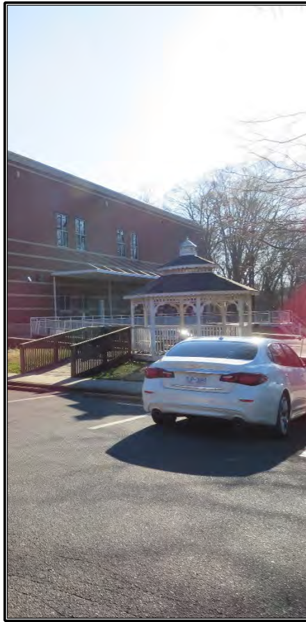
Figure 15. View of gazebo located south of the classroom building, looking northeast.
