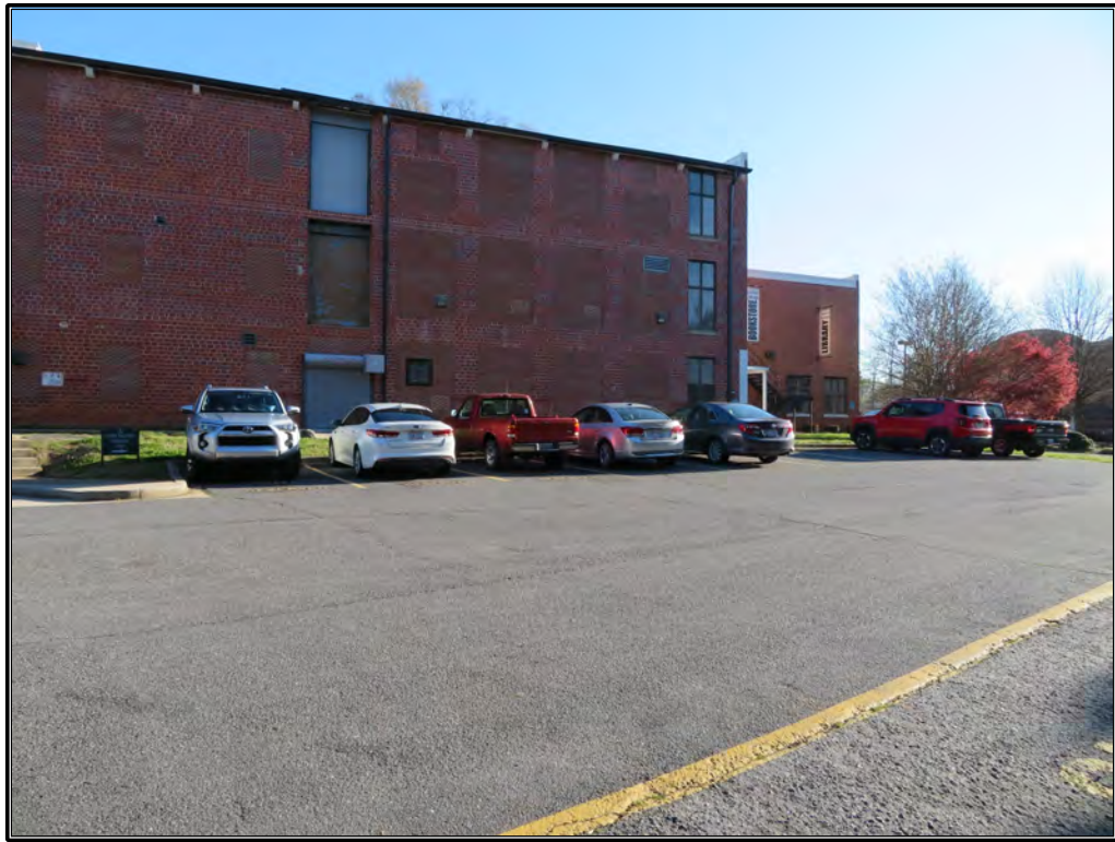
Figure 6. Rear (south) elevation showing infilled windows, looking northeast.
