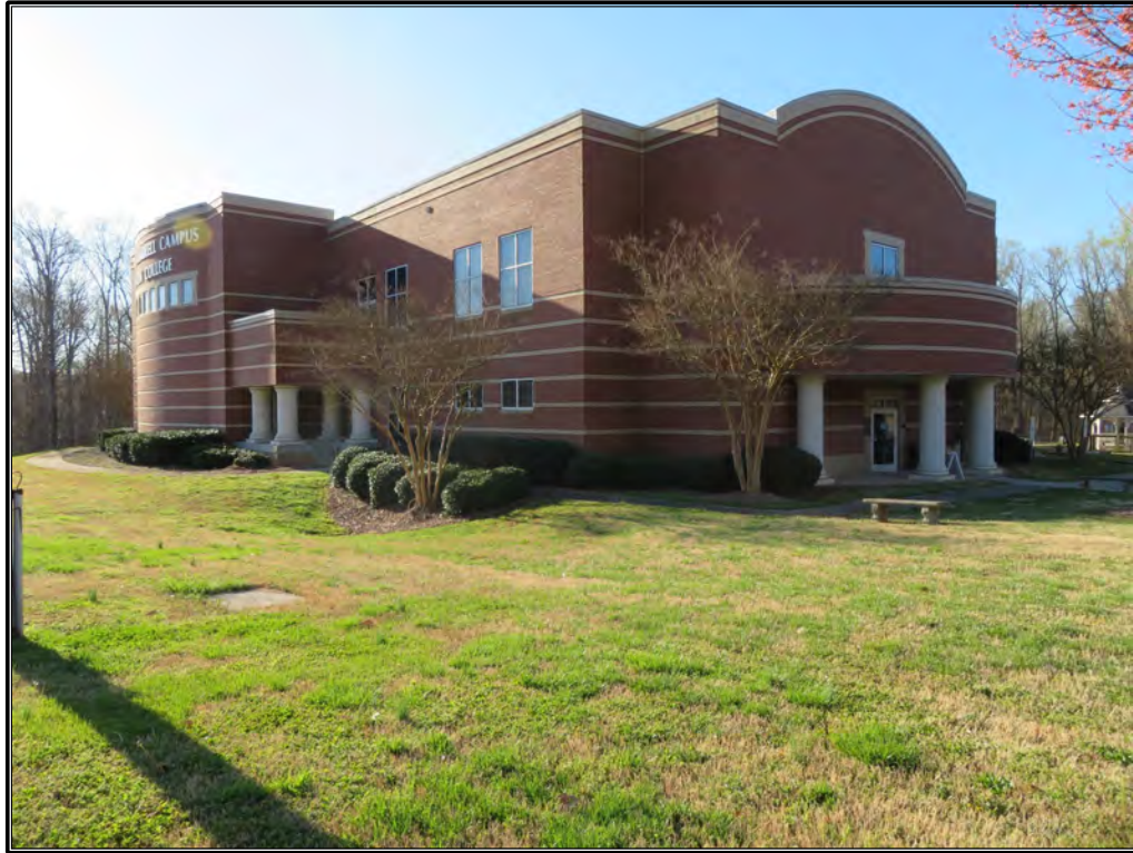
Figure 12. View of classroom building, façade (north) and west elevation, looking southeast.
