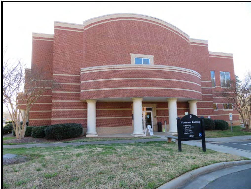
Figure 13. View of classroom building, west elevation, looking southeast.
