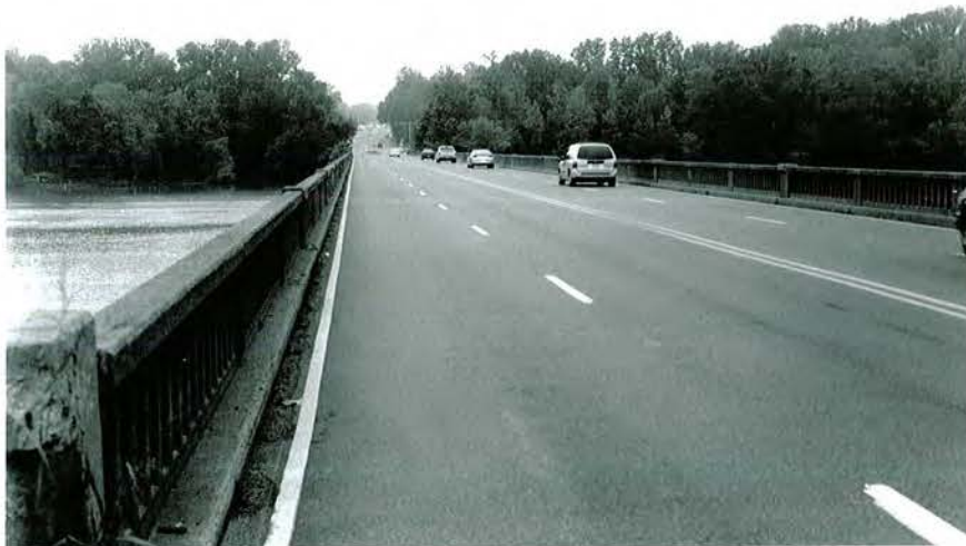
191:16. Through view looking west.
