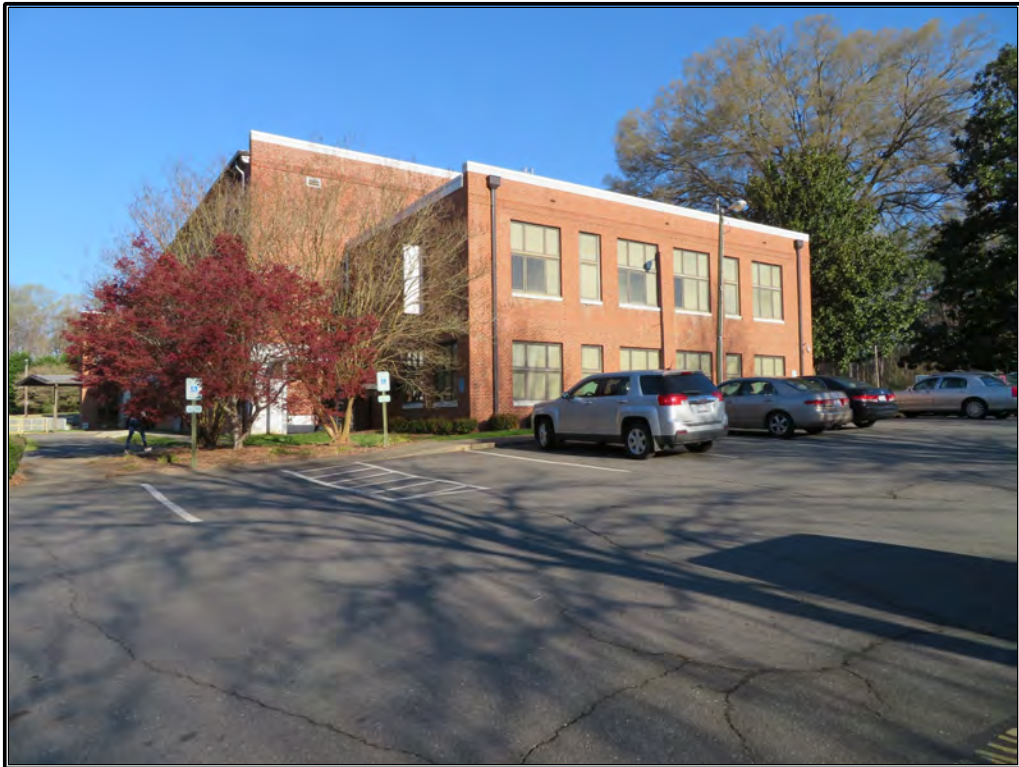
Figure 8. View of east elevation, looking northwest.
