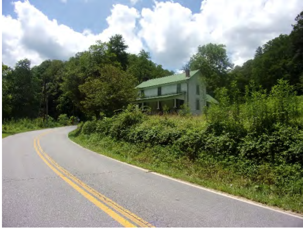
Figure 37. Caldwell Farm I-House, view to the southwest
