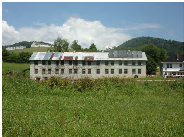
Figure 24. Chicken House #1, view of south elevation; the Joseph S. Wells House is visible at right.
