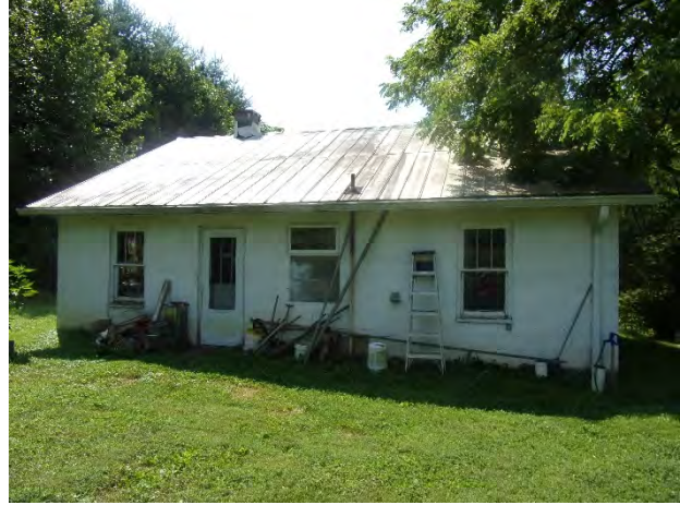
Figure 30. Tenant House #2 (Barn House), view of the north elevation
