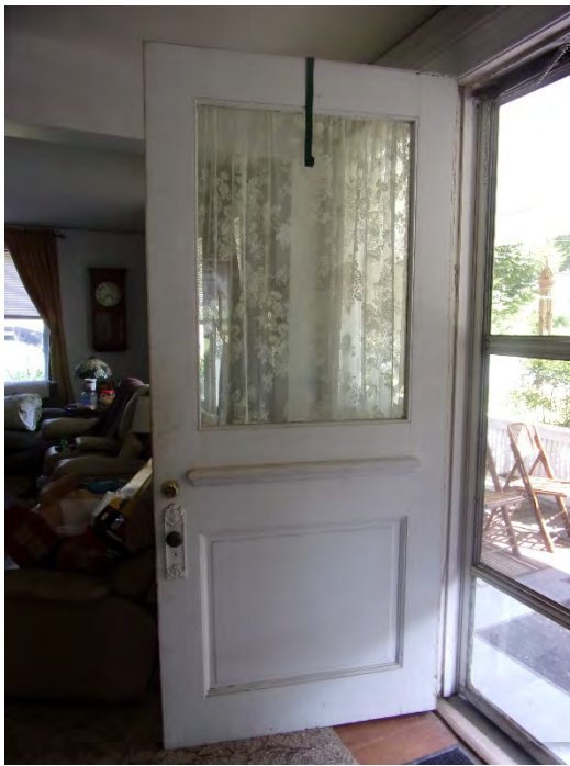
Figure 12. Joseph S. Wells House, front door detail
