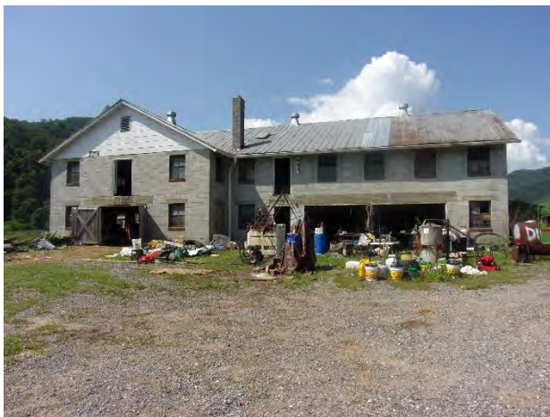
Figure 23. Chicken House #1, view of east elevation
