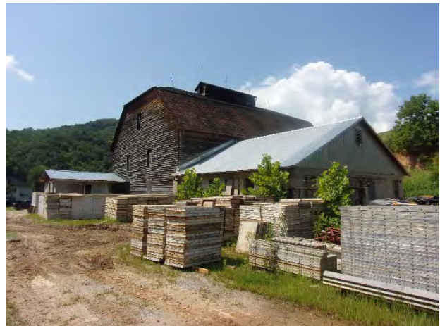
Figure 18. Joseph S. Wells Barn, view to the southwest
