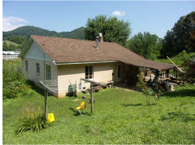
Figure 28. Tenant House #1, oblique view of the south and west elevations
