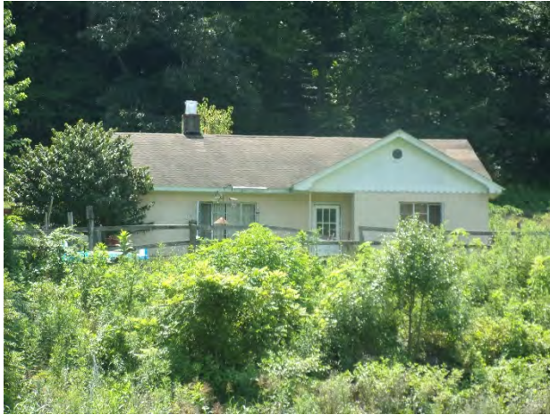
Figure 27. Tenant House #1, view of north façade
