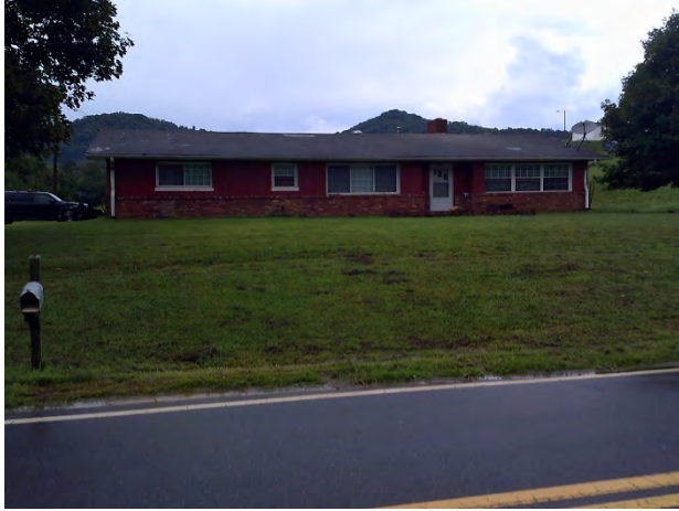
Figure 21. Maurice Wells House, view of south façade
