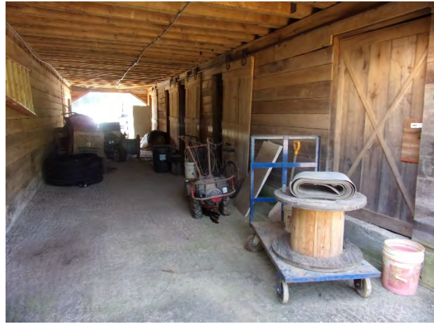
Figure 16. Joseph S. Wells Barn, view to the south inside the central bay
