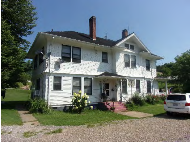
Figure 4. Joseph S. Wells House, view of south elevation
