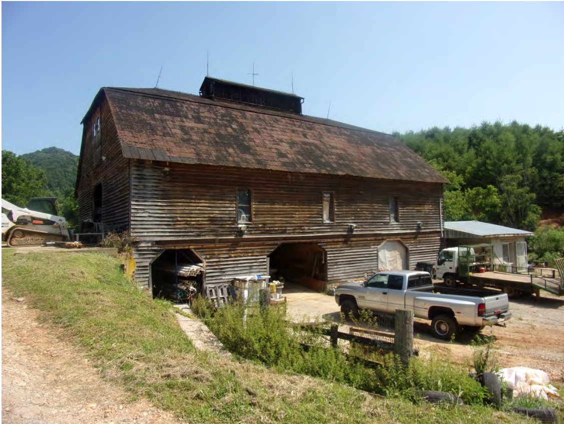
Figure 14. Joseph S. Wells Barn, oblique view of west and south elevations; the milk house is visible at right
