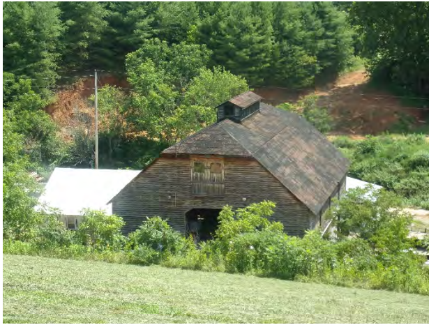
Figure 15. Joseph S. Wells Barn, view of west elevation from above
