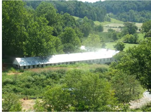
Figure 26. Chicken House #2, view of north and west elevations from above
