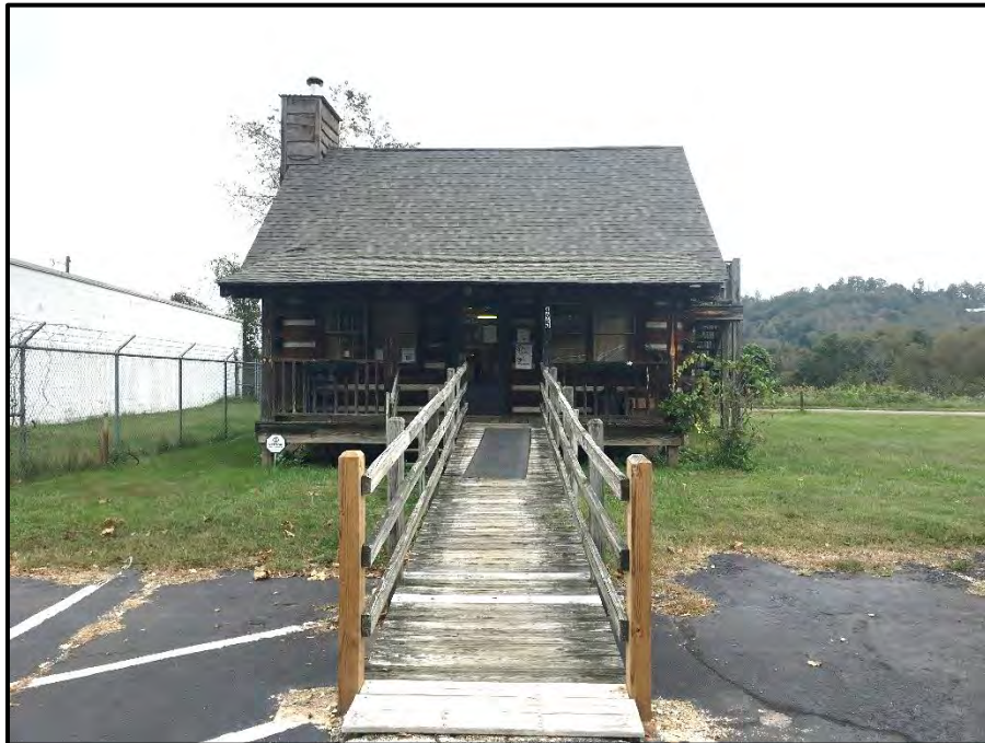
Figure 7. Log House, Looking Northeast.
