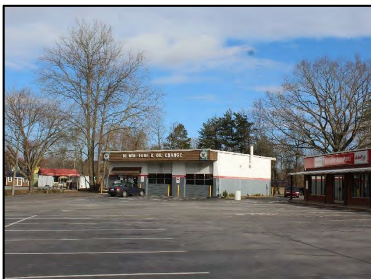
Figure 13. Service Garage, 507 New Leicester Highway, Looking North.
