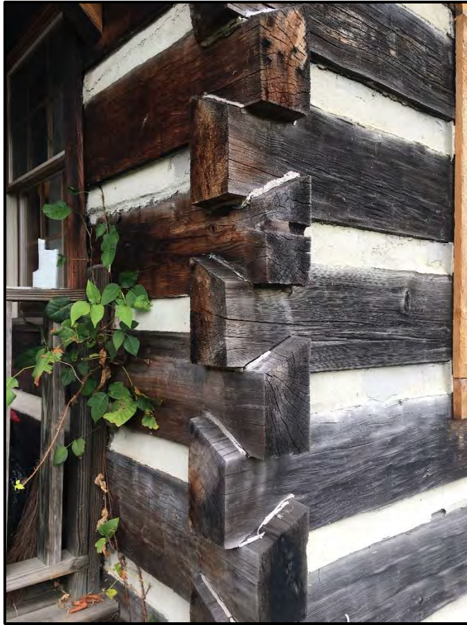
Figure 11. Detail of Corner Notching, Looking Northeast.
