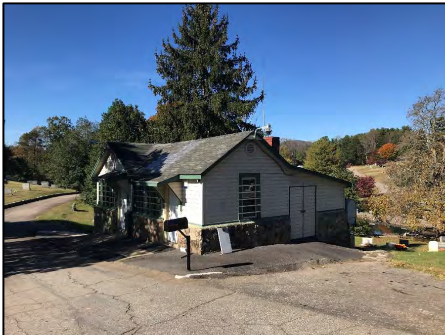
Figure 32. Green Hills Cemetery Office, Looking West.
