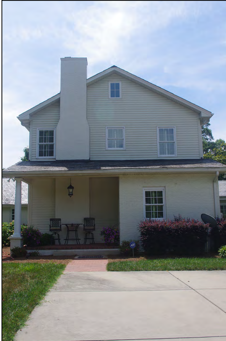
PLATE 8: West Elevation of Rear Ell, McIlwain-Suggs House (UN0484), Union County, North Carolina
