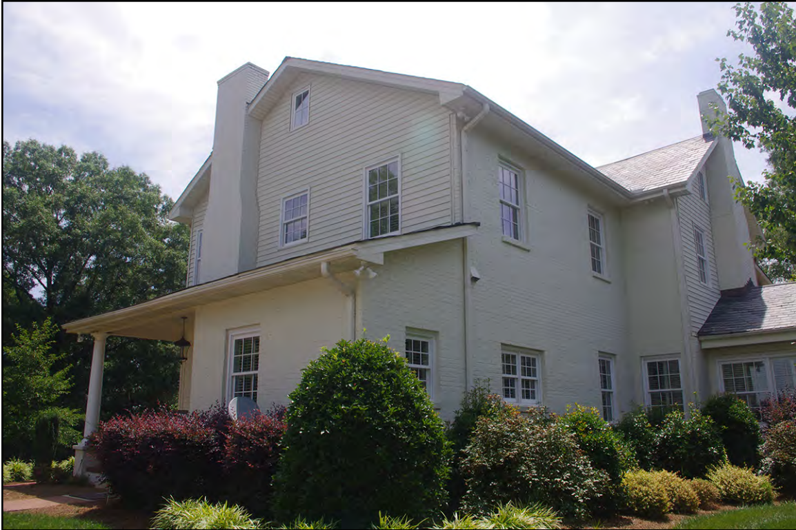
PLATE 9: Oblique View of South Elevation, McIlwain-Suggs House (UN0484), Union County, North Carolina
