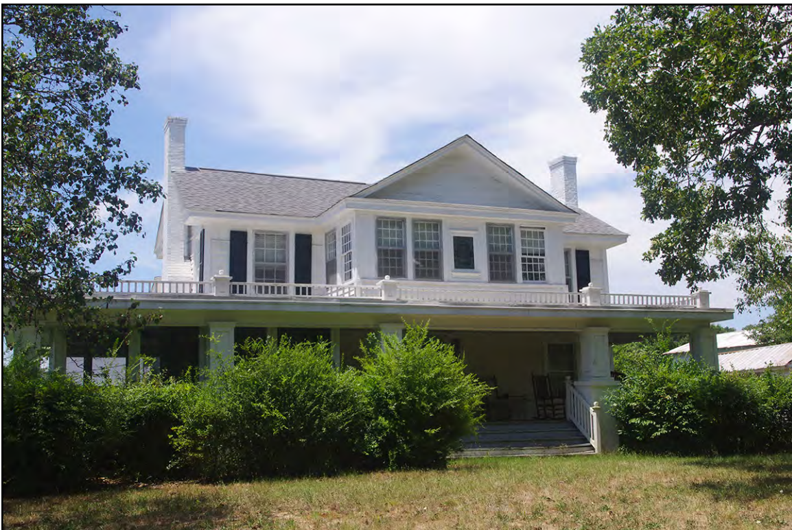
PLATE 21: William Bivens House (UN0830), South Elevation, Union County, North Carolina
