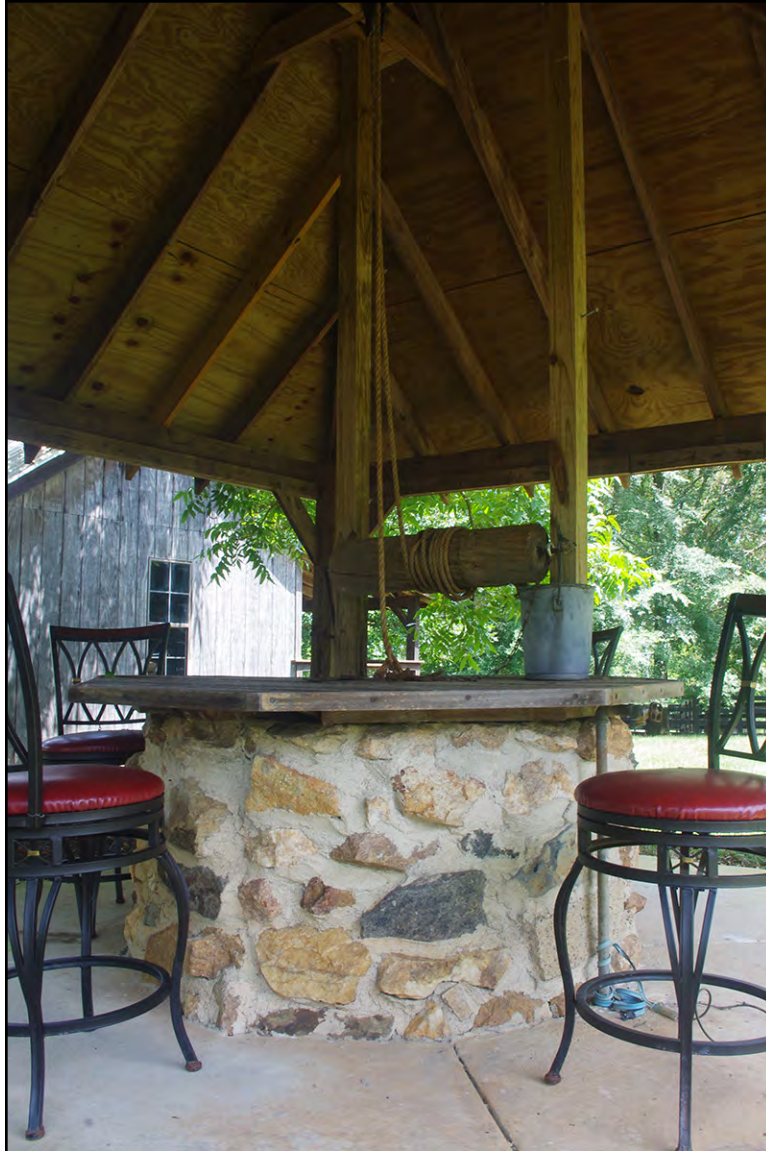
PLATE 16: Detail of Well House, Looking Northwest, McIlwain-Suggs House (UN0484), Union County, North Carolina
