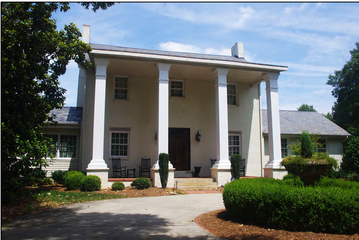
PLATE 3: East Elevation Detail of Main Block, McIlwain-Suggs House (UN0484), Union County, North Carolina
