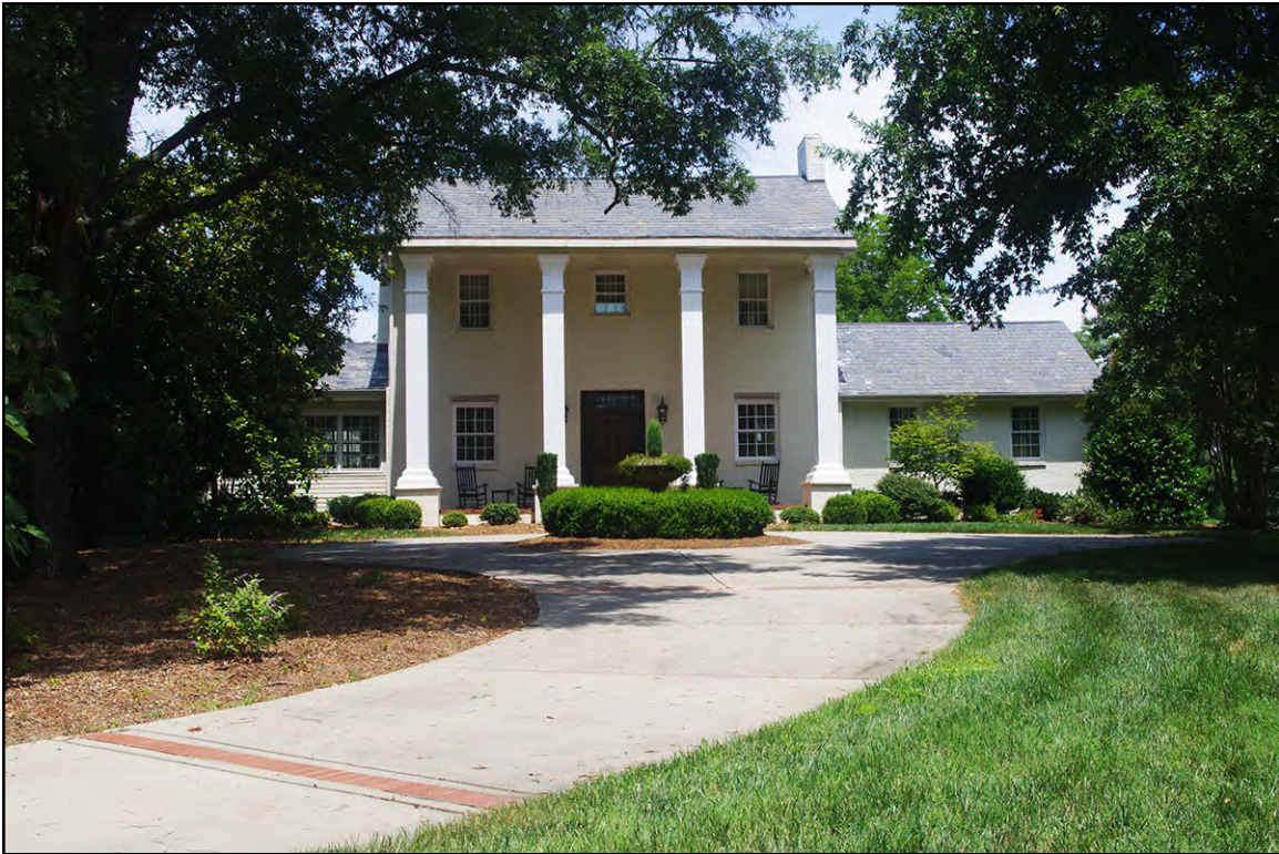
PLATE 1: East Elevation, McIlwain-Suggs House (UN0484), Union County, North Carolina
