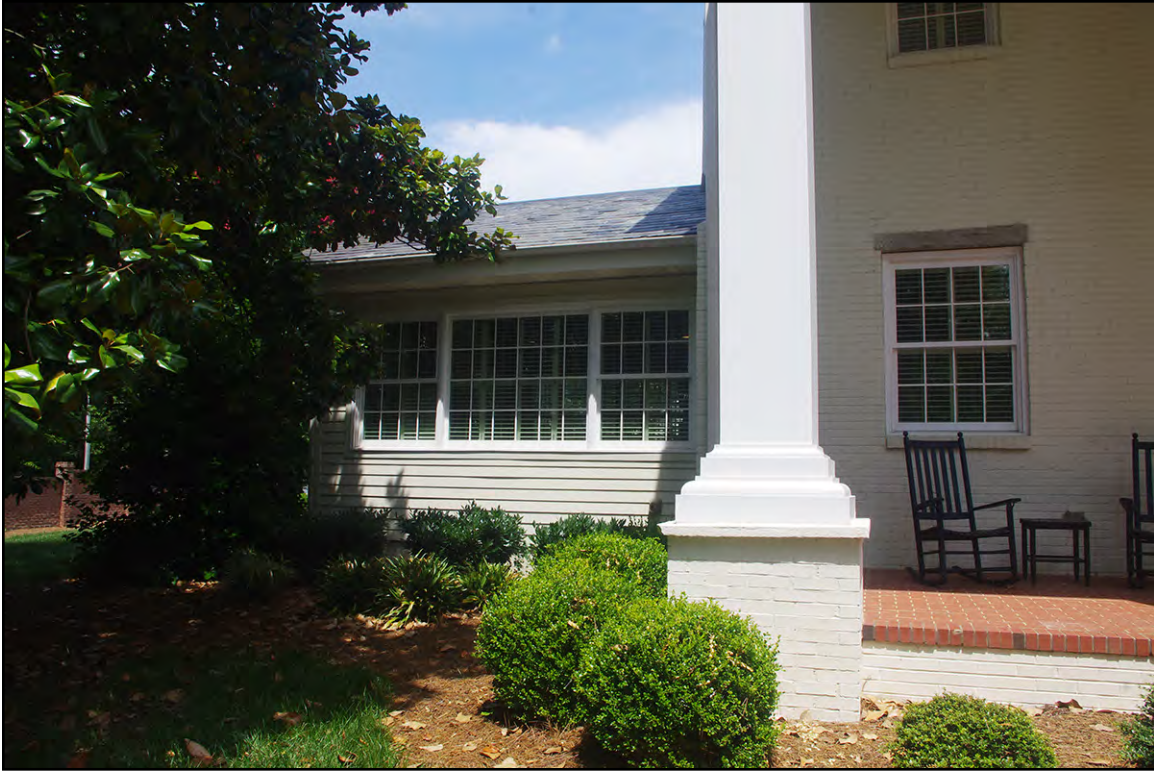
PLATE 5: East Elevation, Detail of Southern Side Wing, McIlwain-Suggs House (UN0484), Union County, North Carolina
