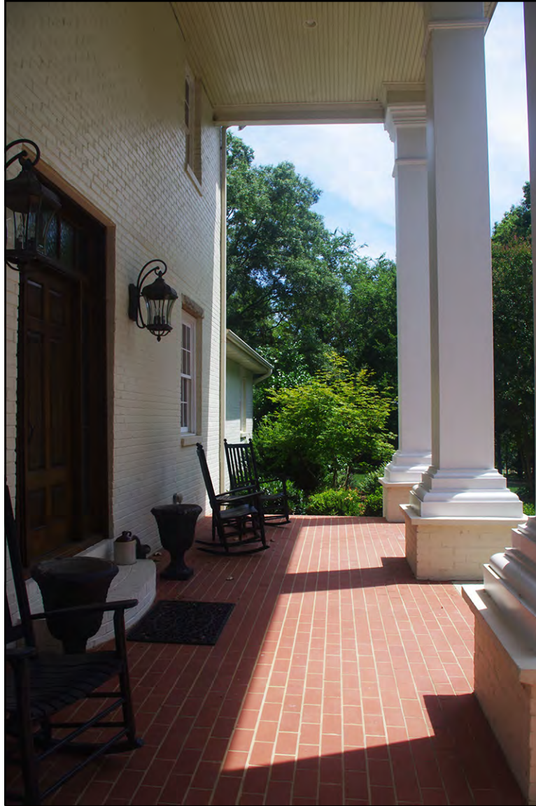
PLATE 4: Looking North from Front Porch of McIlwain-Suggs House (UN0484), Union County, North Carolina
