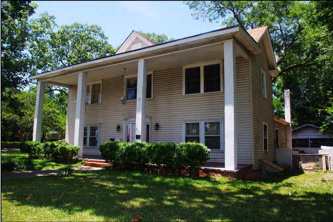
PLATE 20: W.H. Krauss House (UN0653), South Elevation, Union County, North Carolina
