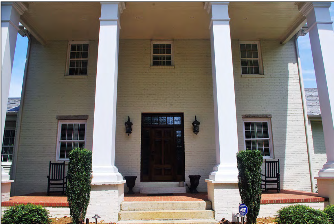
PLATE 25: East Elevation, Detail of Main Block, McIlwain-Suggs House (UN0484), Union County, North Carolina
