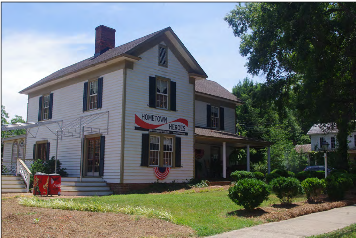
PLATE 23: Adams-Davis House (UN0147), Oblique of View North and West Elevations, Union County, North Carolina
