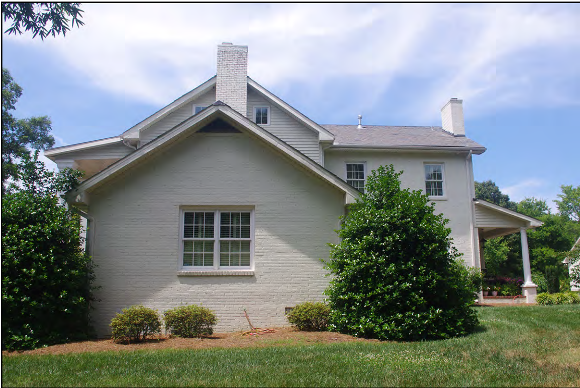
PLATE 6: North Elevation, McIlwain-Suggs House (UN0484), Union County, North Carolina
