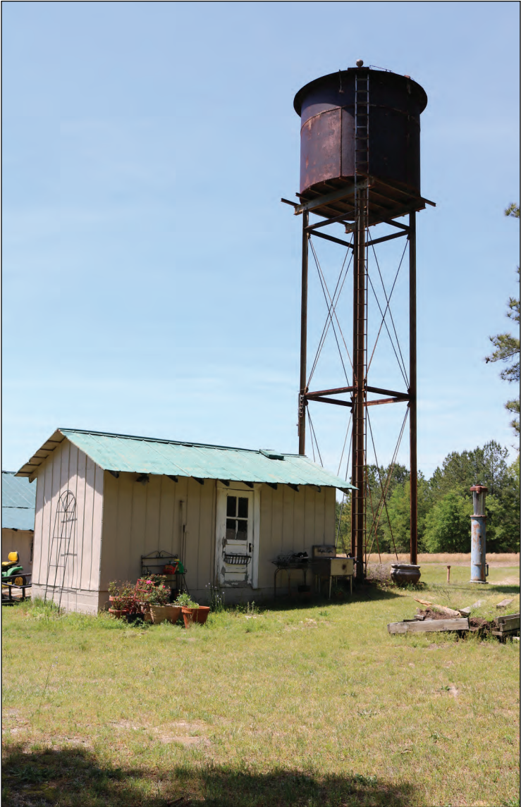
Figure 3.21. Water Tower, Looking Northwest.
