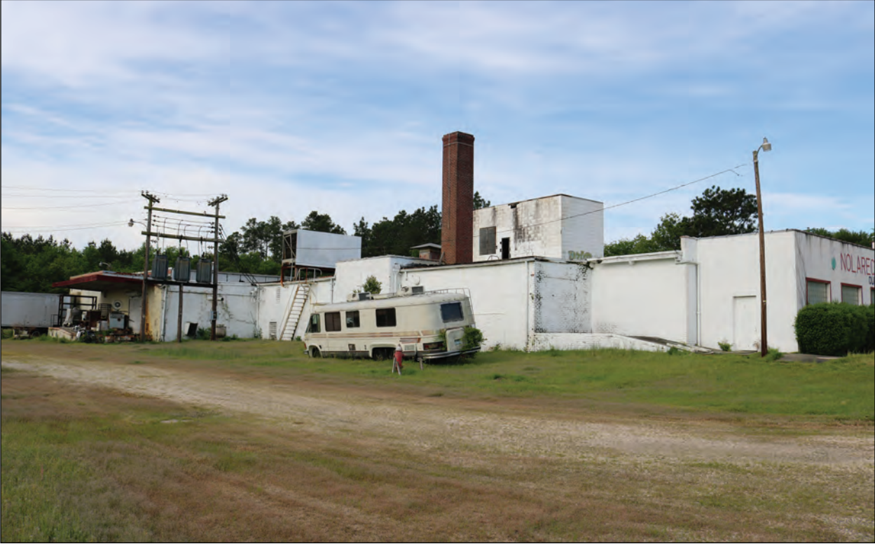
Figure 5.5. Aberdeen Hosiery Mills Co., East Elevation, Looking Southwest.
