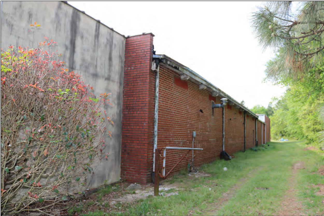
Figure 5.9. Aberdeen Hosiery Mills Co., West Elevation, Looking Southeast.
