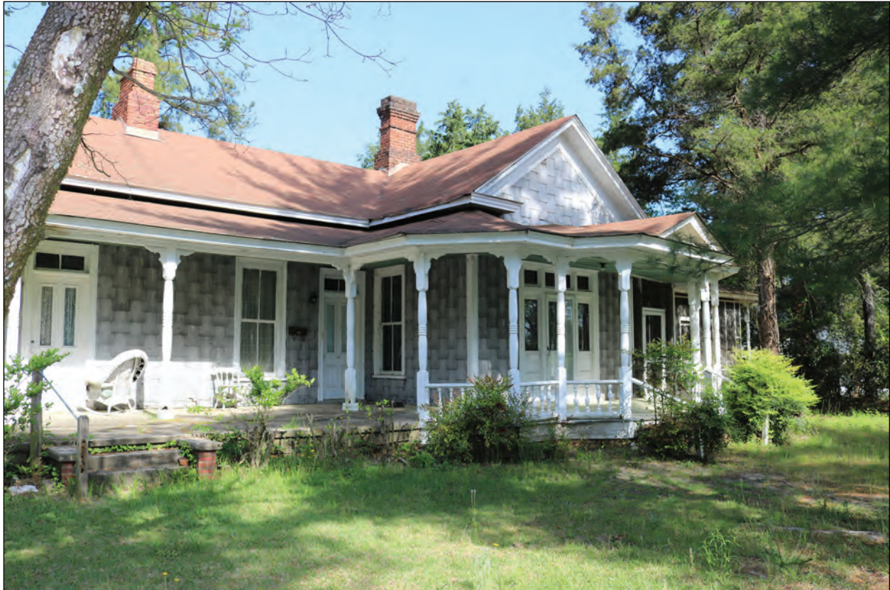
Figure 6.1. Hugh A. Keith House, Façade, Looking Northwest.
