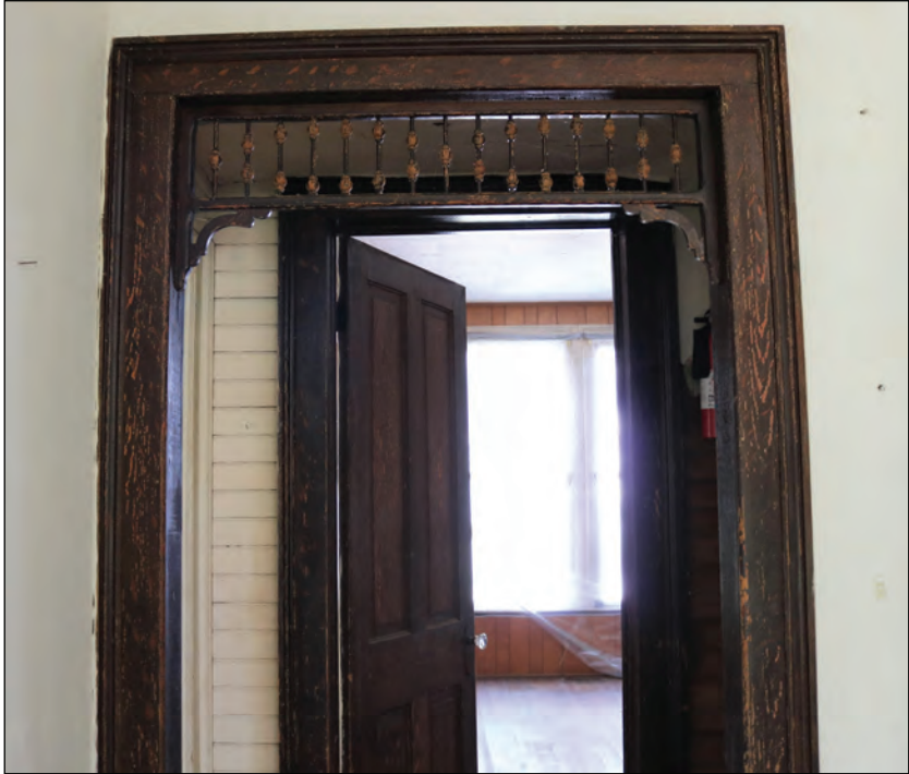
Figure 6.21. Hugh A. Keith House, Detail of Spindled Grille in the Formal Sitting Room.
