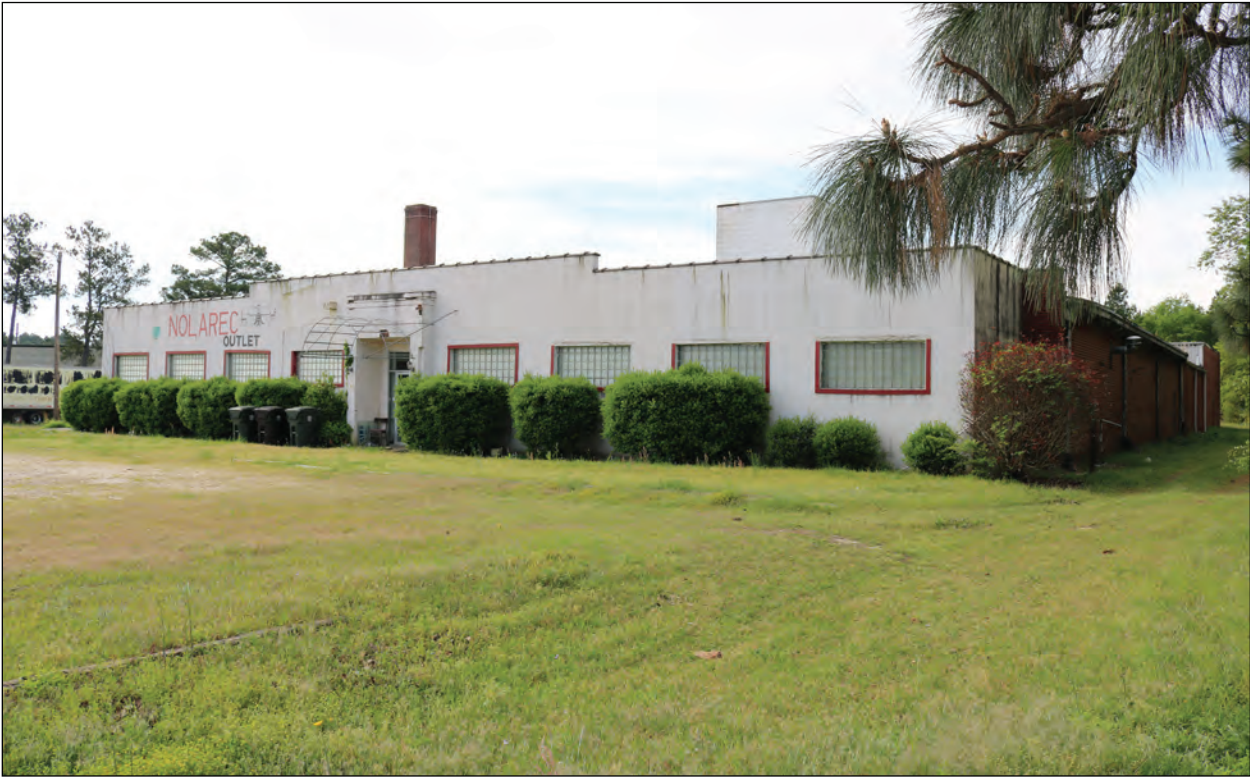
Figure 5.3. Aberdeen Hosiery Mills Co., Façade and West Elevation, Looking Southeast.
