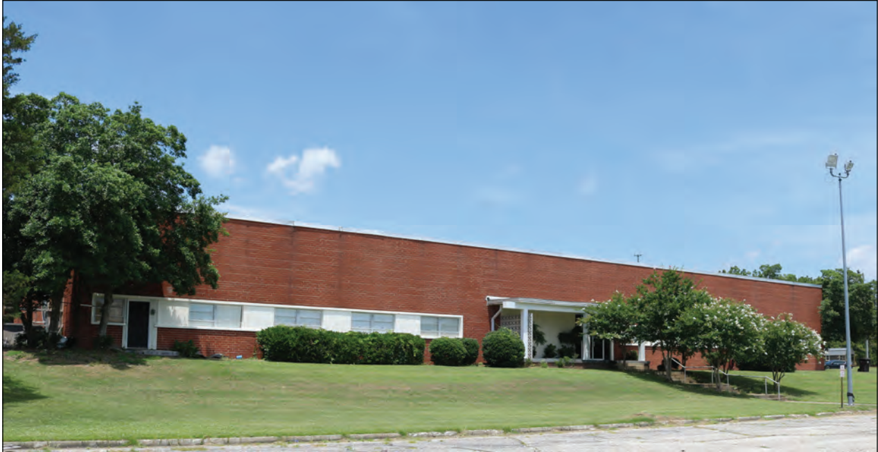
Figure 4.18. Gulistan Carpet Showroom, Looking Southeast.
