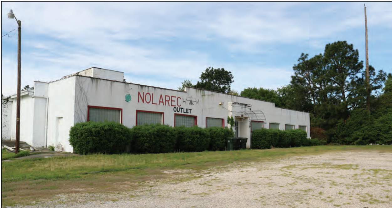
Figure 5.1. Aberdeen Hosiery Mills Co., Façade, Looking Southwest.
