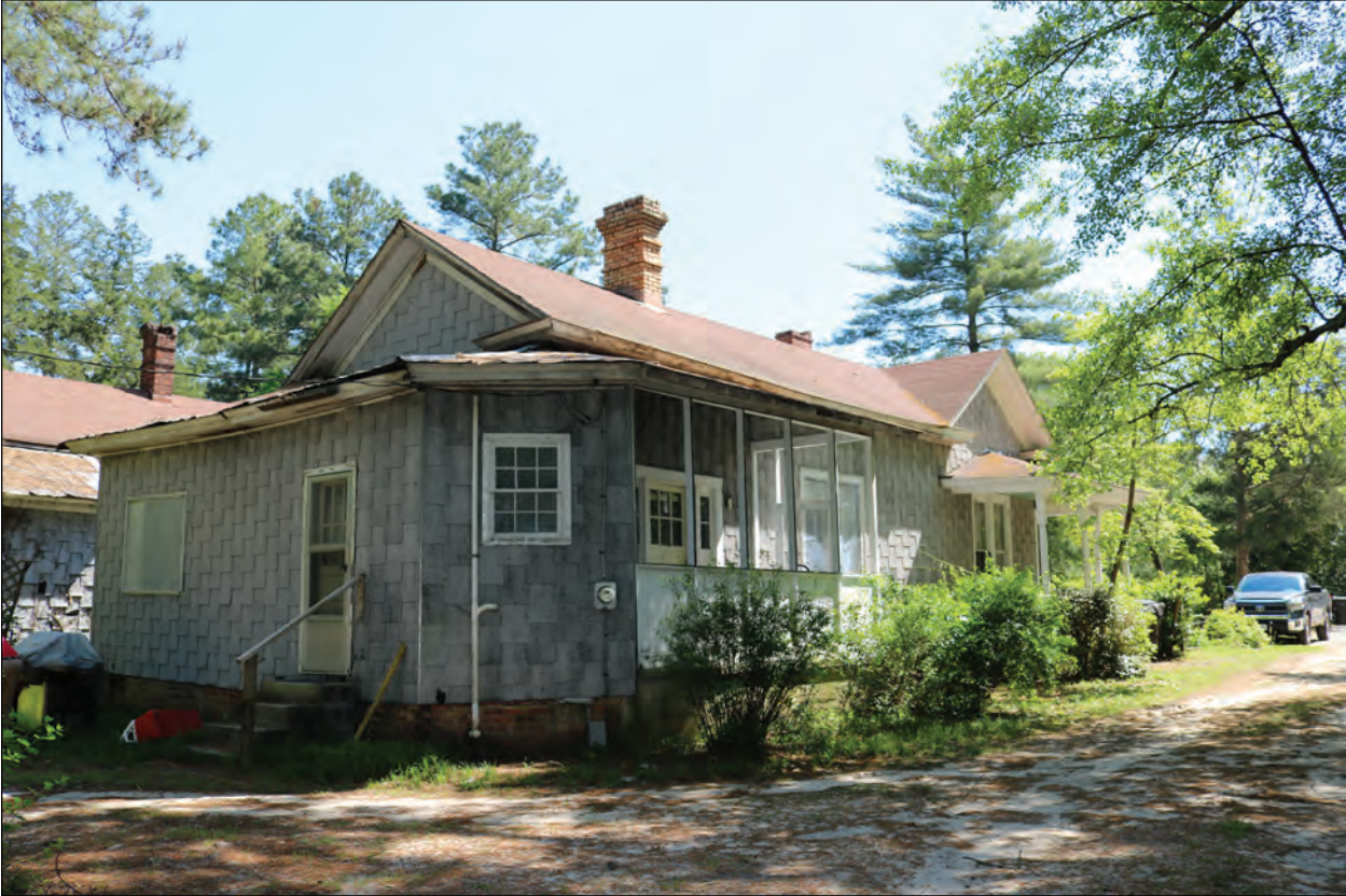
Figure 6.14. Hugh A. Keith House, South and West Elevations, Looking Northeast.
