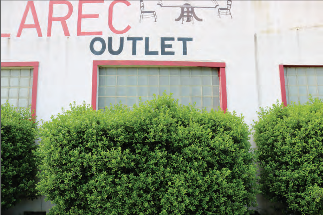
Figure 5.11. Aberdeen Hosiery Mills Co., Window Detail, Looking South.
