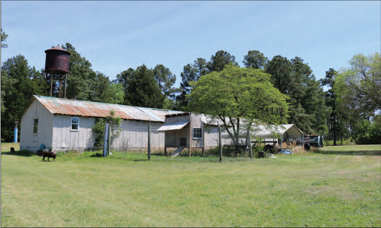
Figure 3.27. Packhouse, Looking Southeast.
