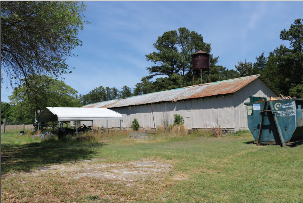
Figure 3.28. Packhouse, Looking Northeast.
