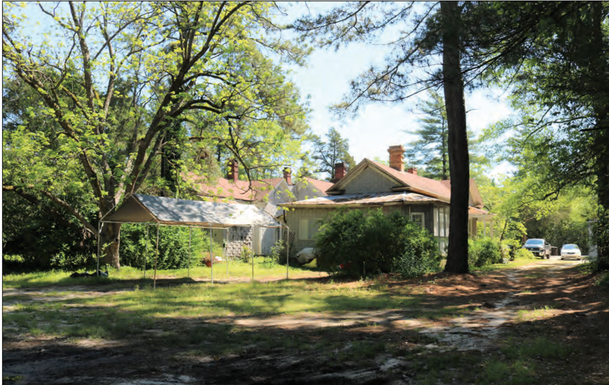
Figure 6.16. Hugh A. Keith House, Rear Elevation and Site, Looking Northeast.
