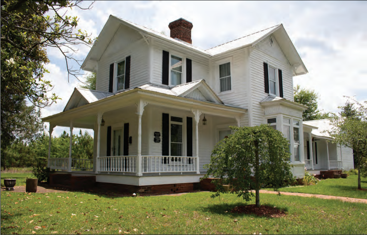
Figure 6.37. John Evander Phillips House (MR0599), Looking Southeast.
