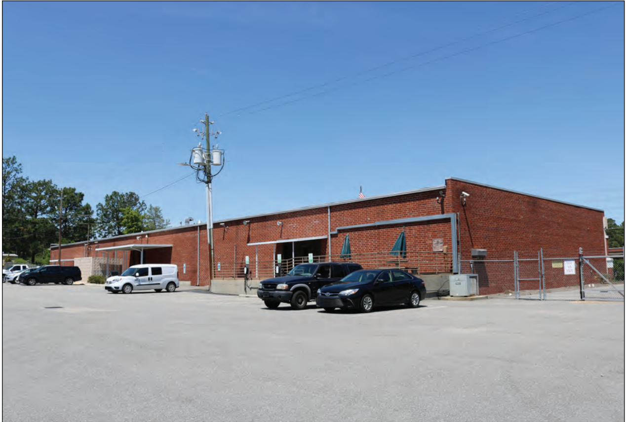
Figure 4.9. Amerotron Executive Office, East and South Elevations, Looking Northwest.
