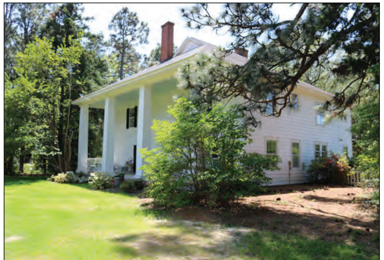
Figure 3.4. Chapin's Orchard, Façade and North Elevation, Looking Southwest.
