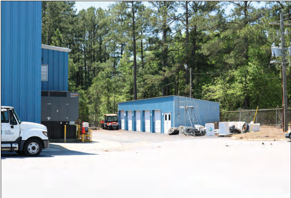
Figure 4.15. Garage, Looking Southwest.
