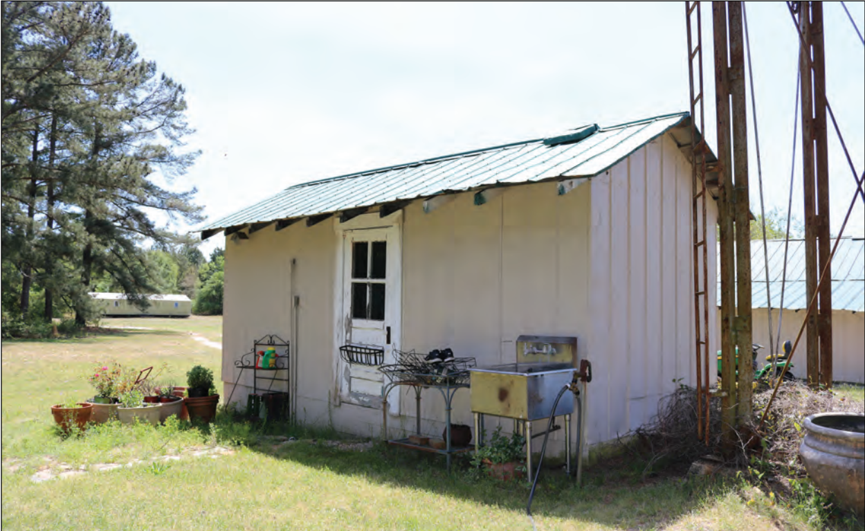
Figure 3.24. Pumphouse, Looking Southwest.
