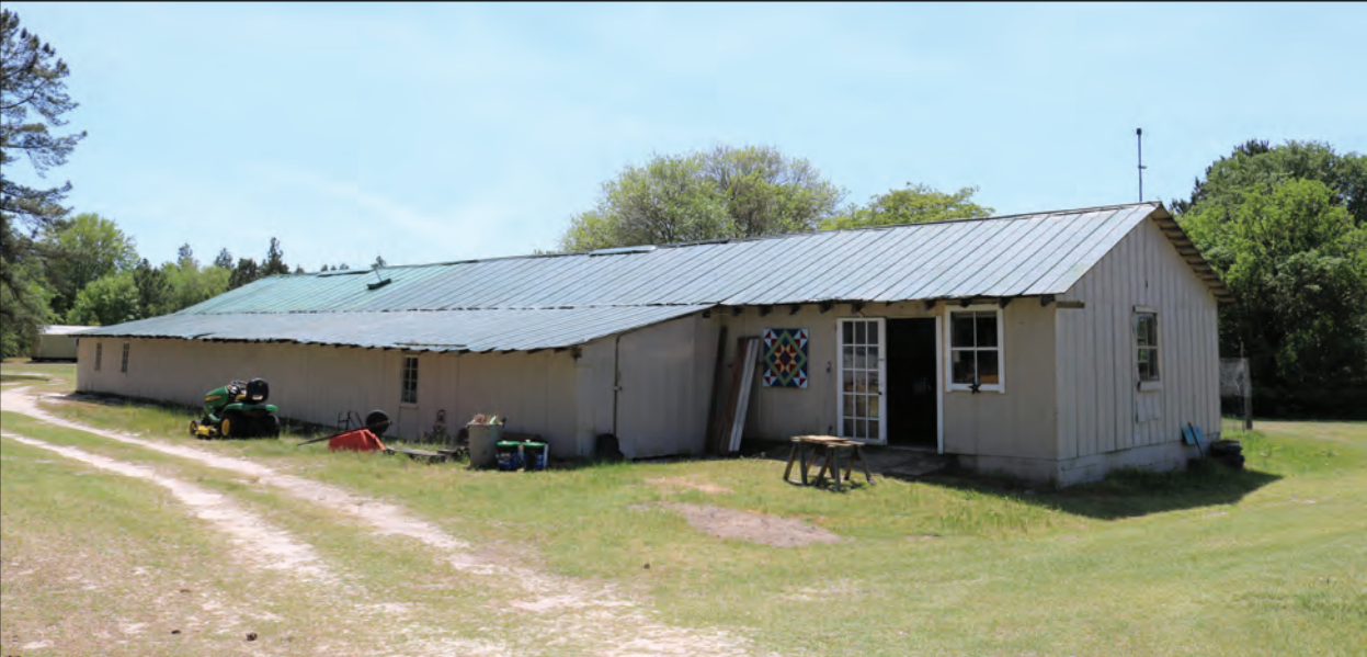
Figure 3.26. Packhouse, Looking Southwest.
