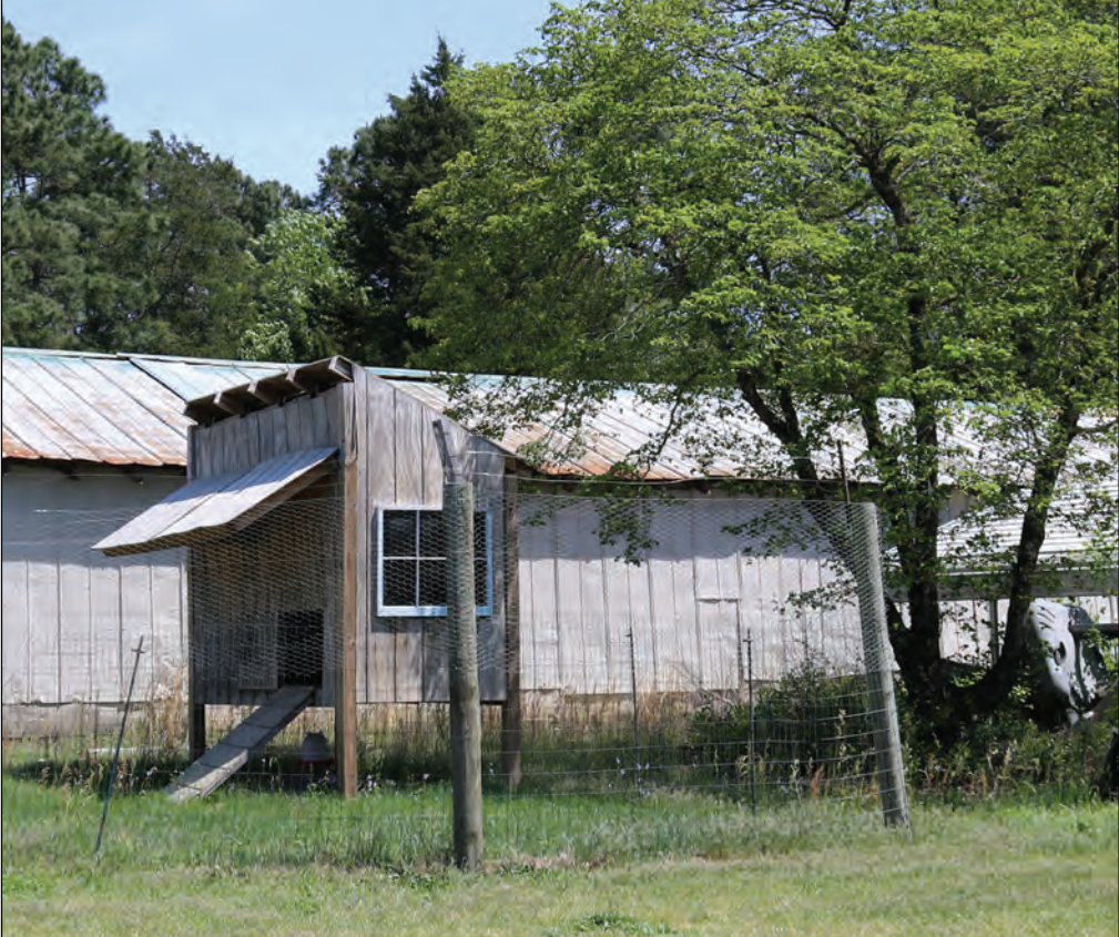
Figure 3.29. Chicken Coop, Looking Southeast.
