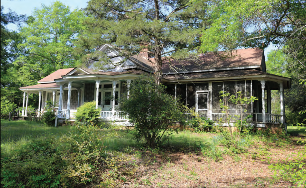
Figure 6.7. Hugh A. Keith House, Façade Looking West.
