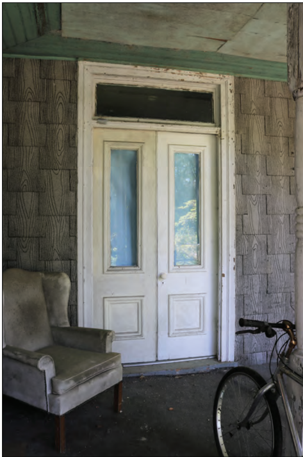
Figure 6.17. Hugh A. Keith House, Original Main Entrance on the Façade.
