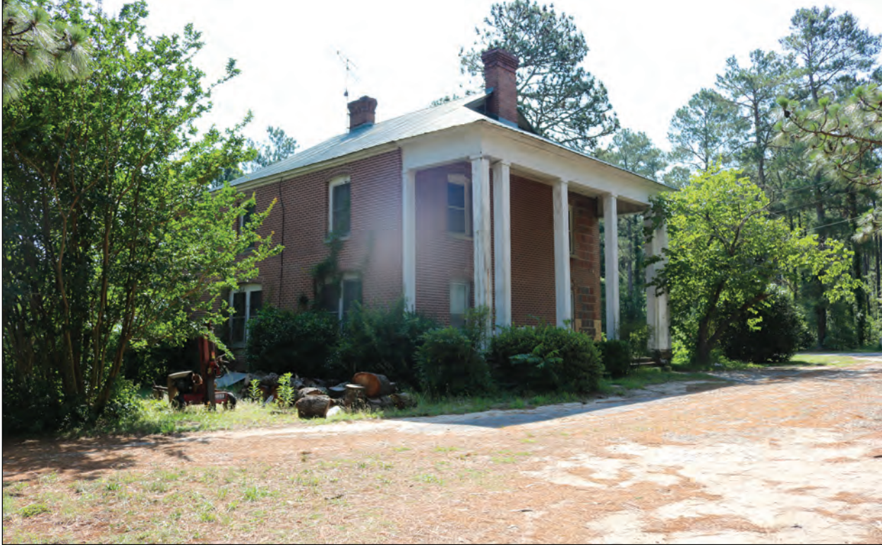
Figure 3.37. 1495 NC 211, Looking Northeast.
