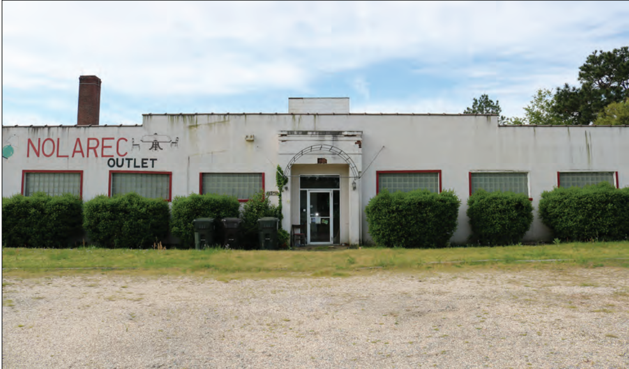
Figure 5.10. Aberdeen Hosiery Mills Co., Main Entrance, Looking South.
