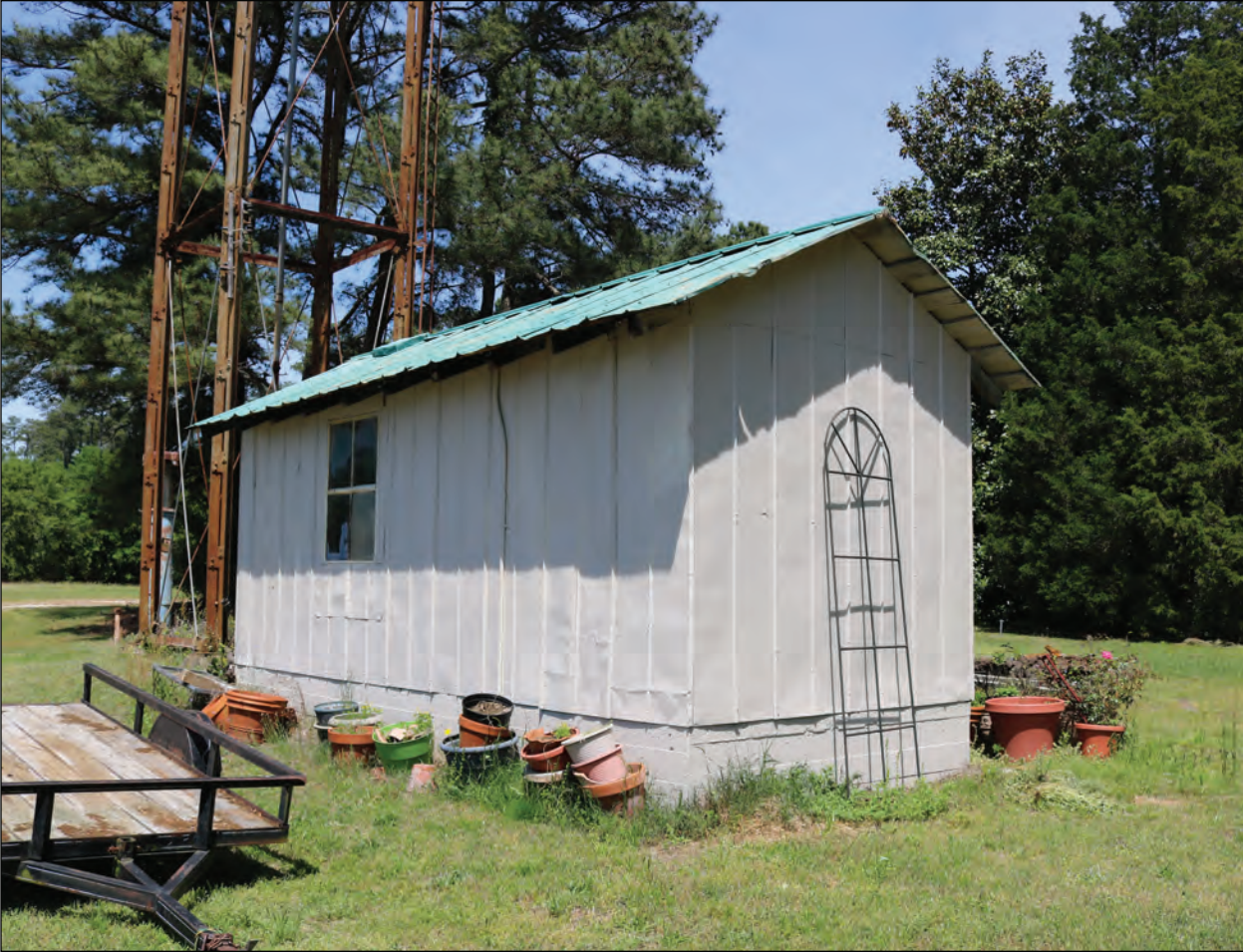
Figure 3.25. Pumphouse, Looking Northeast.
