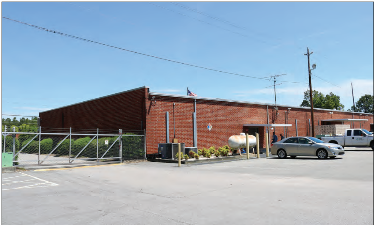
Figure 4.8. Amerotron Executive Office, West and South Elevations, Looking Northeast.
