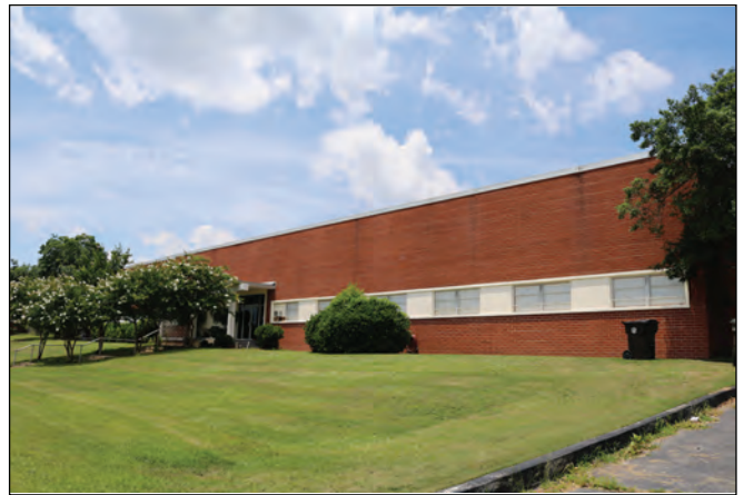
Figure 4.17. Gulistan Carpet Showroom, Looking Northeast.
