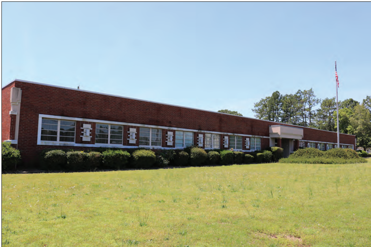
Figure 4.1. Amerotron Executive Office, Façade, Looking Southwest.
