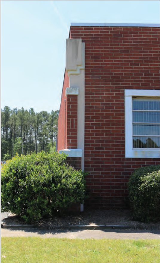
Figure 4.6. Amerotron Executive Office, Corner Detail, Looking South.
