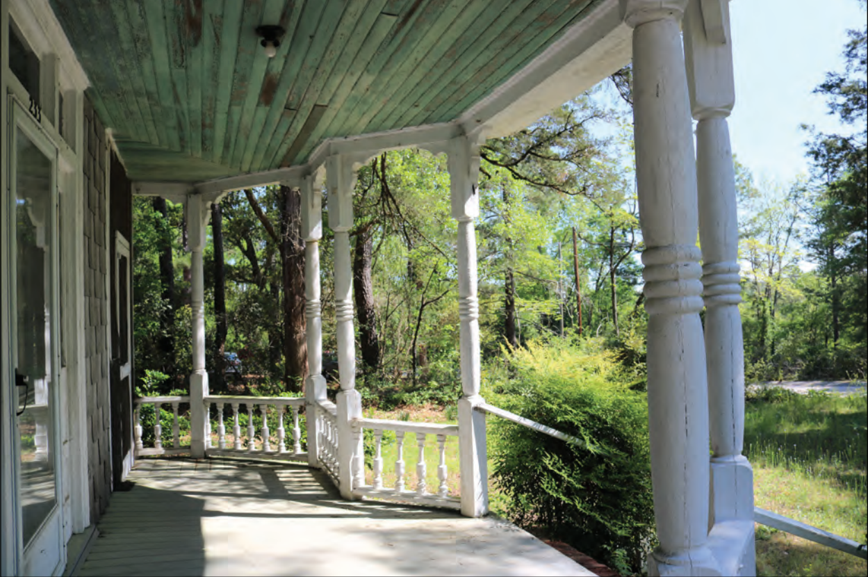
Figure 6.10. Hugh A. Keith House, Porch, Looking Northeast.
