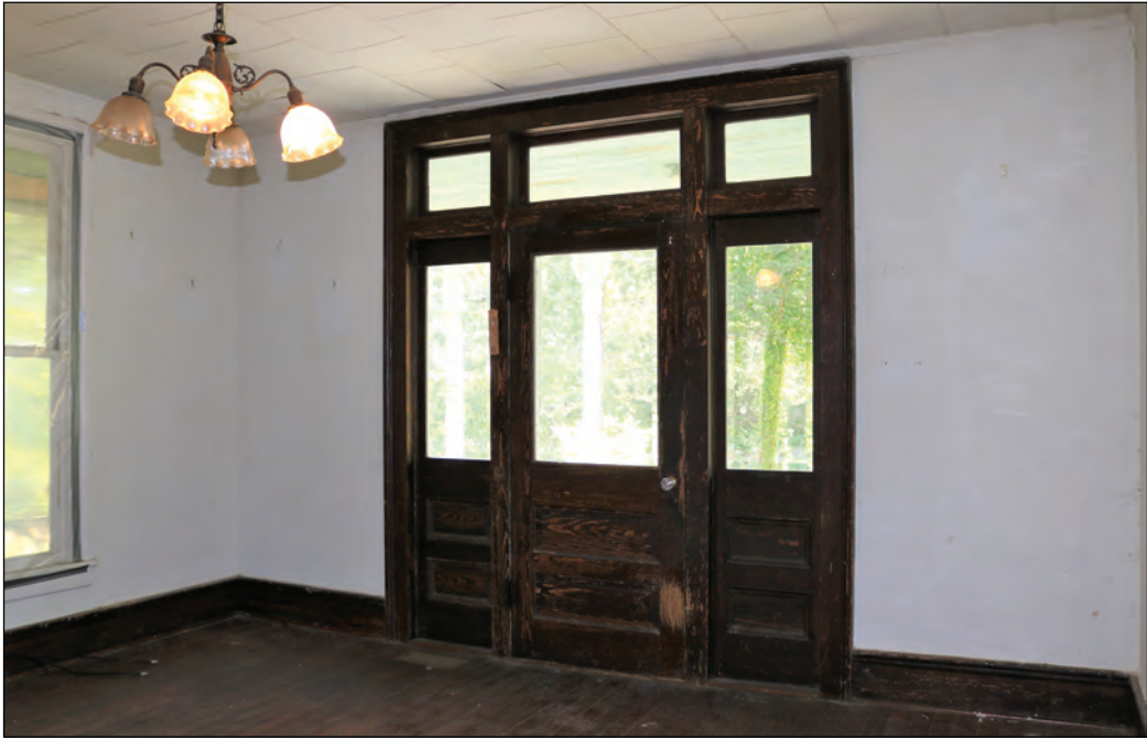
Figure 6.20. Hugh A. Keith House, Interior of the Main Entrance, Looking Southeast.
