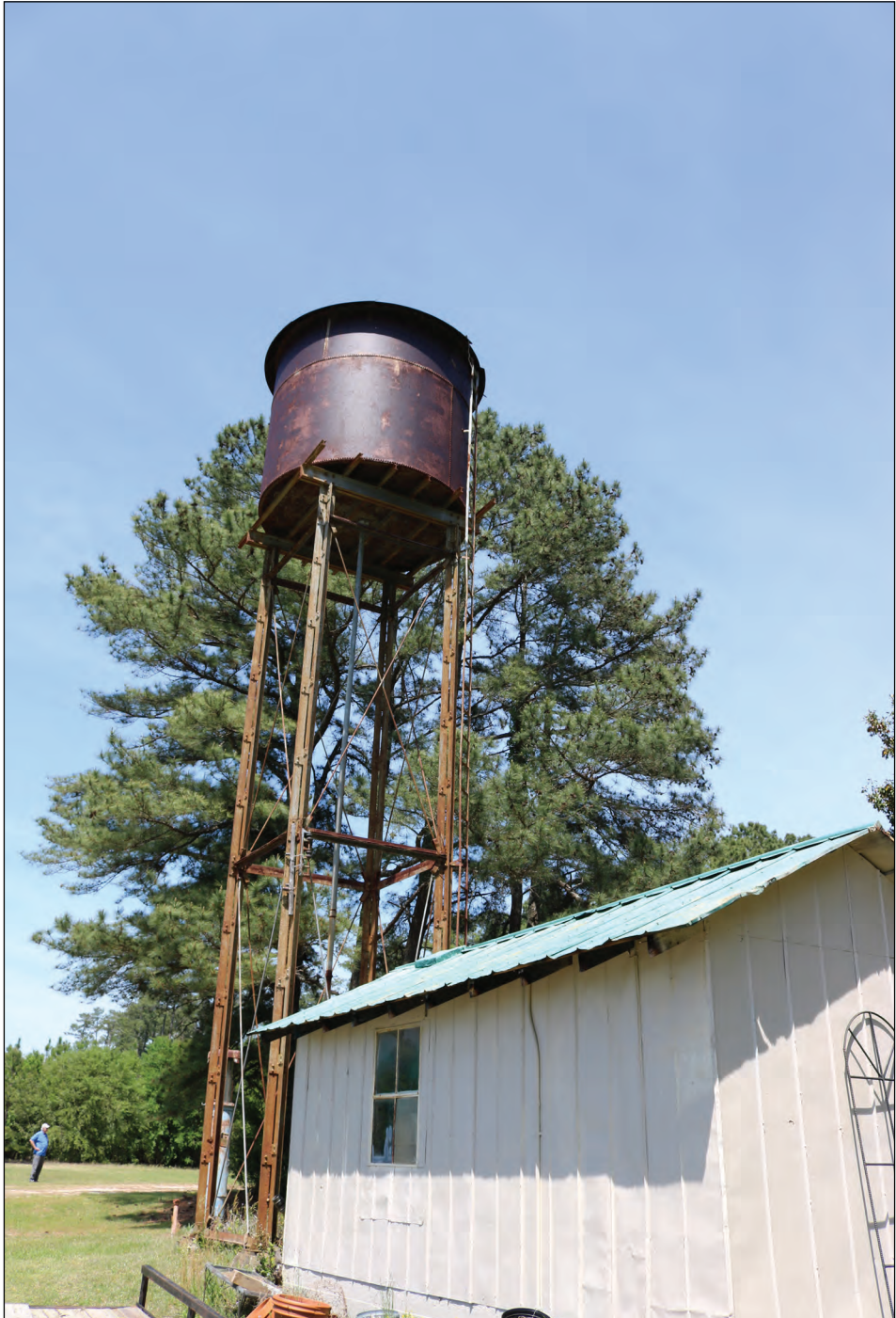
Figure 3.22. Water Tower, Looking Northeast.
