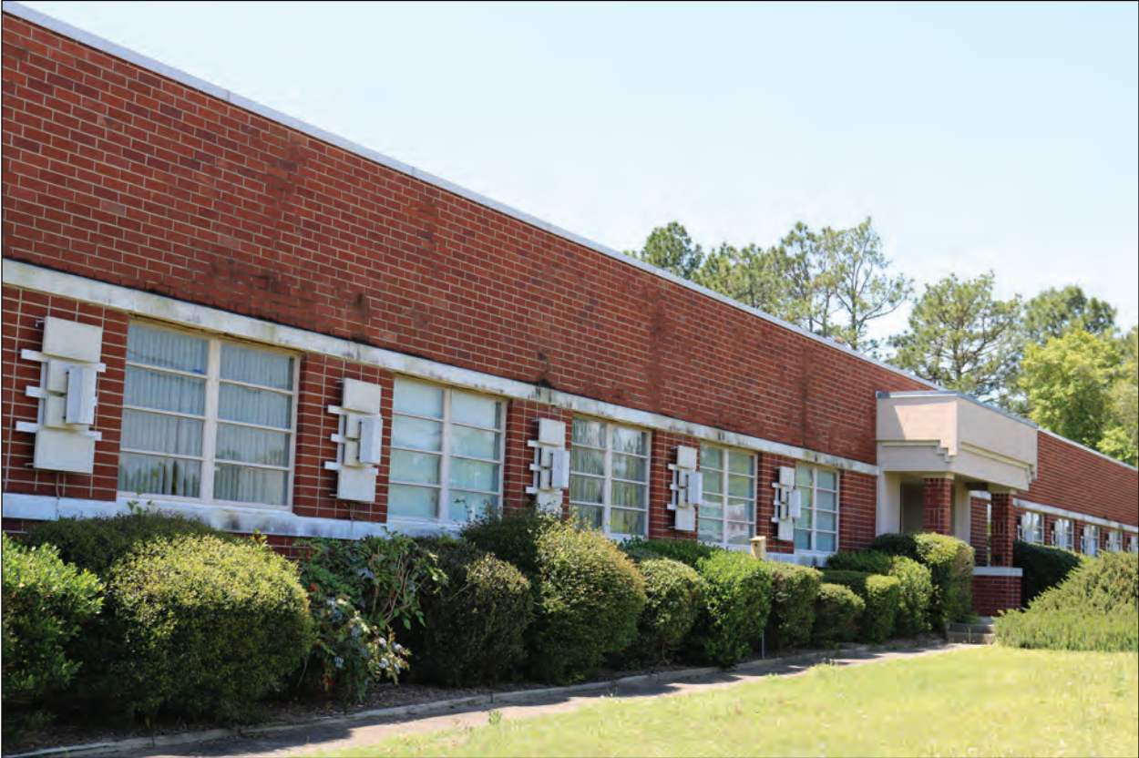
Figure 4.4. Amerotron Executive Office, Window and Entry Detail, Looking Southwest.
