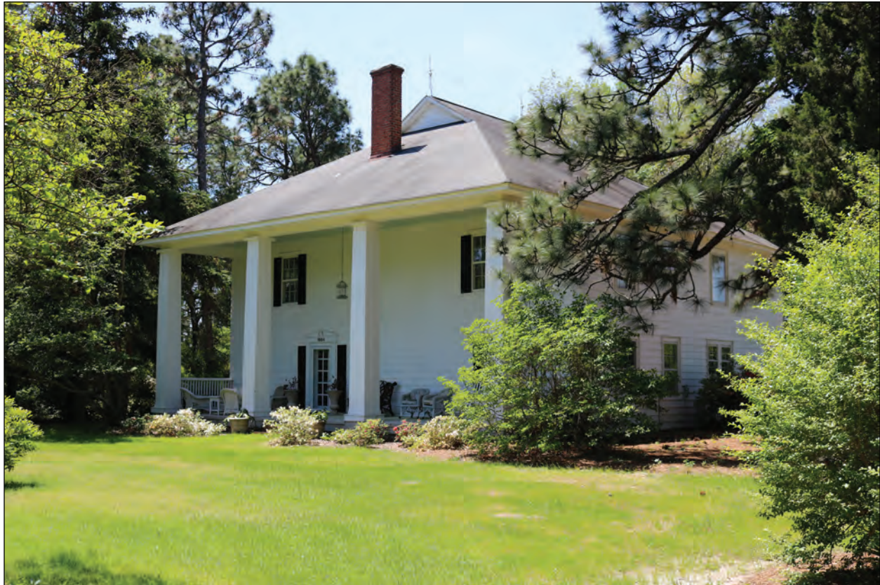
Figure 3.1. Chapin’s Orchard, Façade and North Elevation, Looking Southwest.
