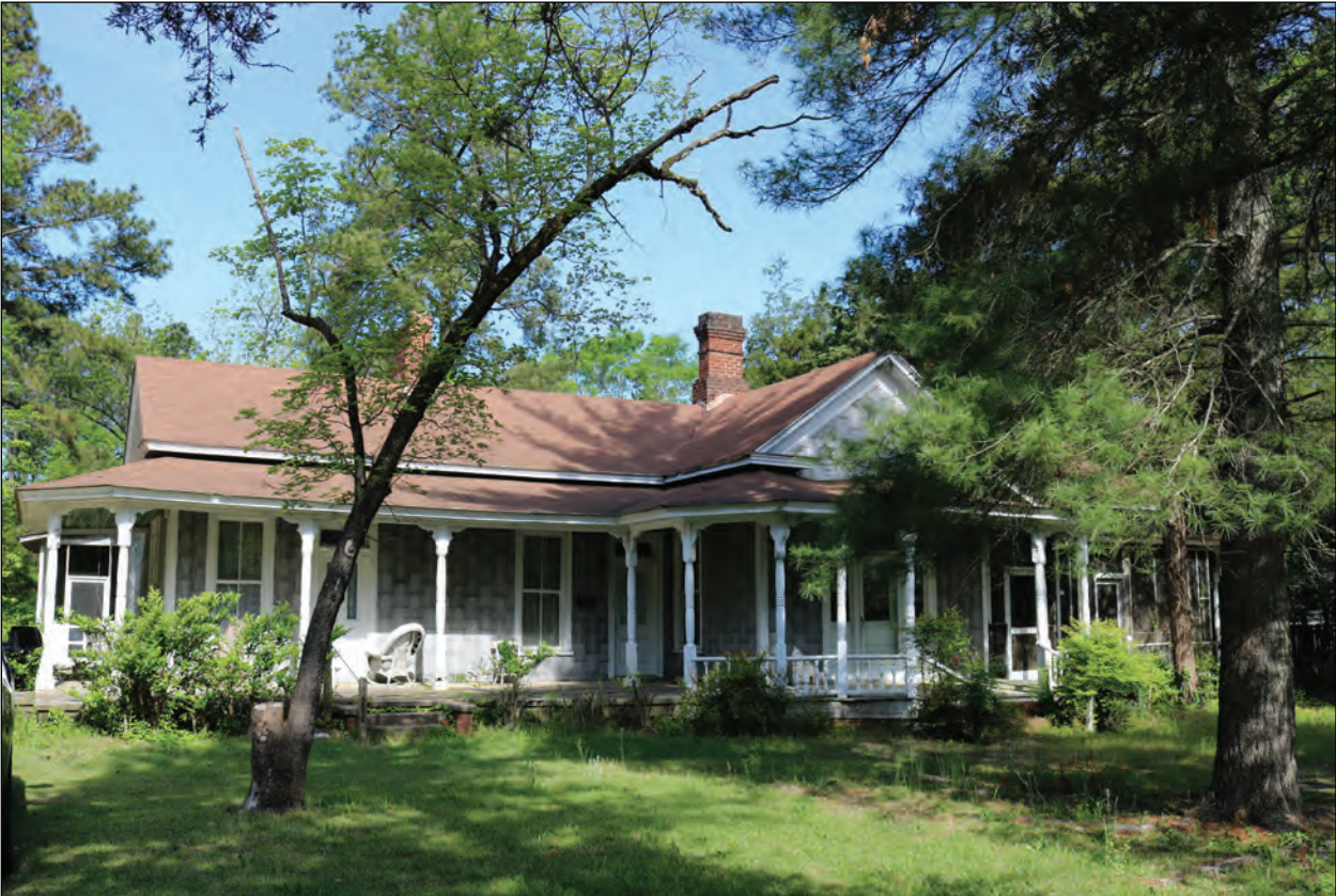
Figure 6.8. Hugh A. Keith House, Façade, Looking Northwest.
