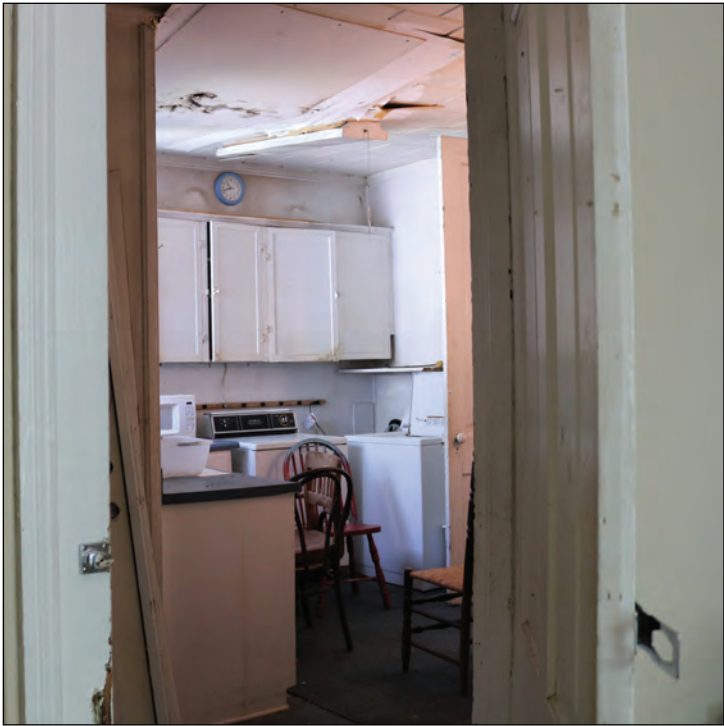
Figure 6.28. Hugh A. Keith House, Added Kitchen.
