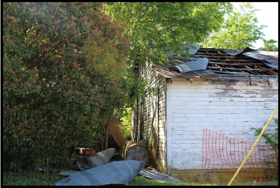
Figure 11: Wood's Store, Looking Southeast.
