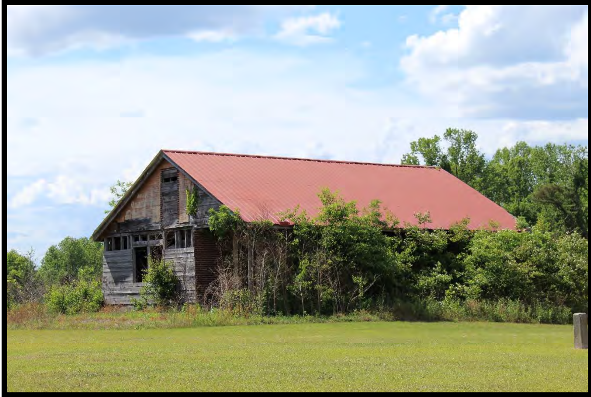
Figure 20: Store (CD1441), Looking Southeast.
