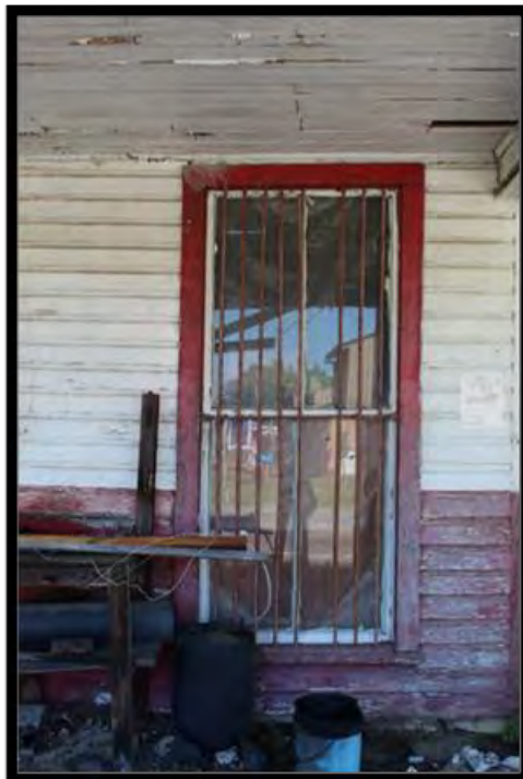
Figure 8: Wood's Store, Detail of Window, Looking North.
