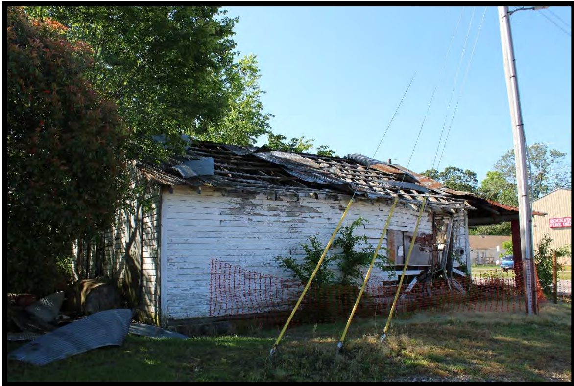
Figure 12: Wood's Store, Looking Southeast.
