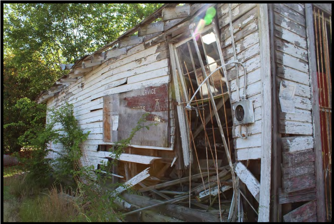
Figure 10: Wood's Store, Looking East.
