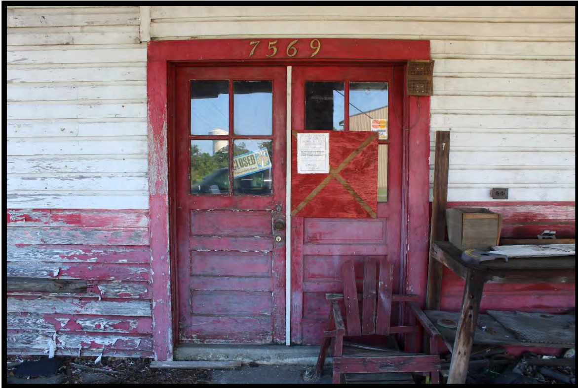
Figure 7: Wood's Store, Detail of Double-Leaf Door, Looking North.
