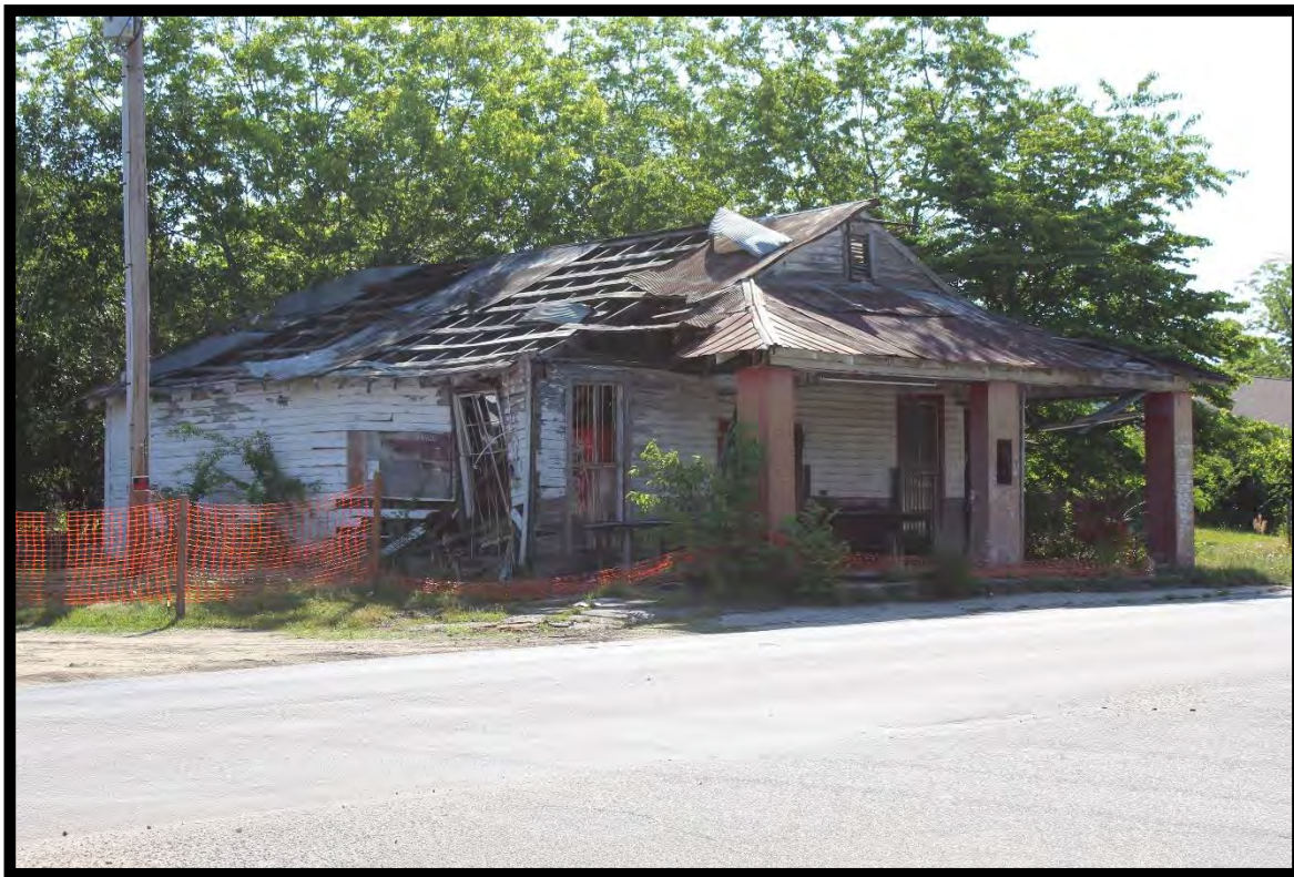
Figure 5: Wood's Store, Looking Southeast.
