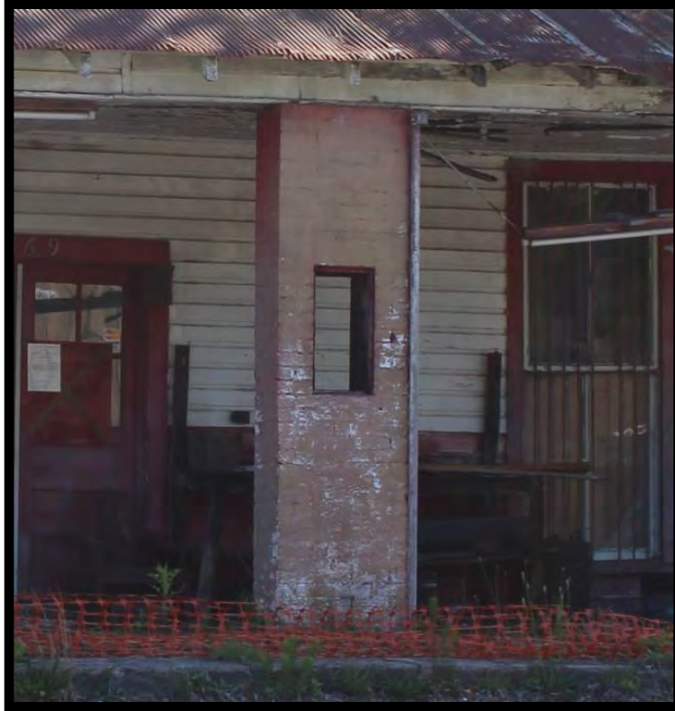
Figure 6: Wood's Store Brick Pier Opening and Pipe, Looking North.
