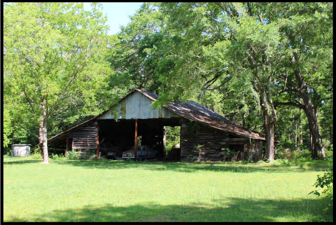
Figure 13: Carmichael-Lindsay House, Barn, Looking Northwest.
