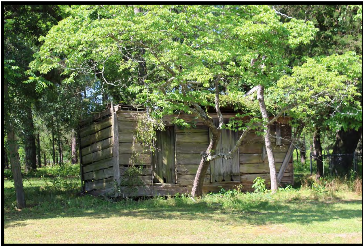
Figure 10: Carmichael-Lindsay House, Side-Gabled Structure, Looking Southwest.
