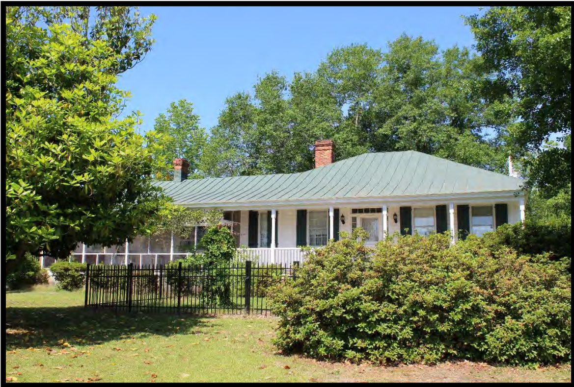
Figure 3: Carmichael-Lindsay House, Looking Northwest.
