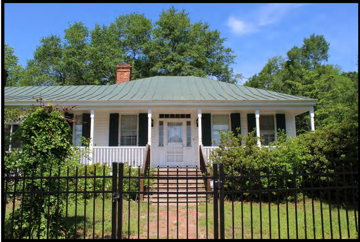
Figure 7: Carmichael-Lindsay House, Looking Northwest.
