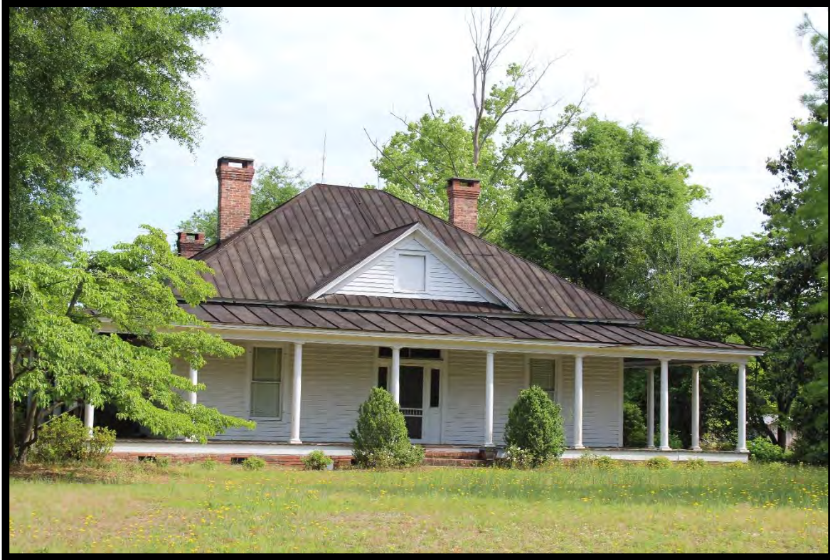
Figure 22: James L. Cooley House (SC0039), Looking Northeast.
