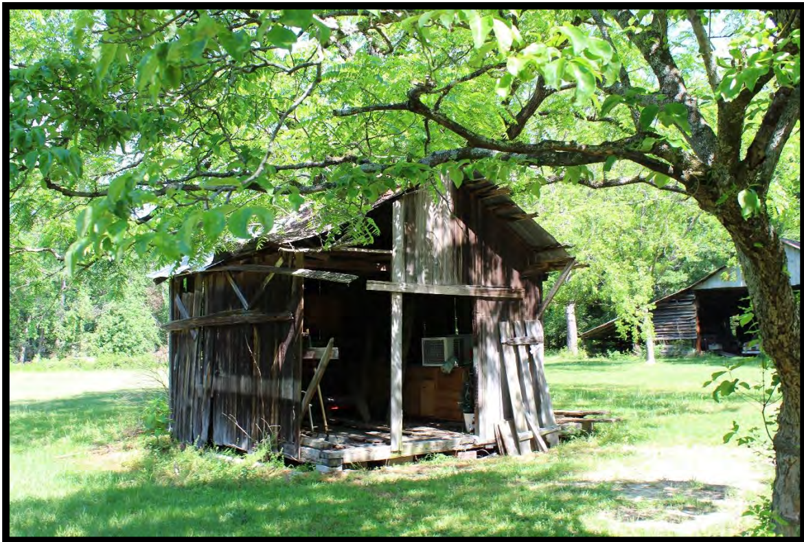
Figure 12: Carmichael-Lindsay House, Front-Gabled Structure, Looking Northwest.
