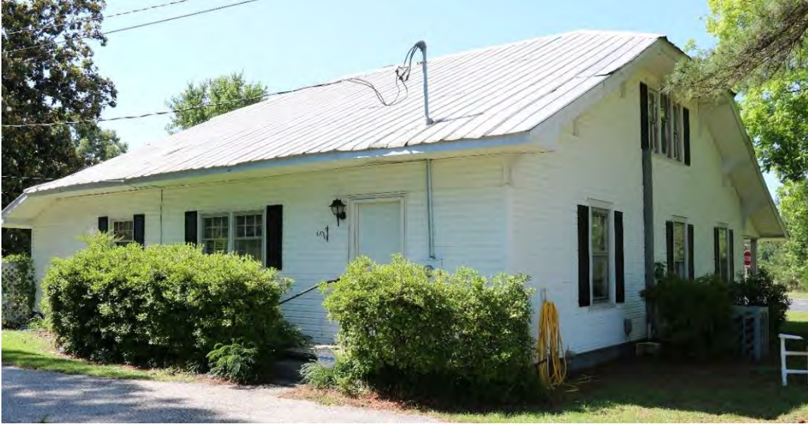
Figure 9. 1928 house, rear (north) and side (west) elevations, view facing southeast.
