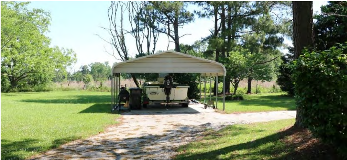
Figure 10. C.1990 carport, view facing north.
