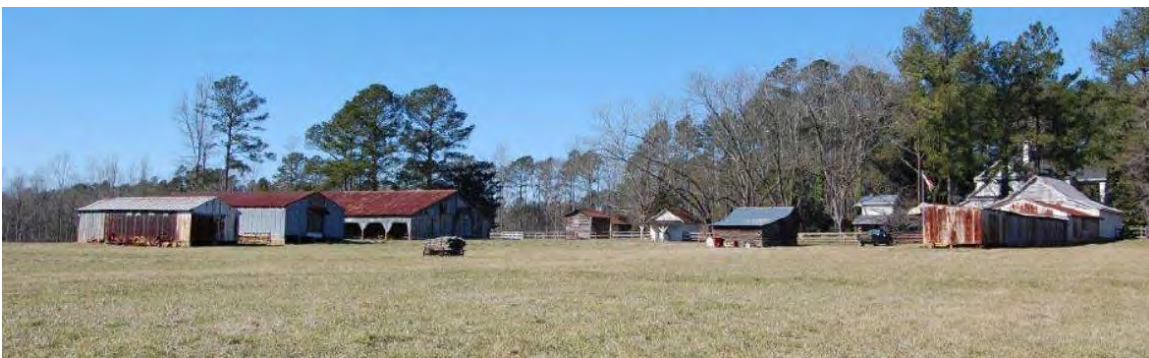
Figure 26. View of the Johnson Farm, showing the cohesive collection of outbuildings. 31
