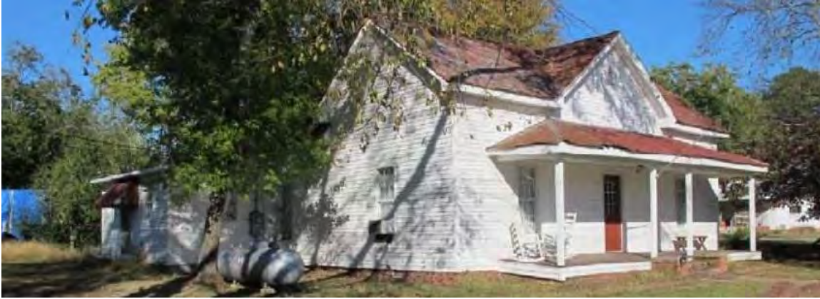
Figure 42. House at 8733 US 401 North (HT0174) with intact front porch. 43
