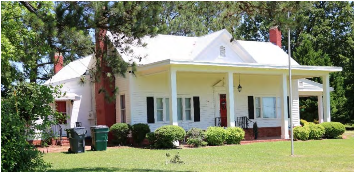
Figure 30. 1920 farmhouse at the Ted L. Penny Farm. South-facing facade and side (west) elevation, view facing northeast.
