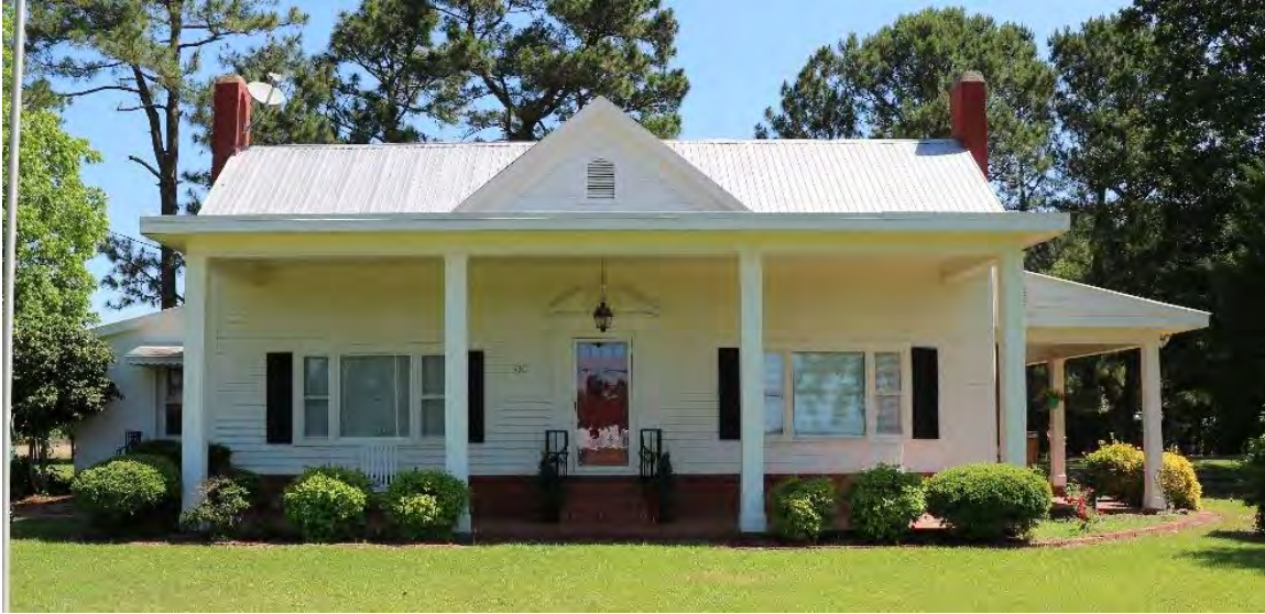
Figure 32. Facade, with Southern Colonial details added c.1950, including addition of a larger covered patio, door pediment, and fenestration replacements.
