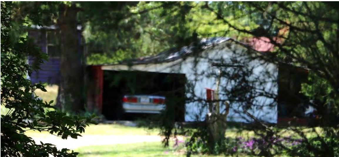
Figure 23. C.1930 Shed A, view facing south/southeast.
