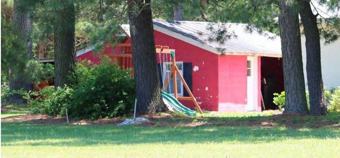
Figure 34. C.1955 garage, facade (south) and side (west) elevation, view facing northeast.
