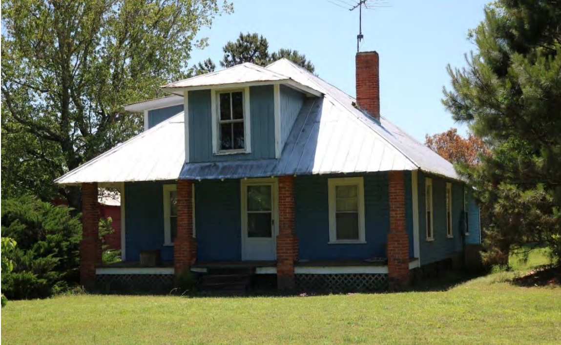
Figure 18. 1915 house, facade and side (west) elevation, view facing southeast.
