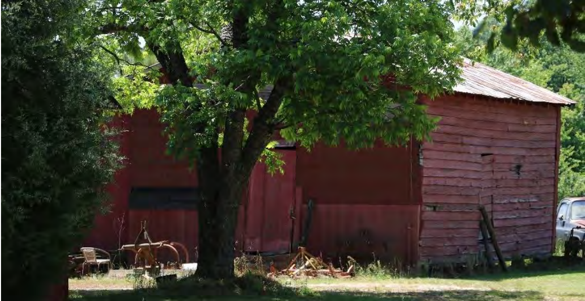
Figure 22. C.1915 large frame shed, view facing south/southeast.
