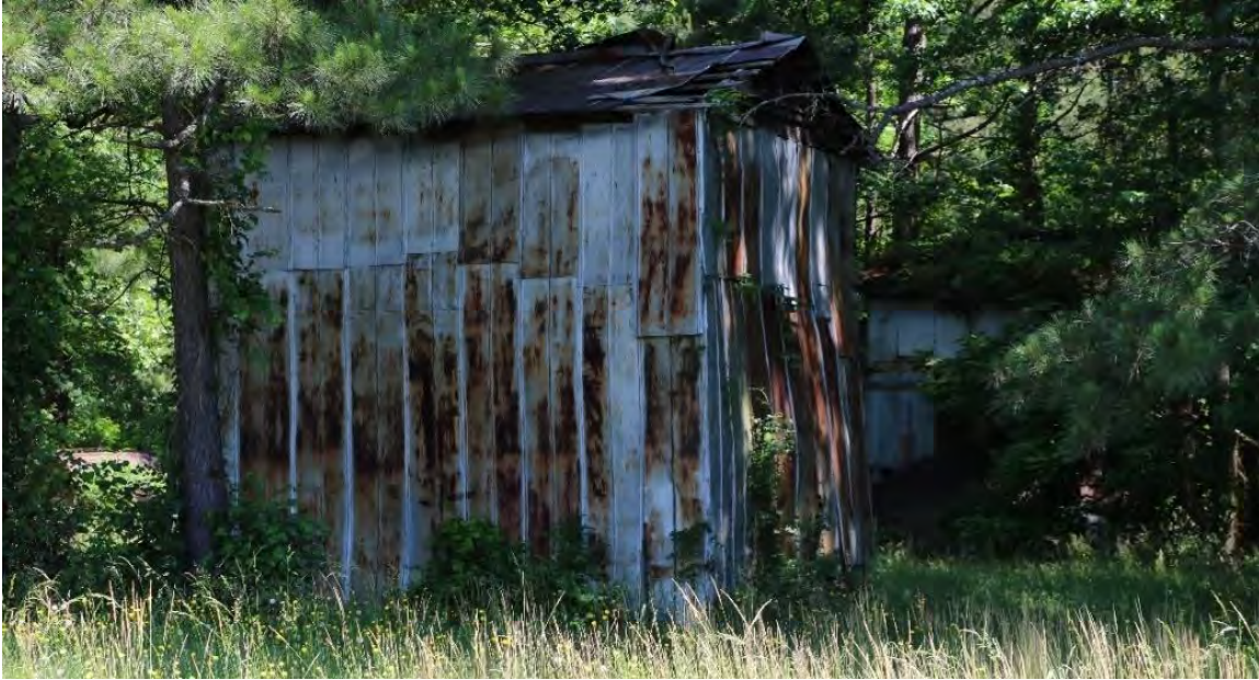
Figure 36. Two c.1920 frame sheds (Shed B at left and Shed C at right), view facing north.
