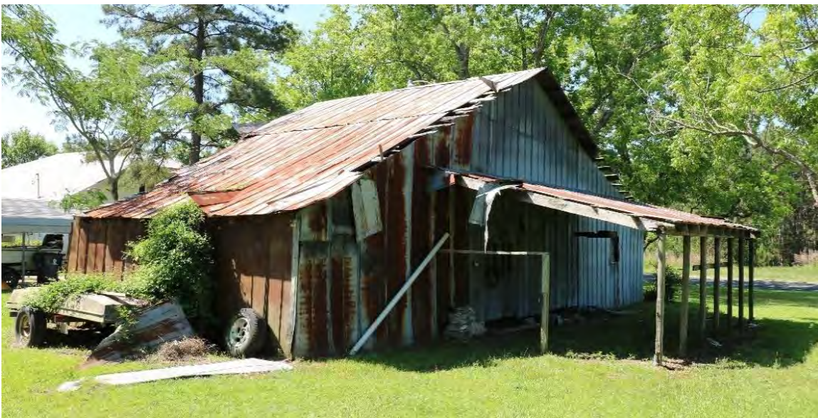
Figure 12. C.1930 barn, side (north) and rear (west) elevations, view facing southeast.
