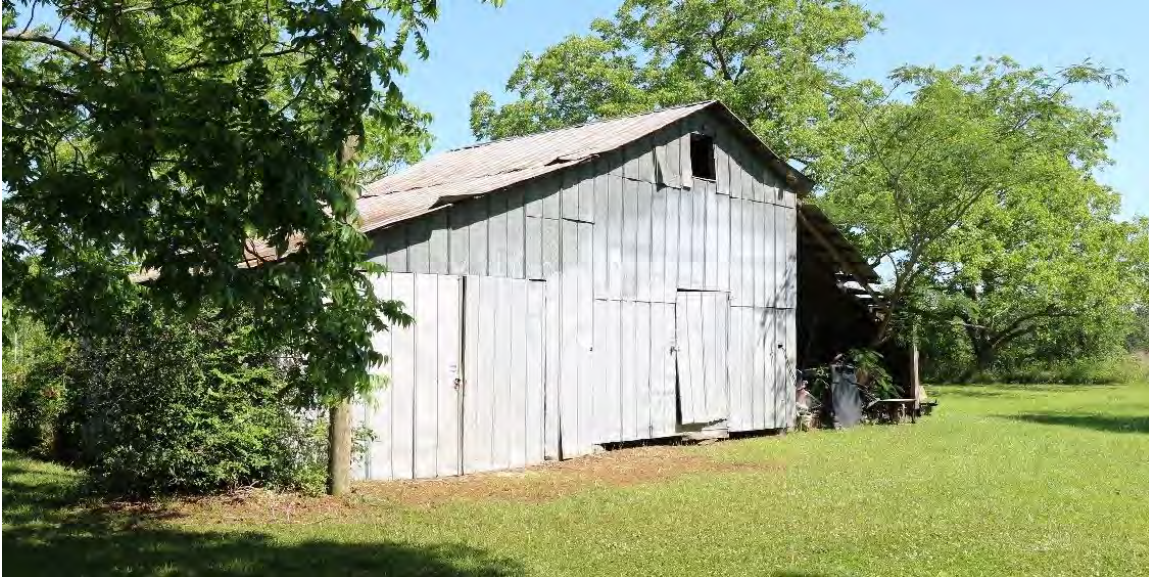
Figure 11. c.1930 barn, east facade, view facing north/northwest.
