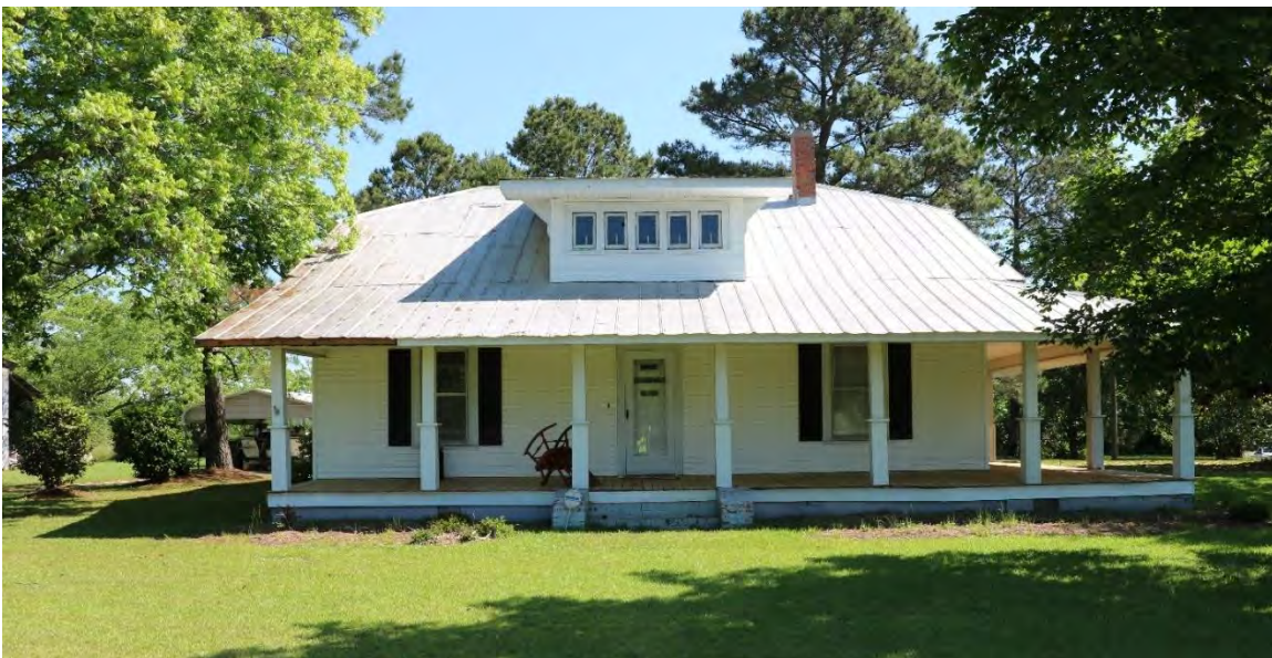
Figure 6. 1928 house at 270 Sheriff Johnson Road. South-facing facade, view facing north.
