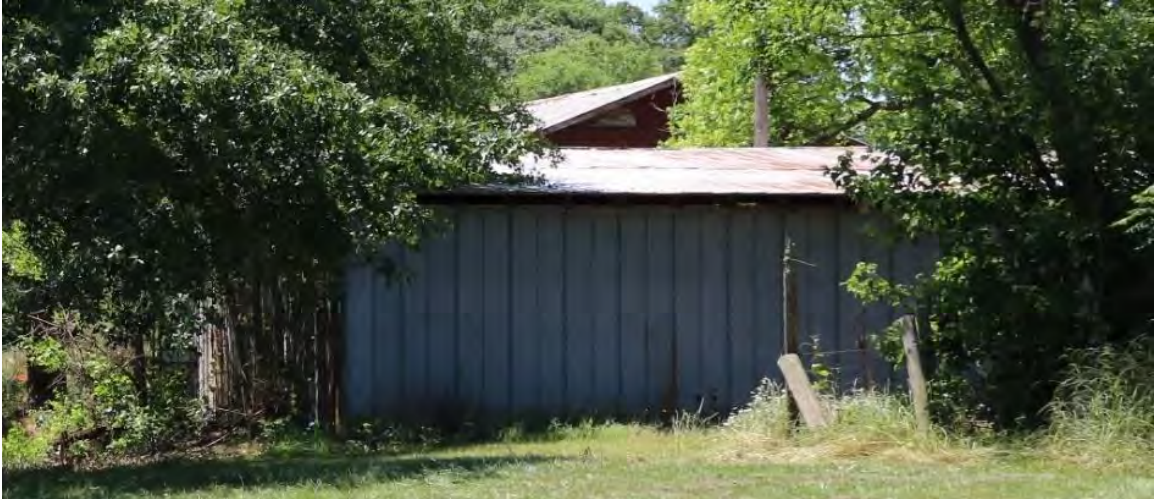
Figure 20. C.1915 vehicle storage shed, view facing south.
