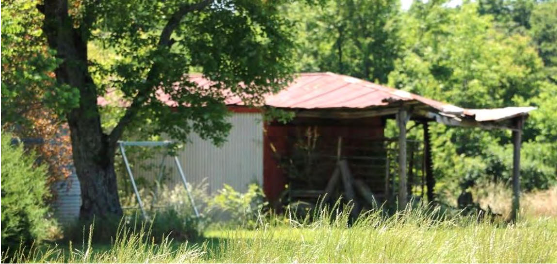
Figure 24. C.1930 Shed B, view facing south/southeast.
