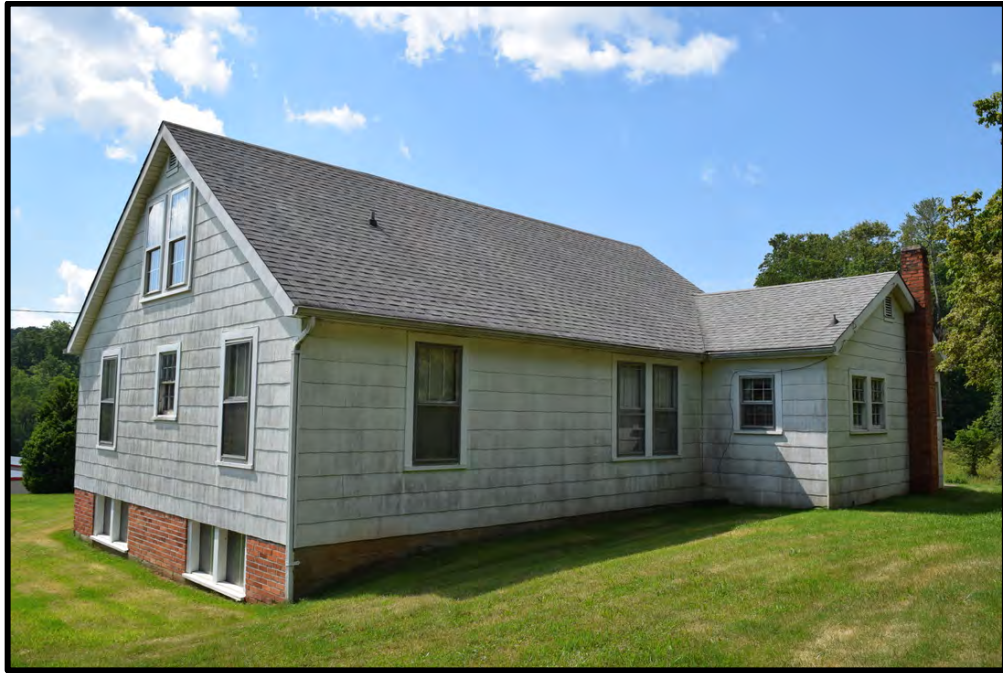
Cox House northwest corner, view to the southeast
