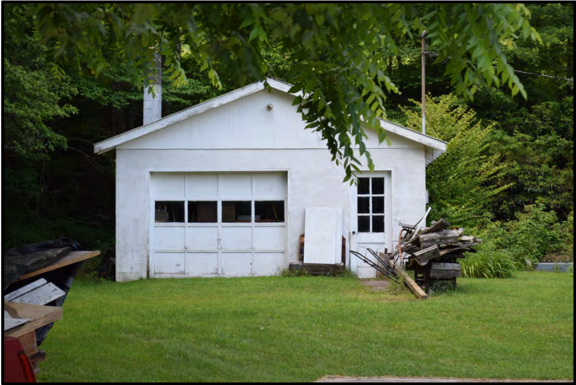
Garage, view to the southwest
