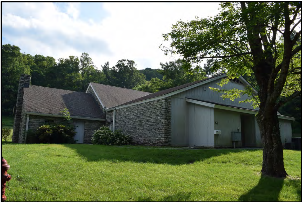
Rear elevation, view to the south-southwest
