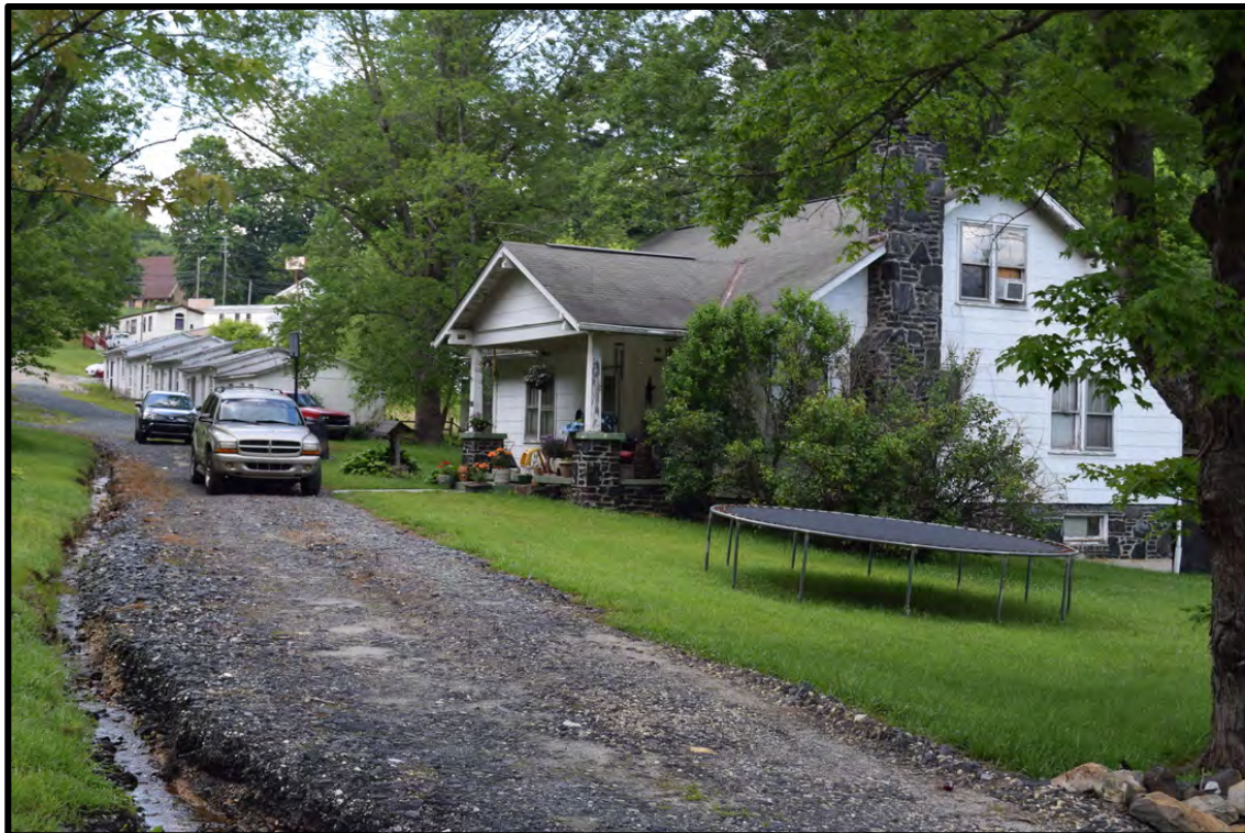
Daisy and Pete Ellis House with motor cabins in the background, view to the north
