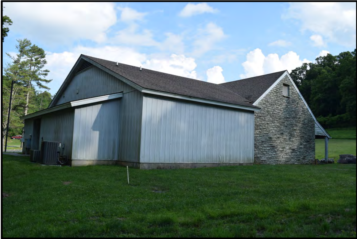
Rear corner of 2001 ell, northwest corner, view to the southeast
