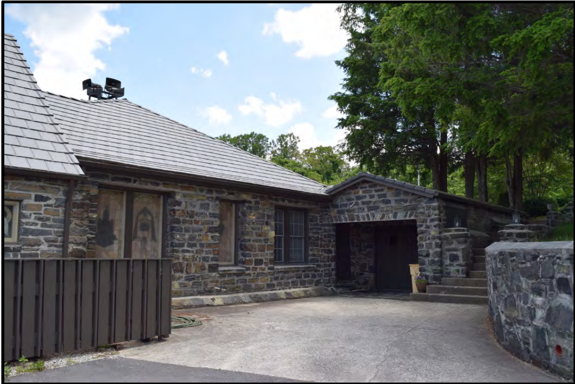
Southwest (rear) corner of the church, view to the northeast
