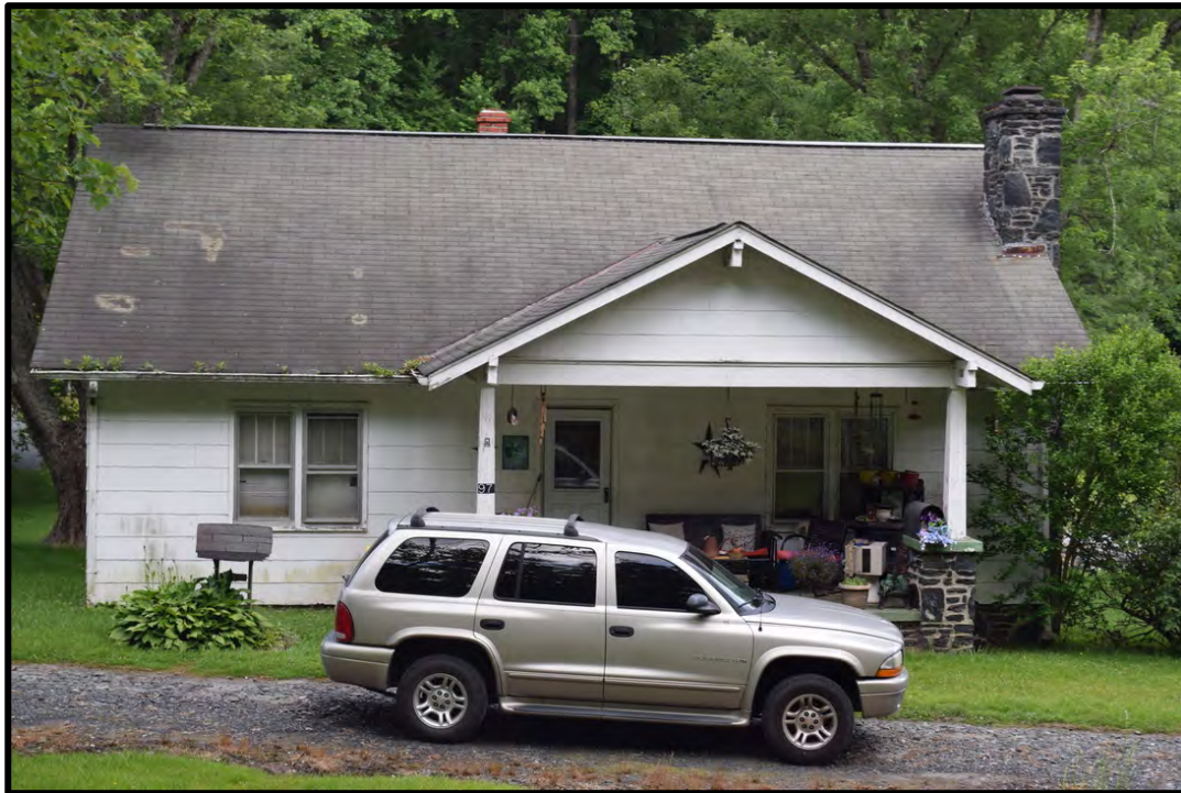
Ellis House facade, view to the east
