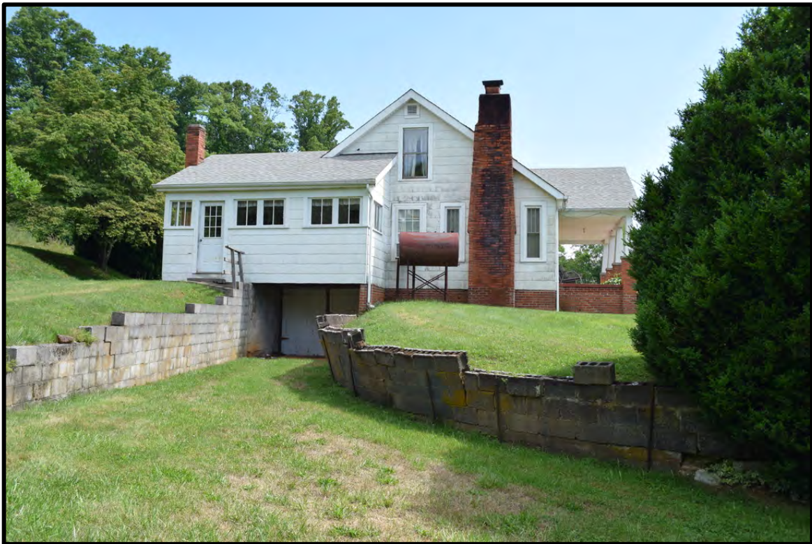
Cox House south elevation, view to the north
