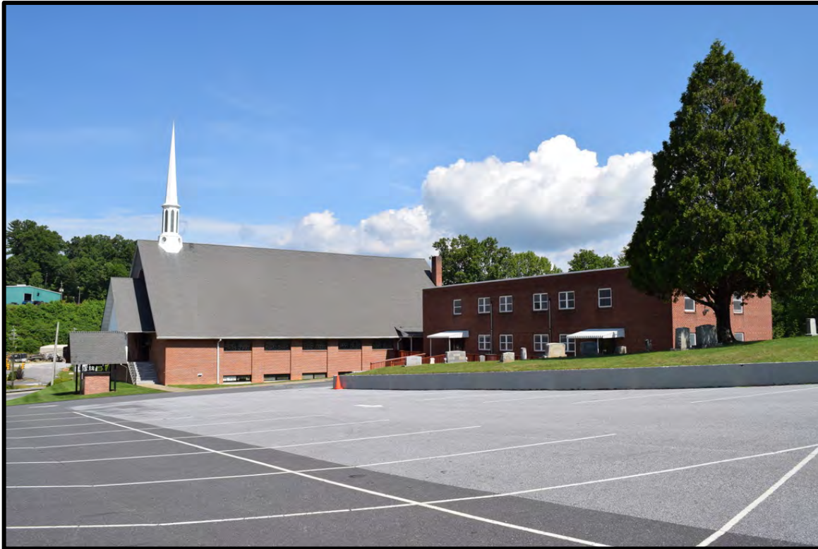
Church (1966) and education building (1957), view to the northwest
