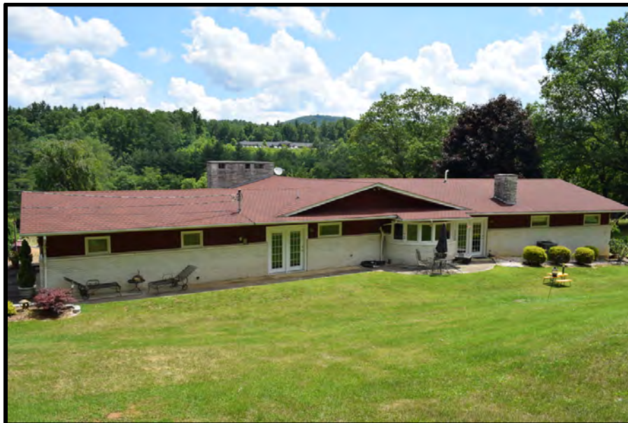
Phillips House rear elevation, view to the east
