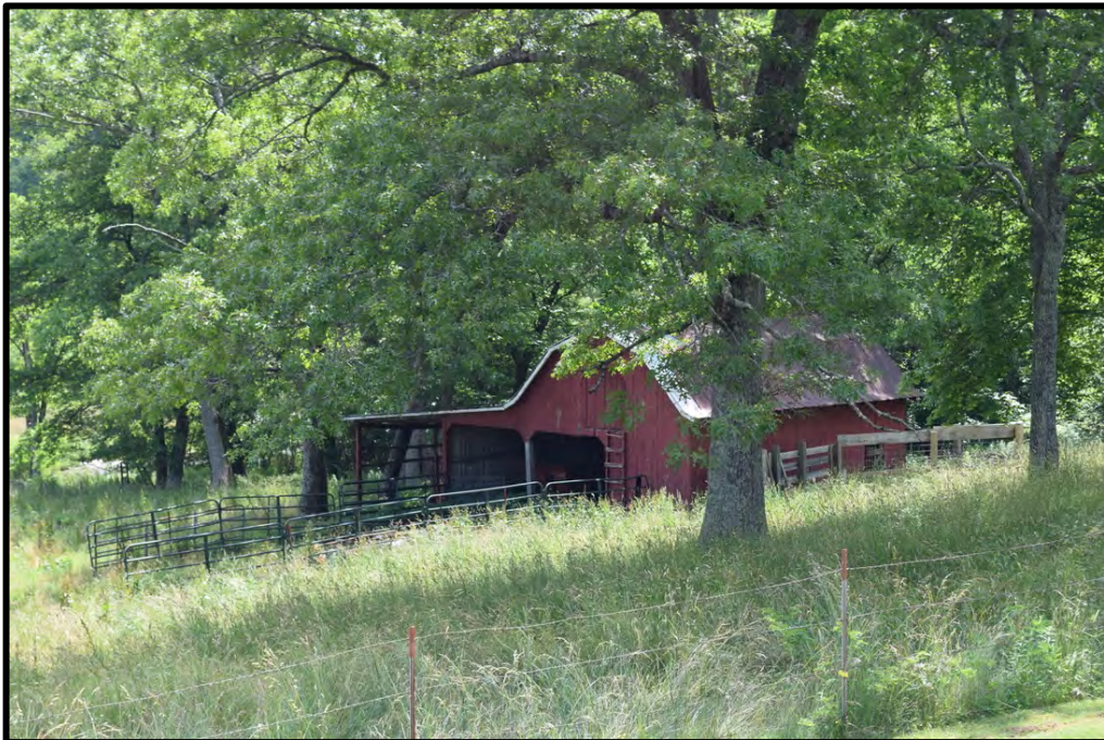
1970s barn southeast of the house, view to the southeast
