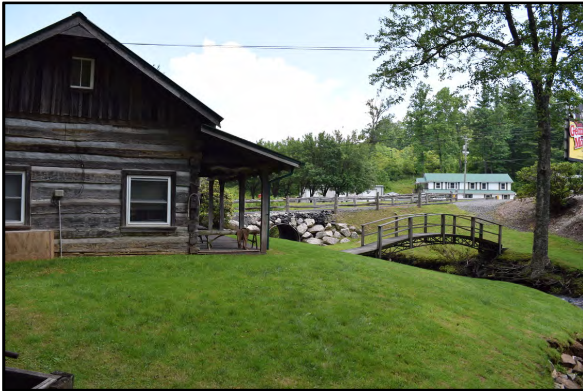
South elevation of house and foot bridge, view to the north
