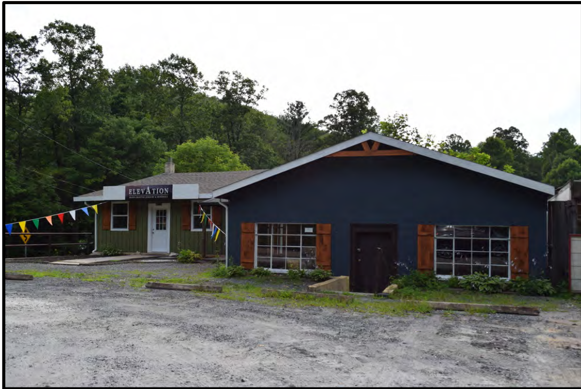
1954 Bea Hensley Forge in foreground with 1972 addition to the left, view to the west
