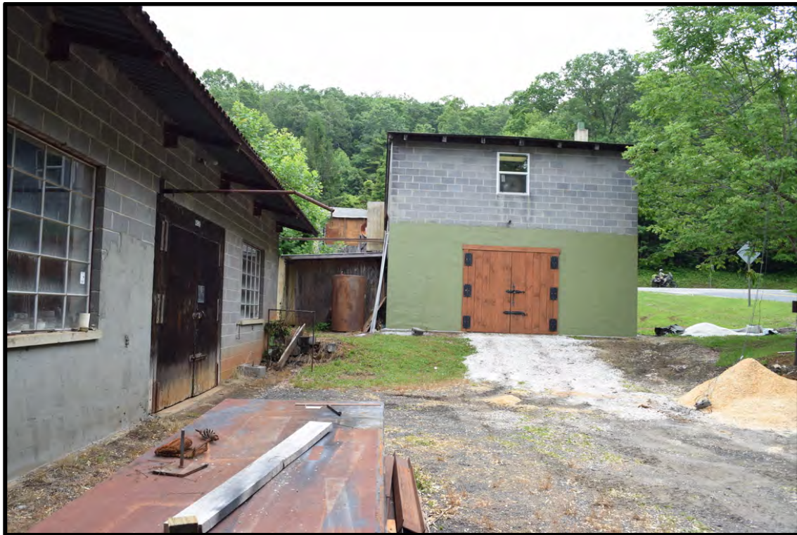
Rear of the 1972 building and front of 1969 forge (on the left), view to the east
