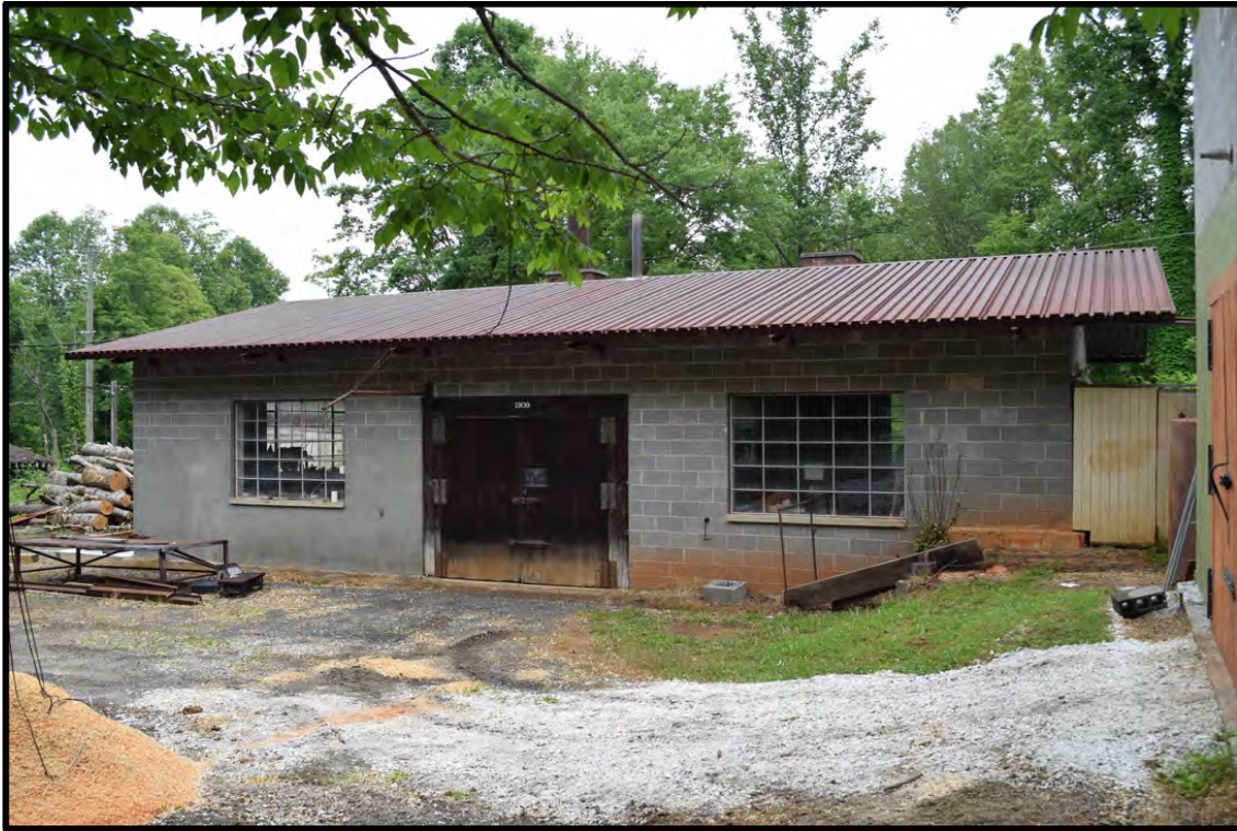
1969 forge, view to the north
