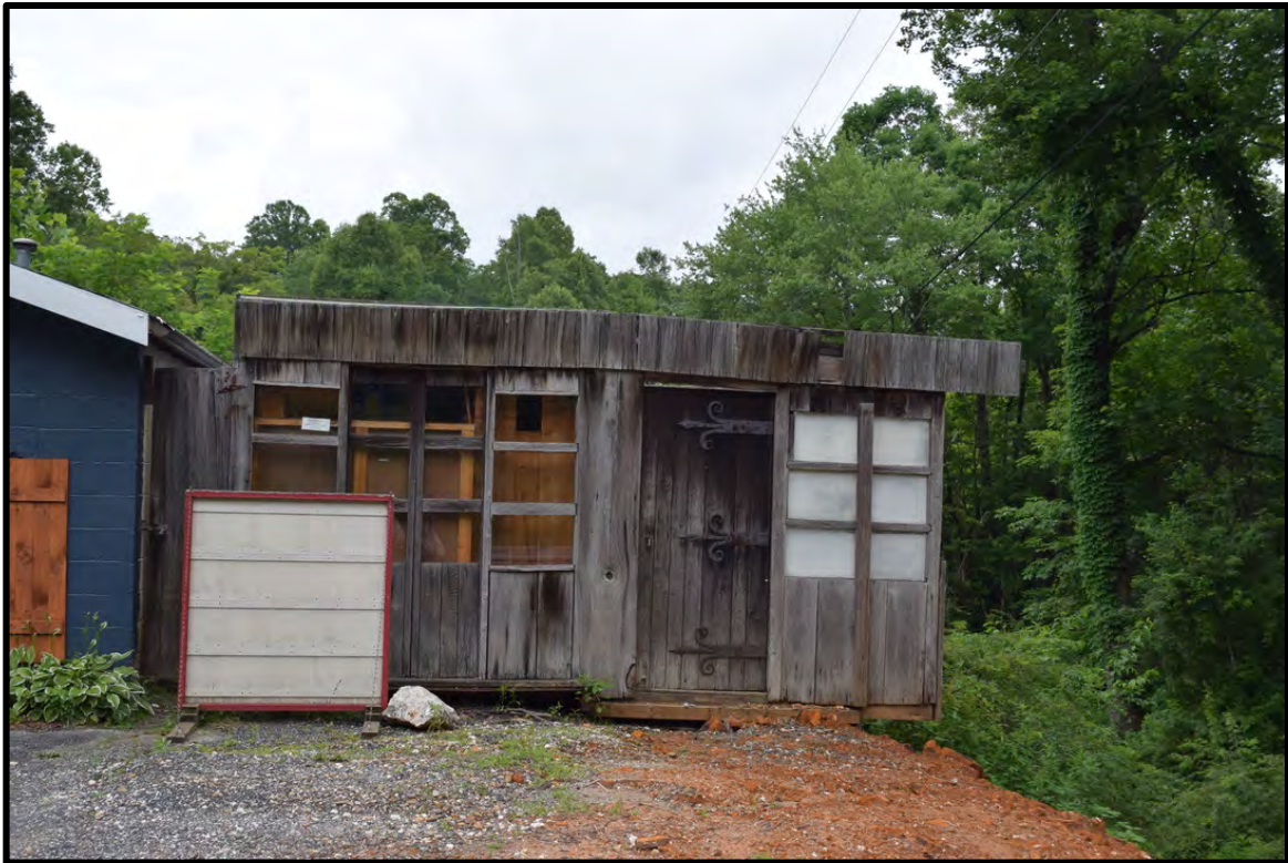
Temporary addition on north side of forge, view to the west (to be removed in 2019)
