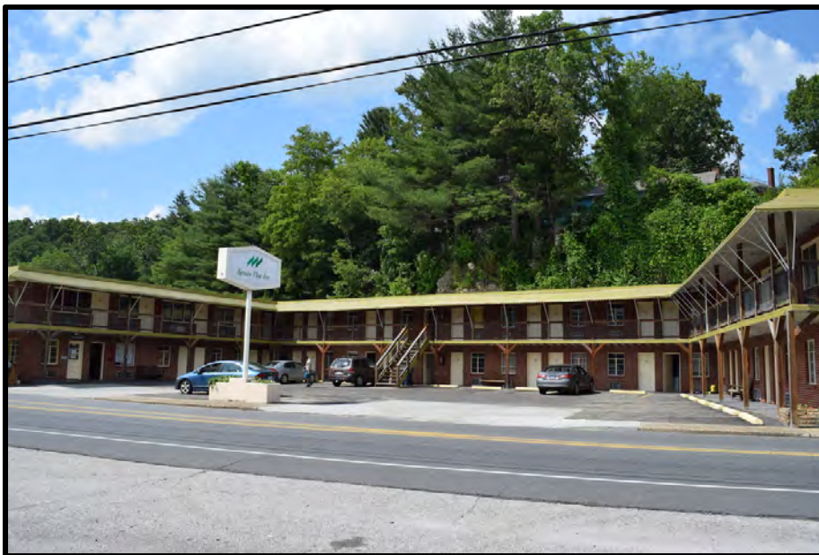
Original Baker Motel (1956) on Oak Street, view to the north
