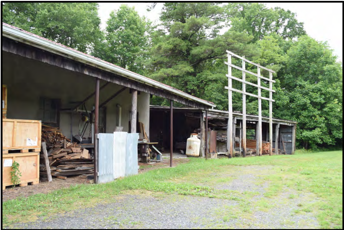
West side of shop and saw mill, view to the south
