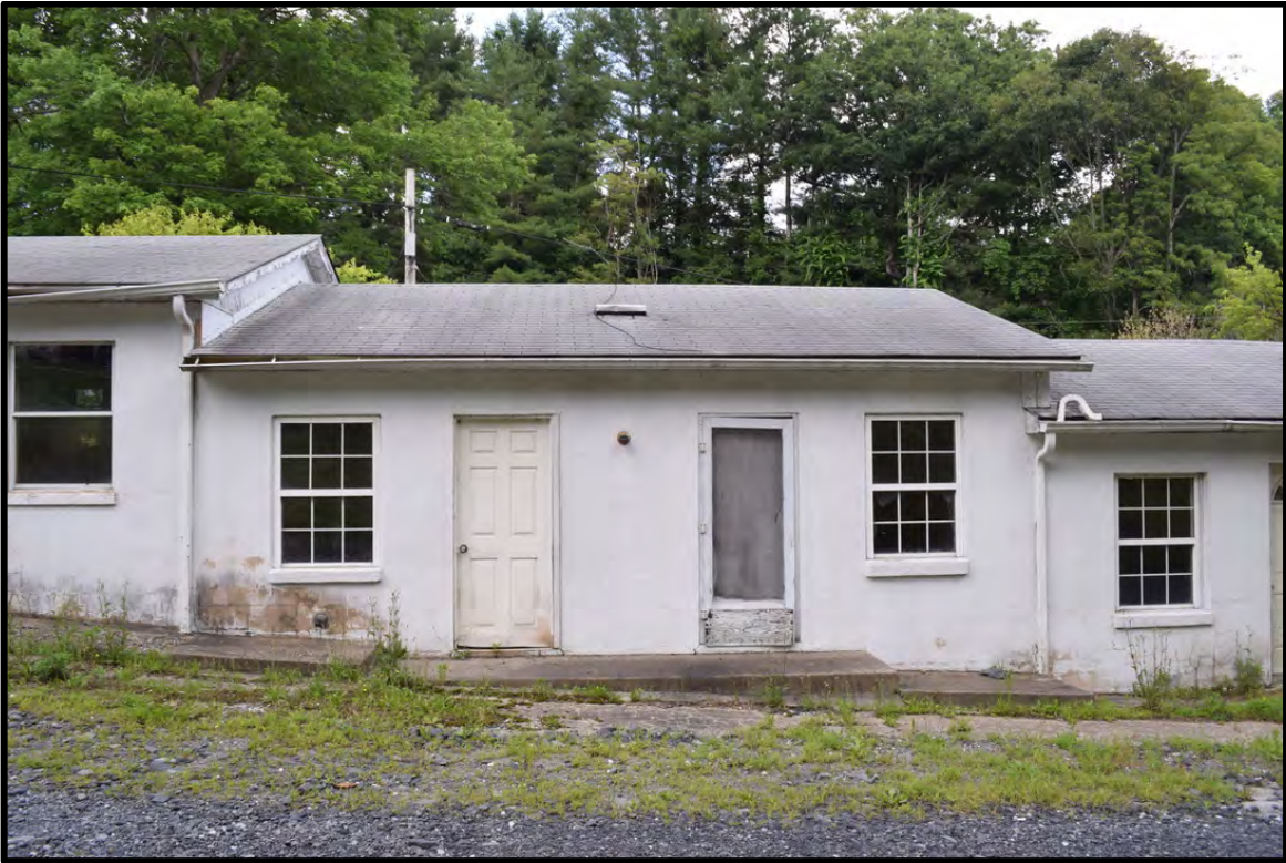
Unit number 2 in motor court, view to the east
