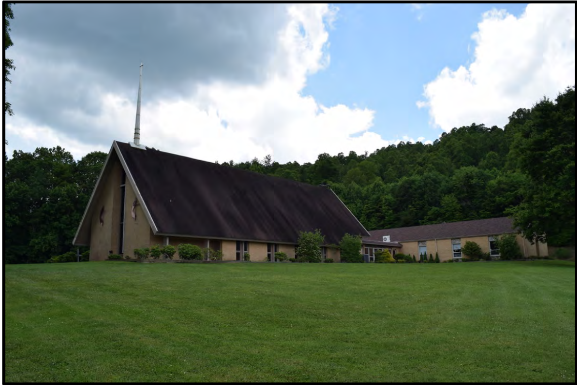
Spruce Pine United Methodist Church (1966), view to the southwest
