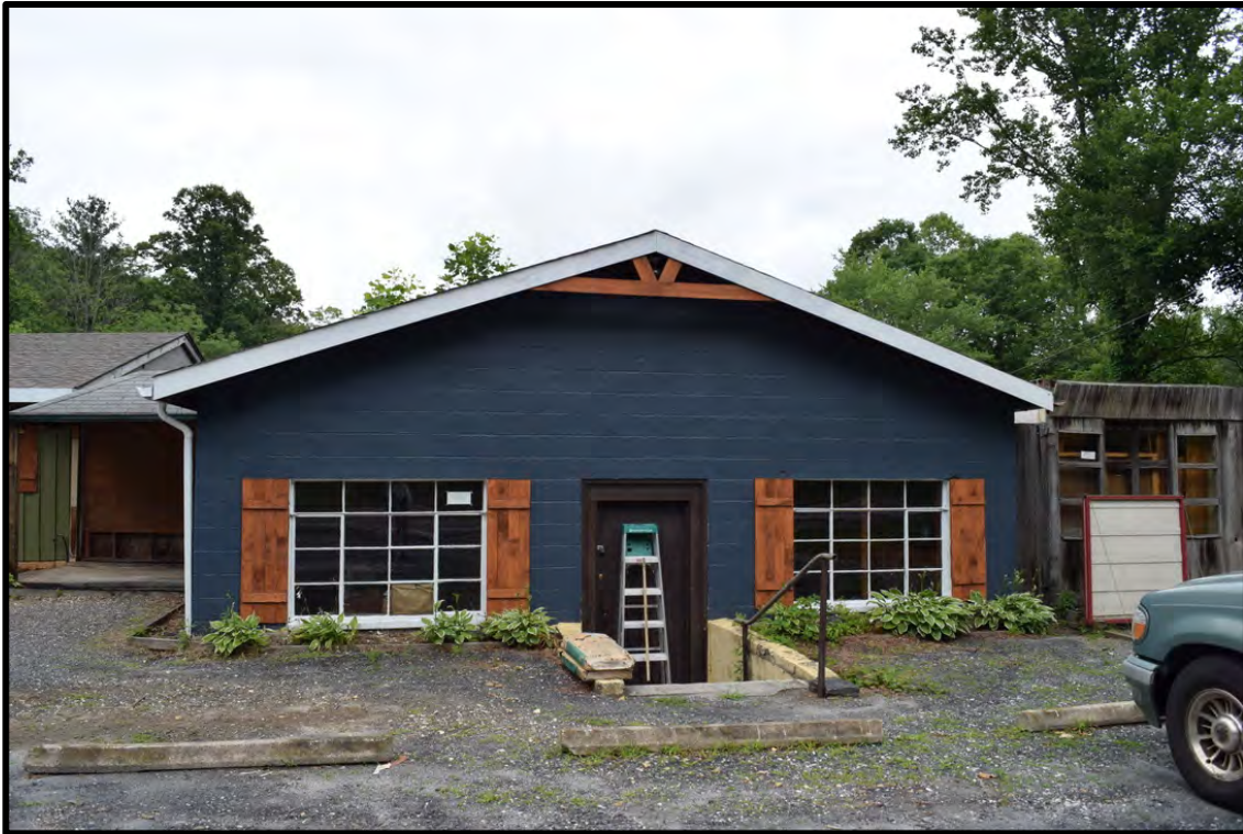
1954 Forge, view to the west
