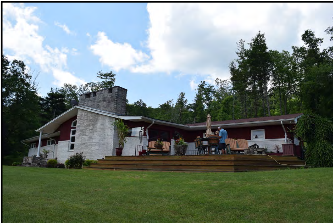
Front (northeast) corner of house, view to the southwest
