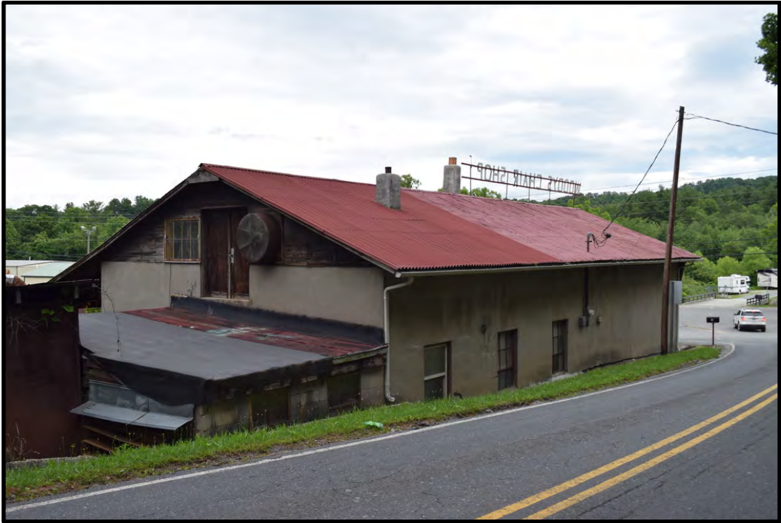
Southeast corner, view to the north
