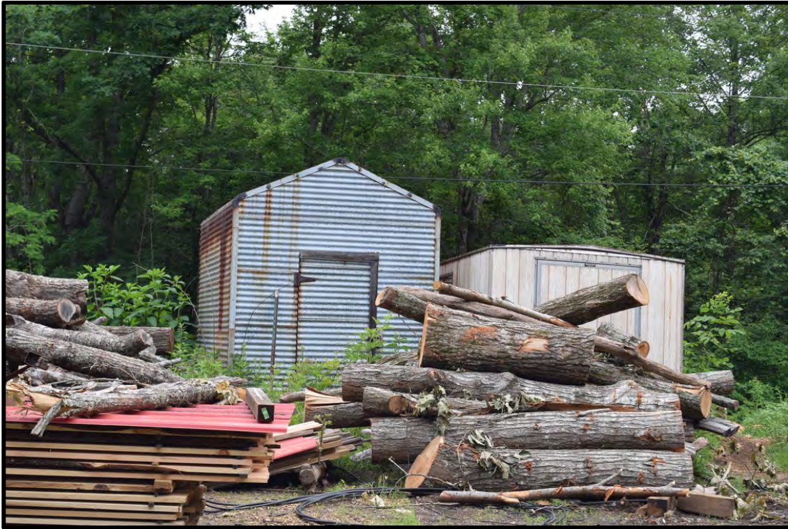
Storage buildings, view to the north
