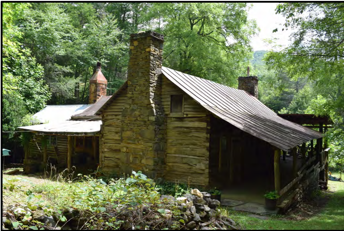
Henry Willis House (NR) view to the southwest
