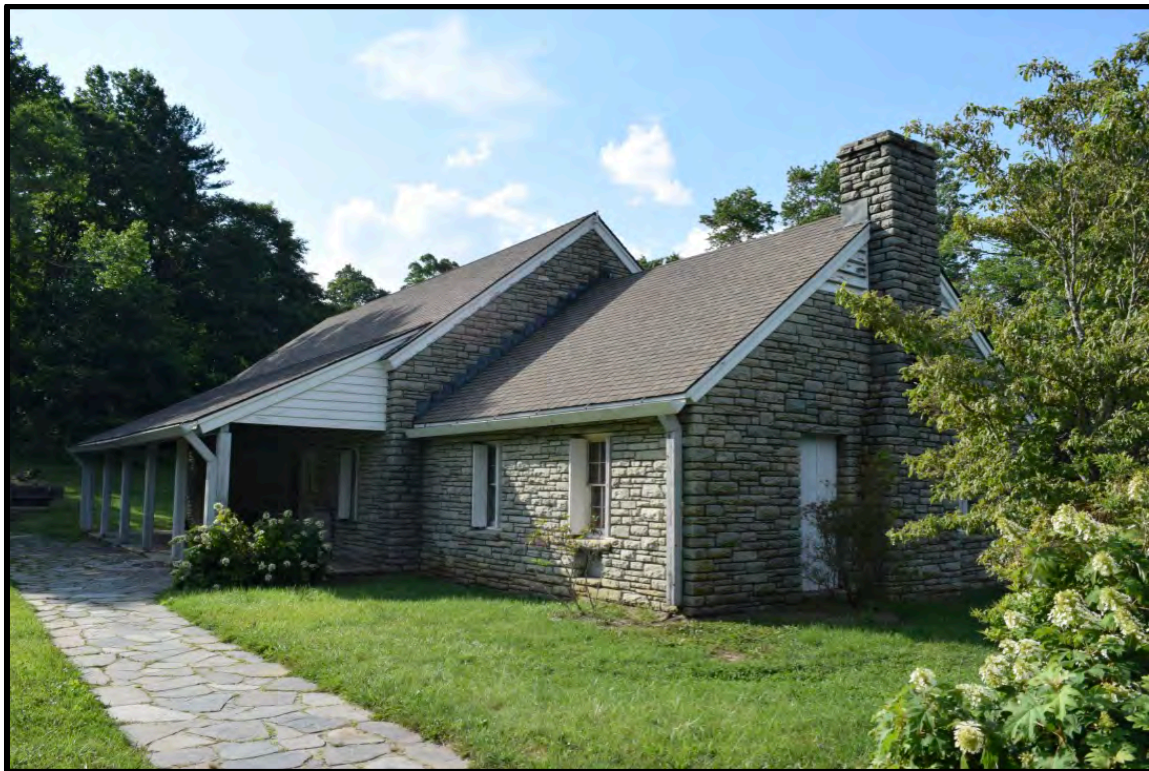
Front corner, view to the northwest
