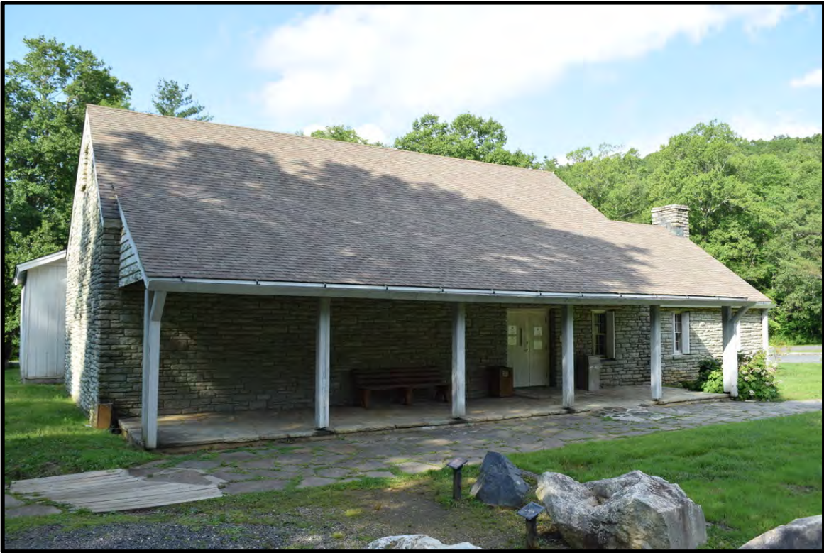
Museum facade, view to the north-northeast
