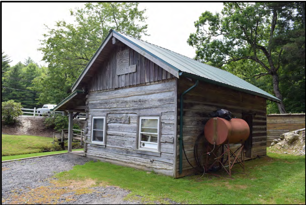
Northwest corner, view to the southeast
