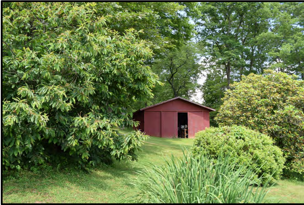
1970s barn northwest of the house, view to the north
