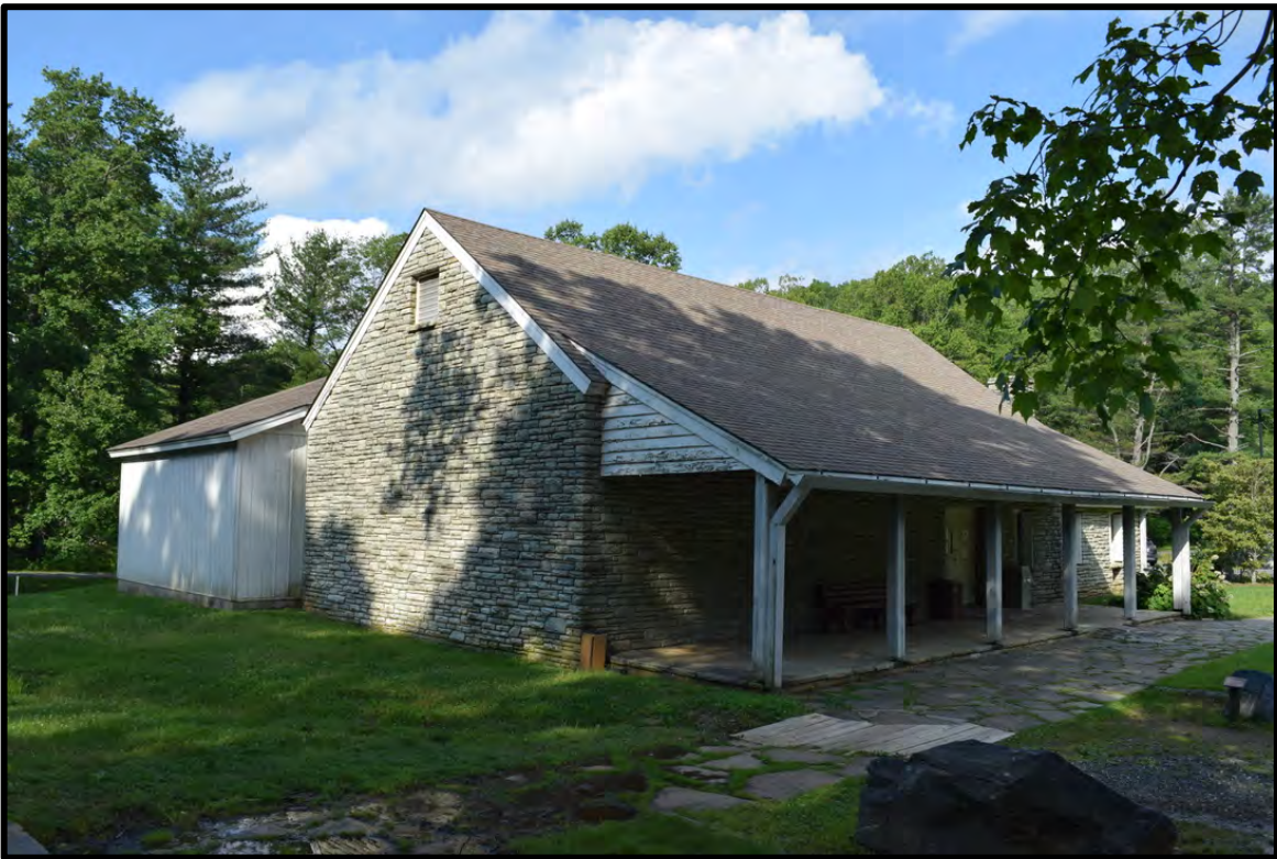
Museum, southwest corner, view to the northeast
