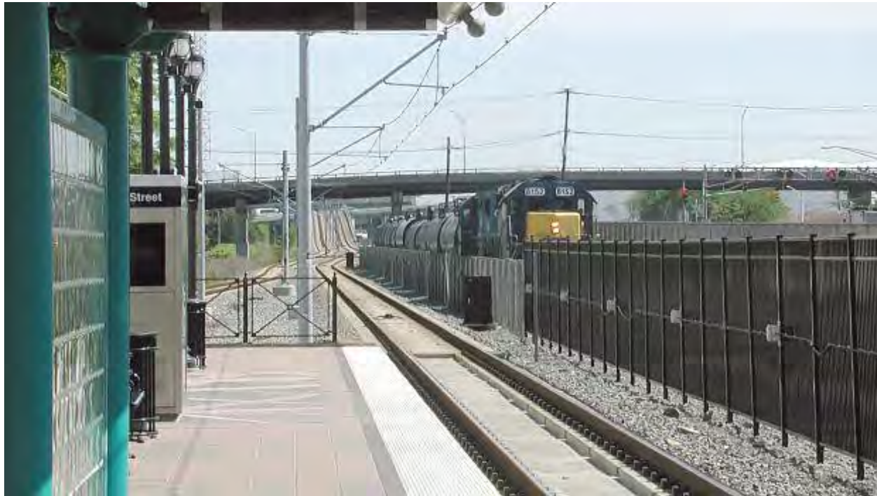
Figure 5: HUDSON-BERGEN LIGHT RAIL TRACKS ADJACENT TO CSX (NJ)
