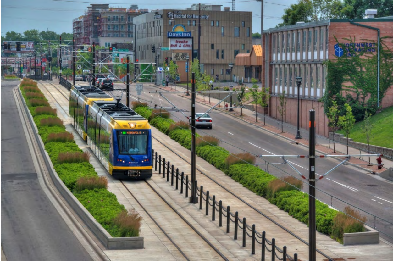
Figure 8: EXCLUSIVE CENTER RUNNING TRANSIT LANES—GREEN LINE LRT (TWIN CITIES, MN)
