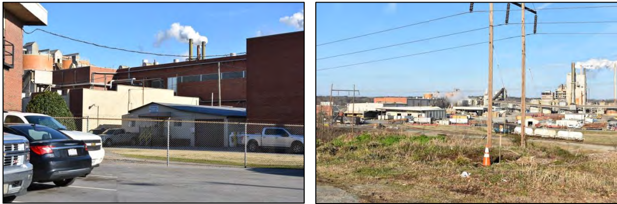
Figure 68. Left, detail of west elevation of 1958 paper mill building; right, view from southeast of mill with 1958 building looming on skyline at center left
