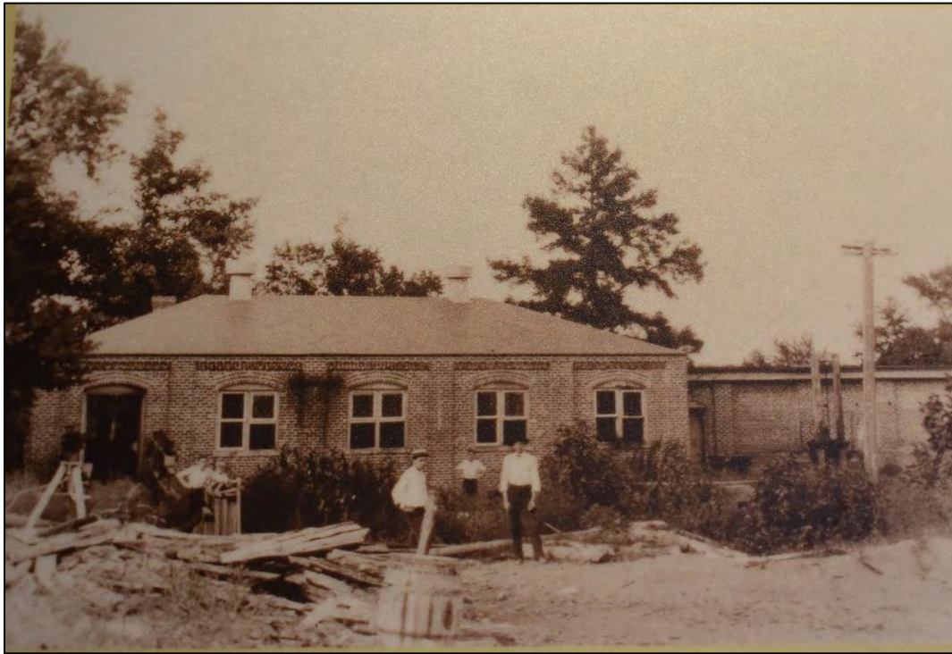
Figure 19. Power Plant, ca. 1910 (image credit: Roanoke Canal Museum and Trail)
