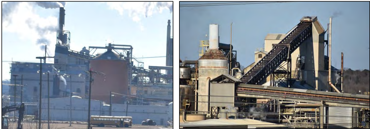
Figure 61. Left, looking west at chemical pulp mill with one-story, original/early walls of paper mill visible in foreground; right, looking northwest at mill at chemical pulp mill with numerous modern appendages and accretions of processing equipment
