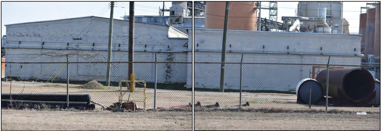
Figure 58. Composite view of west elevation of paper mill; note that all bays are filled in
