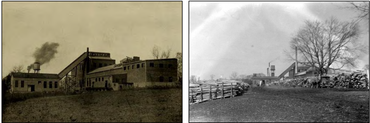
Figure 79. View of “Sulphate fibre mill” from south, 1909, at left (source: Joseph H. Wallace & Co.); view from same direction, perhaps 1920s, at right (source: Images of North Carolina)
