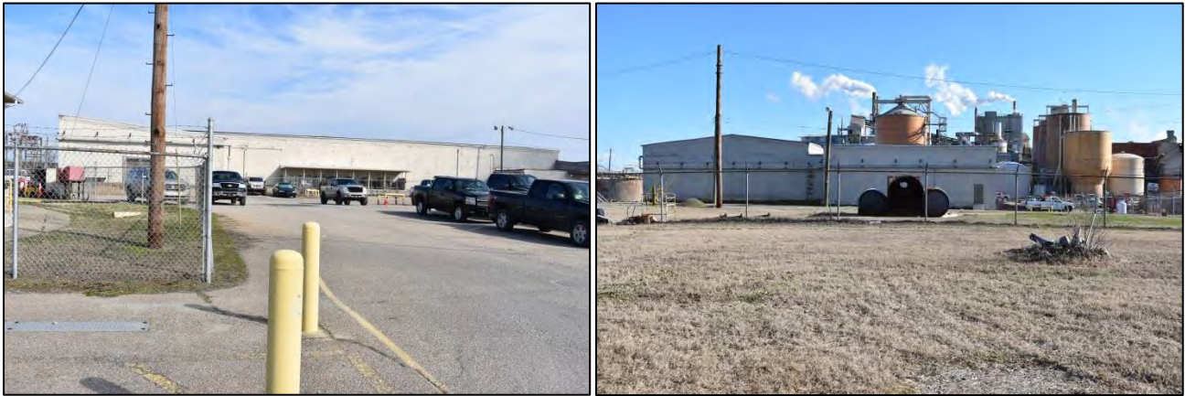
Figure 57. Left, south elevation of early portion of paper mill with all original bays filled in; right, west elevation
