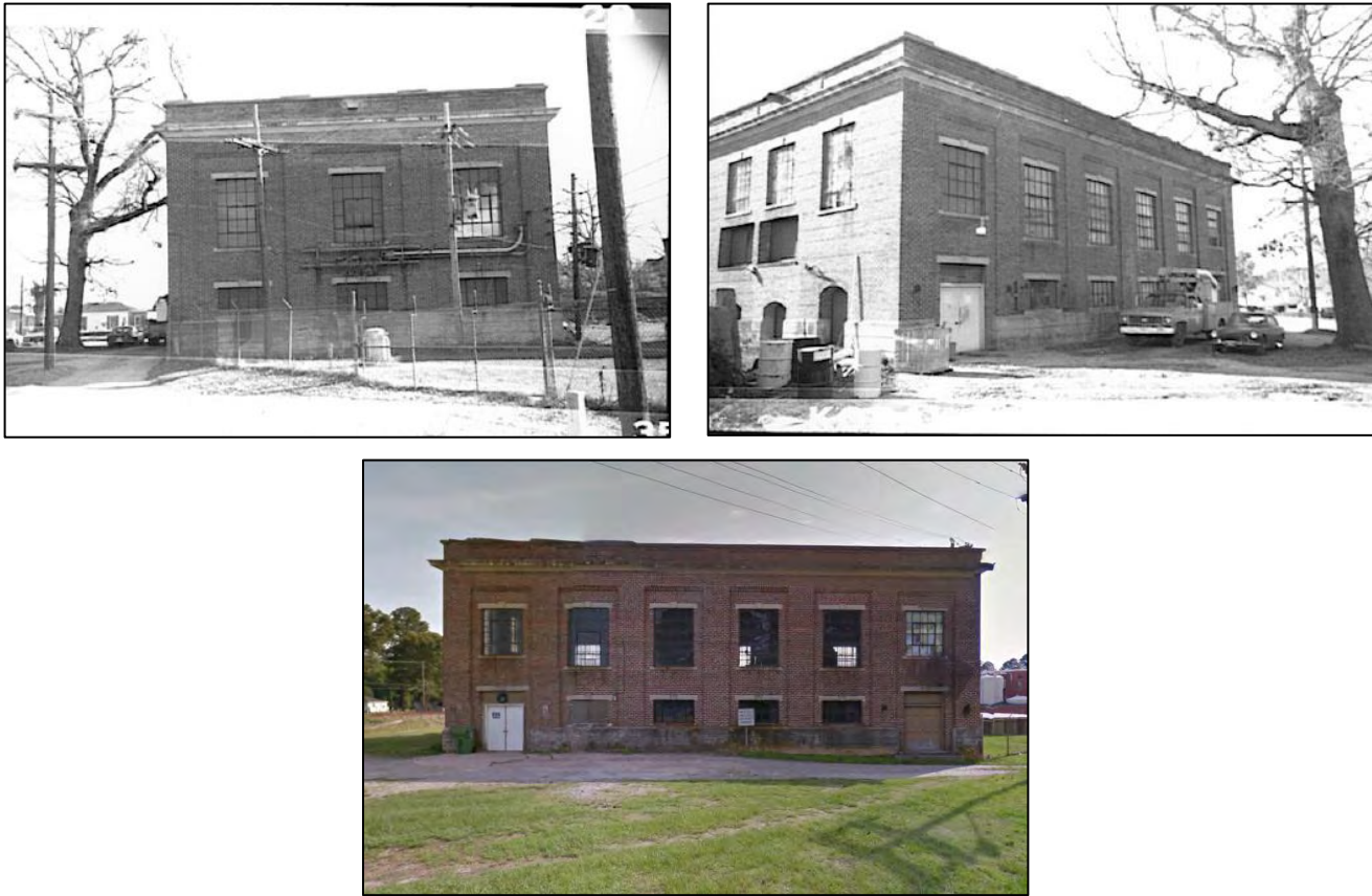
Figure 32. Top, Enfield Electric Power Plant and Water Works (HX0408) at time of 1990 survey (photo credit: NC HPO); bottom, ca. 2013 view of power plant (image credit: Google Streetview)
