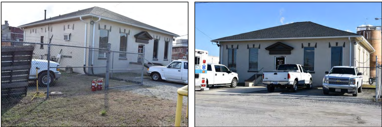
Figure 63. Former office building—north and west front elevations, at left, and west front elevation, at right
