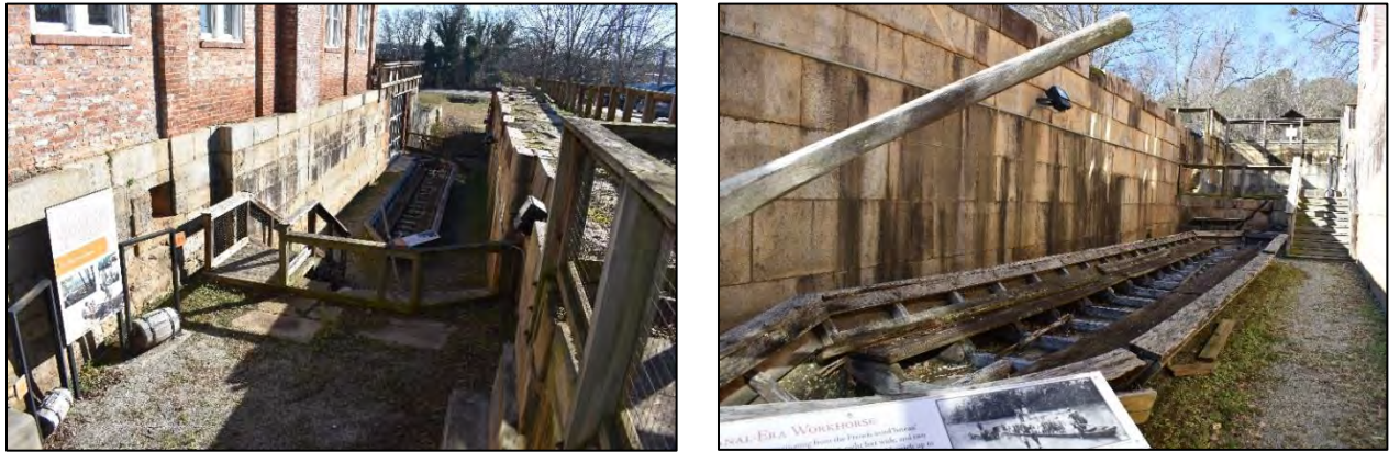
Figure 15. Left, view down into lock (looking east); right, view into lock (looking west)
