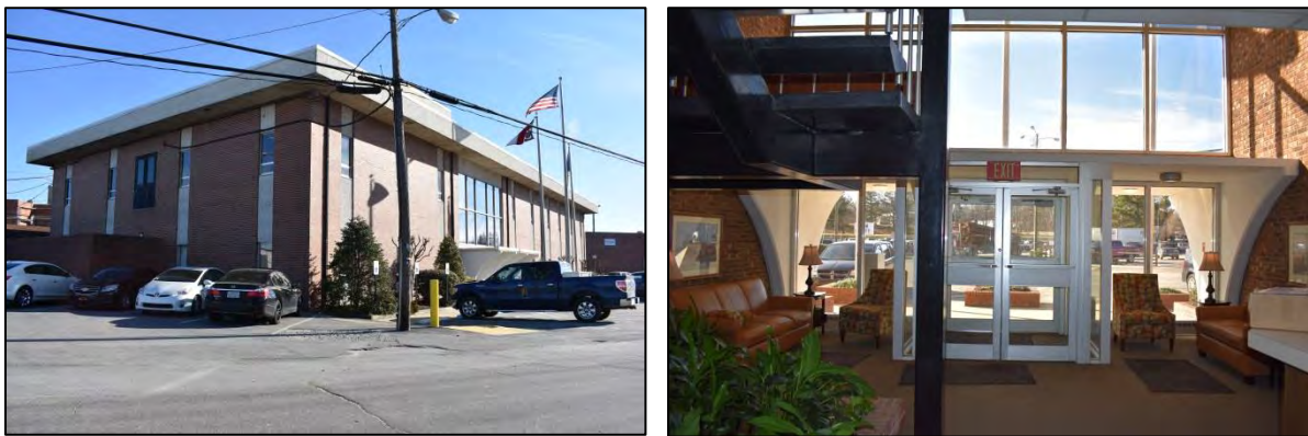
Figure 69. North side and west front elevations of ca.1970 office building and full-height lobby
