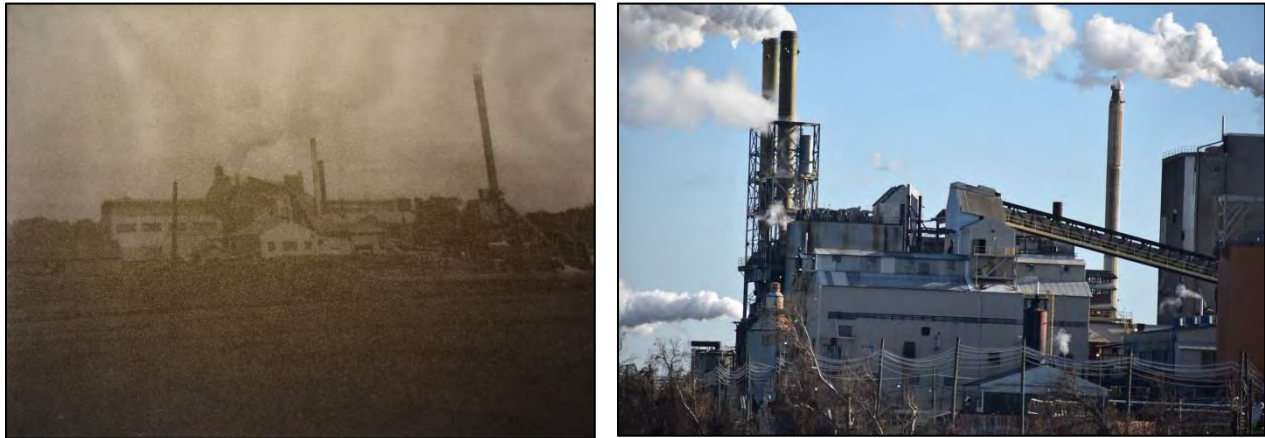
Figure 60. Left, looking southeast at chemical pulp mill in 1945 and, right, at present
