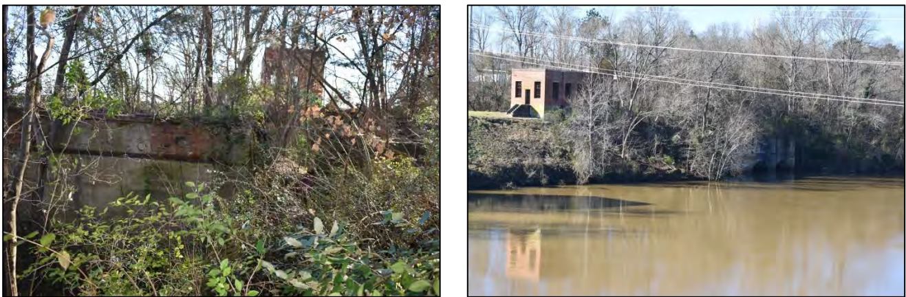
Figure 41. Plant No. 1—left, looking east over plant wall with Switch House in background; right, view of Switch House at left and plant wall along water at right
