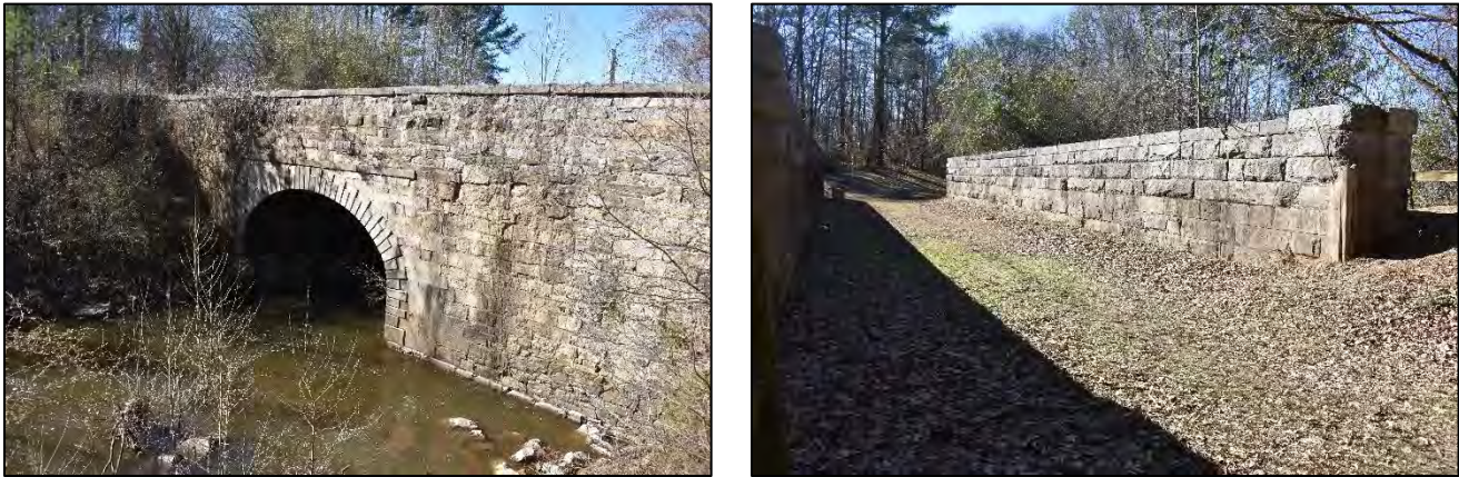
Figure 7. Left, view of aqueduct arch over Chockoyotte Creek; right, view of canal channel spanning the creek
