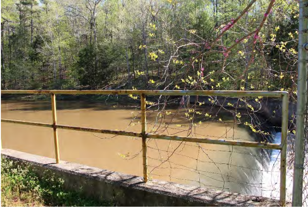
Figure 28. Spillway across Eno River, view looking northeast.
