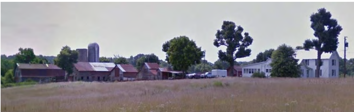
Figure 16. 1912 Lloyd Dairy Farm showing farmhouse at right and cohesive grouping of outbuildings. Google Street View image.
