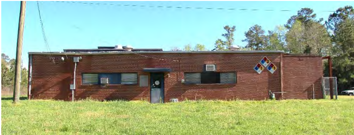
Figure 18. South-facing facade of the 1968 Orange-Alamance Water System building, view looking north.
