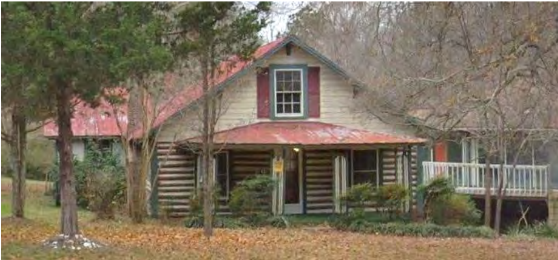
Figure 14. Rustic log house at 618 NC 86 in Hillsborough. Google Street View image.
