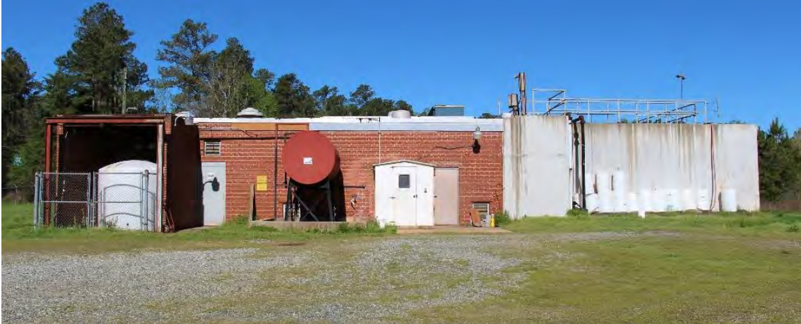
Figure 21. Side (east) elevation, view looking west.
