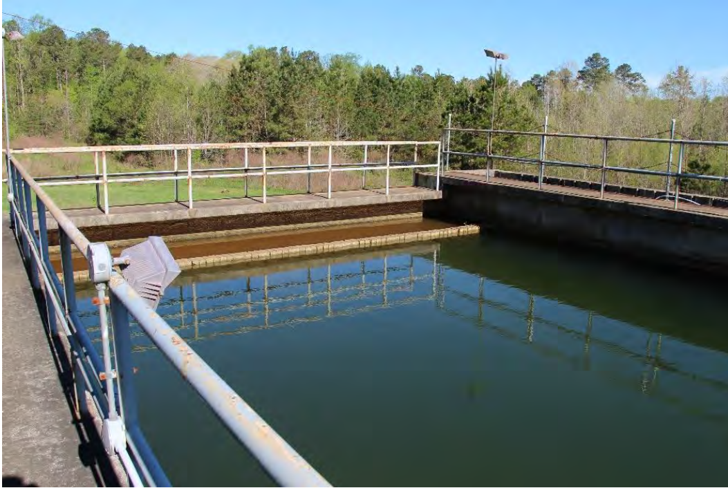
Figure 25. Settling basin and catwalk.
