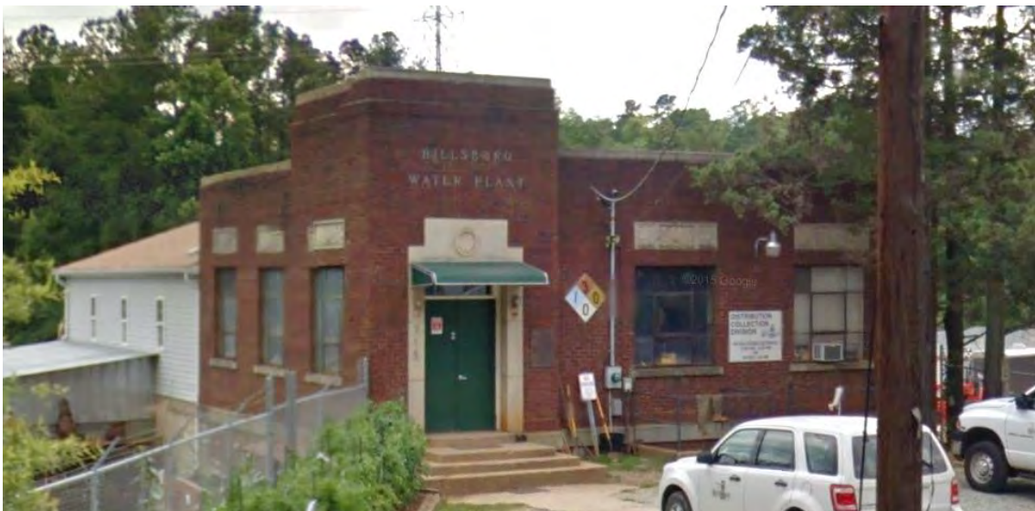
Figure 34. Town of Hillsborough Water Treatment Plant. Google Street View image.
