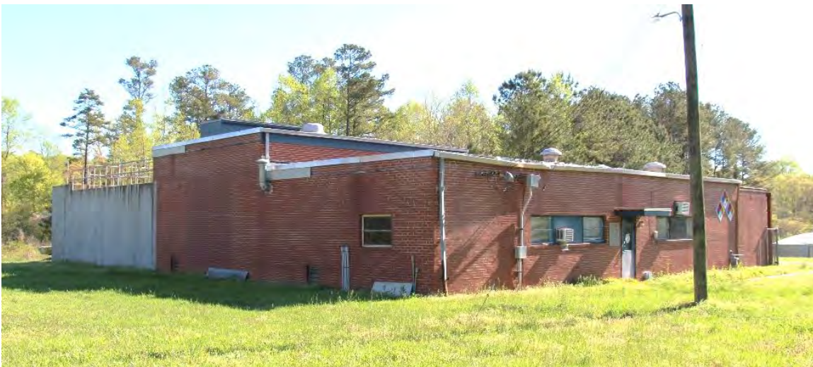
Figure 20. Facade (south) and side (west) elevation, view looking northeast.
