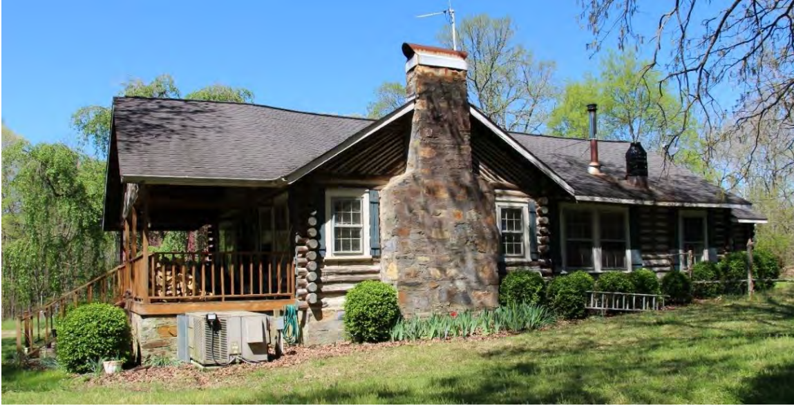
Figure 7. c.1925 log house, side (east) elevation, view facing west.
