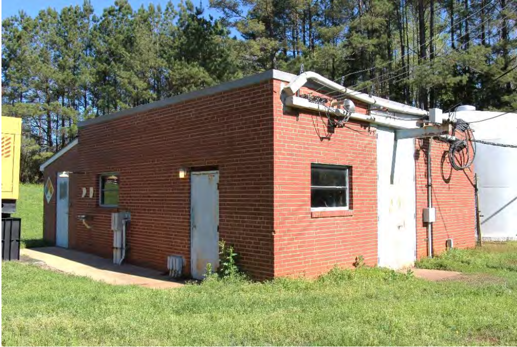
Figure 27. Pumping station, view looking northwest.
