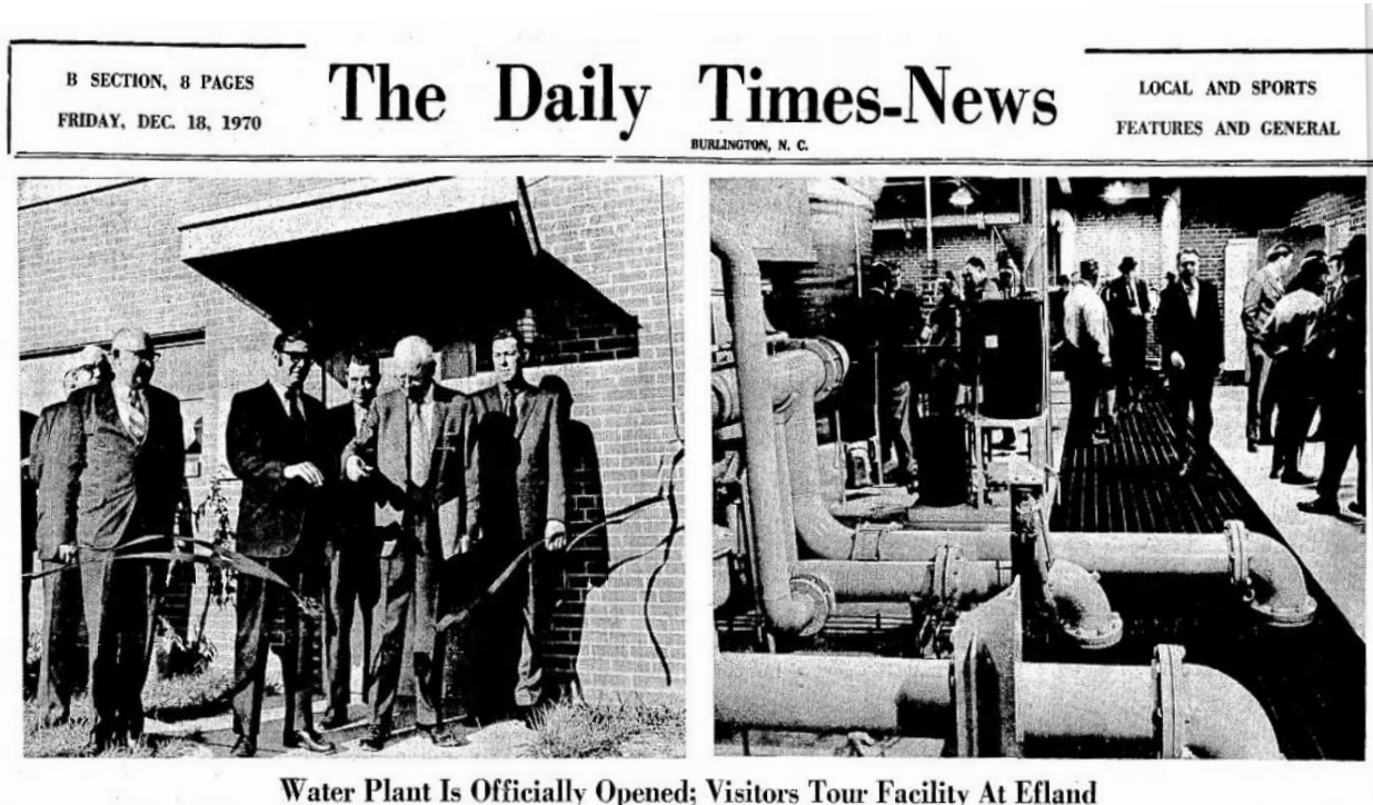
In the photo at left, the ribbon is cut in official... Mabona... Water Plant Is Officially Opened; Visitors Tour Facility At Efland
