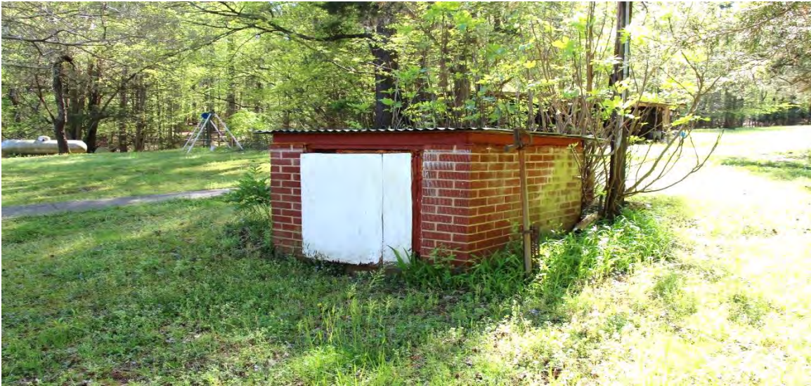
Figure 26. C.1960 pumphouse, view facing southwest.
