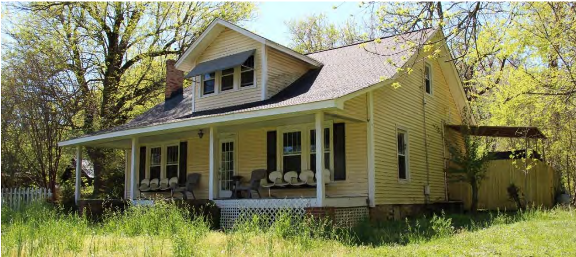
Figure 14. Tapp House 1, facade (east) and side (north) elevation, view facing west/southwest.
