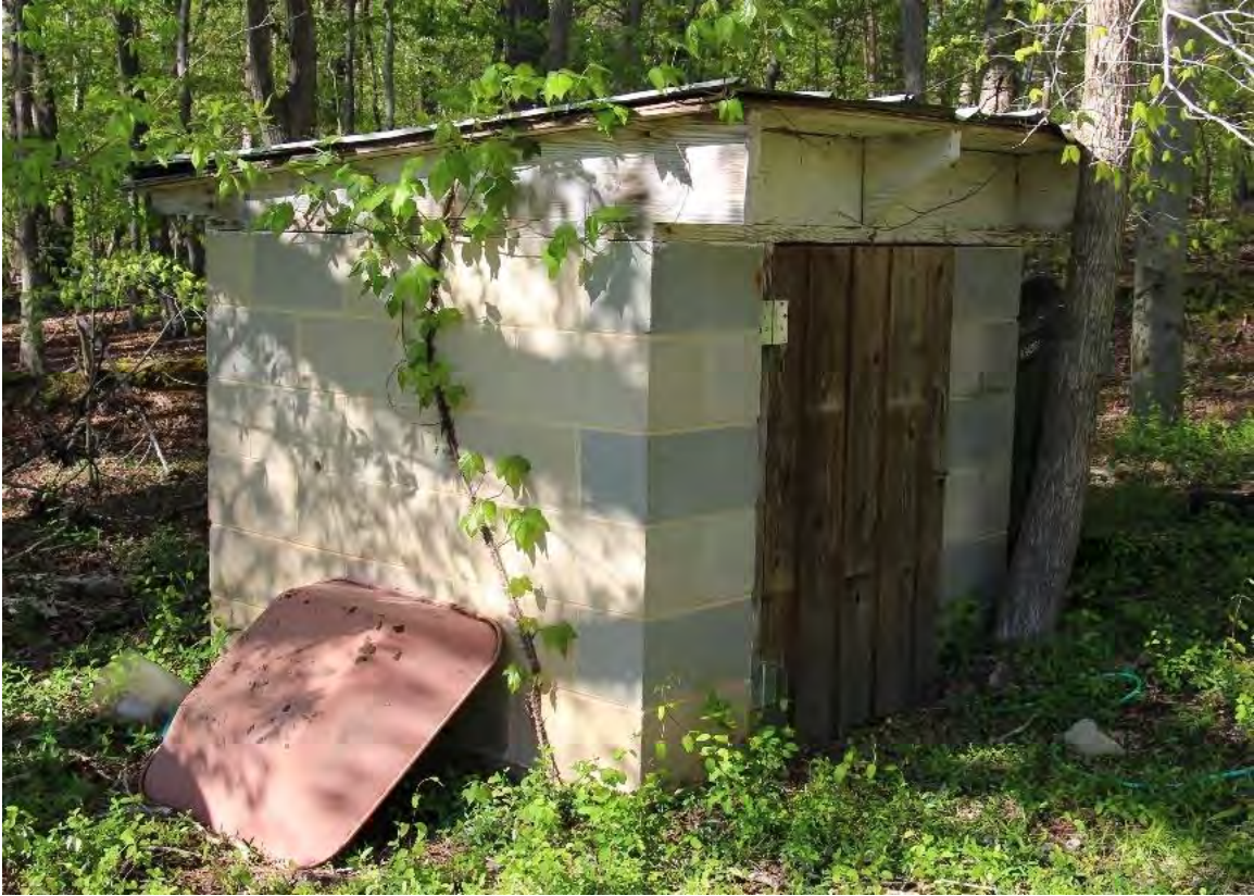
Figure 37. C.1950 concrete pumphouse, view facing northwest.
