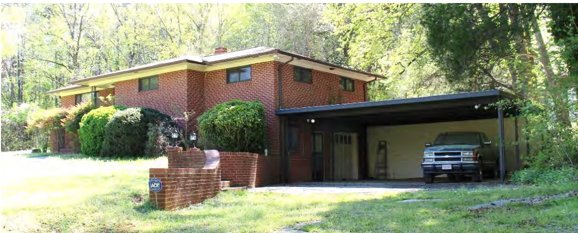
Figure 24. 1959 Tapp House 2 facade (east) and side (north) elevation , view facing southwest.
