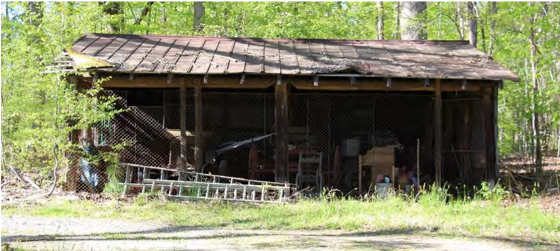
Figure 36. C.1950 metal-clad shed, view facing north.
