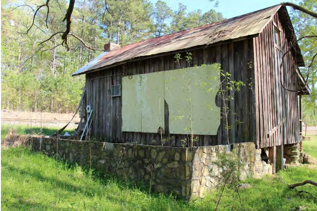
Figure 42. 1883 post office building, rear elevation, view facing southwest.
