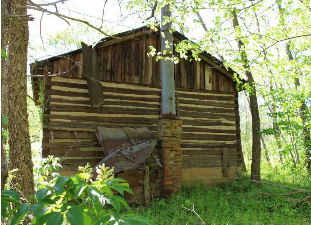
Figure 45. C.1875 tobacco barn, rear elevation, view facing northwest.
