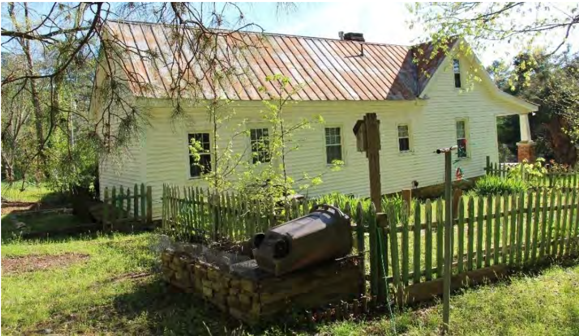
Figure 32. The side (north) elevation of the c.1885 main house, view facing southwest.
