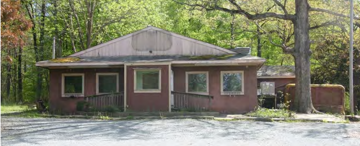
Figure 56. Facade (north) of the dining room/kitchen component, view looking south.
