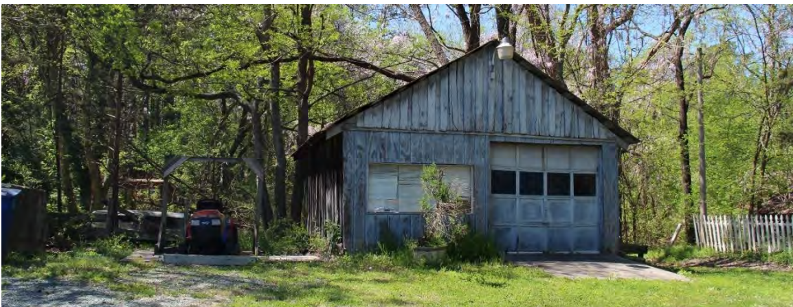
Figure 19. C.1930 garage, view facing west.
