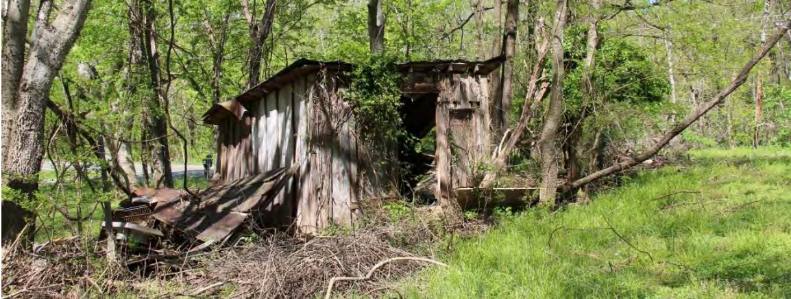
Figure 17. C.1930 shed, view facing north.
