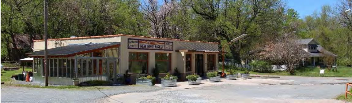
Figure 74. Former gas station (OR3174) at left and Tapp House 1 (OR3175) at right. View facing northwest.
