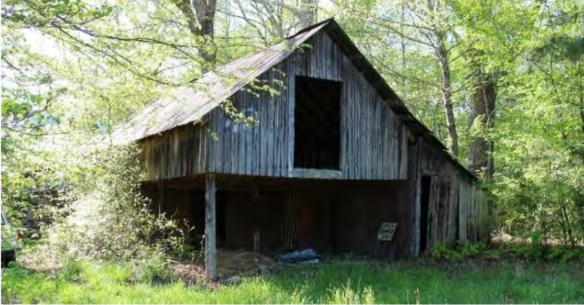
Figure 33. C.1900 main barn outbuilding, view facing west.
