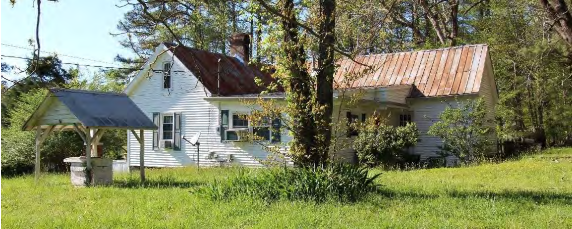
Figure 31. The side (south) elevation of the c.1885 main house, including shed-roof addition, and well, view facing northwest.
