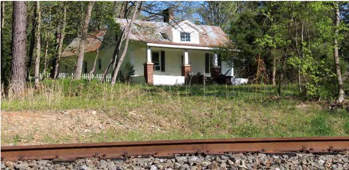
Figure 29. The c.1885 main house on the farmstead with the railroad in the foreground, view facing southeast.
