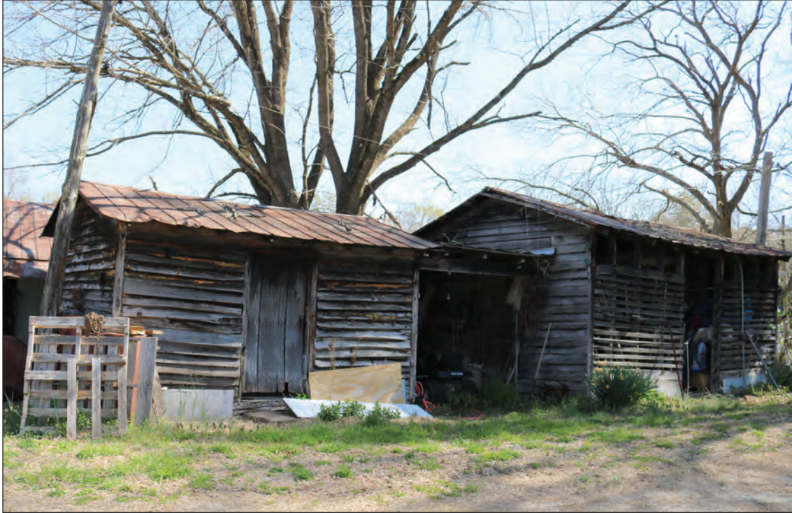
Figure 3.22. Corn Crib and Storage Building, Looking Northeast.
