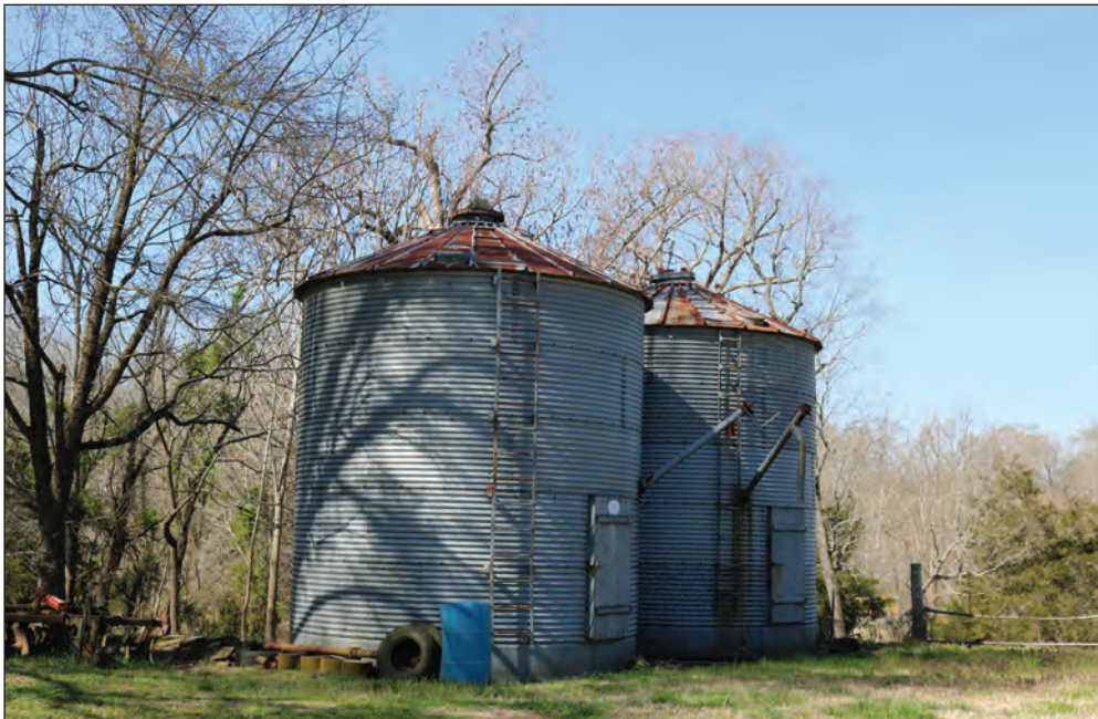
Figure 3.24. Corrugated Metal Silos, Looking West.
