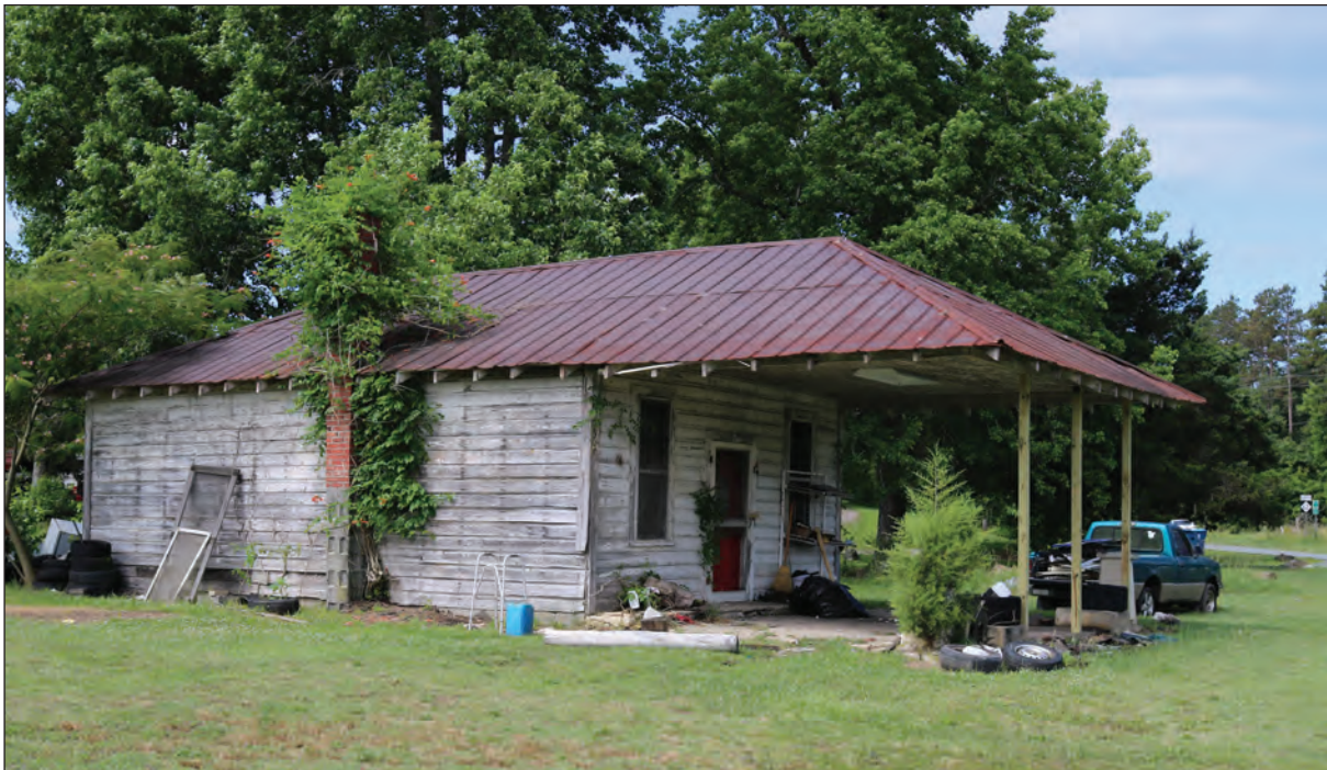
Figure 3.71. Coble's Store (GF1924), Looking Southeast.
