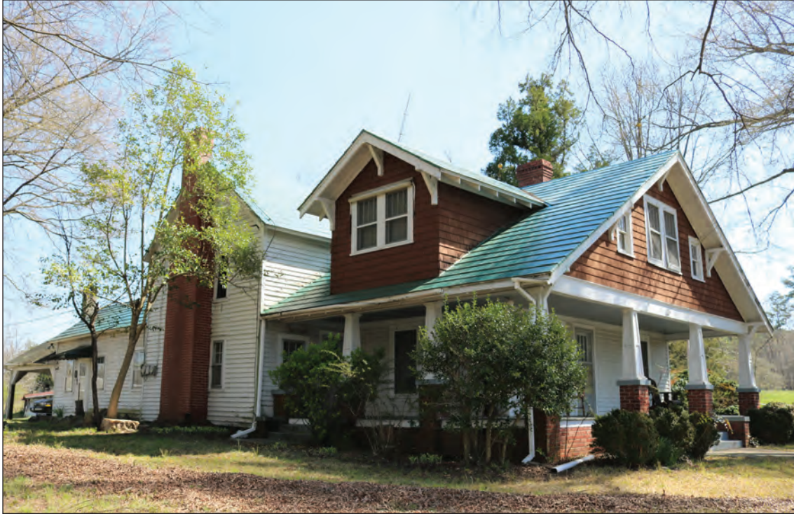
Figure 3.8 David Daniel Coble Farm House, Façade and West Elevation, Looking Northeast.
