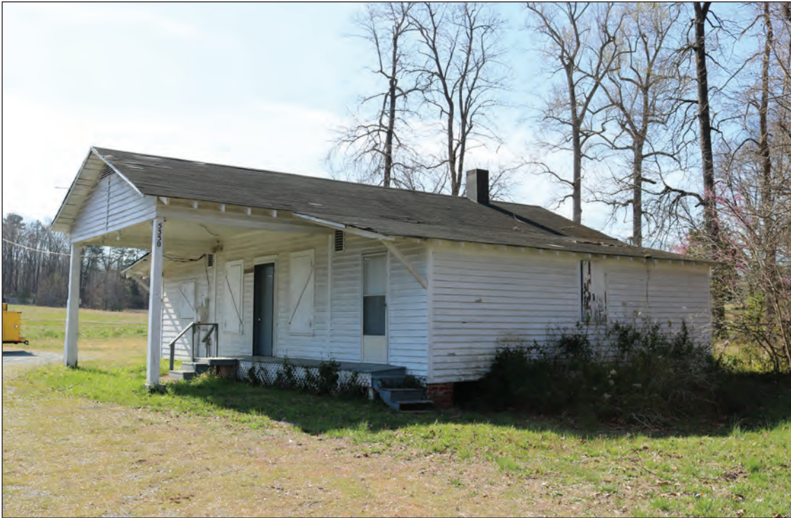
Figure 3.62. Coble Farm Store and Filling Station, Façade, and West Elevation, Looking Southeast.
