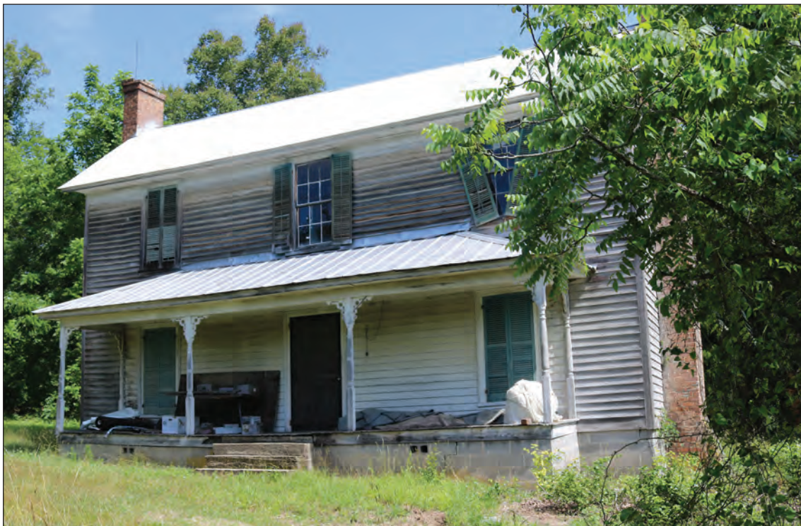
Figure 5.2. Thomas R. Greeson House (GF1923), Looking North.
