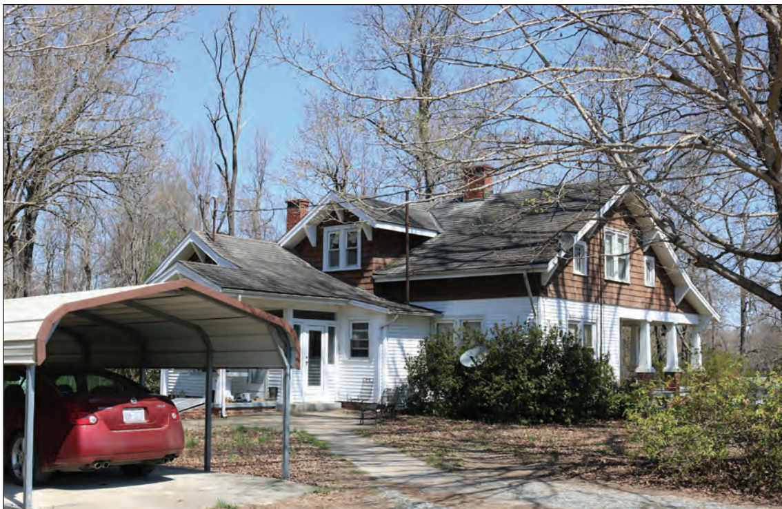
Figure 3.43. Shafter Coble Farm House, South and East Elevations, Looking Northwest
