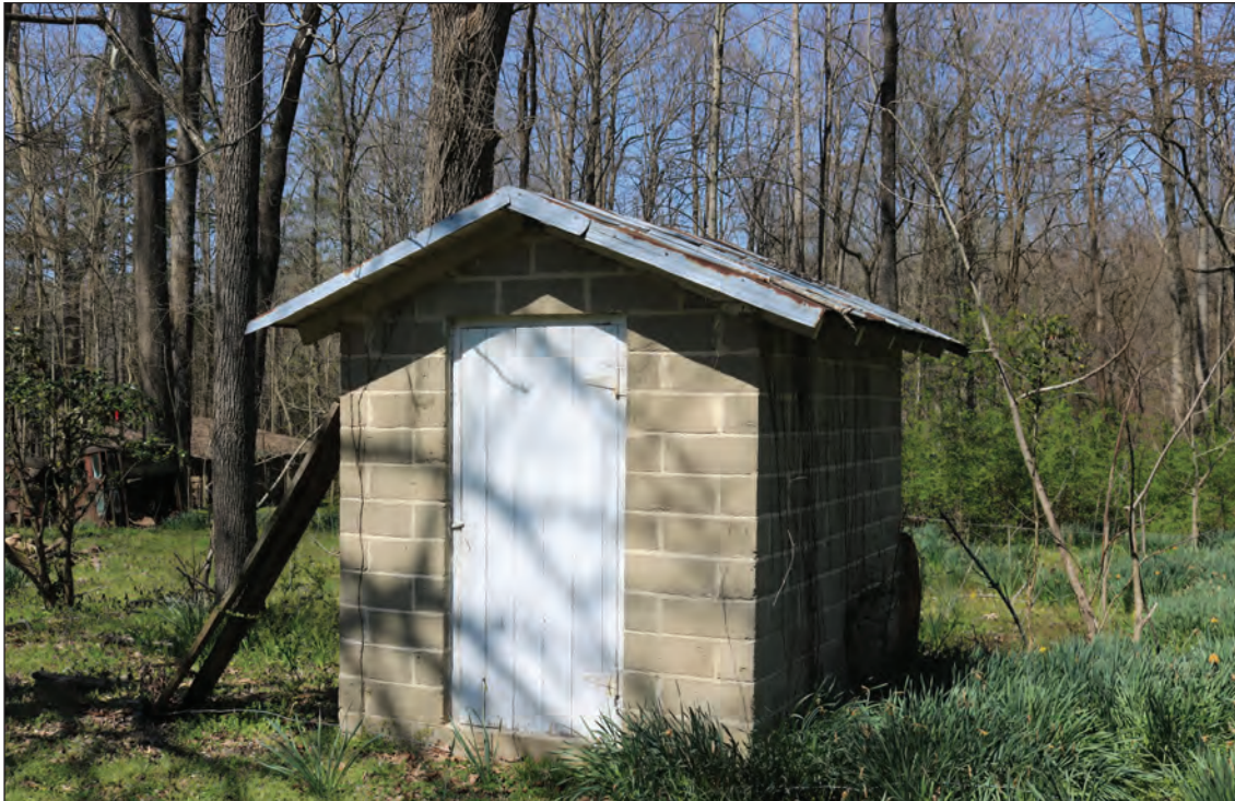
Figure 3.46. Pumphouse, Looking West.
