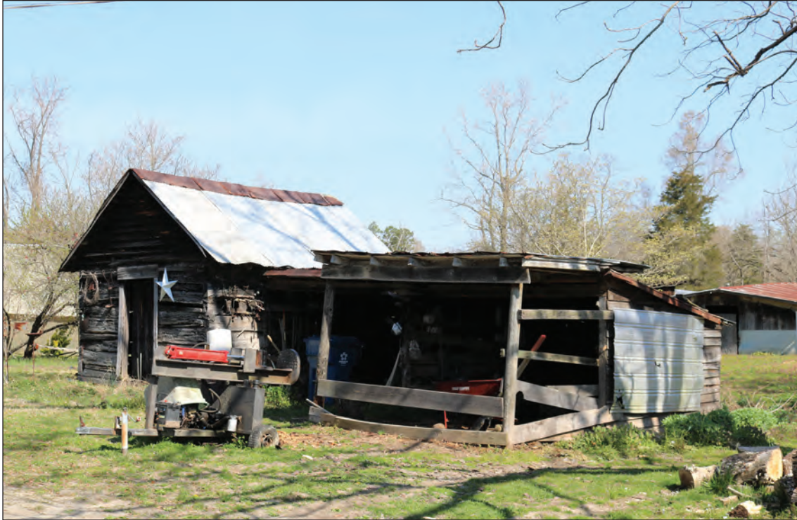
Figure 3.20. Smokehouse, Looking Northwest.
