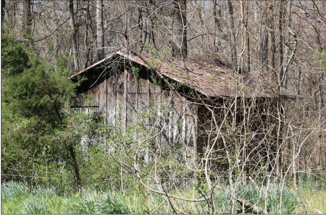
Figure 3.45. Board and Batten Storage Shed, Looking Northwest.
