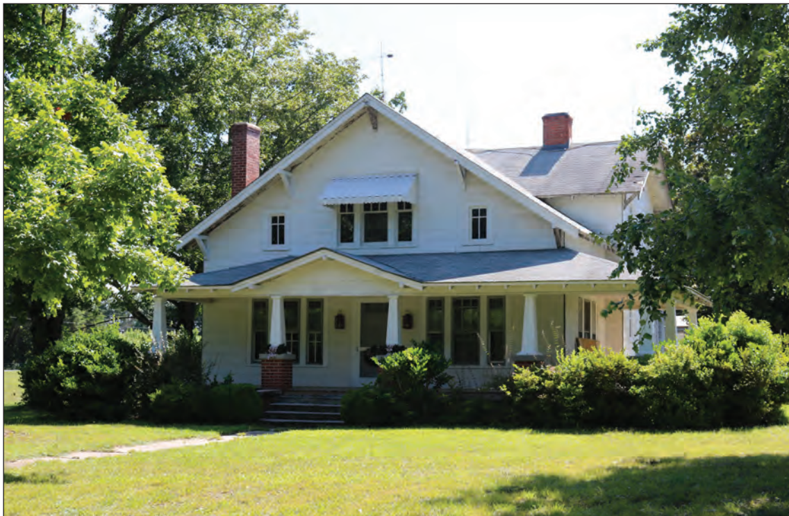
Figure 5.6. 4307 Old Julian Road, Looking Northeast.
