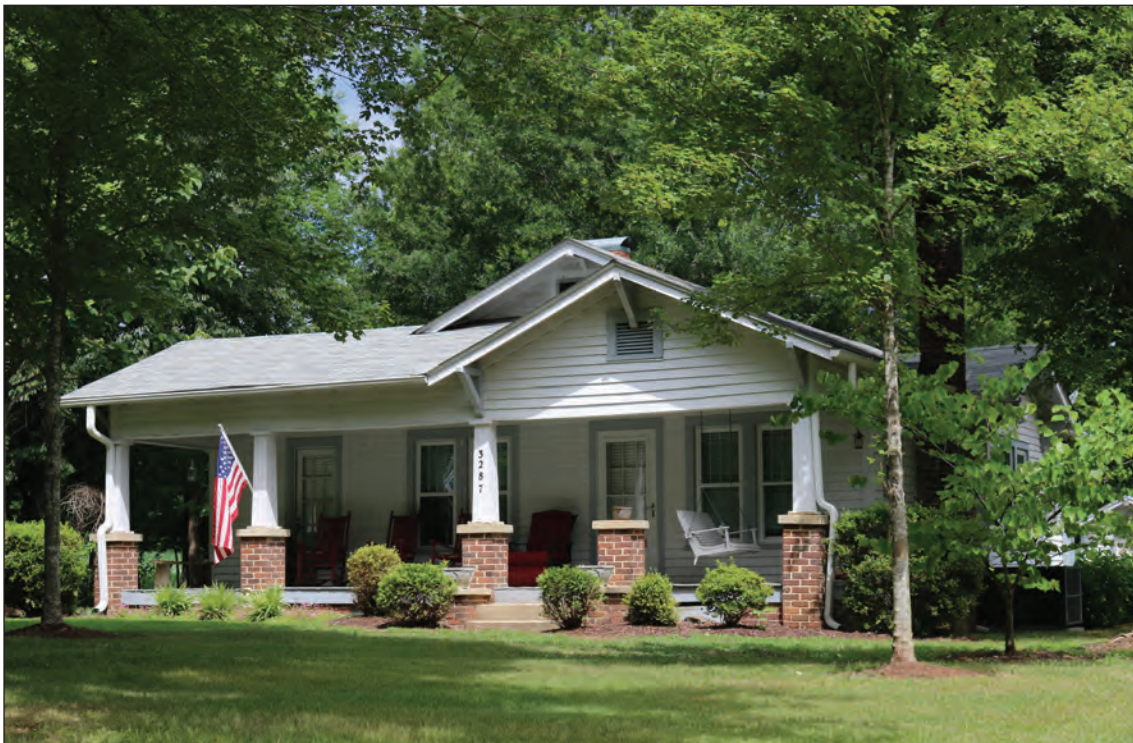
Figure 5.4. Moser Farm (GF8985), Looking West.
