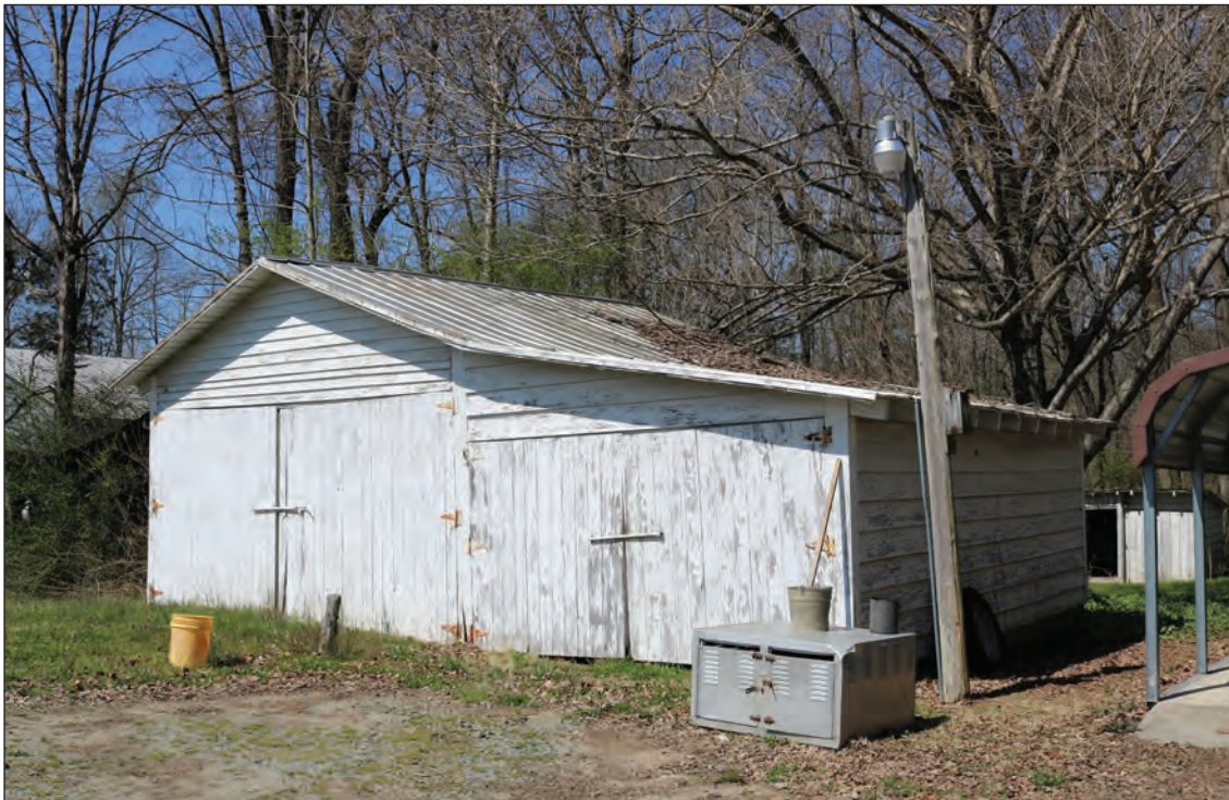
Figure 3.49. Garage, Looking Southwest.
