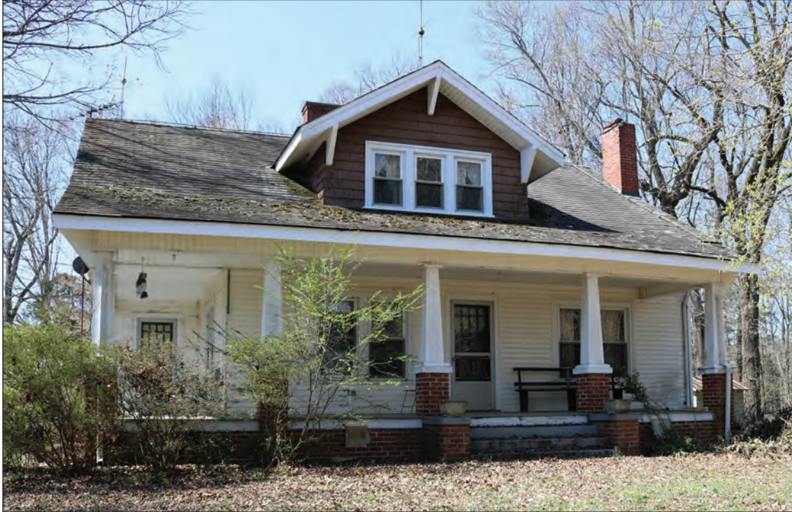
Figure 3.40. Shafter Coble Farm House, Facade, Looking Southwest.
