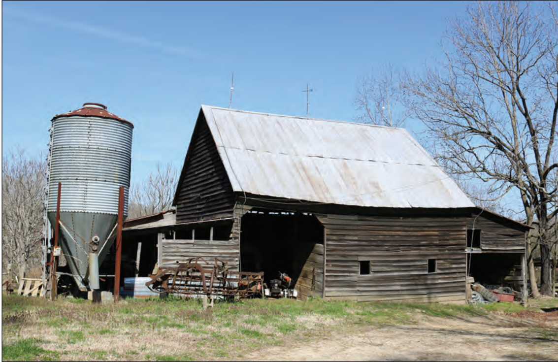
Figure 3.25. Barn and Corrugated Metal Silo, Looking Northwest.
