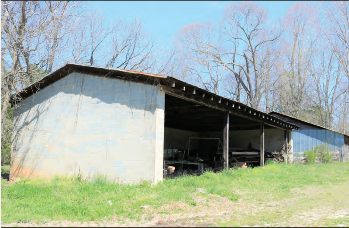
Figure 3.60. Farm Equipment Shed, Façade and South Elevation, Looking Northwest.
