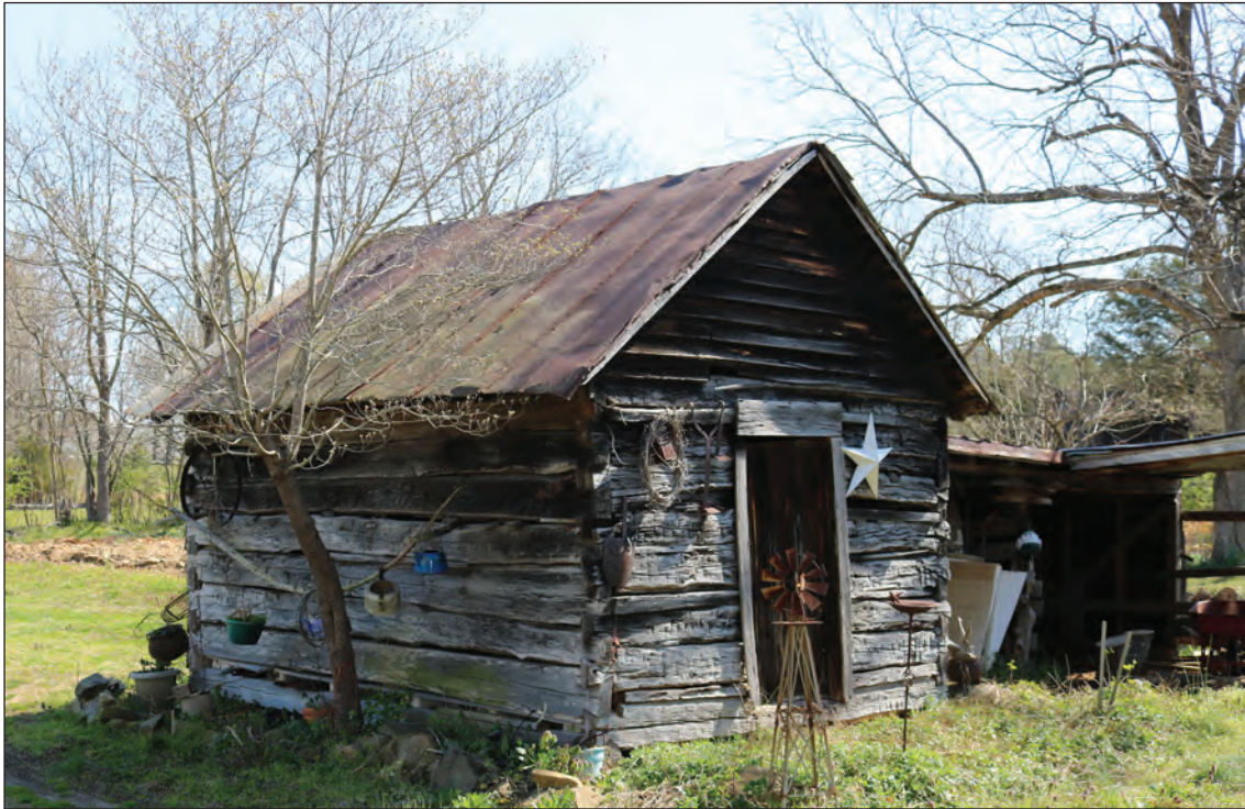
Figure 3.19. Smokehouse, Looking Northeast.
