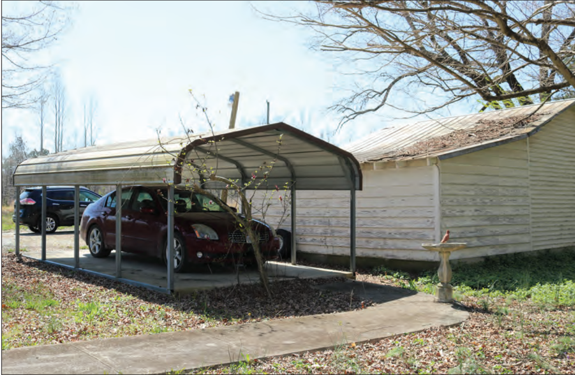
Figure 3.50 Carport, Looking Southeast.
