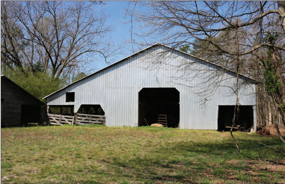
Figure 3.54. Barn, Looking West.
