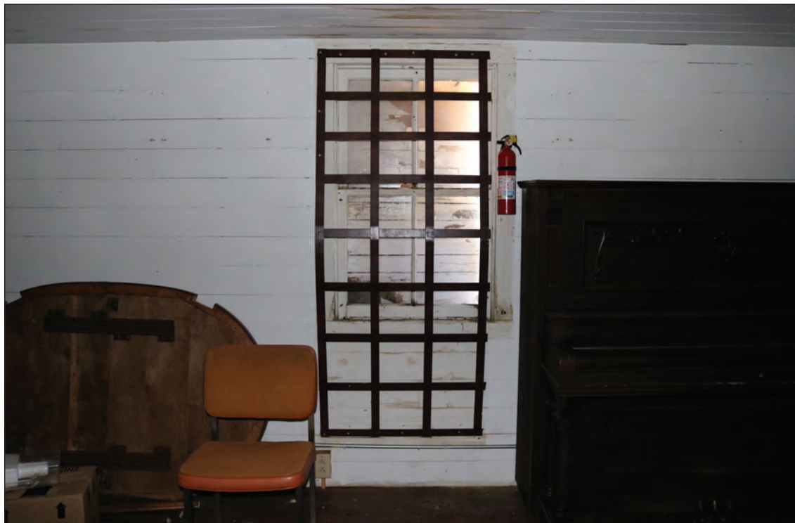
Figure 3.69. Coble Farm Store and Filling Station, Cast Iron Safety Grate, Looking West
