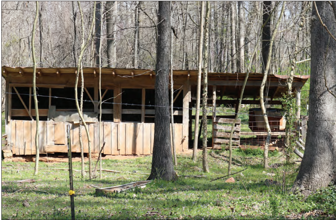
Figure 3.53. Large Chicken Coop, Looking North.
