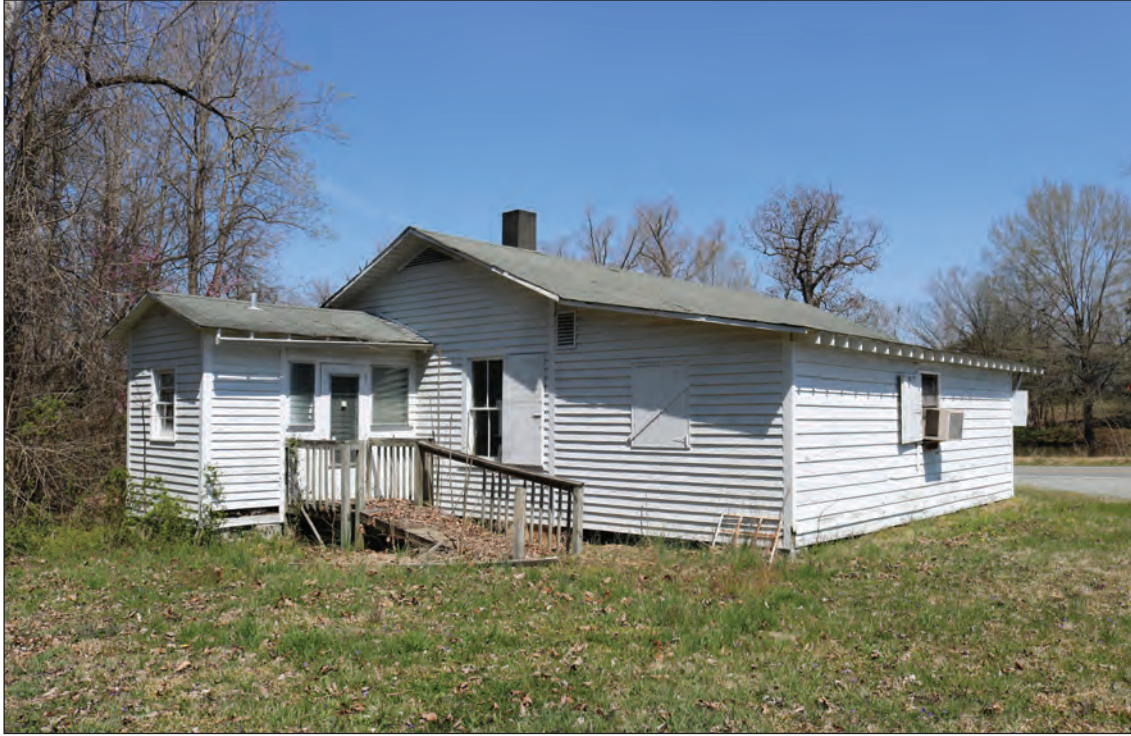
Figure 3.63. Coble Farm Store and Filling Station, South and West Elevations, Looking Northwest.
