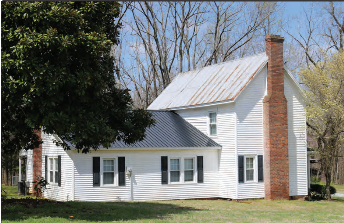
Figure 3.73. C.A. Coble Farm, East and South Elevations, Looking Northwest.
