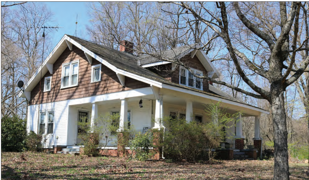
Figure 3.38. Shafter Coble Farm House, Façade and East Elevation, Looking Southwest
