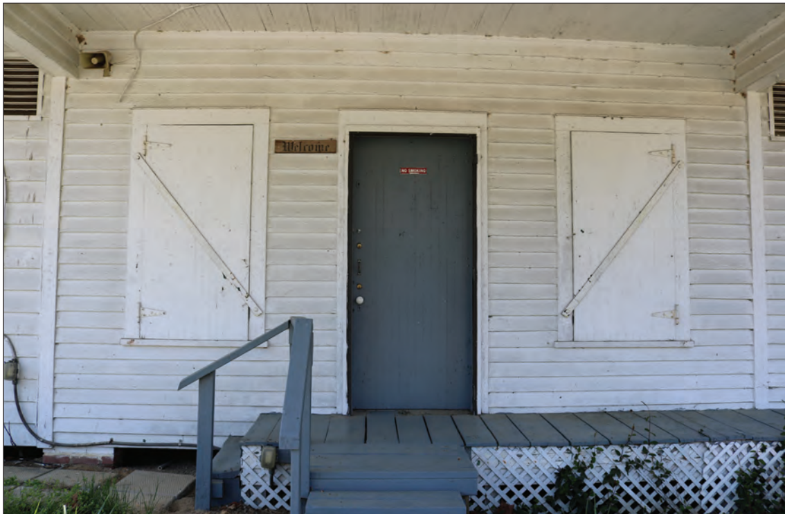
Figure 3.64. Coble Farm Store and Filling Station, Main Entrance, Looking South.
