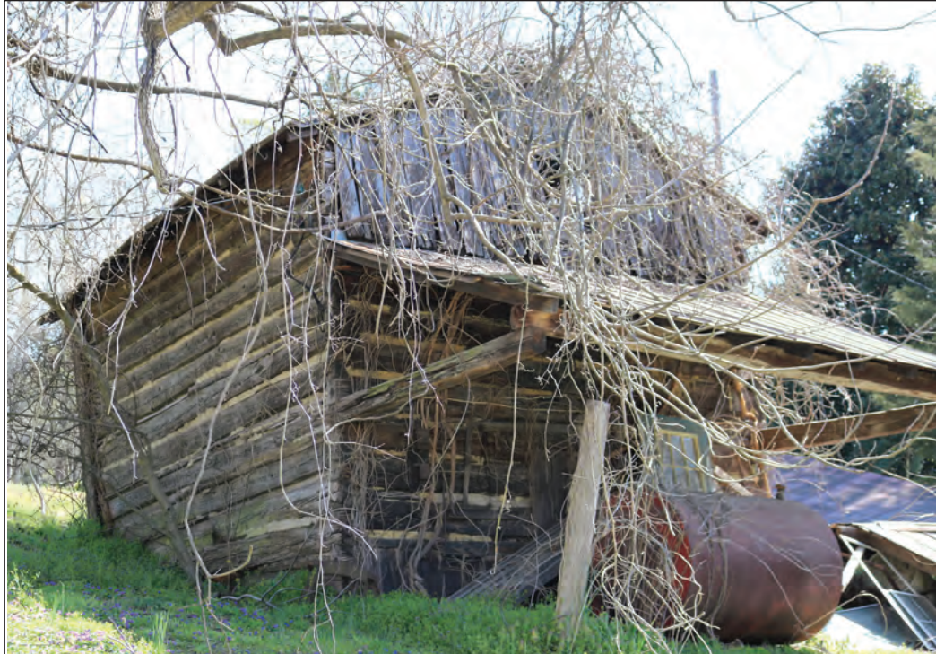
Figure 3.36. Barn, Looking Northeast.
