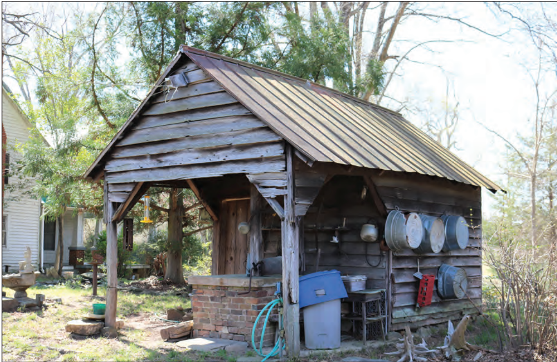
Figure 3.21. Wellhouse, Looking Southeast.
