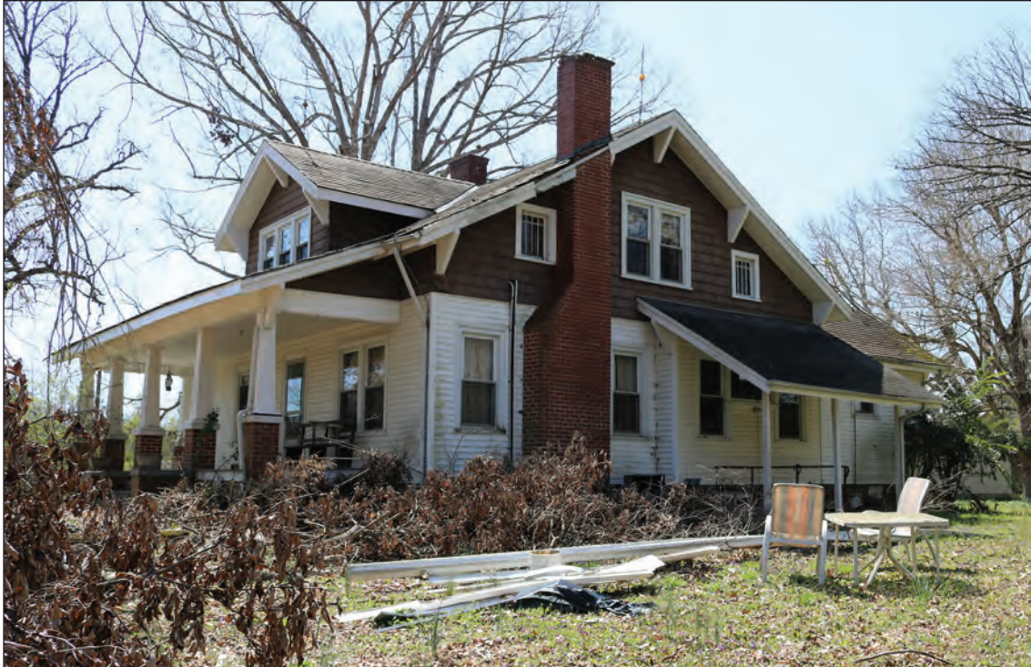
Figure 3.41. Shafter Coble Farm House, Façade and West Elevation, Looking Southeast.
