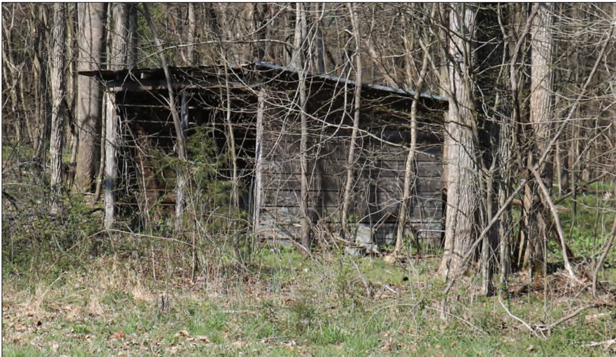
Figure 3.70. Shed, Looking Southwest.
