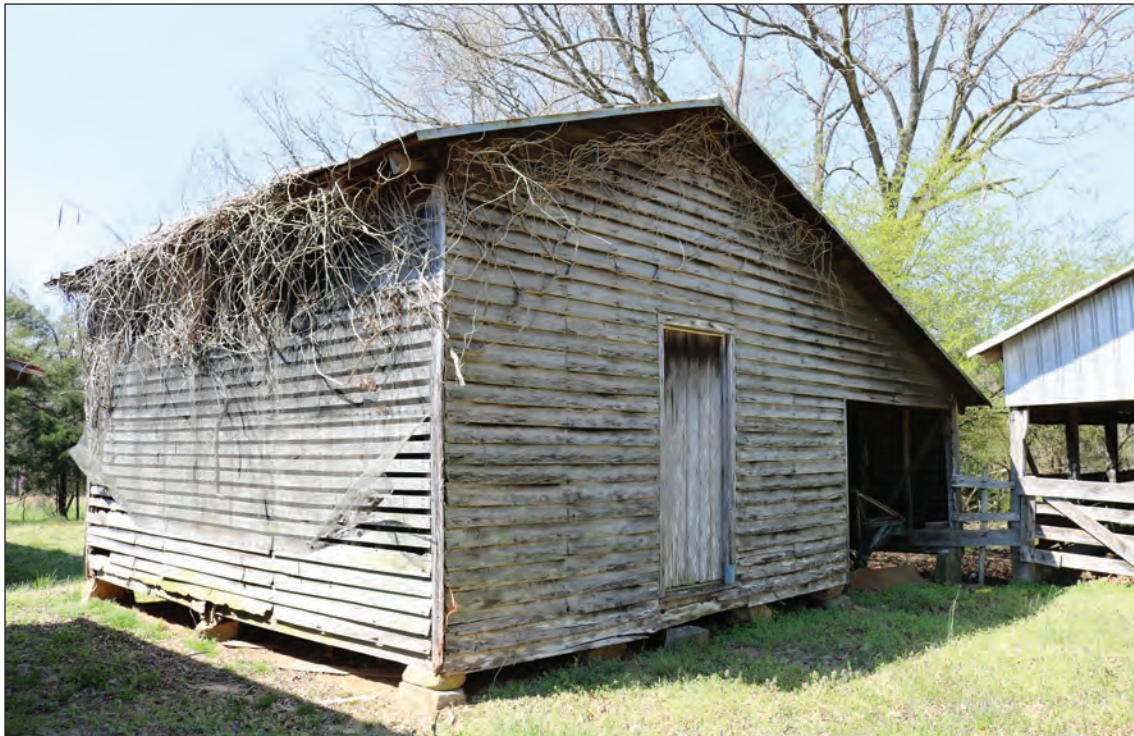
Figure 3.59. West Tobacco Packhouse, Façade and East Elevation, Looking Southwest.
