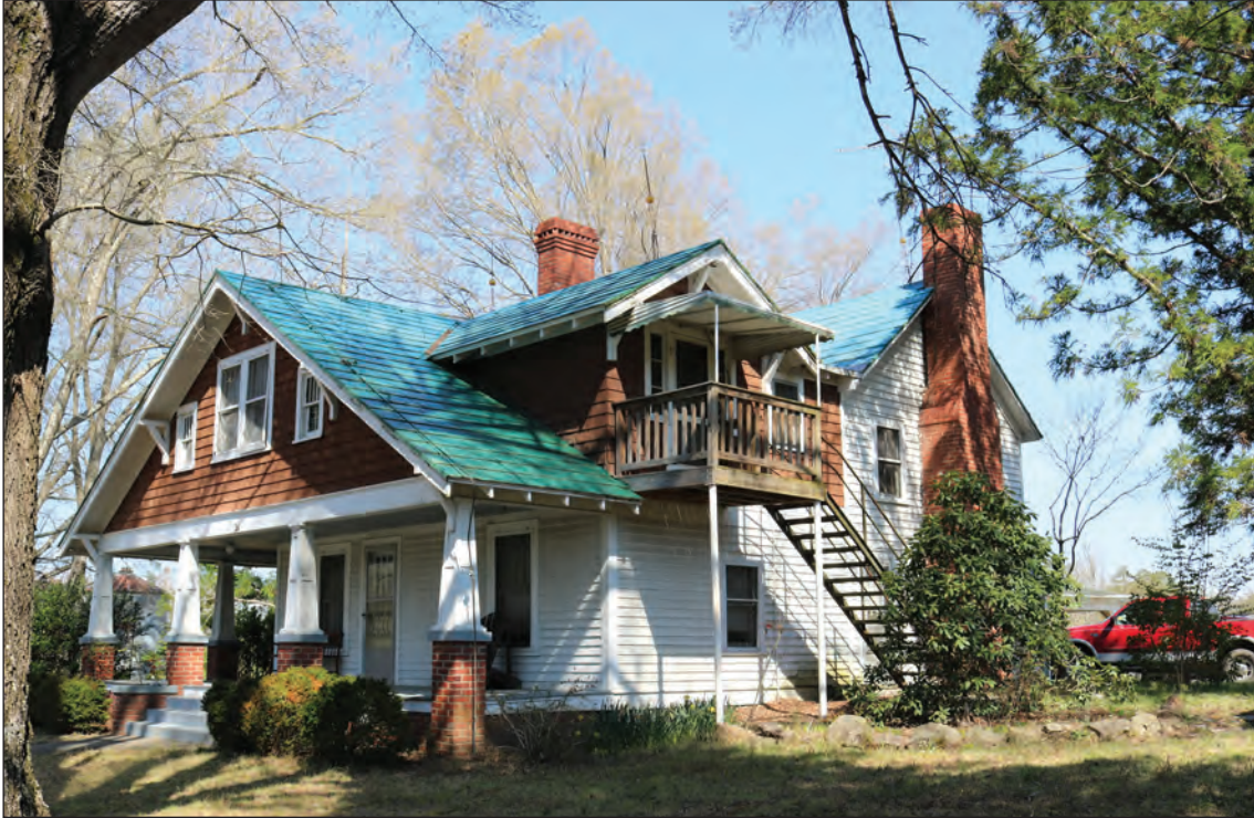
Figure 3.10. David Daniel Coble Farm House, Façade and East Elevation, Looking Northwest.
