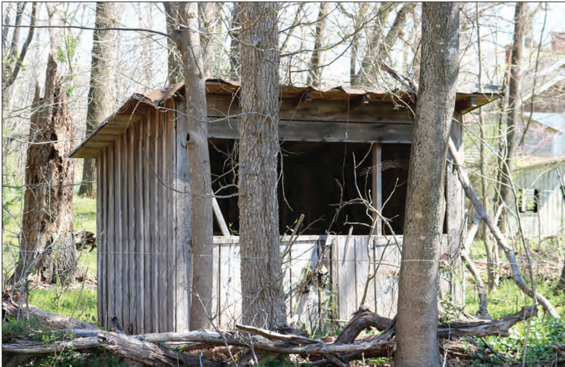
Figure 3.52. Circa 1940 Canted Roof Storage Coop, Looking North.
