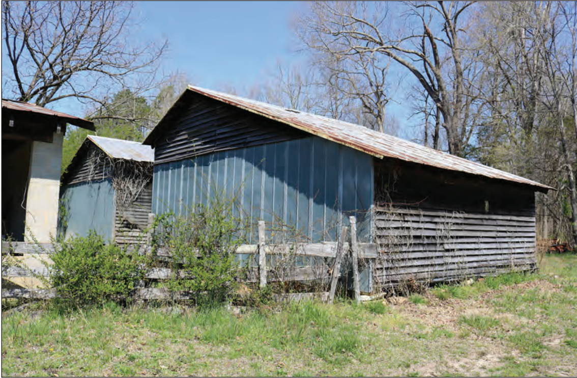
Figure 3.58. East Tobacco Packhouse, East and South Elevations, Looking Northwest.
