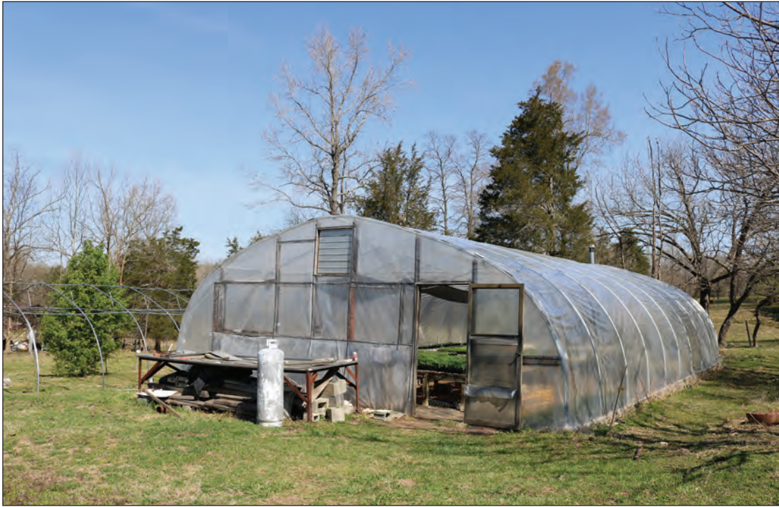
Figure 3.31. Greenhouse Complex, Looking North.
