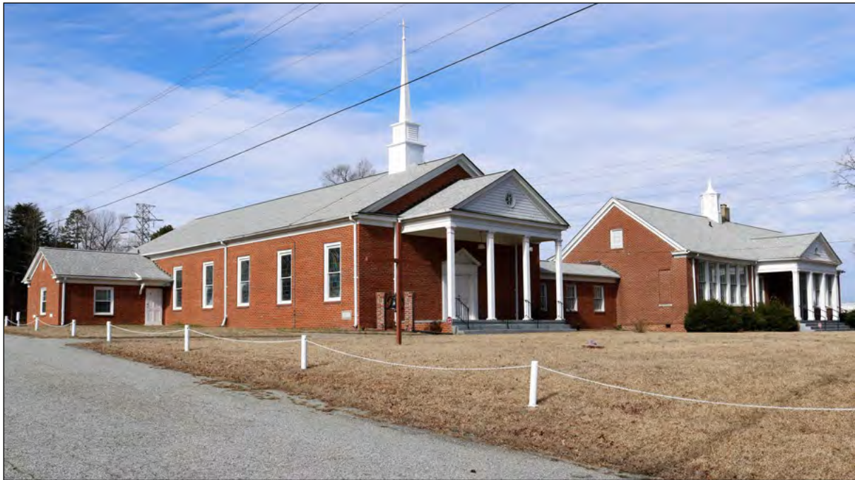
A. Looking Northwest
