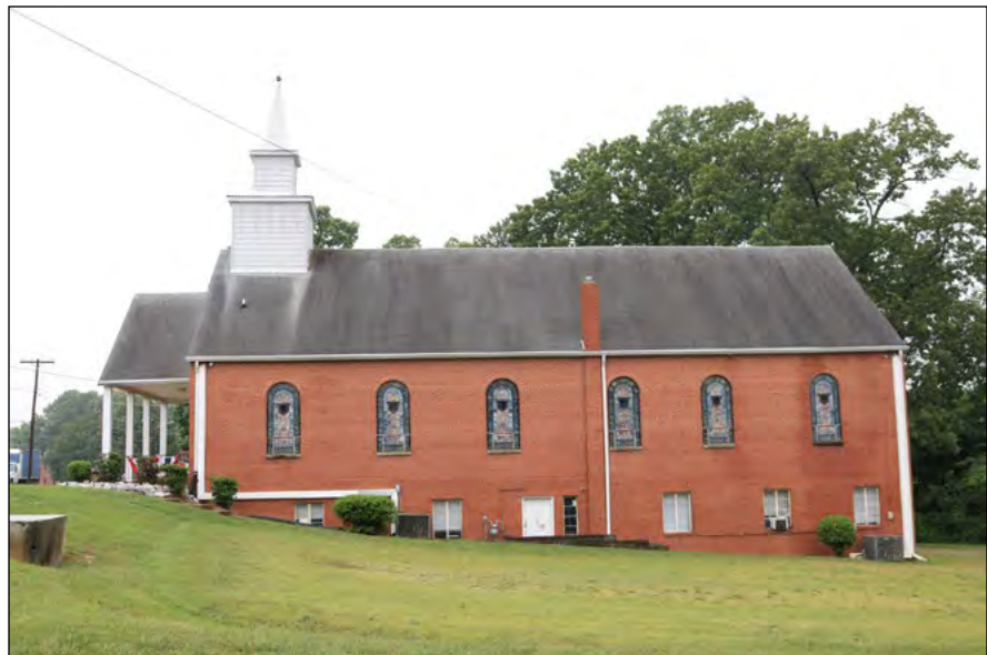
B. Church, Looking West
