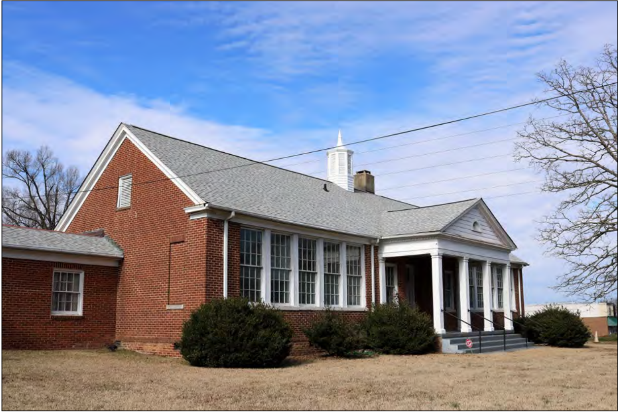
A. Looking Northwest
