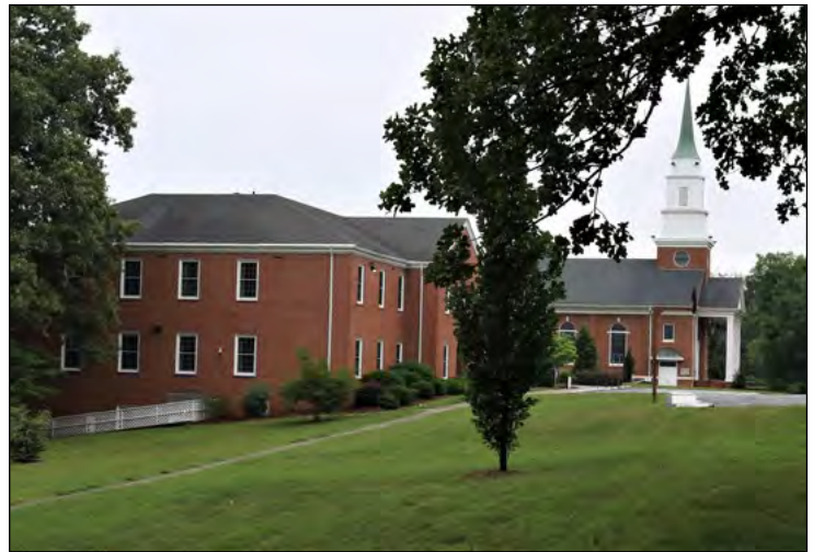
B. Sanctuary and Educational Wing, Looking North
