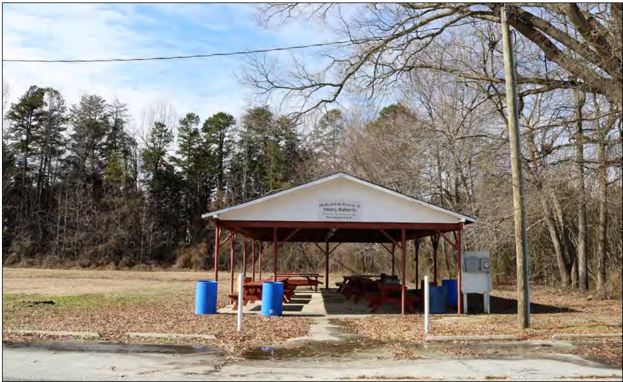
B. Looking West at Picnic Pavilion
