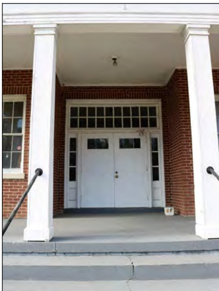
B. Looking Southwest
