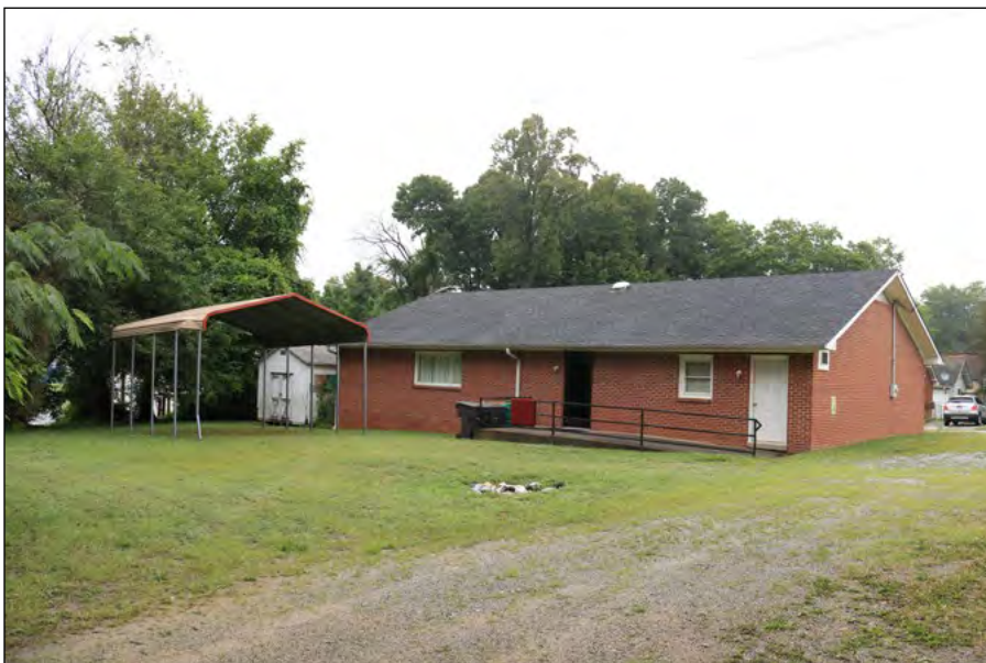
C. Support Building, Looking Northeast
