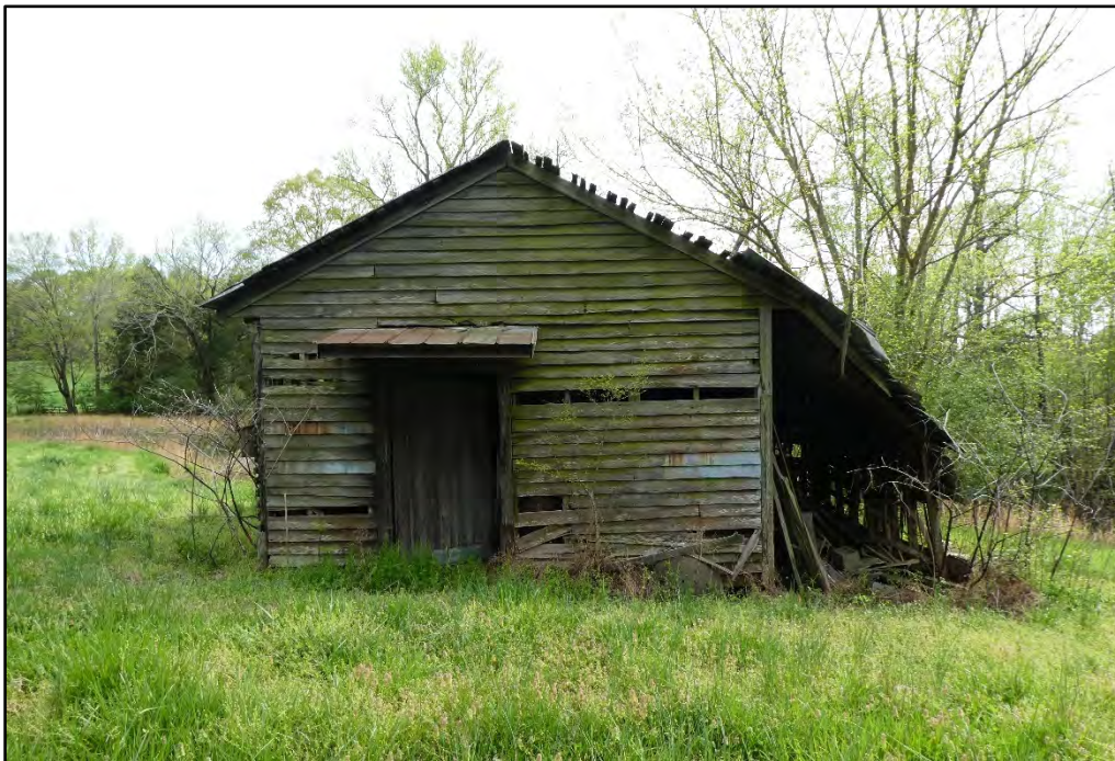
Figure 17. North elevation of Corn Crib A (Site Plan # 2), taken facing south.
