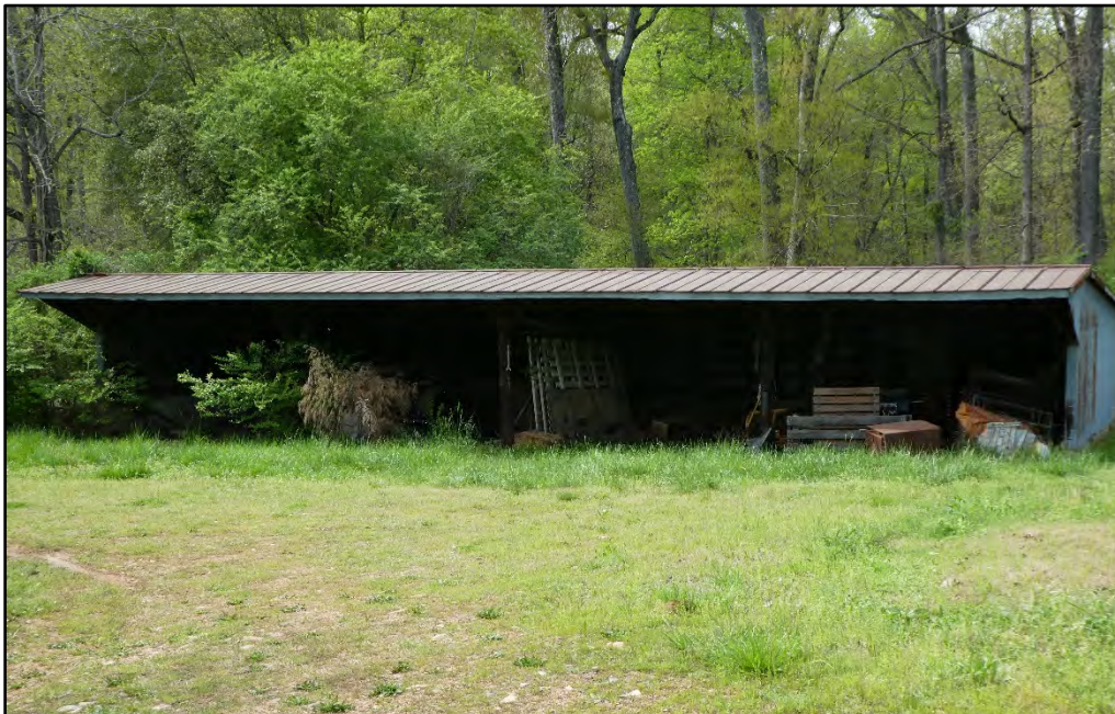
Figure 34. Machine Shed A (Site Plan # 10), southeast elevation, taken facing west-northwest.
