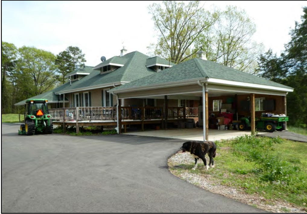
Figure 13. North and west elevations of the farmhouse today, showing new deck, carport, and hardscaping, taken facing southeast.
