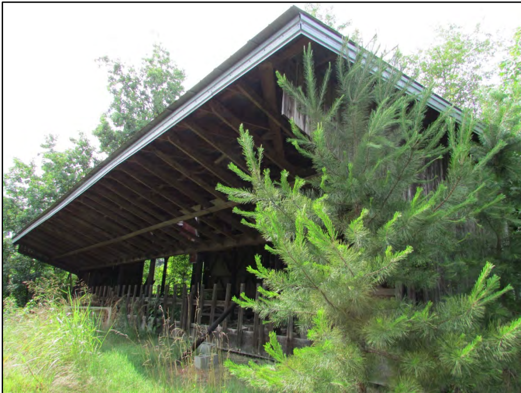
Figure 48. Livestock Shelter (Site Plan # 22), taken facing northwest.
