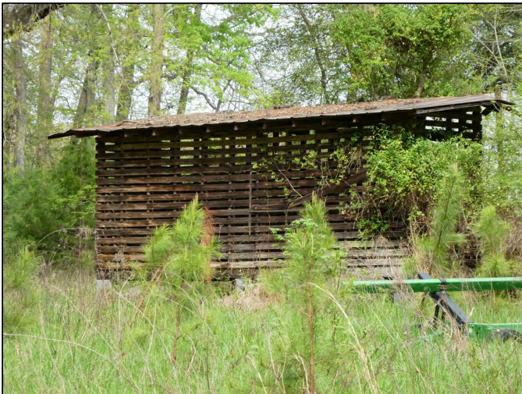
Figure 42. Corn Crib B (Site Plan # 20), west elevation, taken facing northeast.
