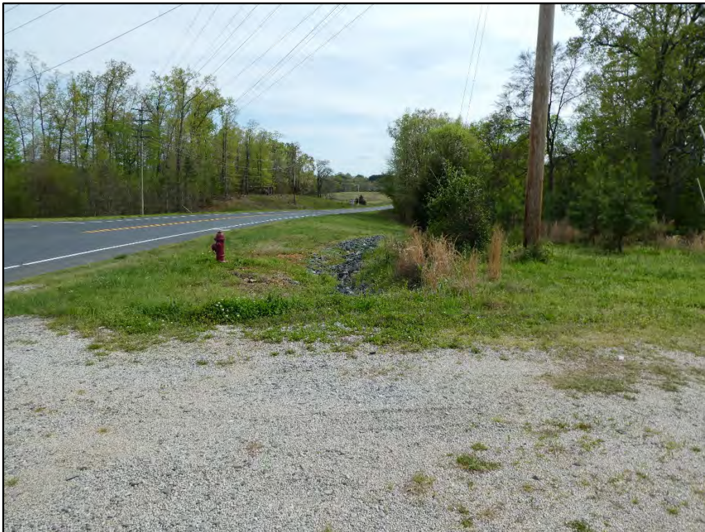
Figure 5. View of the Northeast Connector looking south from the back or secondary access road to the Moss-Coble farmstead. Shed (Site Plan #22) is hidden in the trees on the lefthand side of the photograph.
