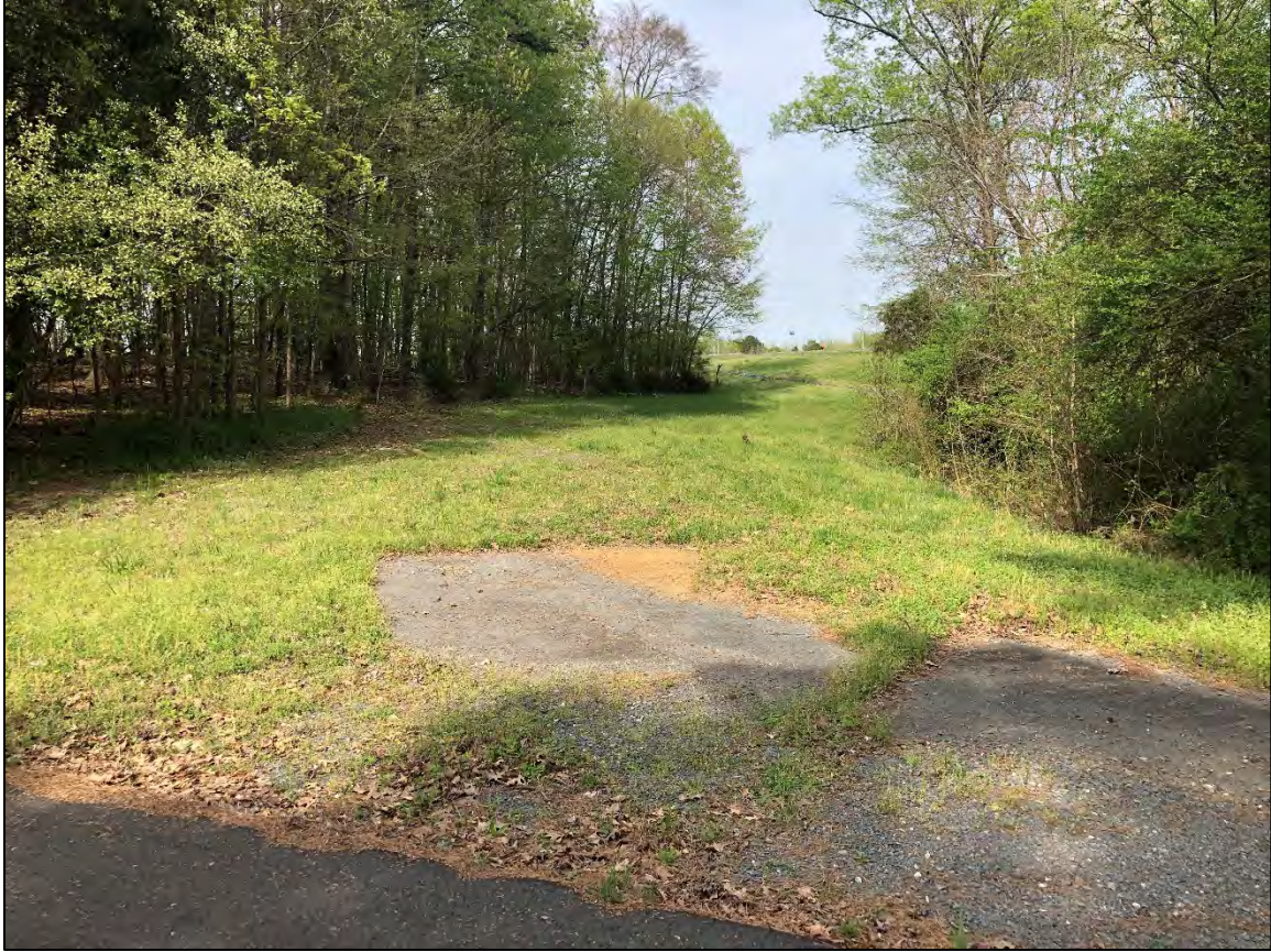
Figure 10. Former route of Moss Spring Road, taken facing northeast toward Northeast Connector from the paved driveway.
