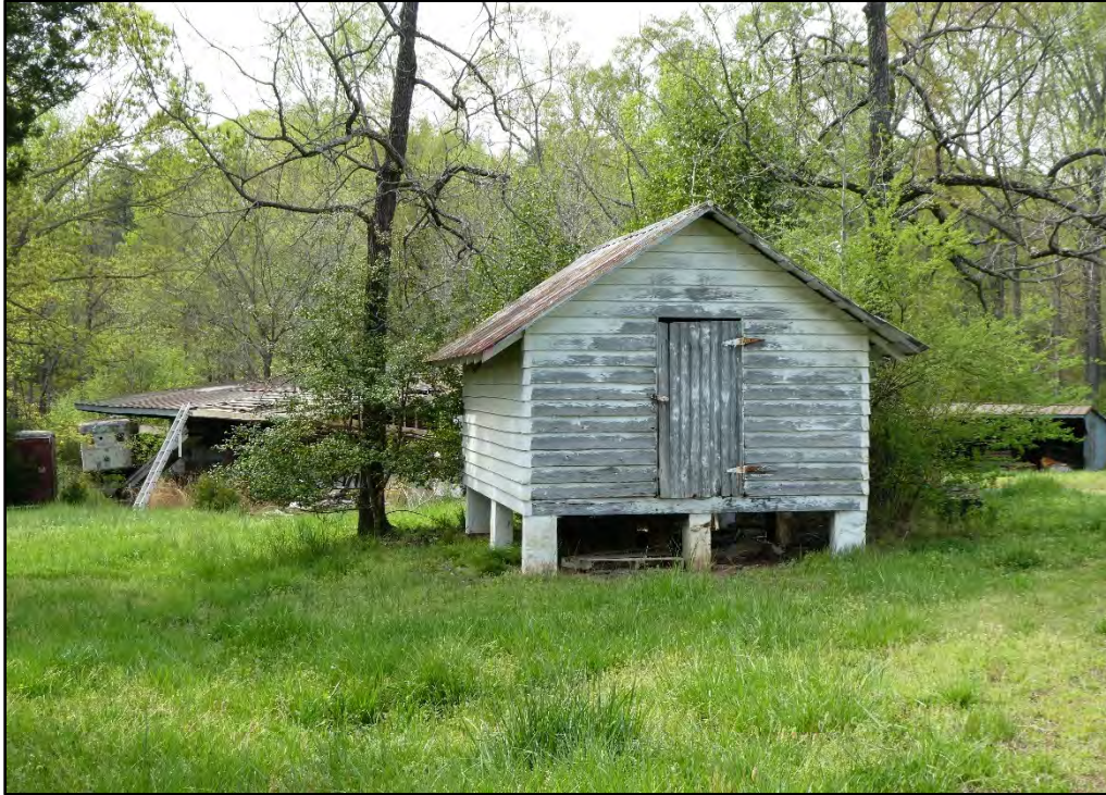
Figure 29. Granary A (Site Plan # 9), east elevation, taken facing west-northwest.
