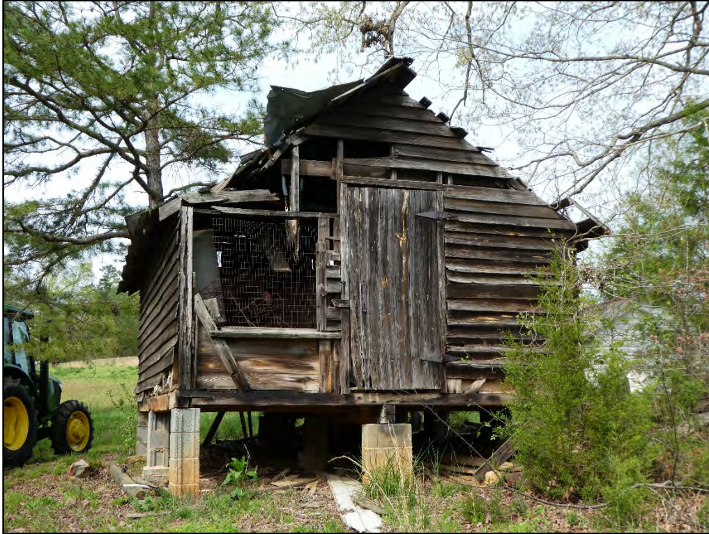
Figure 23. South elevation of Coop A (Site Plan #5), taken facing north.
