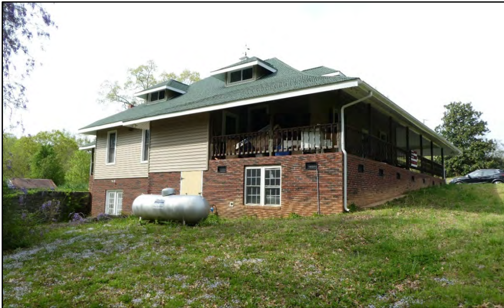
Figure 14. Current view of south elevation of the dwelling, taken facing north.
