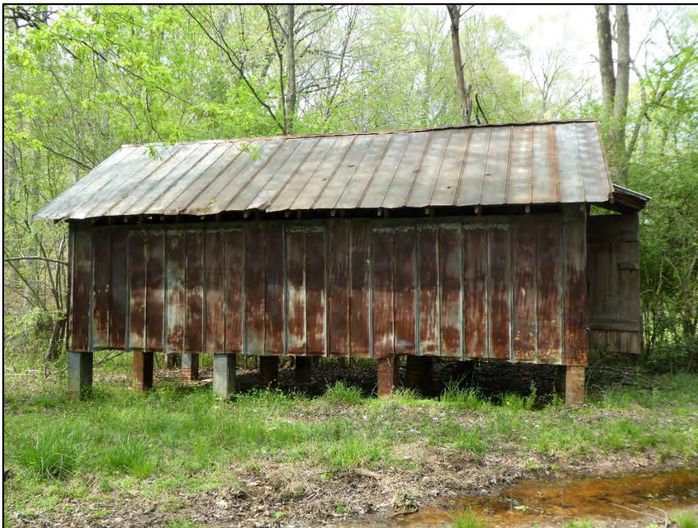
Figure 38. Granary B (Site Plan # 17), south elevation, taken facing north.
