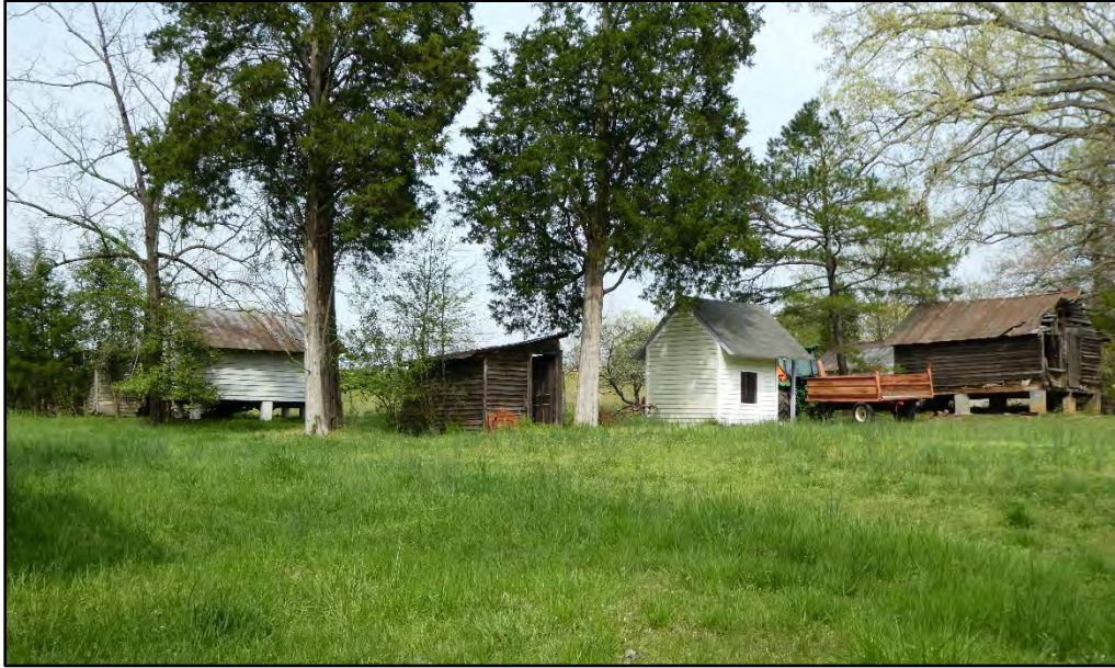
Figure 27. From left to right, Granary A, Coop B, Playhouse, and Coop A (Site Plan # 9, 11, 12, and 5), taken facing northeast.
