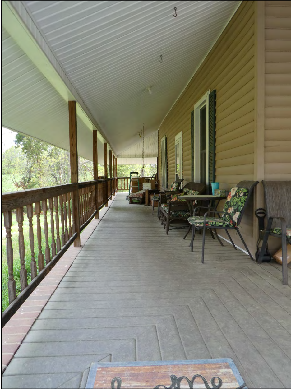
Figure 15. Detail of wraparound porch as seen in 2019, illustrating new framing, ballusters, composite decking, vinyl siding, vinyl windows, and applied vinyl shutters, taken facing west.
