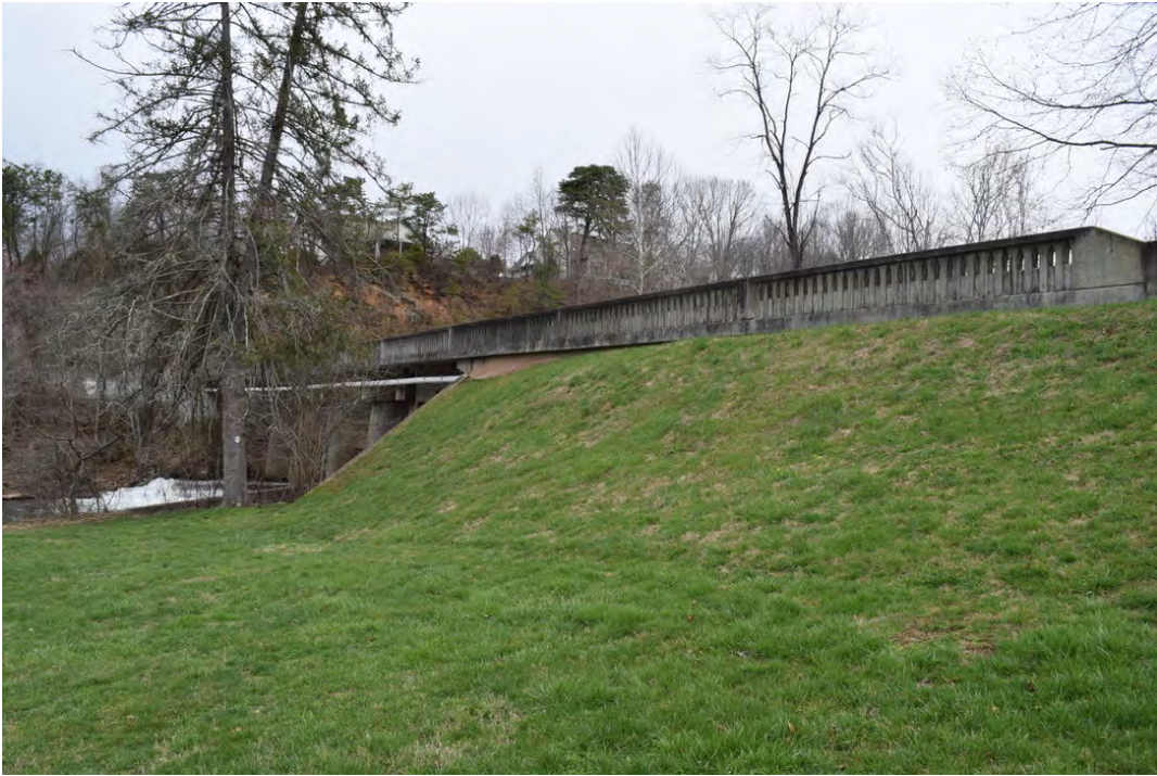
Hill below bridge approach on south end, view to the northeast
