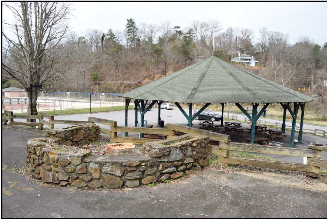
Merry-Go-Round shelter, view to the northwest
