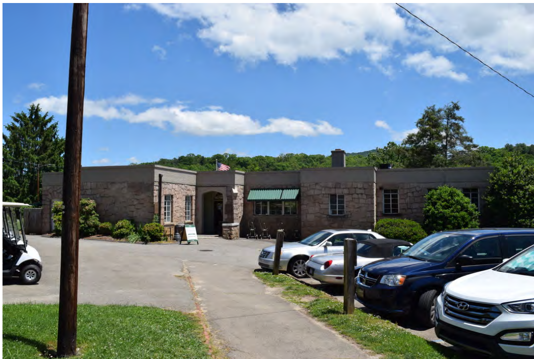
1927/1956 Clubhouse, view to the southeast
