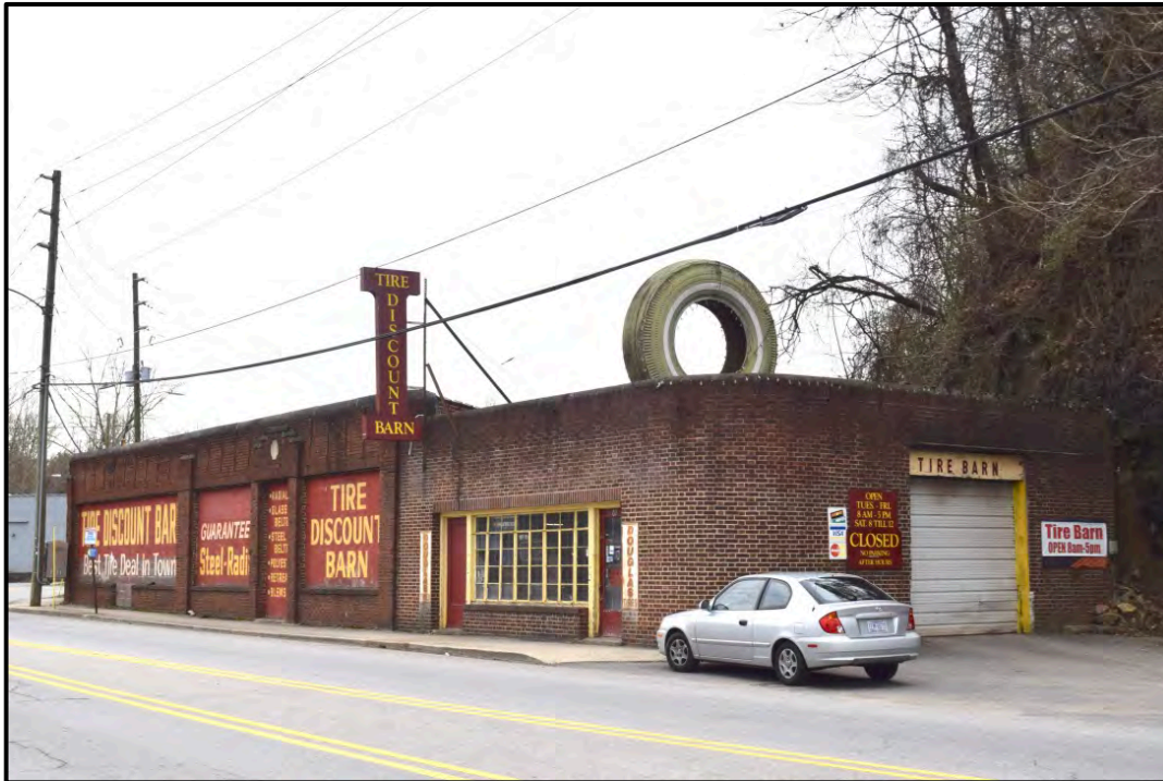
Discount Tire Barn on London Road, view to the south
