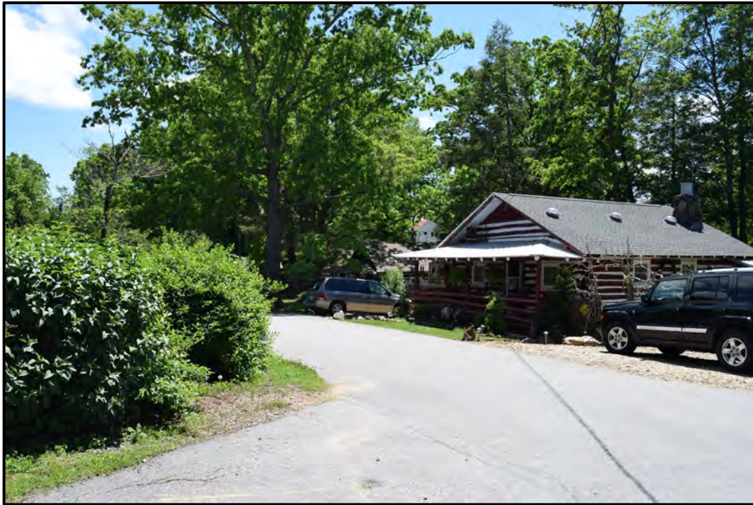
32 Spruce Drive, view to the southwest
