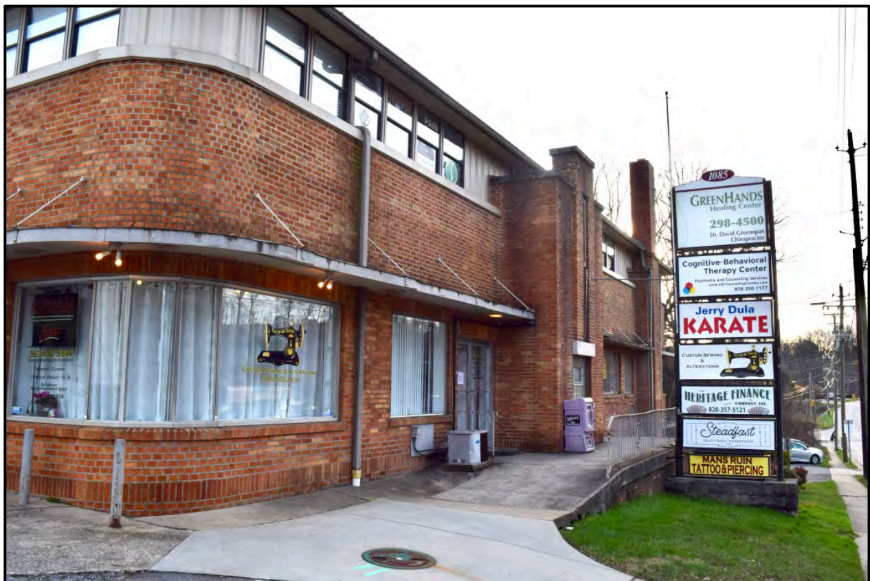
Northeast (front) corner, view to the southwest
