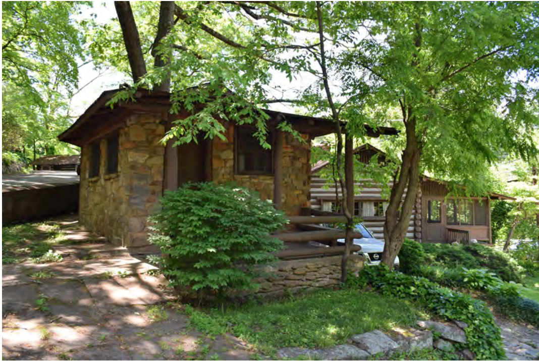
Stone building at the northwest corner of Rhododendron Drive and Cottage Drive, view to the west
