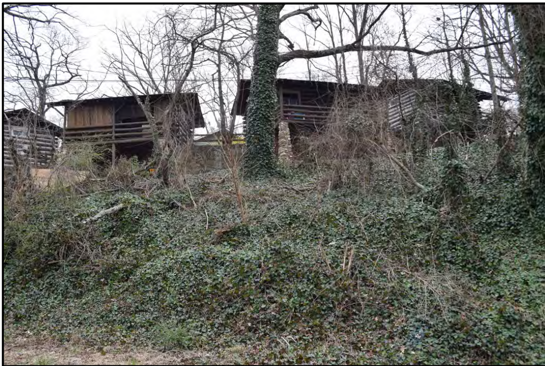
Rear (north) elevations of cabins on Cottage Drive seen from Swannanoa River Road, view to the south
