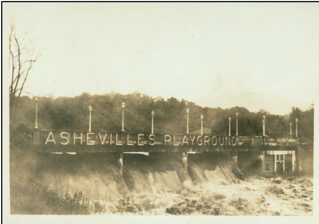
Flood waters under the dam in 1940. Photo courtesy North Carolina Collection, Pack Memorial Public Library, Asheville, North Carolina
