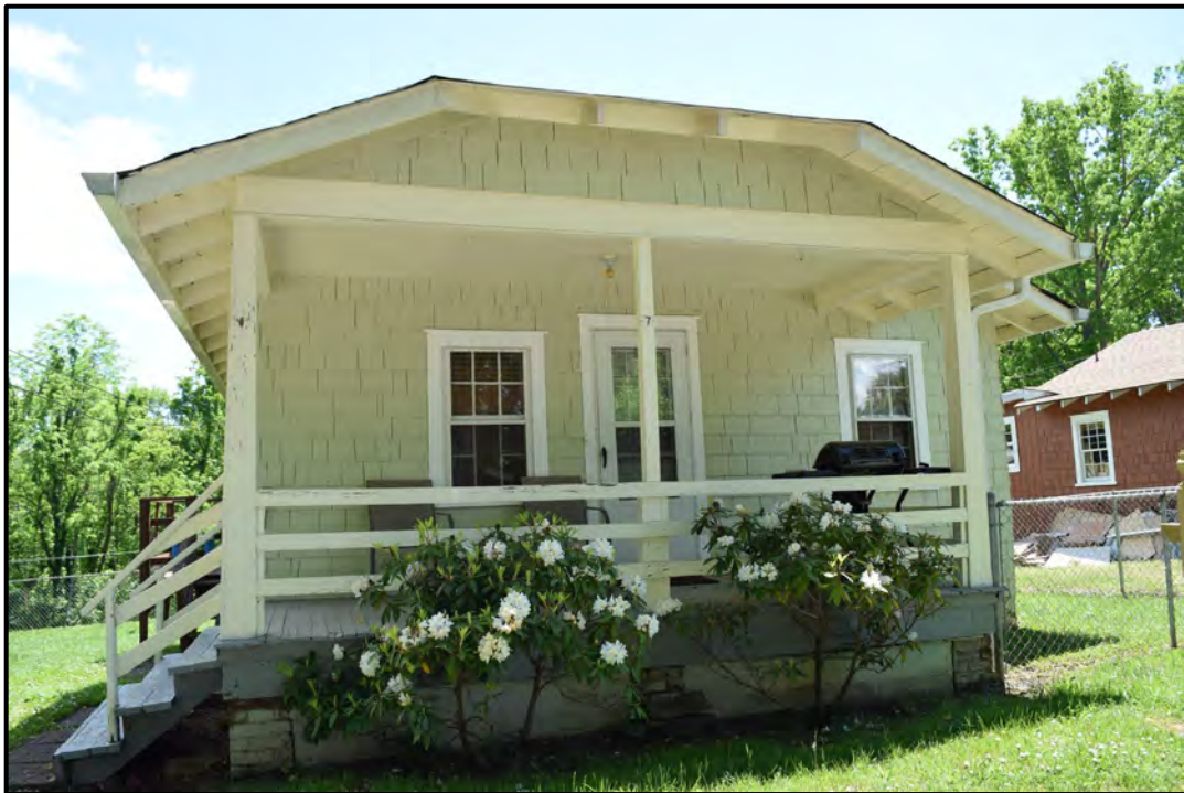
Circa 1932 bungalow at 32 Spruce Drive, view to the south
