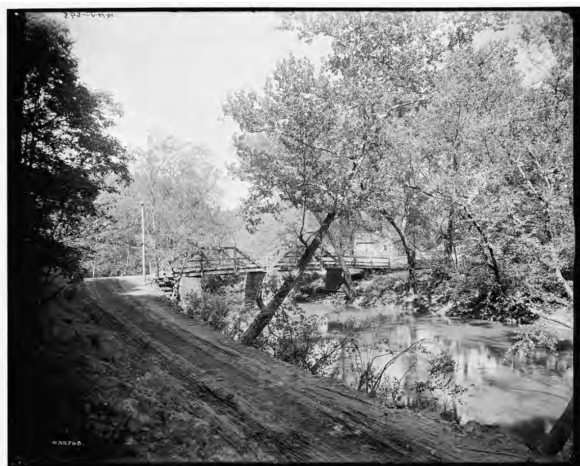
Image of the 1887 Asheville city waterworks and wooden bridge replaced in 1924 by the current concrete bridge, dam, and power house. The waterworks closed around 1915 and the equipment was abandoned. Photo from the Library of Congress. Detroit Publishing Co., William Henry Jackson, Photographer. Waterworks on the Swannanoa, Asheville, N.C. [Between 1895 and 1910].
