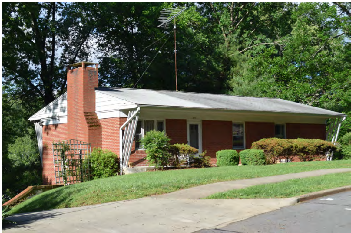
Ranch house with modernist elements at 79 Arthur Street, 1952, view to the southwest
