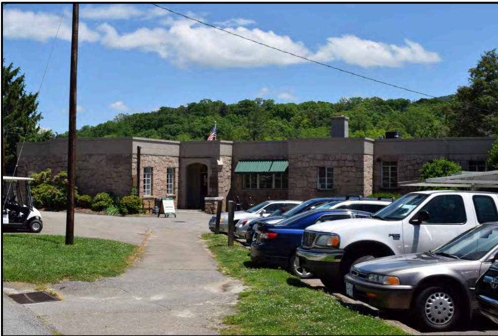
1927/1956 Clubhouse, view to the southeast
