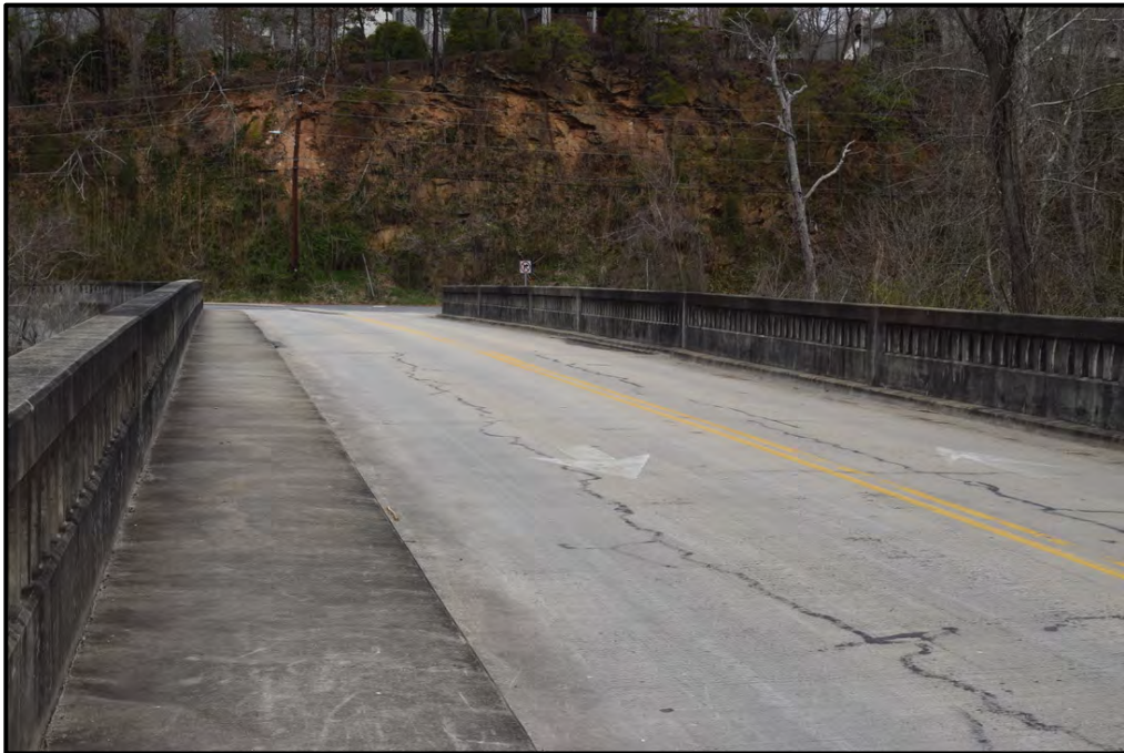
Bridge deck, view to the north
