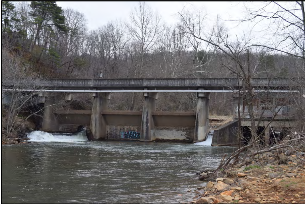
Swannanoa River Bridge, Dam, and Power House, view to the east-northeast
