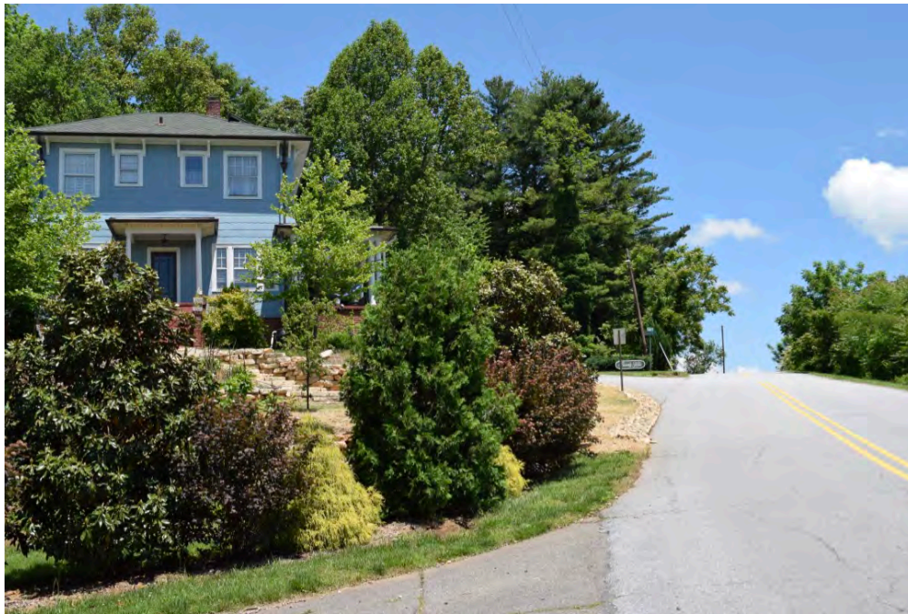
Ada N. and Dr. LaBruce Ward House, built at 271 Fairway Drive in 1936
