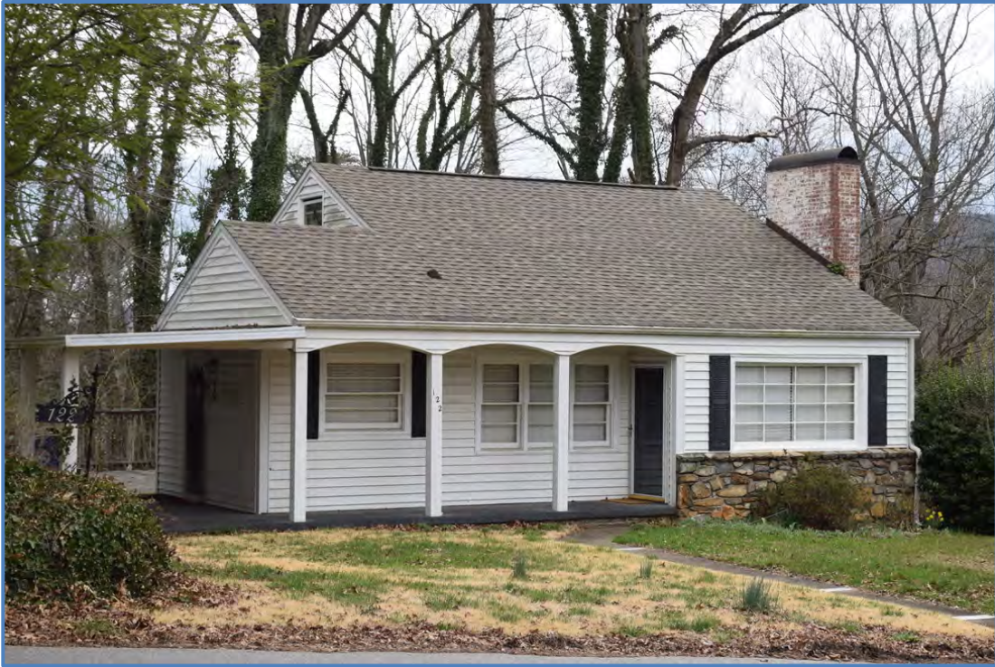
The 1953 Monimia MacRae House at 122 Beverly Road, view to the east-northeast
