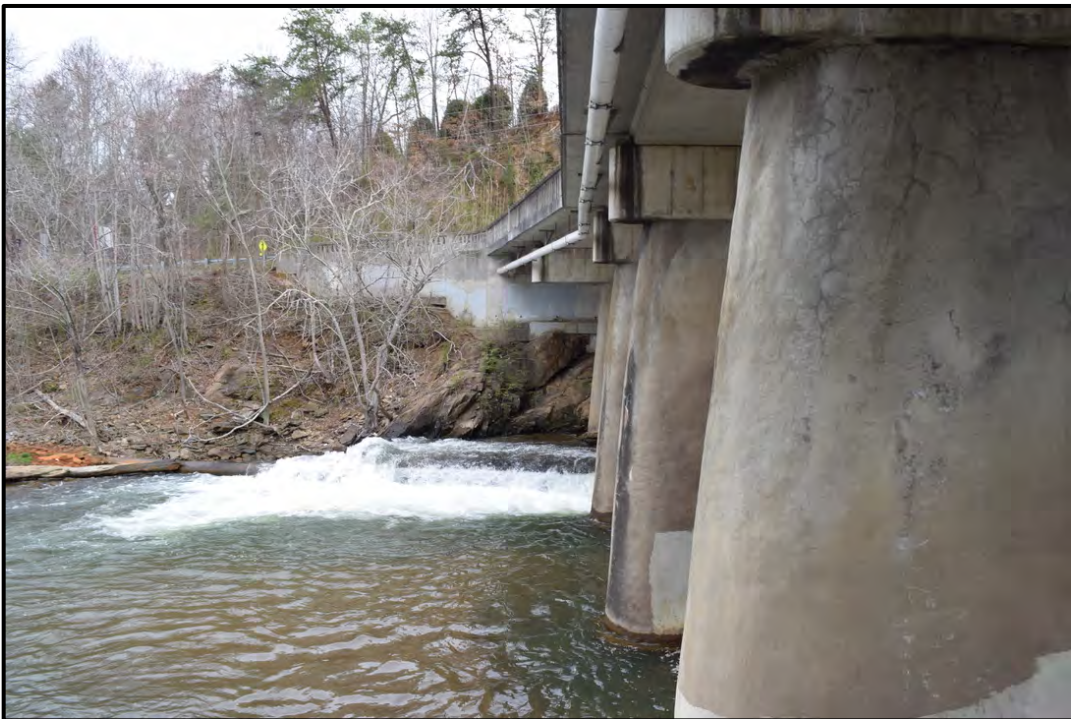
West side of bridge and Swannanoa River, view to the north
