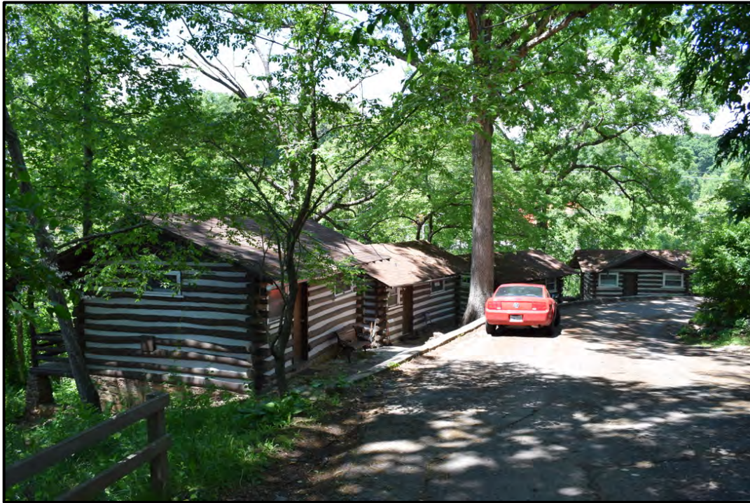
Cabins at 16, 17, 18, and 19 Cottage Drive, view to the east-northeast
