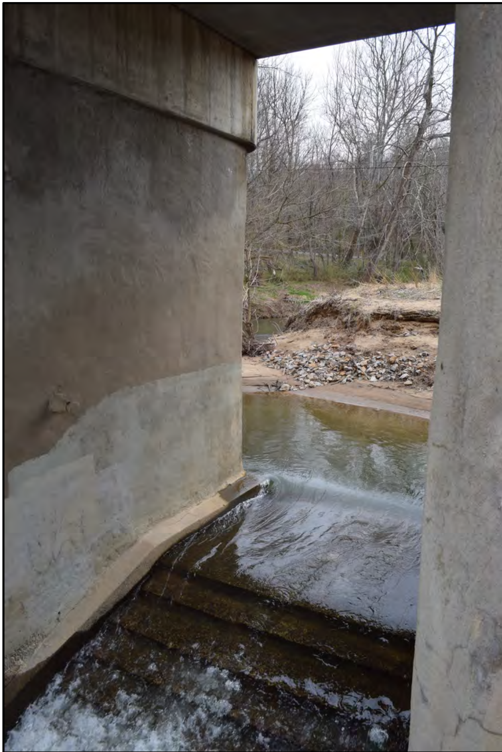
Spillway on south end of bridge, view to the east-northeast
