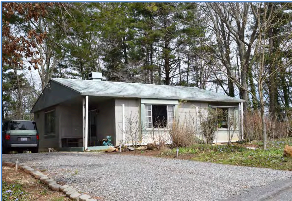
Bruce A. and June L. Elmore Lustron House at 70 Hampden Road, 1949, view to the northeast
