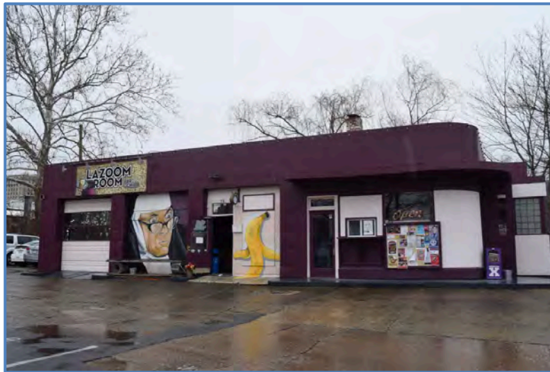
Former Esso Station on Biltmore Avenue, view to the east
