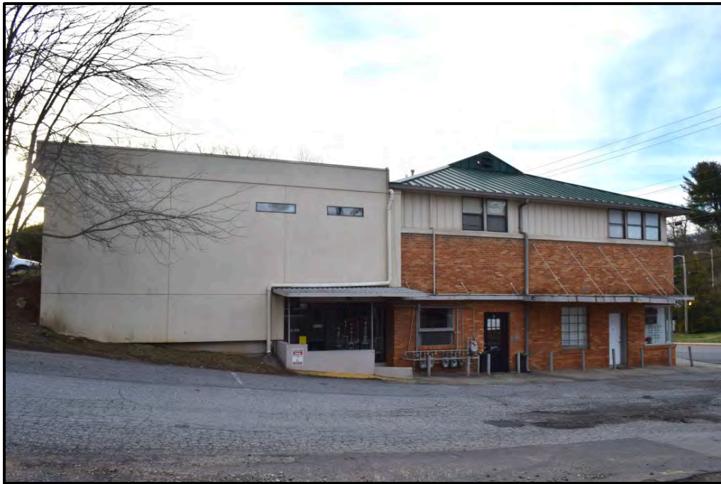
East elevation, view to the west
