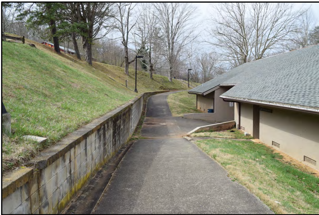
Walkway along south side of bathhouse, view to the west
