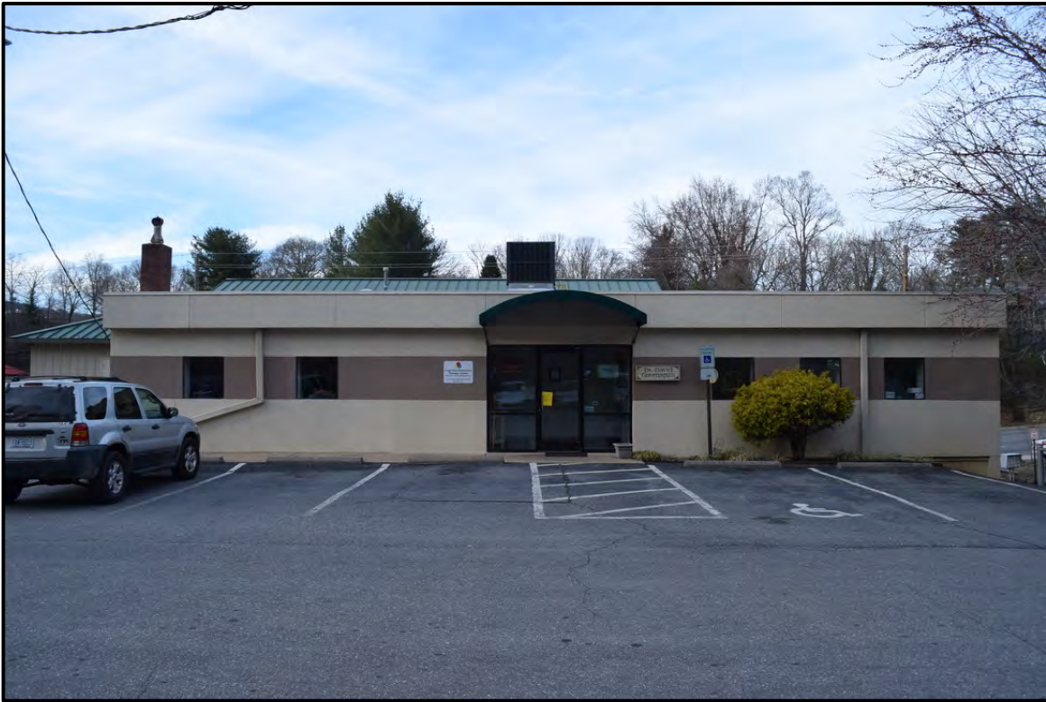
Modern rear addition, view to the north
