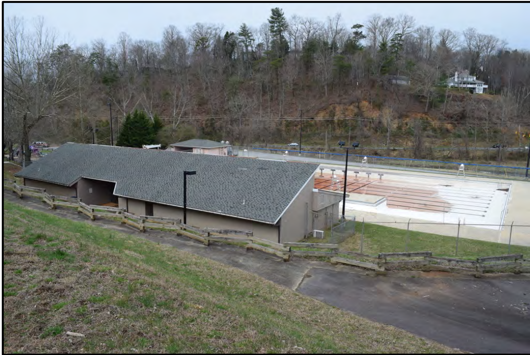
Bathhouse and pool view to the north
