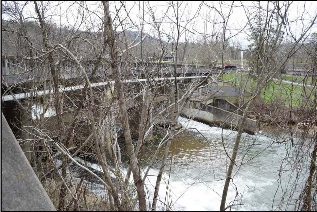
Northwest corner of bridge from Azalea Road, view to the southeast
