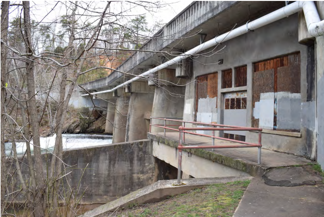
Power house under south end of bridge, view to the north
